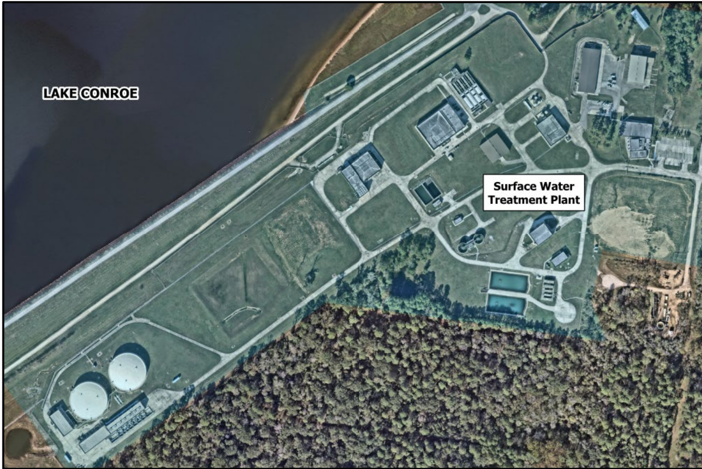
Surface Water Treatment Plant (Constructed in 2015)
