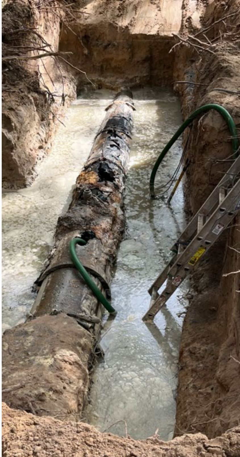
Pictures of 2023 Repair to Lift Station No. 5 Force Main
