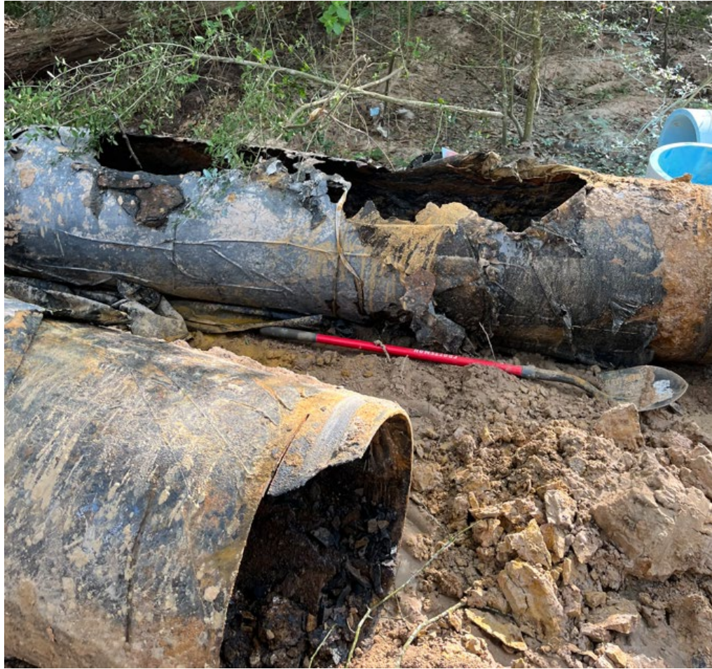
Pictures of 2023 Repair to Lift Station No. 5 Force Main
