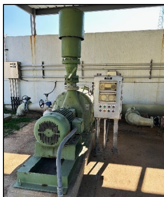
Digester Blower - In for maintenance.
