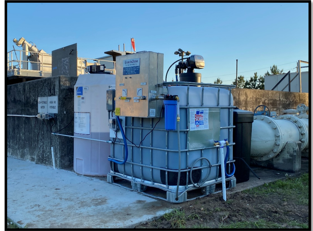
Chemical Feed System
