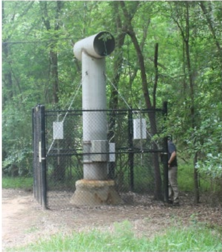
Figure 1: Tin Man Collection System Exhaust Structure (prior to removal)
