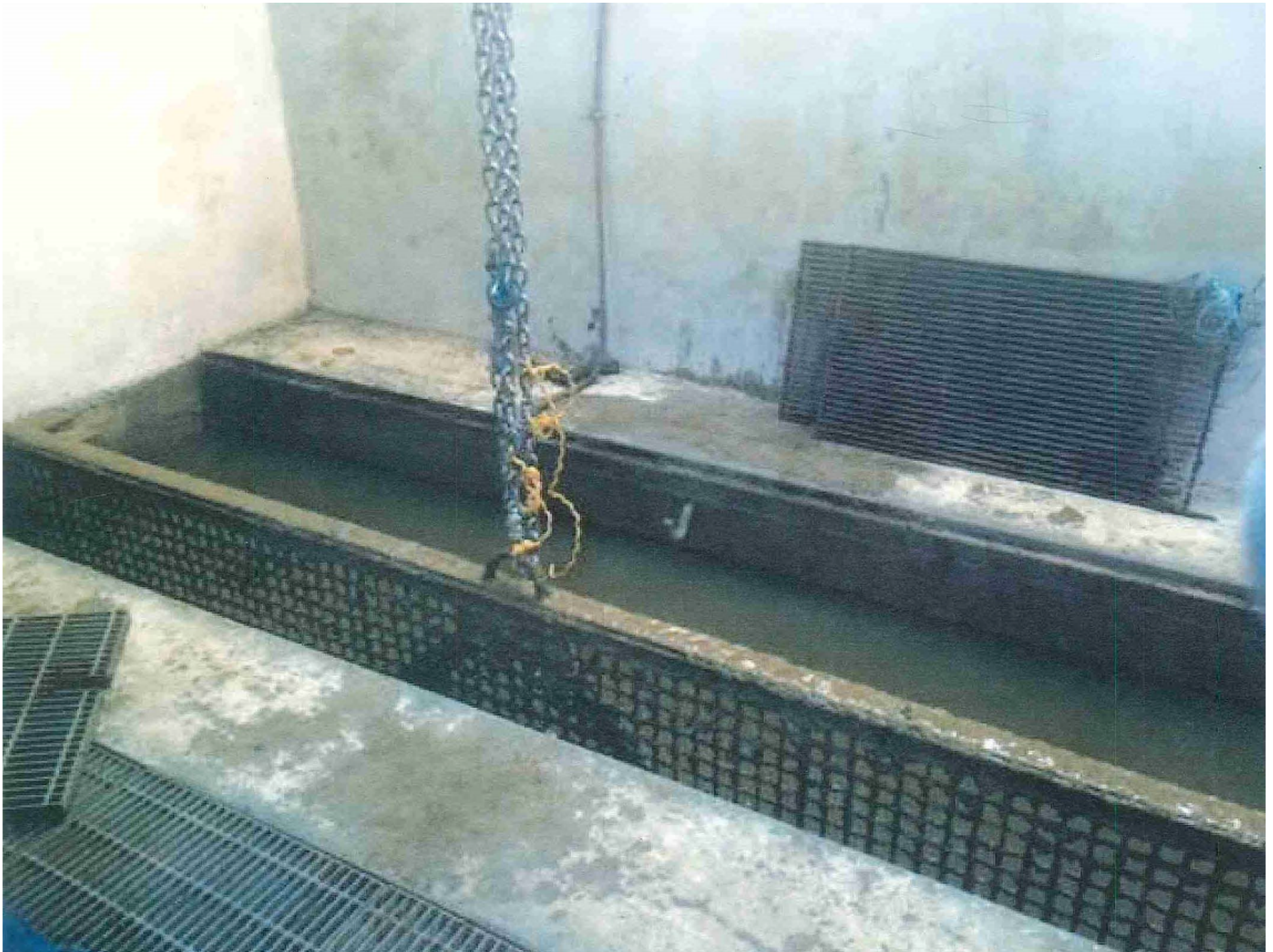
Screen at Lake Houston Pump Station
