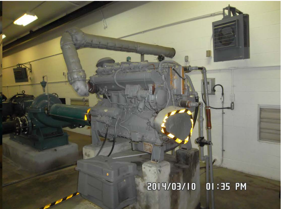
Water Booster Pump Auxiliary Engine
