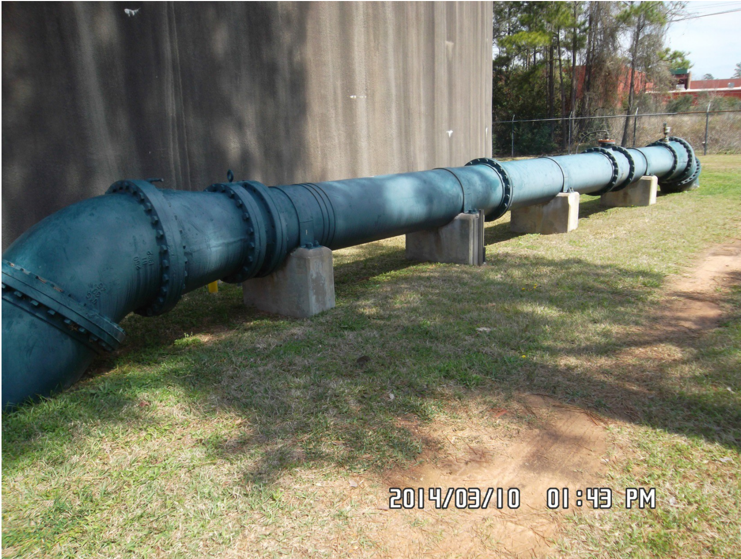
Water Plant above-ground Piping, Valves and Appurtenance
