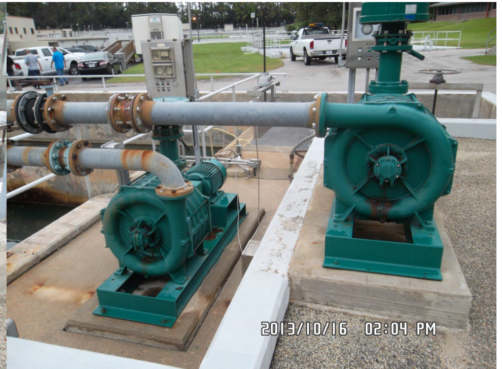
Post Aeration Blowers and Piping – Front View
