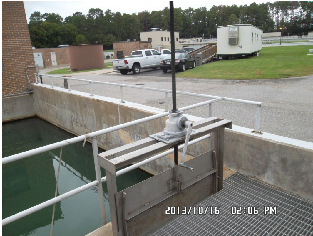
Sluice Gate Crank Valve – Post Chlorine Contact Basin
