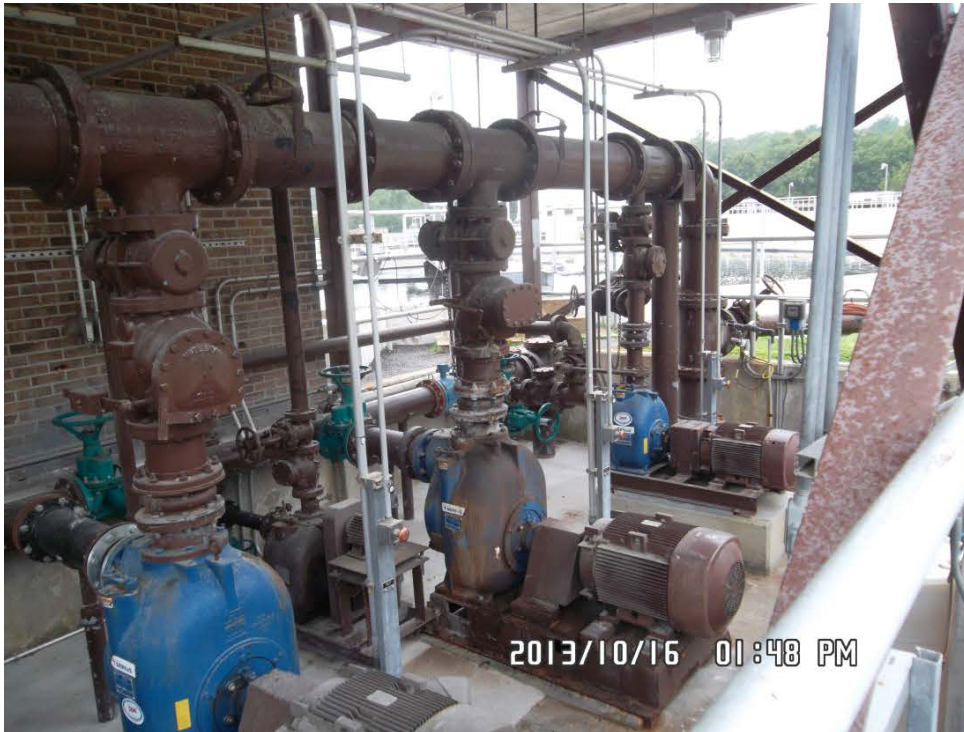
Return Pumps, Scum Pumps and Piping Front View
