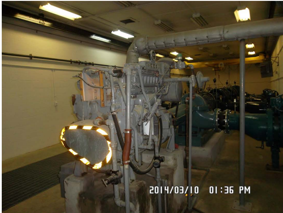
Water Booster Pump Auxiliary Engine
