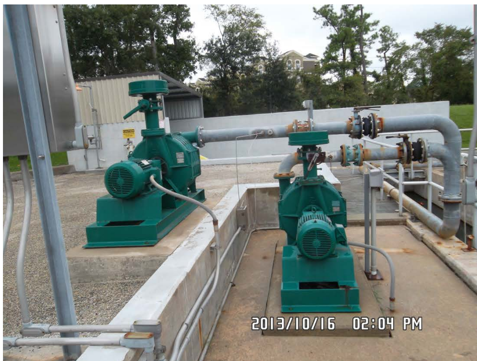
Post Aeration Blowers and Piping Front View
