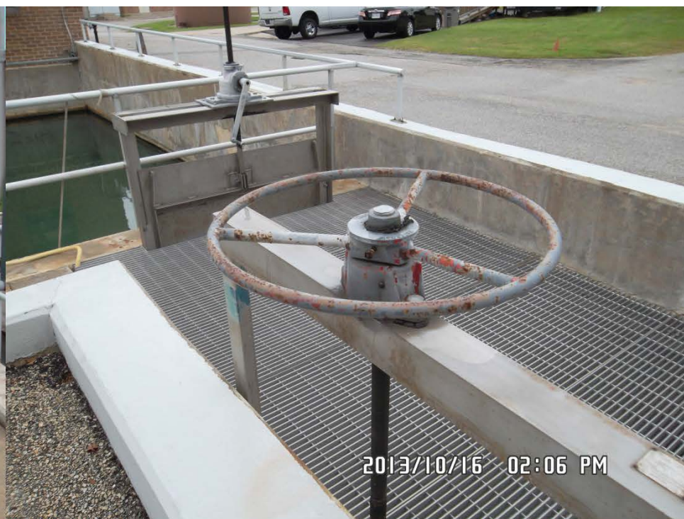
Sluice Gate Wheel – Post Chlorine Contact Basin
