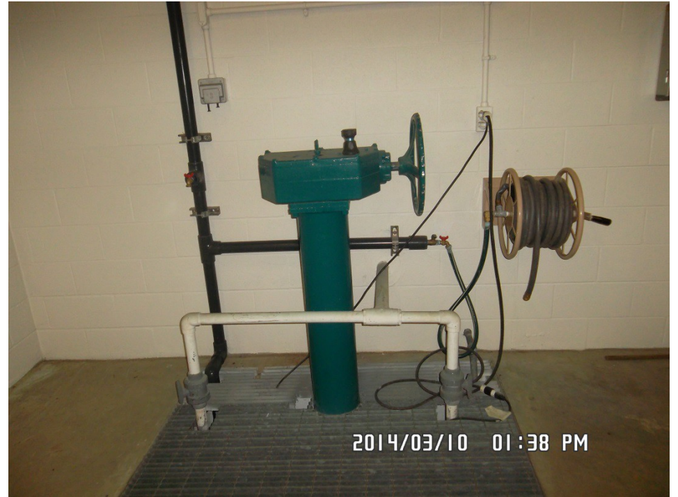
Valve Risers with Handwheels
