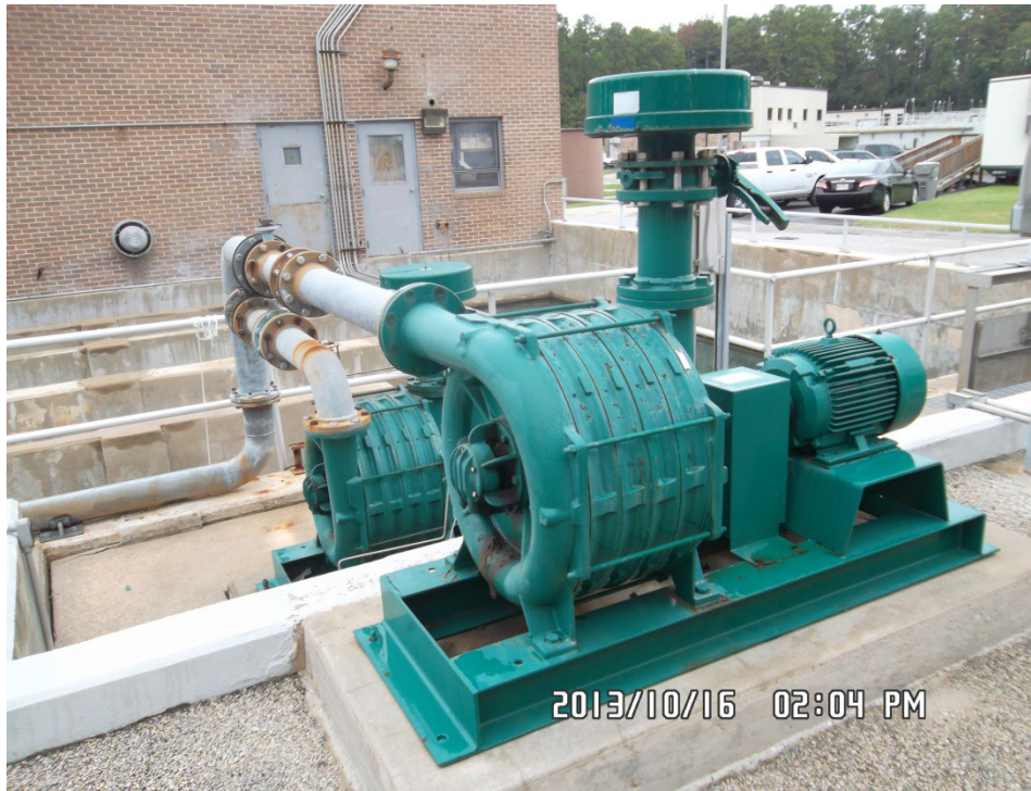
Post Aeration Blowers and Piping – Side View
