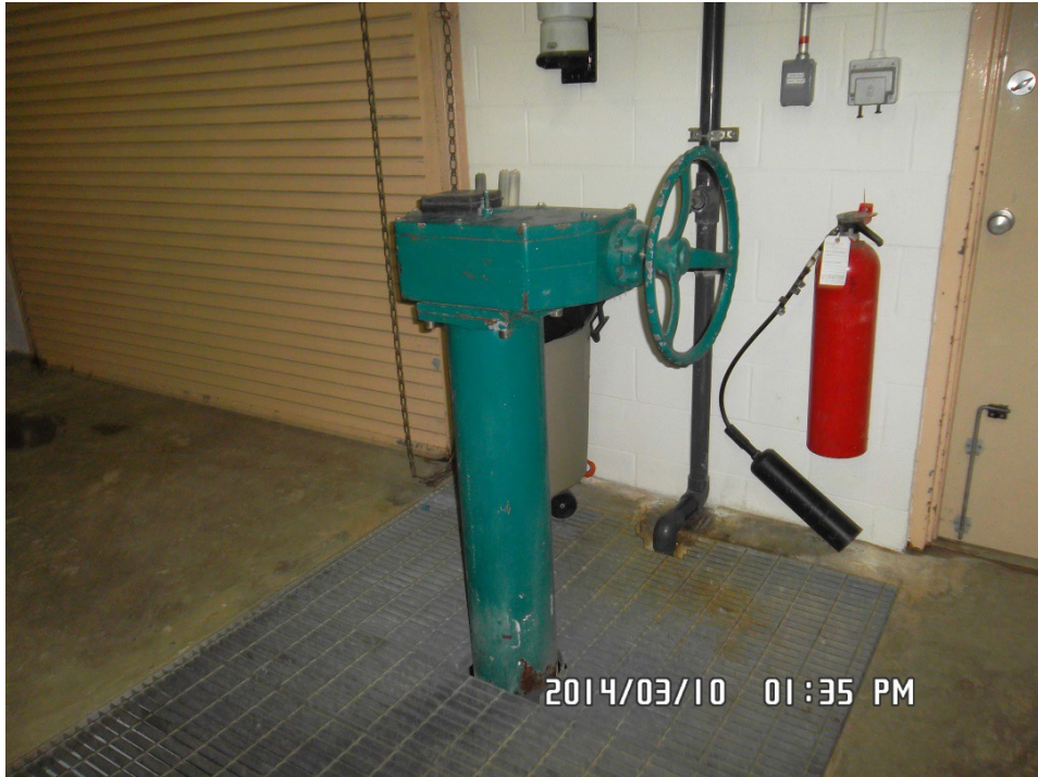
Valve Risers with Handwheels
