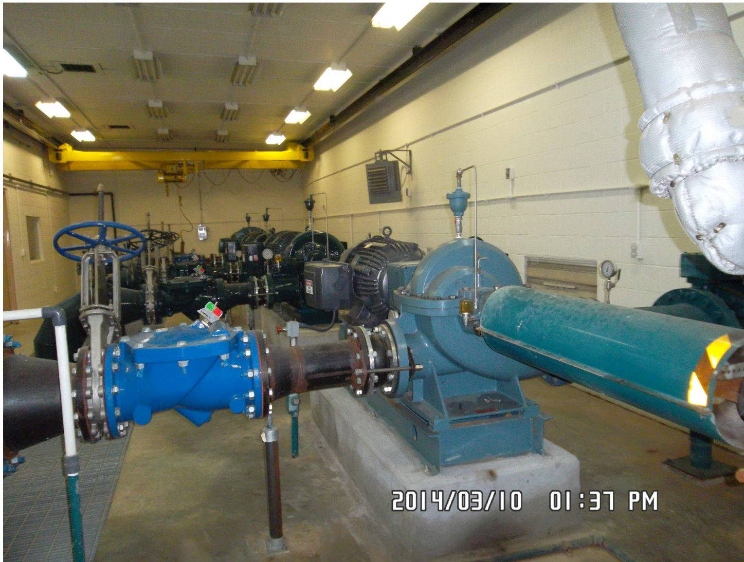
Water Booster Pumps and Piping
