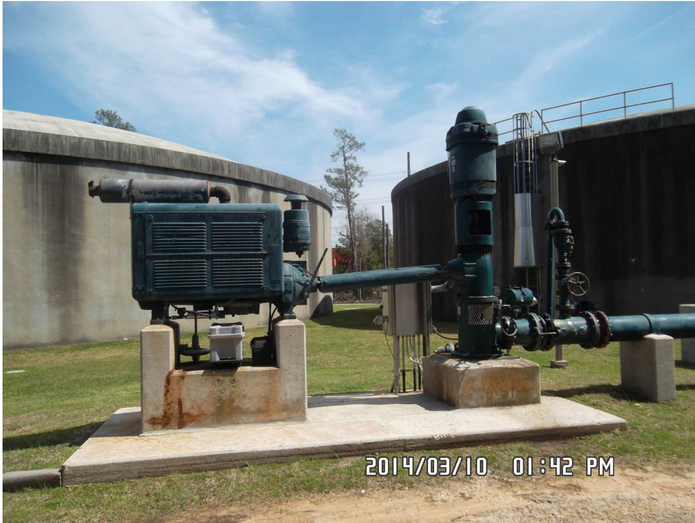
Water Well Pump, Motor and Auxiliary Engine
