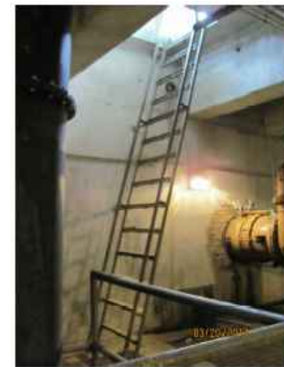
PHOTOGRAPH 1- SHIPS LADDER ACCESS
