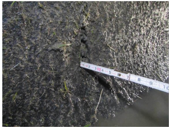
IMG_4028. Surface Spalling @ 100 ft (A)
