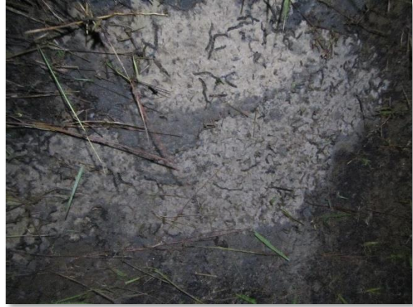
Photo 3-6. Surface Delamination (Typ.)
