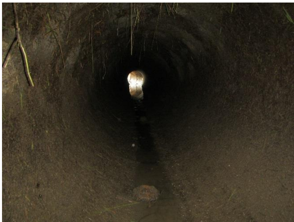
IMG_3970. 60-inch Pipe (B)
