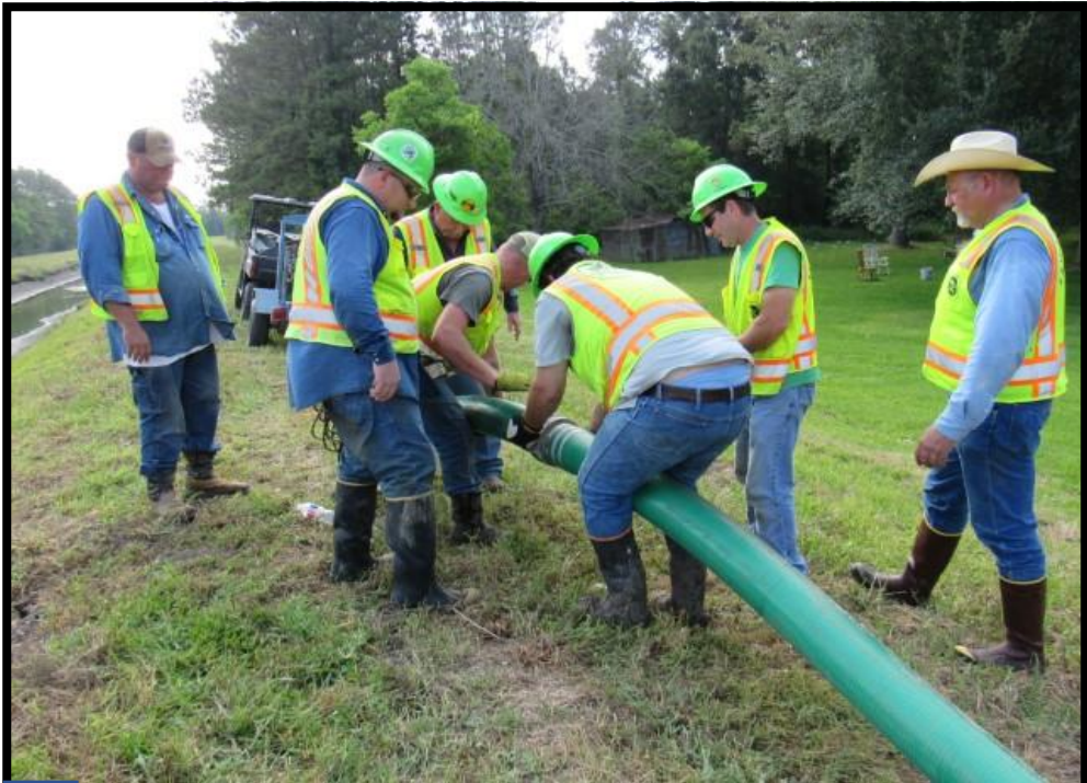
Dewatering pump suction line installation.
