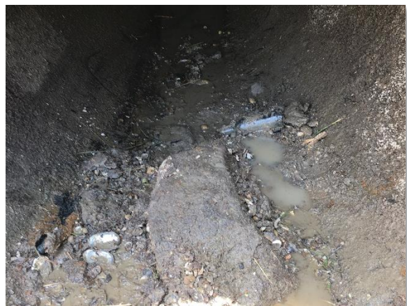
Photo 3-19. Debris Cast in Pipe Invert
