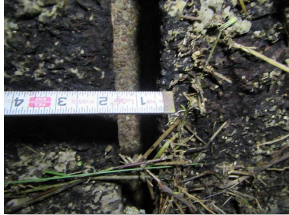
Photo 3-11. 1.5-inch Joint Gap at 10 ft
