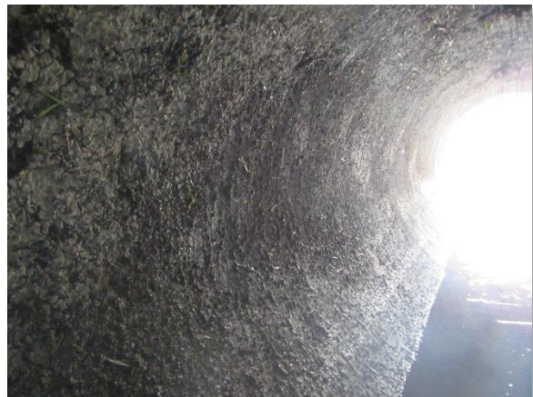
IMG_4030. 48-Inch South Pipe Wall (B)
