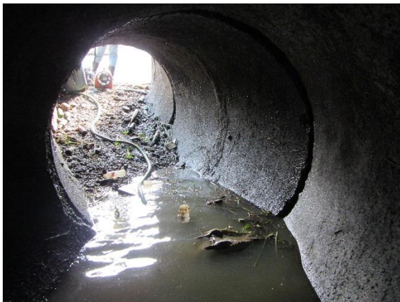
IMG_3979. 60-inch Pipe Outlet and 3.5-inch Joint Gap at Change in Direction
