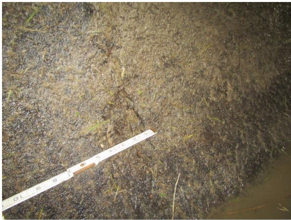
IMG_4027. Surface Spalling @ 100 ft (A)
