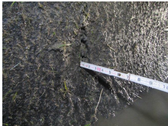
Photo 3-15. Surface Spalling at 100 ft (B)
