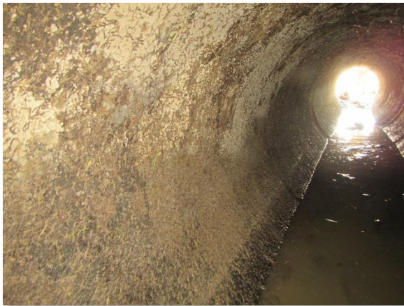
IMG_4057. 48-inch North Pipe Wall (C)
