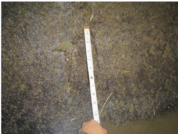
Photo 3-14. Surface Spalling at 100 ft (A)
