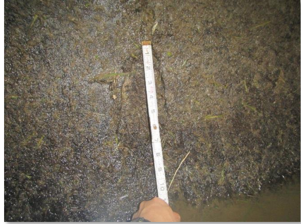
IMG_4026. Surface Spalling @ 100 ft (A)
