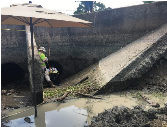
Photo 3-8. 48-inch South Inlet Structure
