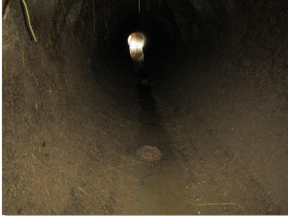
IMG_3972. 60-inch Pipe (C)
