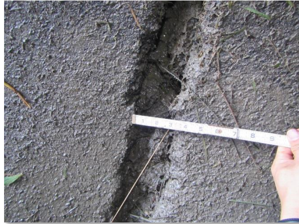
Photo 3-2. Pipe Joint Gap (15 ft)
