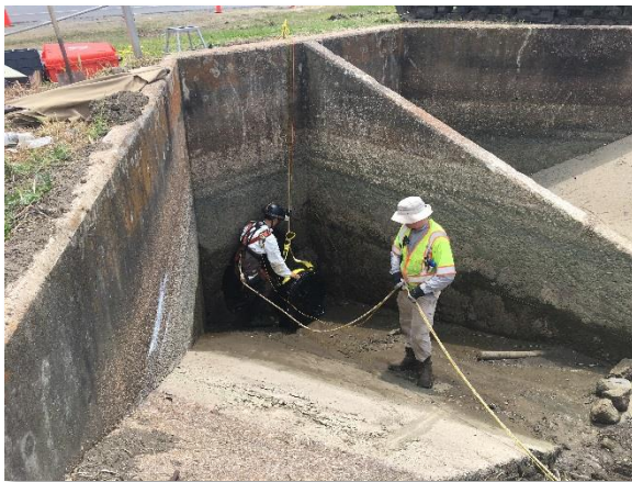
Photo 3-16. 48-inch North Inlet Structure
