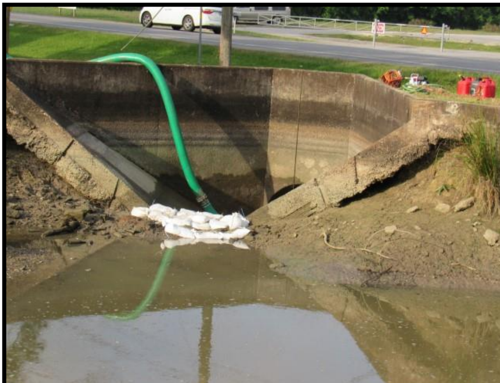
Cofferdam and pump suction at 60-inch downstream structure (looking upstream).
