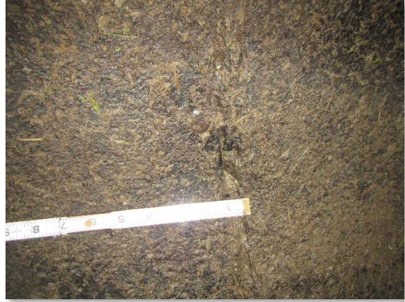
IMG_4054. Pipe Joint (Typ.)
