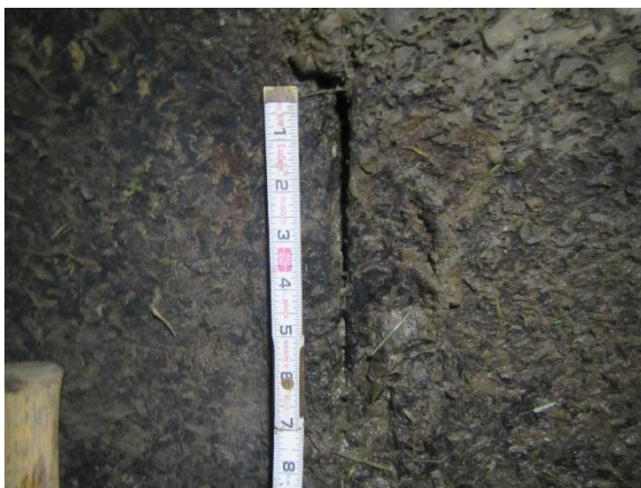
Photo 3-18. Small Joint Gap (Typ.)
