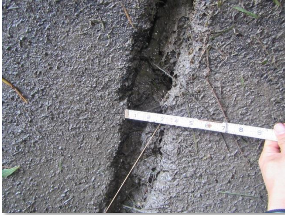
IMG_3957. 3.5-Inch Joint Gap at Inlet Change in Direction (A)
