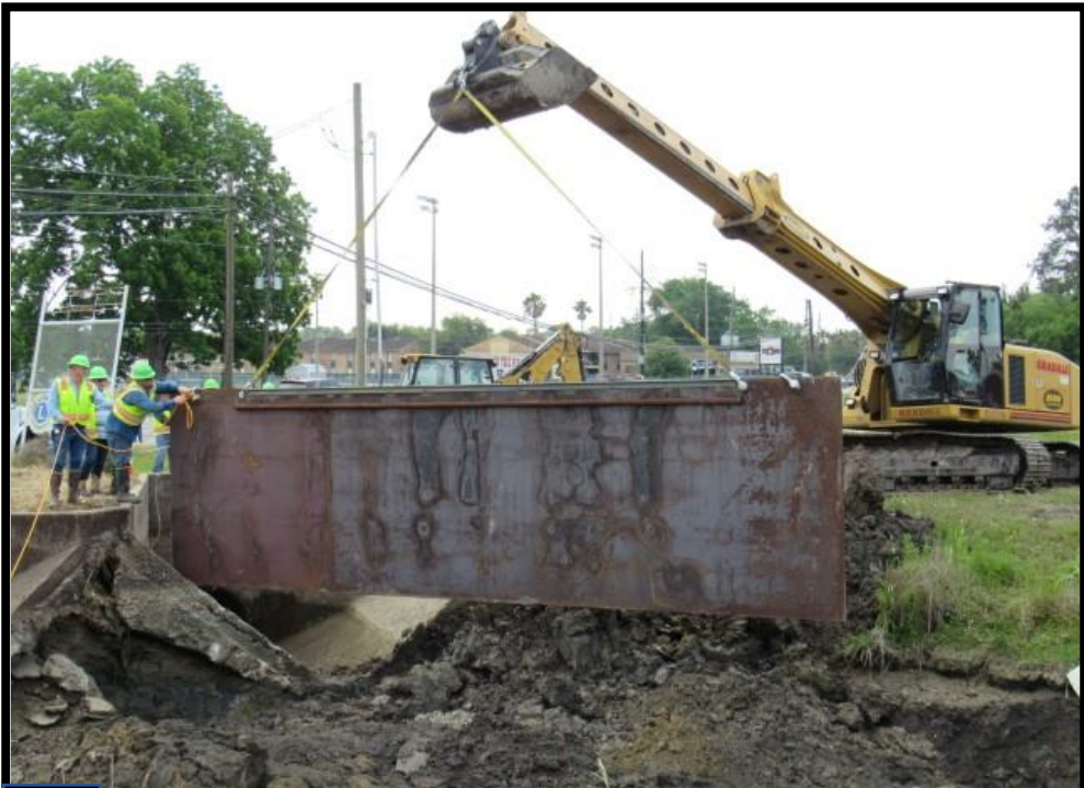
Steel plate installation at 60-inch bypass intake structure. (looking downstream/southeast)
