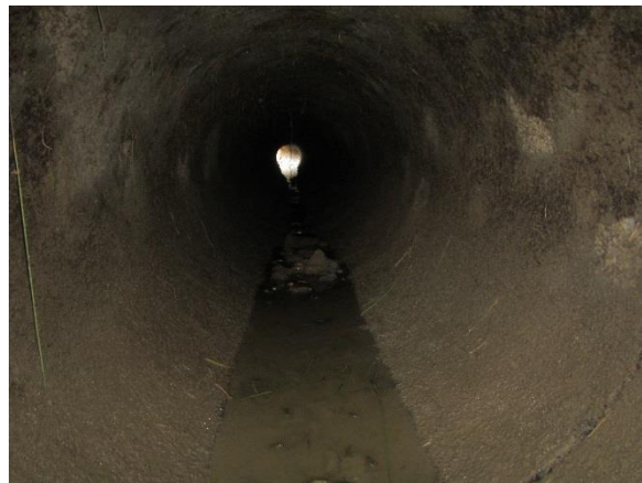
Photo 3-4. 60-inch Pipe Condition (Typ.)
