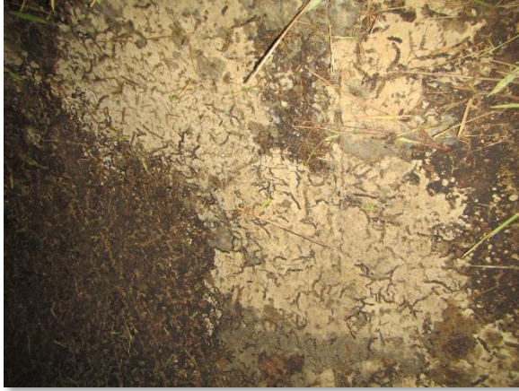
IMG_4053. 48-inch North Pipe Surface
