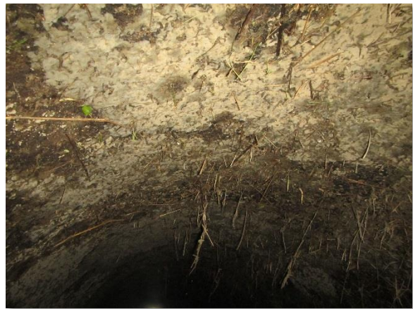
IMG_4052. Pipe Crown (A)
