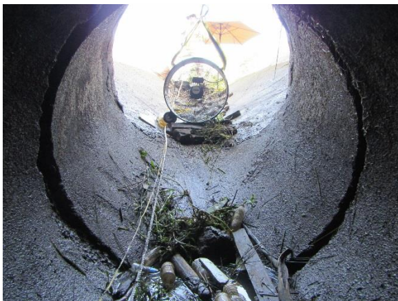
IMG_3955. Pipe Inlet (Upstream View)
