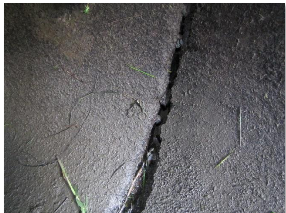
IMG_3962. Pipe Joint Missing Mortar @ 80 ft
