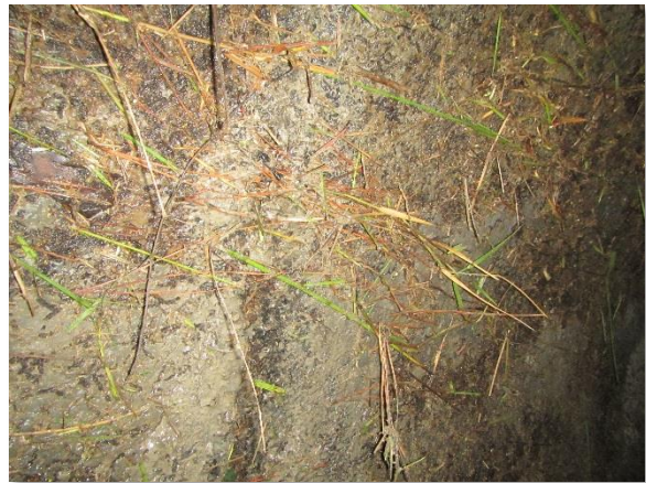
IMG_3967. 60-Inch Pipe Wall
