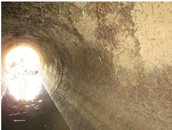
IMG_4029. 48-inch South Pipe Wall (A)
