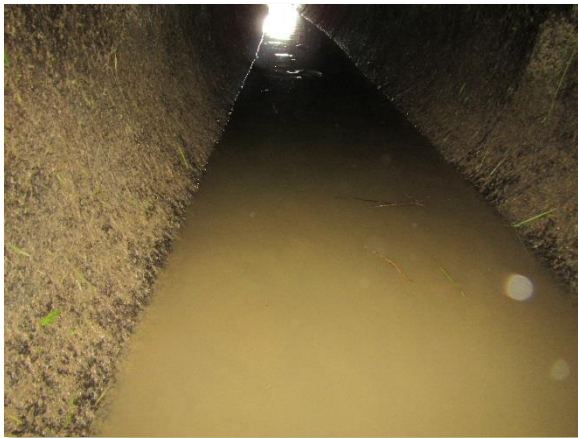
Photo 3-12. Possible Pipe Sag
