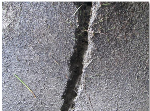
IMG_3956. Pipe Joint Missing Mortar @ 10ft
