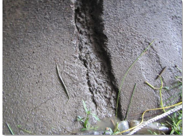
IMG_3958. 3.5-Inch Joint Gap at Inlet Change in Direction (B)
