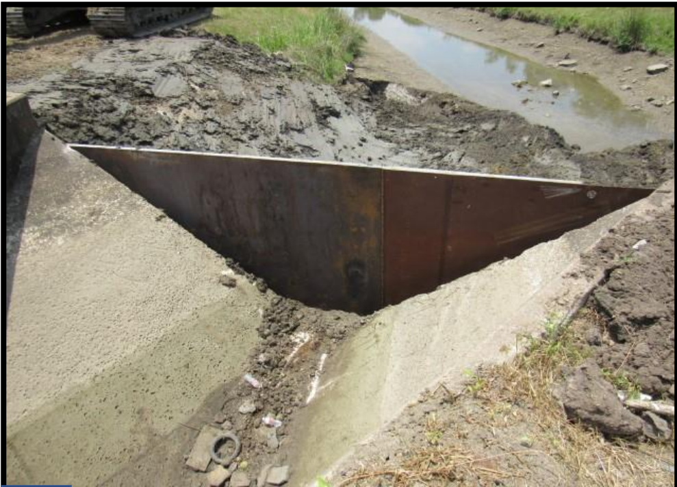
Final installation of steel plate at 60-inch bypass intake structure. (looking upstream)
