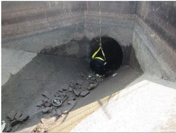
IMG_3953. 60-inch Inlet Structure
