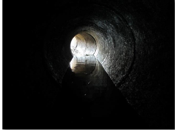
IMG_3973. 60-inch Pipe Outlet
