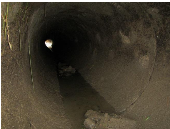
IMG_3961. 60-Inch Pipe and Debris
