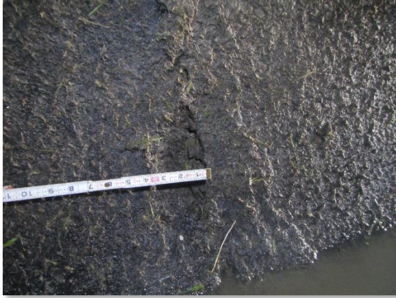
IMG_4025. Surface Spalling @ 100 ft (A)
