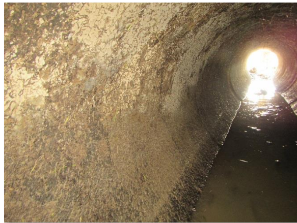
Photo 3-17. Pipe Surface (Typ.)
