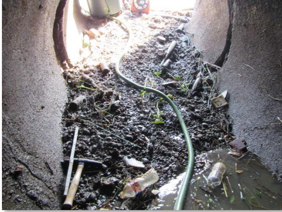
IMG_3981. Debris at 60-inch Pipe Outlet (A)
