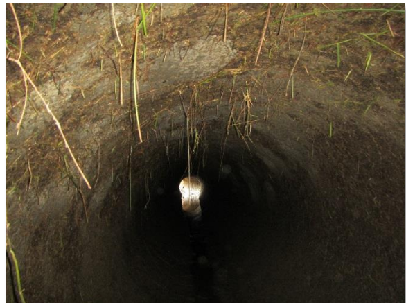
IMG_3971. 60-Inch Pipe Crown
