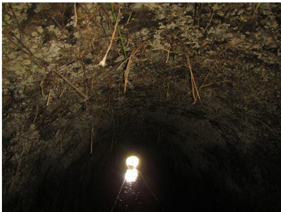
IMG_4061. Pipe Crown (B)
