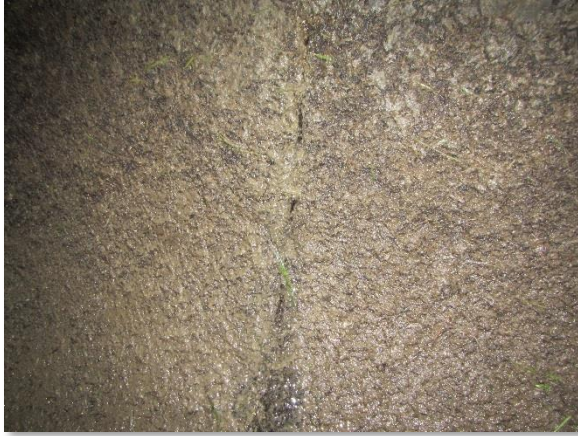
Photo 3-5. Surface Profile and Pipe Joint (Typ.)
