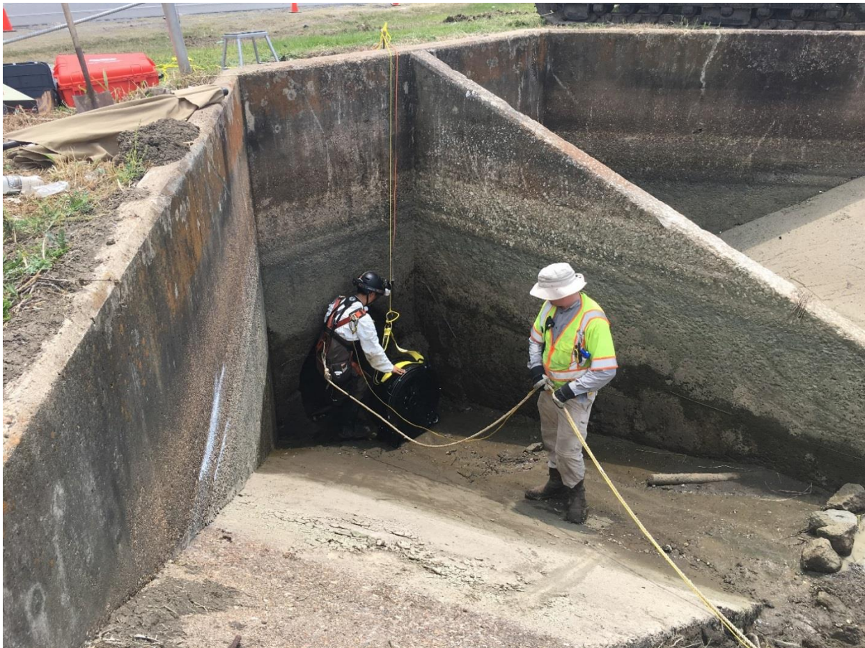
Photo 2-1. Confined Space Entry at SJRA Siphon 7 48-inch North
