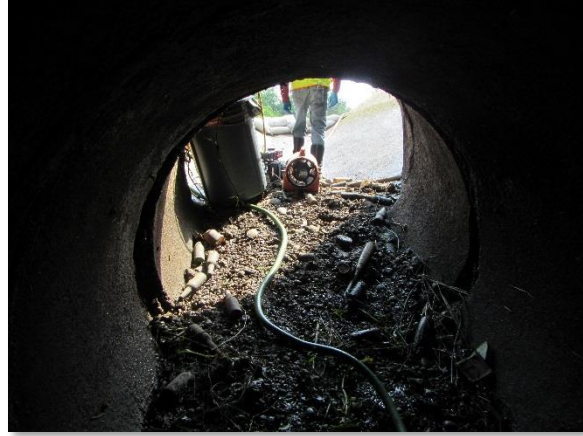
IMG_3982. Debris at 60-inch Pipe Outlet (A)
