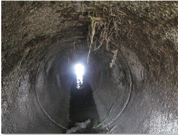
IMG_4037. 48-inch North Pipe
