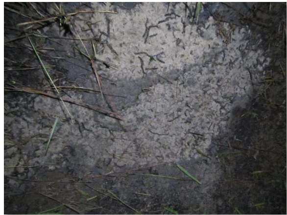
IMG_3978. Surface Delamination (Typ.)
