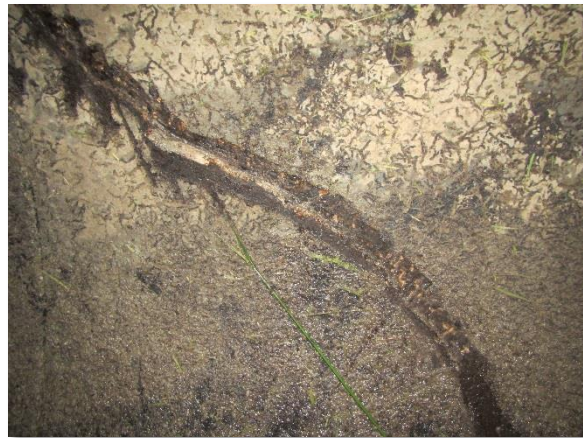
Photo 3-13. Possible Diagonal Cold Joint
