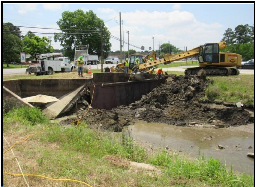
Steel plate installation at 60-inch bypass intake structure. (looking downstream/southeast)
