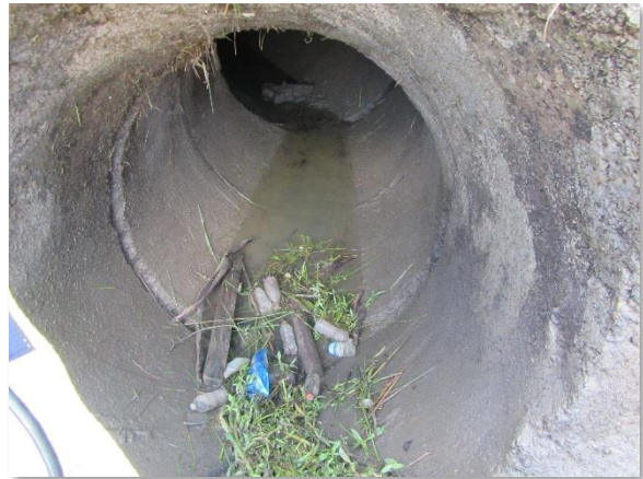
IMG_3954. Pipe Inlet
