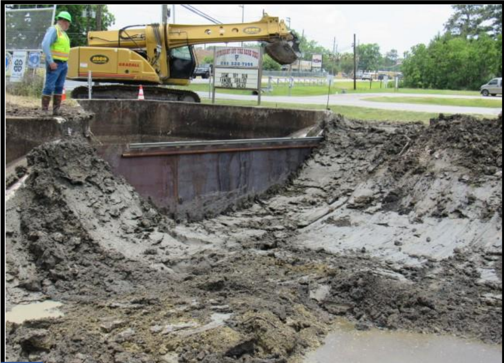
Backfill and re-grading behind steel plate. (looking downstream/southeast)
