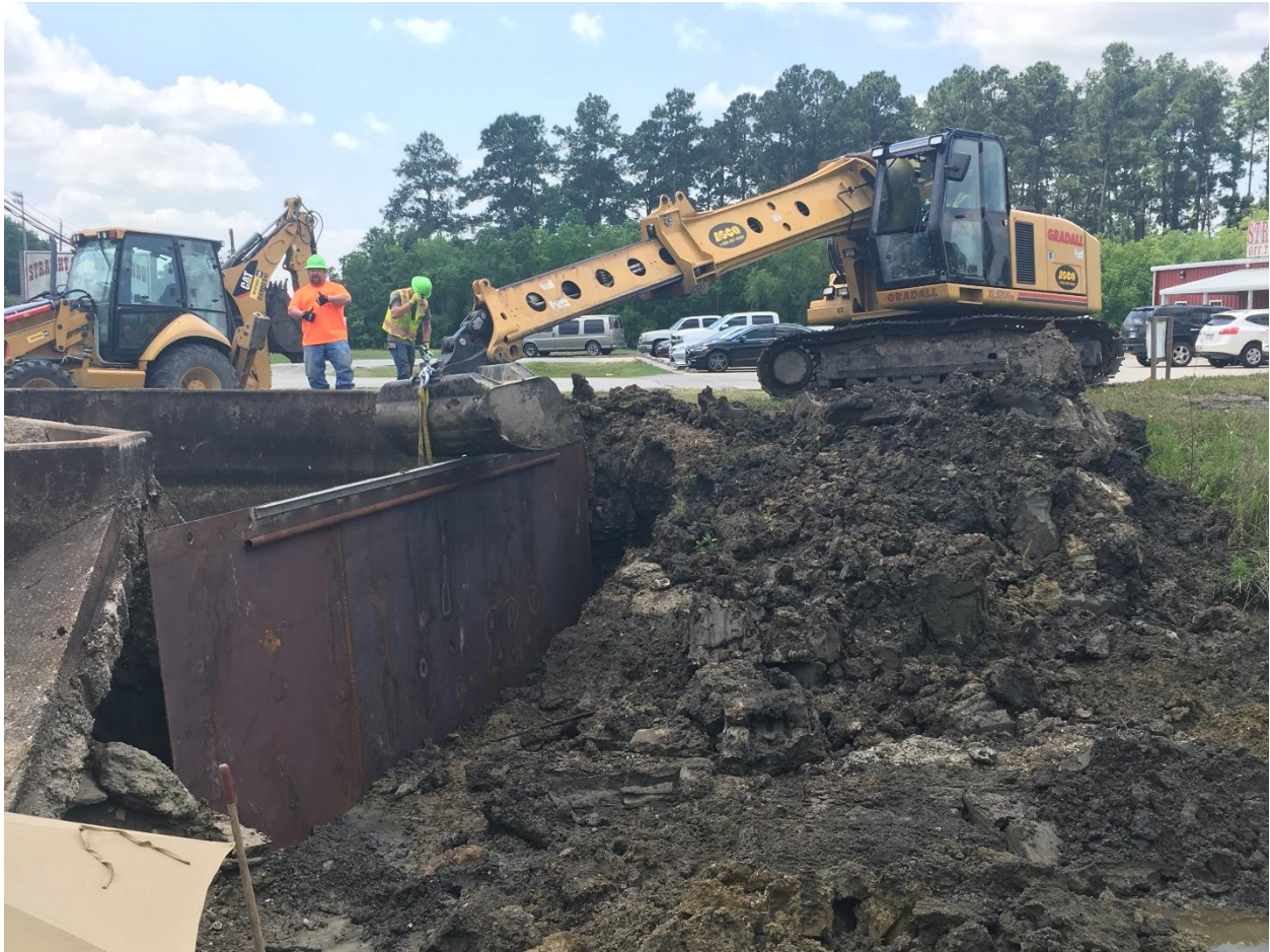
Photo 3-7. Steel Plate Installation at 60-inch Inlet Structure (Performed by SJRA)
