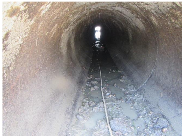
IMG_4069. 48-inch North Pipe Looking Upstream
