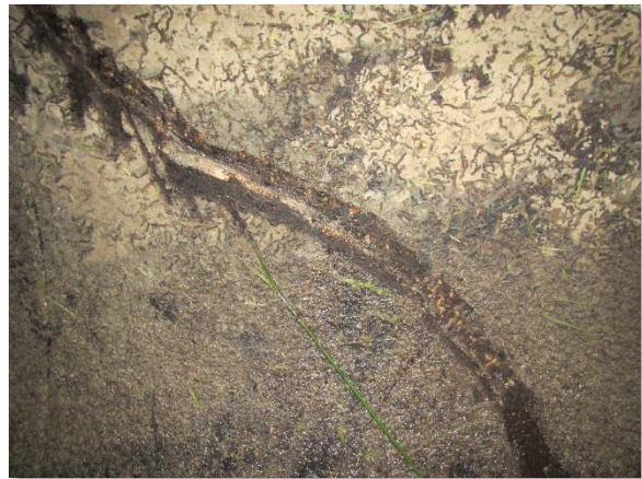
IMG_4019. Diagonal Cold Joint at 60 ft
