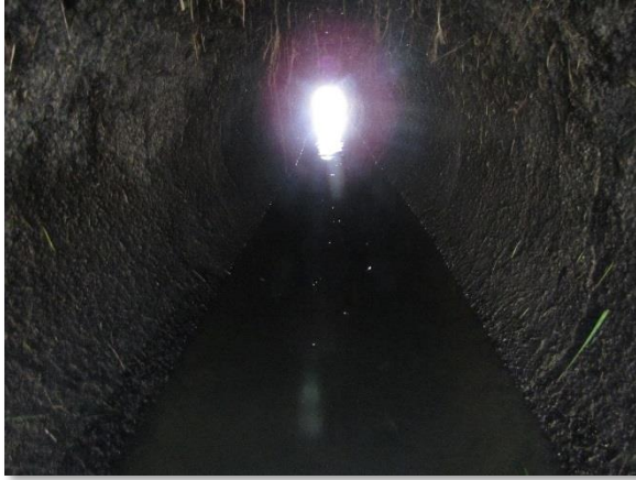
IMG_4011. 48-inch South Pipe (A)
