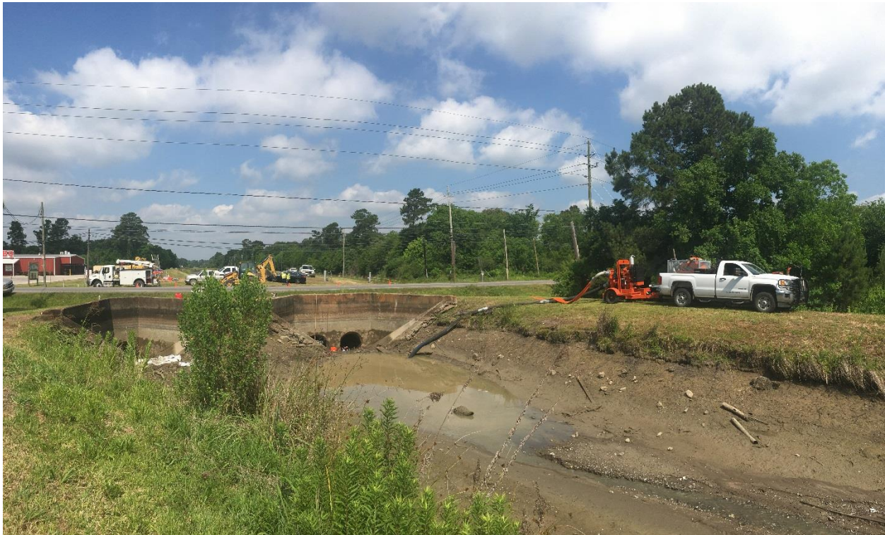
Photo 2-2. Dewatering at Downstream End of Siphon 7
