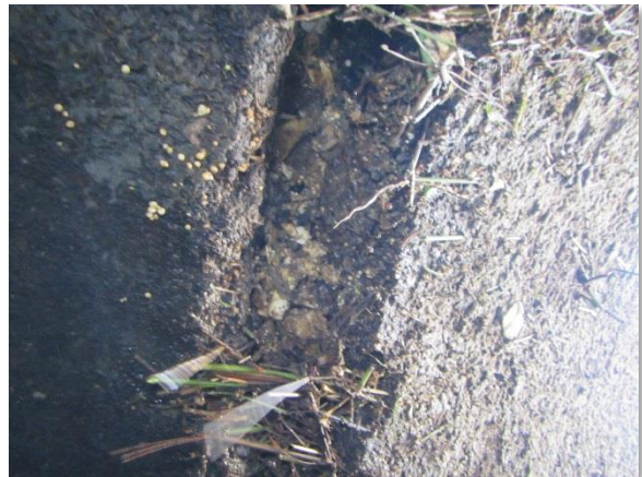
IMG_3960. 3.5-Inch Joint Gap at Inlet Change in Direction (D)
