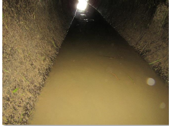
IMG_4017. Pipe Invert @ 50 ft
