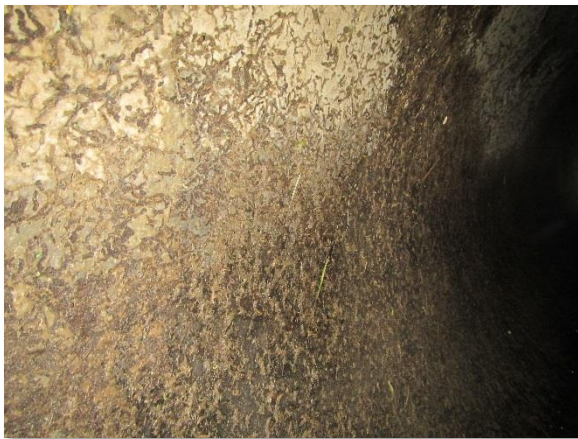
IMG_4051. 48-inch North Pipe Wall (B)
