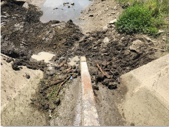
Photo 3-20. Removed Debris (Typ.)
