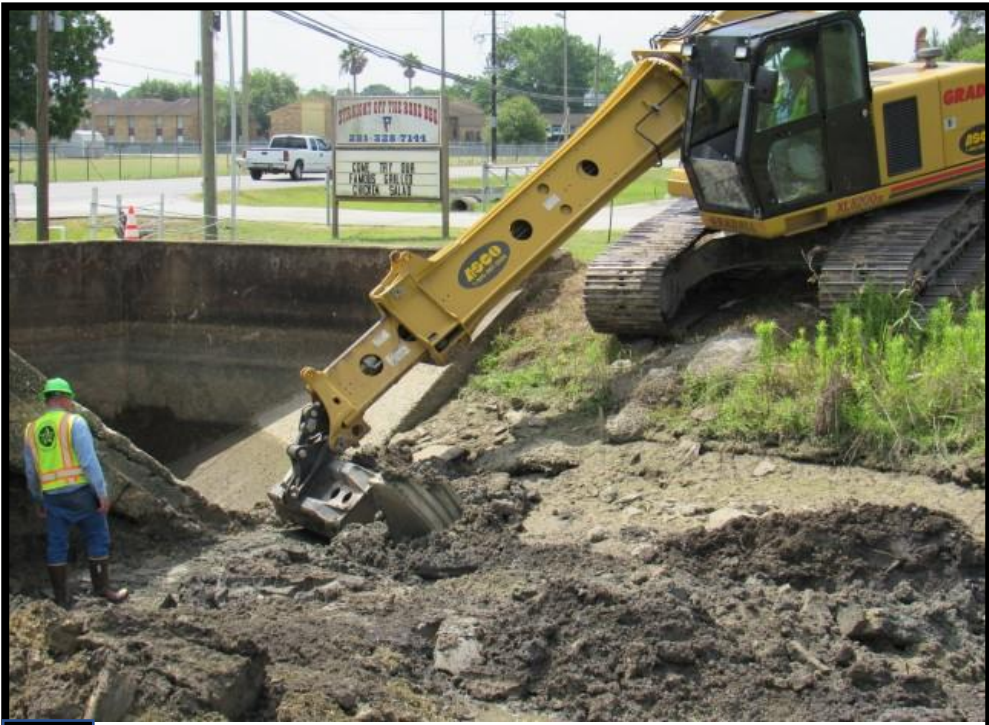
Grading for plate installation at the upstream of 60-in bypass. (looking downstream/southeast)
