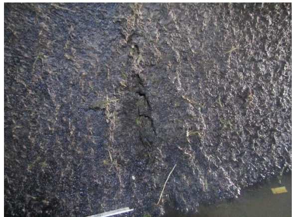
IMG_4024. Surface Spalling @ 100 ft (A)
