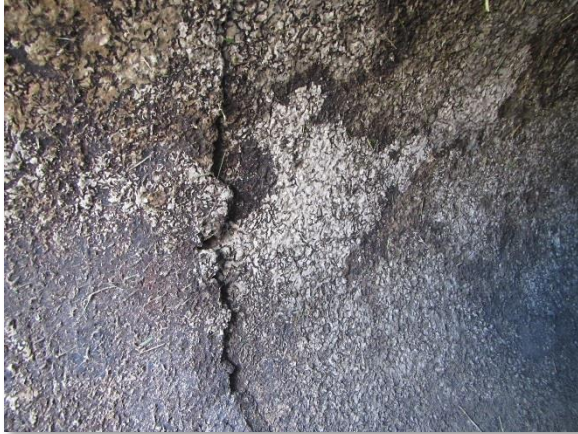
Photo 3-10. Surface Delamination at Joint (Typ.)
