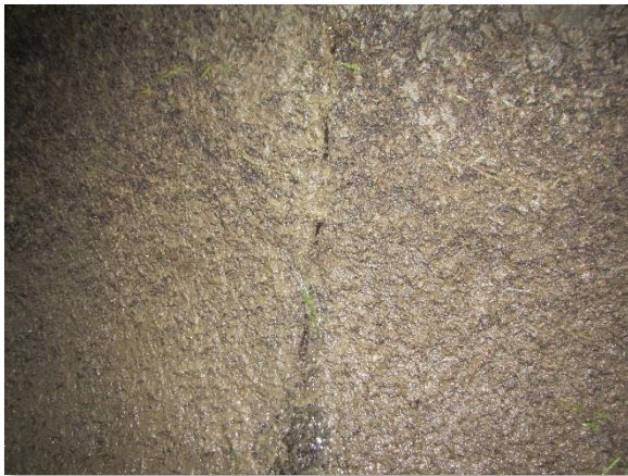
IMG_3966. Pipe Joint (Typ.)
