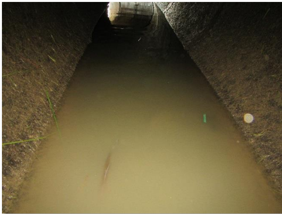
IMG_3974. Pipe Invert
