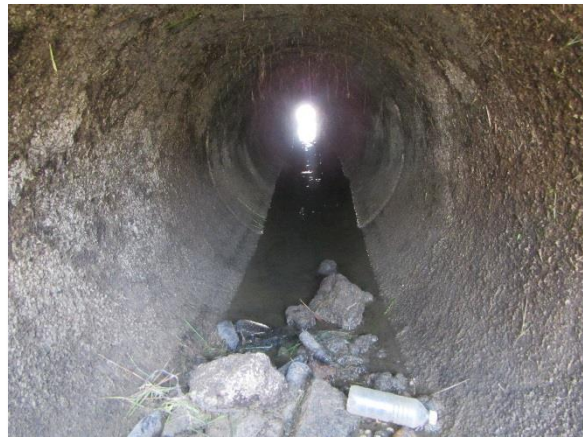
Photo 3-9. Pipe Profile and Debris (Typ.)
