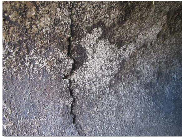
IMG_4005. Delamination at Pipe Joint (Typ.)
