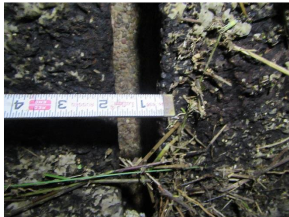
IMG_4009. Pipe Joint Missing Mortar @ 10ft
