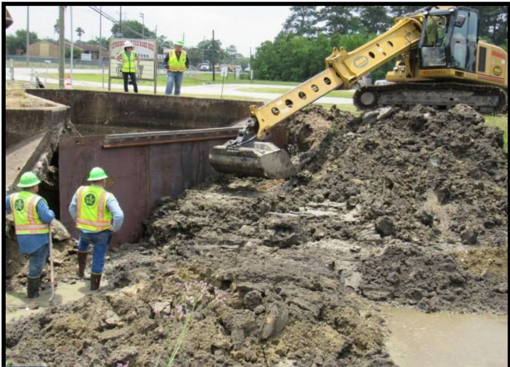
Backfilling behind steel plate. (looking downstream/southeast)
