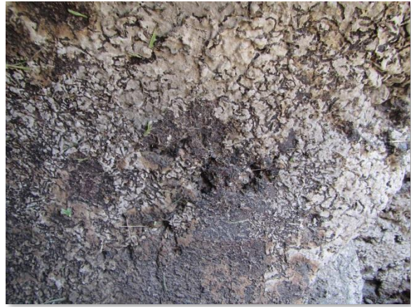
IMG_4038. 48-inch North Pipe Wall (A)
