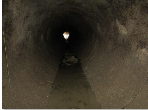
IMG_3964. 60-inch Pipe (A)
