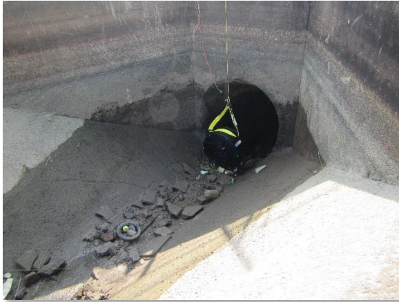
Photo 3-1. 60-inch Inlet Structure
