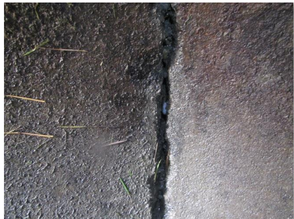
IMG_3980. Pipe Joint Missing Mortar at Last Joint
