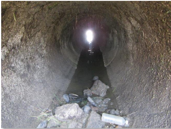
IMG_4004. Debris at Pipe Inlet
