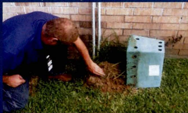
Randy Acreman inspects an Aerator on an OSSF System
