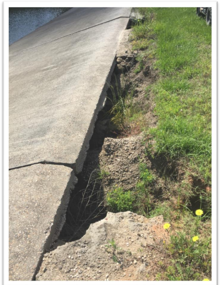
Above: Typical undermining of original Outlet Channel slope paving.
