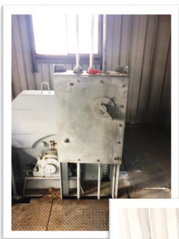
Left: Old starter cabinet exterior.
