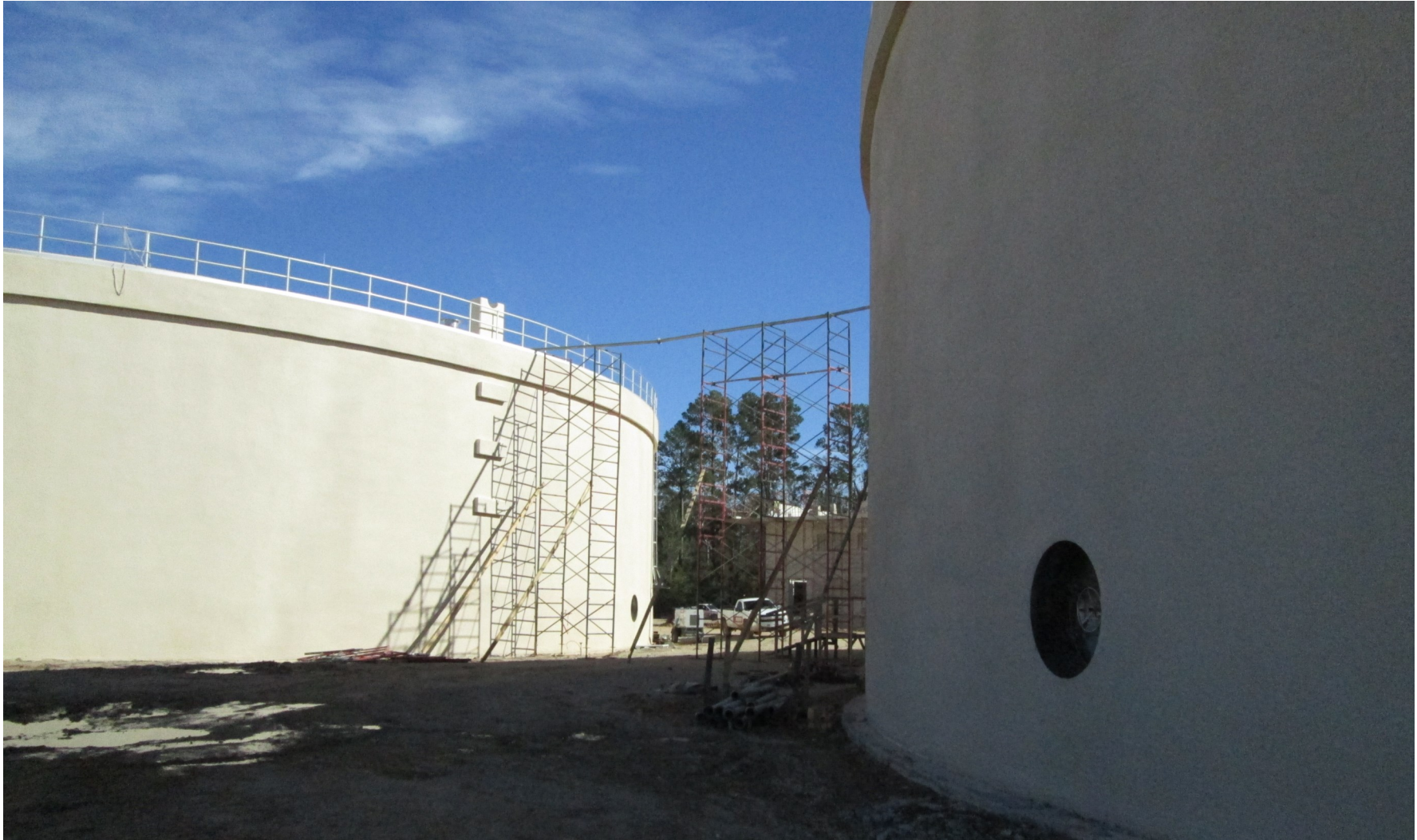
⑧ Ground Storage Tank No. 2 preparing for water tightness test (leak testing?)
