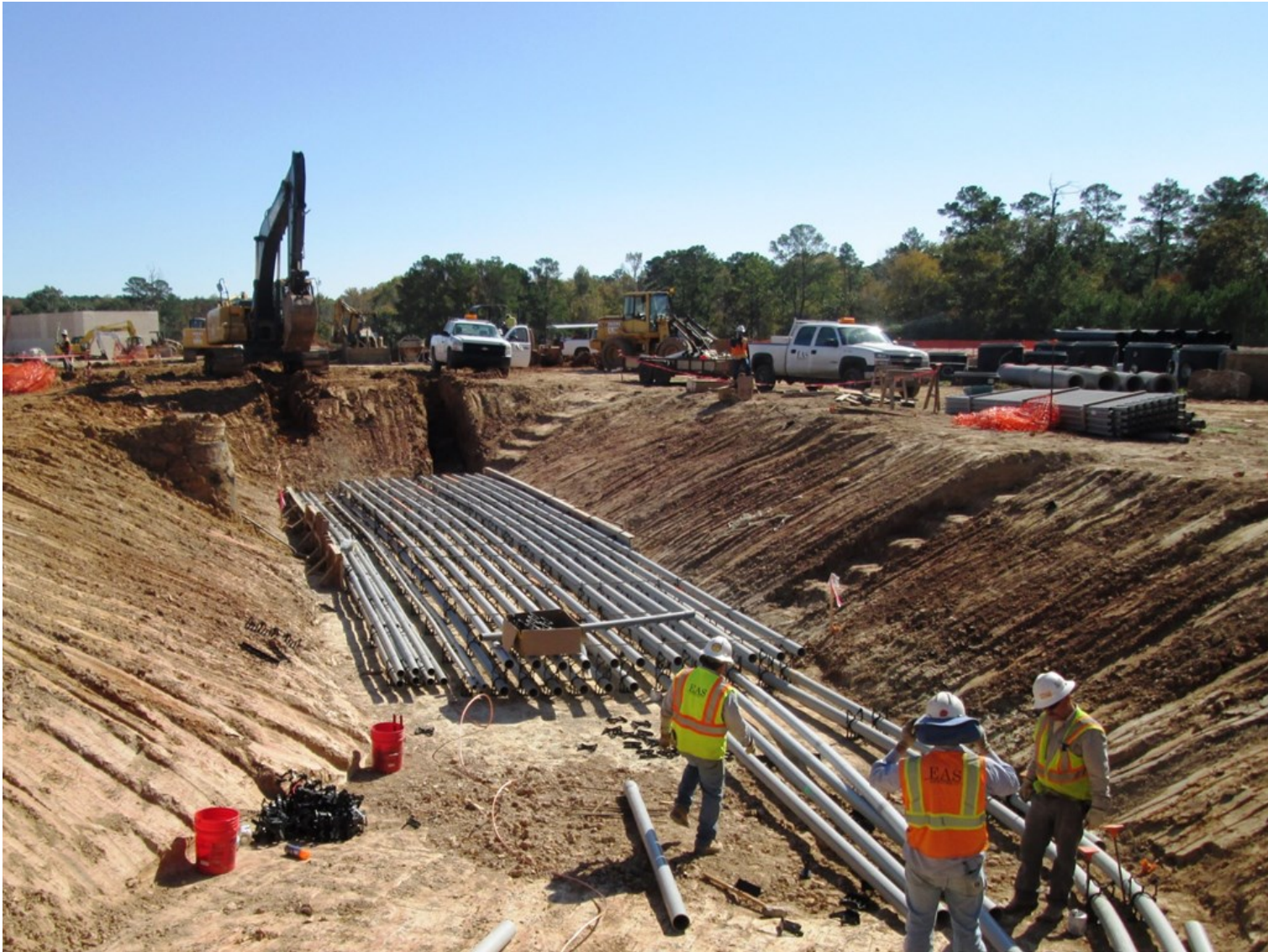
15 Electrical duct bank from Electrical Building to the High Service Pump Station
