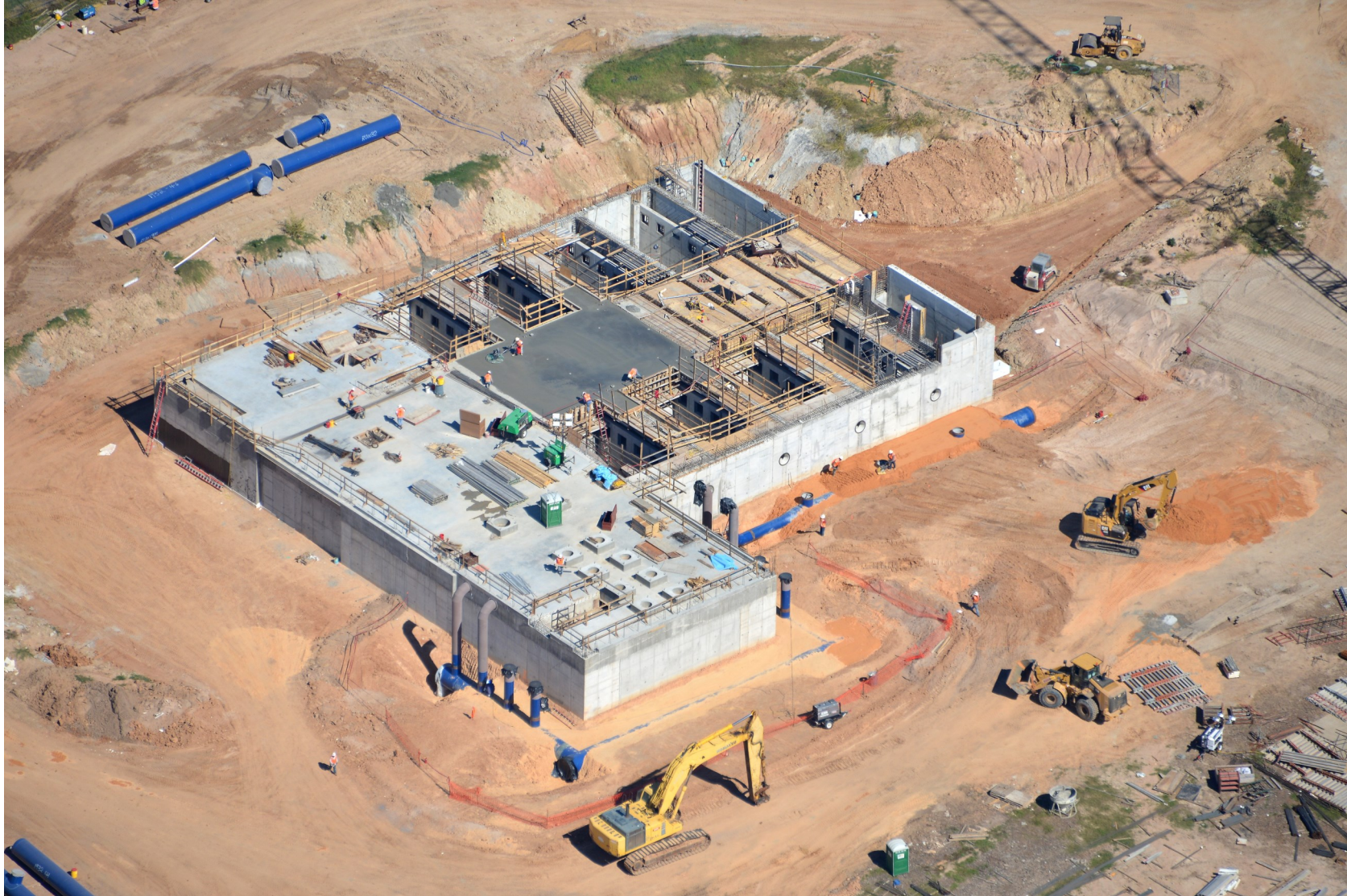
⑦ Aerial view of Granular Activated Carbon Facilities second floor concrete deck installation
