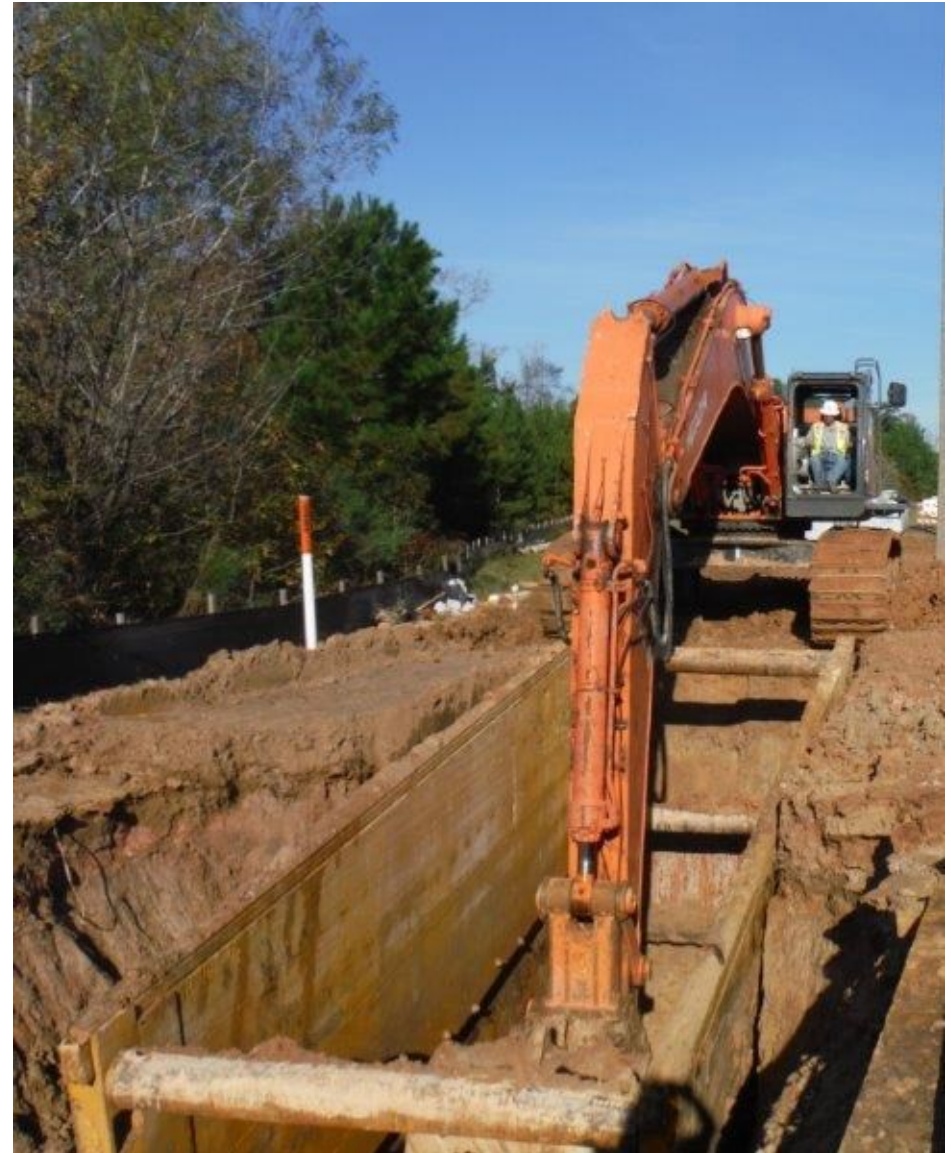
① Segment T2 - 54-inch pipe installation along Fish Creek Thoroughfare
