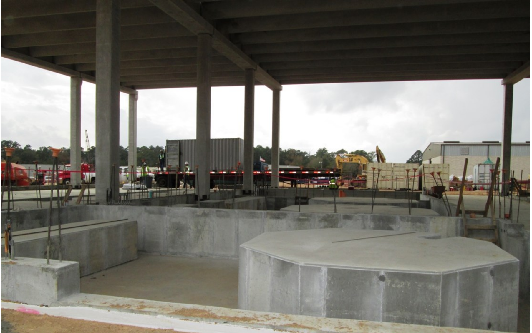
16 Chemical Building foundation and precast structure complete
