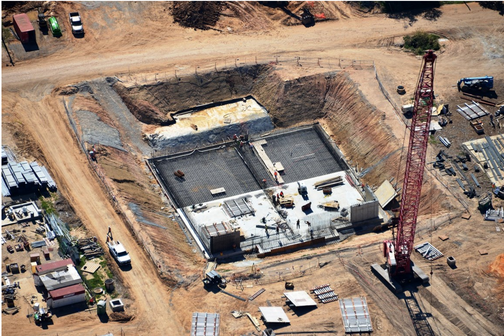
17 Aerial View of Backwash Equalization Basin foundation installation
