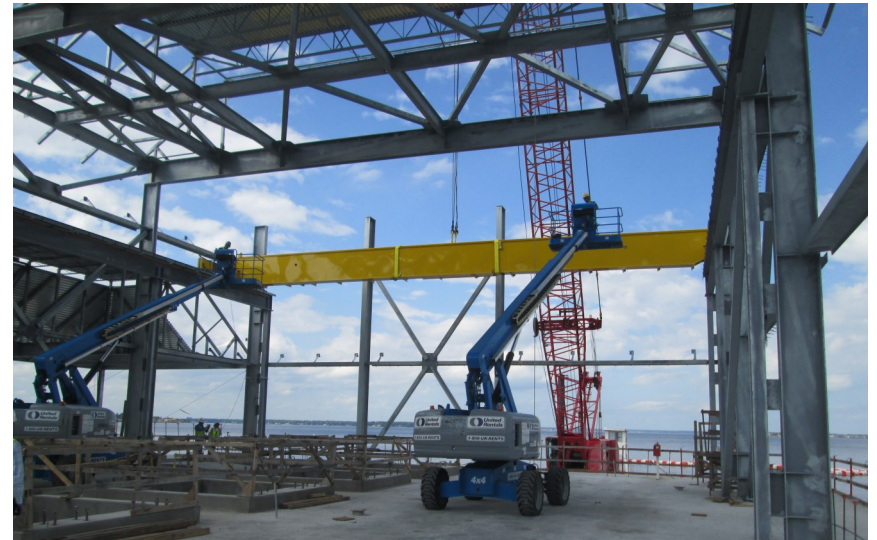
① ② ③ 30-ton bridge crane installed and building steel erection at Raw Water Intake Station
