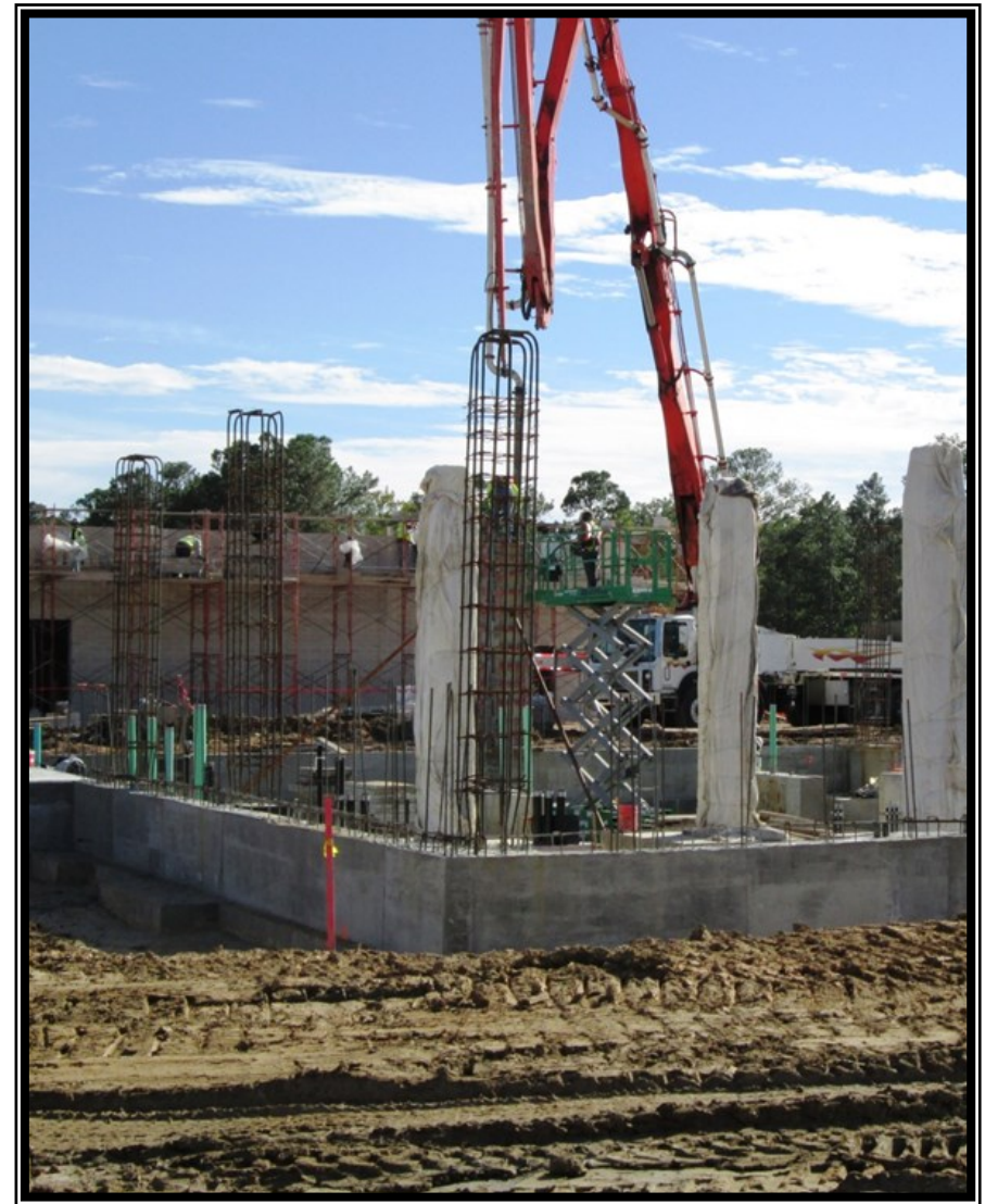
Surface Water Facilities — Concrete columns at Dewatering Building
