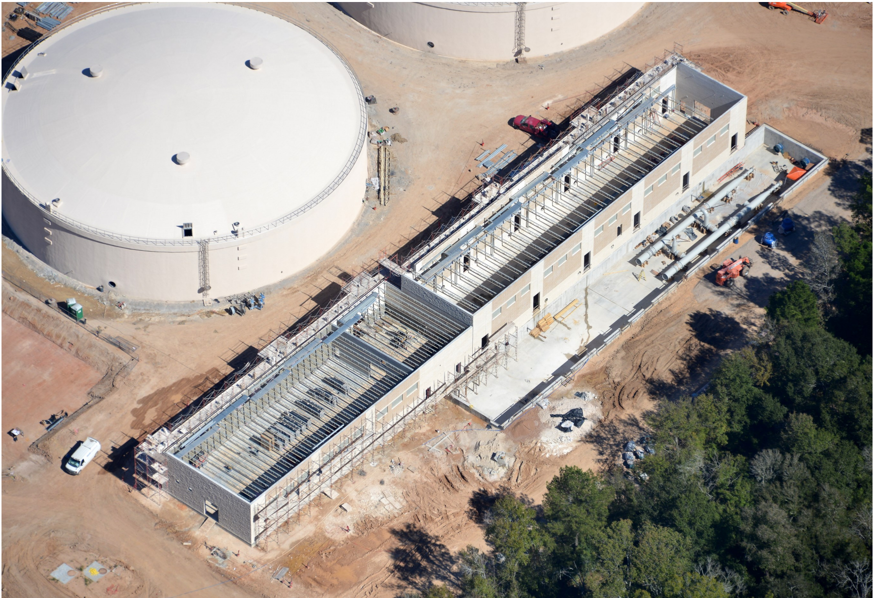
9 Aerial view of HSPS roof framing installation
