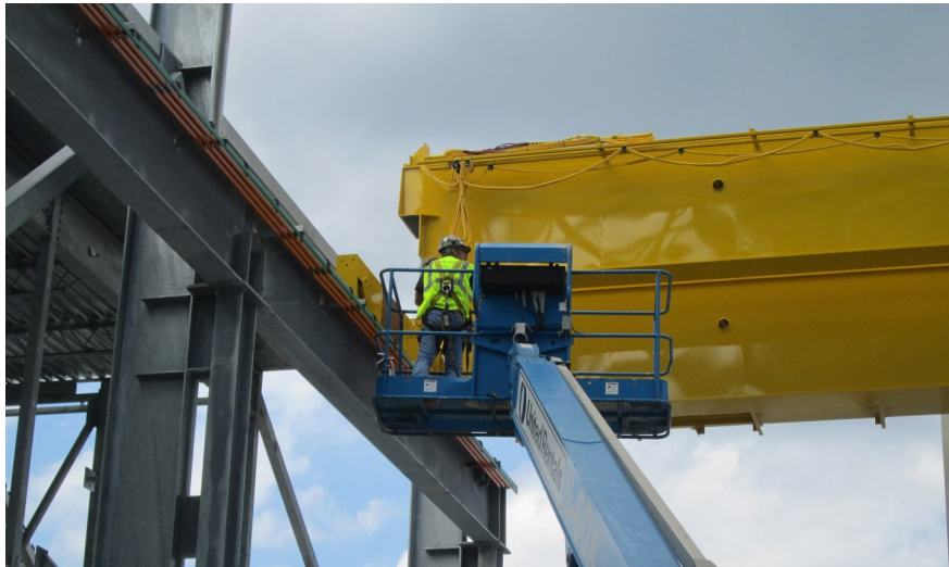
① ② ③ 30-ton bridge crane installed and building steel erection at Raw Water Intake Station
