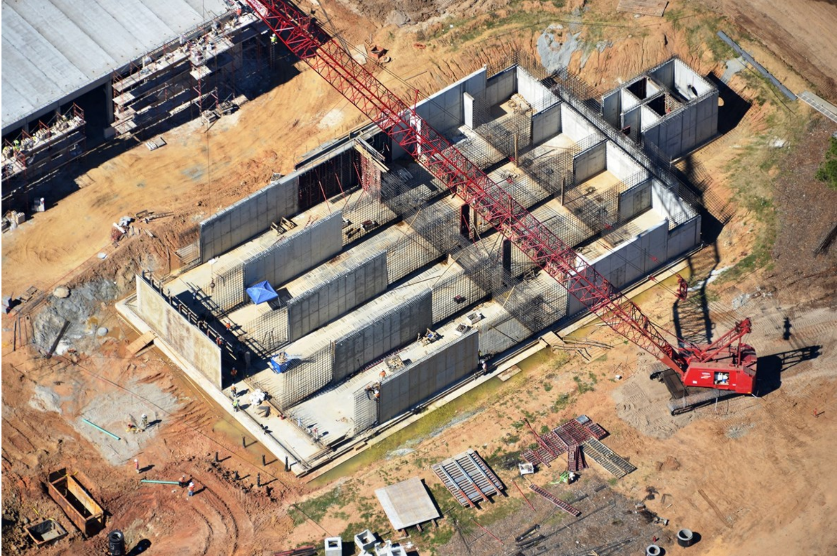
④ Aerial view of Pretreatment foundation installation
