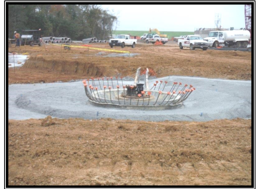
Above: SWF—Base of sludge thickener at solids dewatering area
