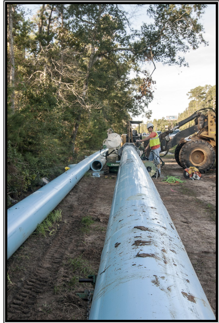
Segment W1A — Welded PVC pipe along FM 2978
