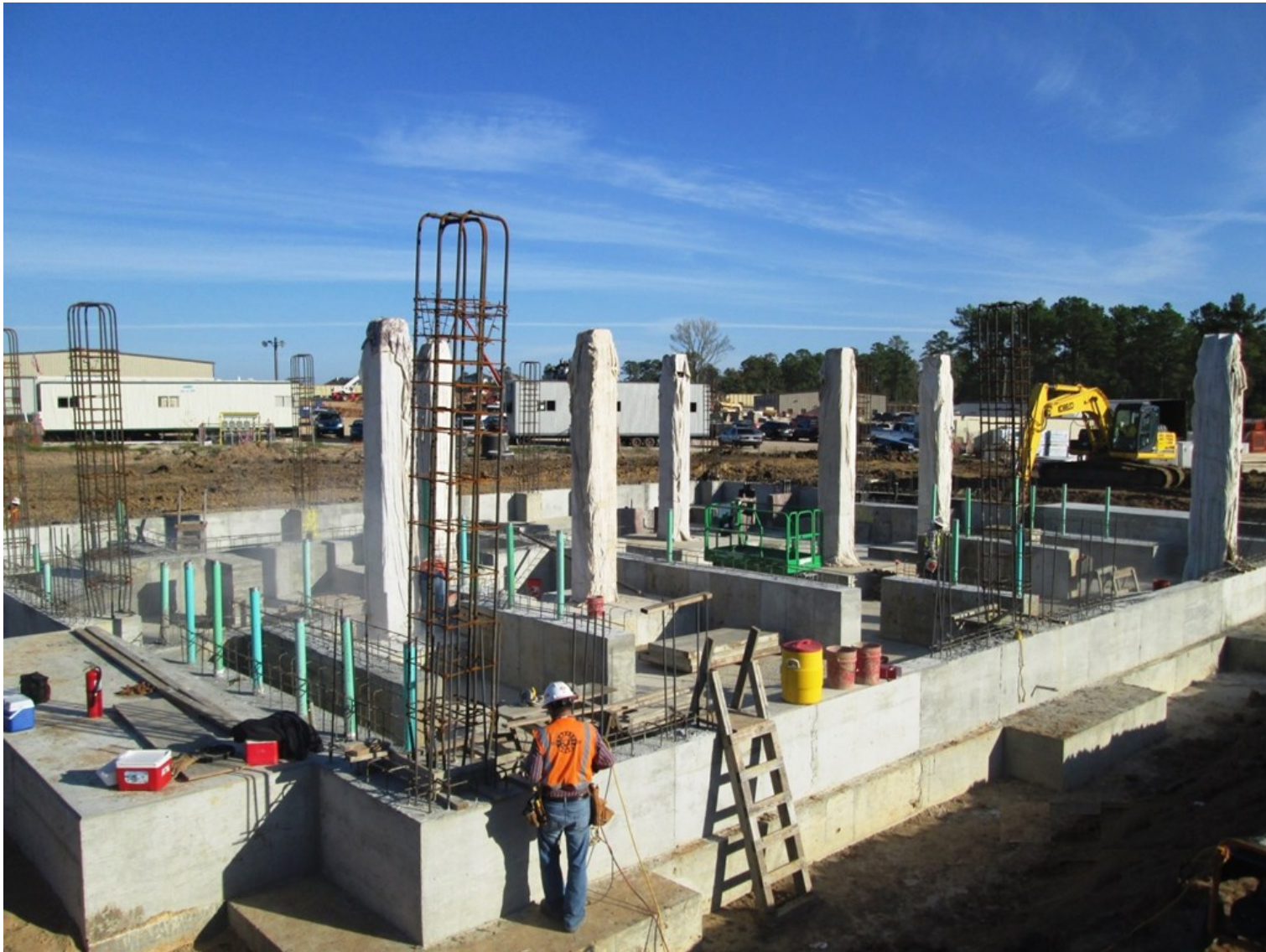
19 Installation of cast-in-place concrete columns
