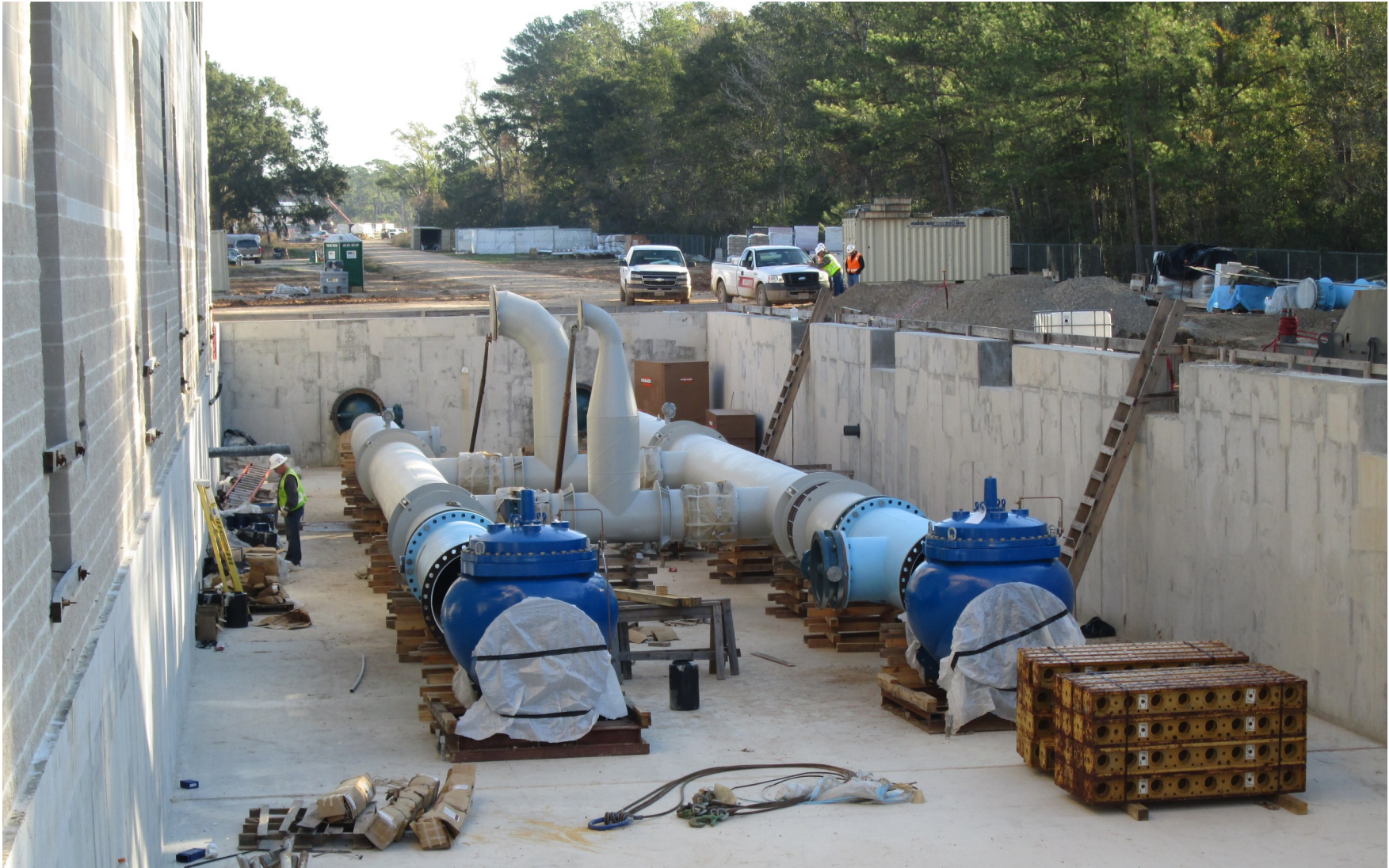
13 High Service Pump Station Discharge Bay Piping
