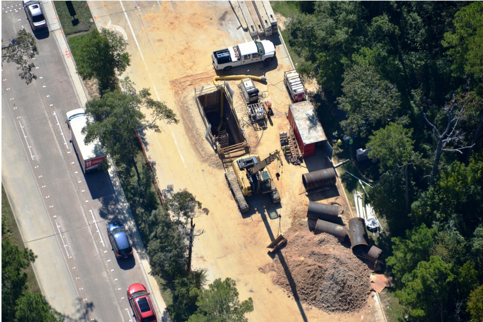
① Segment W2A - Tunnel operation utilizing 60-inch casing along Research Forest Drive at Shadowbend Place
