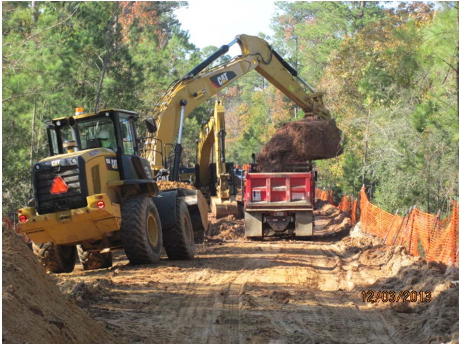
① Segment W1B - Open cut operation along future Research Forest Drive
