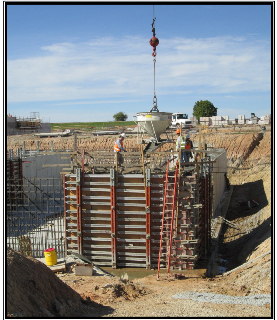
Surface Water Facilities—Placement of concrete along southeast wall at GAC
