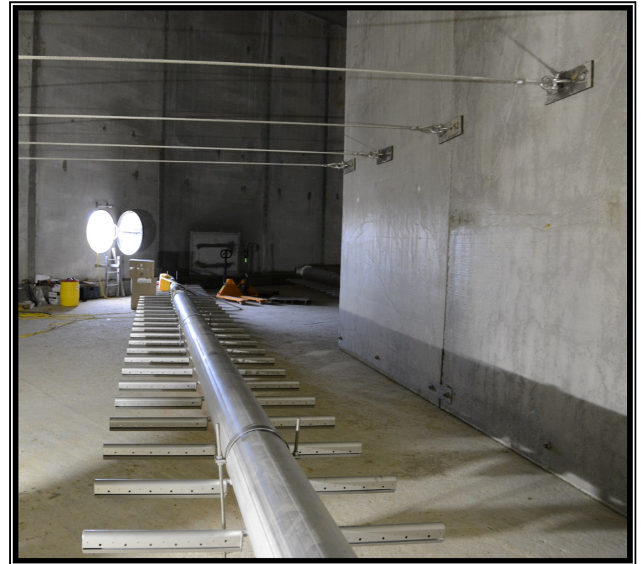
Surface Water Facilities—View of aeration system inside Ground Storage Tank
