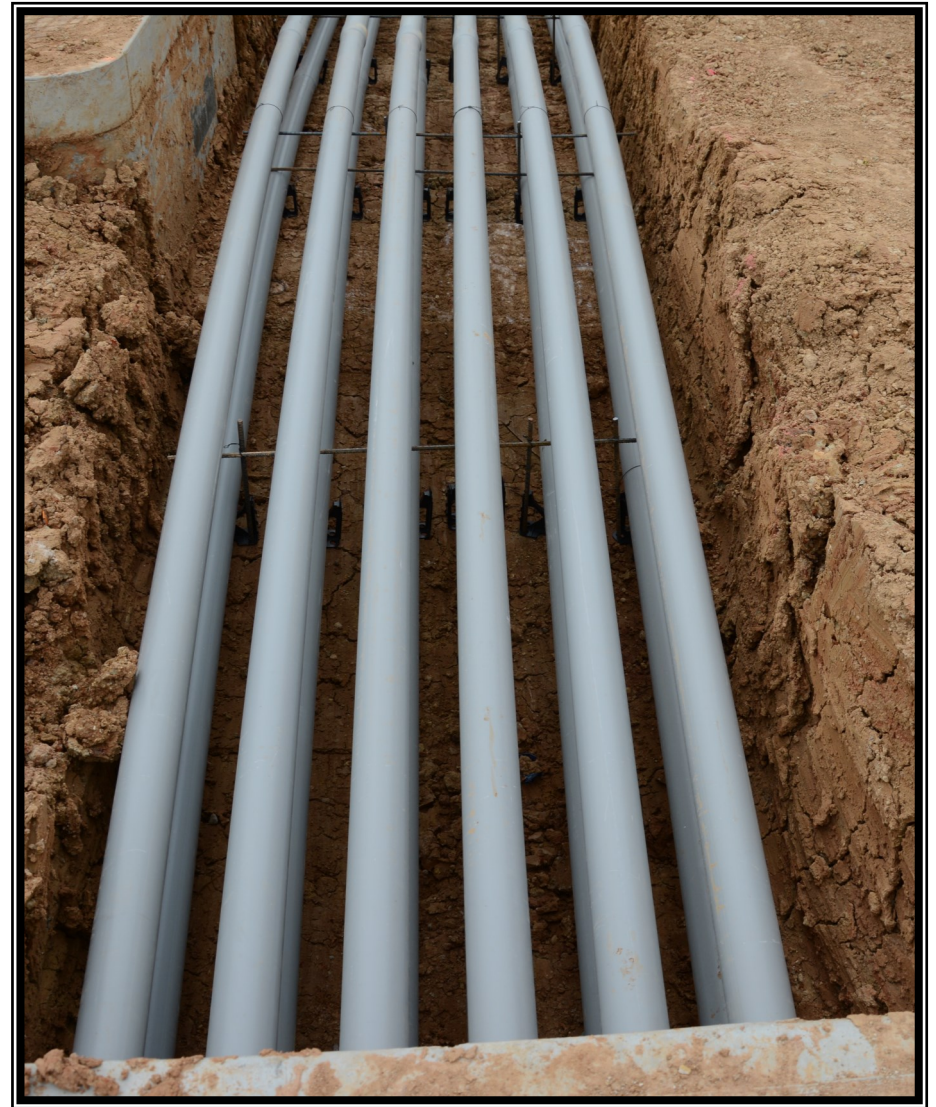
Surface Water Facilities— Electrical duct bank installation near Electrical Building
