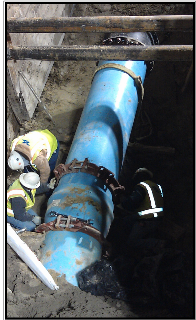
Restrained joint installation along Segment W2A
