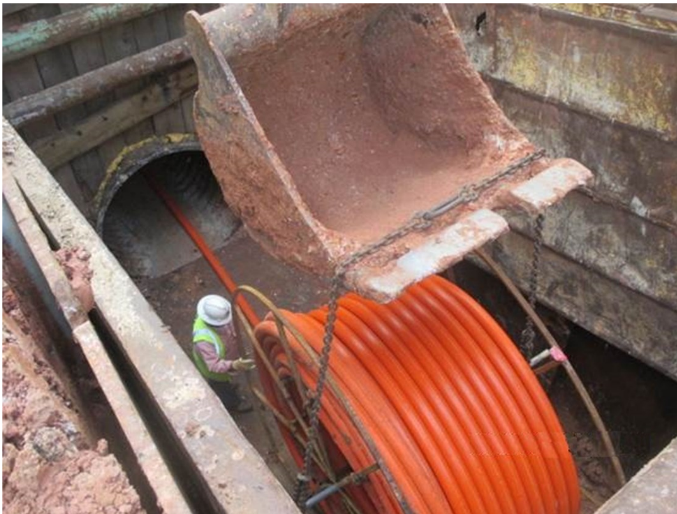
❶ Segment W1B - Fiber optic conduit installation along Research Forest Drive near Alden Bridge Drive
