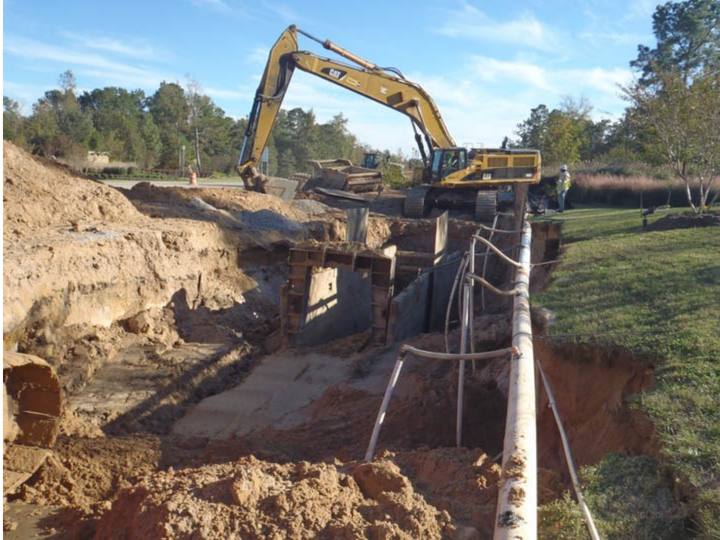
❶ Segment T3—54-inch pipe installation along Fish Creek Thoroughfare near Lake Creek
