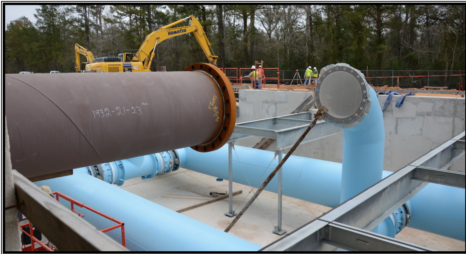
Surface Water Facilities—HSPS discharge header
