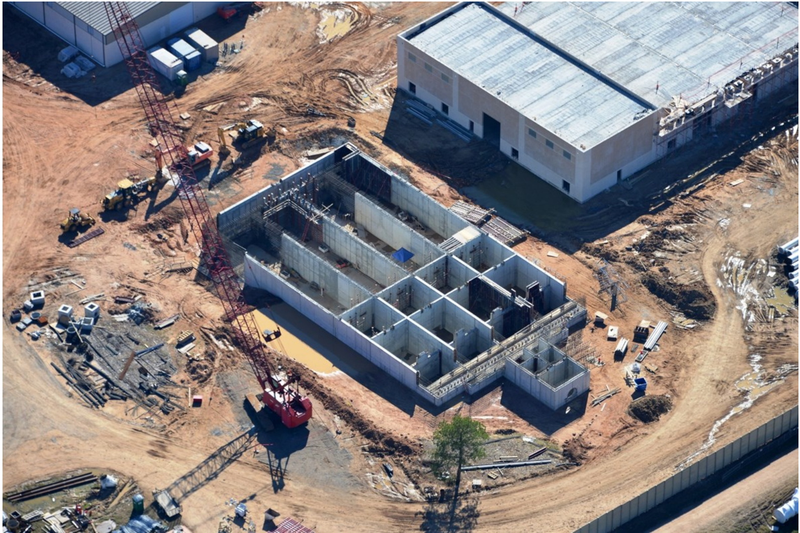
② Aerial view of intermediate concrete walls at the Pretreatment Facilities
