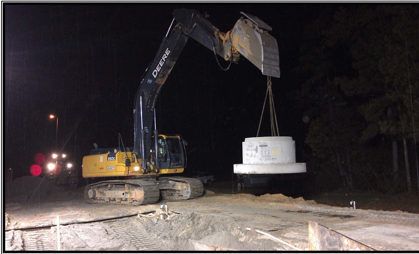
Installation of valve access manhole along Segment W2A
