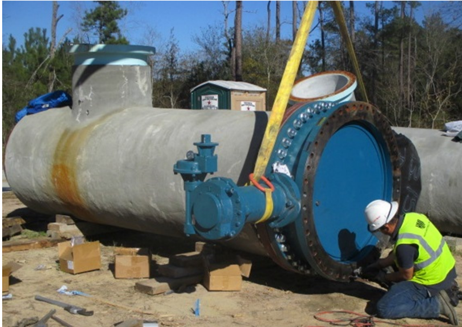
① Segment W1A—48-inch pipe and butterfly valve installation along future Research Forest Drive
