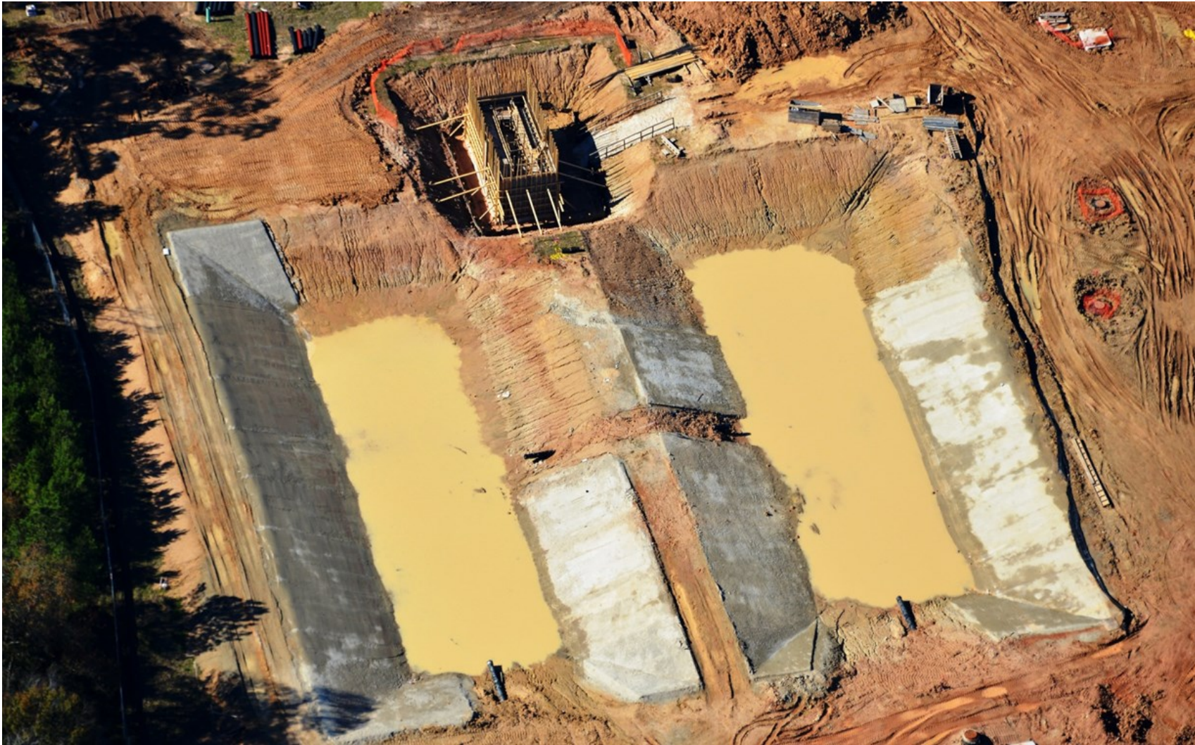
⑪ Aerial view of water recovery basins and pump station foundations
