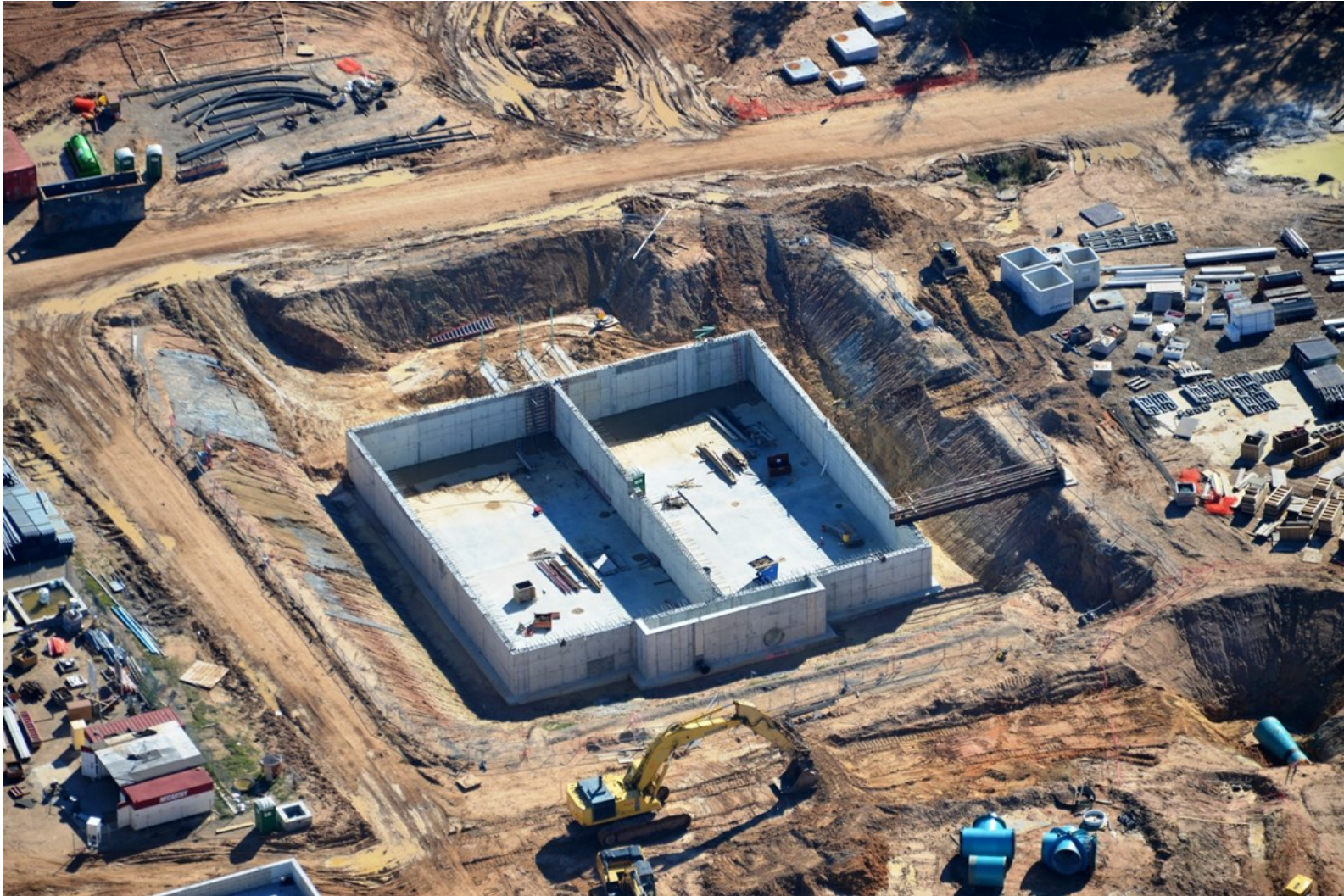
⑧ Concrete walls complete, walkways under construction at Backwash Equalization Basin
