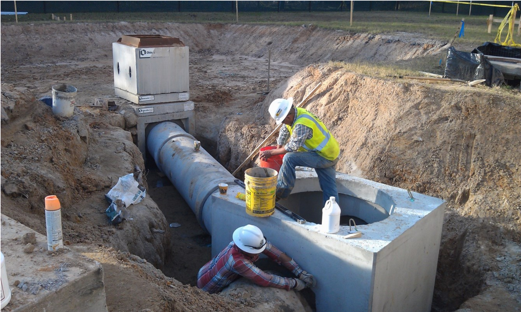
❶ Water Receiving Facilities—South—Stormwater pipe installation at SJRA Water Plant No. 4
