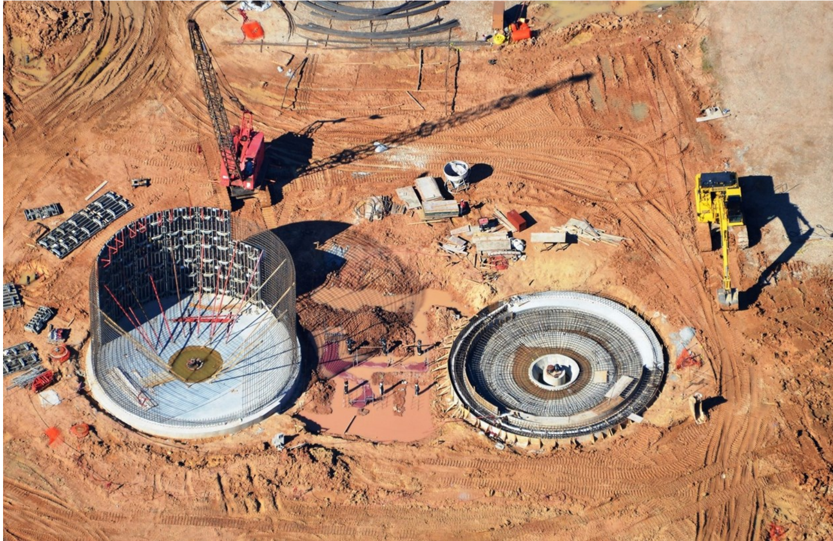
⑩ Aerial view of concrete wall placement at thickeners
