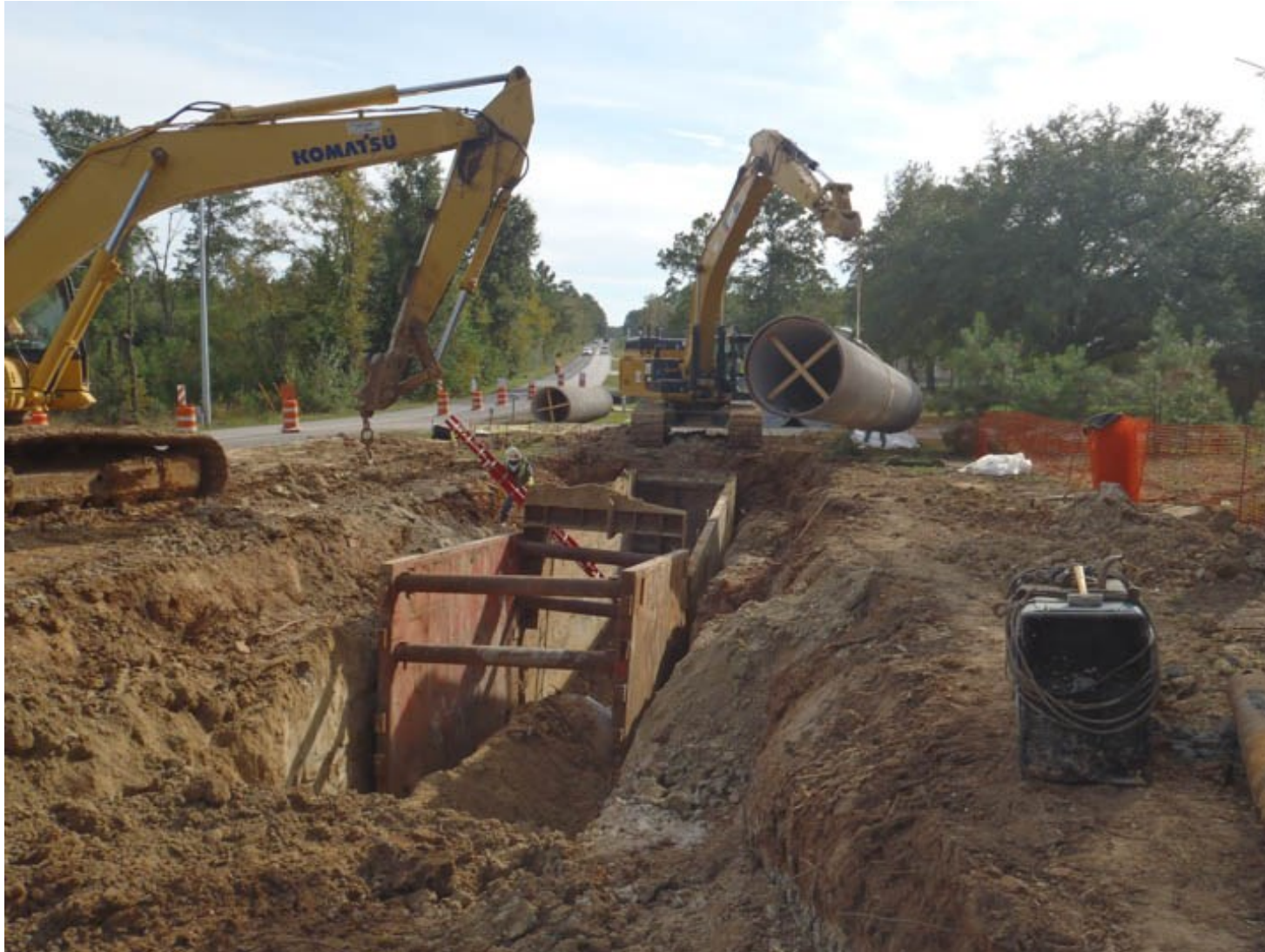
❶ Segment T1 - 60-inch pipe installation along McCaleb Road
