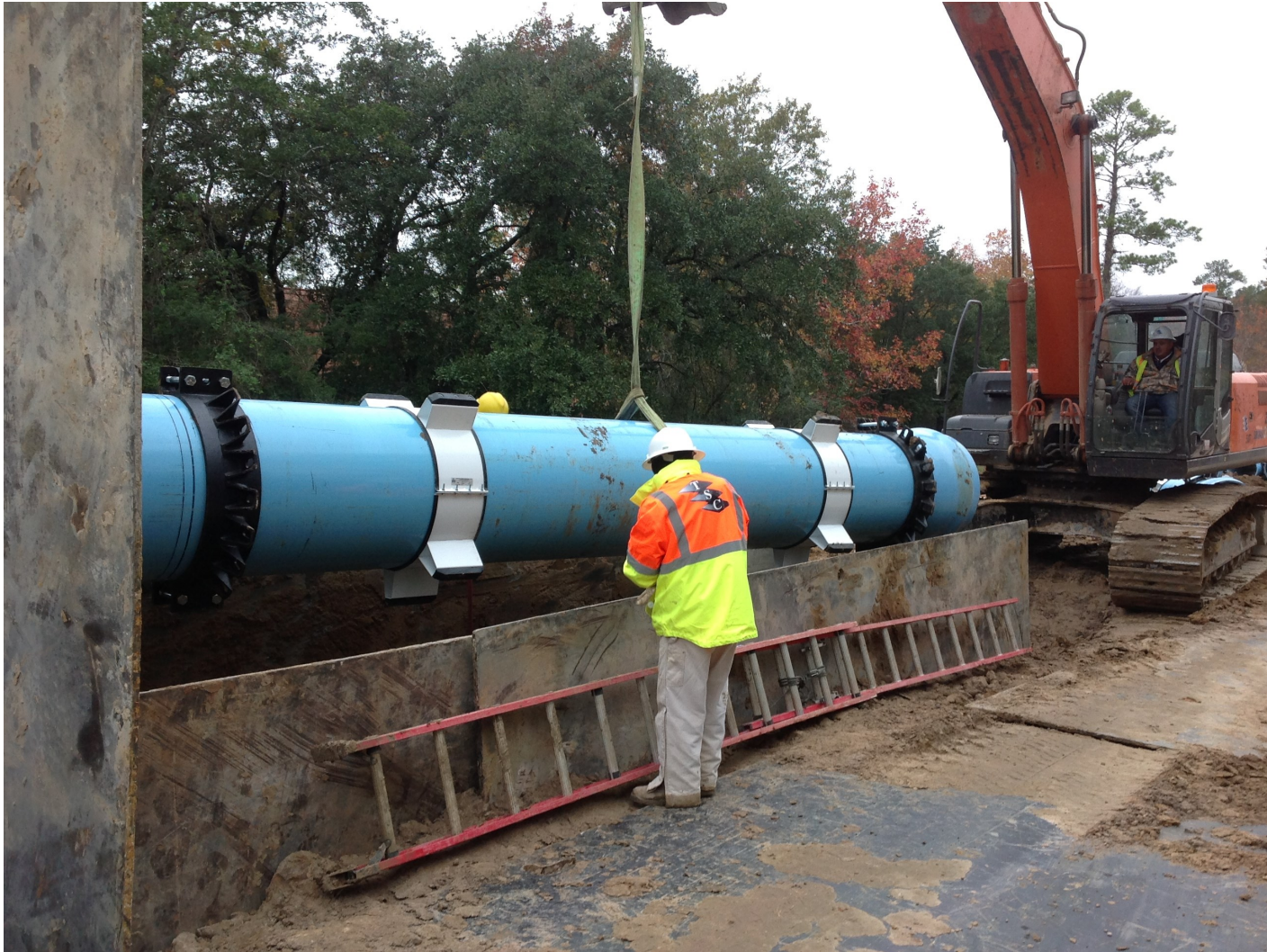
❶ Segment W2B - 30-inch pipe installation along Grogan's Mill Road
