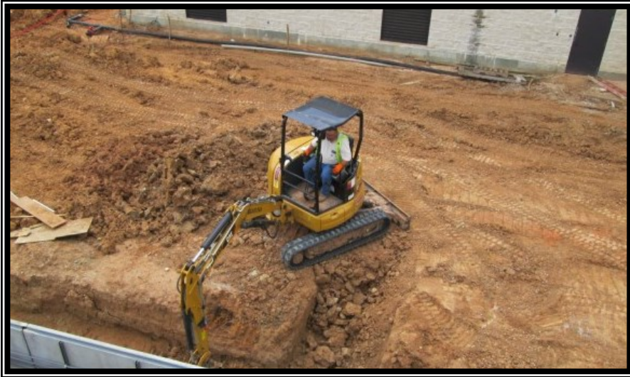
Workers working on the Chemical trench at the Surface Water Treatment Facility
