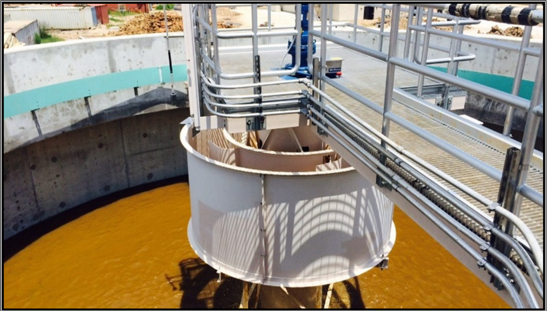
⑤ Sludge Thickeners—Solids received from the Pretreatment Facility for sludge formation
