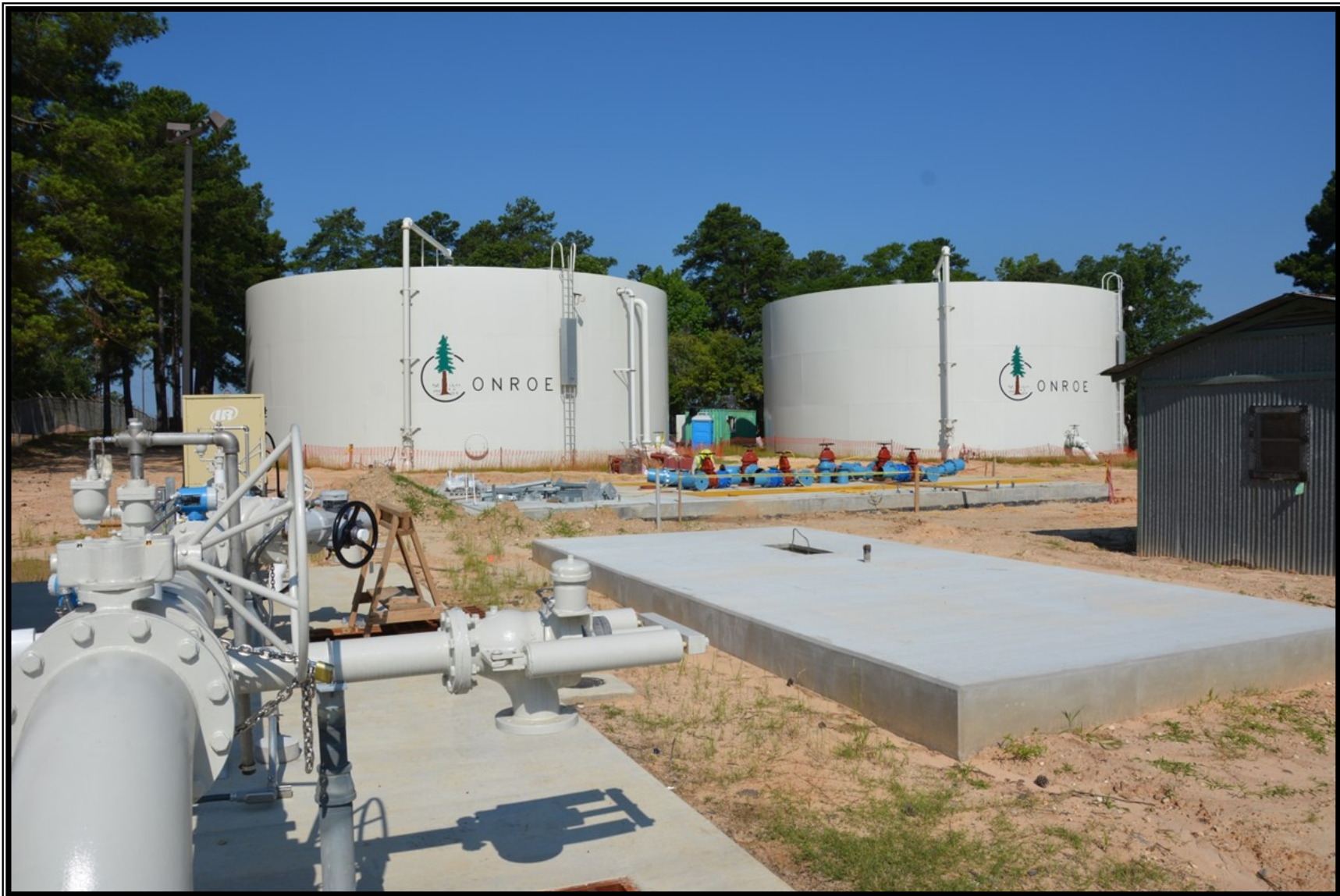
System Improvements—City of Conroe's Water Plant No. 6 (new pump building)
