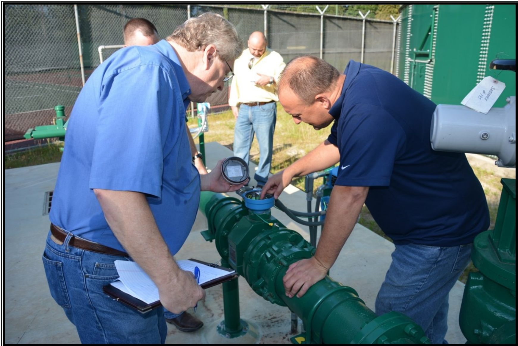
System Improvements—SJRA staff assisting with check-out at Rayford Road MUD's Water Plant No. 1
