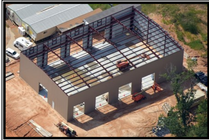
Erected walls at the Maintenance Building
