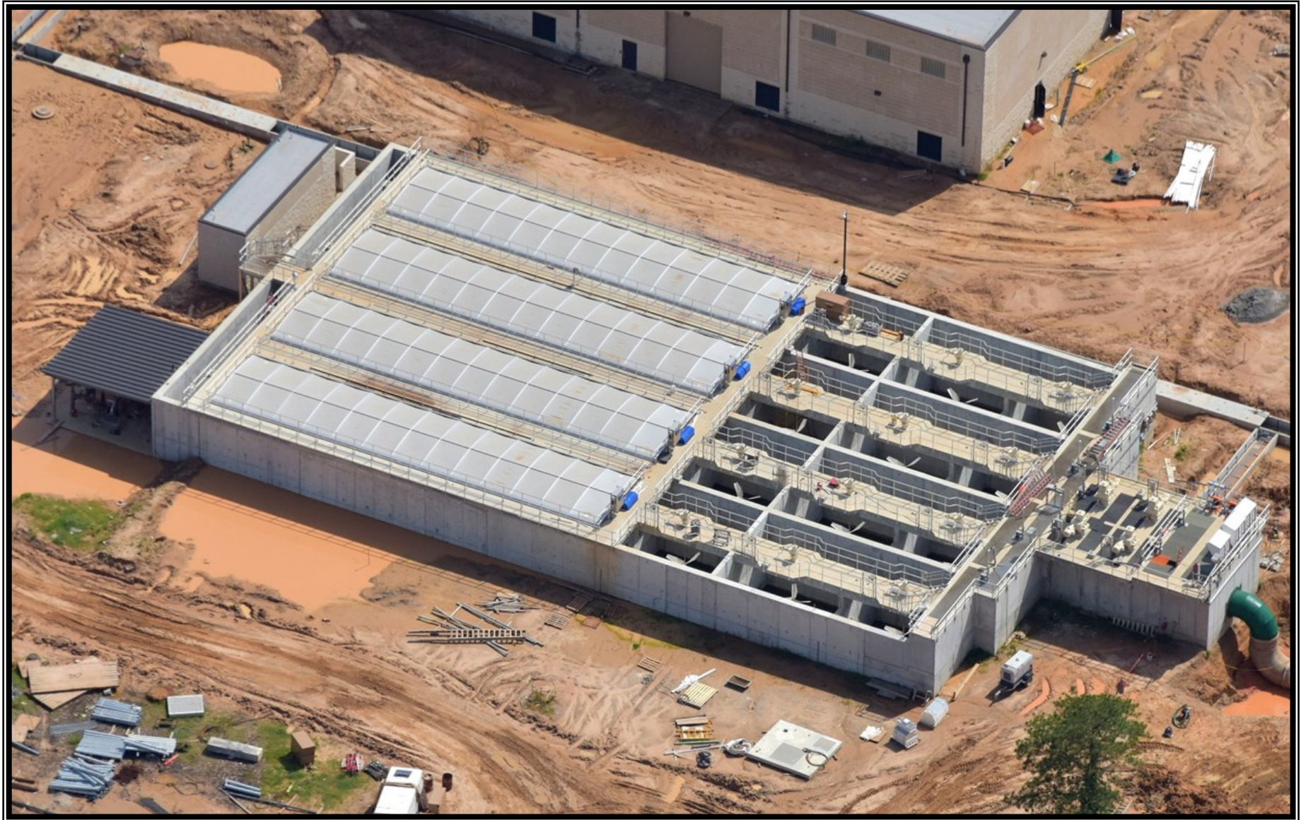
③ Pretreatment Facility—Covers installed over the suspended solids plate settlers
