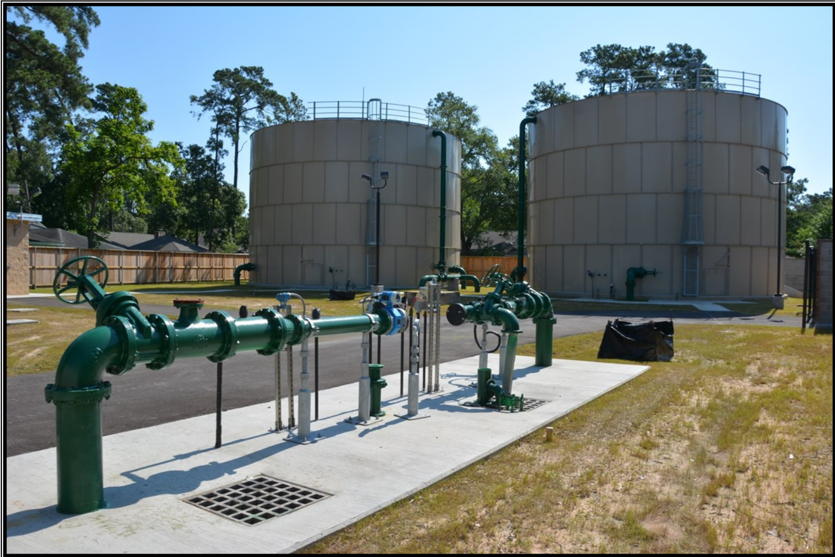
System Improvements - City of Oak Ridge North's Water Plant
