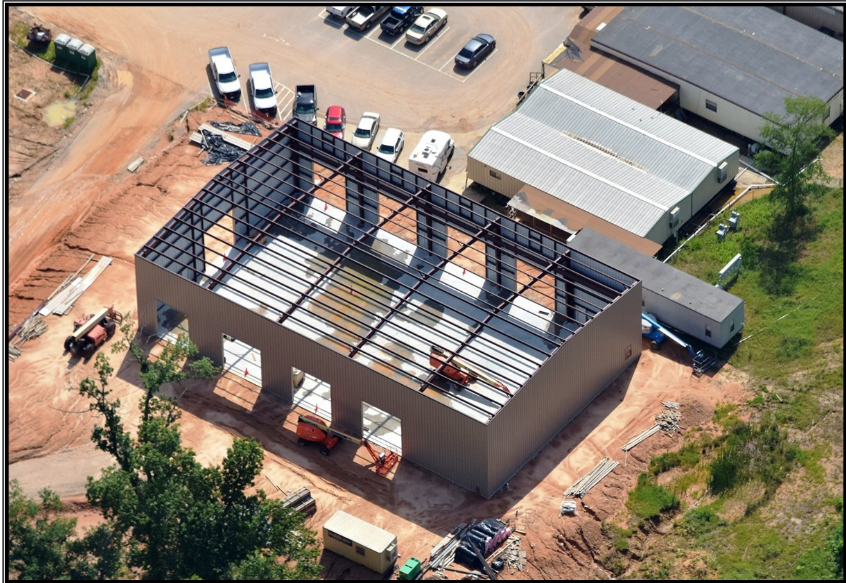
① Maintenance Building — Installation of exterior metal wall panels
