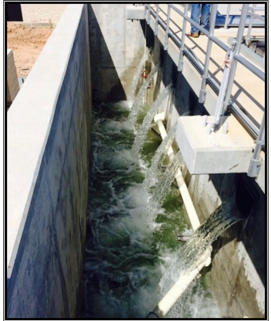
③ Pretreatment Facility—Raw water flowing through the Pretreatment Basin
