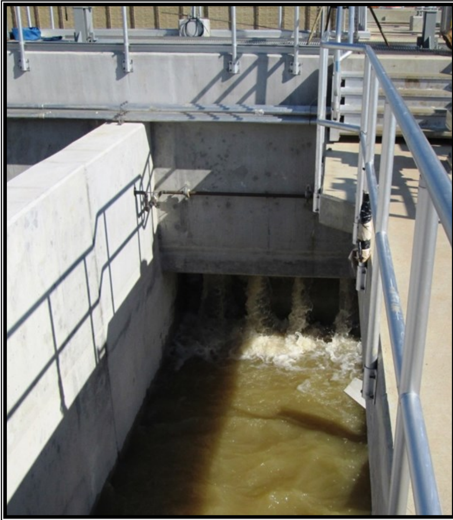
③ Pretreatment Facility—Raw water flowing through the Pretreatment Basin
