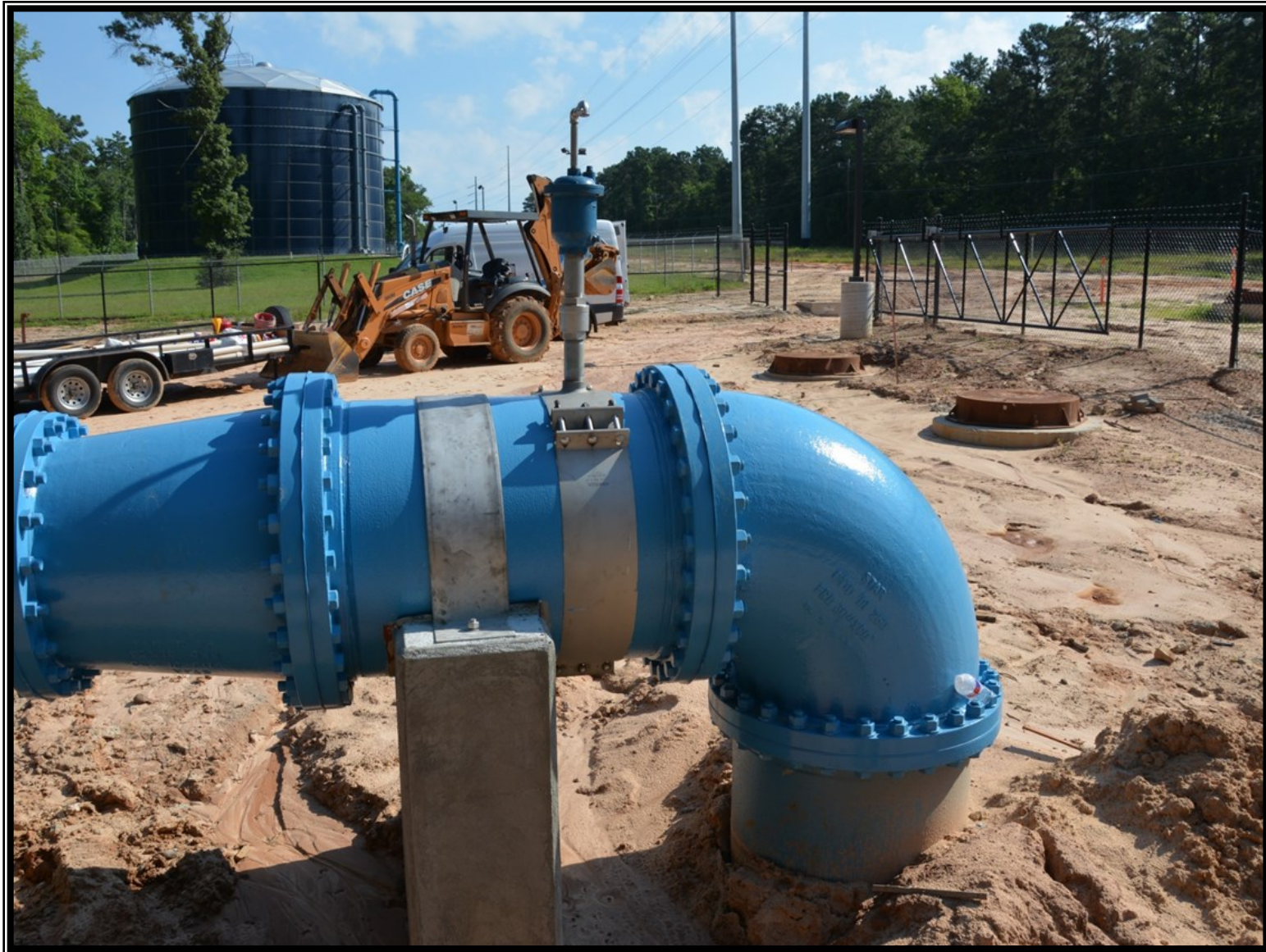
① Standpipe yard piping complete; only site paving remains
