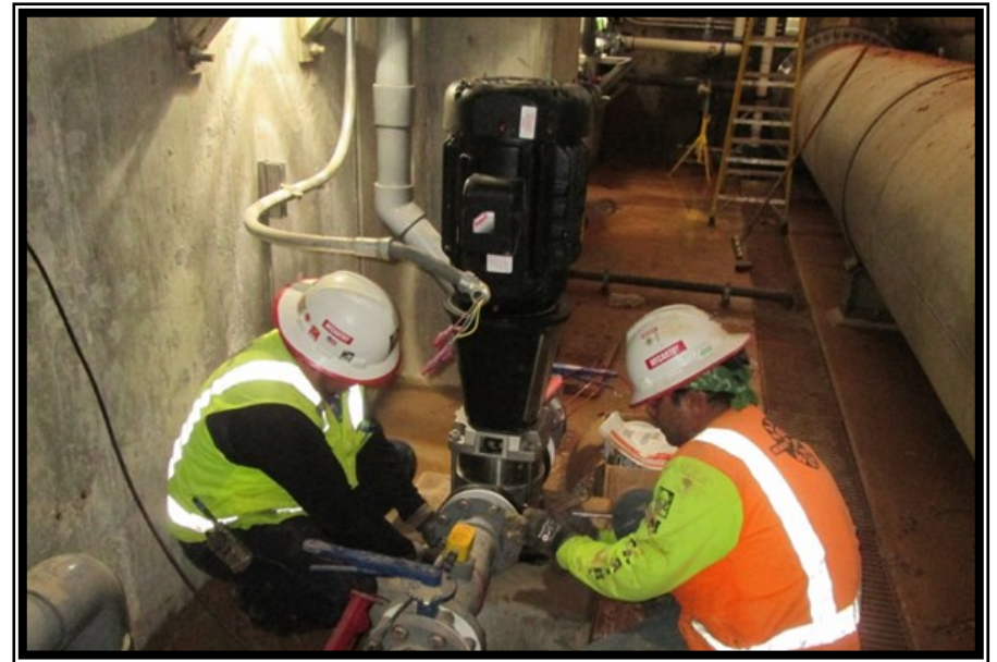
Workers processing mechanical piping at the Granular Activated Carbon (GAC) Building
