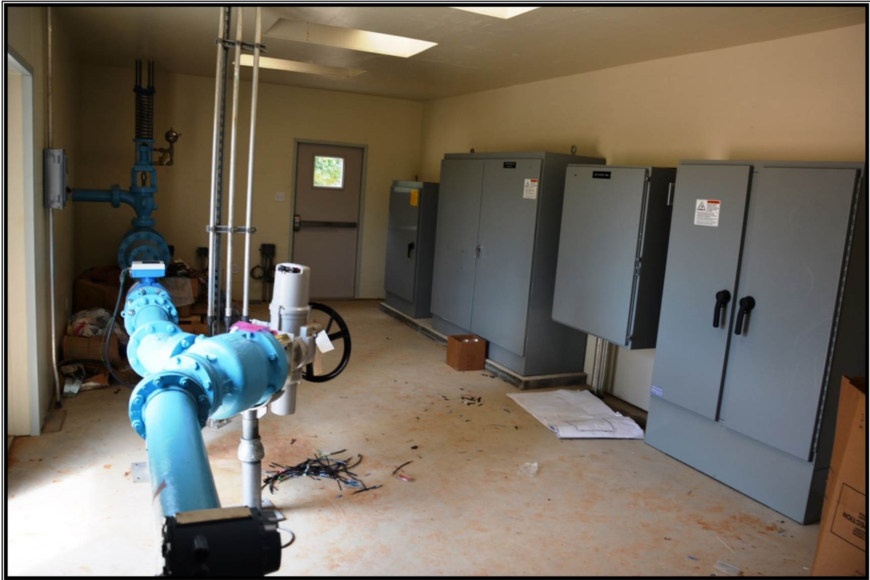
System Improvements—PLC panel and flow control valve completed at Mid South's Water Plant
