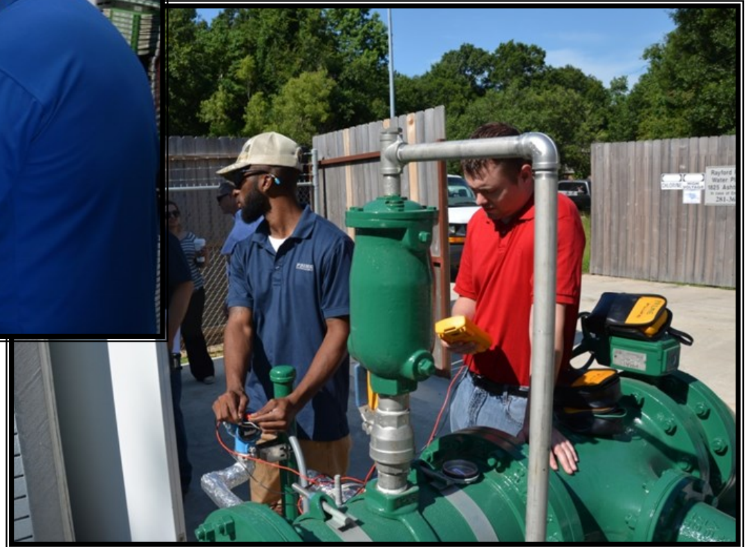
System Improvements—SCADA PLC communication check-out at Rayford Road MUD's Water Plant No. 2
