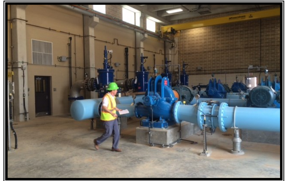
Above—SCADA staff checking out the various systems Left—SCADA staff checking out and troubleshooting the system Bottom—Risk Management Fund representative appraising facilities for insurance purposes
