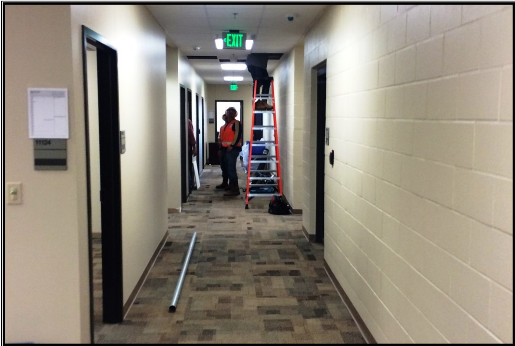
SJRA staff installing fiber optic cable conduit in the GRP Operations Building
