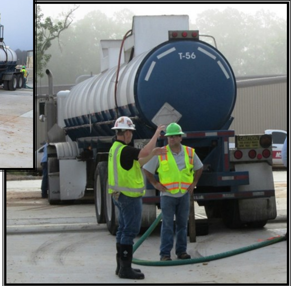
② Chemical System — The first chemical delivery (Aluminum Chlorohydrate)
