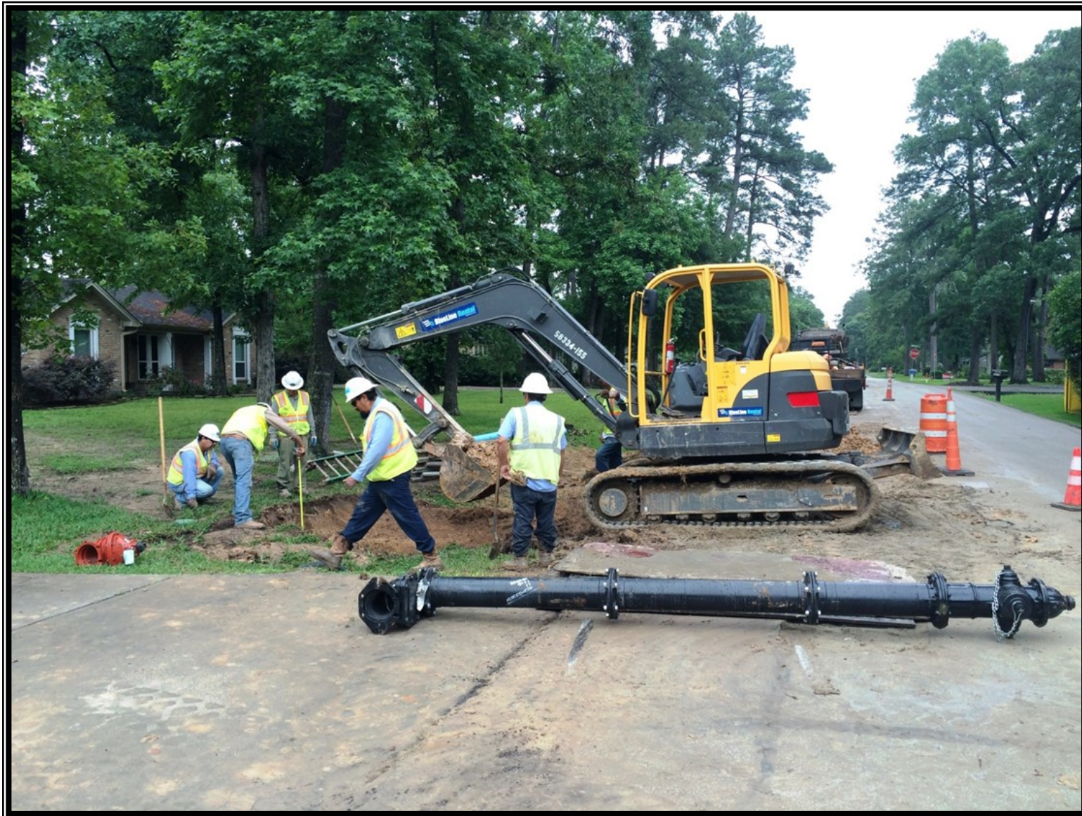
① Installation of flushing hydrant adjacent to 16-inch waterline along Maplewood Drive
