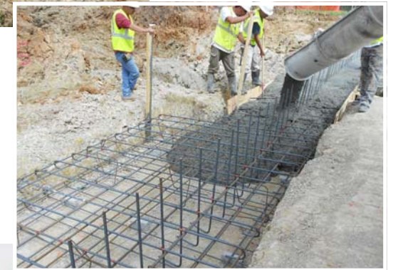
GRP Building No. 1 construction
