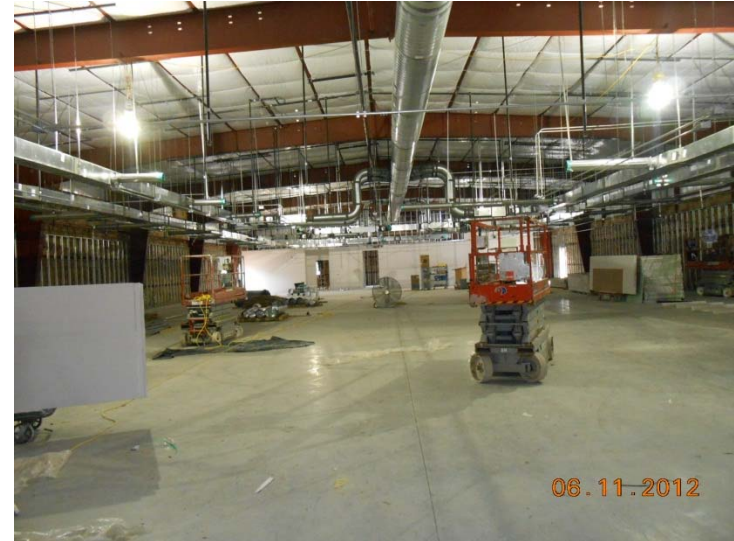
June 11, 2012 – GRP Building No. 1 Interior
