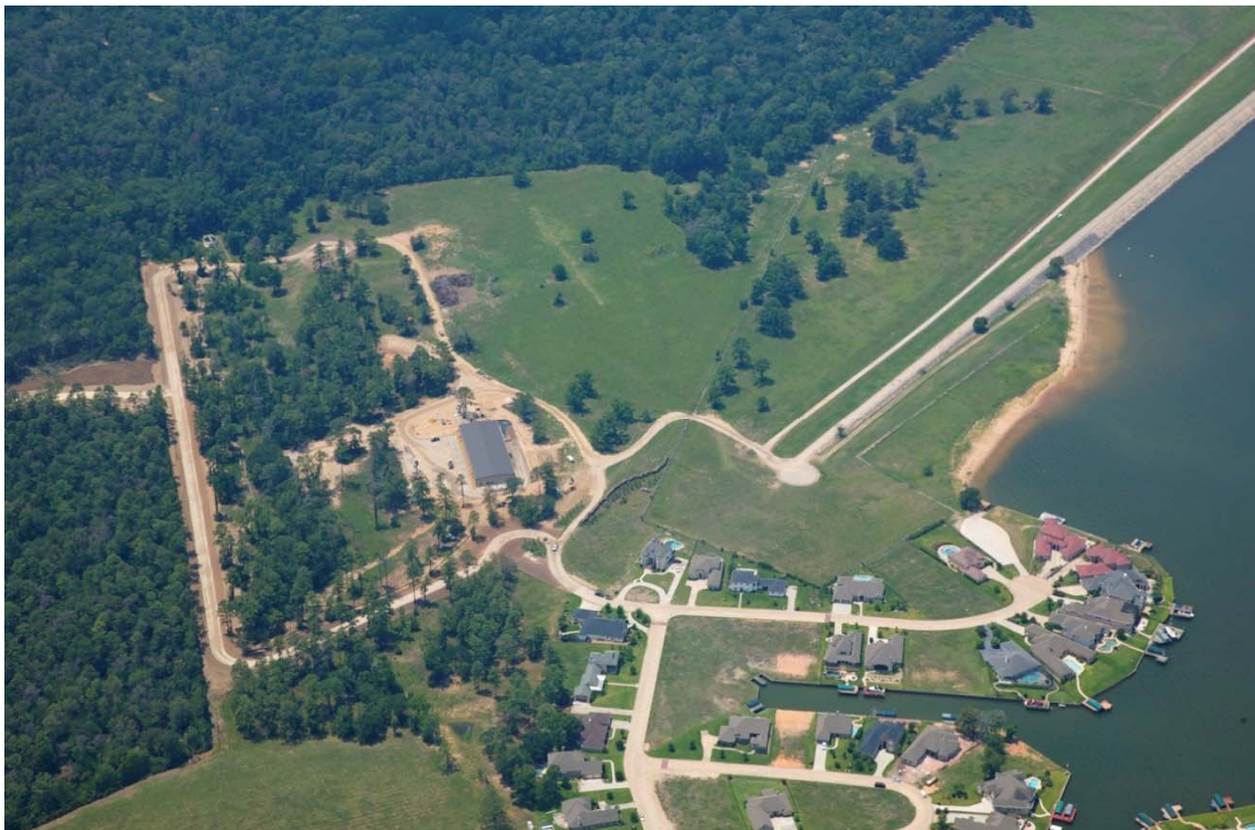
Surface Water Facility Site
