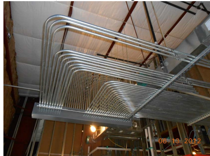
June 13, 2012 – GRP Building No. 1 Electrical Conduit
