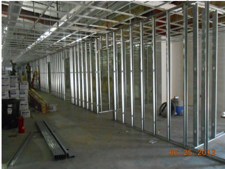
June 25, 2012 – GRP Building No. 1 Interior Walls Framed
