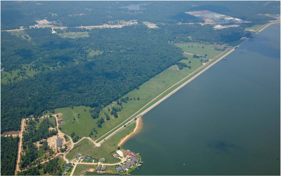
Surface Water Facility Site
