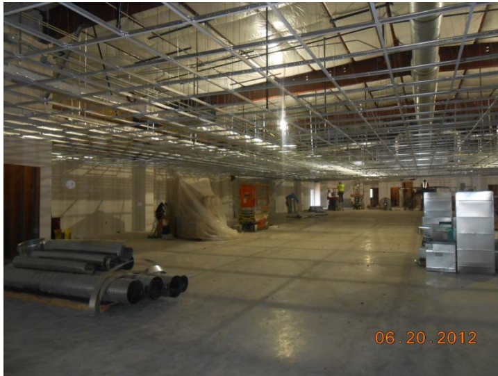
June 20, 2012 – GRP Building No. 1 Ceiling Grid
