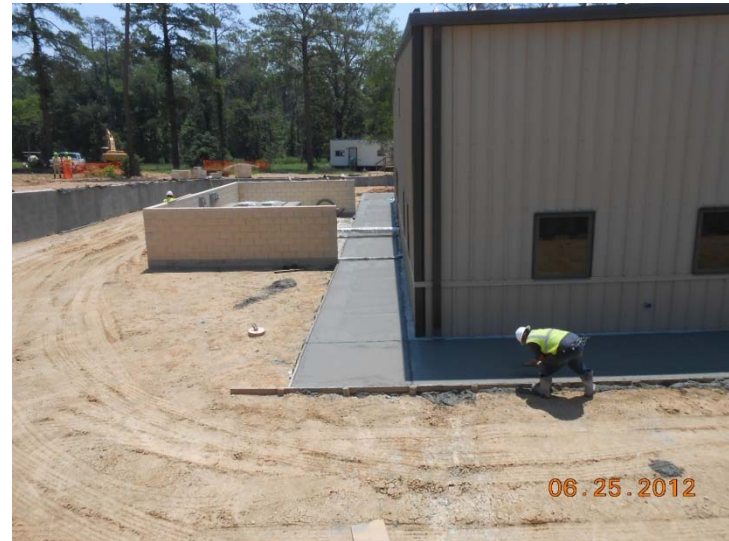
June 25, 2012 – GRP Building No. 1 Sidewalk Pour
