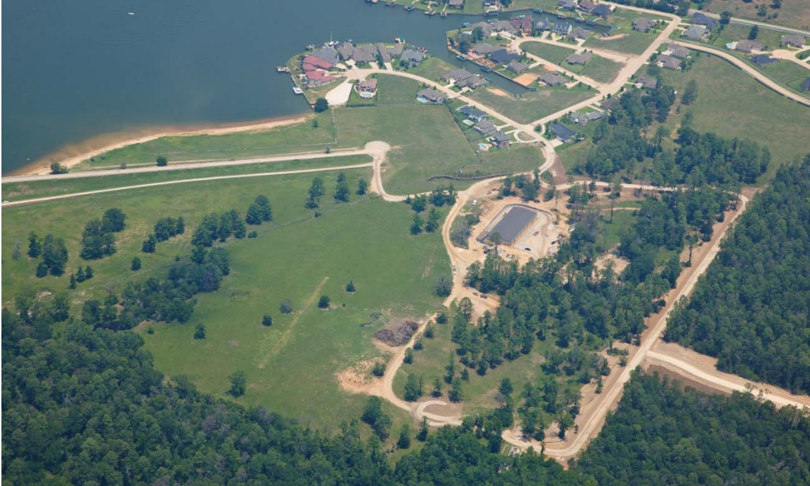
Surface Water Facility Site
