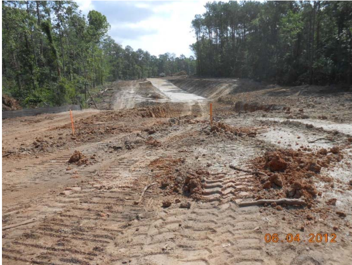
June 4, 2012 – SWF Access Road Construction
