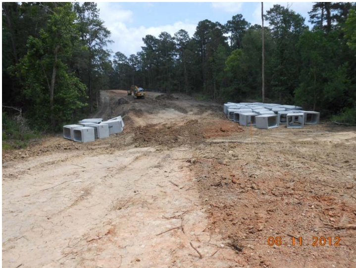
June 11, 2012 – SWF Access Road Construction
