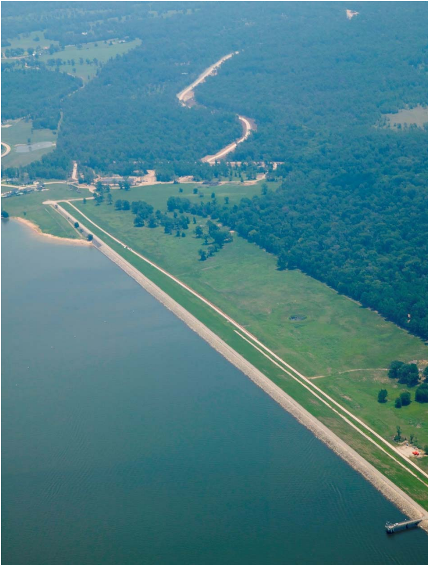
Surface Water Facility Site
