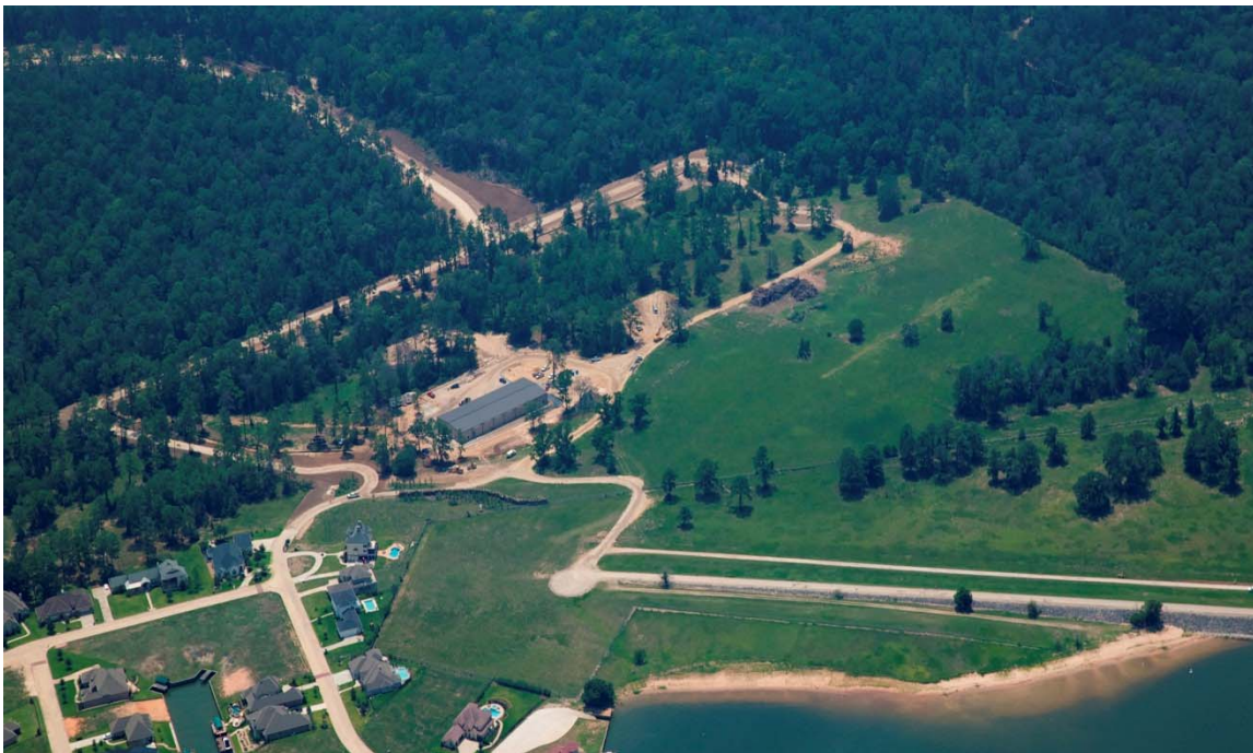
Surface Water Facility Site
