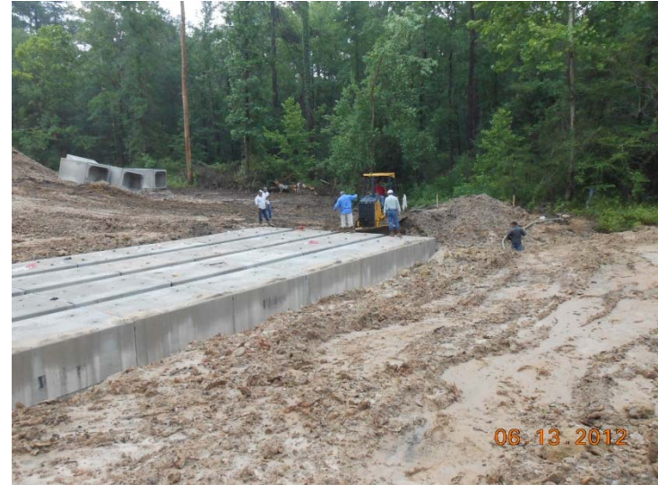
June 13, 2012 – SWF Access Road Construction
