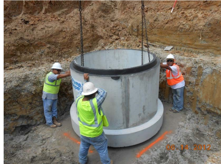
June 14, 2012 – Aligning New Lift Station Wet Well
