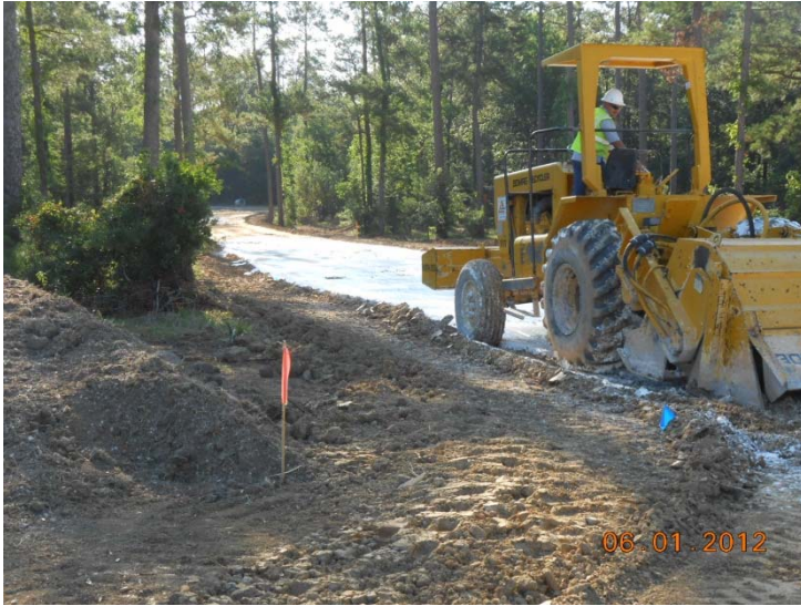
June 1, 2012 – AquaTexas Sanitary Sewer/Road Relocation
