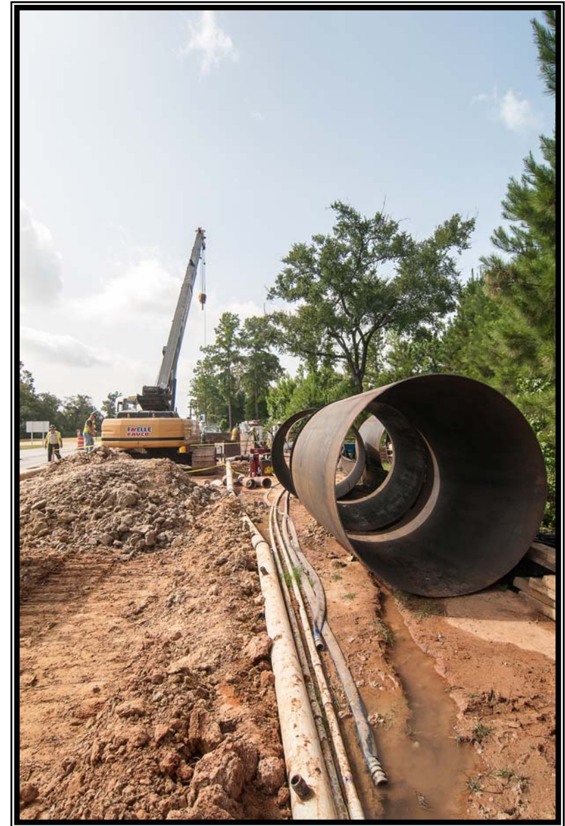
Segment T2 - Construction Along Fish Creek at Mulligan Drive
