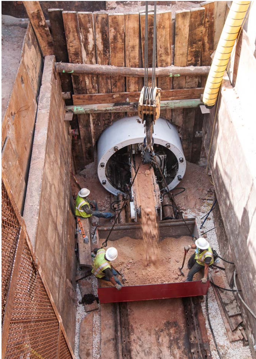
② Excavated Material Removed by Conveyor Belt
