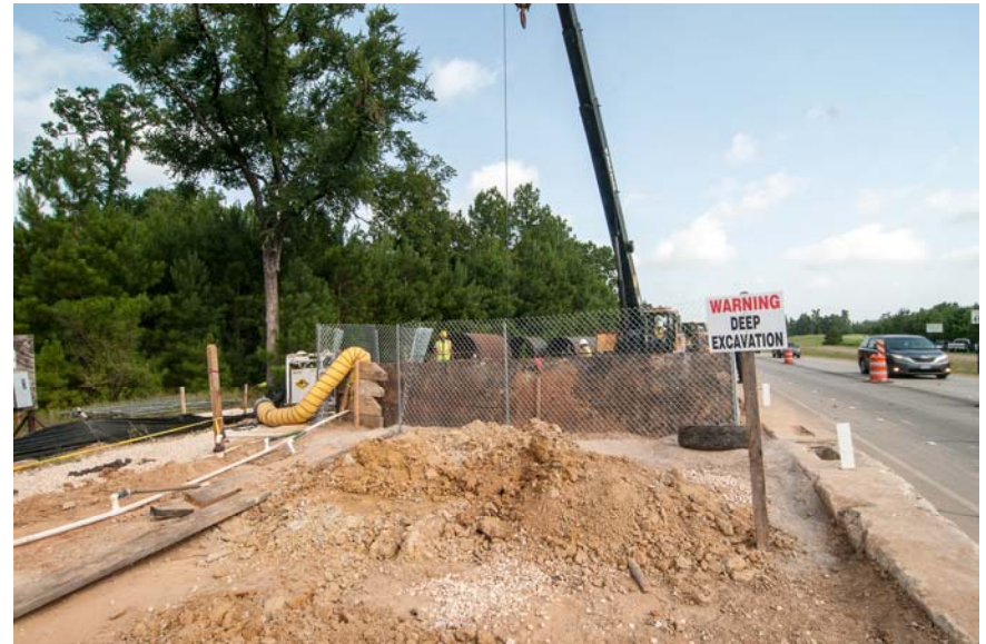
9 Tunnel Shaft for Segment T2 - Fish Creek at Mulligan Drive
