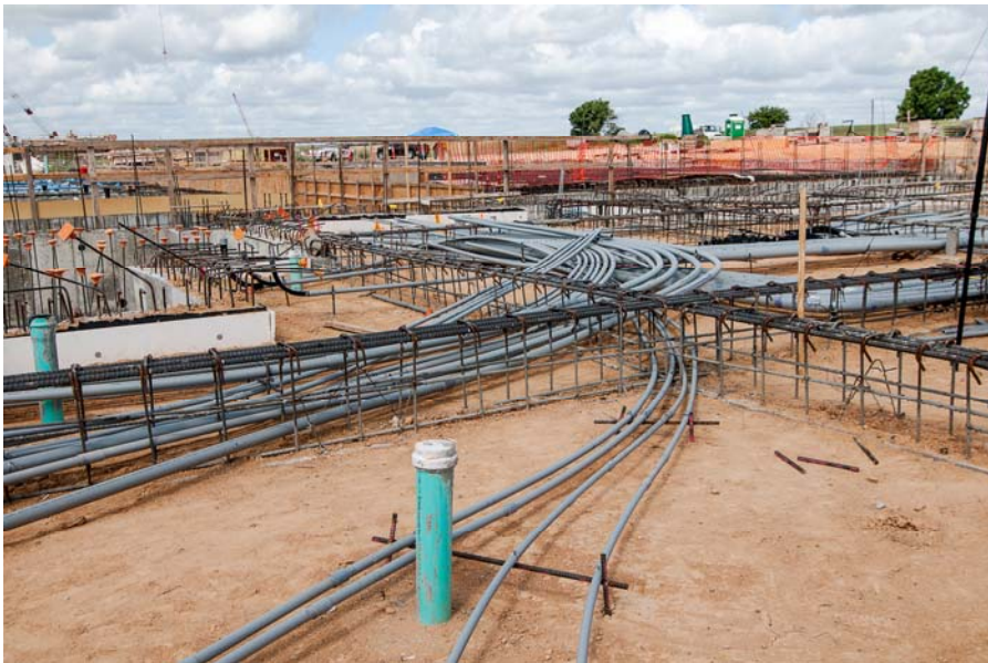
10 11 12 13 Backfilling and Electrical Conduit Installation at Membrane Facilities
