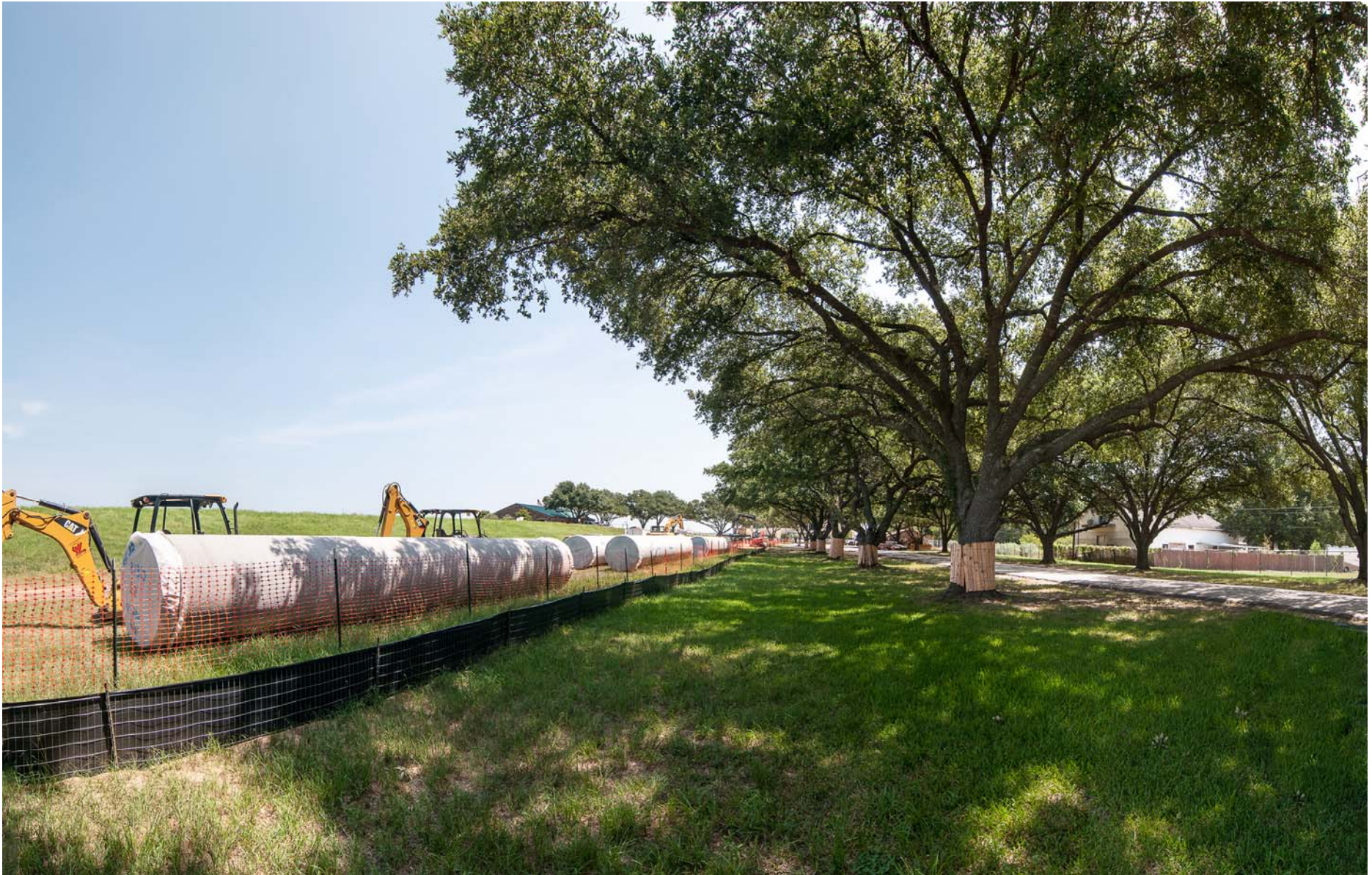
⑤ Segment T1 - Entrance at Dam Site Road
