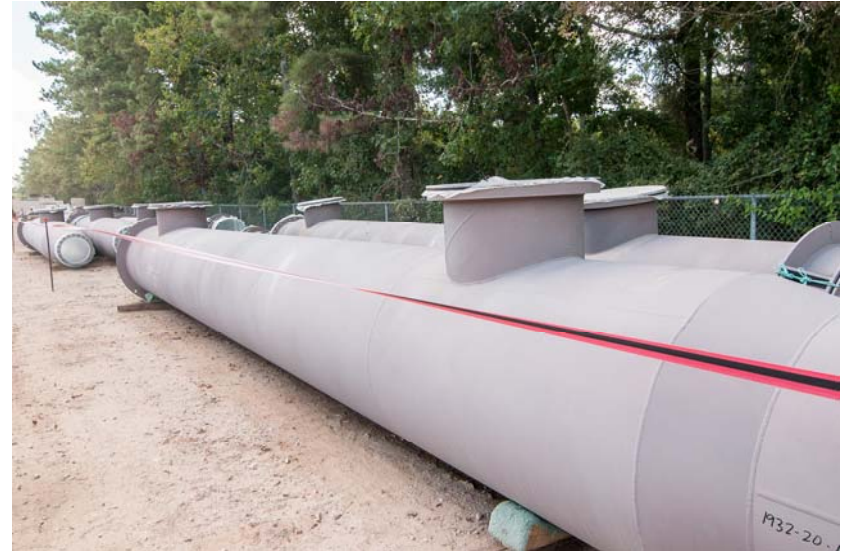
⑧ High Service Pump Station - Manifold Piping On-site
