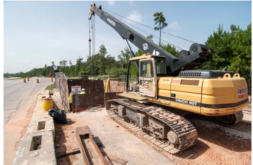
③ Tunnel Boring Machine Access Excavation
