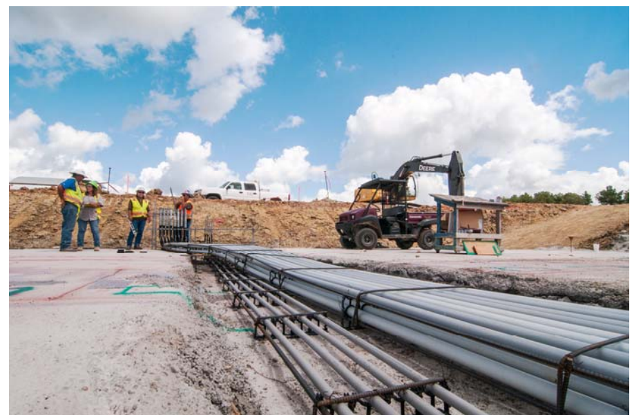
17 Conduit Installation at Electrical Switchgear Building
