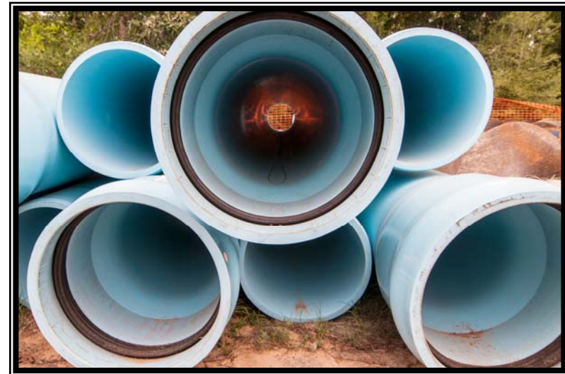
Below: PVC Pipe Used at Research and Kuykendahl (Segment W2B)
