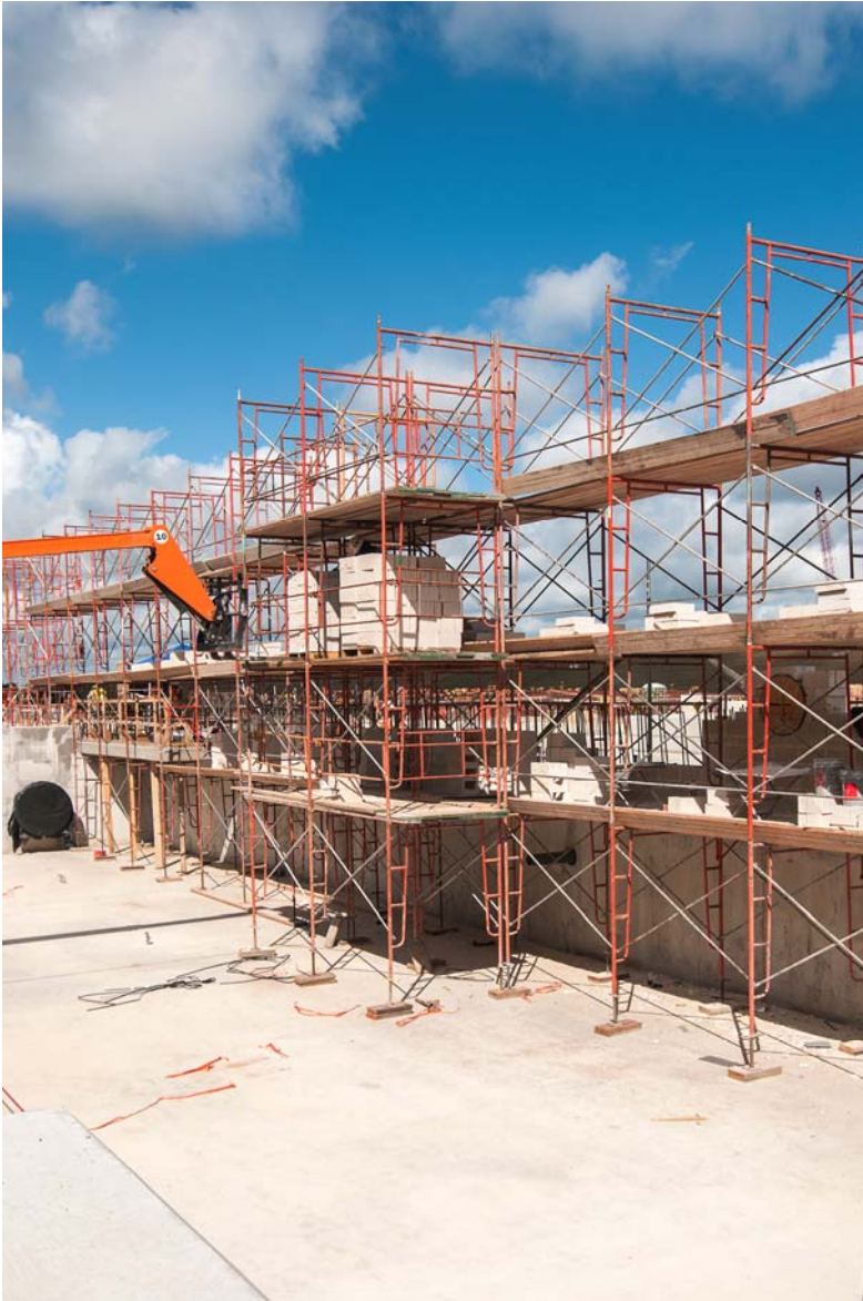
⑦ High Service Pump Station - Scaffolding for Masonry Work
