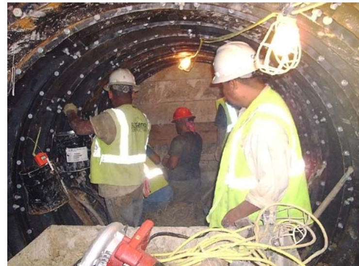
9 Segment T1 Tunnel Under Highway 105
