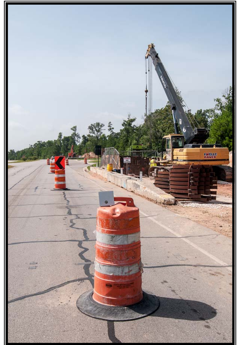
Segment T2 - Construction Along Fish Creek
