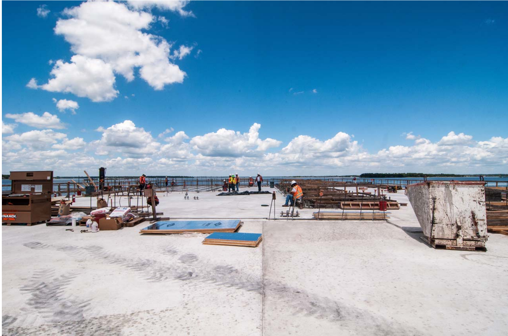
② Raw Water Pump Station - Future Pump Building Location
