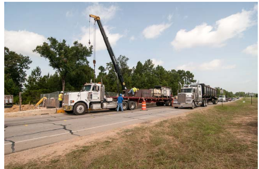
④ Construction Equipment Unloaded at Fish Creek and Mulligan Drive
