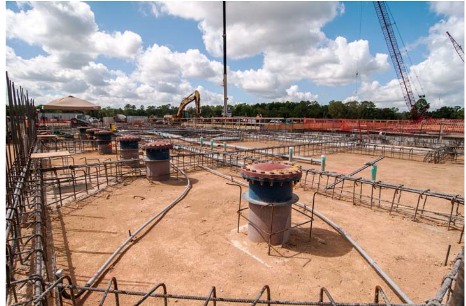
10 11 12 13 Backfilling and Electrical Conduit Installation at Membrane Facilities
