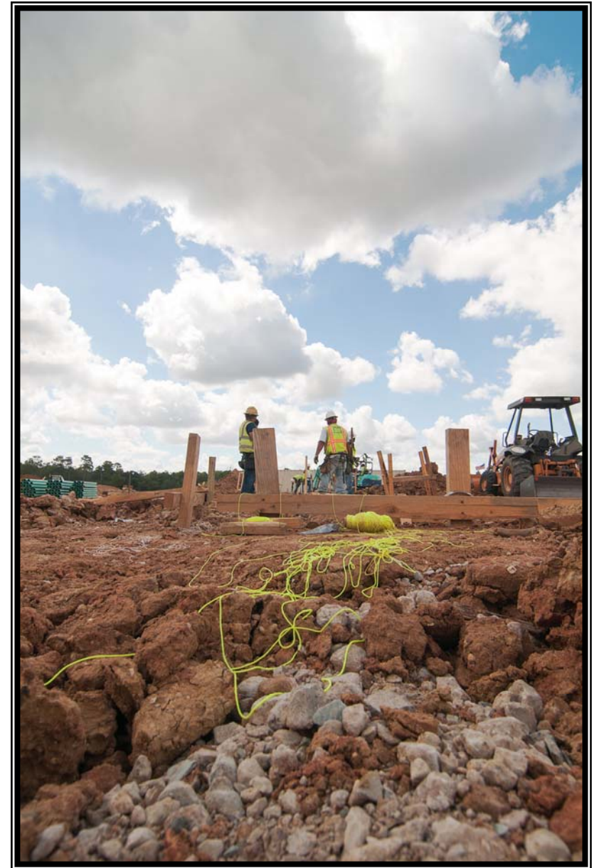
Surface Water Facilities - Construction at Warehouse
