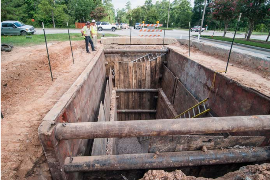
① ② ③ Segment W1B Installation of Tunnel Shaft for Boring Under Crownridge at Research Forest
