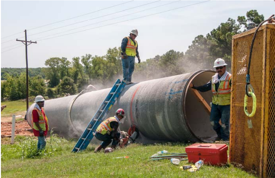
② Segment T1 Workers Cut a Section of 60-inch Pipe
