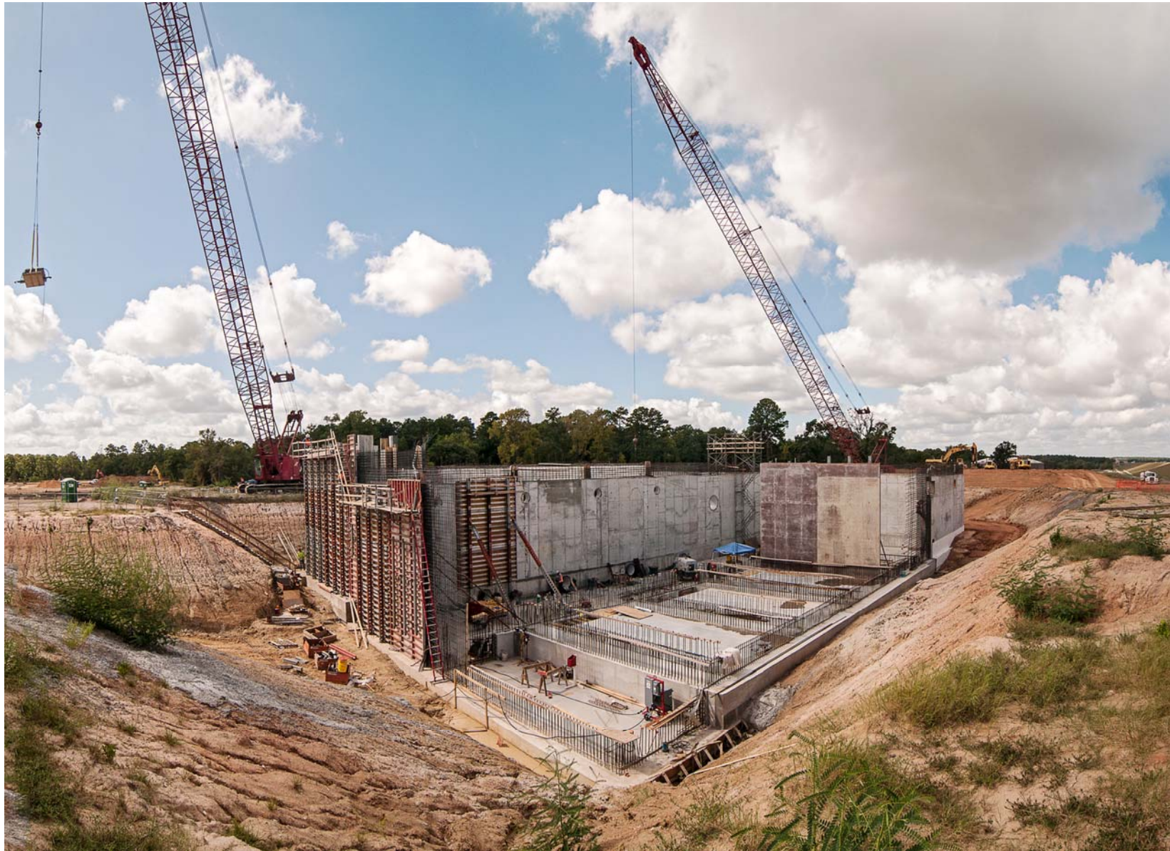
⑥ GAC Facility - Basin Walls Under Construction
