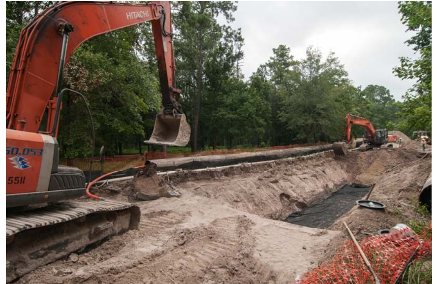
⑤ Segment W1B Future Kuykendahl 16-inch and 20-inch Waterline Crossing
