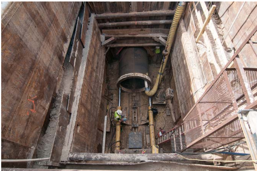
10 Installation of Liner Pipe for Segment T2 - Fish Creek at Mulligan Drive
