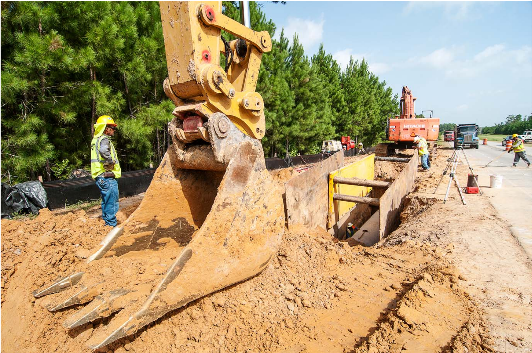
⑤ 60-inch Pipe Installed by Open Cut Construction Along Fish Creek Thoroughfare
