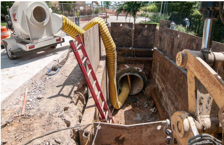
④ Segment T1 Tunnel Access at G&A Building
