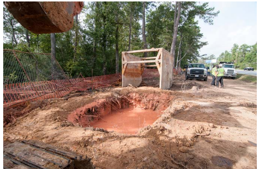
① ② ③ ④ Segment W1A Along FM 2978 - Trenchless Construction of 16-inch Waterline
