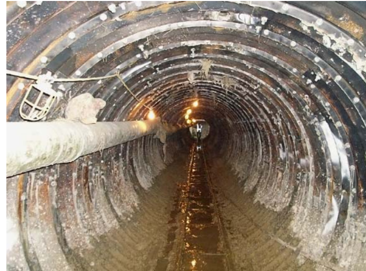
8 Segment T1 Tunnel Under Highway 105
