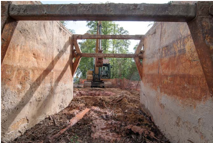
① ② ③ ④ Segment W1A Along FM 2978 - Trenchless Construction of 16-inch Waterline
