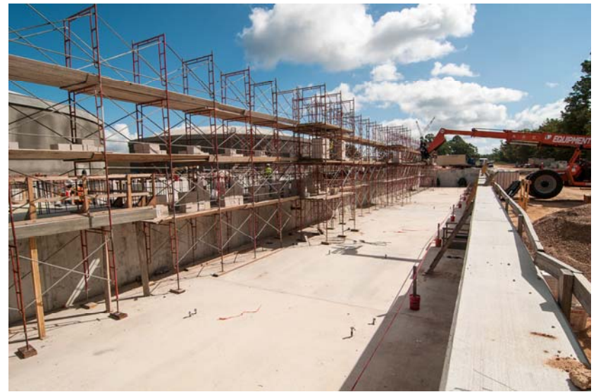
⑨ High Service Pump Station Discharge Bay
