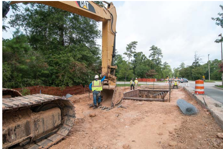
① ② ③ Segment W1B Installation of Tunnel Shaft for Boring Under Crownridge at Research Forest
