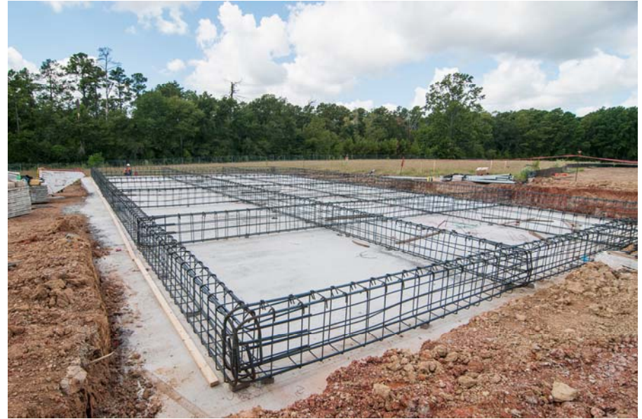
15 Installation of the Generator Building Begins
