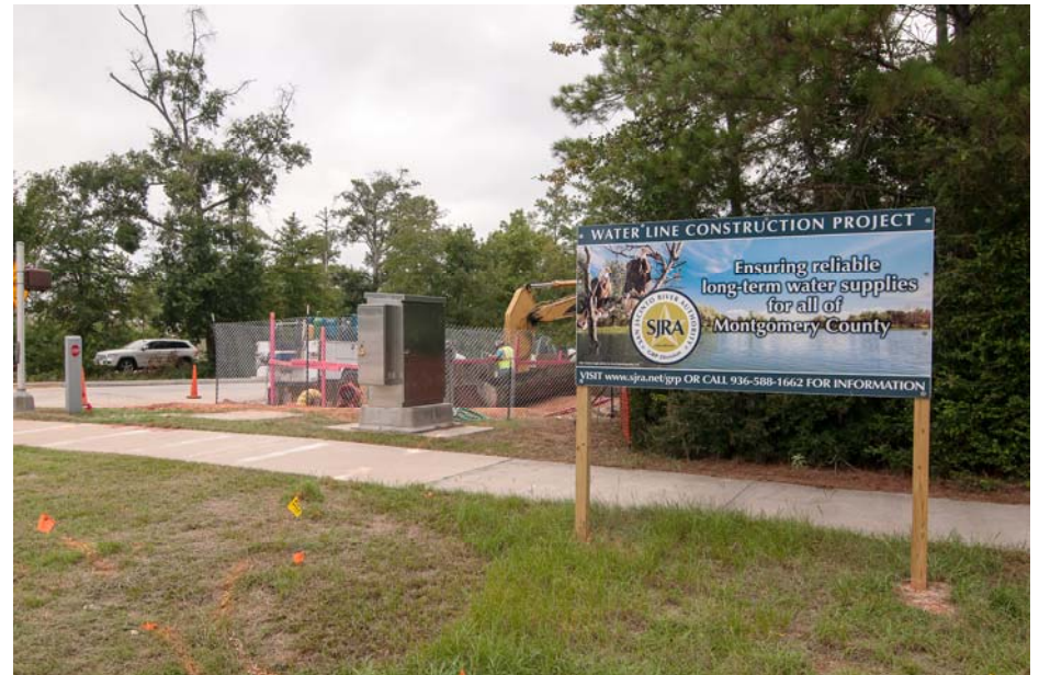
SJRA Project Sign - Located at Construction Sites
