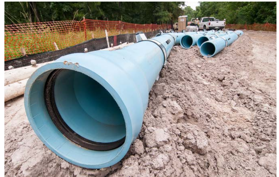
⑥ Segment W1B - 20-inch PVC Pipe Fitted with Spacers for Installation in Casing Pipe
