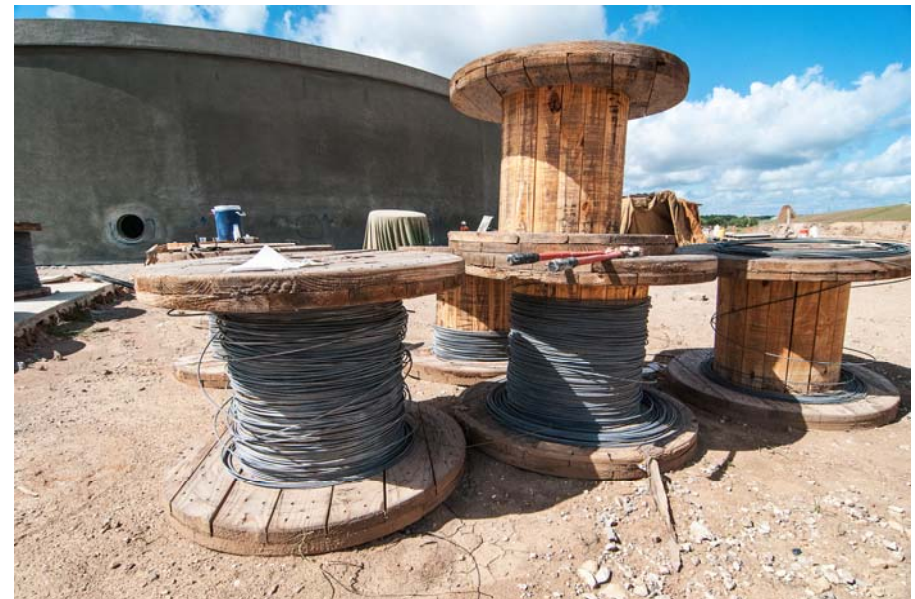
③ ④ ⑤ Inside GST No. 2, Wire Wrapping GST No. 1, and Spools of Wire Used in Wrapping Process
