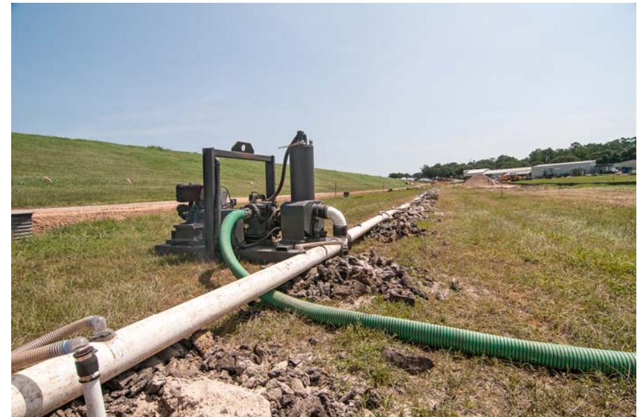
⑥ Segment T1 Dewatering Operation
