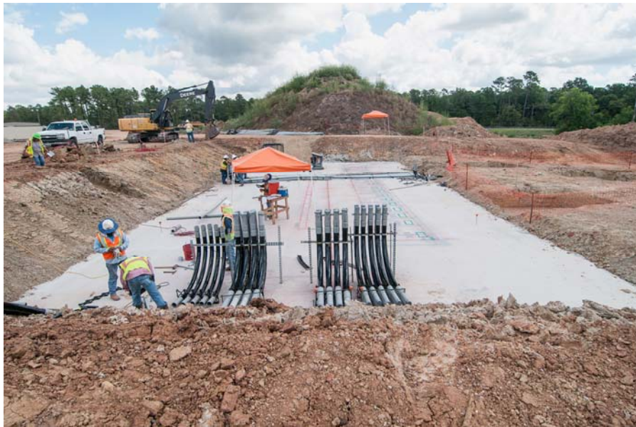
16 Switchgear Building Pad
