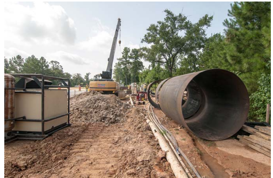
11 Liner Pipe for Segment T2 - Fish Creek at Mulligan Drive
