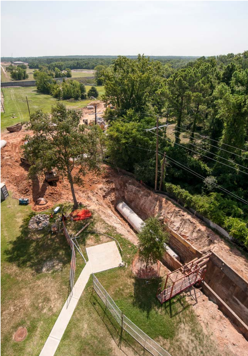
1 Segment T1 from G&A Building
