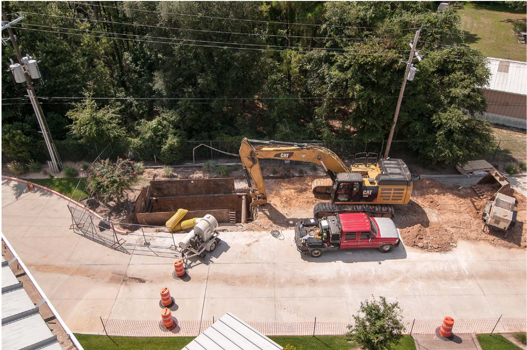
① Segment T1 Pipe Installation at G&A Building
