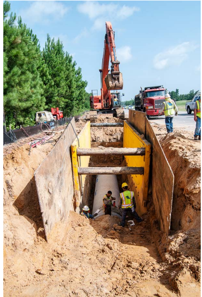
⑥ ⑦ 60-inch Pipe Installation Along Fish Creek Thoroughfare
