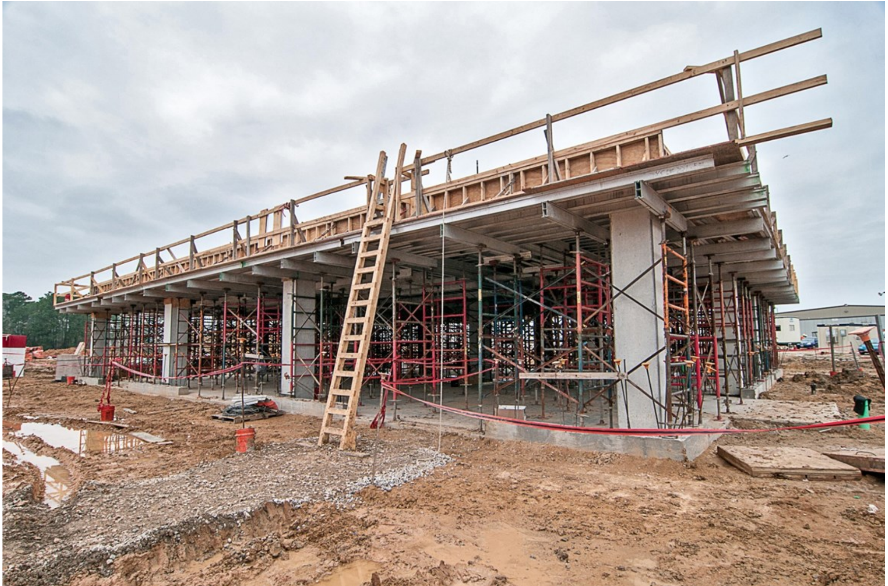
9 Second floor deck installation at Dewatering Building
