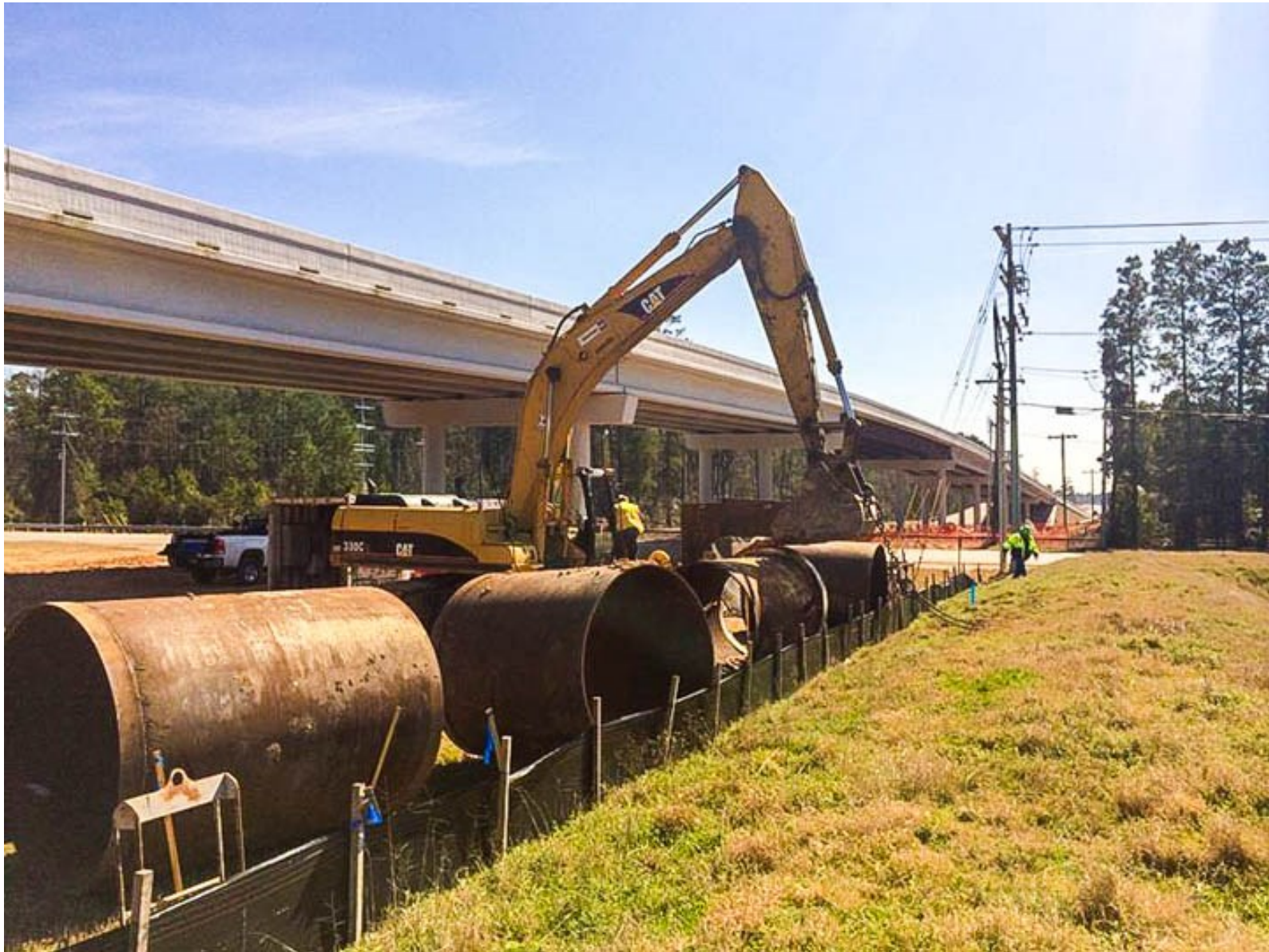
① Segment T2 - Tunnel operation for FM 2854 and BNSF Railroad crossing
