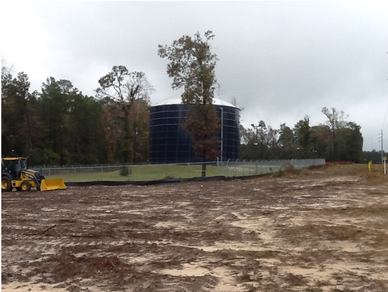
① Cleared Standpipe site adjacent to Conroe Water Plant No. 21
