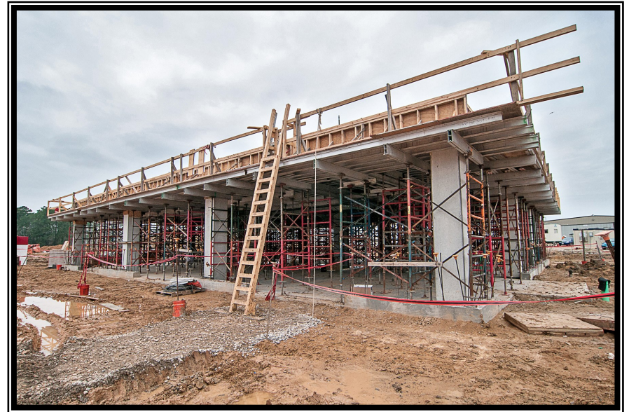
Above: Belt Press Building at Surface Water Facilities
