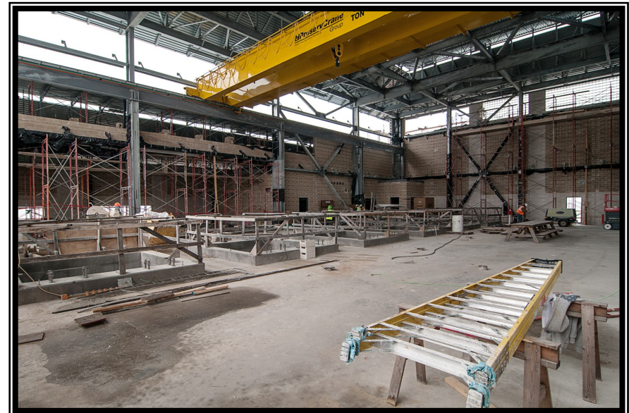
Below: Inside view of Intake Pump Station at Surface Water Facilities
