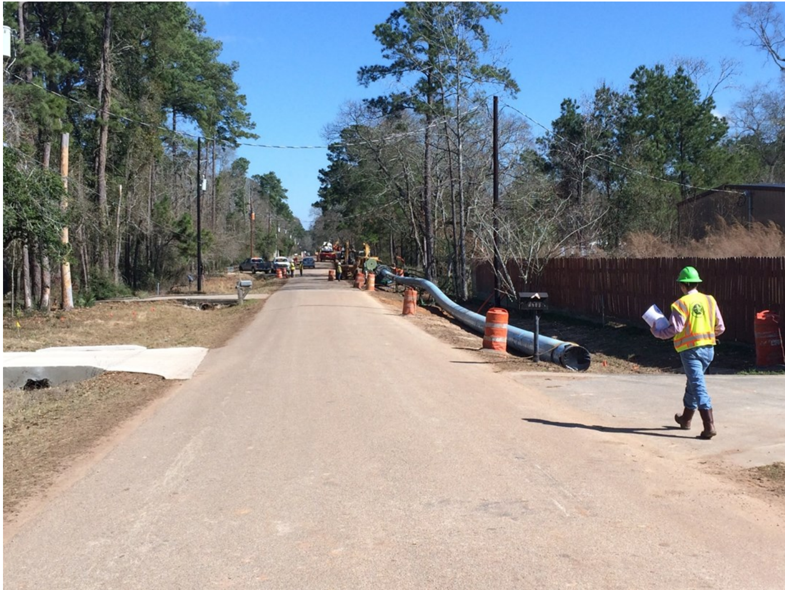
① Segment W4 - Pipe fusing operation along Southline Road
