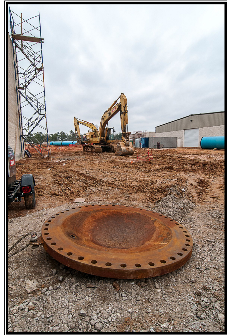
Construction materials outside of the Membrane Building at Surface Water Facilities
