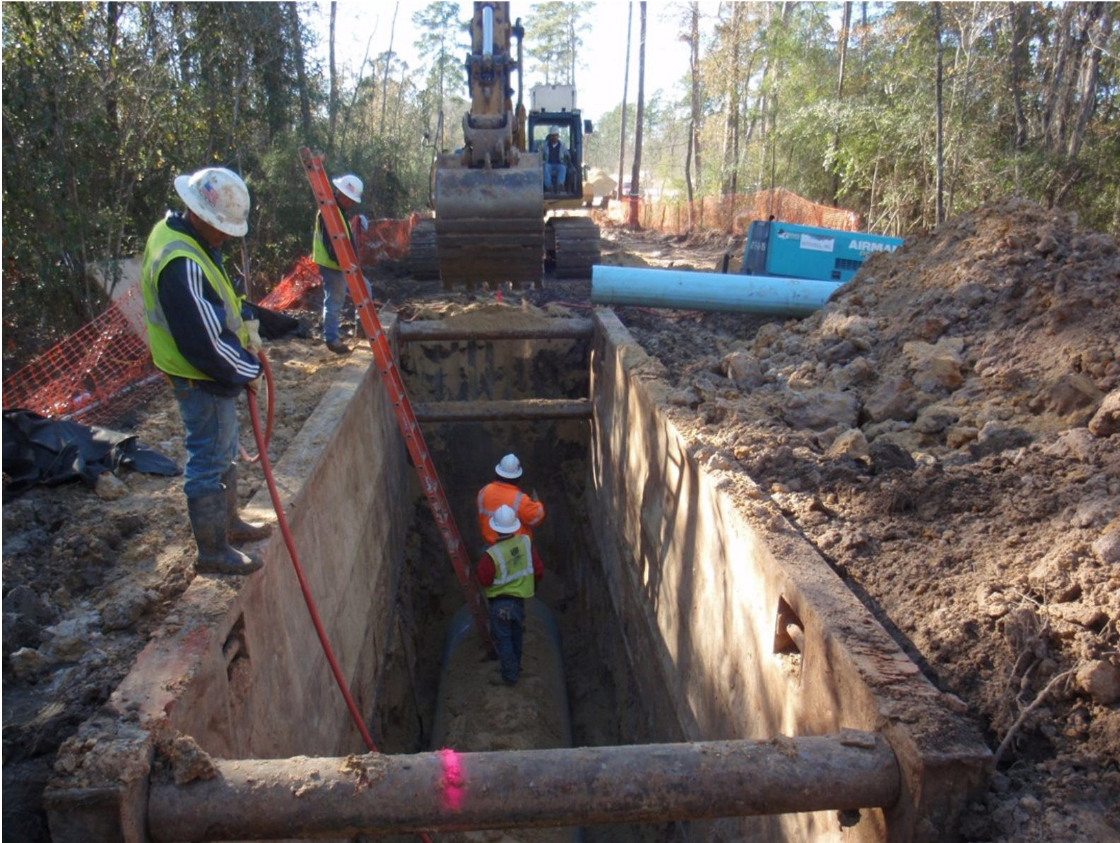
① Segment W1A—48-inch pipe installation along future Research Forest Drive
