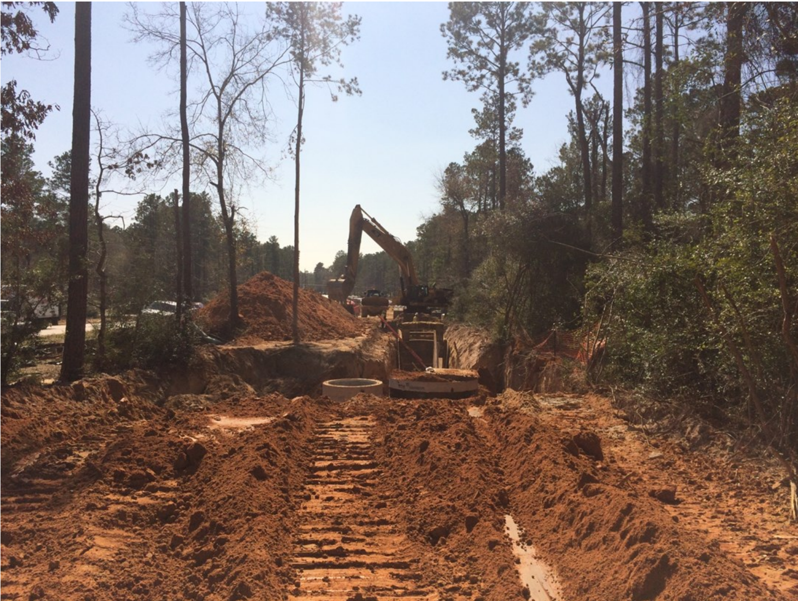
① Segment T3—54-inch pipe installation along Fish Creek Thoroughfare
