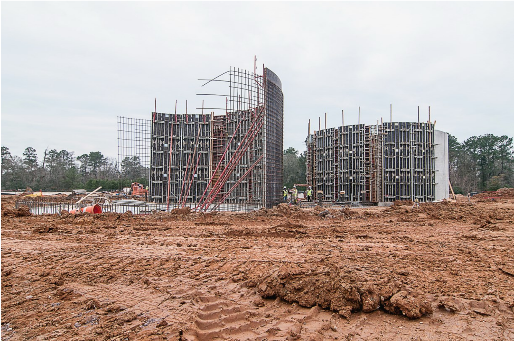
⑩ Wall construction of thickeners
