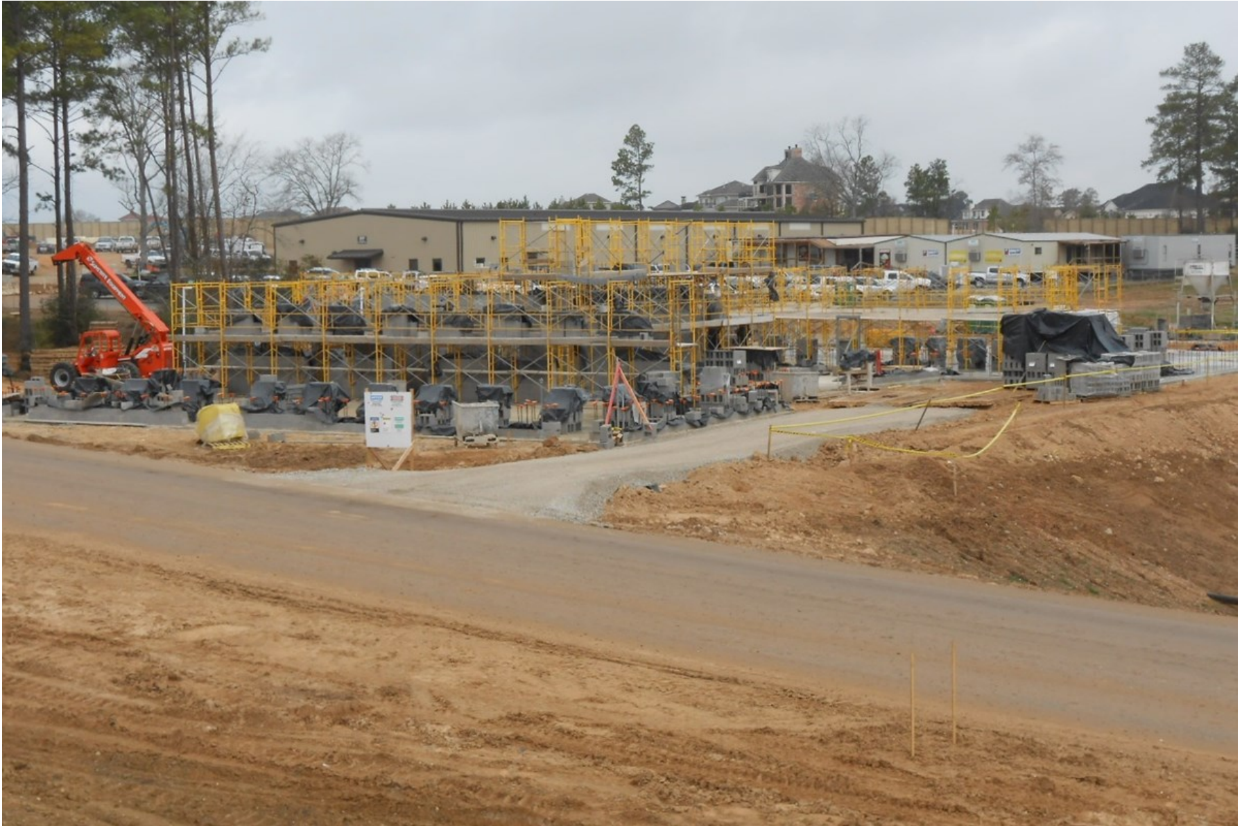
12 Masonry installation at Operations Building
