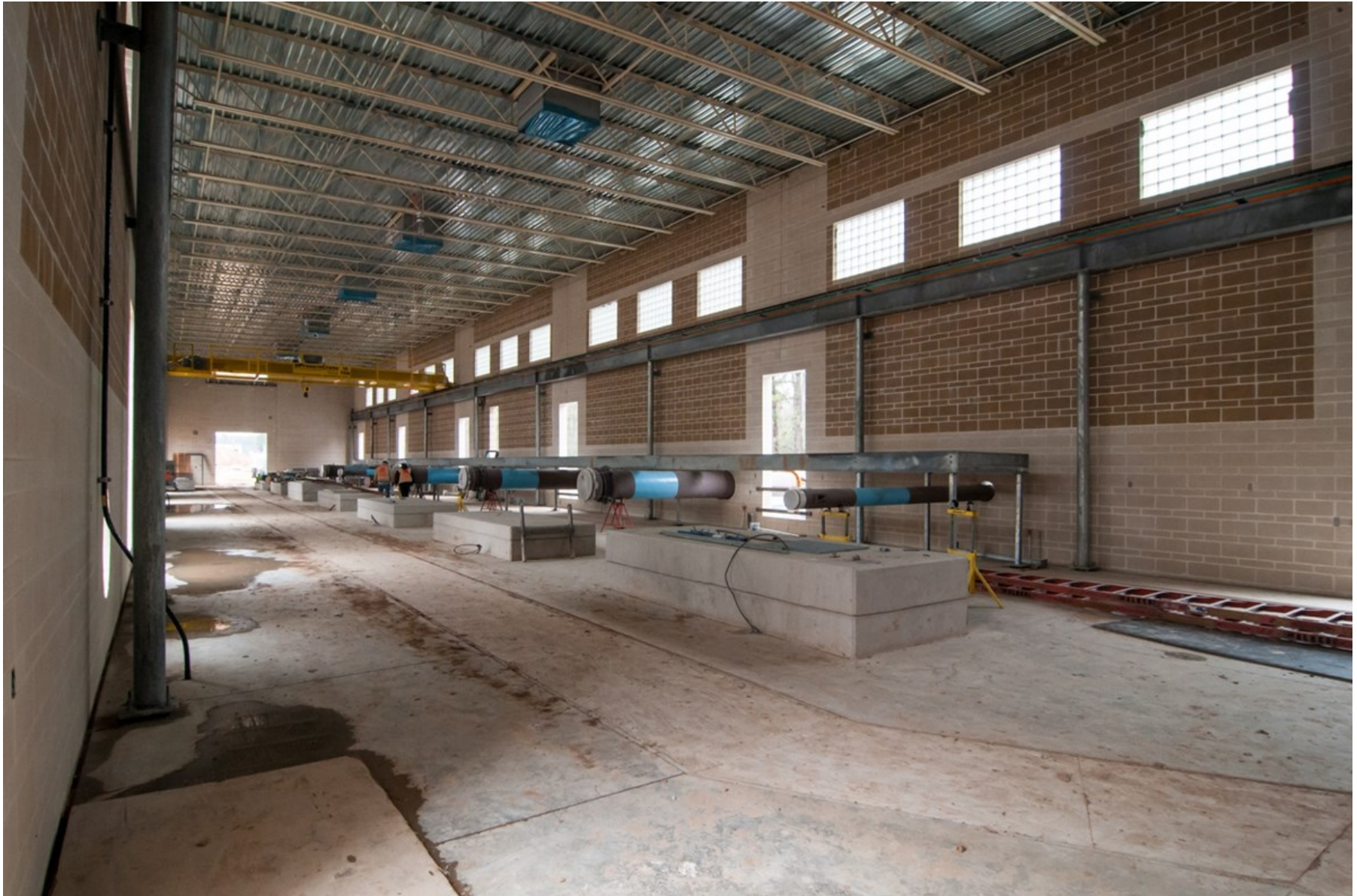
⑤ Pump room at High Service Pump Station
