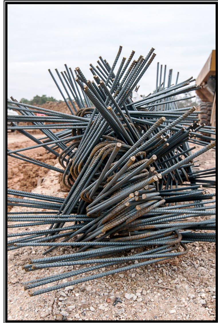
Intertwined rebar at Surface Water Facilities
