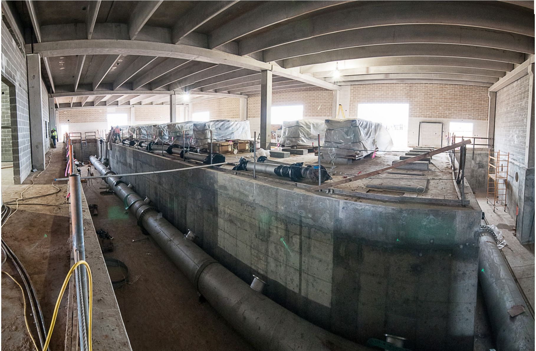
③ Interior pipe trench at Membrane Building
