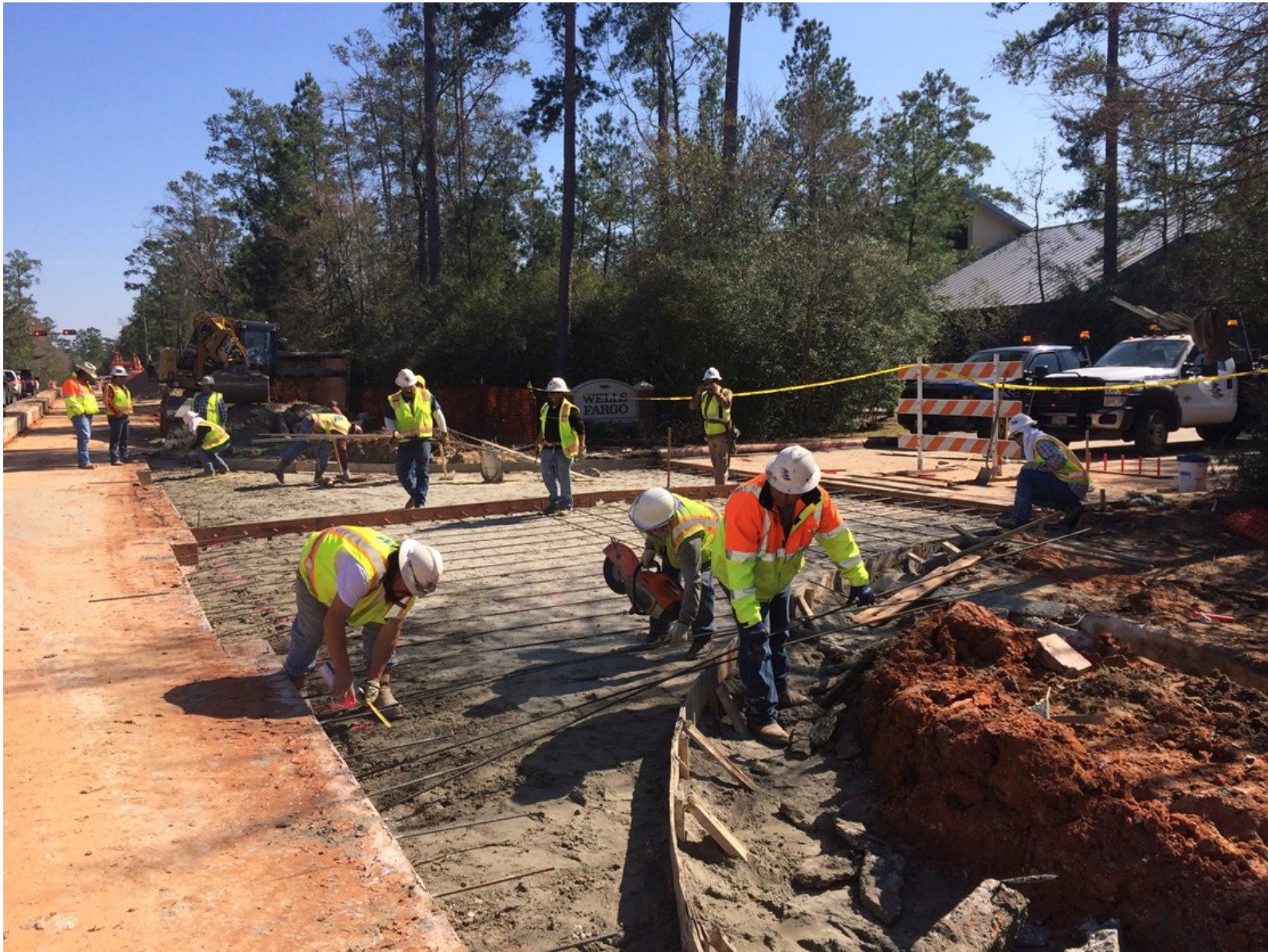
① Segment W1B - Concrete pavement replacement along Research Forest Drive near Kuykendahl Road
