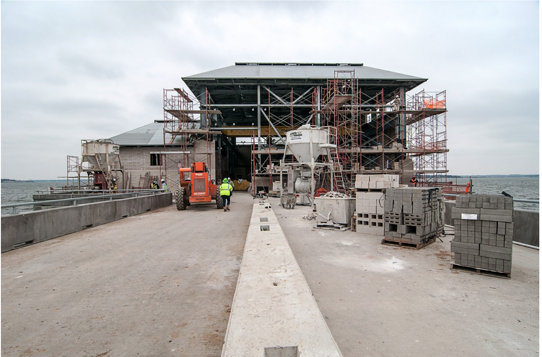
① Masonry installation at Raw Water Intake
