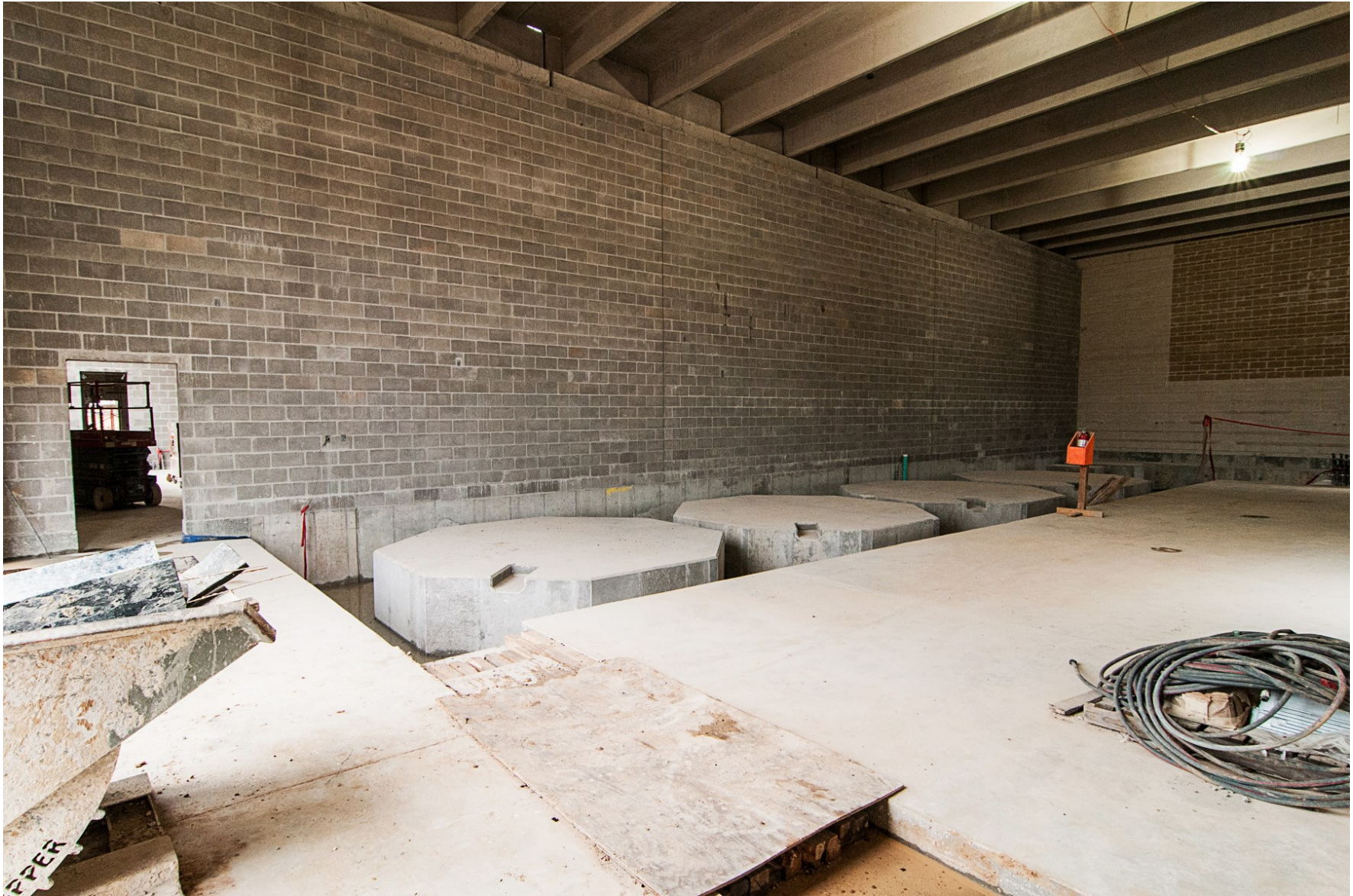
⑦ Interior view of Chemical Storage Basin pedestals
