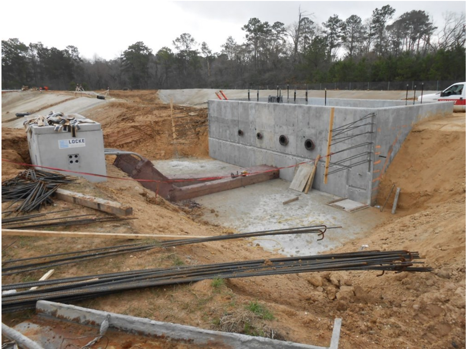
11 Water recovery basins and pump station
