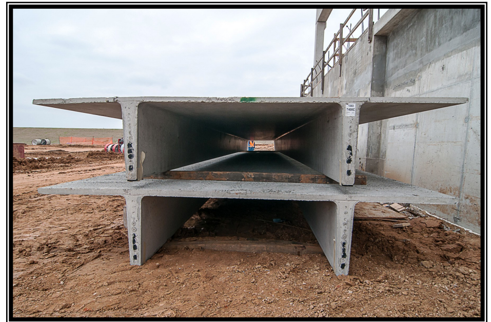
Concrete pre-cast panels outside of GAC Building at Surface Water Facilities
