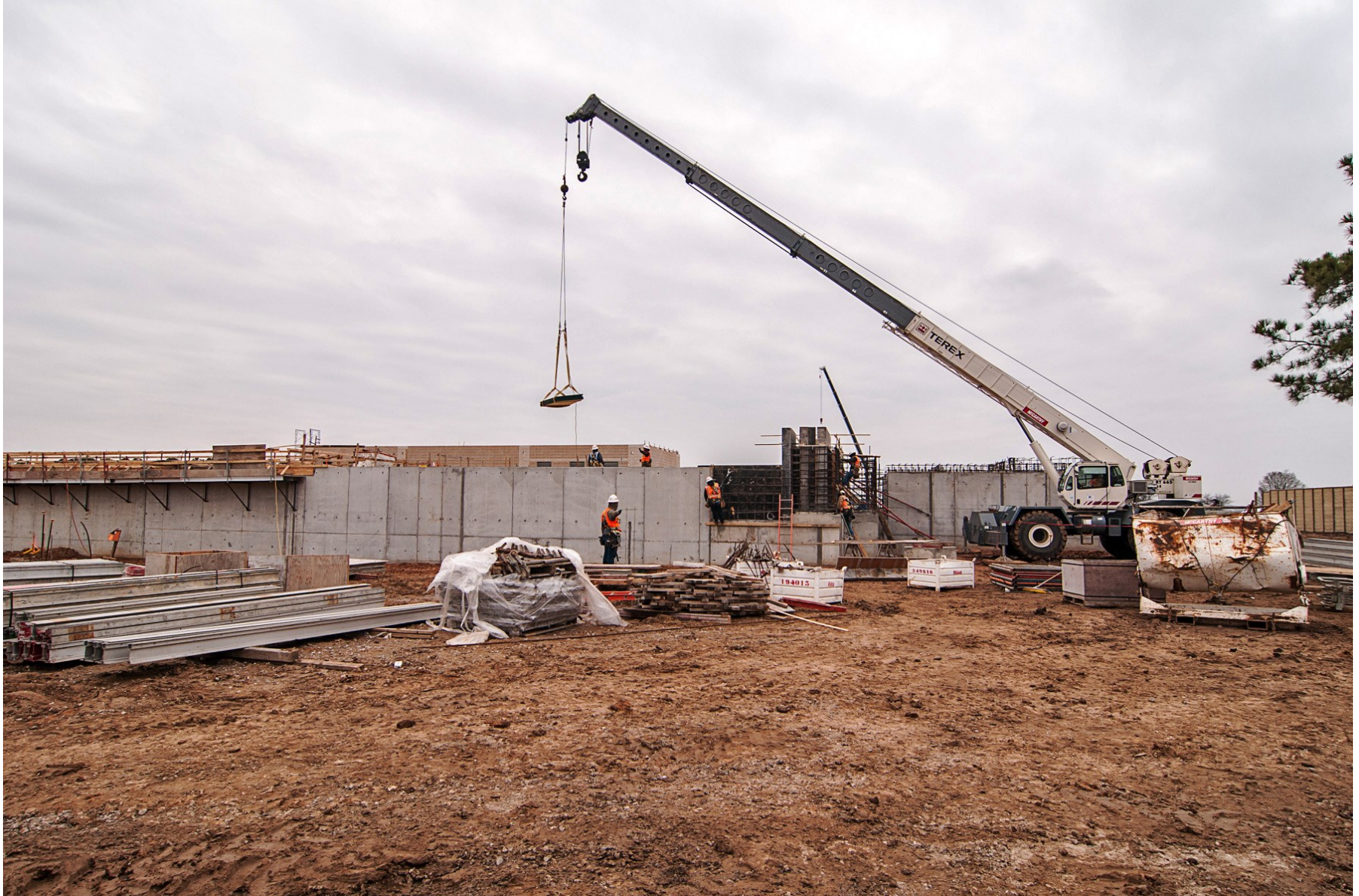
② Elevated walkway construction at the Pretreatment Facilities
