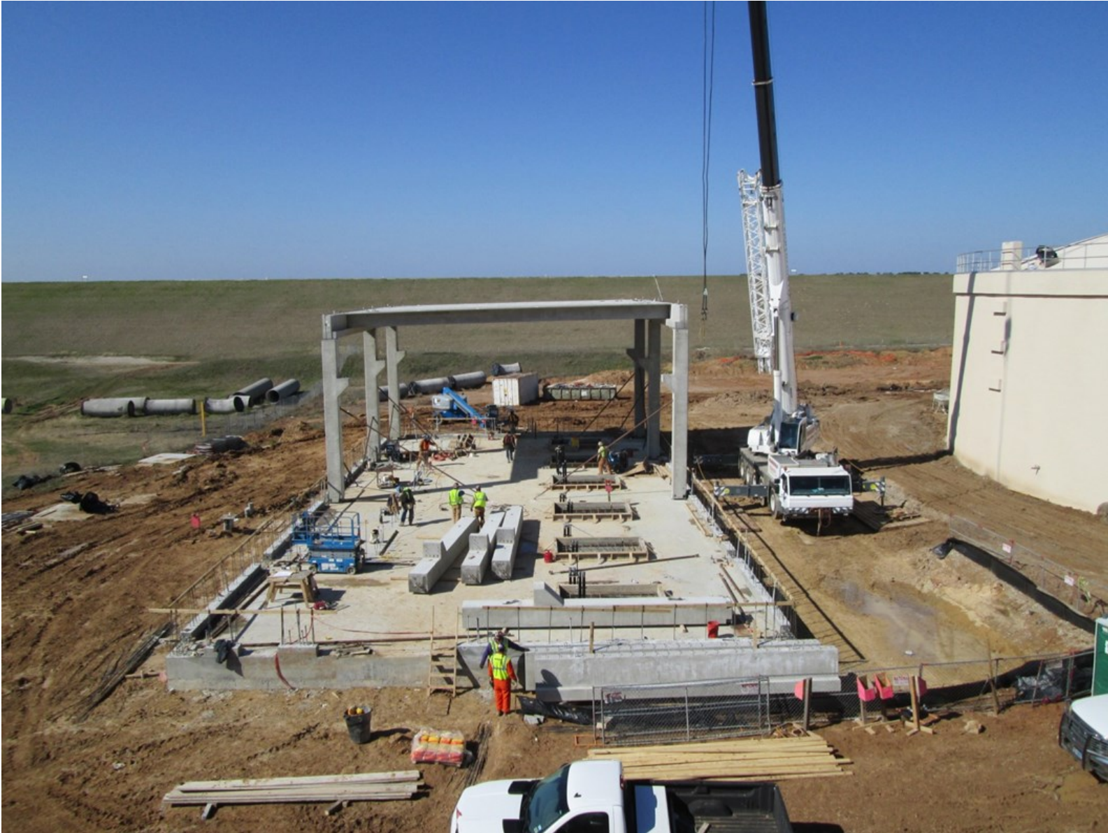
⑥ Pre-cast structure installation at Blower Building
