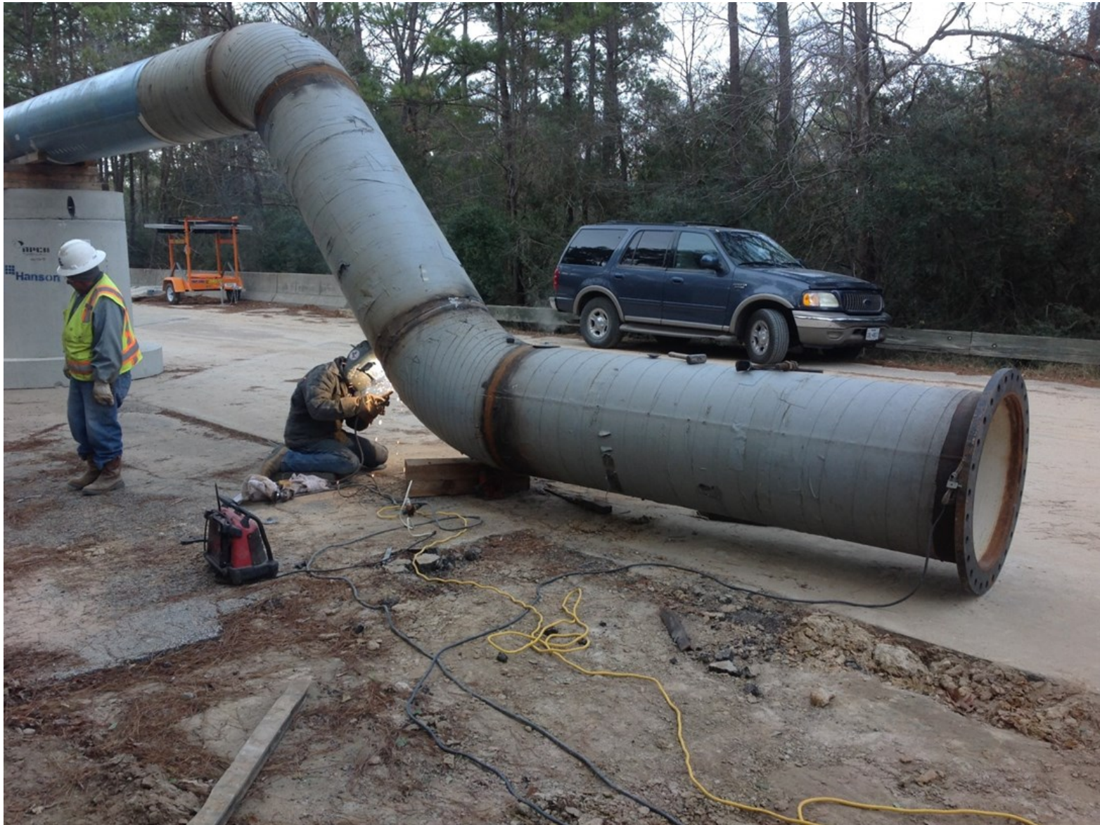
① Segment W2B - 30-inch aerial pipe crossing at Panther Branch along Grogans Mill Road
