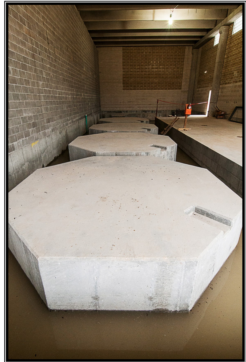
Interior view of chemical storage basin pedestals at Surface Water Facilities
