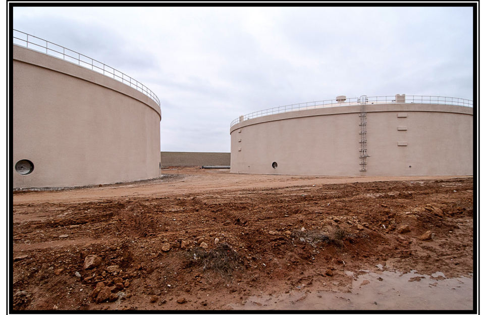
Ground Storage Tank Nos. 1 and 2 at Surface Water Facilities
