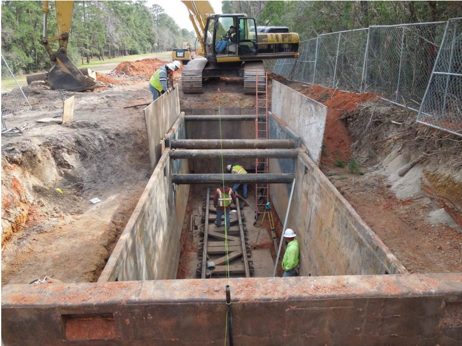
① Segment C2—Tunnel operation for 16-inch pipe crossing Longmire Road
