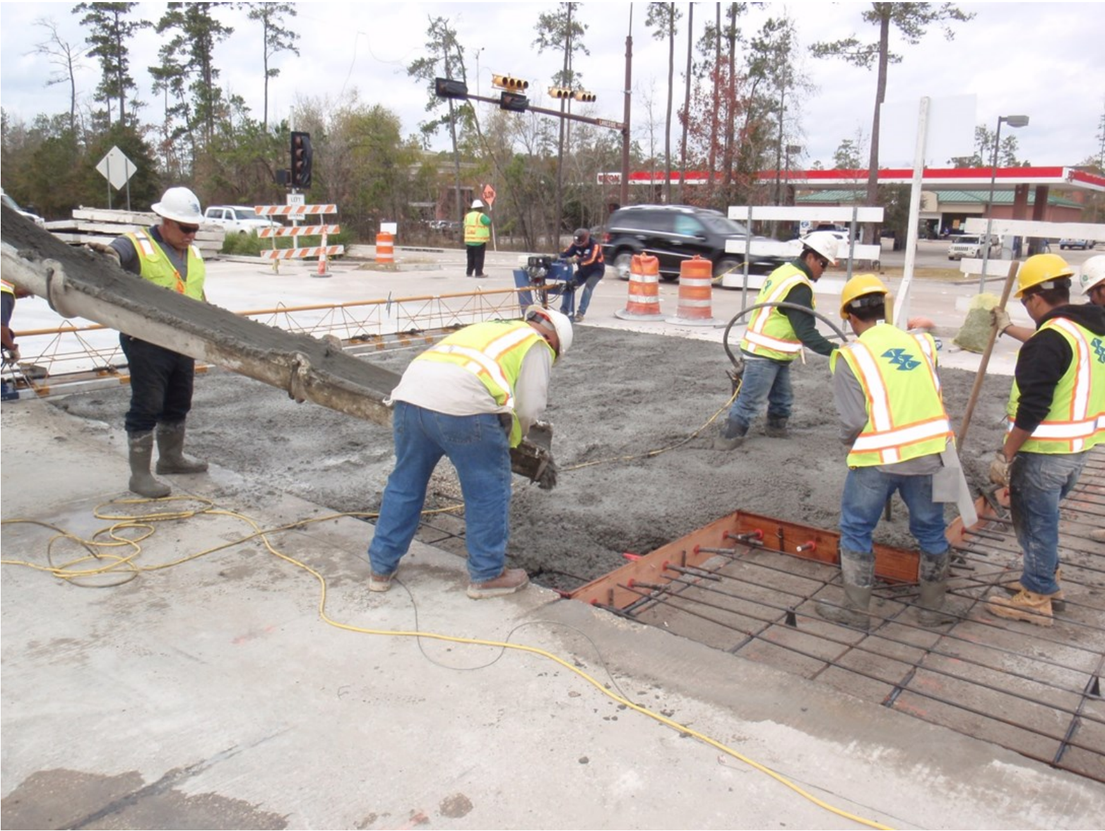
① Segment W2A - Concrete pavement replacement at Research Forest Drive and Lakeside Boulevard
