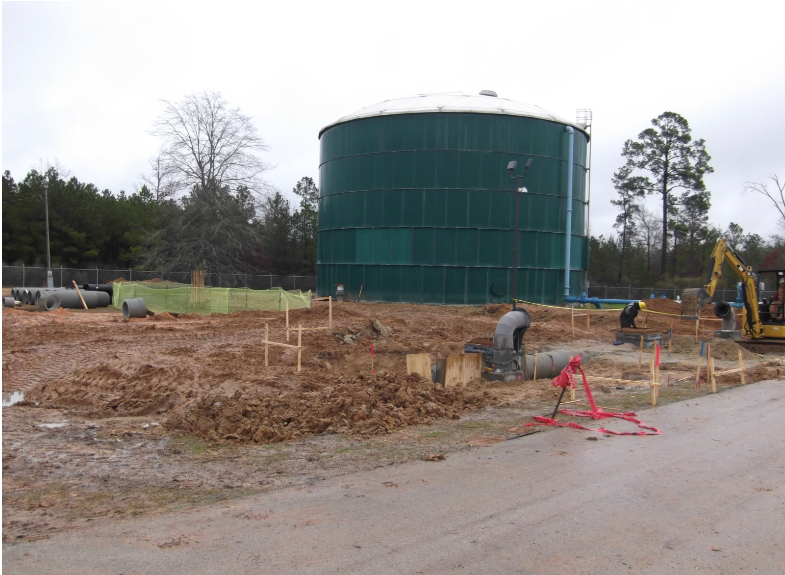
❶ Water Receiving Facilities—North— Yard piping installation at City of Conroe Water Plant No. 20
