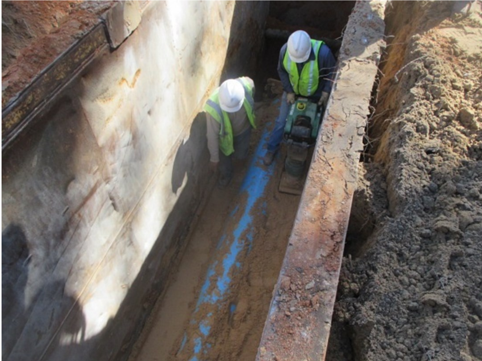
❶ Segment C1B - 16-inch PVC pipe installation along Longmire Road
