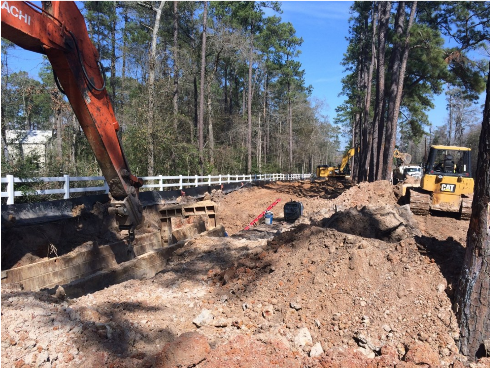
① Segment T1 - 60-inch pipe installation along McCaleb Road
