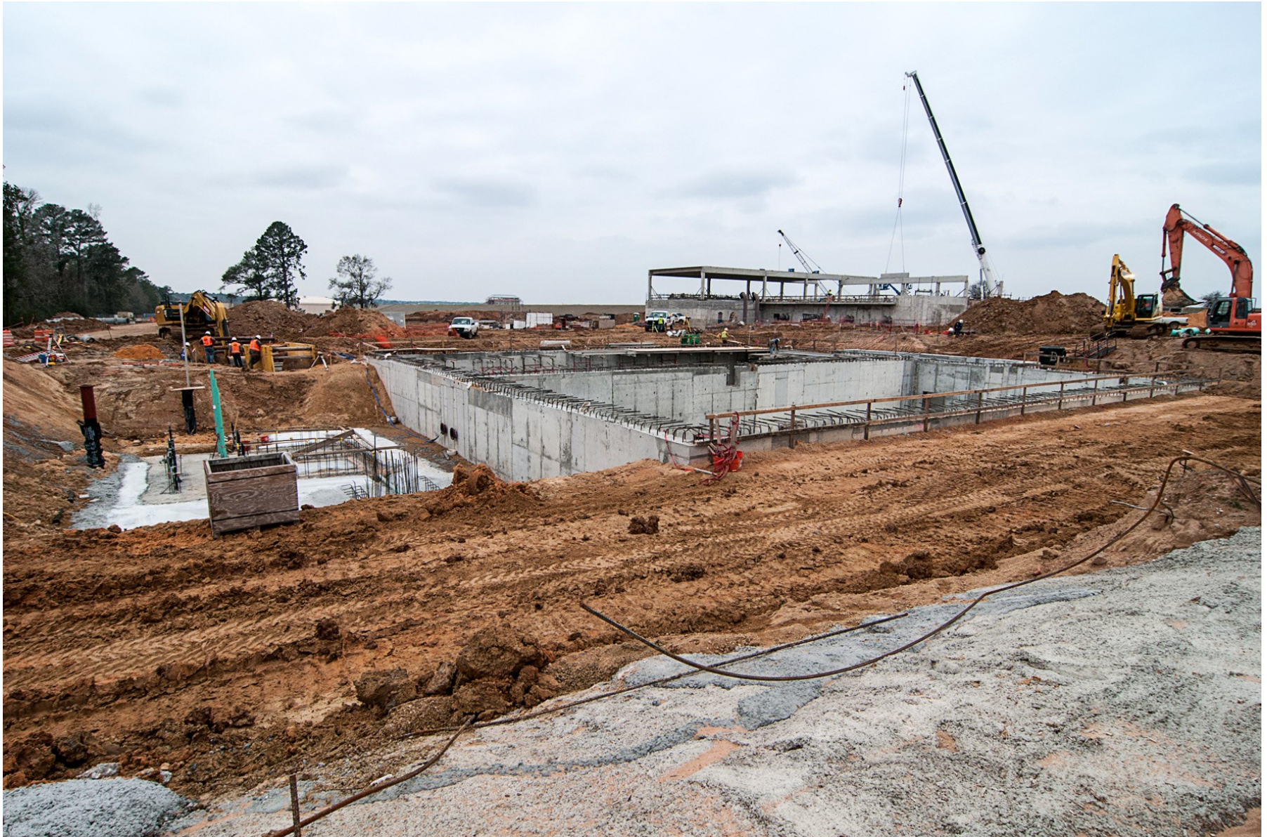
8 Backwash Equalization Basin deck
