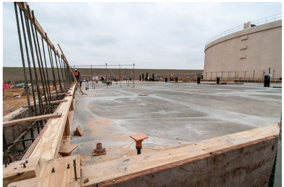
Blower Building Foundation at Surface Water Facilities
