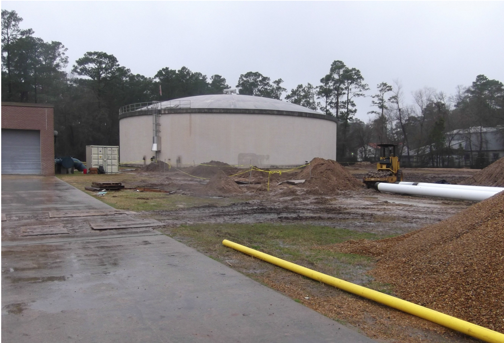
❶ Water Receiving Facilities—South—Yard piping installation at SJRA Water Plant No. 3
