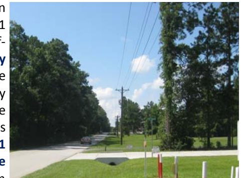
Power Poles along McCaleb Road (Segment T-1)
