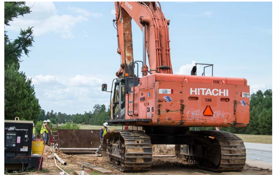
④ Segment T2 Tunnel Pit Crew
