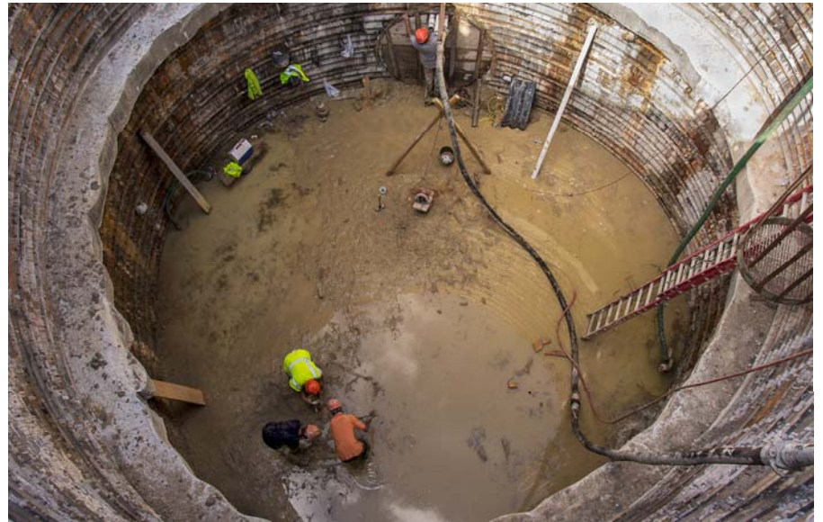
⑤ Segment T1 Tunnel West of Spillway Channel
