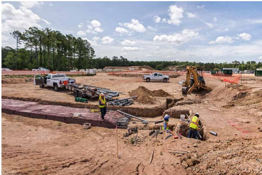
15 Electrical Conduit Installation at Chemical Storage Facilities
