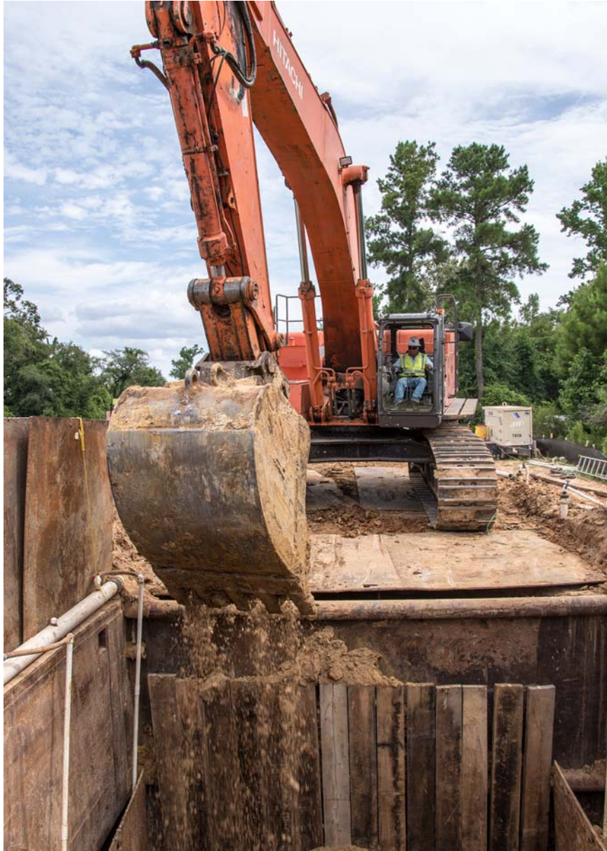
② Segment T2 Tunnel Pit Along Fish Creek Thoroughfare
