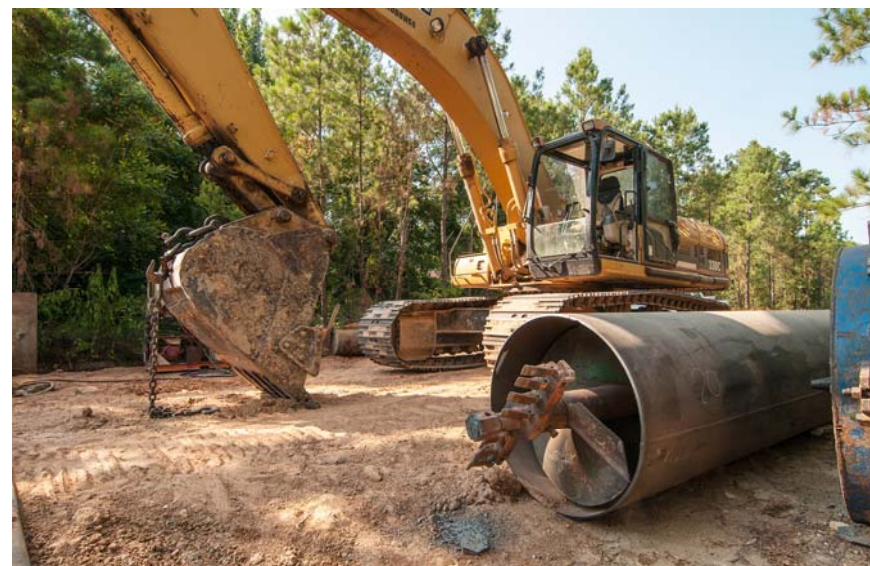
③ Segment W1B Tunneling Equipment
