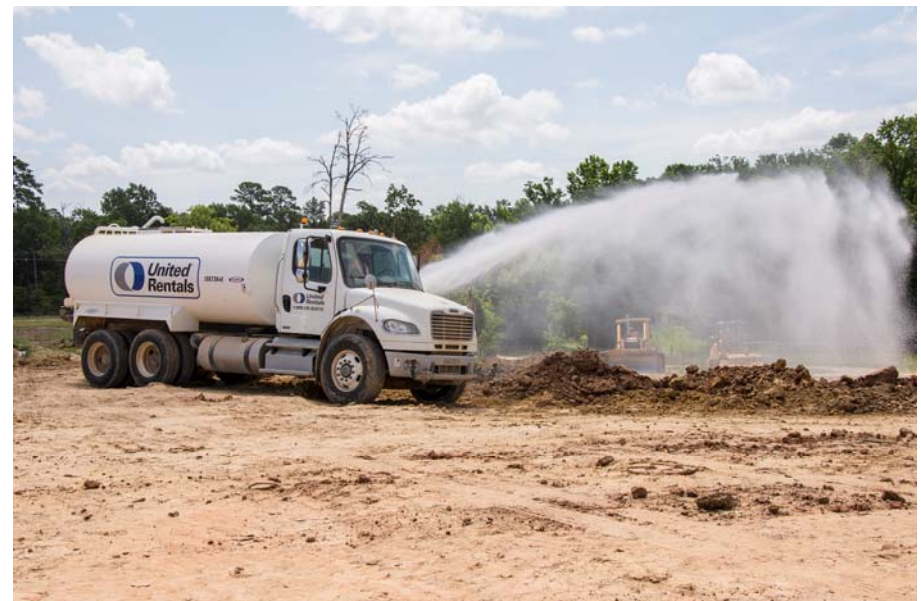
16 Soil Erosion/Stabilization Control
