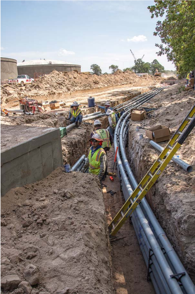
10 Electrical Conduit Installation at High Service Pump Station
