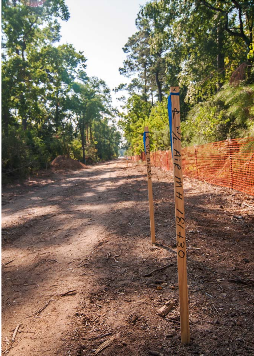
5 Segment W1A Staking and Tree Protection near Research Forest
