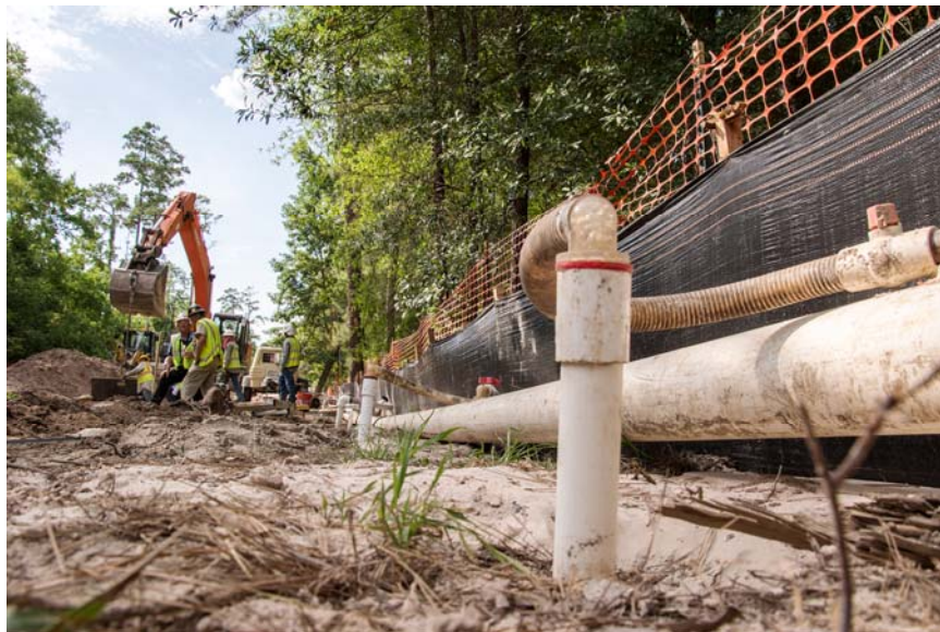
6 Segment W1B Dewatering Operation
