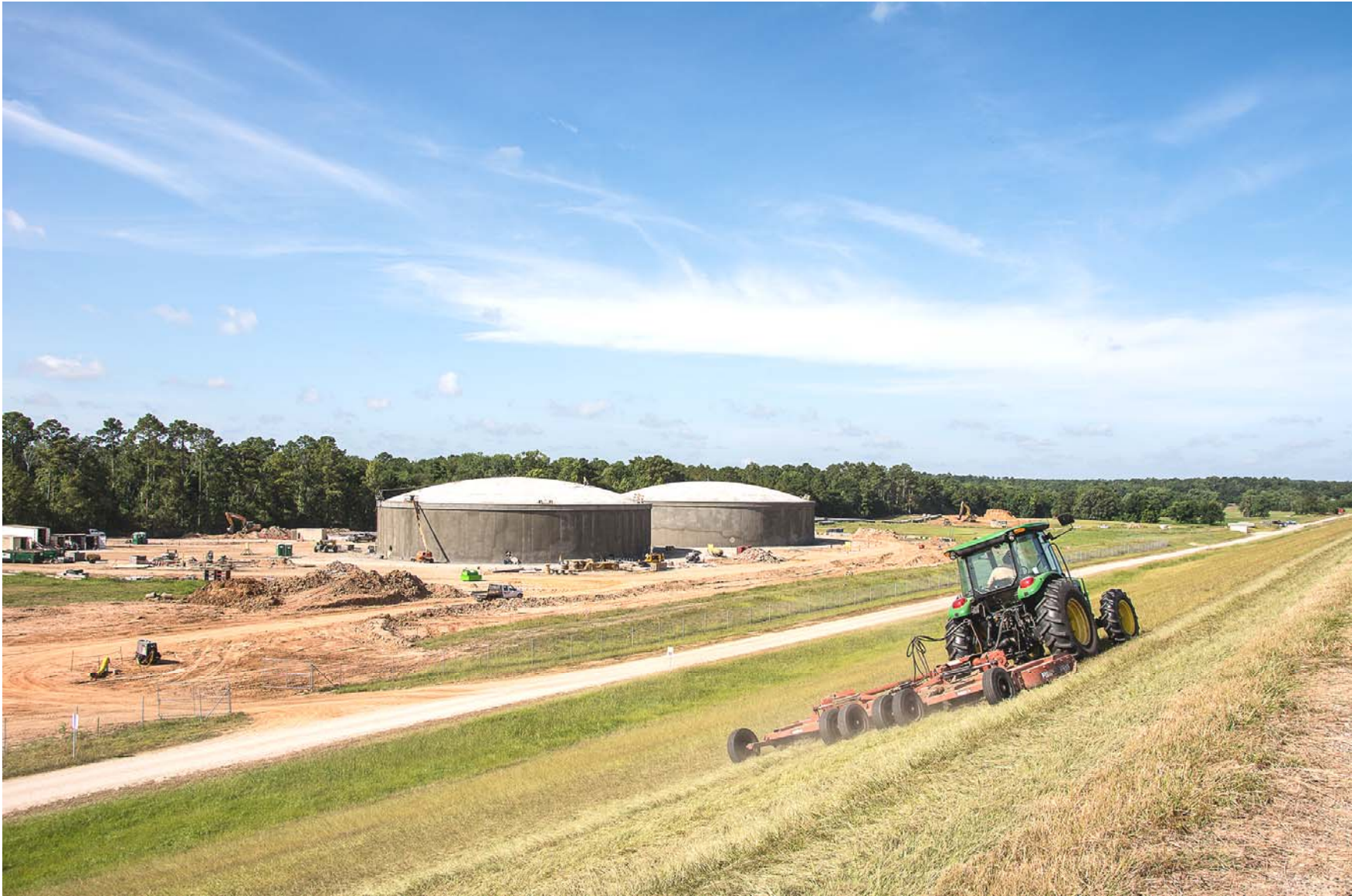
⑤ Ground Storage Tank Nos. 1 and 2
