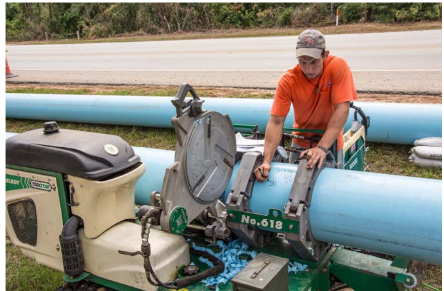
④ Segment W1A PVC Pipe Joint Fusion
