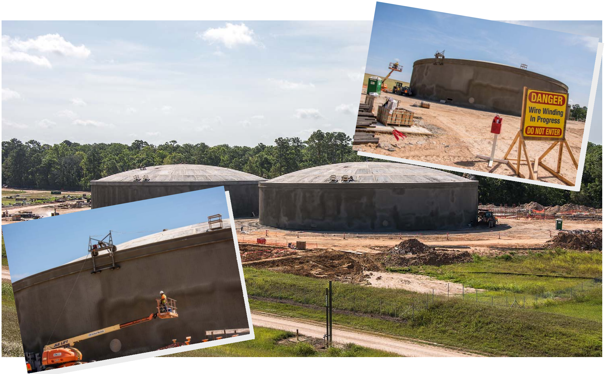
6 7 8 Ground Storage Tank Nos. 1 and 2
