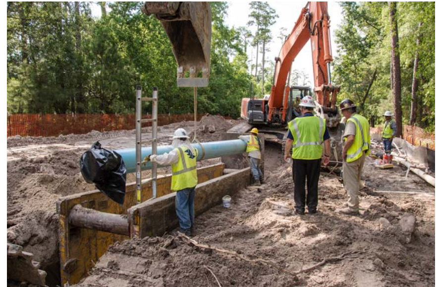
5 Segment W1B 16-inch Well Collection Line - Alden Bridge at Panther Creek
