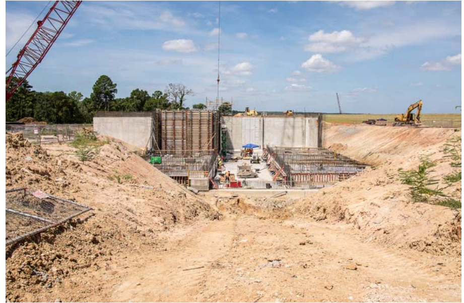
14 Installation of the GAC Wall Begins
