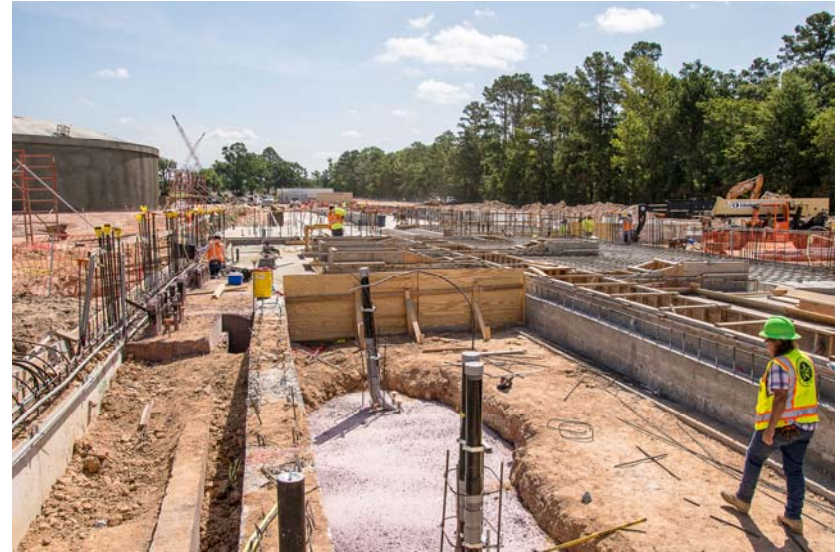
11 Progress on High Service Pump Station
