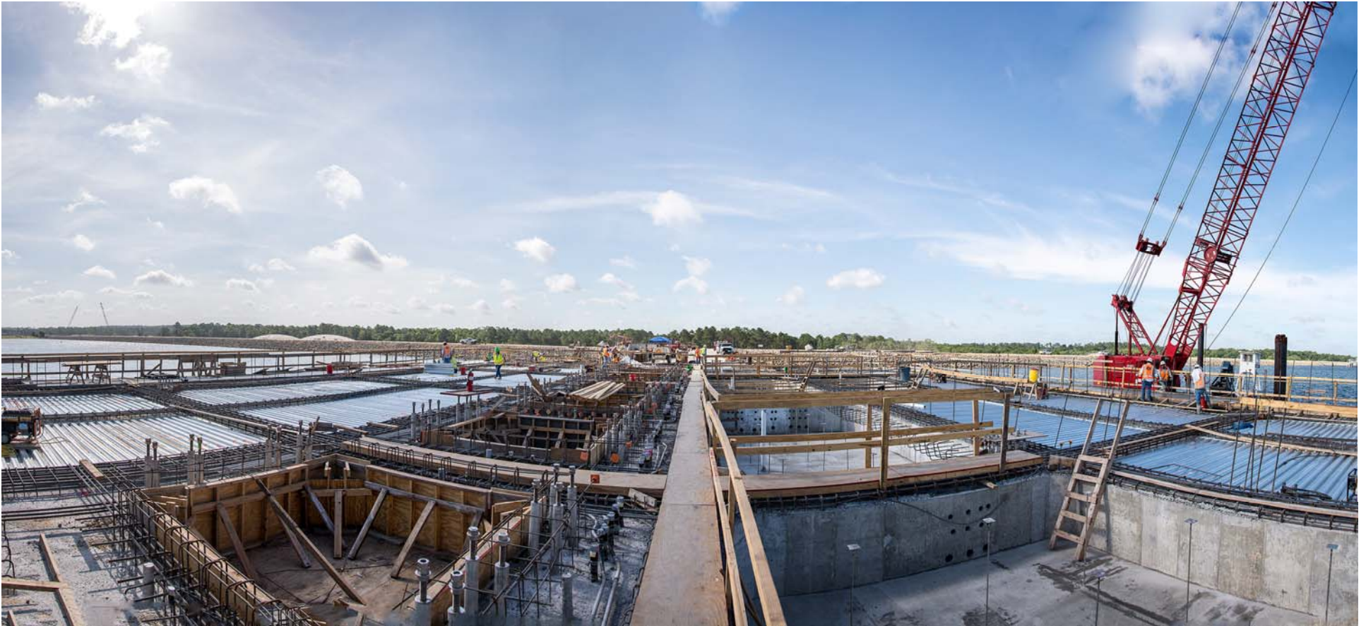
❶ Raw Water Pump Station at end of Pier
