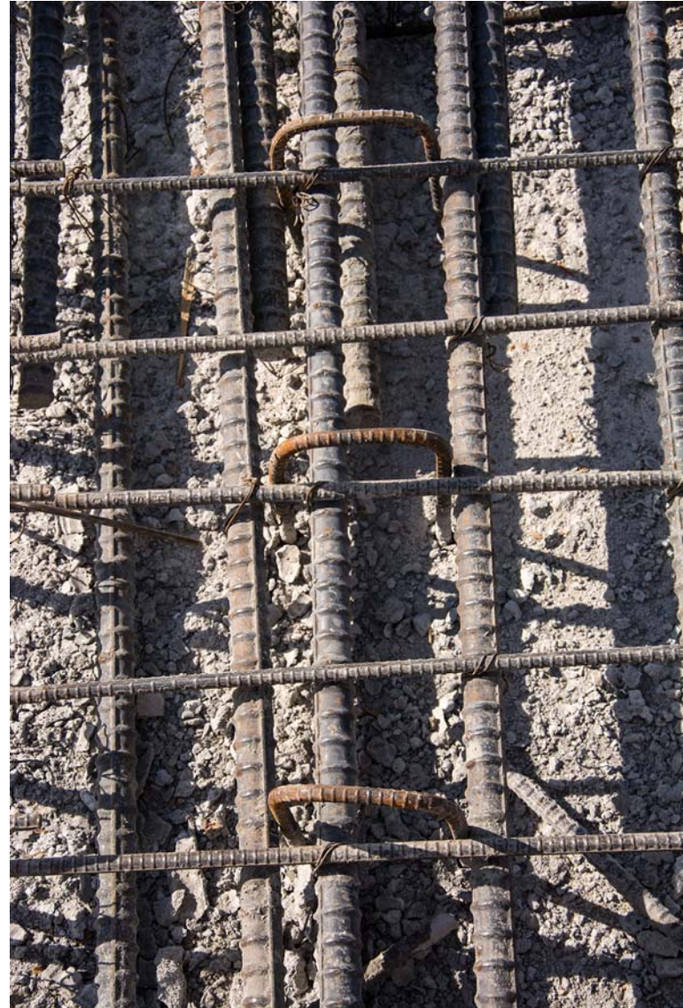
Rebar used in the construction of the High Service Pump Station
