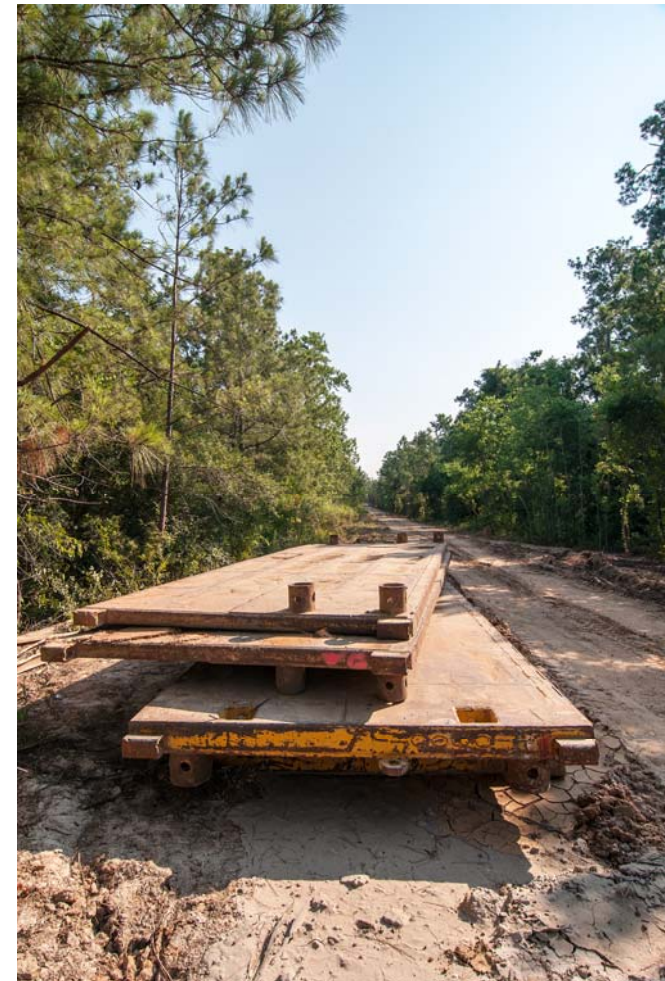
Trench Box at Transmission Segment W1B
