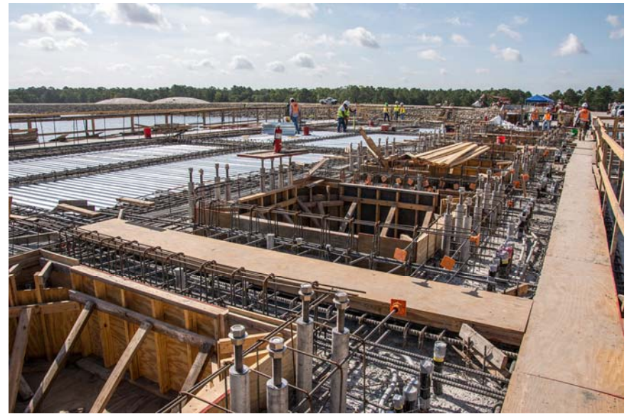
②③④ Raw Water Pump Station - Pier and Foundation nearing completion
