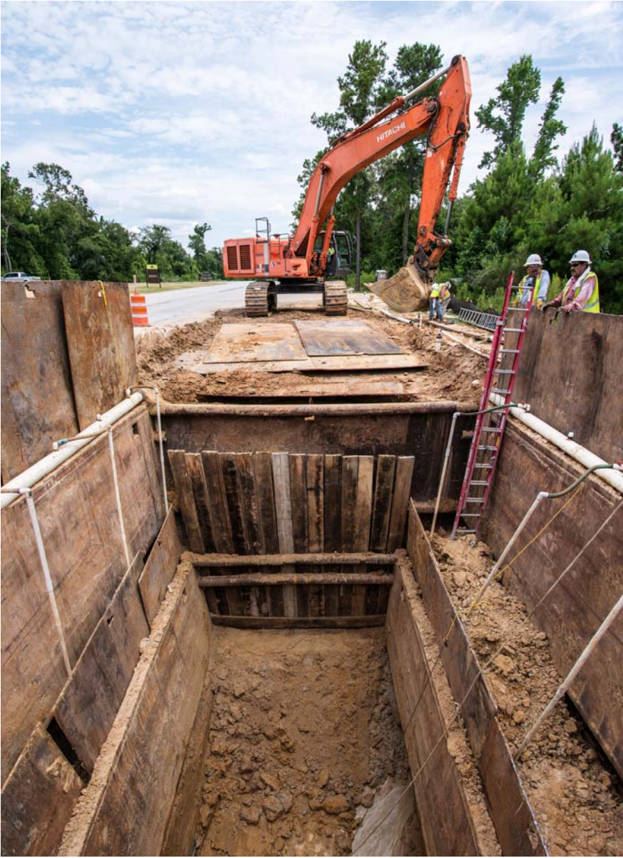
1 Segment T2 Tunnel Pit Installation
