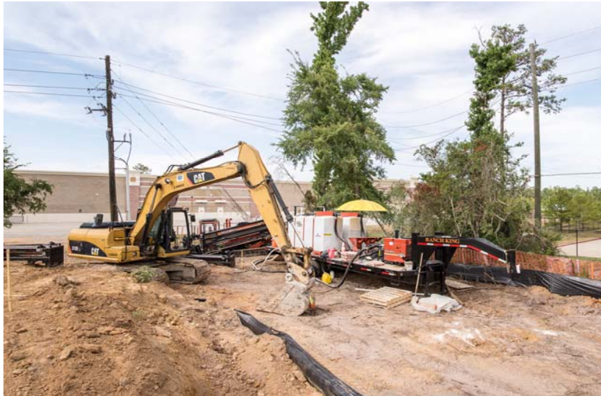
① Segment W1A Tunnel Boring Operation
