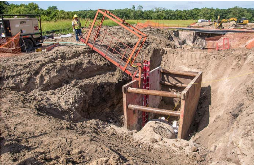
④ Segment T1 60-inch Access For Pipe Welding
