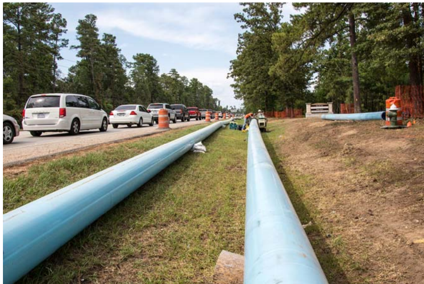
③ Segment W1A Fused PVC Pipe along FM 2978
