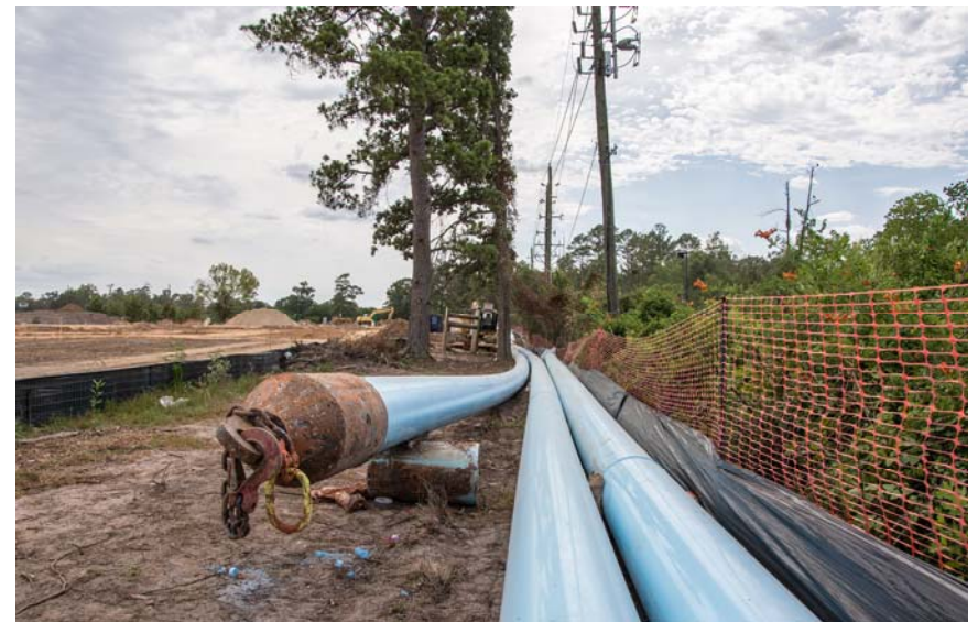
7 Segment W1A Fused PVC Pipe Ready for Installation
