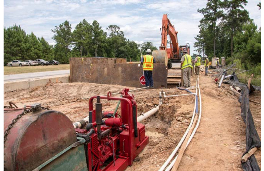
③ Segment T2 Dewatering Pump
