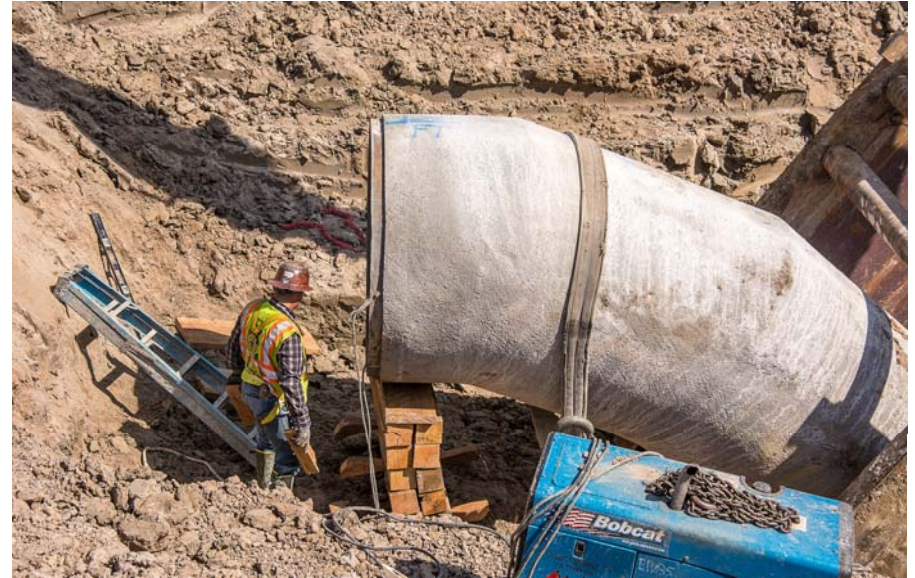
③ Segment T1 60-inch Pipe West of Spillway Channel
