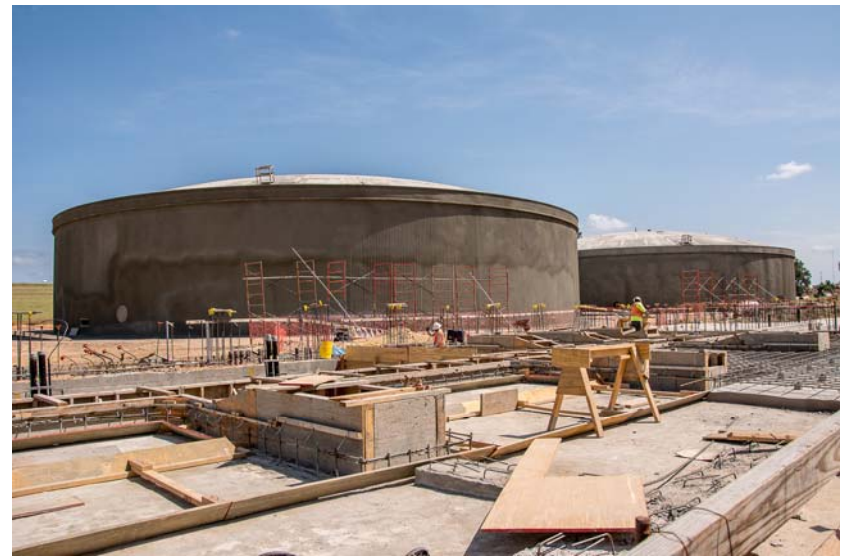
12 Progress on High Service Pump Station
