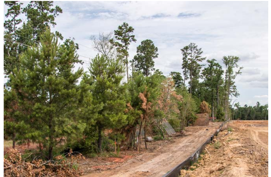
② Segment W1A Completed Section
