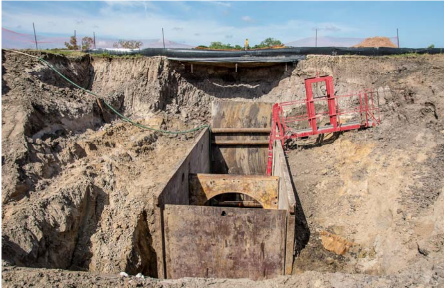
② Segment T1 Tunnel Access East of Spillway Channel
