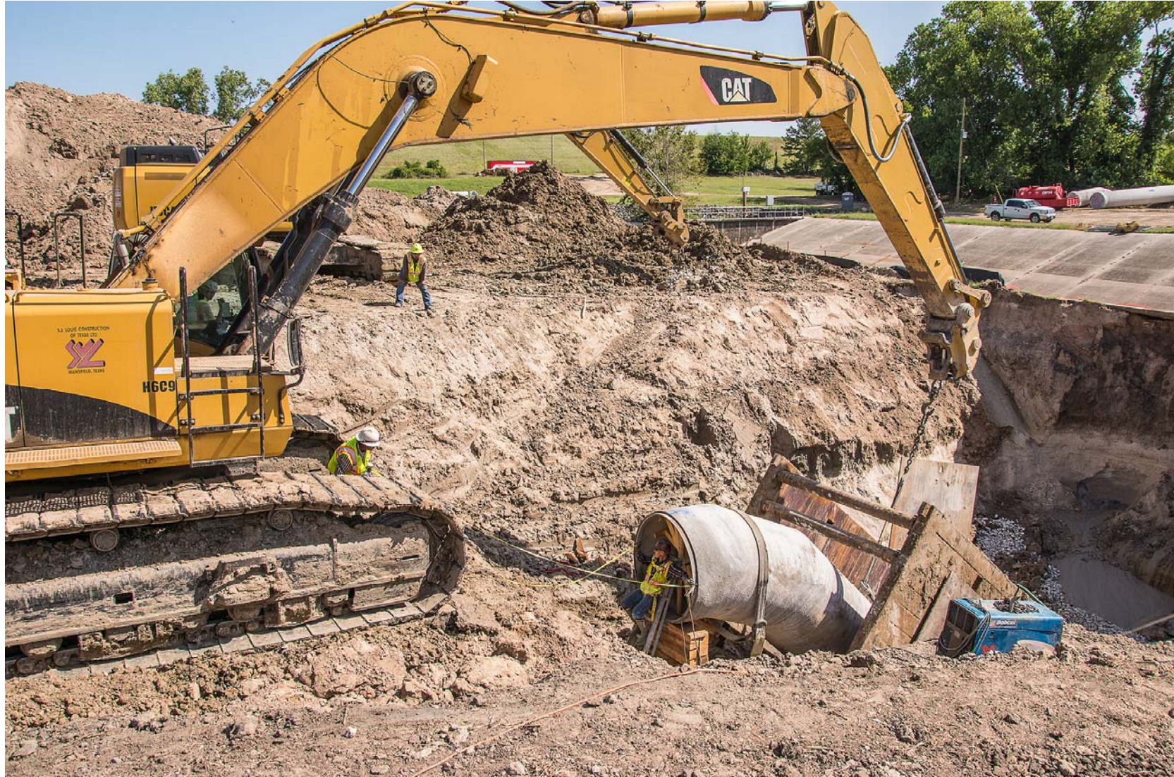
① Segment T1 60-inch Pipe Installation Under Spillway Channel
