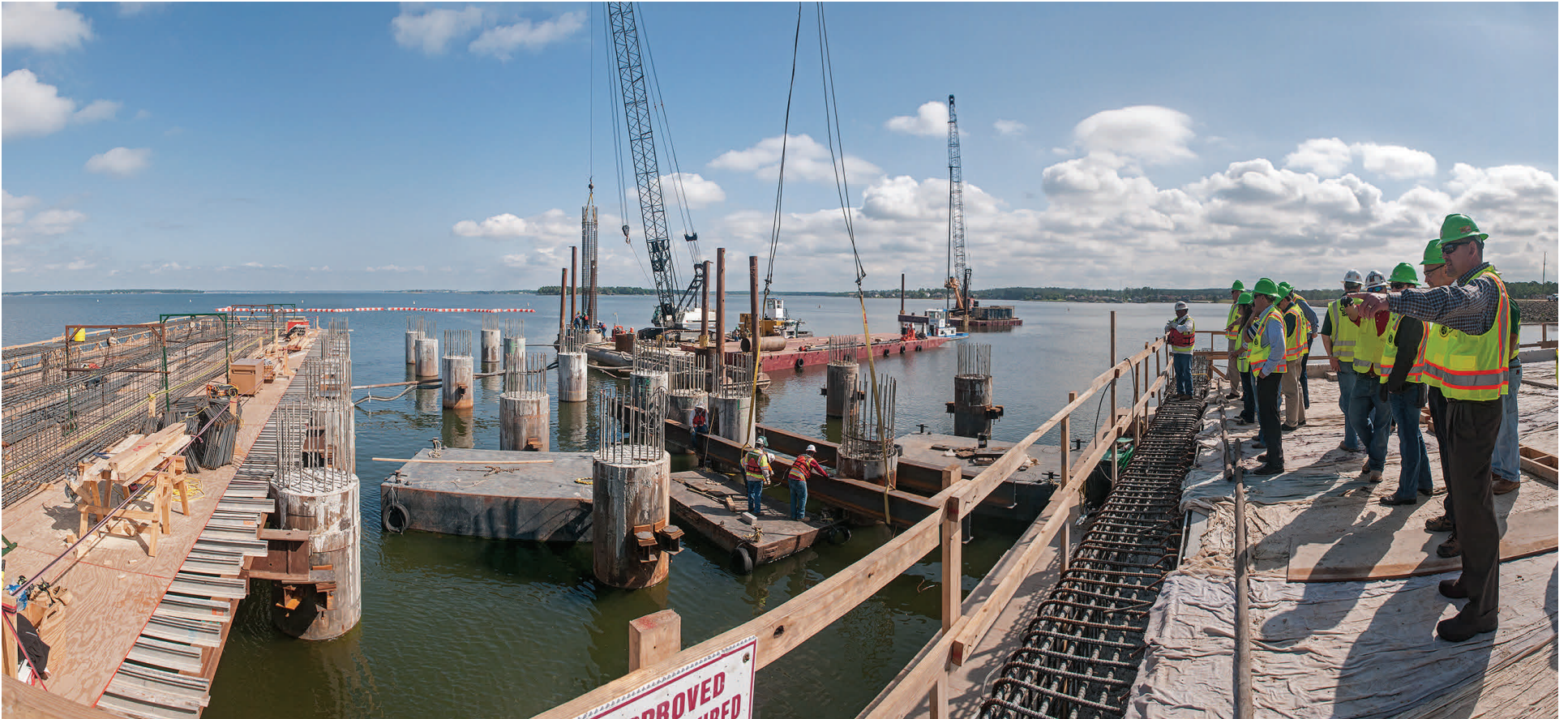
Raw Water Pump Station Site Tour - April 22, 2013
