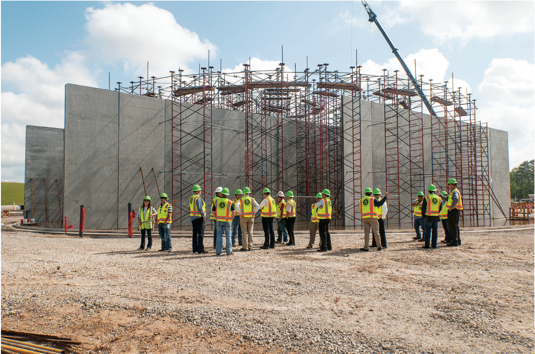
Ground Storage Tank No. 2 Site Tour - Baffle walls completed with scaffolding erection for wall placement - April 22, 2013
