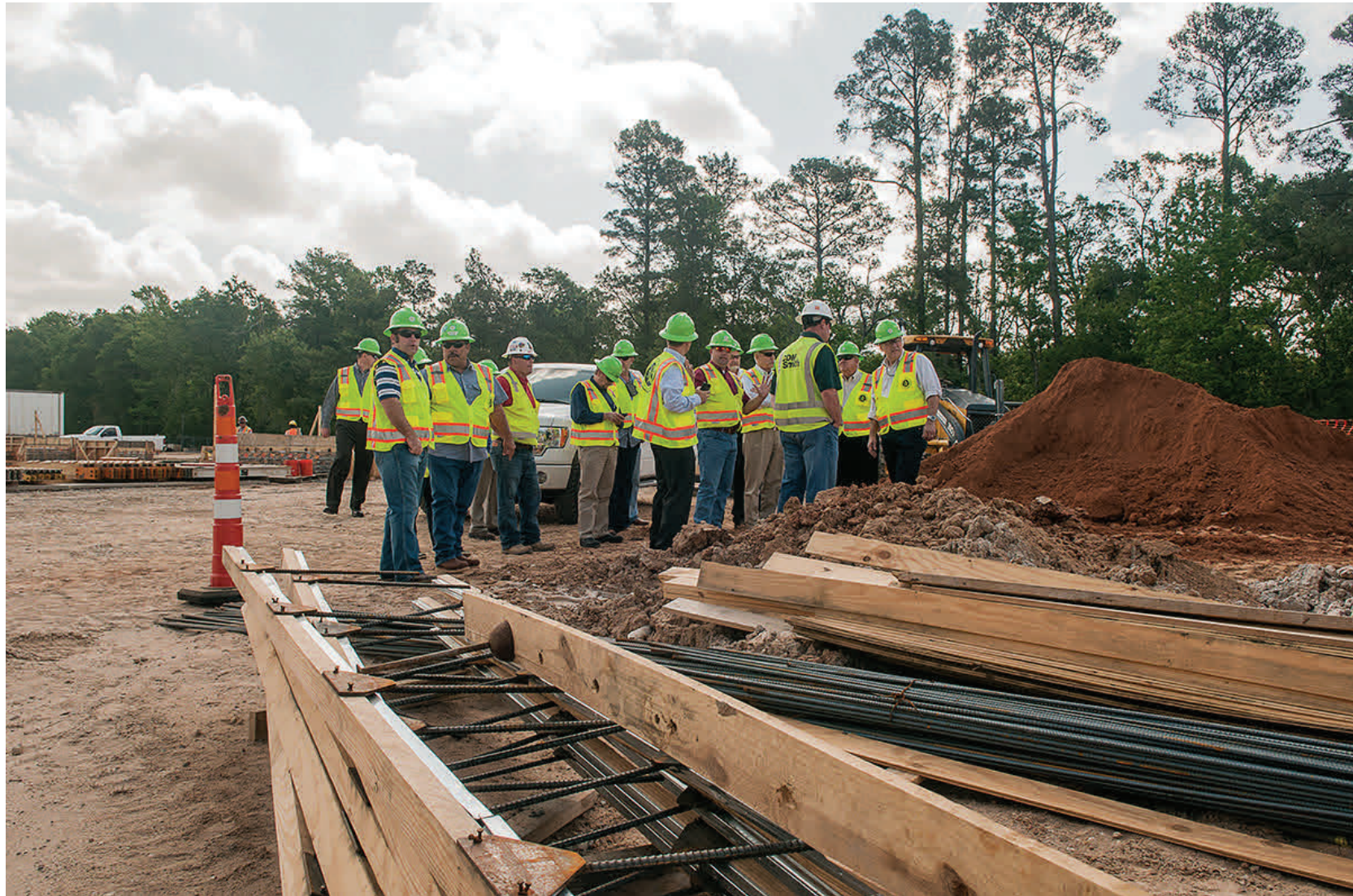
Construction Site Tour - April 22, 2013
