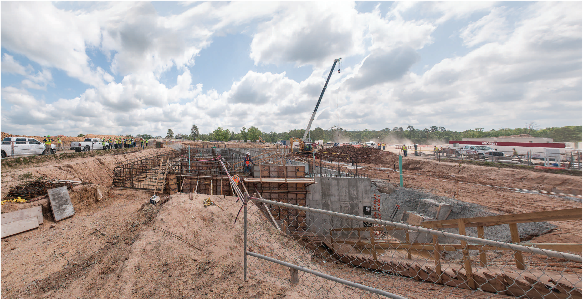
Membrane Facilities - April 22, 2013
