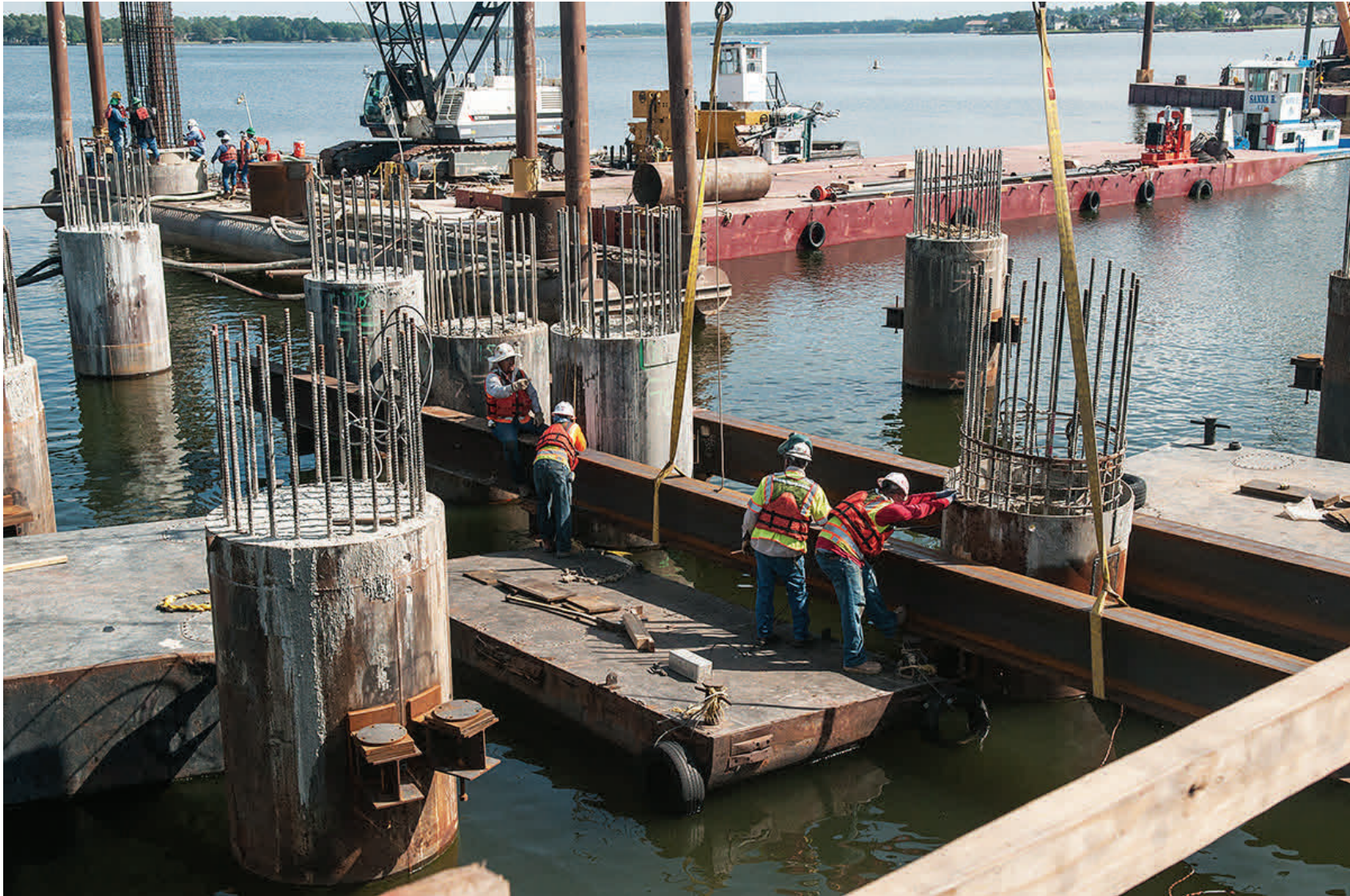
Raw Water Pump Station - Workers assemble temporary construction deck supports - April 22, 2013
