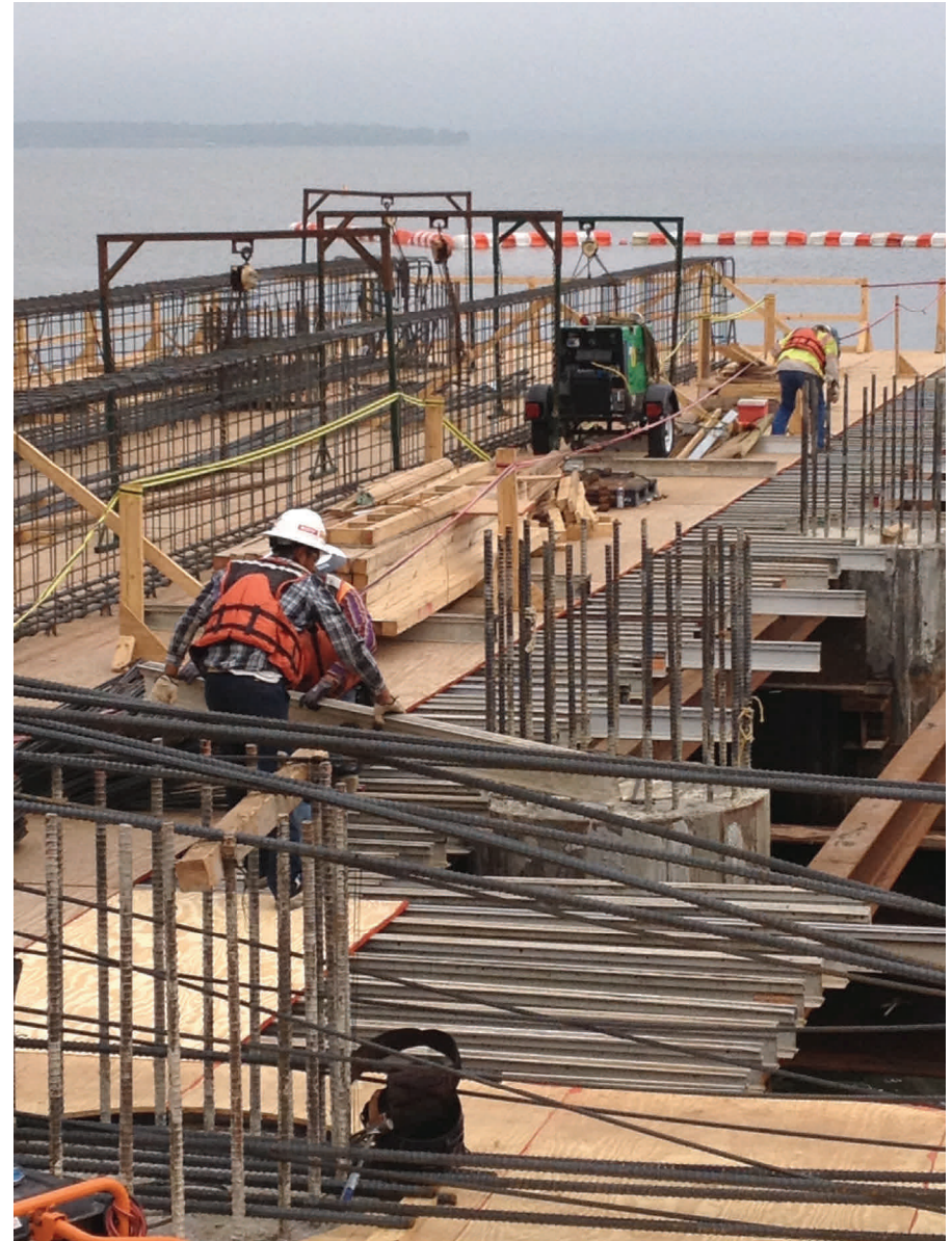
Temporary Construction Platform Installation at Raw Water Pump Station
