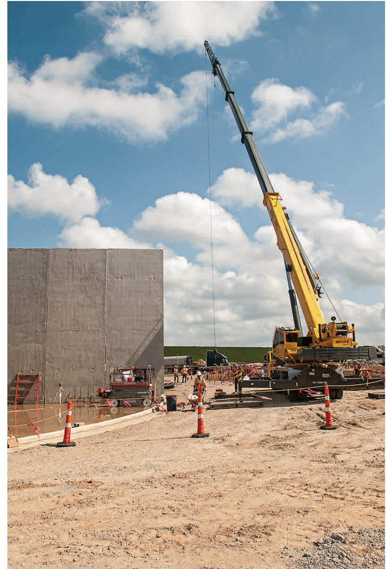
Site work at Ground Storage Tank No. 1 - April 22, 2013
