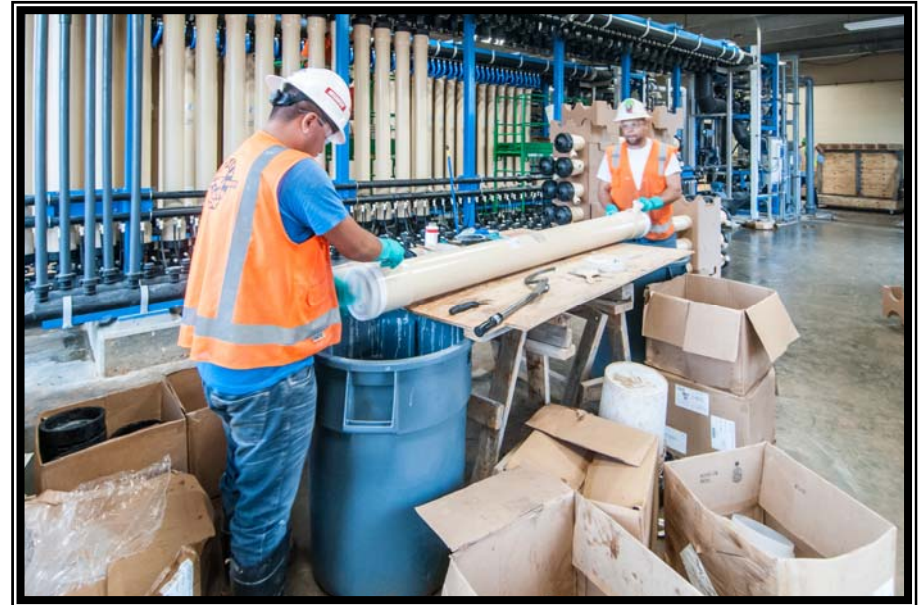
Left, Above, and Bottom: Workers preparing to install membrane cartridges
