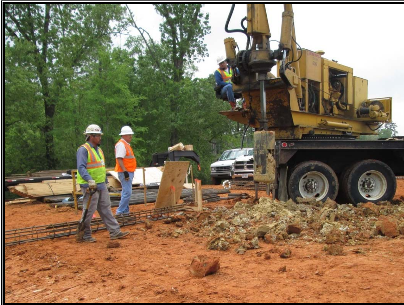
⑤ Maintenance Building — Installation of drilled shafts
