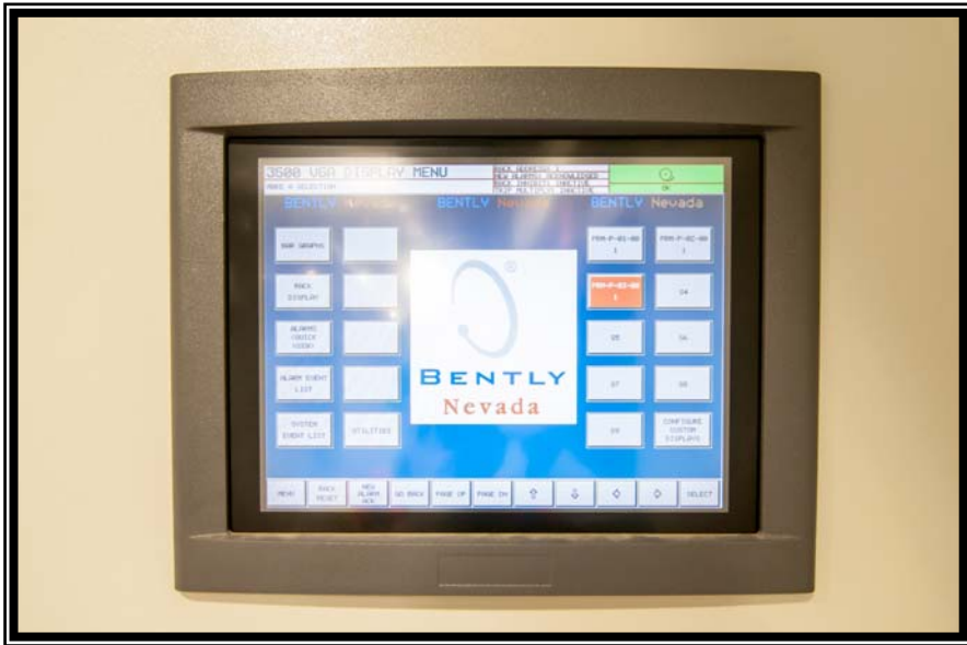
Instrumentation at the Raw Water Intake Facility
