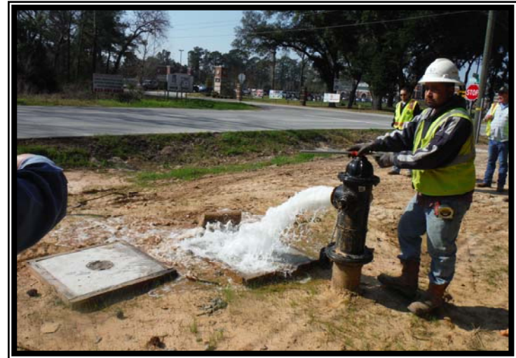
Employees observing construction worker flushing transmission lines
