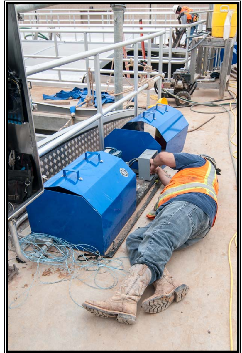
Worker at the Pretreatment Facility installing electrical wiring
