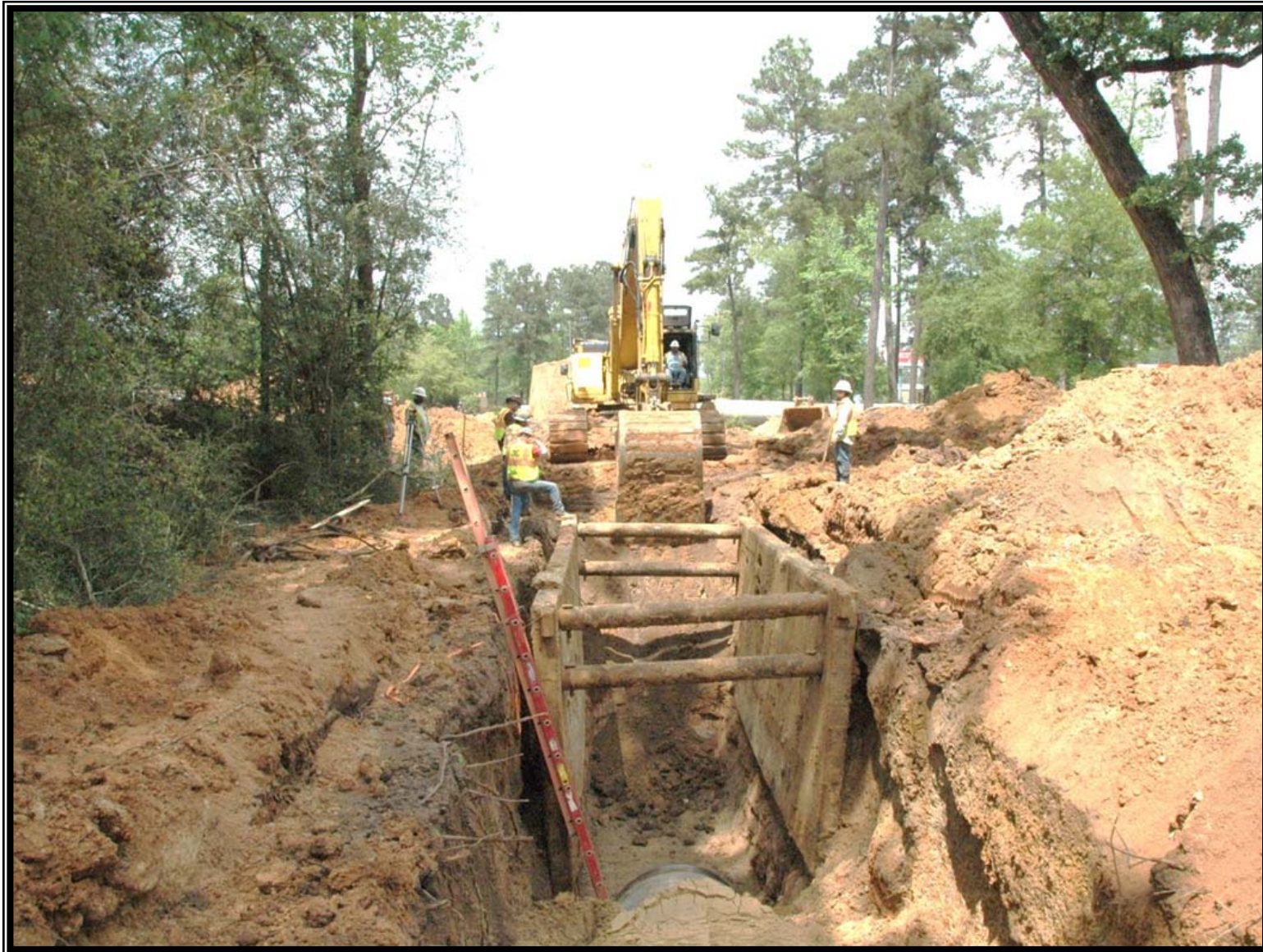
❶ 54-inch open-cut installation along Sendera Ranch Drive
