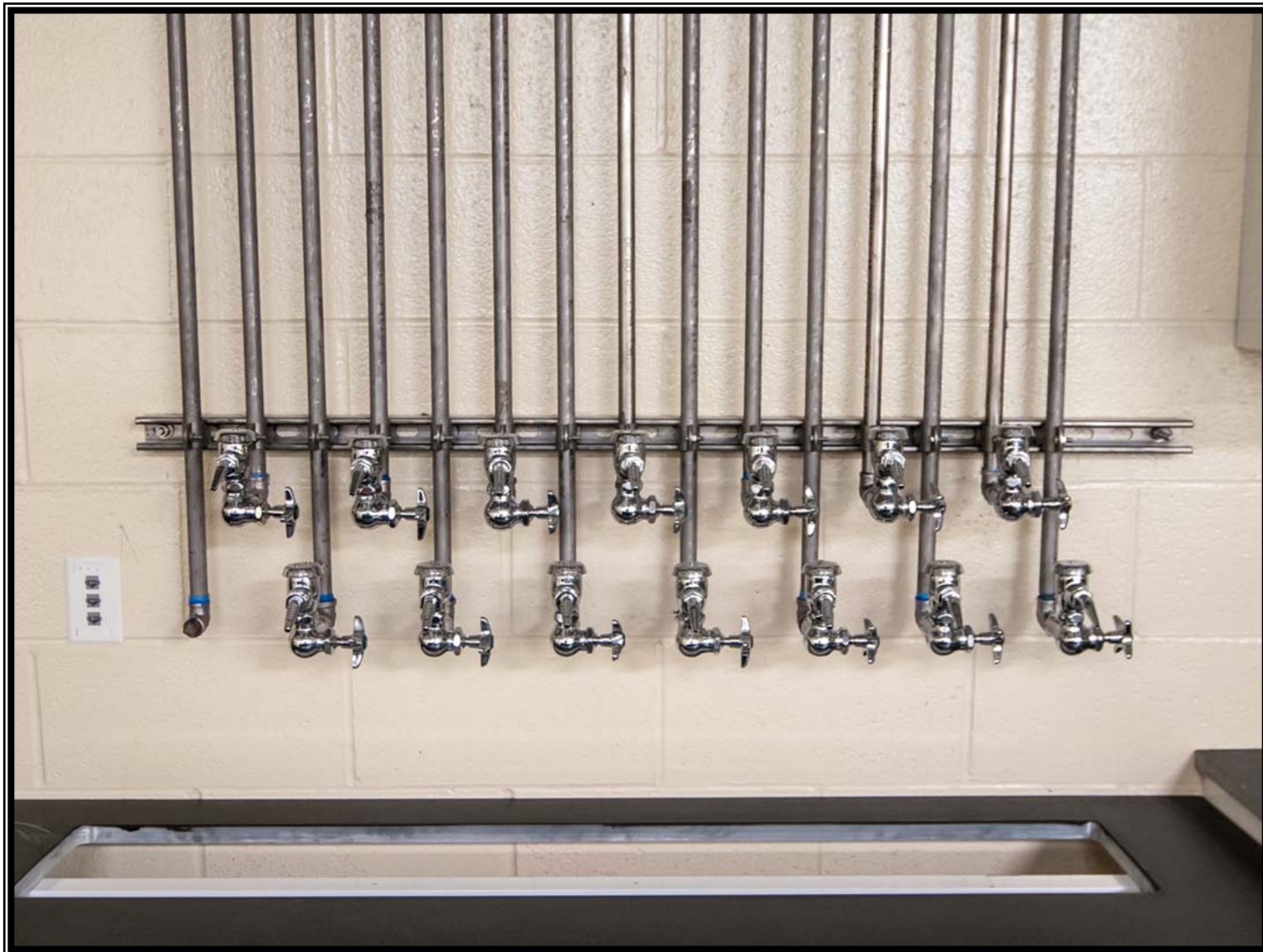
① Membrane Building — Installation of process water sample faucets
