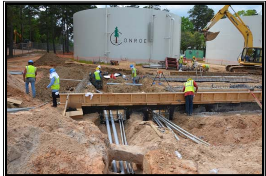
System Improvements at Conroe Water Plant No. 6
