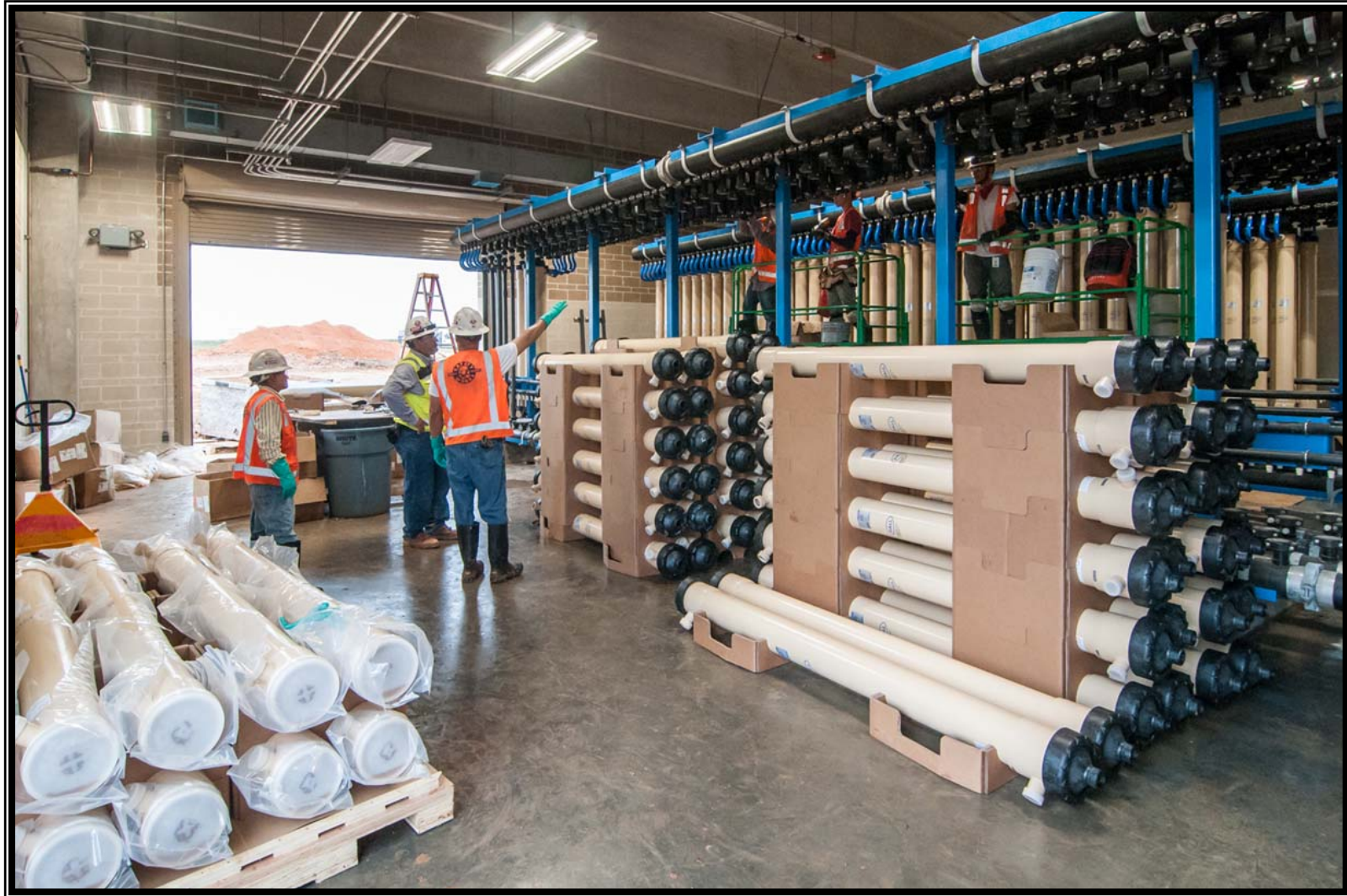
❶ Membrane Building — Installation of membrane cartridges
