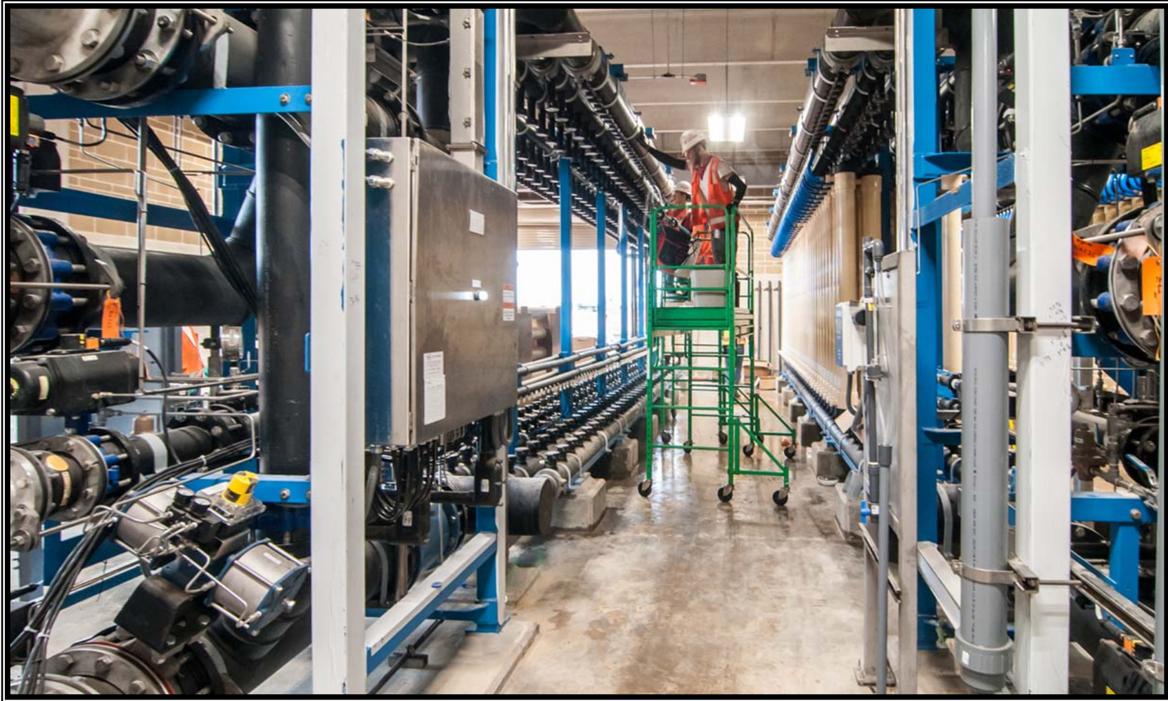
① Membrane Building — Installation of membrane cartridges
