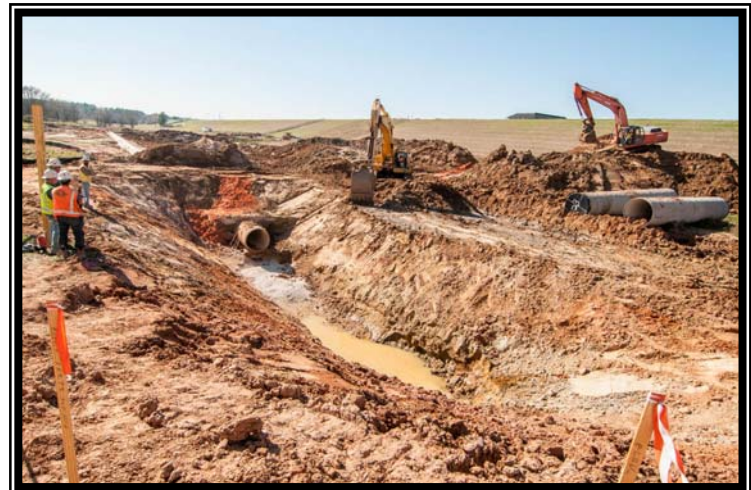
Workers overlooking the installation of a raw waterline at the Surface Water Treatment Plant
