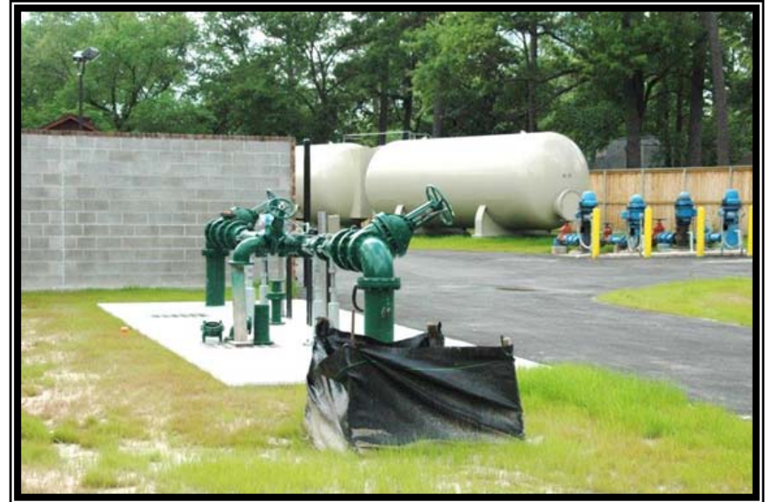
Oak Ridge North Water Receiving Facility
