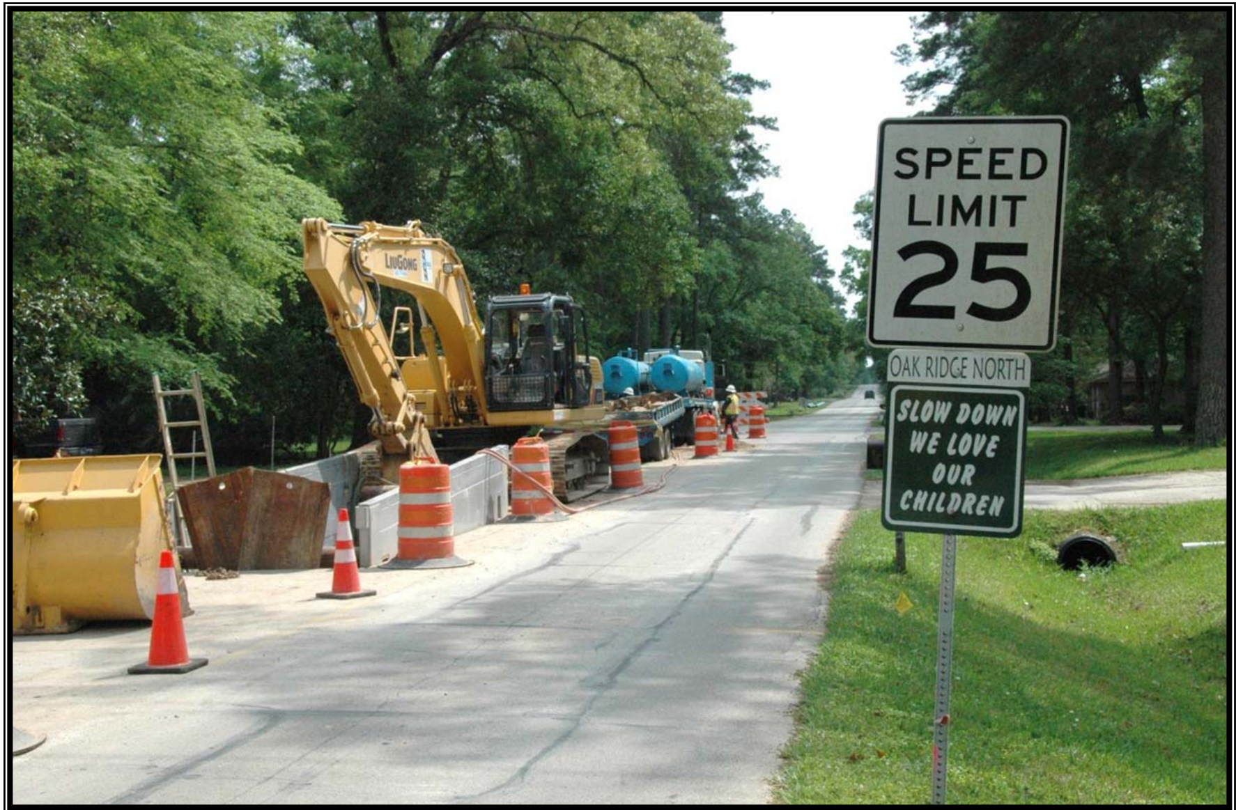
① 16-inch pipe trenchless bore pit installation along Maplewood Drive
