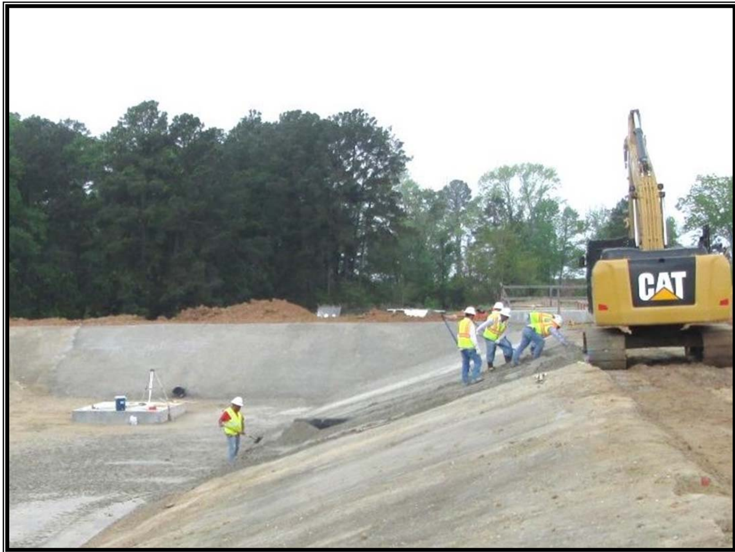
④ Process Water Recovery — Soil cement lining installation
