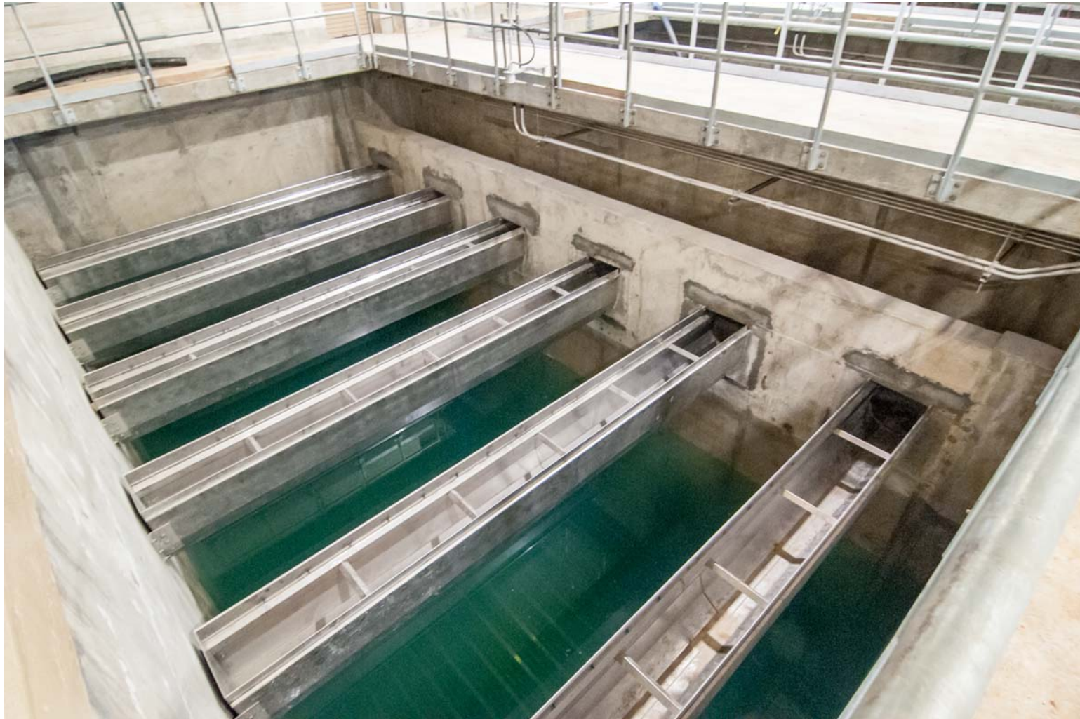
② Granulated Activated Carbon (GAC) Building
