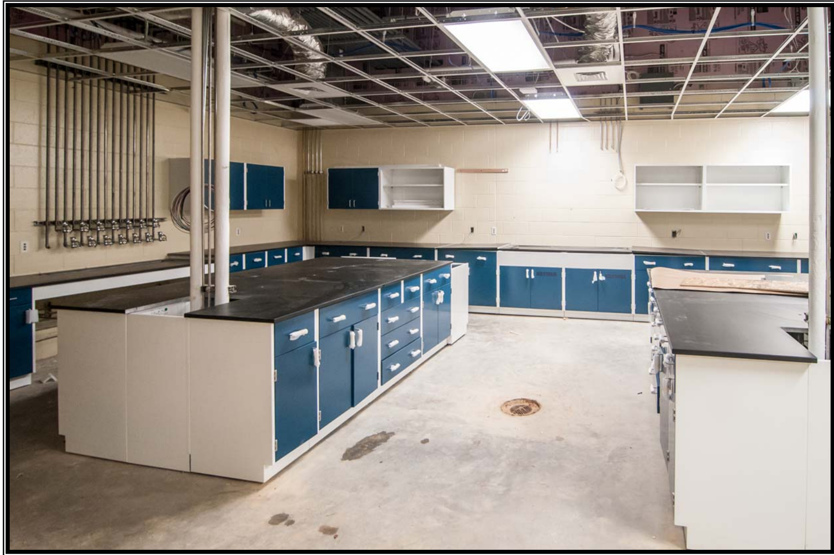
❶ Membrane Building — Lab millwork installation
