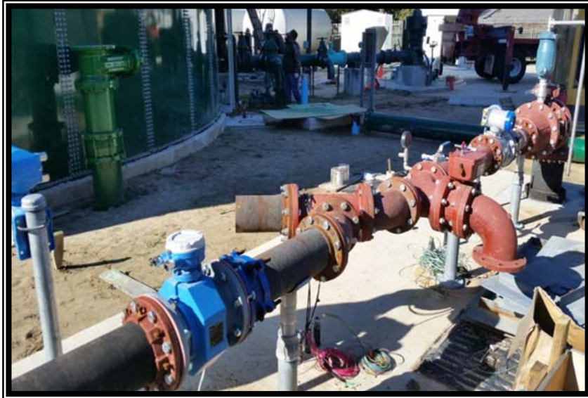
Rayford Road Water Receiving Facility
