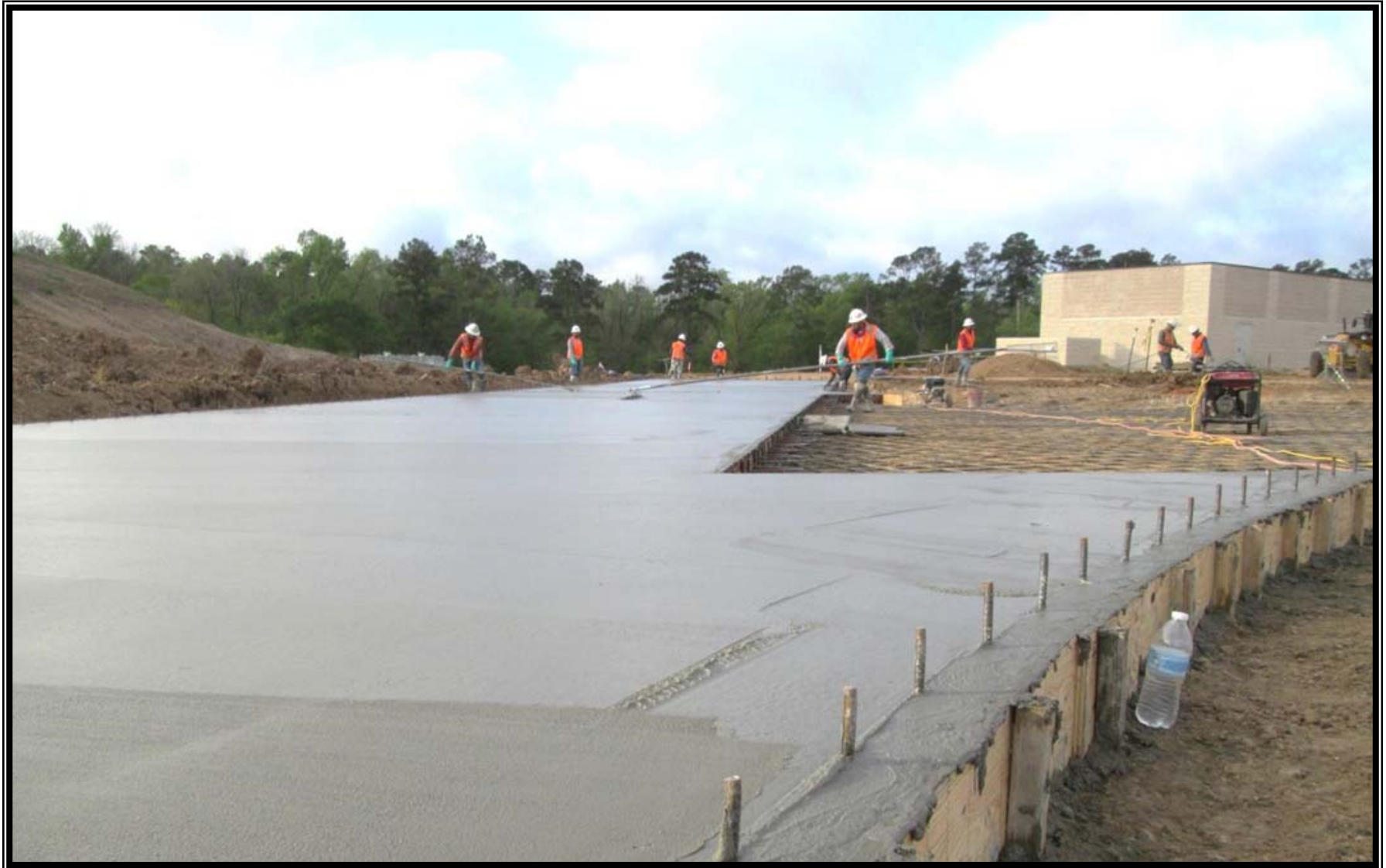
General Site — Roadway installation from main entrance to Power Supply Building
