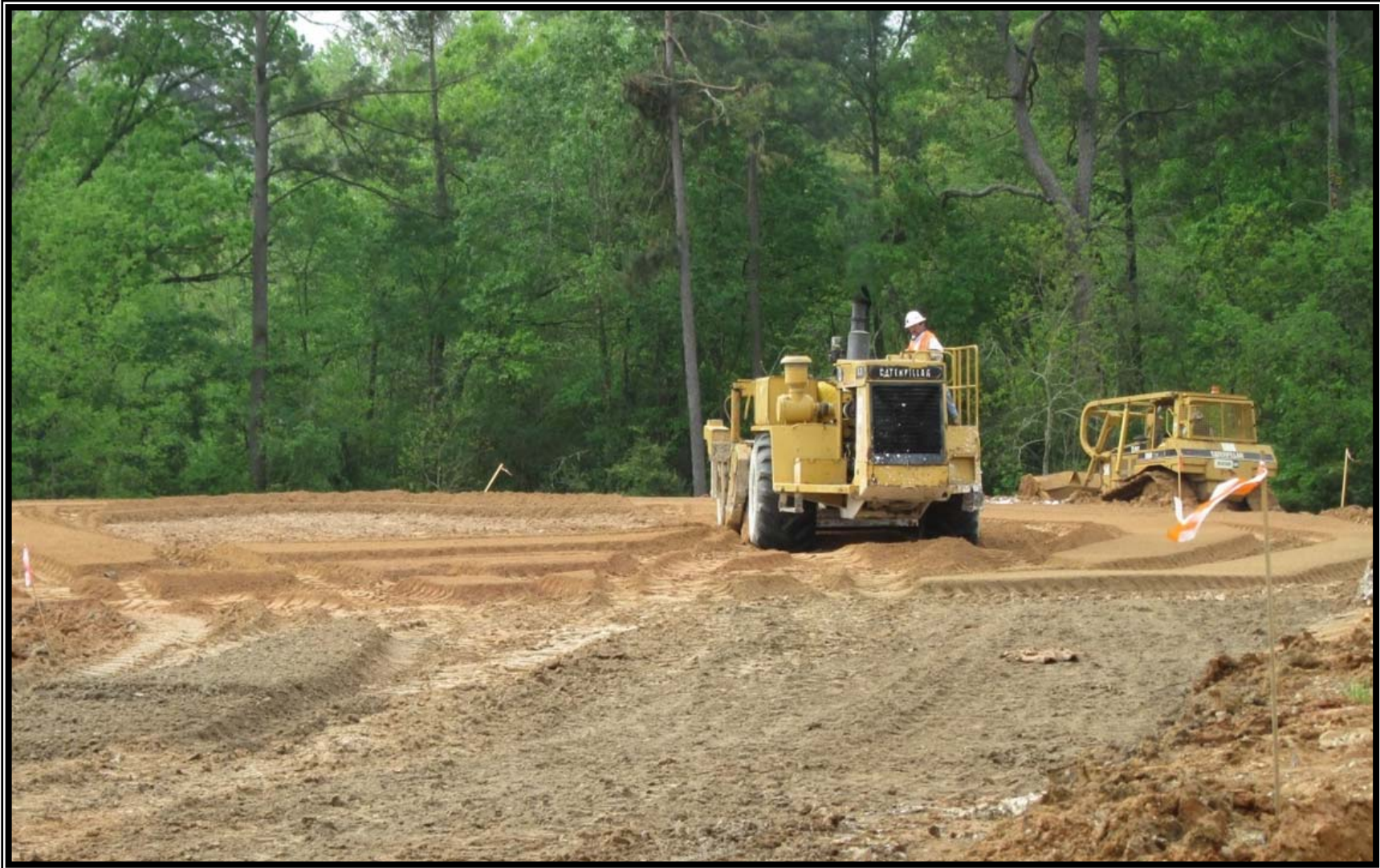
General Site — Stabilization of pavement subgrade
