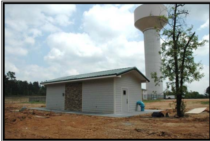
Mid-South Water Receiving Facility
