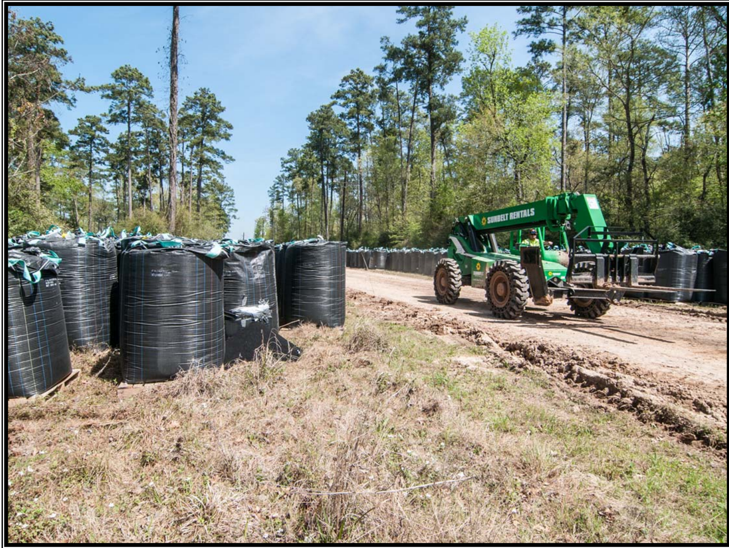
② Granulated Activated Carbon (GAC) — Delivery and storage of 880 tons of GAC
