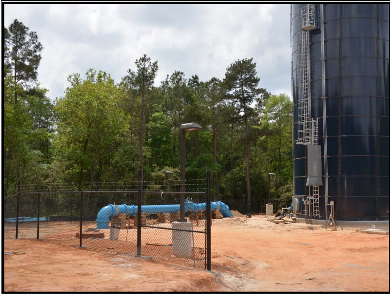
① Final grading, aboveground pipe coating, and fencing completed at Standpipe
