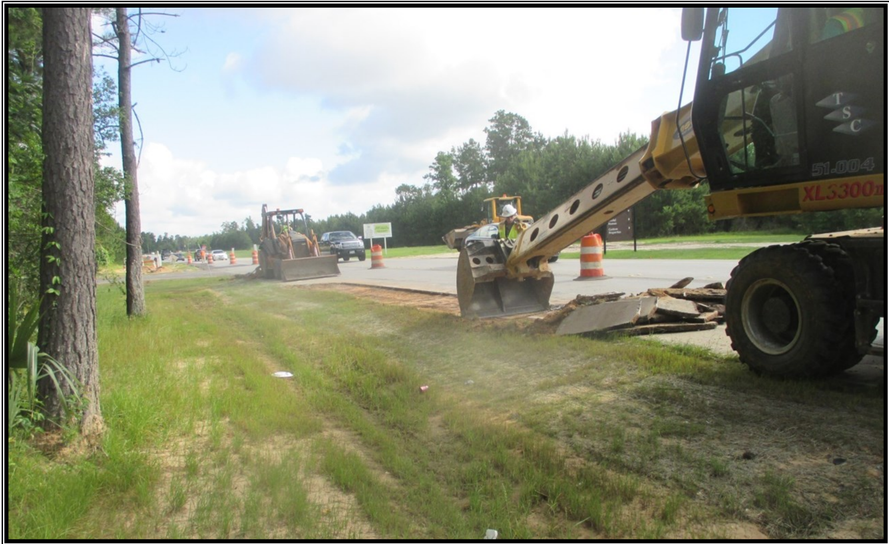
① Segment T2 - Asphalt pavement restoration along Fish Creek Thoroughfare
