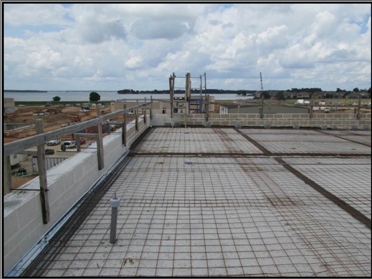
⑥ Preparation of concrete deck placement at the Dewatering Building
