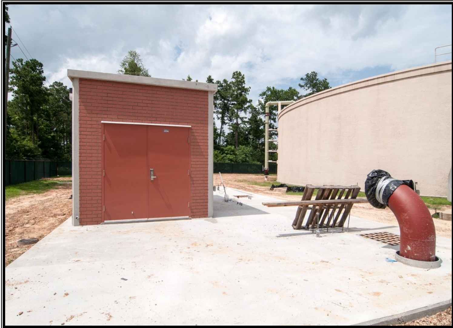
① Surface Water Receiving Facility – South — Metering station at Woodlands Water Plant No. 4
