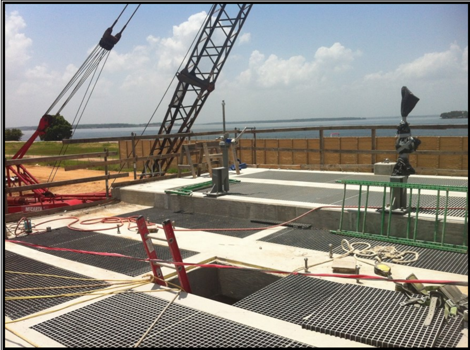
② Grating and sluice gate installation at the Pretreatment Building
