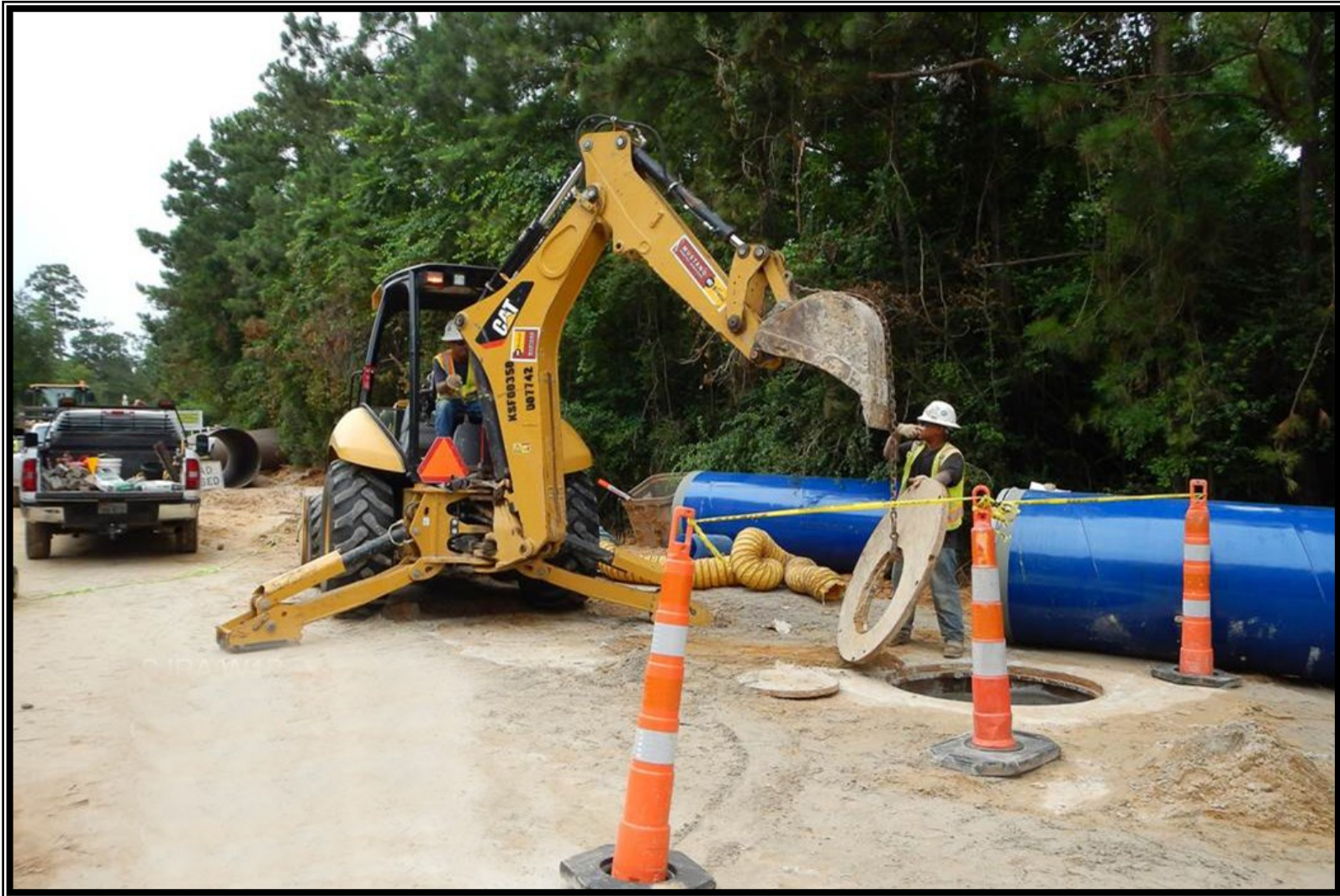
① Segment W1B - Completing manhole installation along Research Forest Drive
