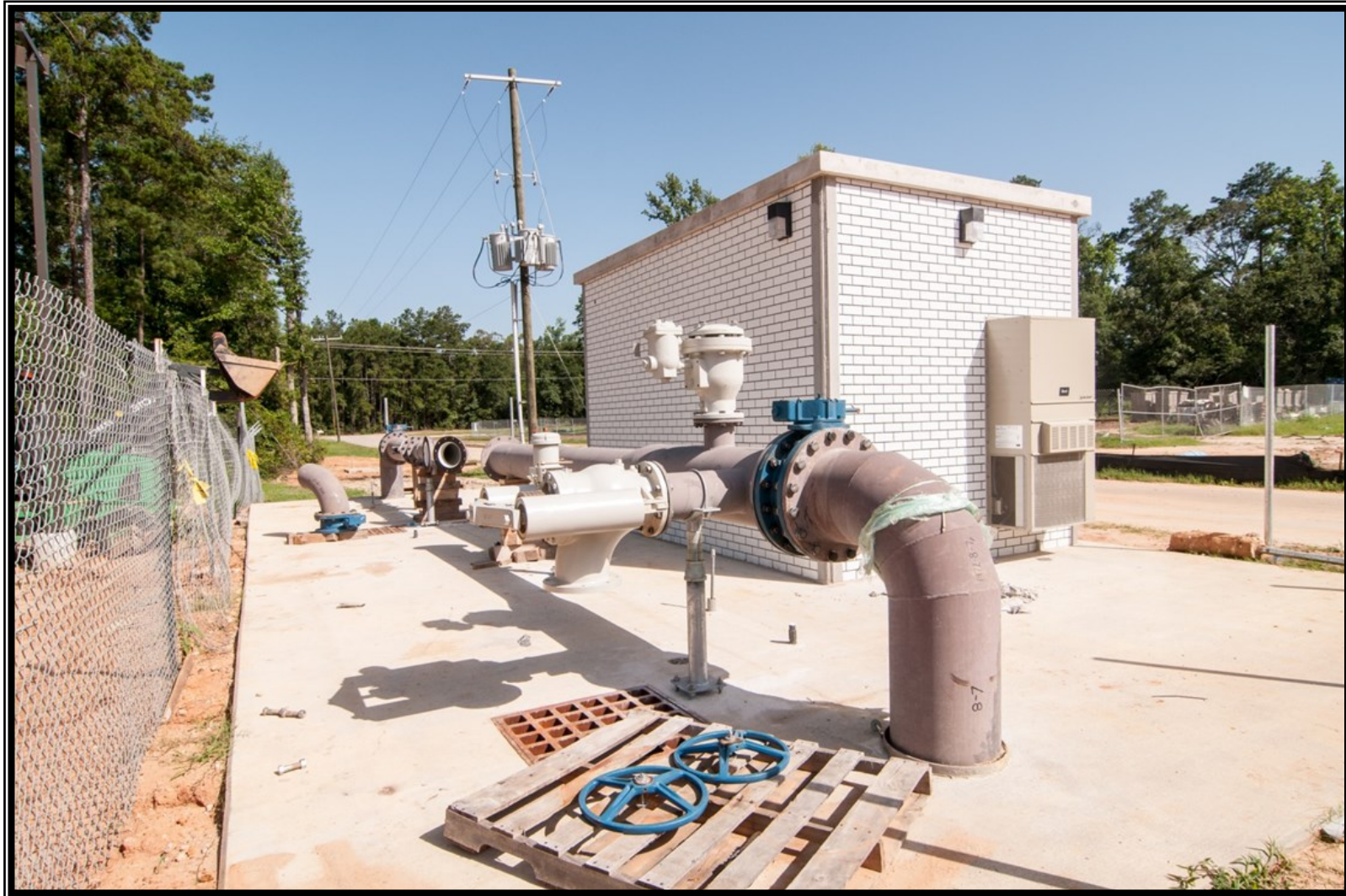
② Surface Water Receiving Facility – North—Piping for metering station at Conroe Water Plant No. 21
