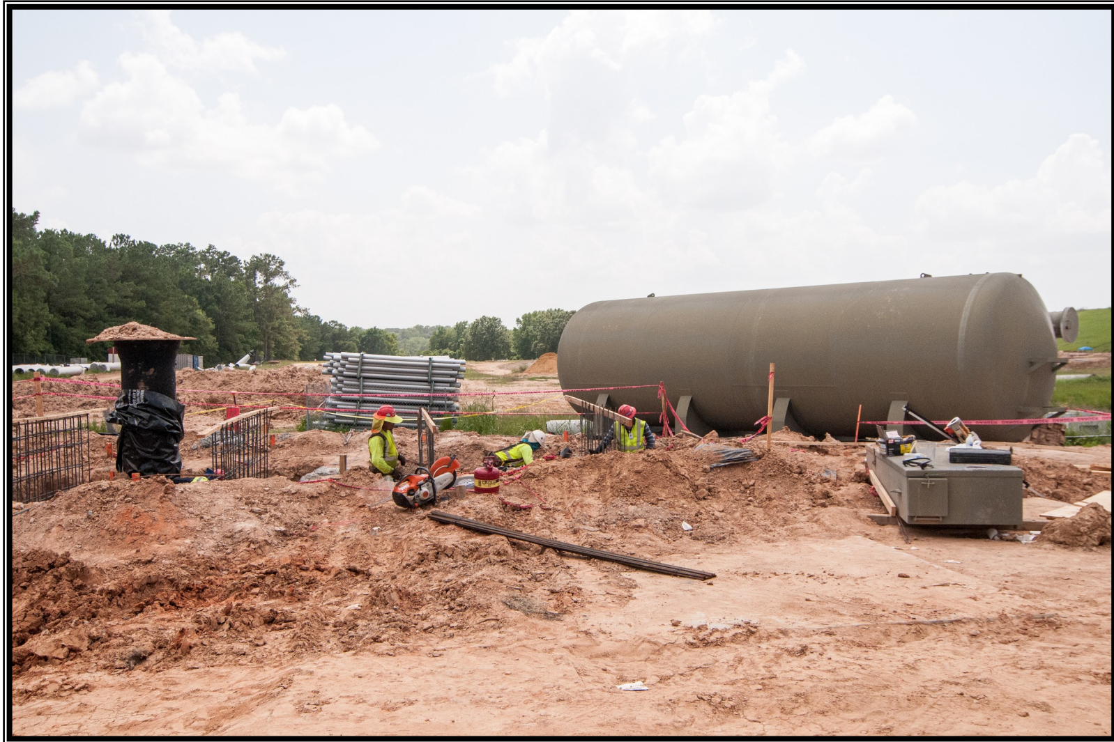
⑤ Installation of hydro-pneumatic pump at the High Service Pump Station
