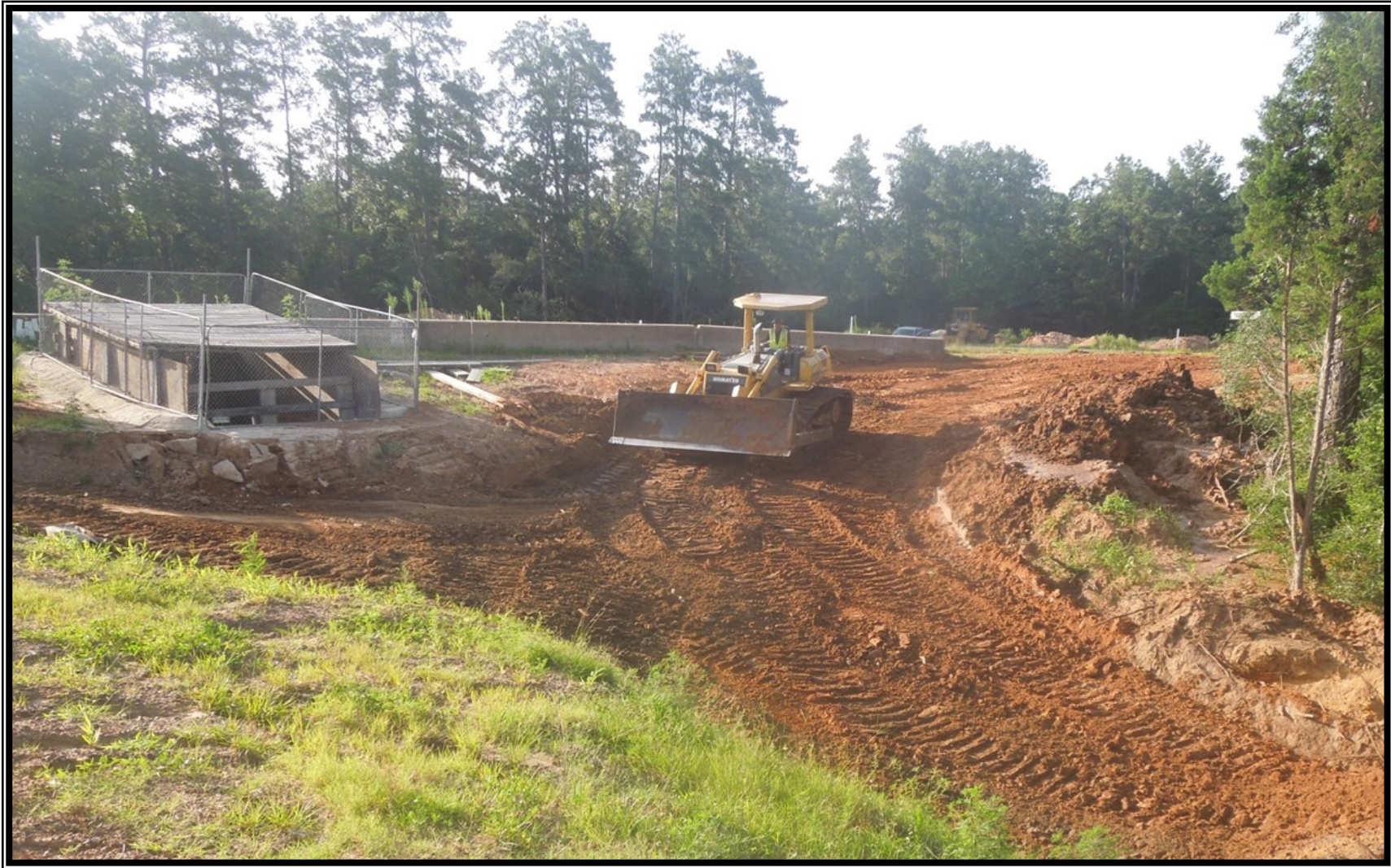
① Segment C4—Bore pit and site grading along FM 830 at I-45 frontage road
