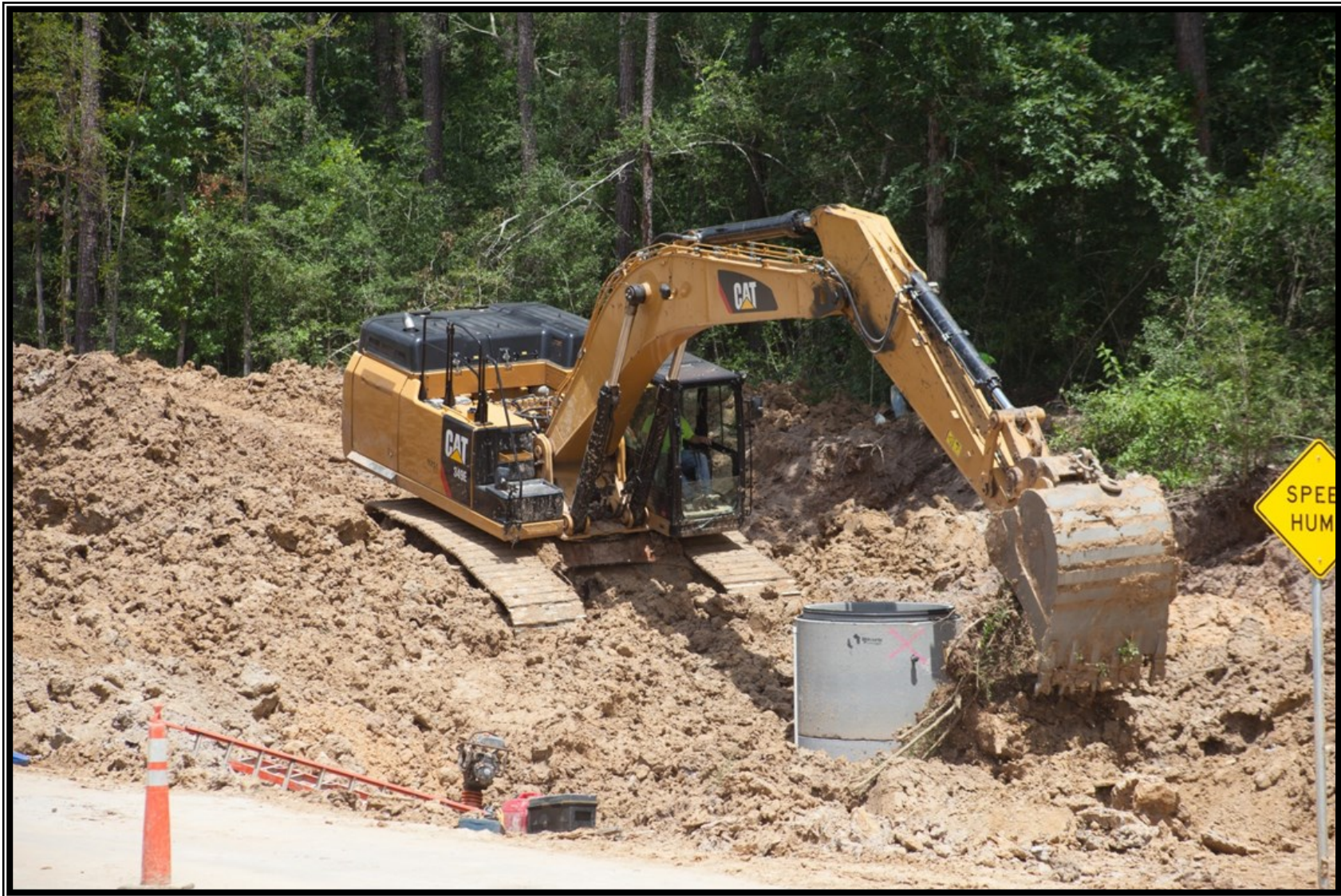
① Segment C1A - Manhole installation along GRP Access Road
