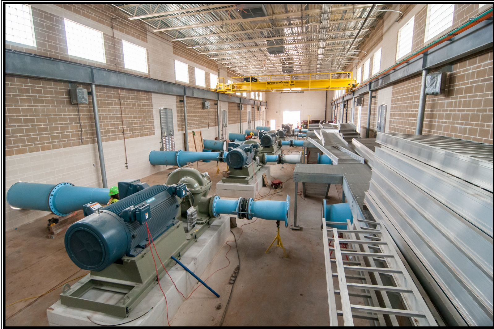
⑤ Installation of finished water discharge piping at the High Service Pump Station
