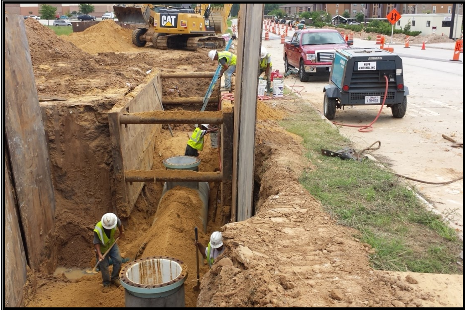
① Segment W1A—48-inch open cut pipe installation along Research Forest Drive
