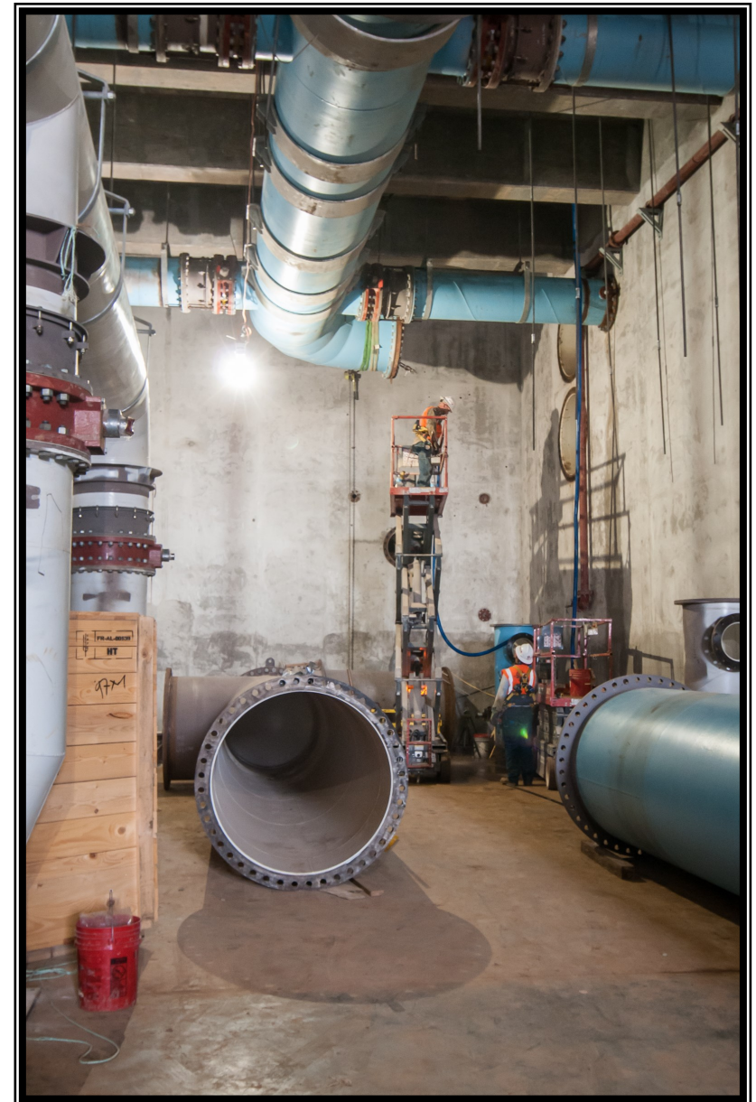
Left: HVAC equipment at Operations Building at SWF Above: Assembly of pipes at Granular Activated Carbon Building at SWF
