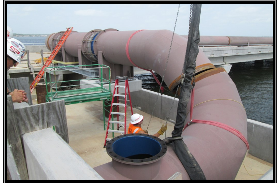
① Delivery, welding and installation of 48-inch pipe at Raw Water Intake and Pump Station
