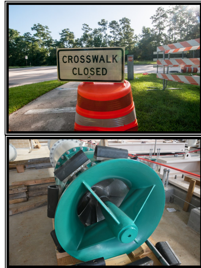
Top: Construction signage at Transmission Line Segment W2A
