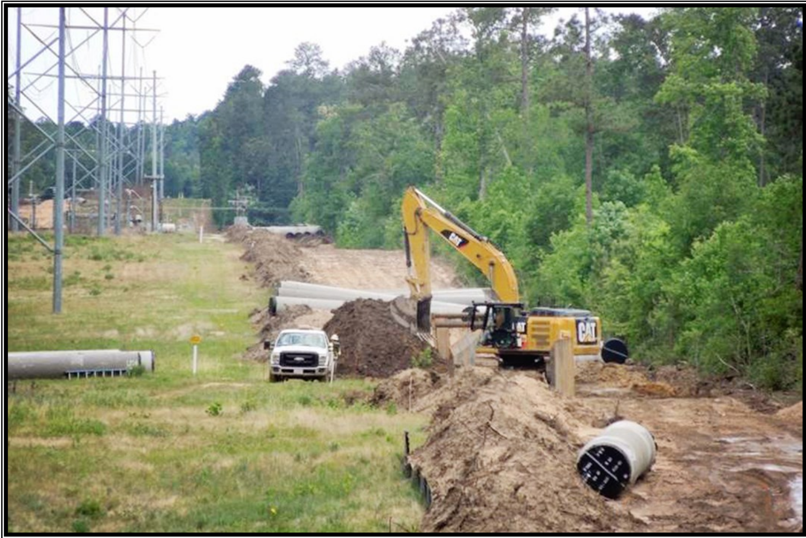
① Segment C2— 36--inch open cut pipe installation along Entergy corridor
