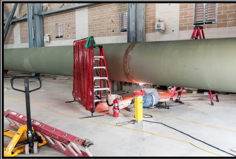
① Delivery, welding and installation of 48-inch pipe at Raw Water Intake and Pump Station
