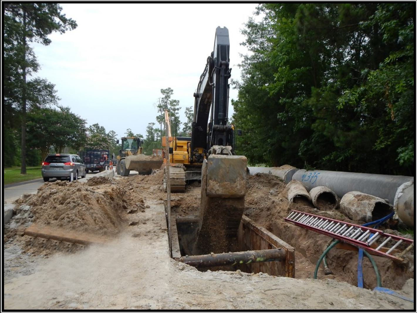
① Segment W2A - Backfilling trench box for 42-inch pipe along Research Forest Drive
