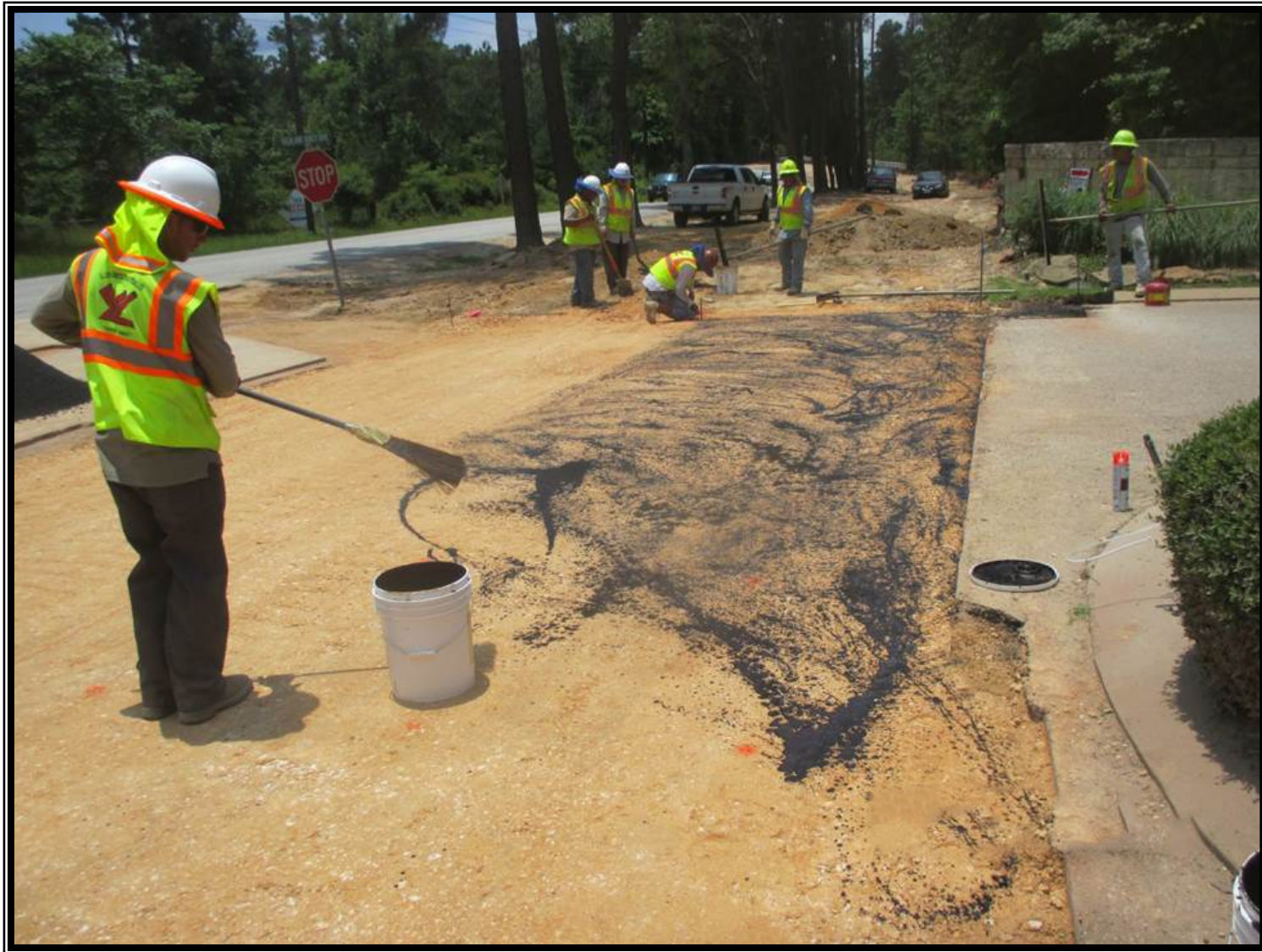
① Segment T1 - Pavement restoration along McCaleb Road at Highland Ranch Drive
