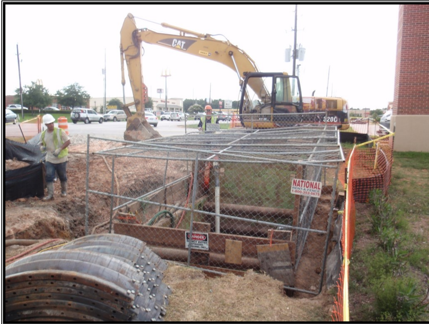
① Segment T3—54-inch trenchless pipe installation along FM 2978
