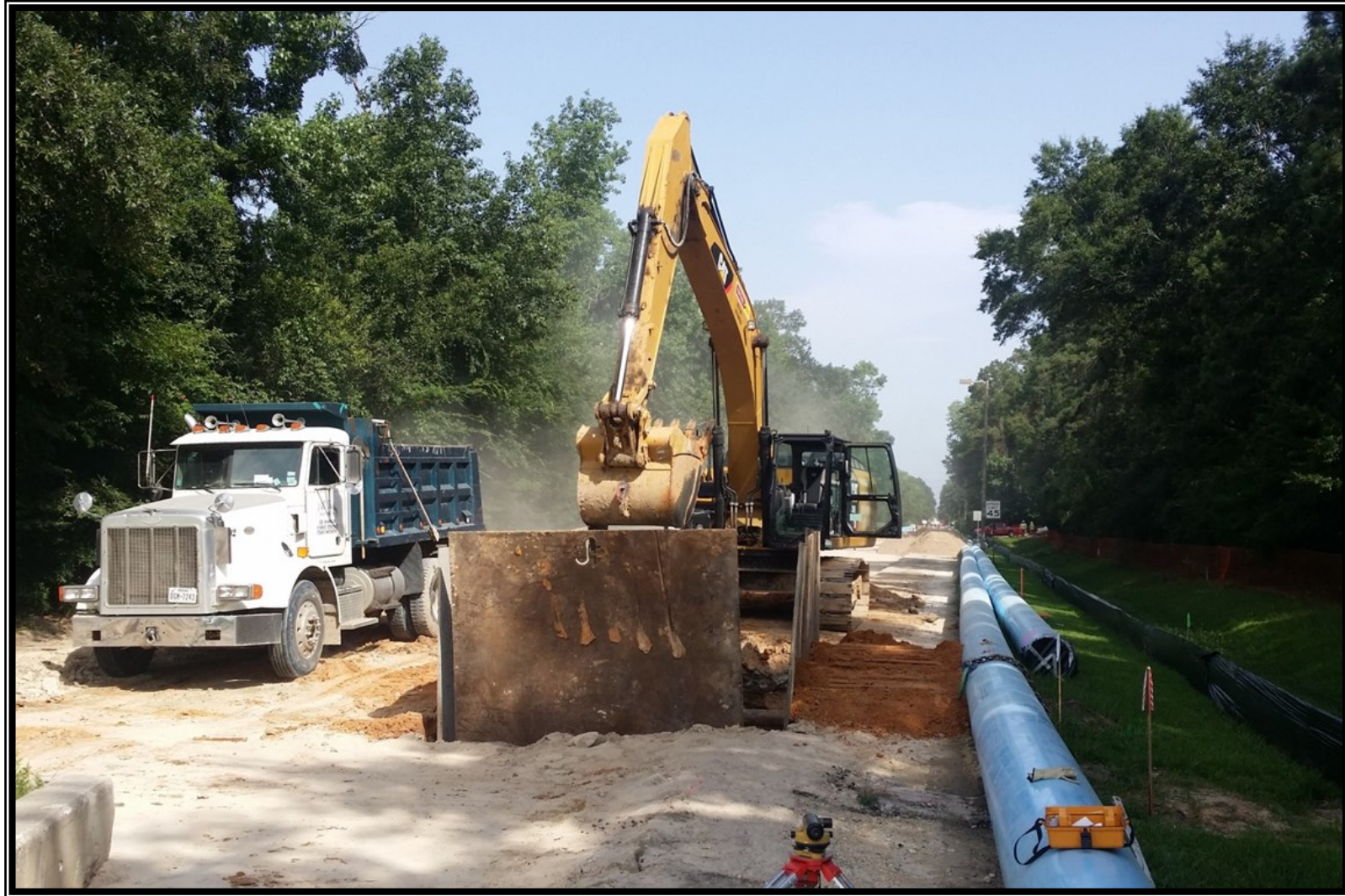
❶ Segment W3A - Bore pit excavation for 24-inch trenchless pipe installation along Grogans Mill Road
