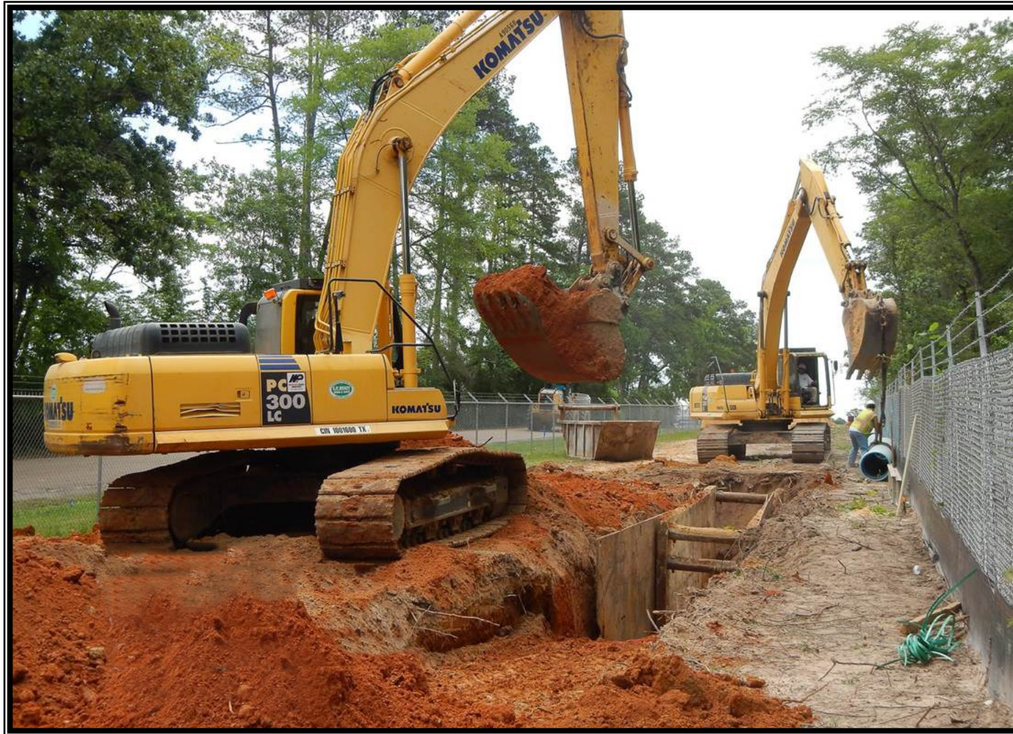
❶ Segment C3— 20-inch open cut pipe installation along Silver Springs Road
