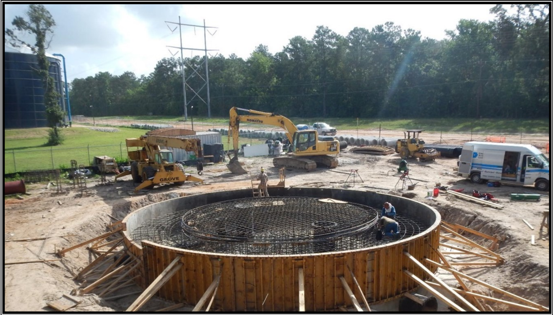
① Surface Water Standpipe—Standpipe foundation reinforcing steel and formwork installation
