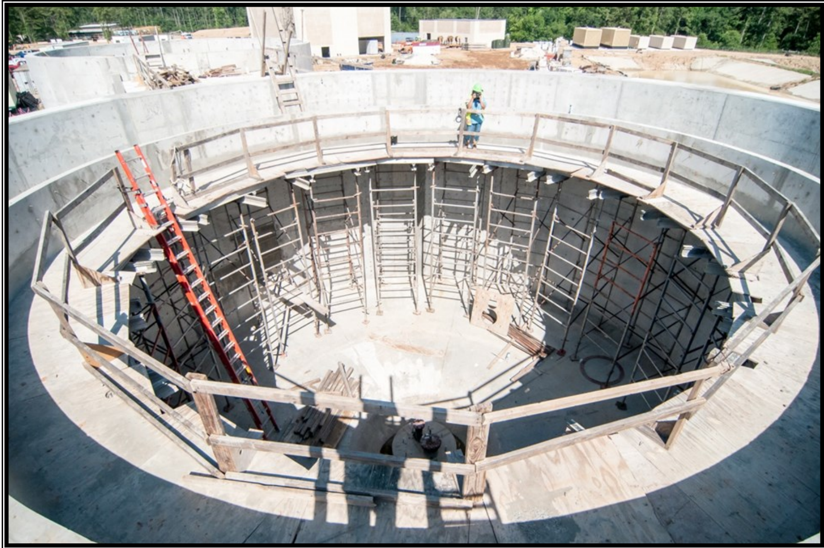
⑦ Shoring for lauder installation at the Sludge Thickeners
