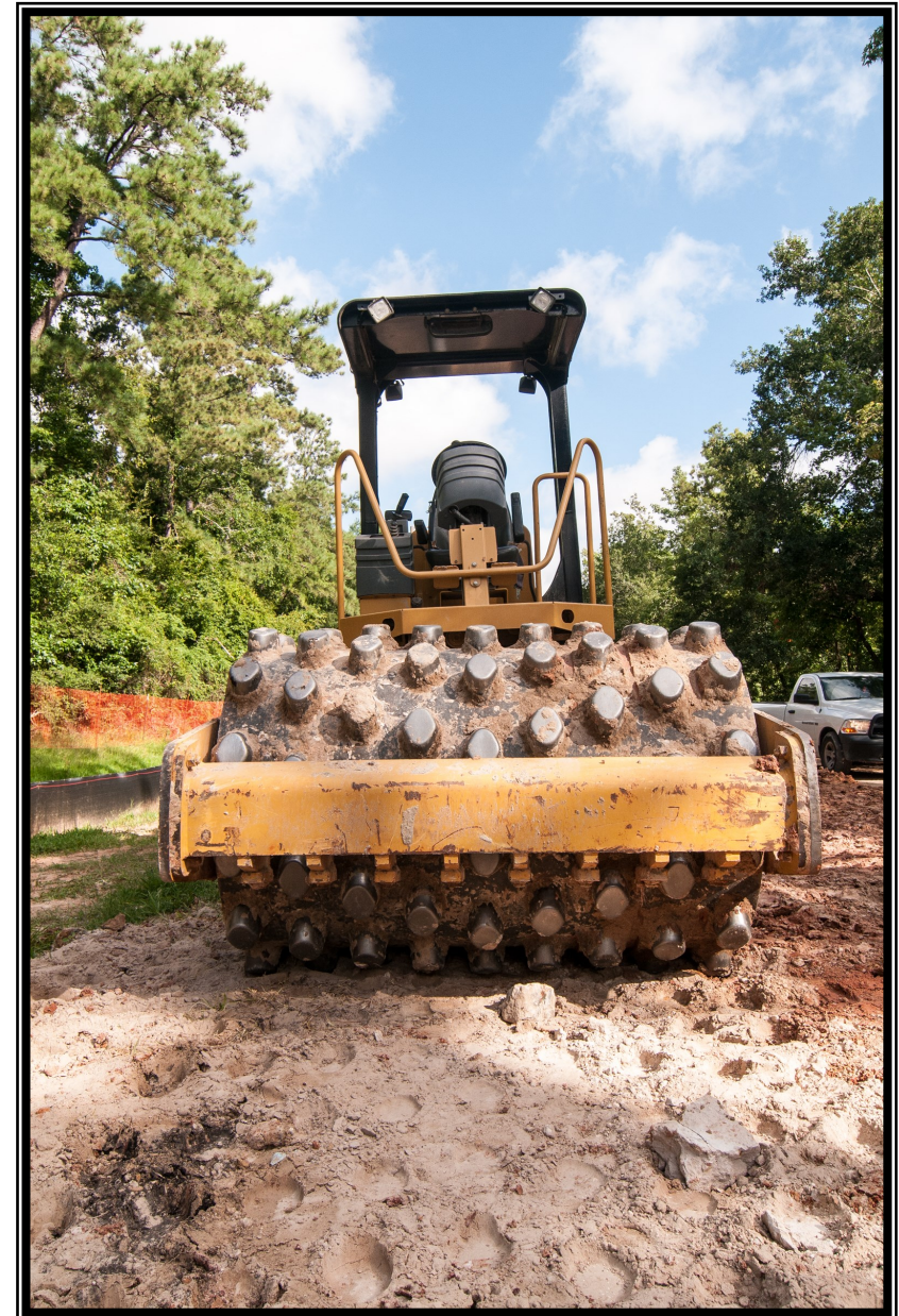
Left: Pump at Raw Water Intake and Pump Station at SWF Above: Construction activities at Transmission Line Segment W3A
