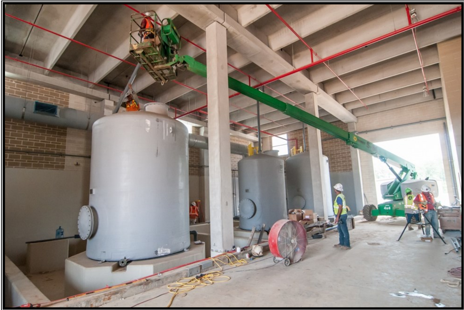
④ Chemical tank and vent pipe installation at the Chemical Storage Facilities
