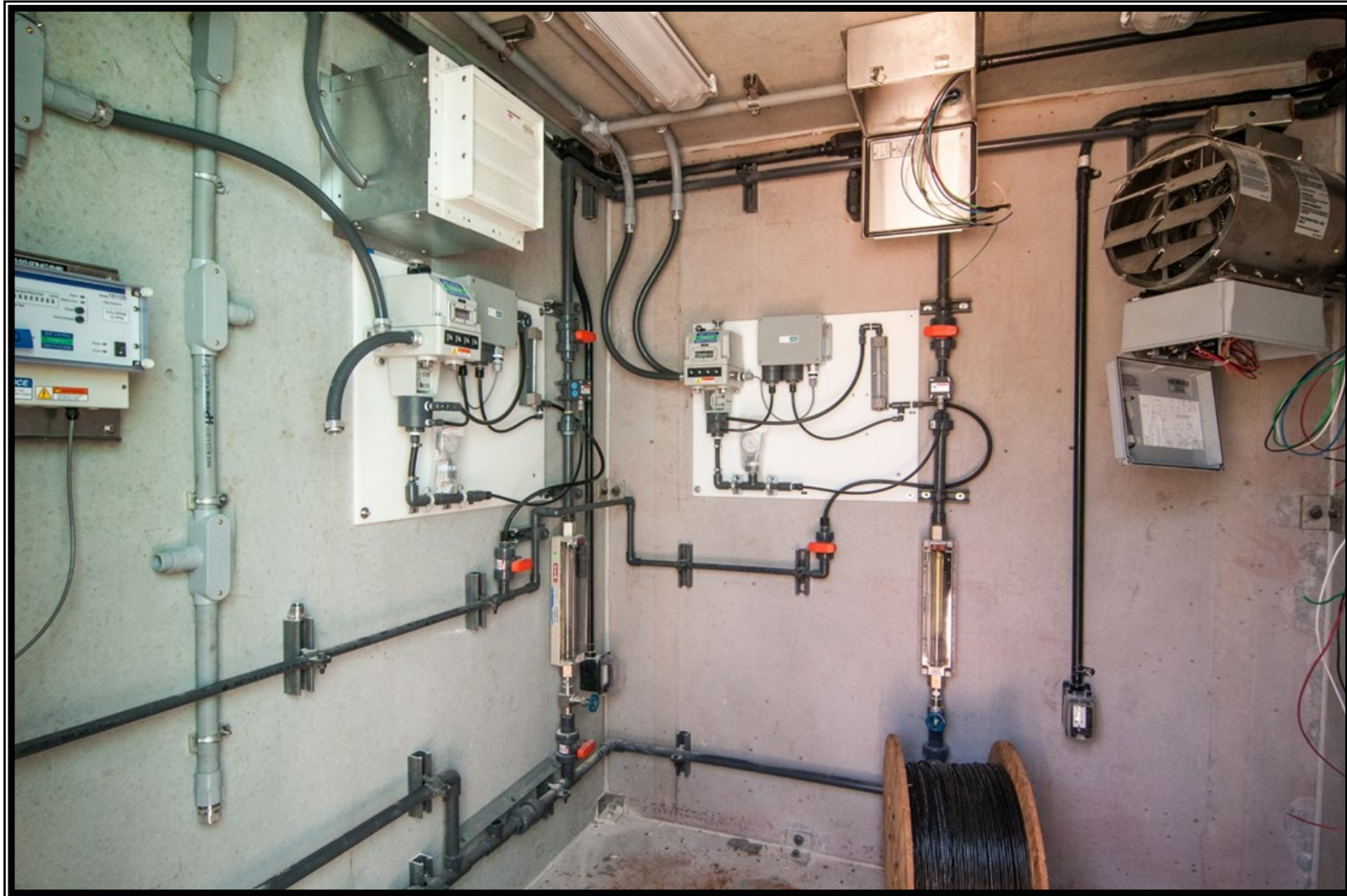
① Surface Water Receiving Facility – North—Interior view of metering station at Conroe Water Plant No. 20
