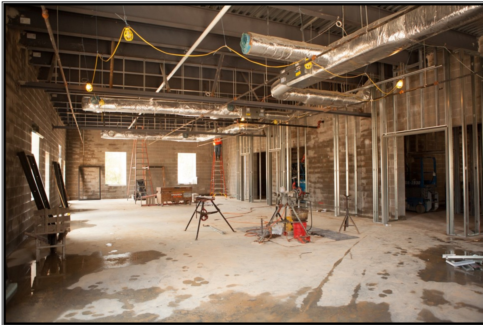
⑨ Wall Framing Installation at the Operations Building
