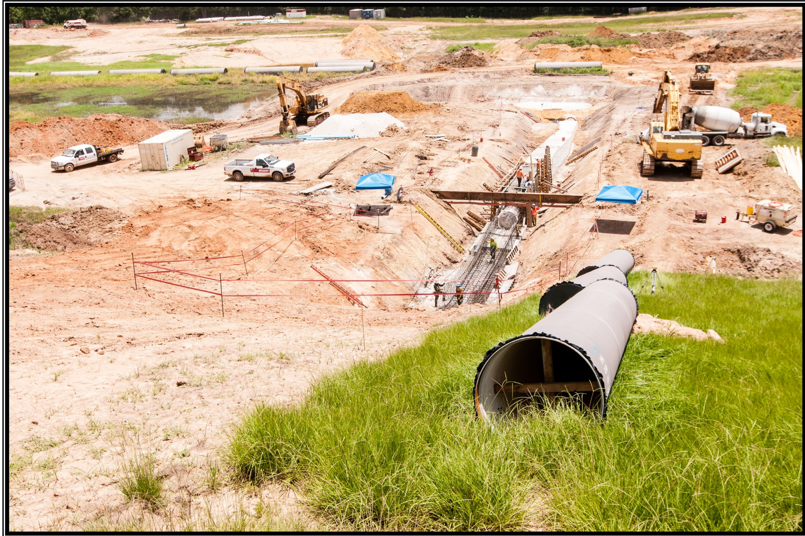
❶ 48-inch pipe installation at toe of dam at Raw Water Intake and Pump Station
