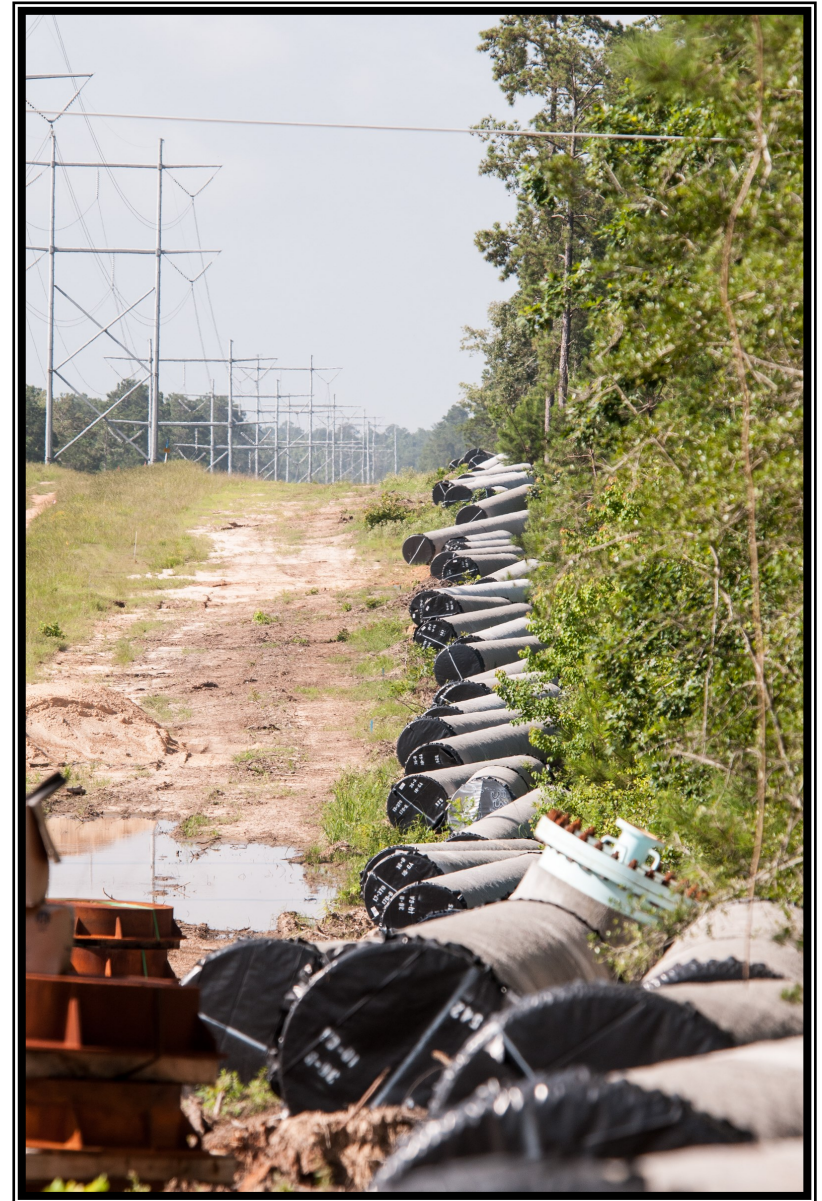
Staging area along Entergy easement at Transmission Line Segment C2
