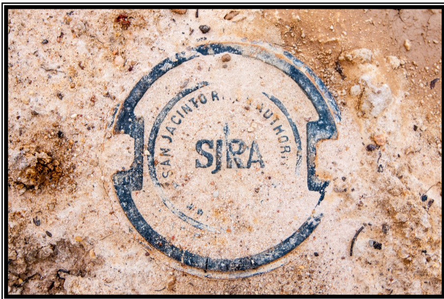
Valve cover at Surface Water Receiving Facility-North in City of Conroe
