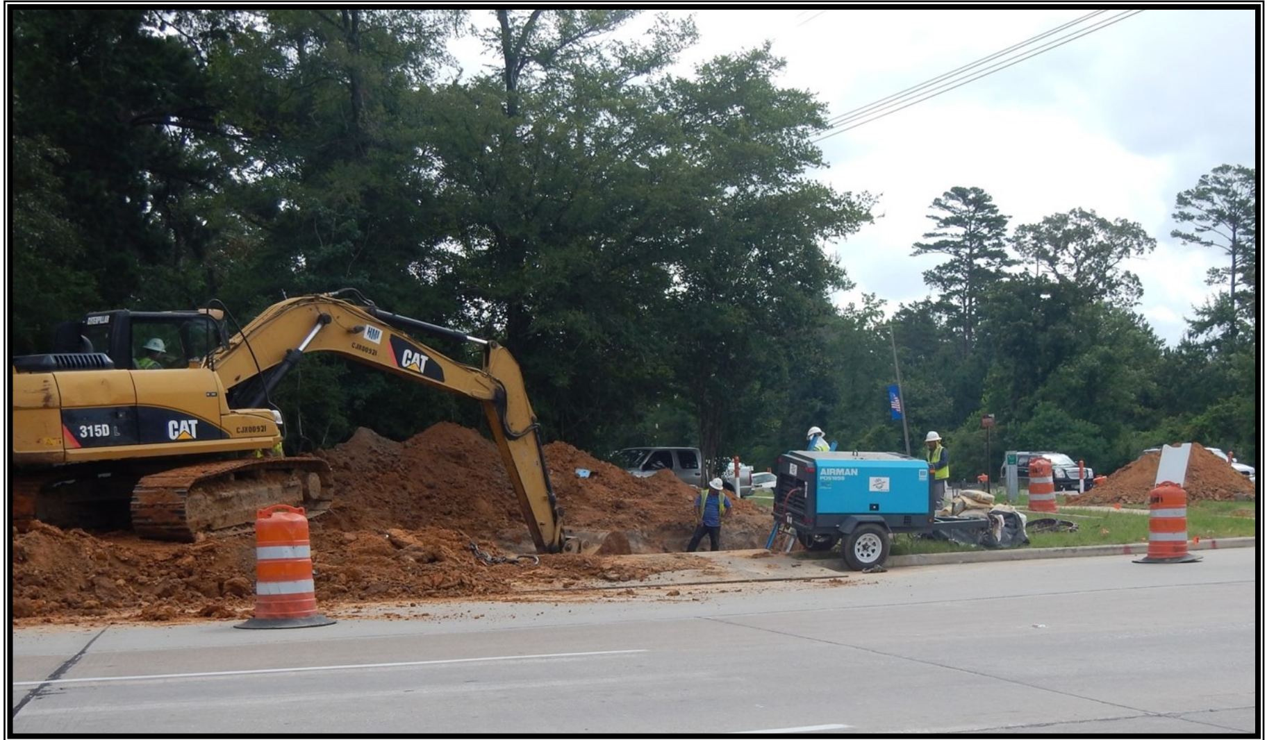
① Segment W4 - 24-inch pipe connection at Gosling Road and Research Forest Drive
