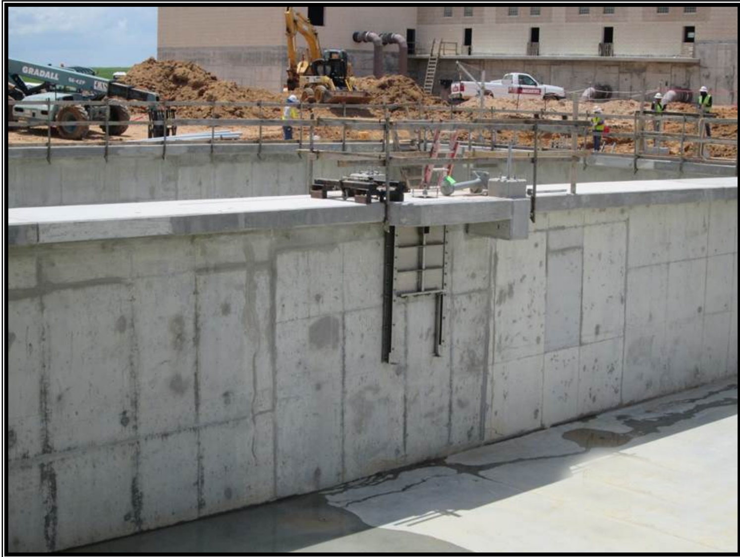
⑧ Sluice gate installation at the Backwash Equalization Basin
