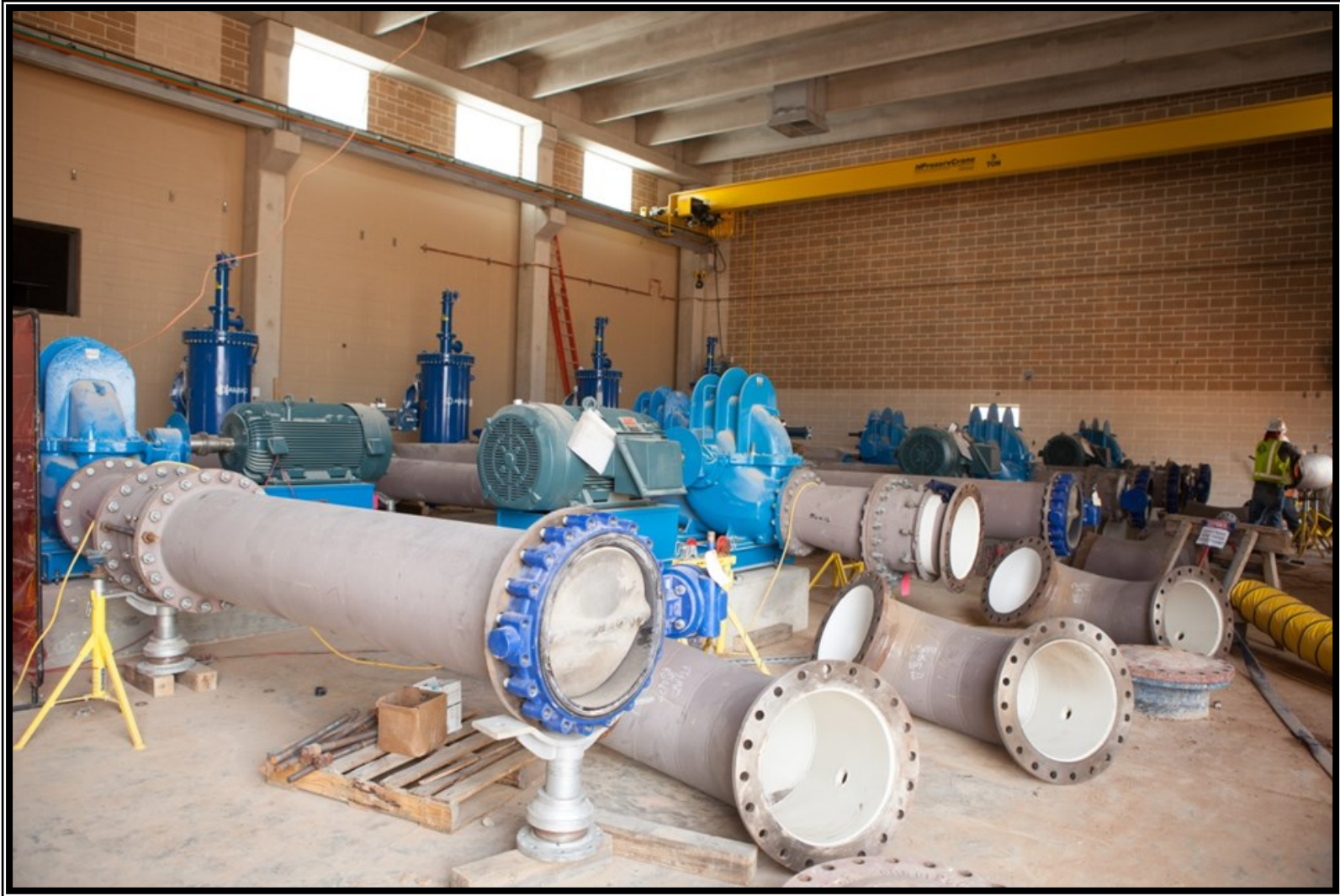
③ Feed pump and piping installation at the Membrane Building
