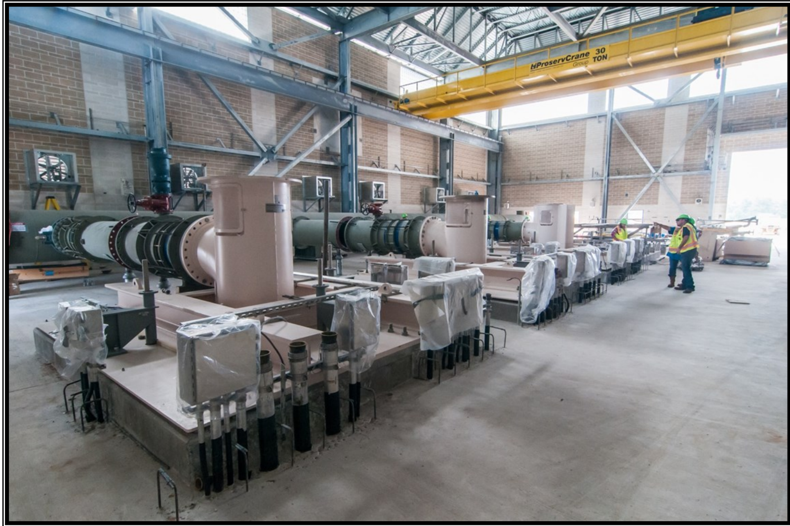
❶ Pump assembly and slide gate installation in the Raw Water Intake and Pump Station
