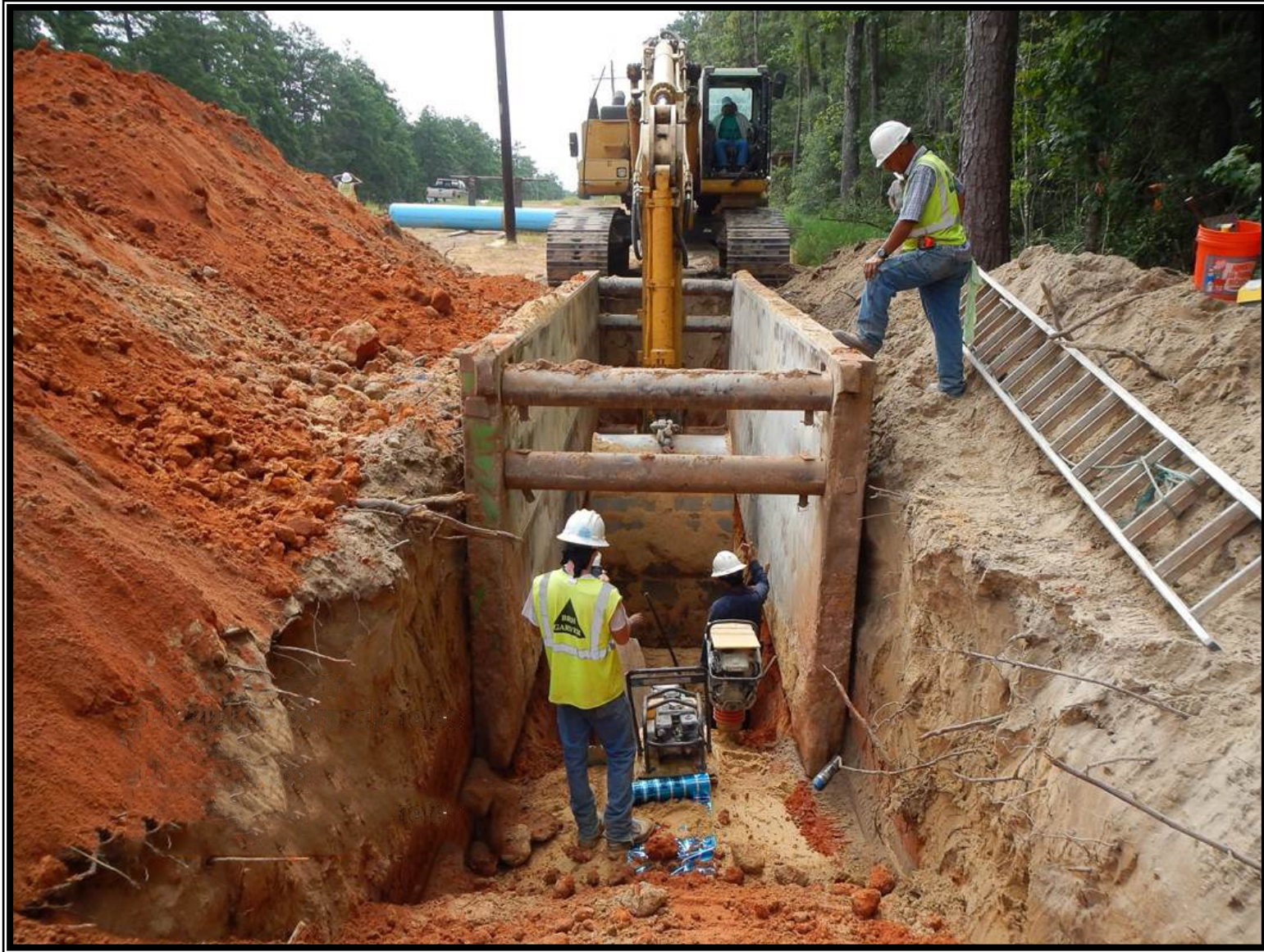
① Segment C4—20-inch waterline installation along FM 830
