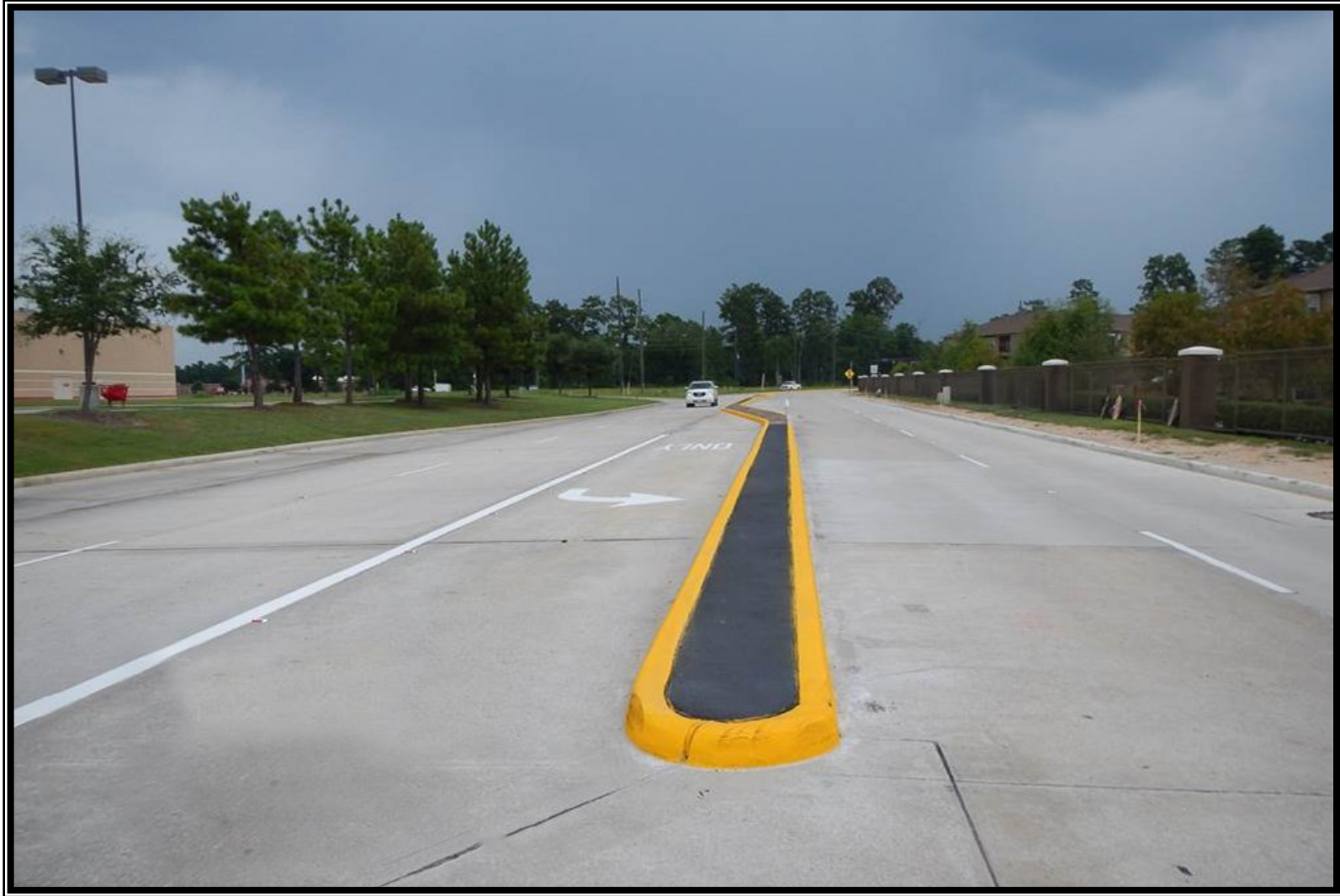
① Segment W1A—Traffic restoration along Research Forest Drive at FM 2978
