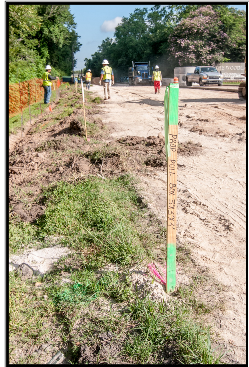
Construction staking along Segment W3A site
