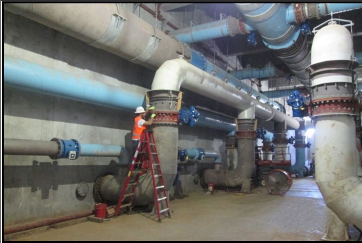
③ Carbon contactor process piping installation at the Granulated Activated Carbon Building
