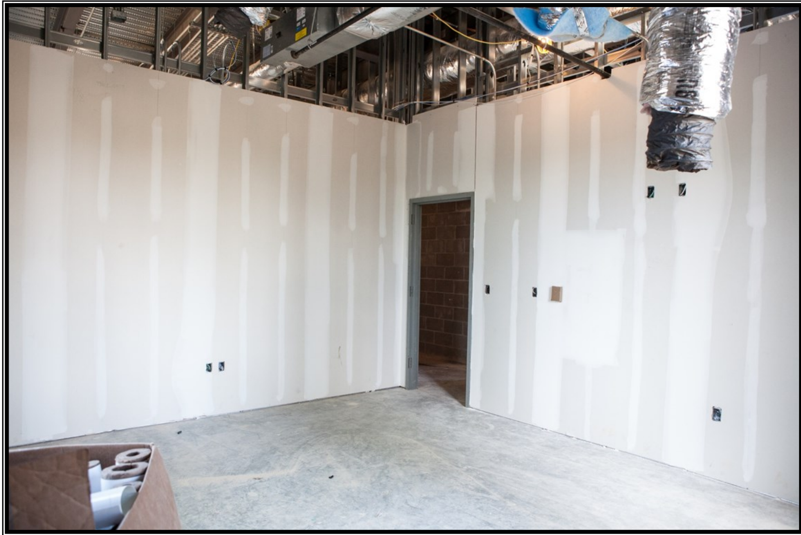
① Drywall installation and finishing in the Operations Building
