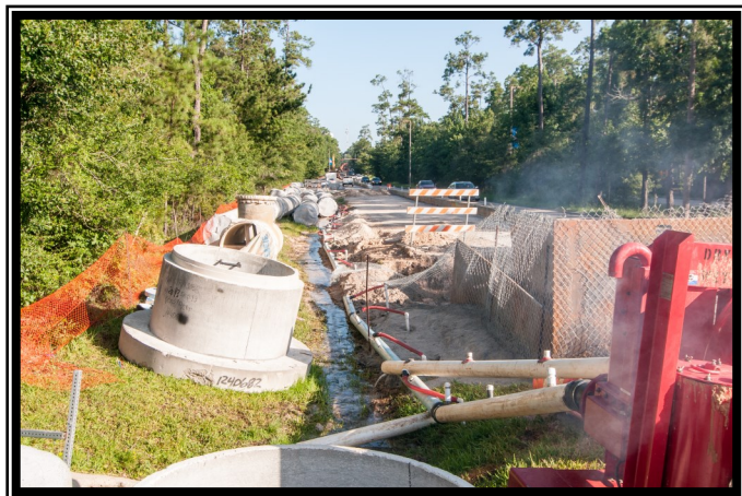
Well-pointing at Segment W2A—The Woodlands High School
