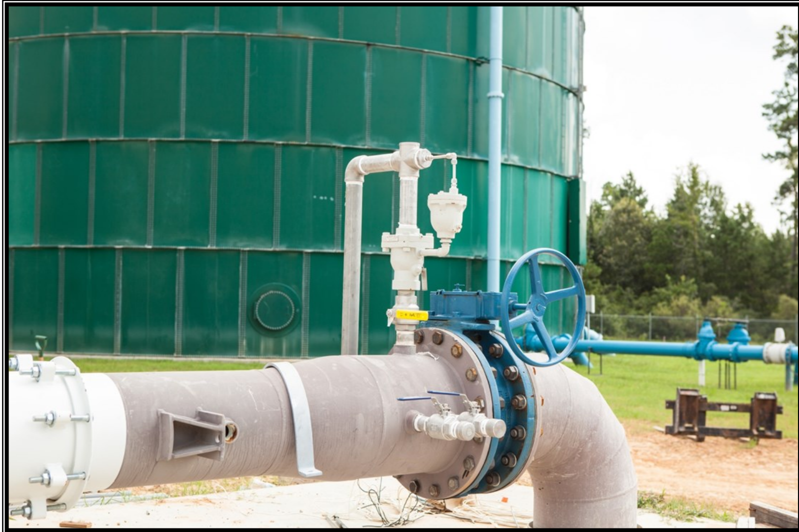
❶ Surface Water Receiving Facility – North— Flow Control Pressure Station assembly at Conroe Water Plant No. 20
