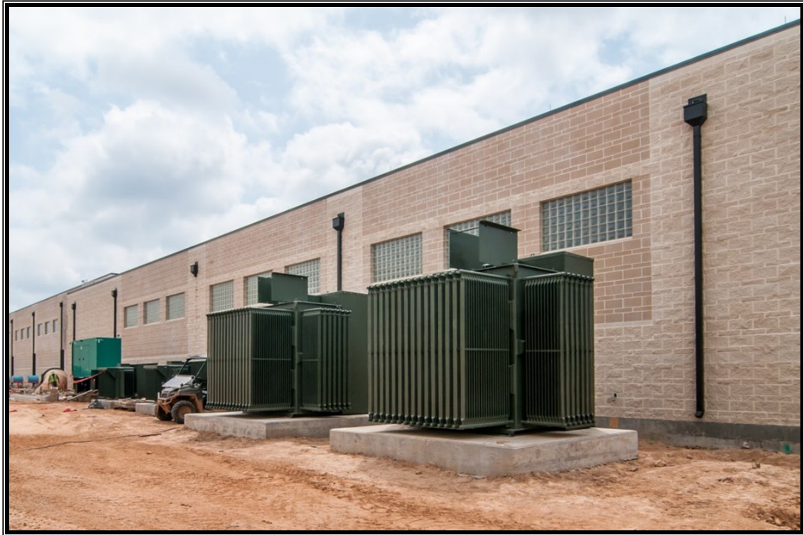
⑤ Transformer installation (12470 V : 4160 V) at the High Service Pump Station
