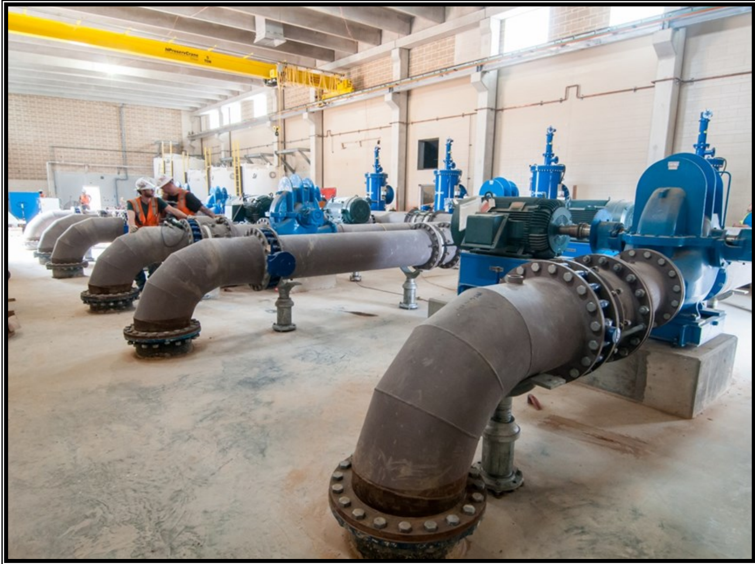
② Feed pump and piping installation at the Membrane Building
