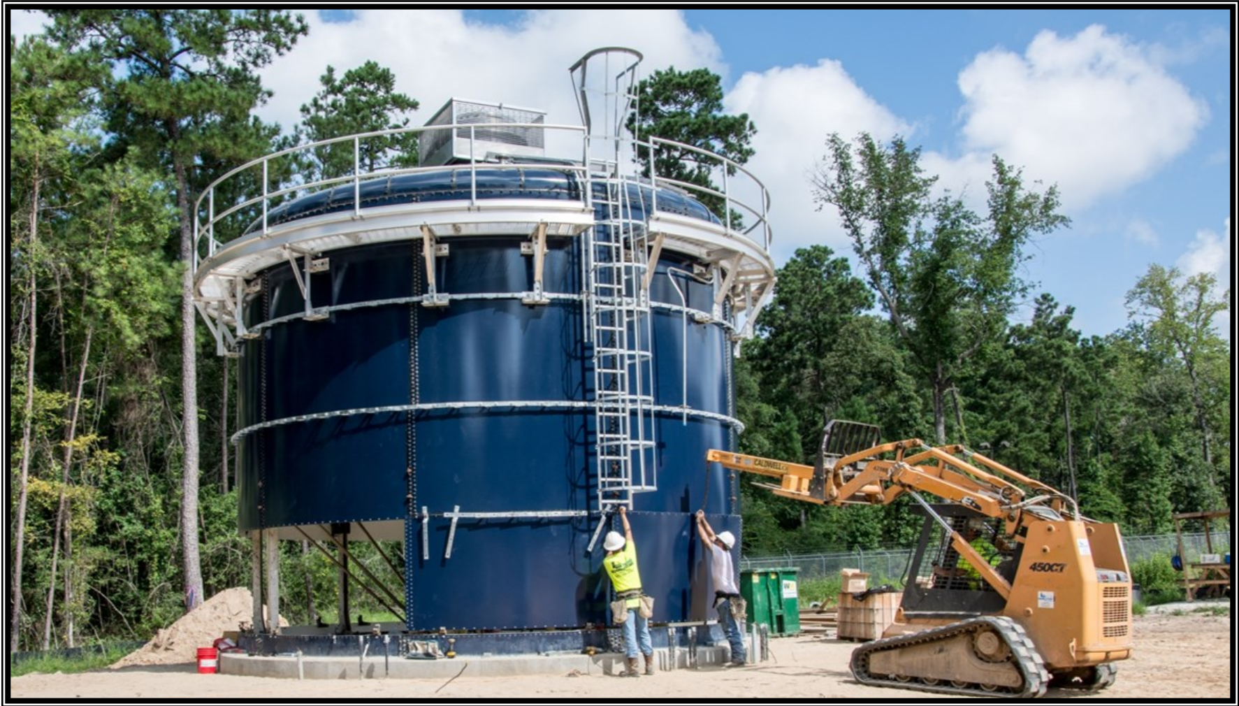
❶ Surface Water Standpipe—Standpipe tank panel installation at Conroe Water Plant No. 21
