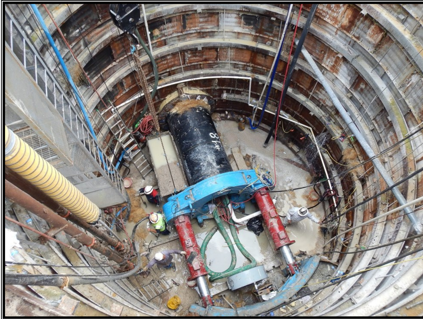
❶ Segment W2B - Bore pit and tunneling bore machine installation for Woodlands Waterway crossing
