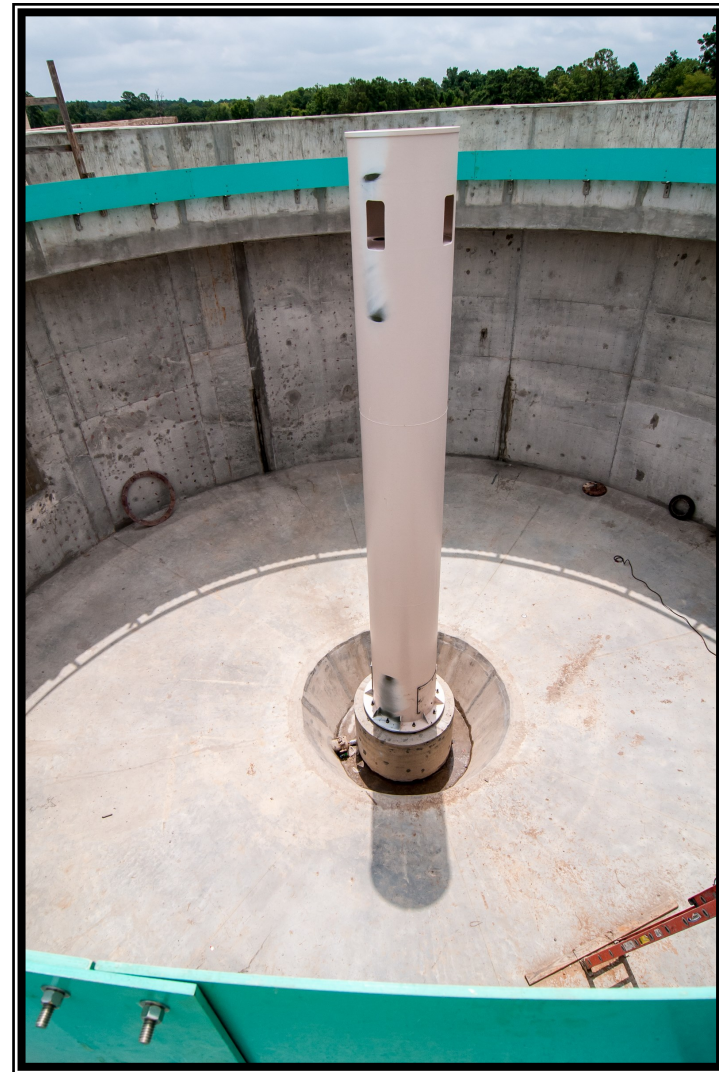
Center column of sludge thickener at the Surface Water Facility
