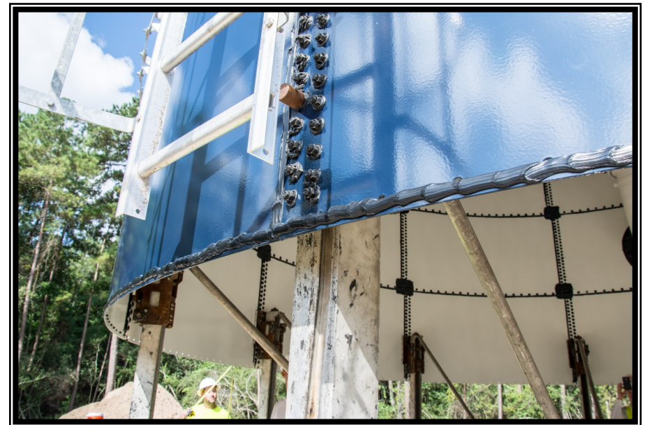
Left: Pumps and filtration at the Membrane Building Above: Standpipe tank panel installation at Conroe Water Plant No. 21
