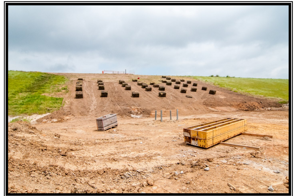
Resodding on slope of dam below the Raw Water Intake
