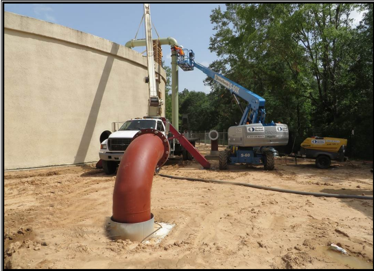
① Surface Water Receiving Facility – South — Riser pipe installation at Woodlands Water Plant No. 1
