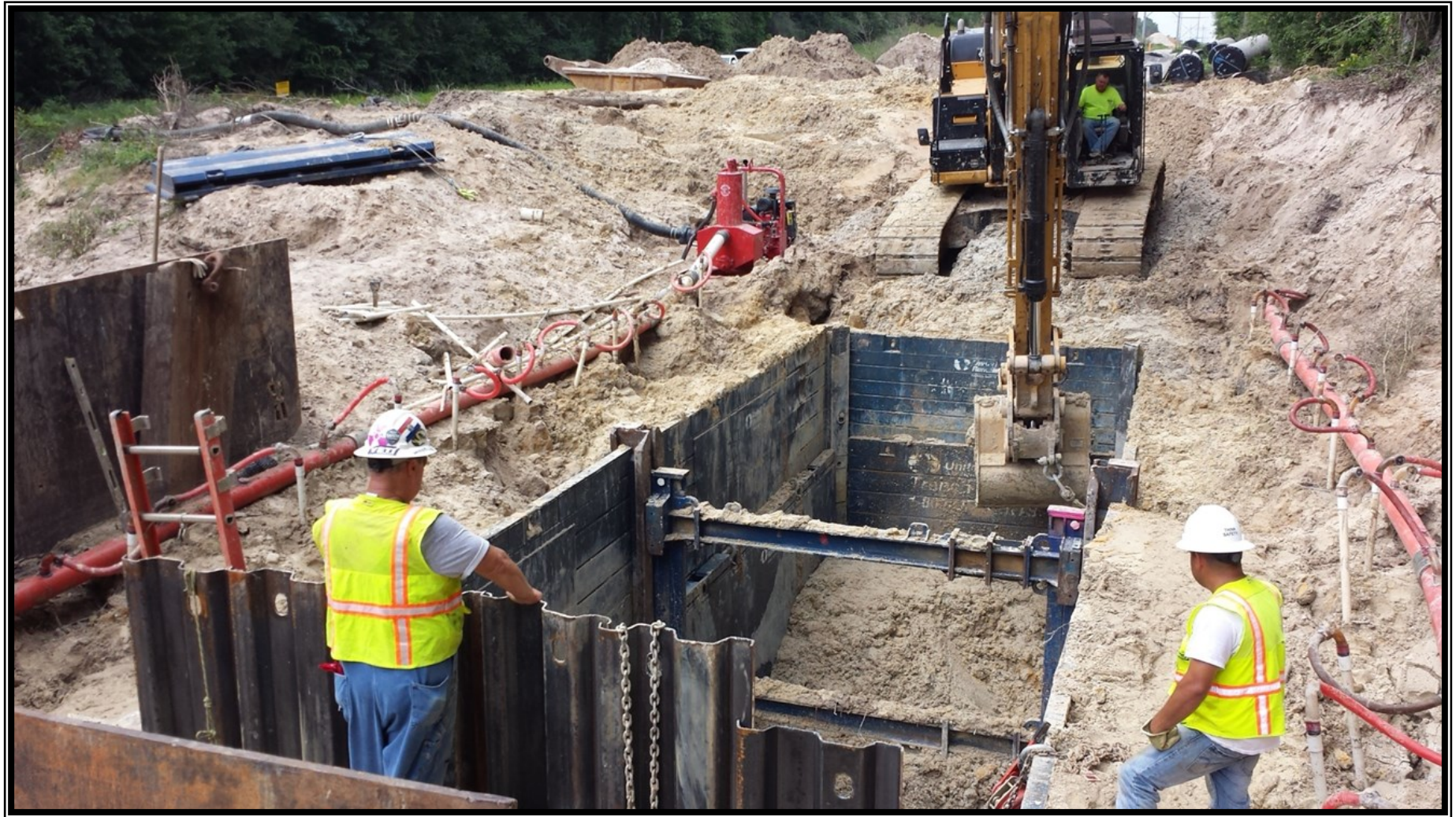
❶ Segment C2— Tunnel bore pit installation along Entergy corridor
