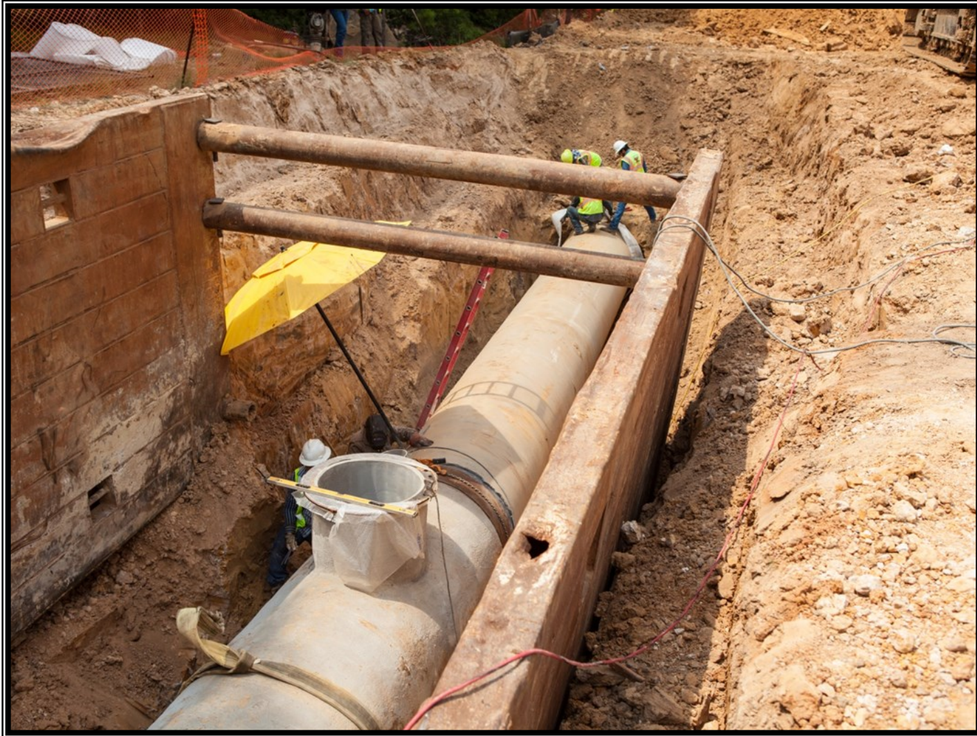
① Segment T3— 54-inch pipe installation along Sendera Ranch Road
