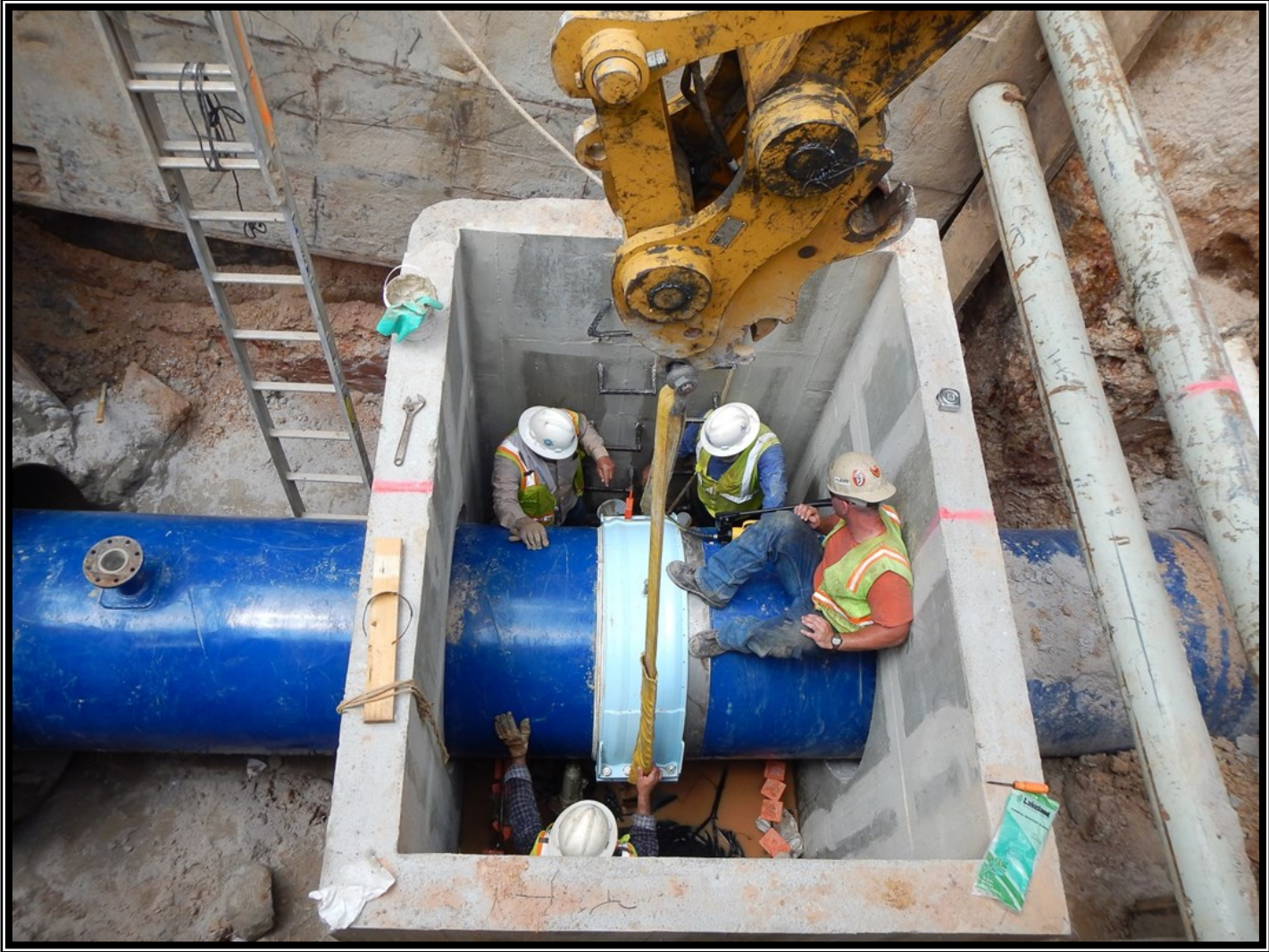
❶ Segment W2A— Expansion joint installation at Big Barn fault crossing
