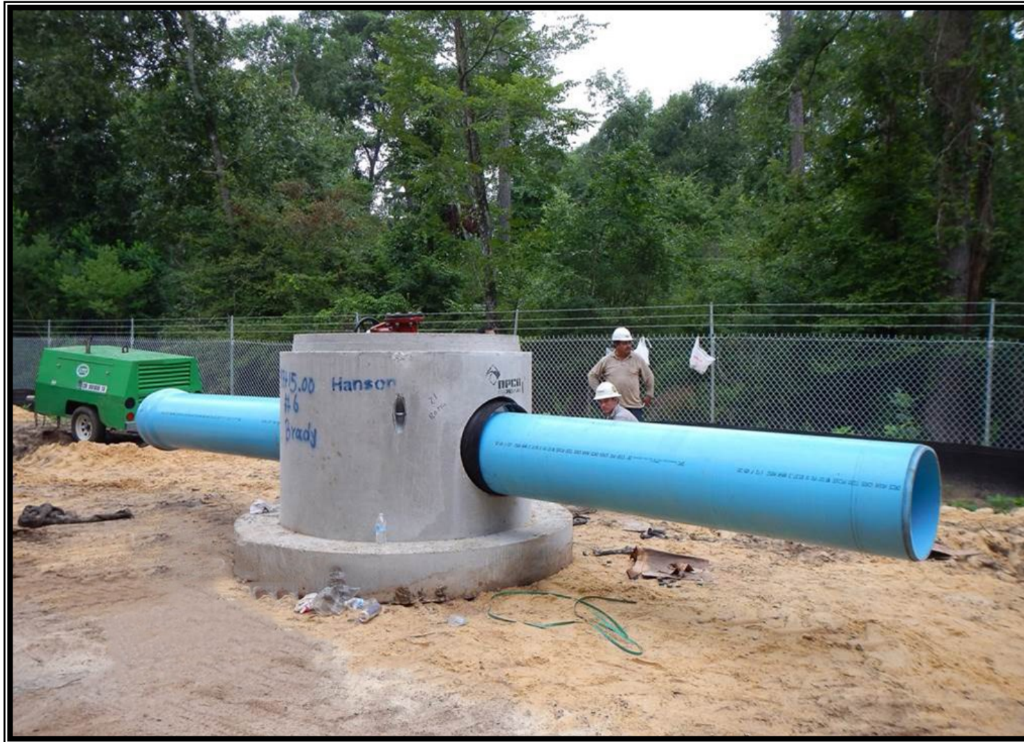
① Segment C3— Manhole installation preparation along Silver Springs Road
