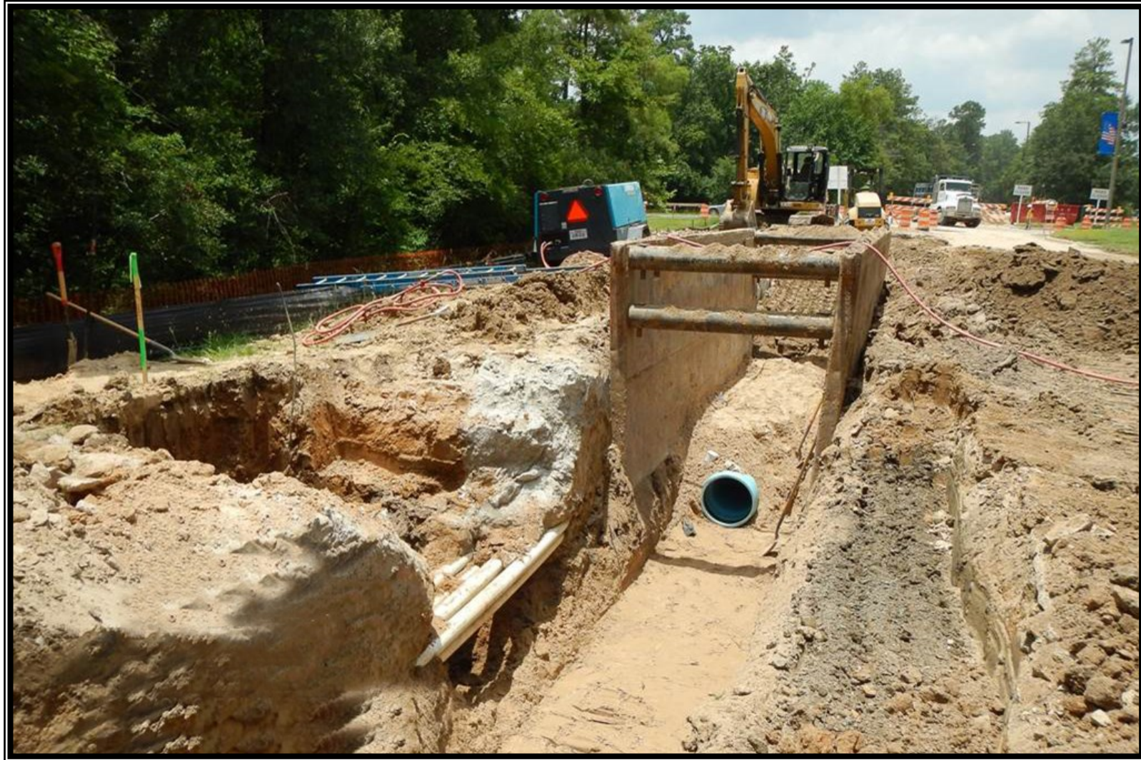
① Segment W3A - 20-inch pipe installation along Grogans Mill Road
