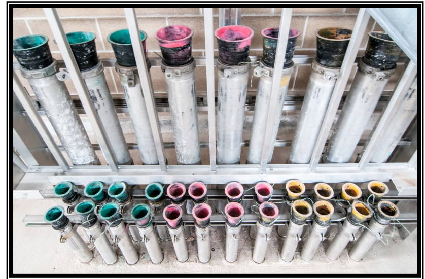
Electrical conduit at Raw Water Intake and Pump Station at Surface Water Facility
