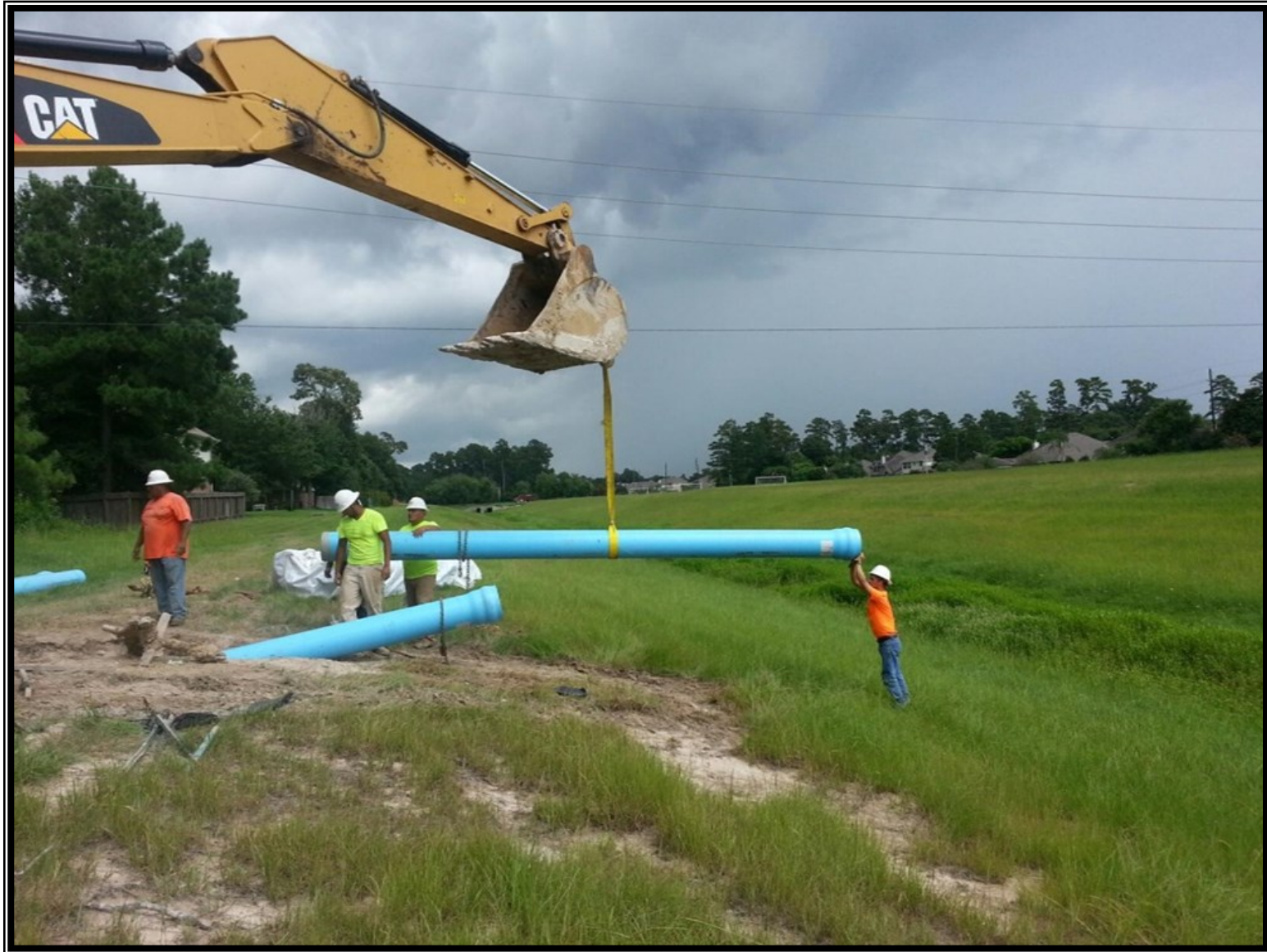
① Segment W3B - 12-inch waterline installation along Montgomery County Drainage District No. 6
