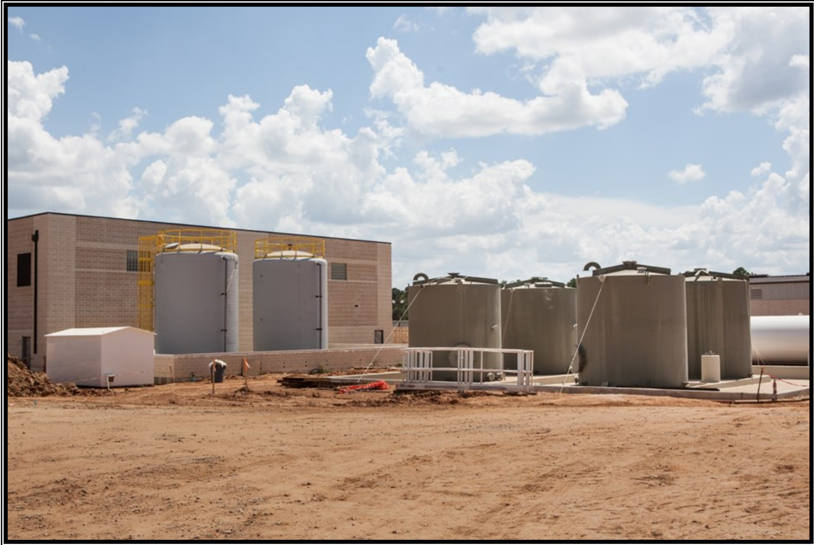
④ Storage tank installation at the Chemical Building
