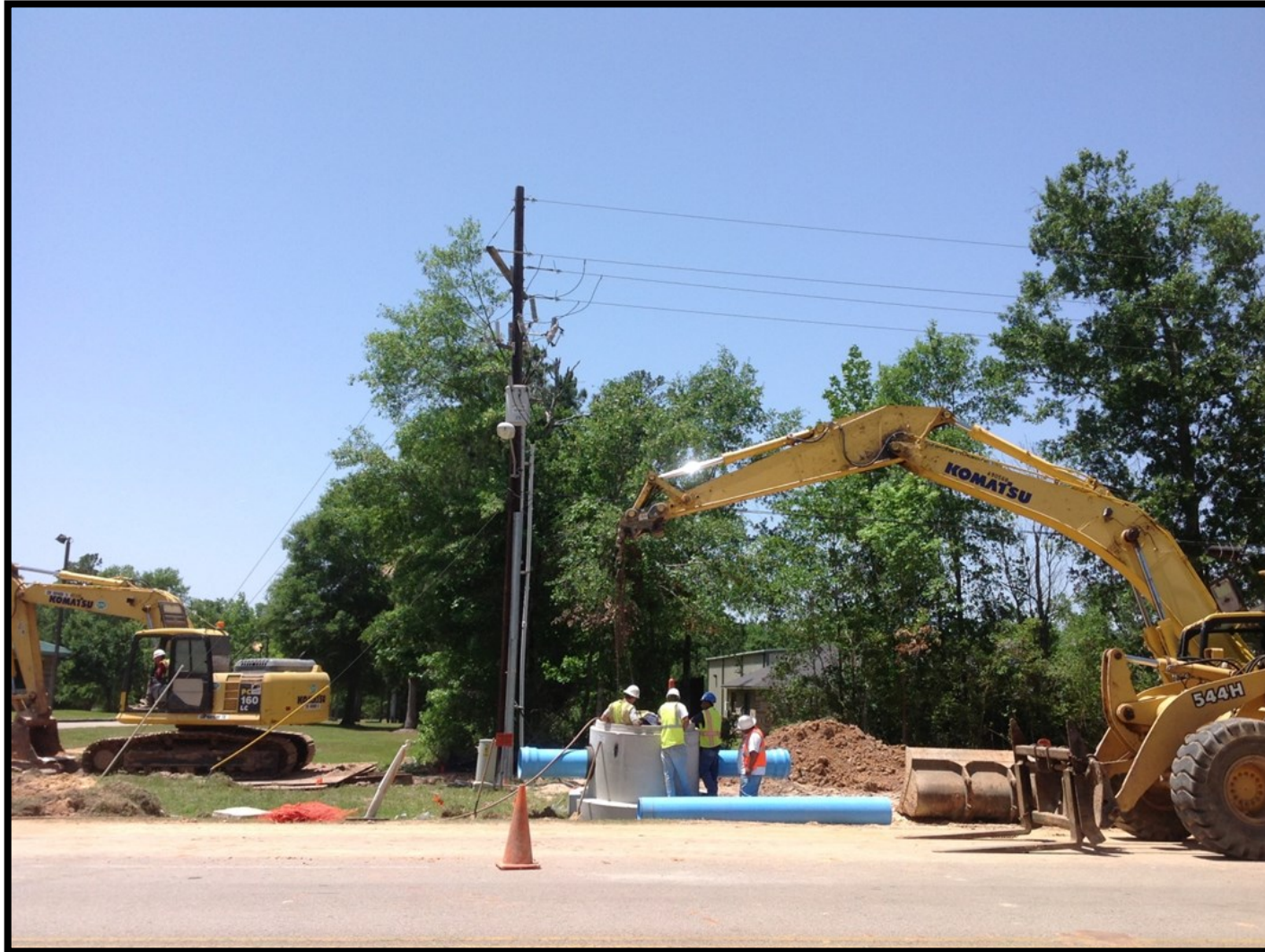
① Segment C3—Valve access manhole installation along Pollock Road
