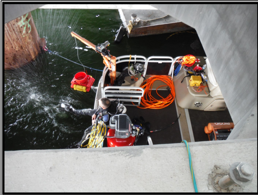
❶ Divers and construction crew preparing for placement of pump barrels into Lake Conroe at Raw Water Intake
