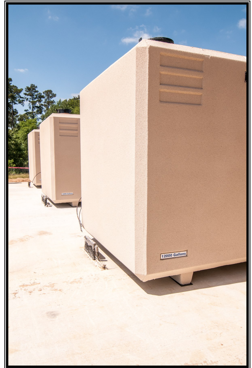
Three 12,000 gallon diesel fuel reservoirs at Surface Water Facility
