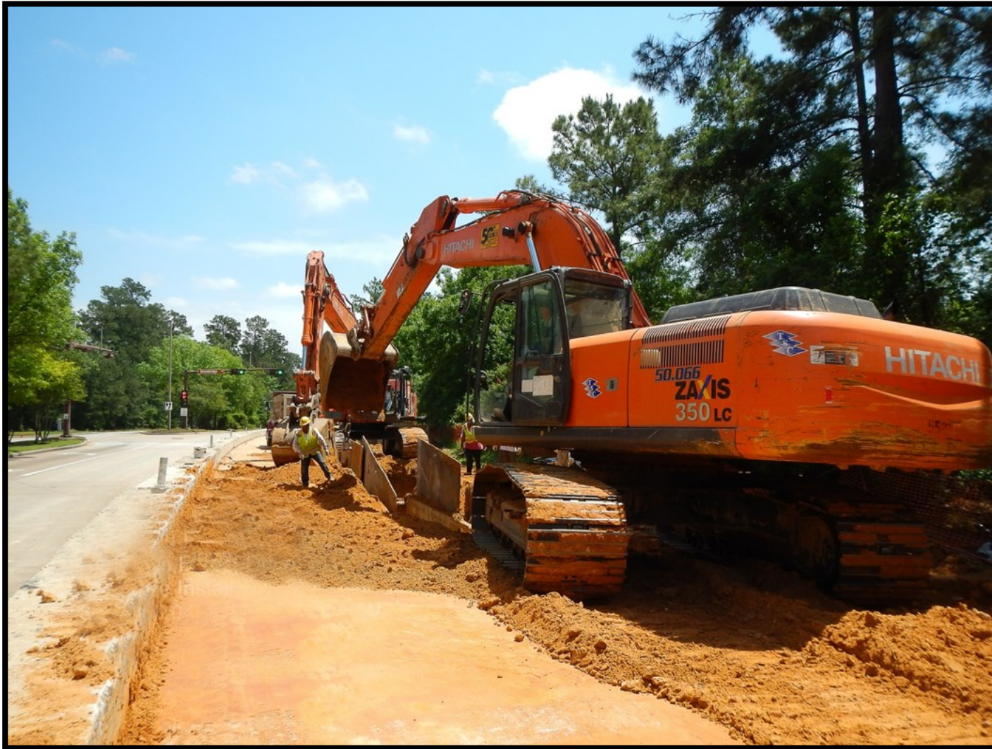
① Segment W1B - 42-inch pipe installation along Research Forest Drive
