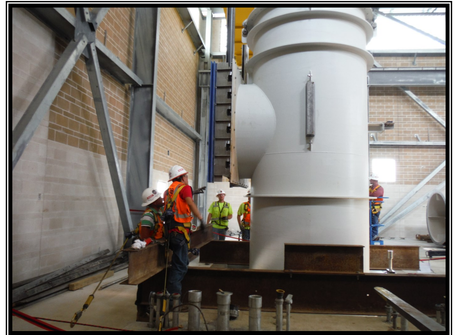
❶ Divers and construction crew preparing for placement of pump barrels into Lake Conroe at Raw Water Intake
