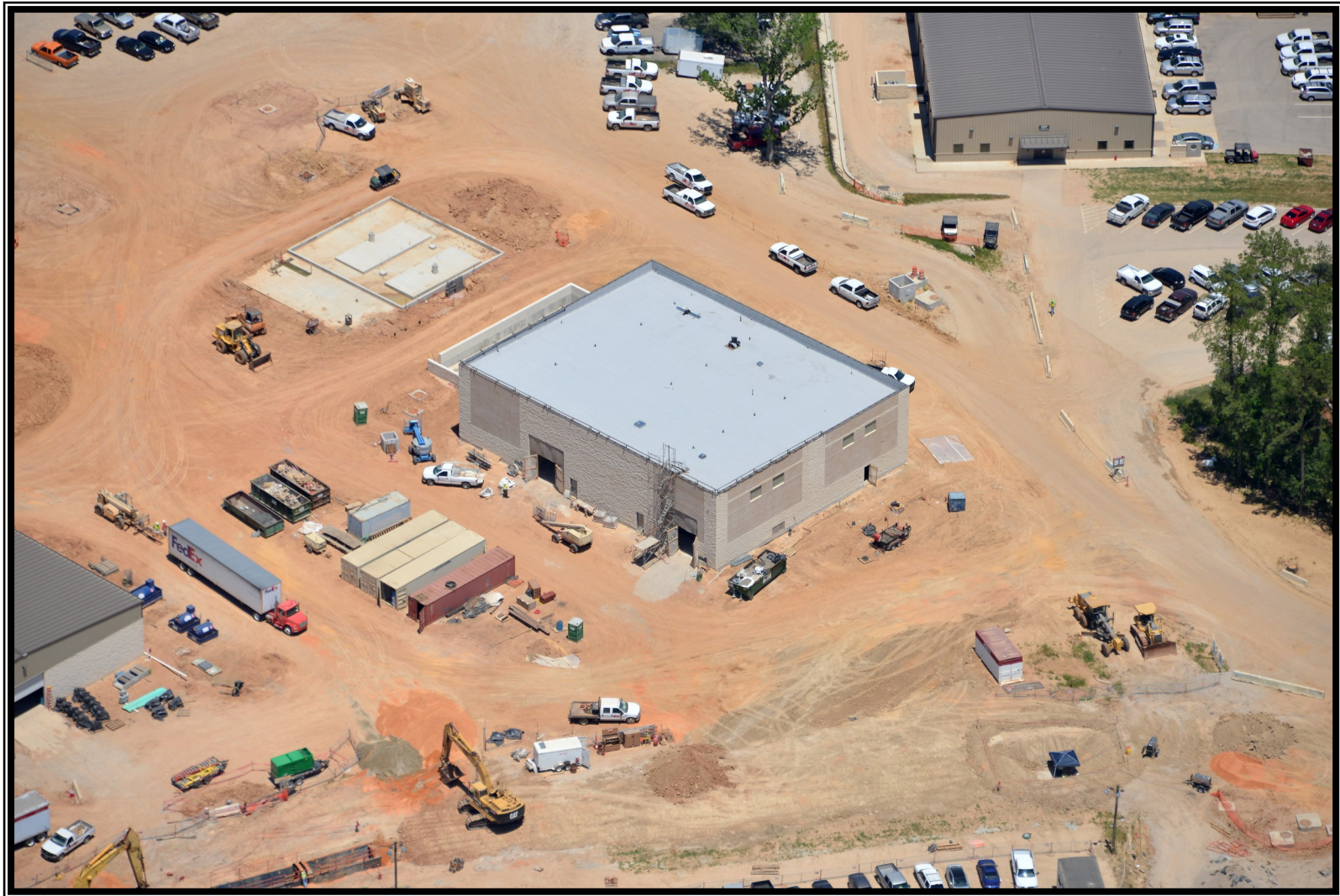
⑤ Aerial view of the Chemical Storage Facilities
