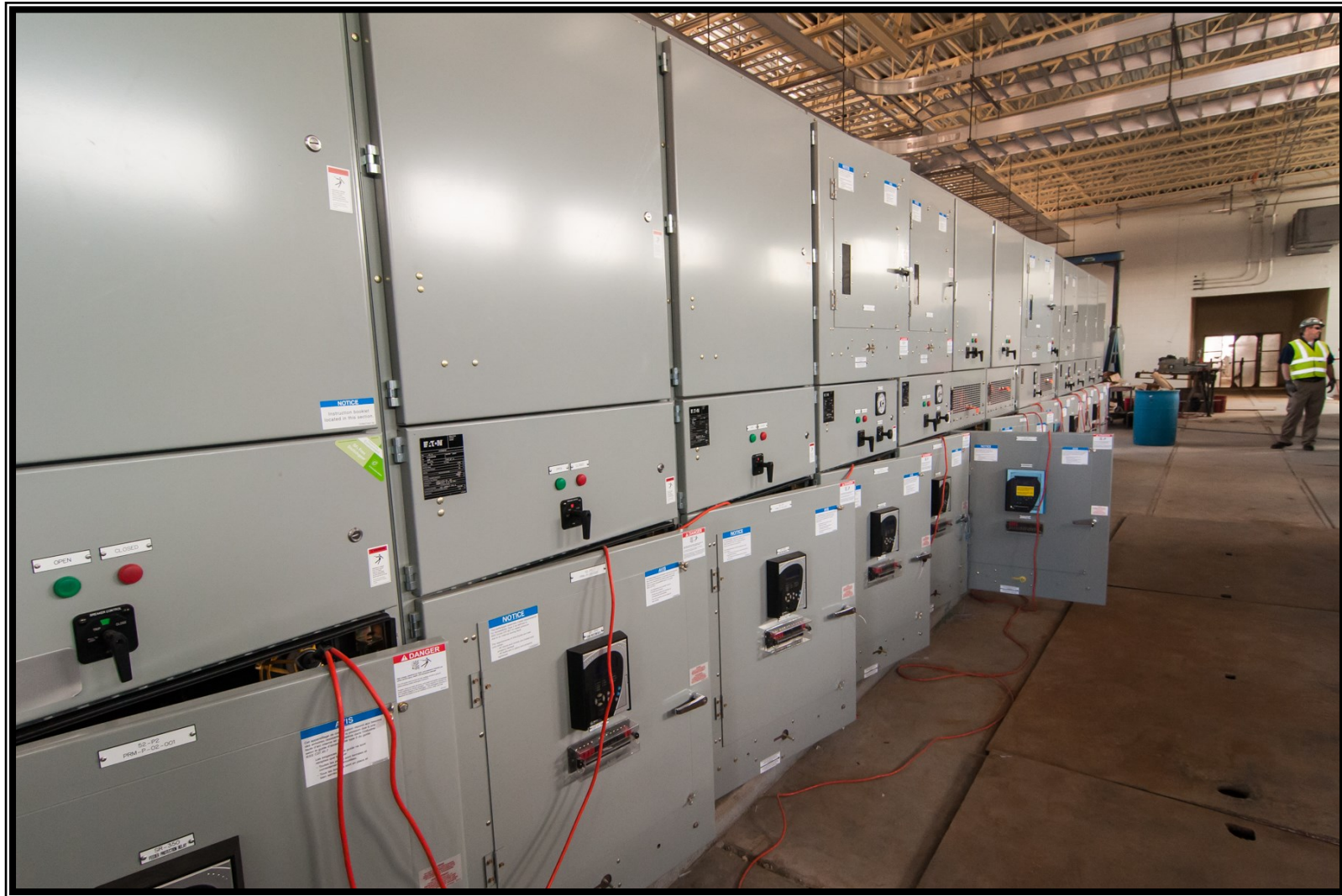
6 Motor control center at High Service Pump Station
