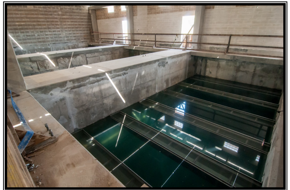
Leak testing contact basins at GAC Building at Surface Water Facilities
