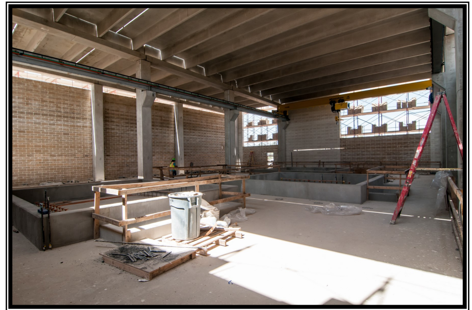
Masonry work at Solids Dewatering Building at Surface Water Facility
