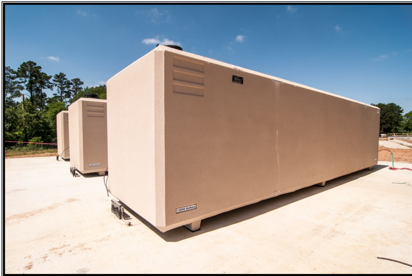
12 Diesel fuel reservoirs at Electrical Facilities
