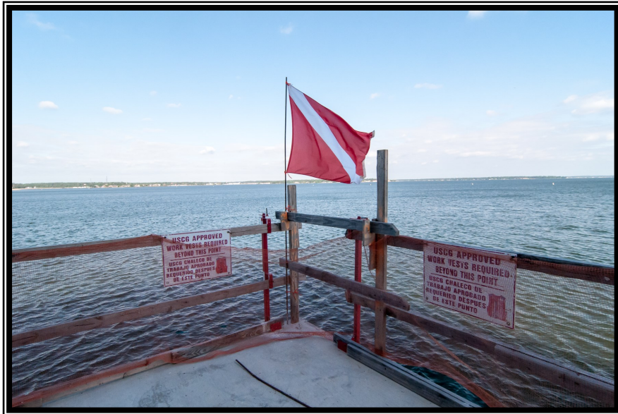
Flag being flown to indicate divers working in the area. Divers installing intake screens in water at Raw Water Intake
