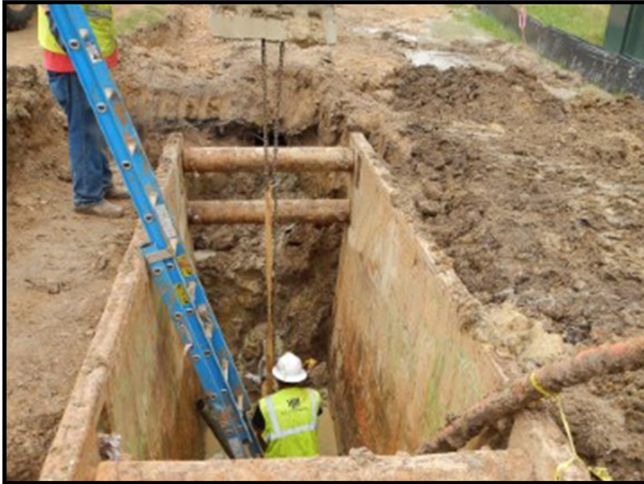
❶ Segment W4 - 24-inch pipe and fiber optic conduit installation on Gosling Road
