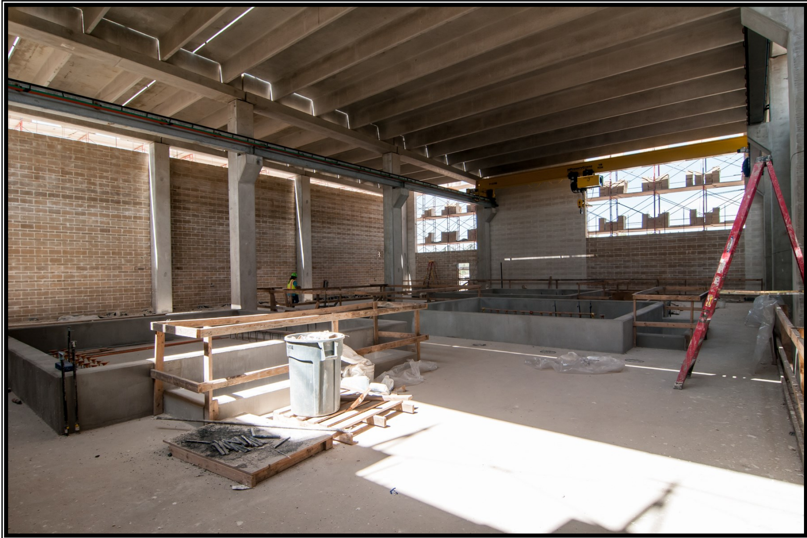
⑧ Masonry installation at Solids Dewatering Building
