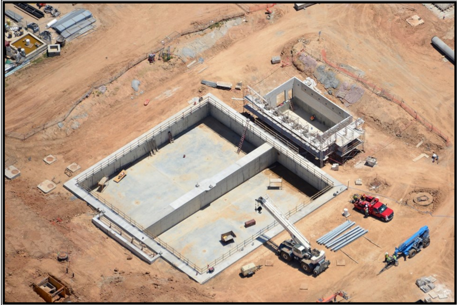
9 Aerial view of the Backwash Equalization Basin
