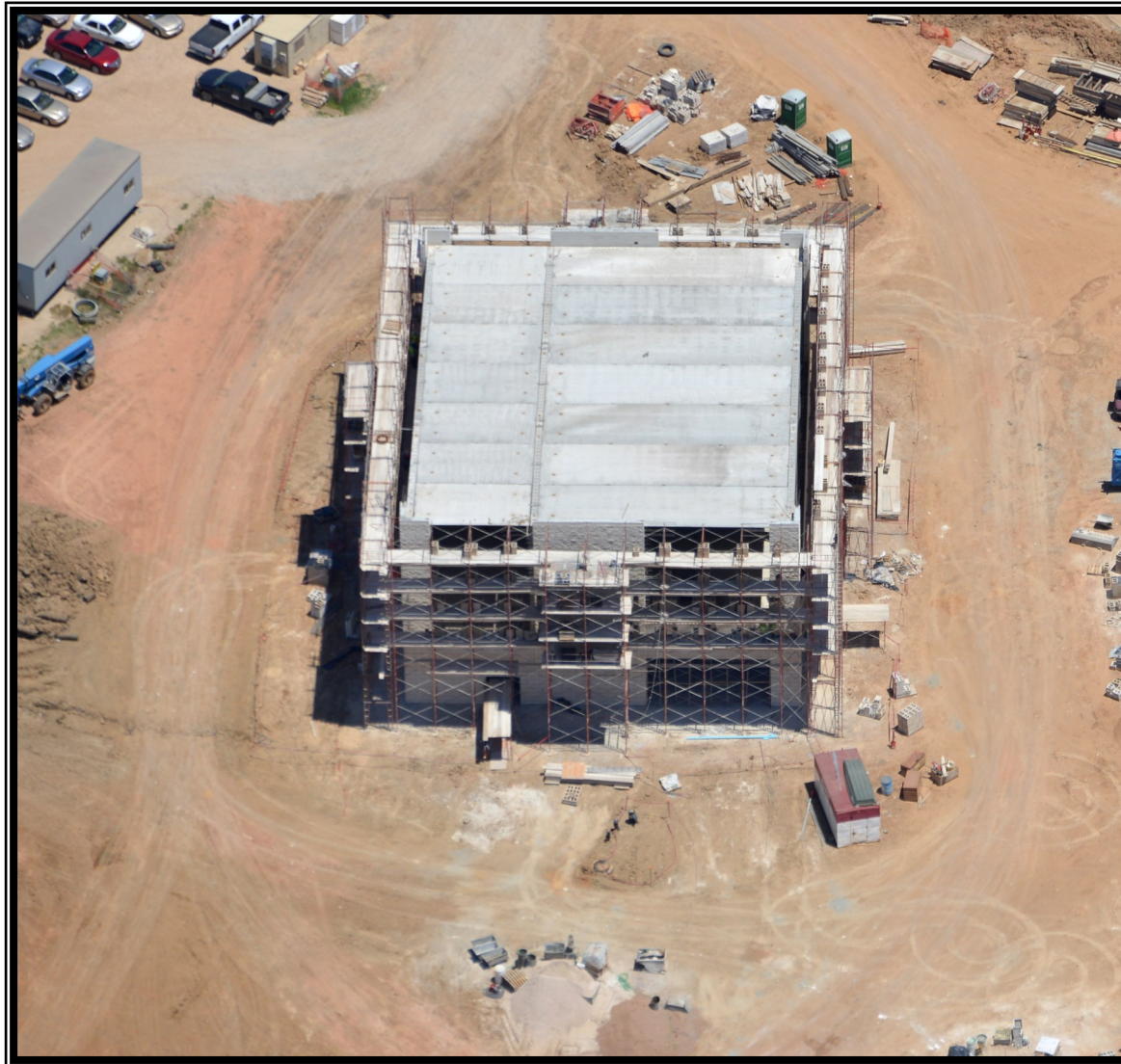
⑧ Aerial view of Solids Dewatering Building
