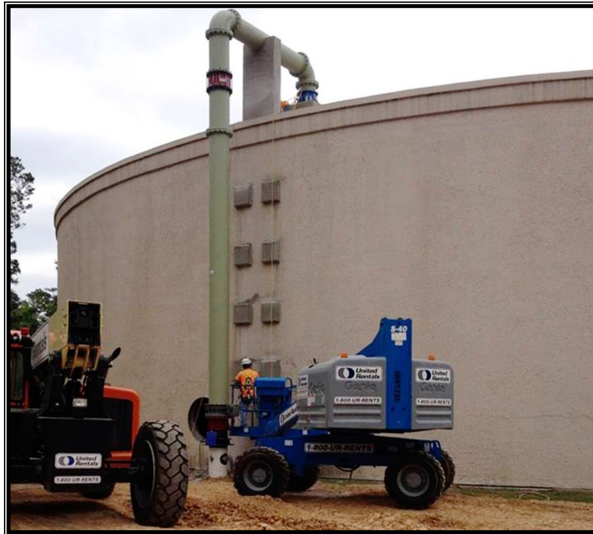
① Surface Water Receiving Facility – South —20-inch ground storage tank connection at SJRA Water Plant No. 4
