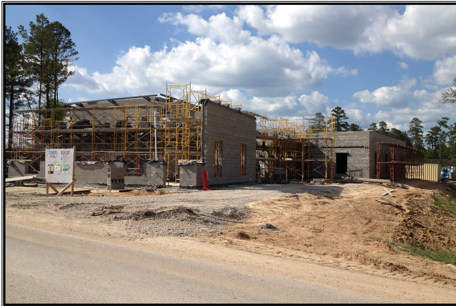
11 Roof framing and masonry installation at Operations Building
