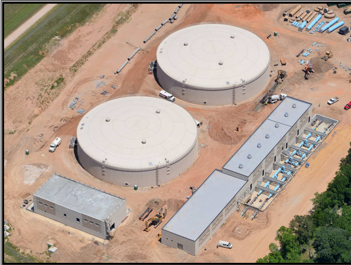
Aerial view of GSTs 1 & 2, High Service Pump Station and Blower Building
