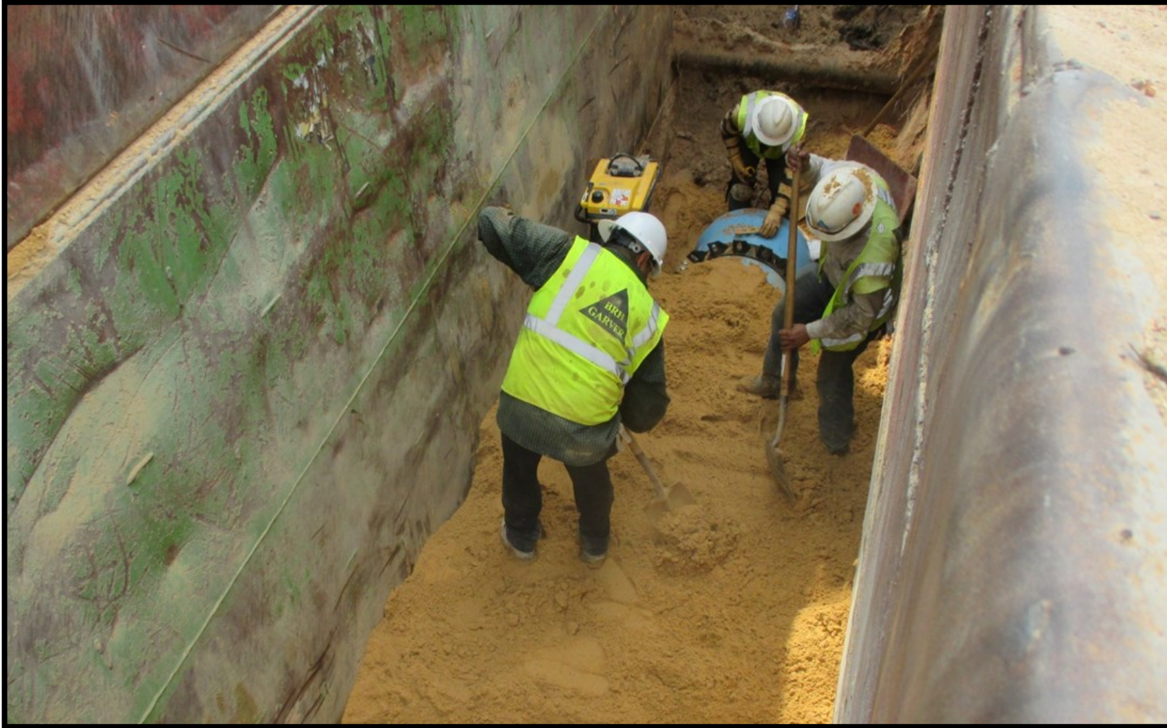
① Segment C4—24-inch pipe and restrained joint installation along FM 830
