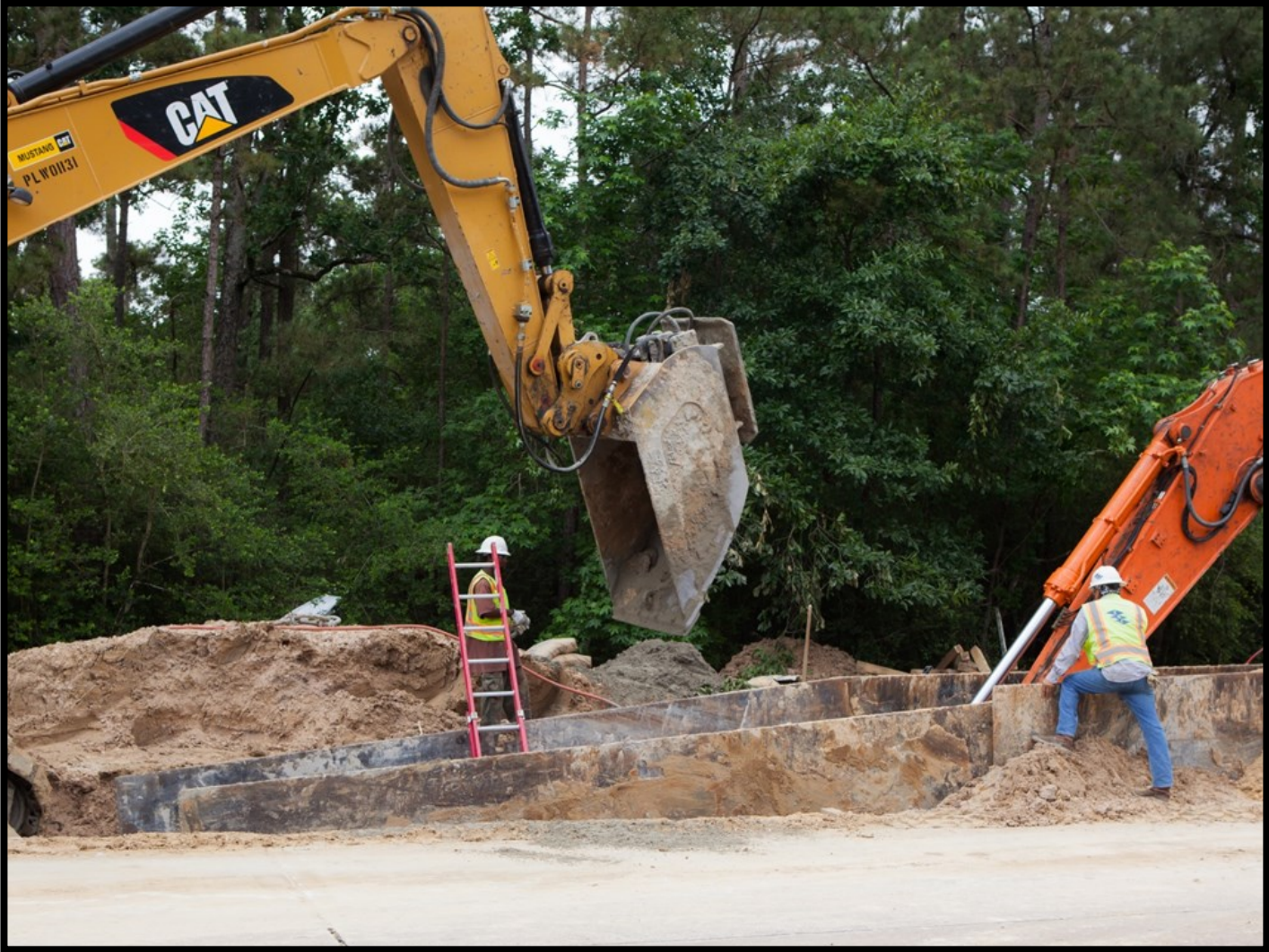
① Segment W2A - 42-inch pipe installation along Research Forest Drive
