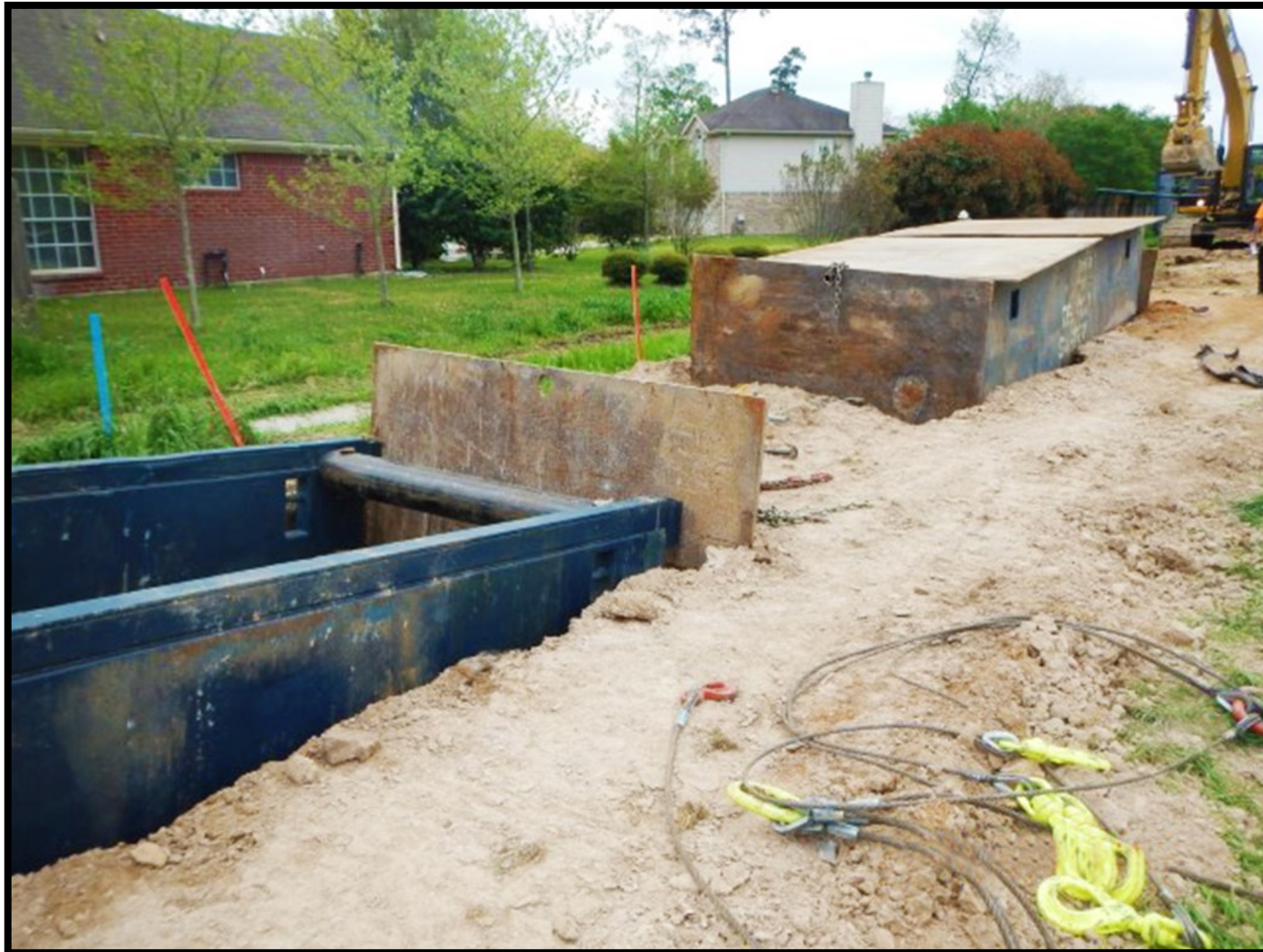
① Segment W3B— Pipe installation along Montgomery County Drainage District right-of-way
