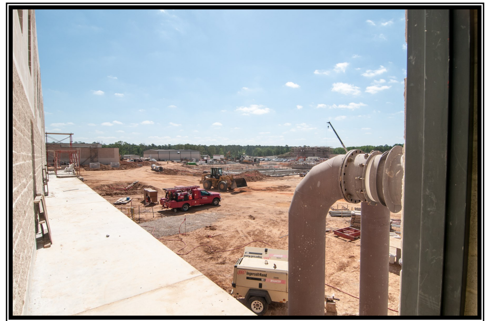
View from GAC Building at Surface Water Facility
