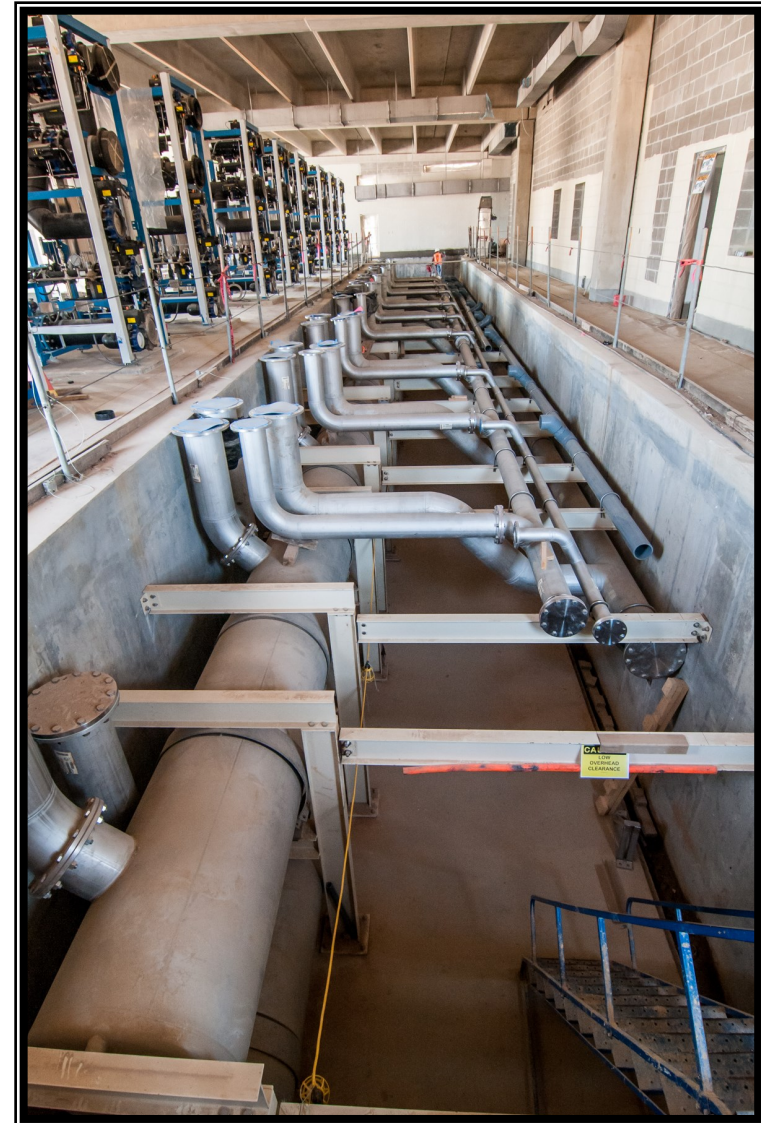
③ Equipment racks and piping at the Membrane Building
