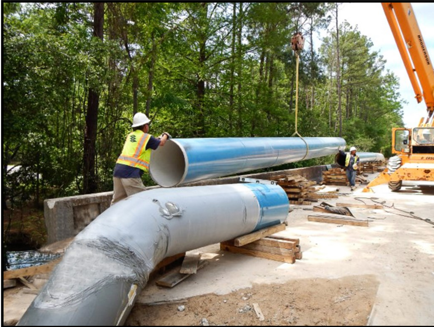
① Segment W2B - 30-inch aerial pipe installation on Grogans Mill Road at bridge crossing
