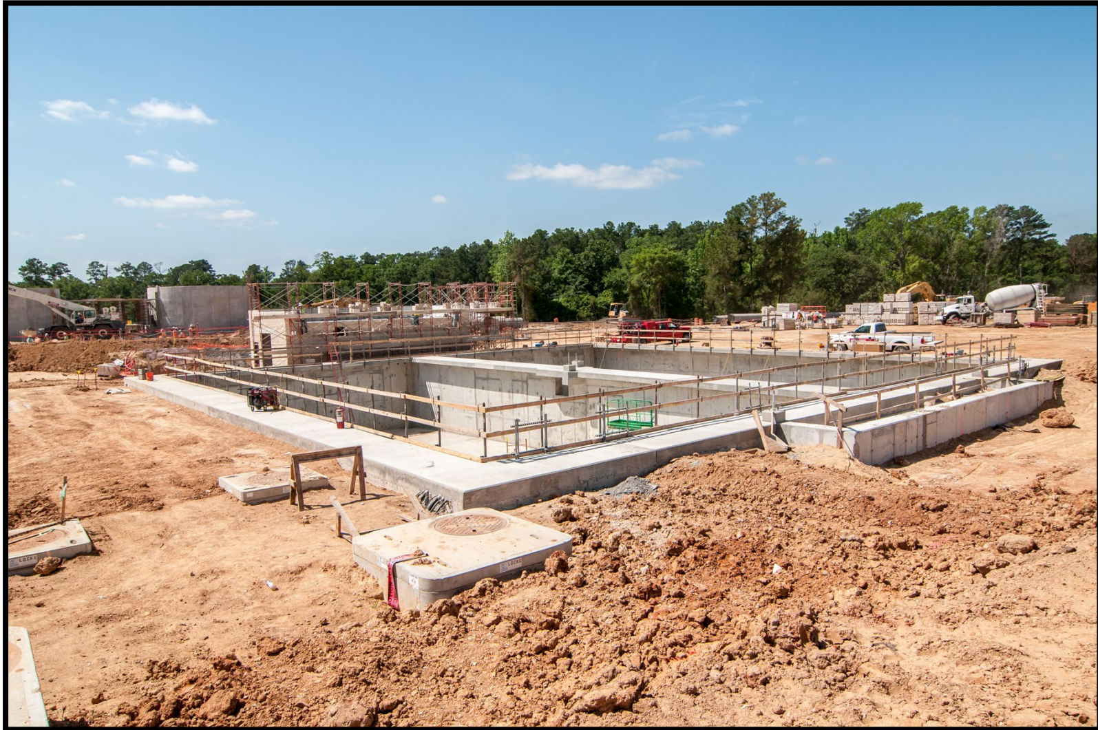
9 Pump station masonry installation at Backwash Equalization Basin
