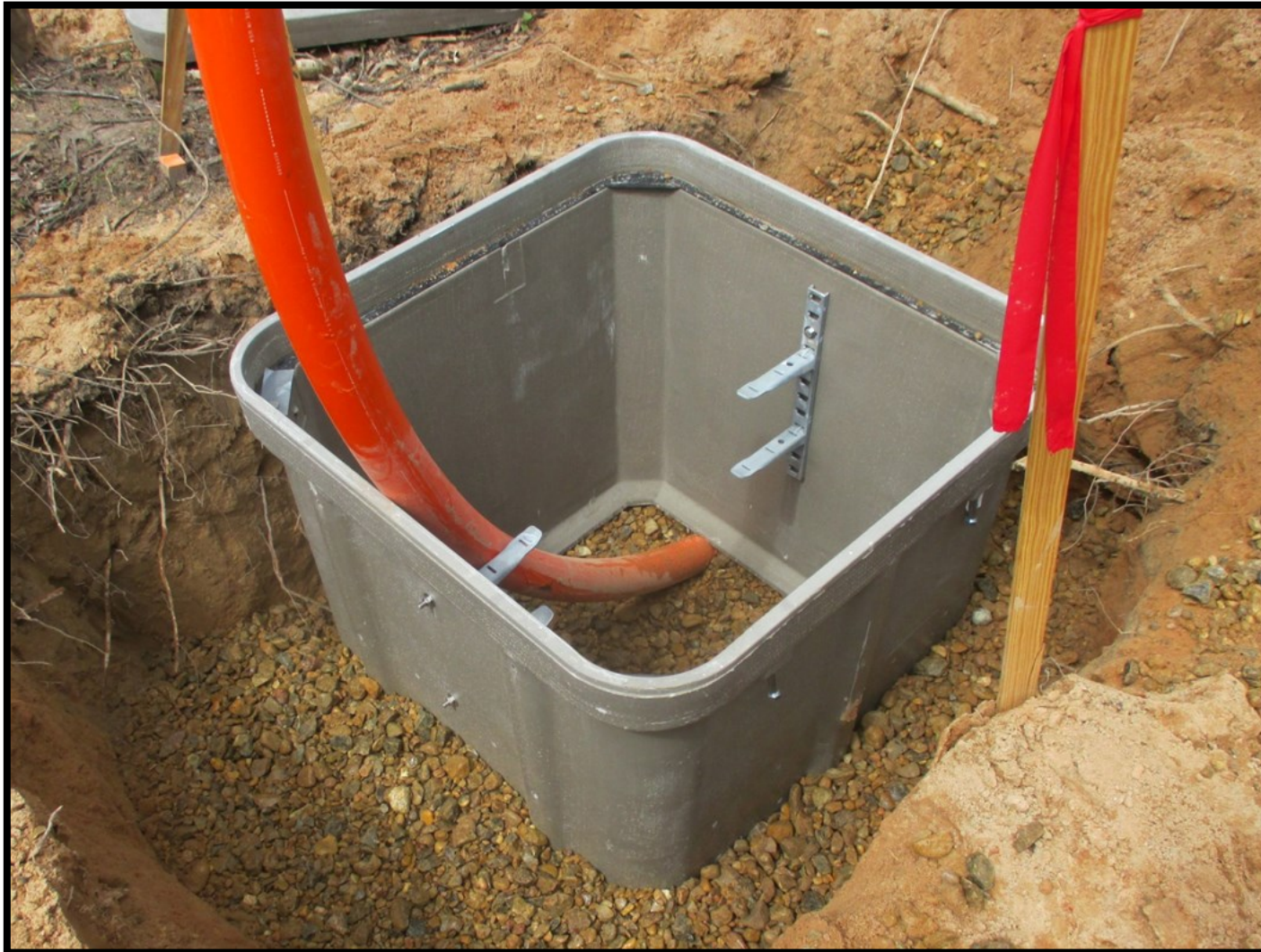
① Segment C1B—Ground box and fiber optic conduit installation
