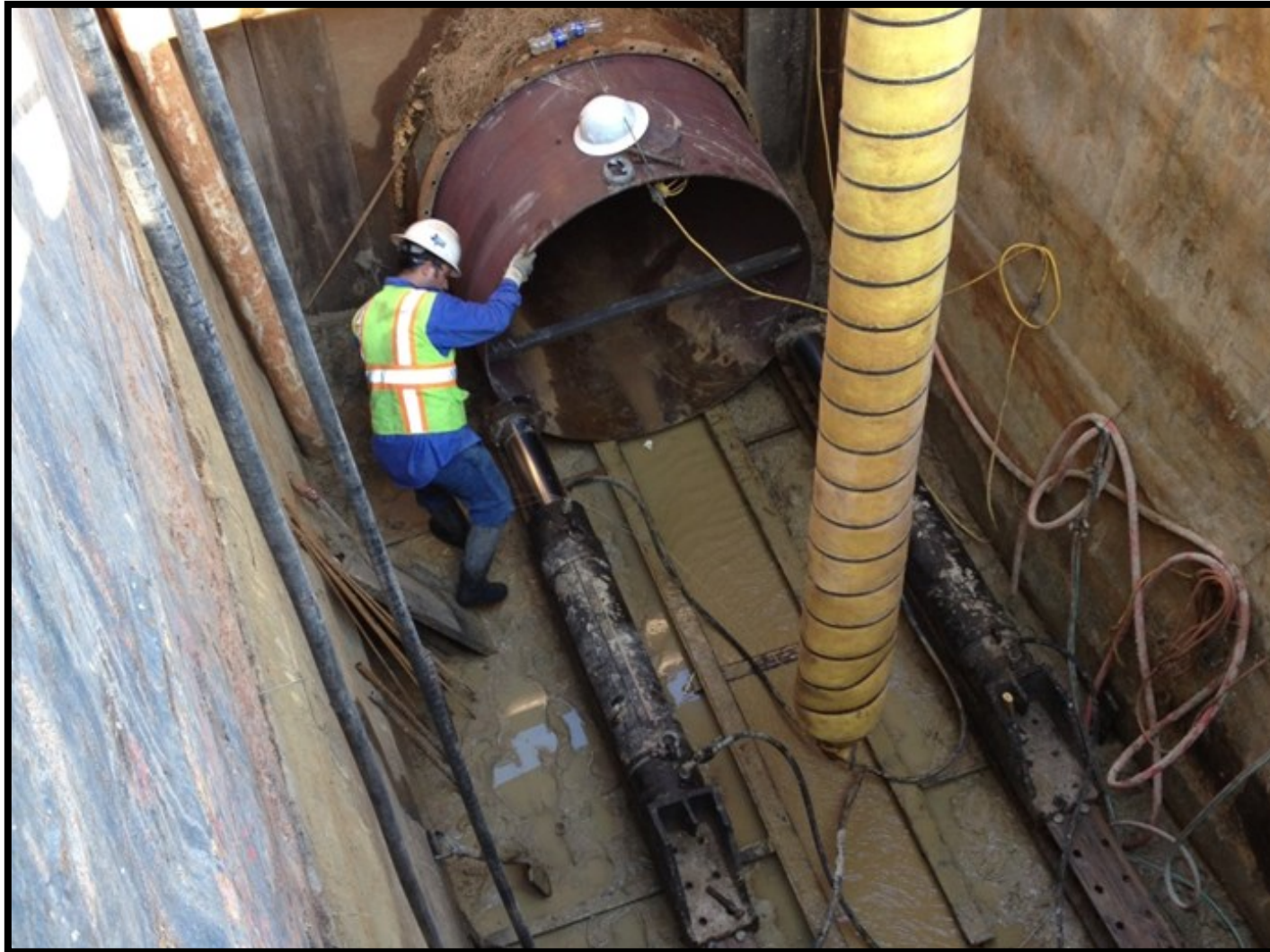
① Segment C1A - Tunnel installation at Longmire Road
