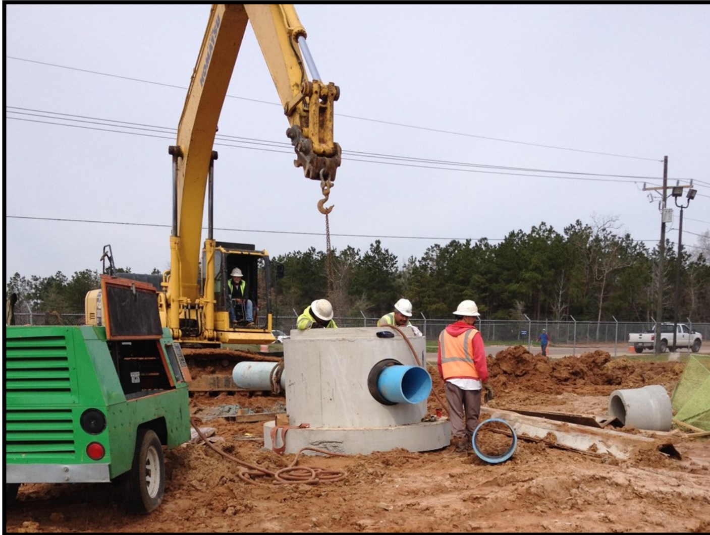
❶ Water Receiving Facilities - North—Valve access manhole installation at Conroe Water Plant No. 20
