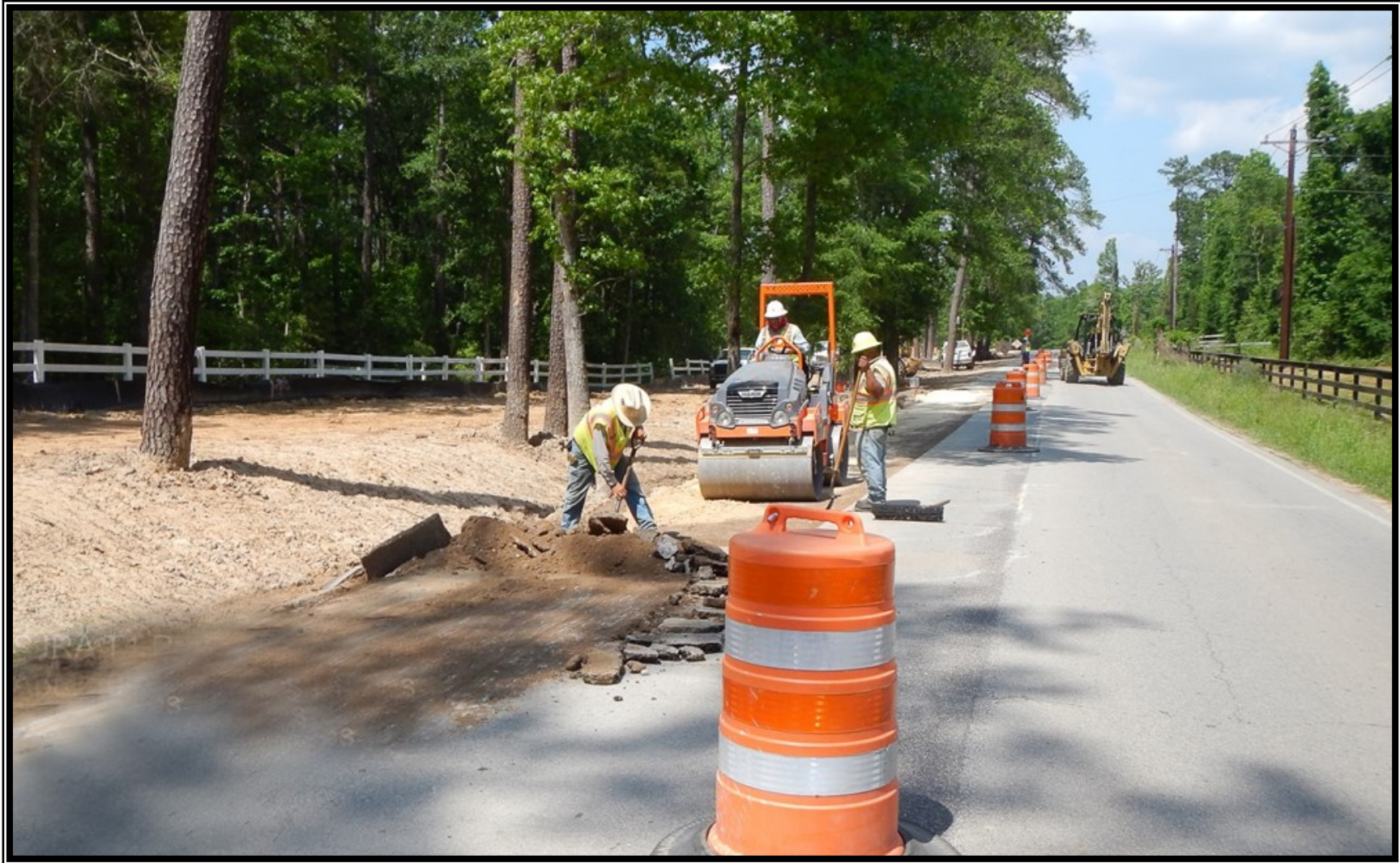
① Segment T1 - Asphalt pavement repairs along McCaleb Road
