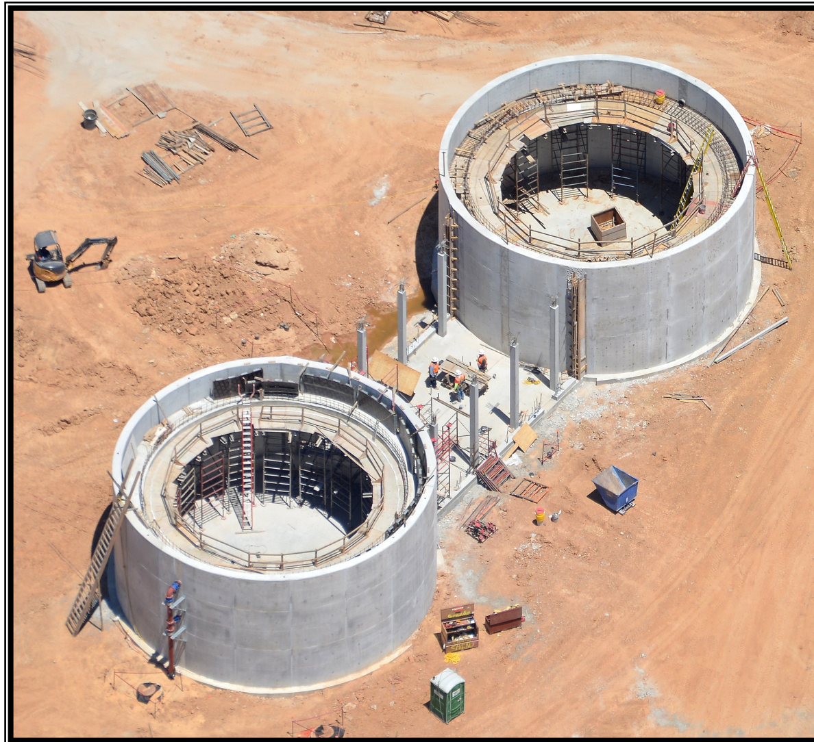
⑩ Aerial view of Sludge Thickeners
