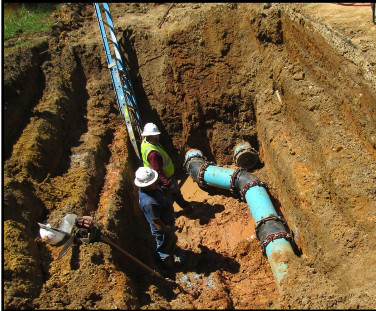
① Segment W1A—12-inch water line relocation at the intersection of Branch Crossing and Research Forest
