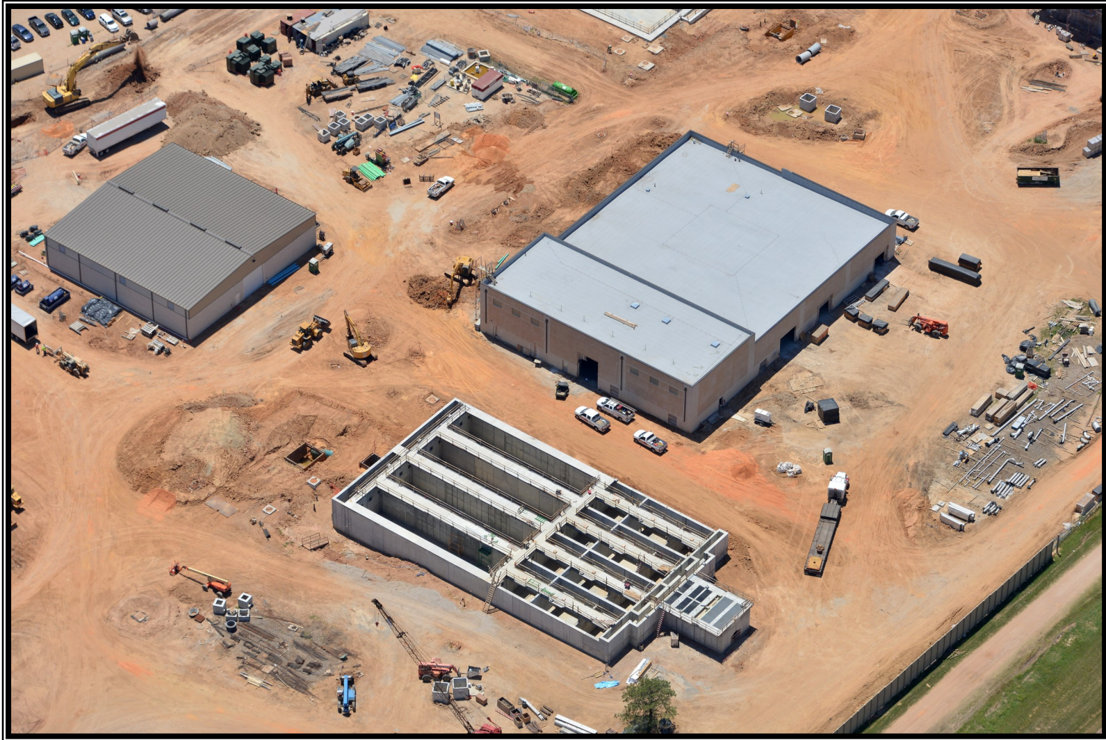
Aerial view of Membrane Building and Pretreatment Facility
