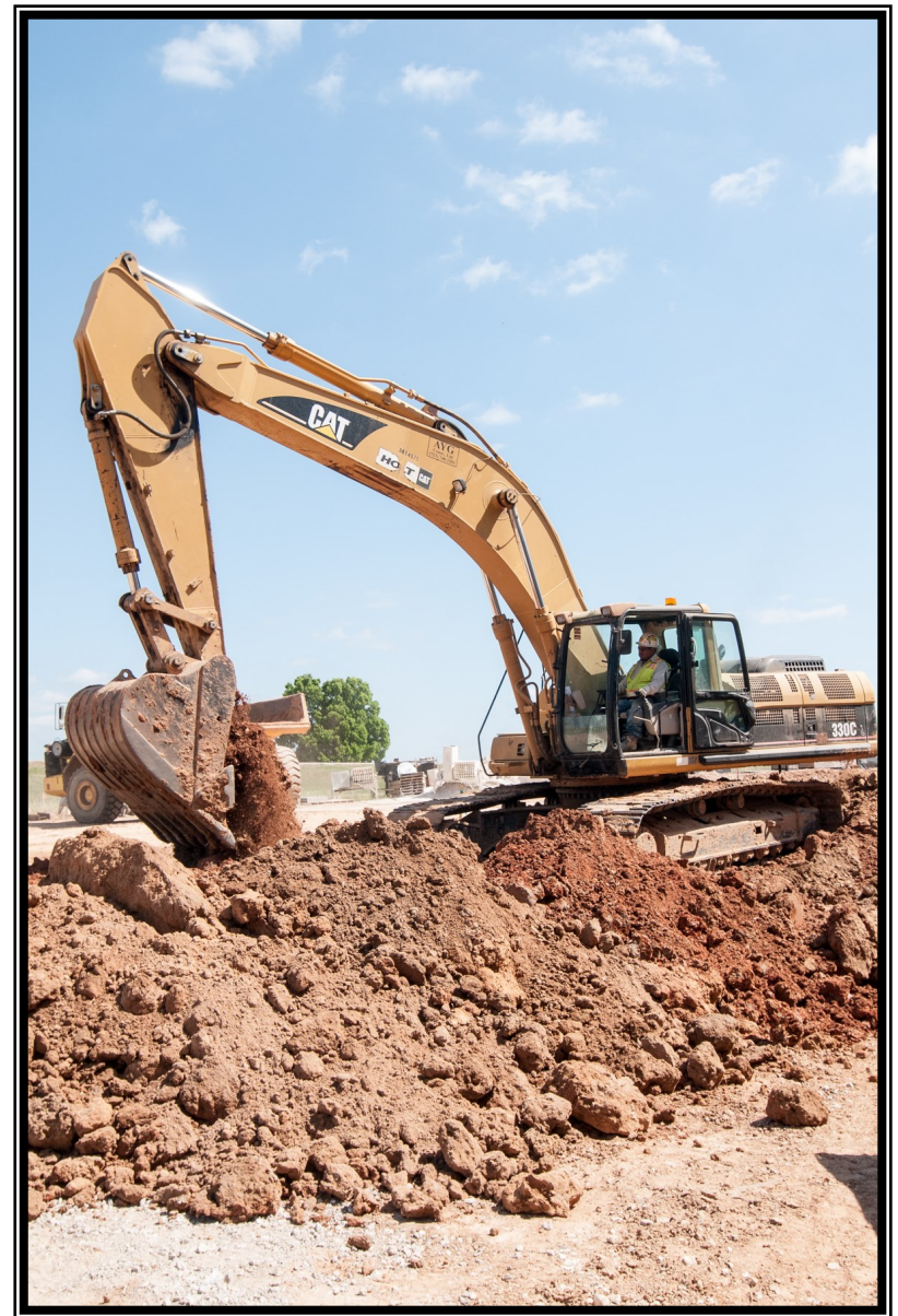
Construction activities at Surface Water Facilities
