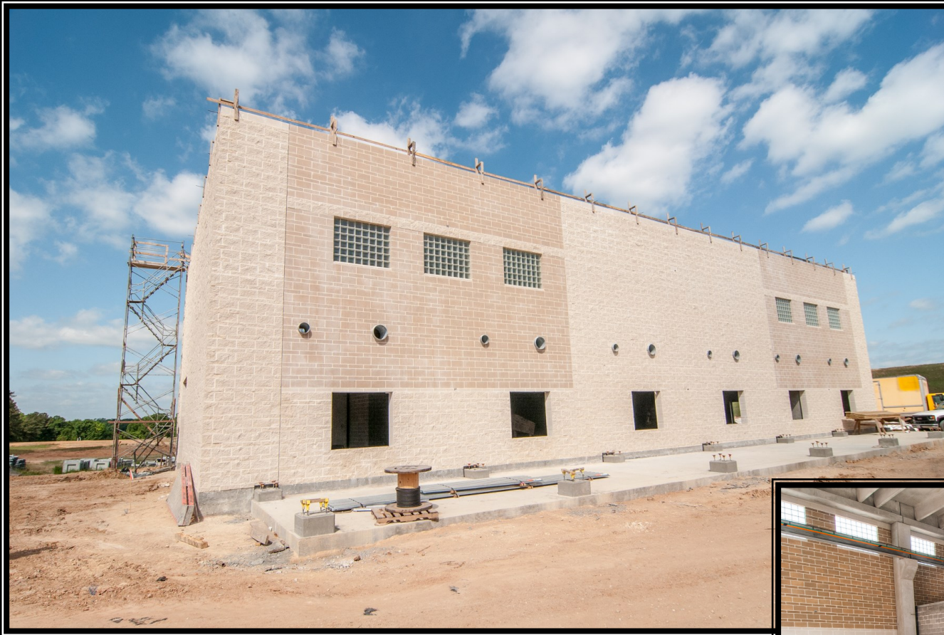
⑦ Exterior view of Blower Building
