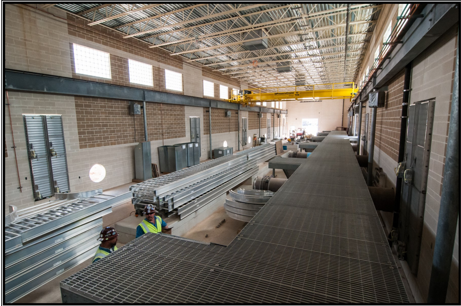
⑥ Interior view of High Service Pump Station
