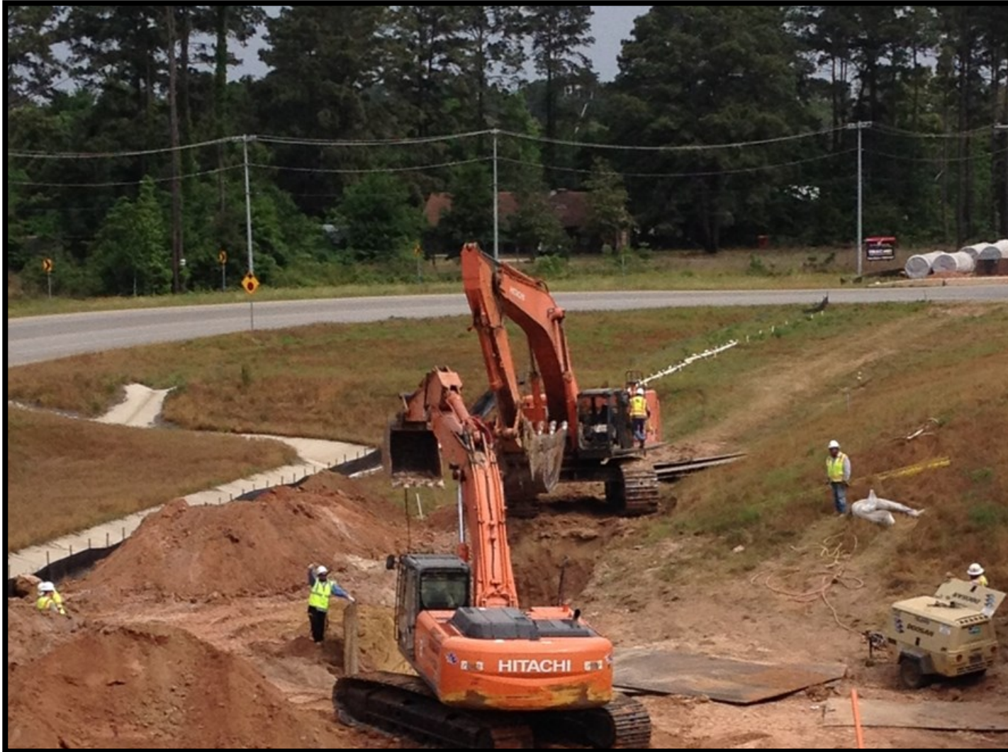
① Segment T2 - 54-inch pipe installation at FM 2854
