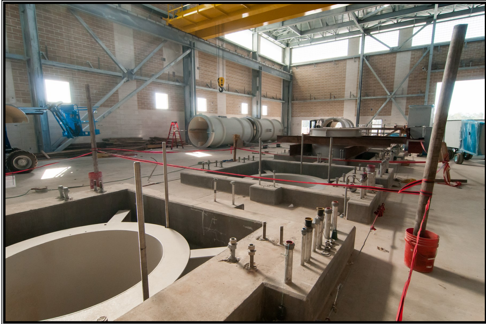
❶ Pump barrels in place at Raw Water Intake and Pump Station
