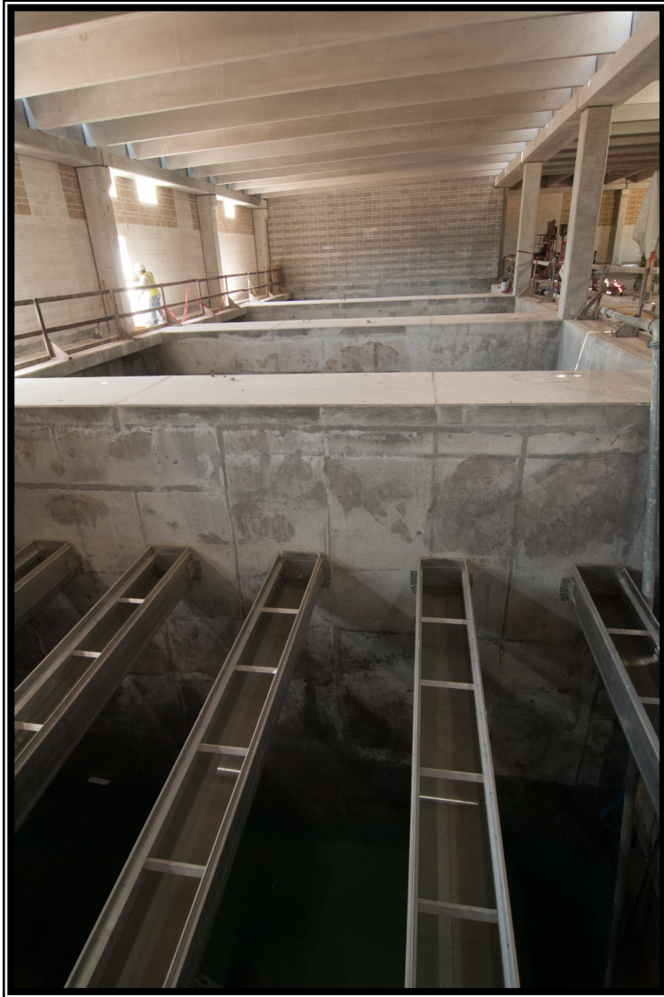
④ Contactor underdrain in Granulated Activated Carbon Building
