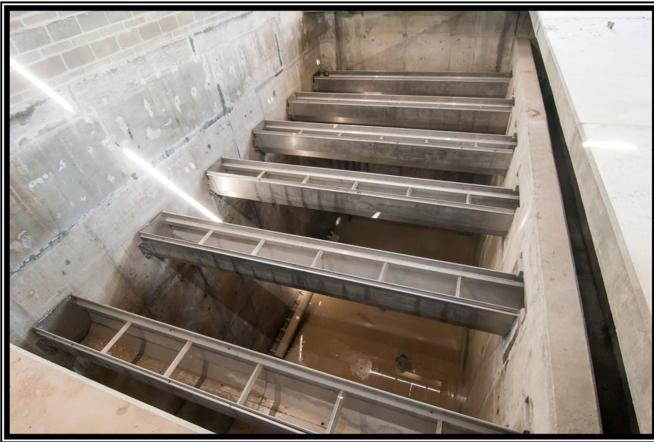
Leak testing contact basins at GAC Building at Surface Water Facilities
