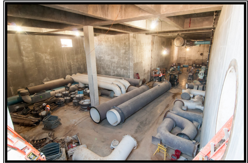
④ Contactor underdrain in Granulated Activated Carbon Building
