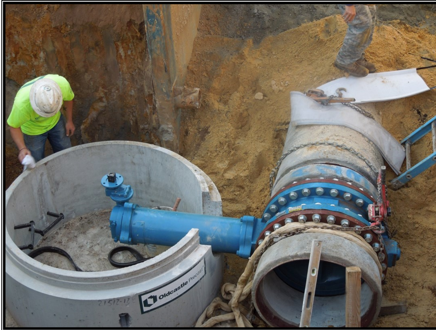
❶ Segment C2— Butterfly valve installation along Entergy easement
