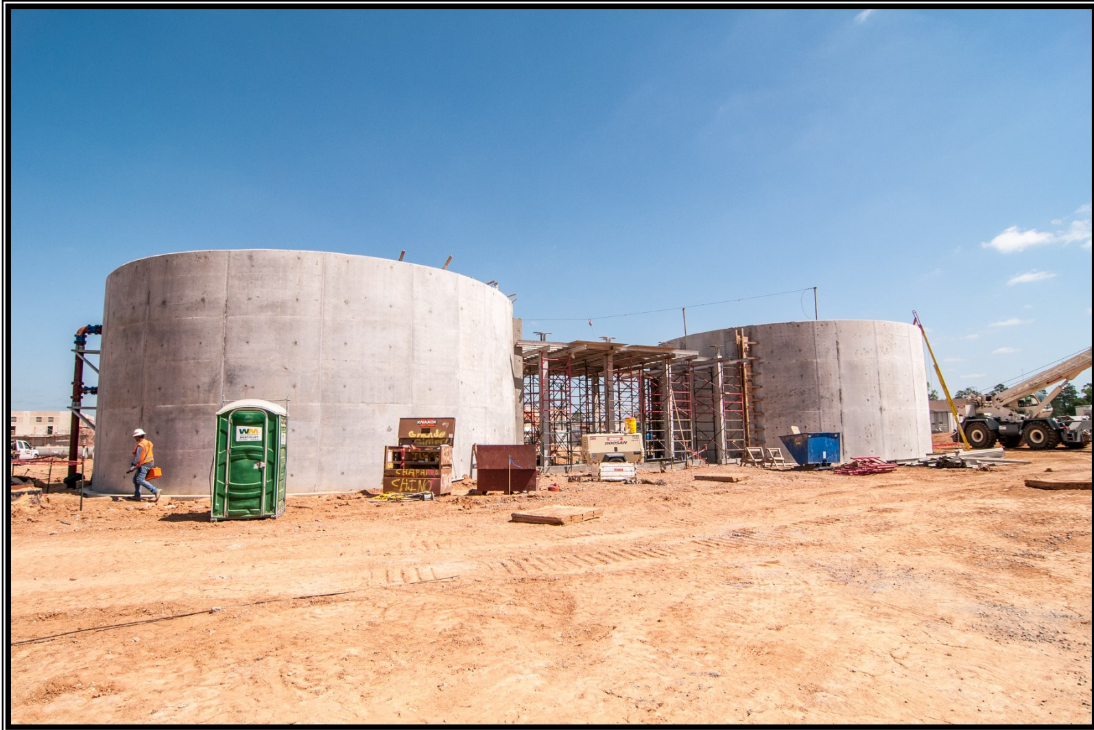
⑩ Concrete column installation continues at Sludge Thickeners
