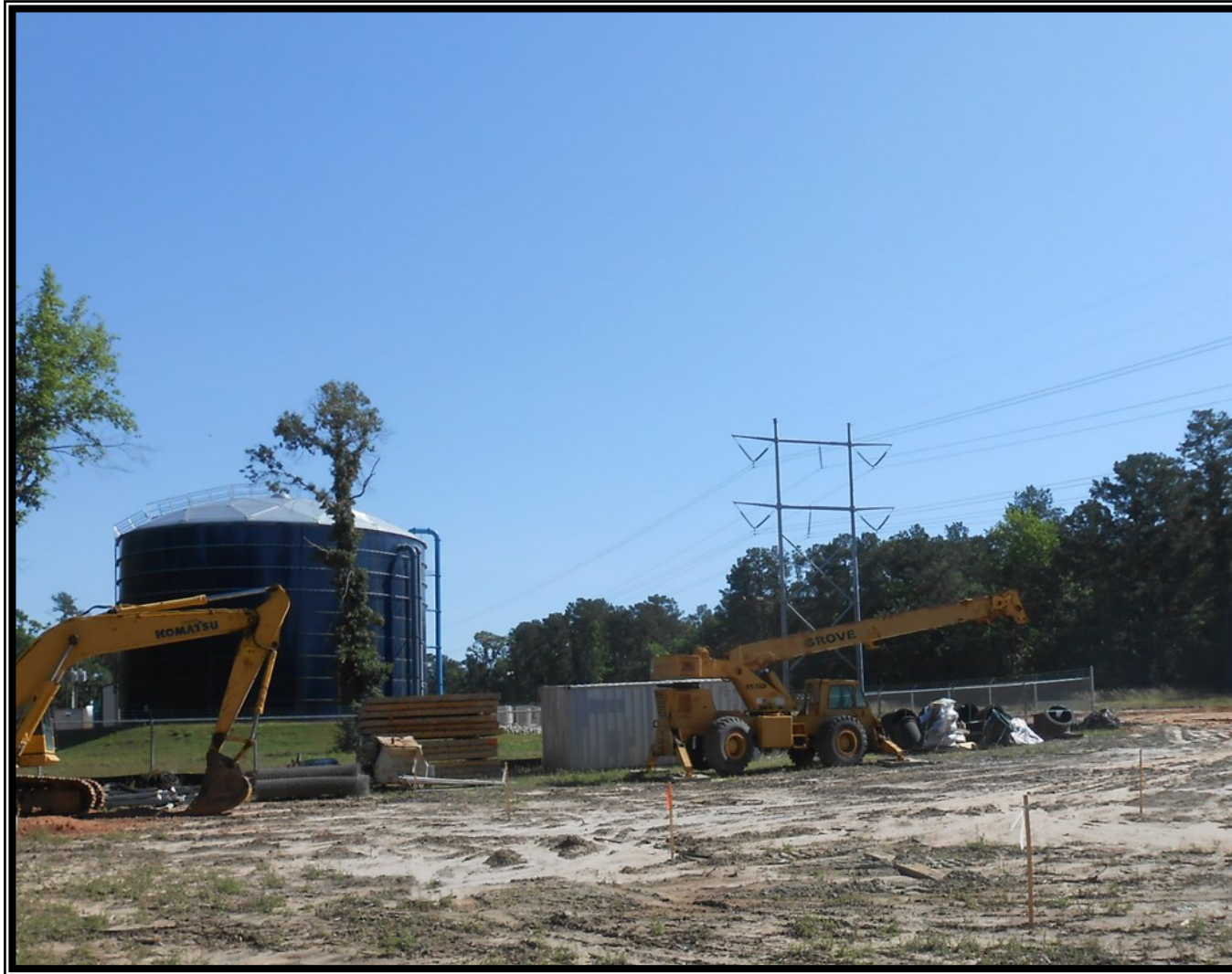
① Surface Water Standpipe—Equipment mobilization and delivery of construction materials
