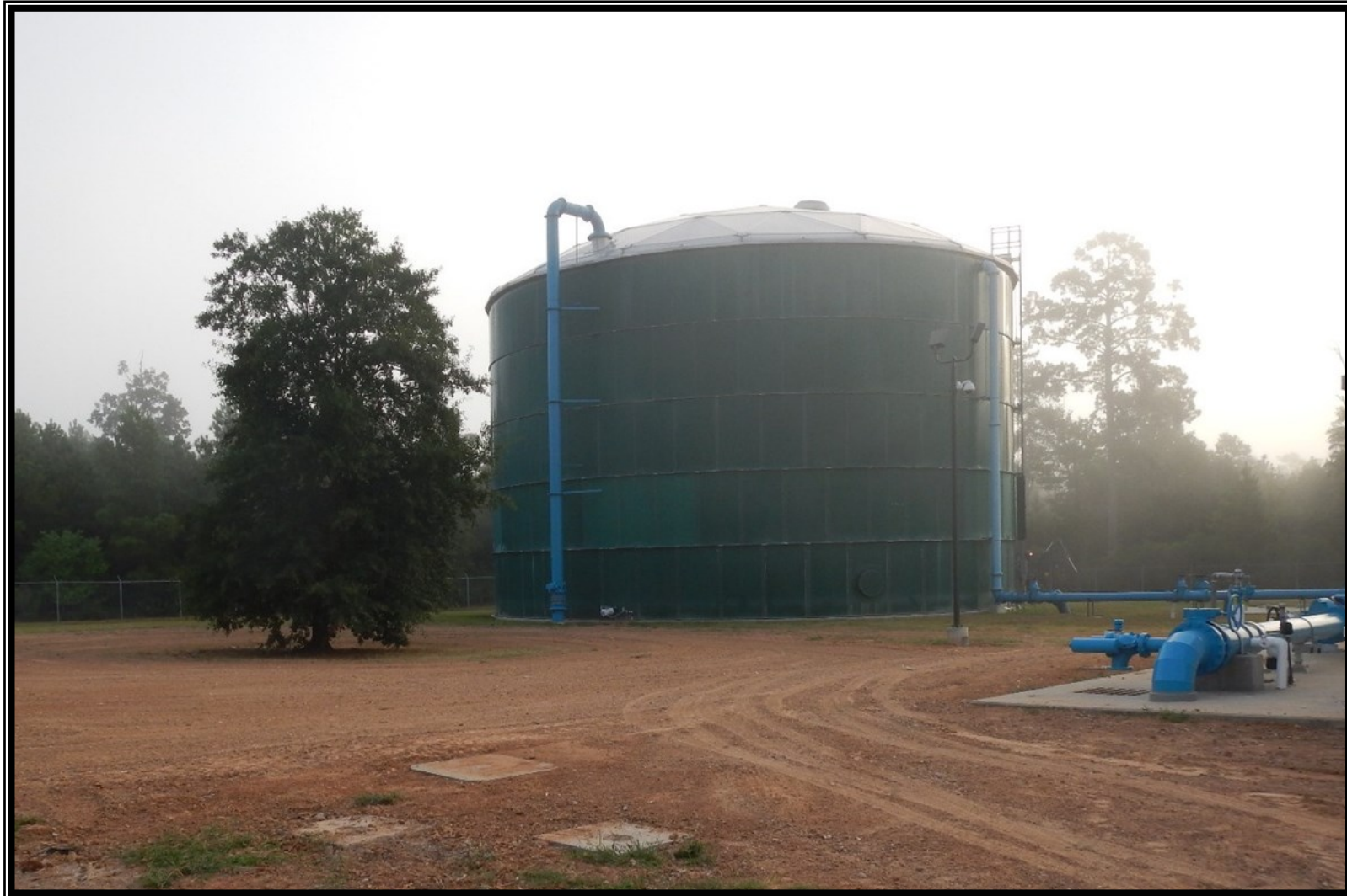
① Surface Water Receiving Facility – North— Site restoration at Conroe Water Plant No. 20
