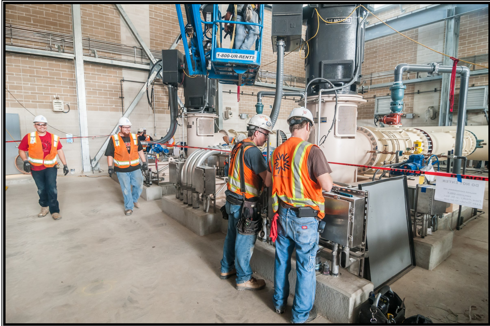
❶ Pump motor installation at the Raw Water Intake and Pump Station
