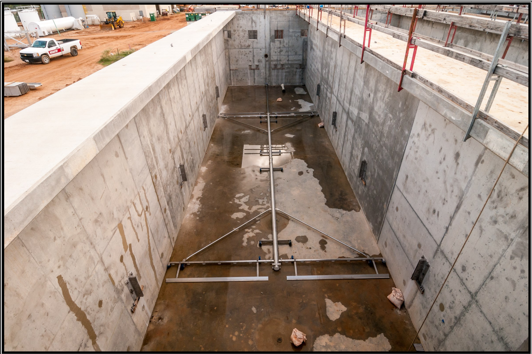
② Hoseless Sludge Collection System installation at the Pretreatment Facility
