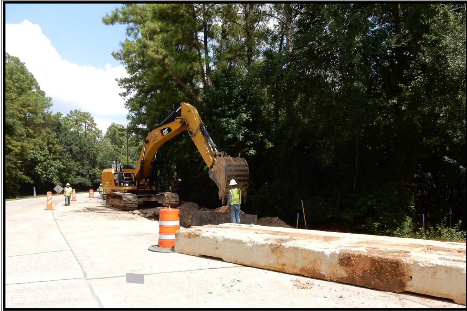
① Segment W3A - 24-inch open-cut pipe installation along South Millbend Drive
