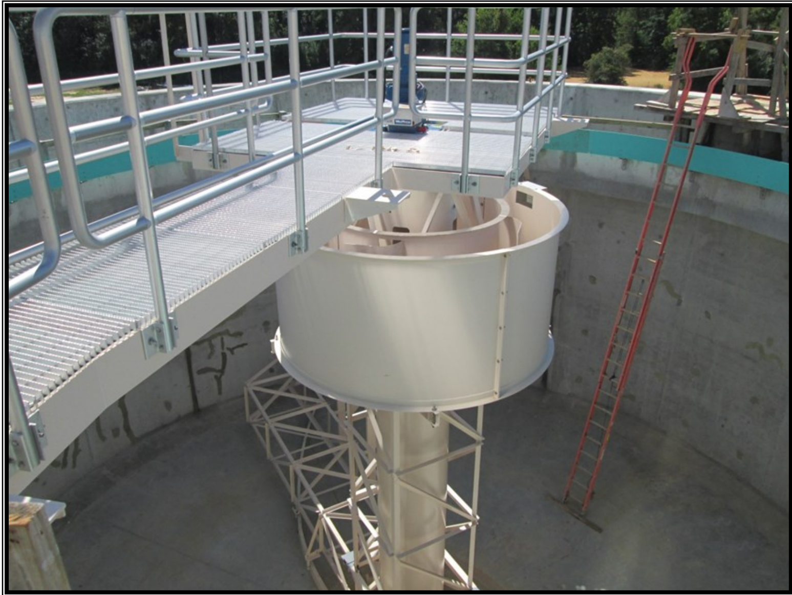
⑥ Stilling well and catwalk installation at the Sludge Thickeners
