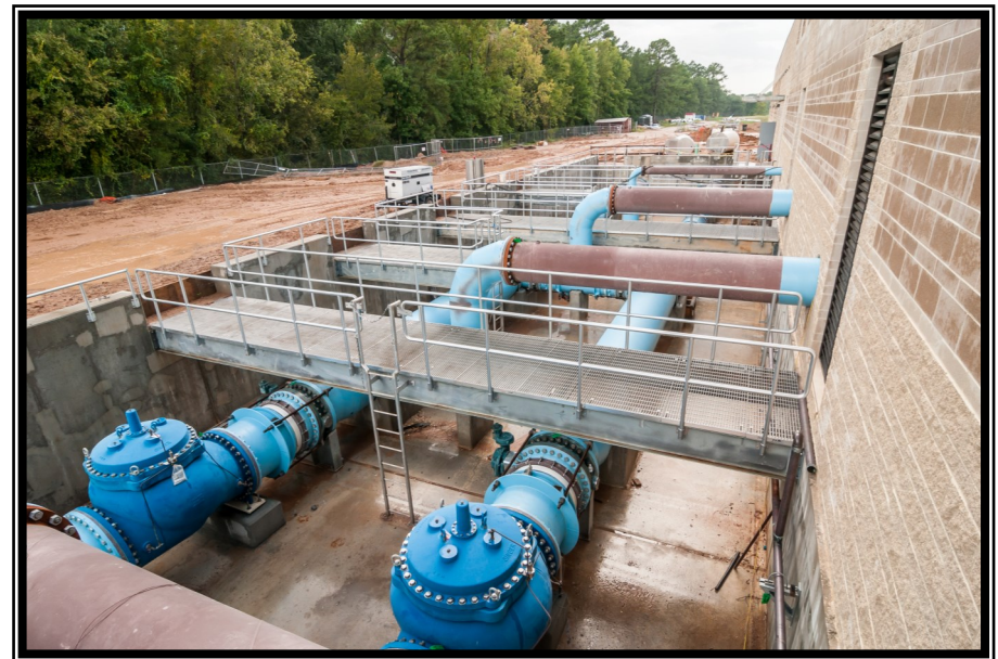
Left: Intake suction header installation at the High Service Pump Station Above: Electrical gear installation at the High Service Pump Station Bottom: Transmission line valves at the High Service Pump Station
