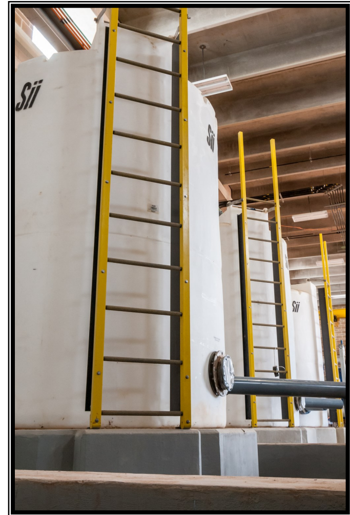
Chemical tanks at the Membrane Building
