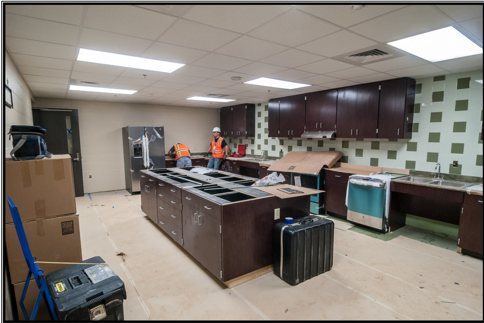
⑦ Kitchen area in the Operations Building
