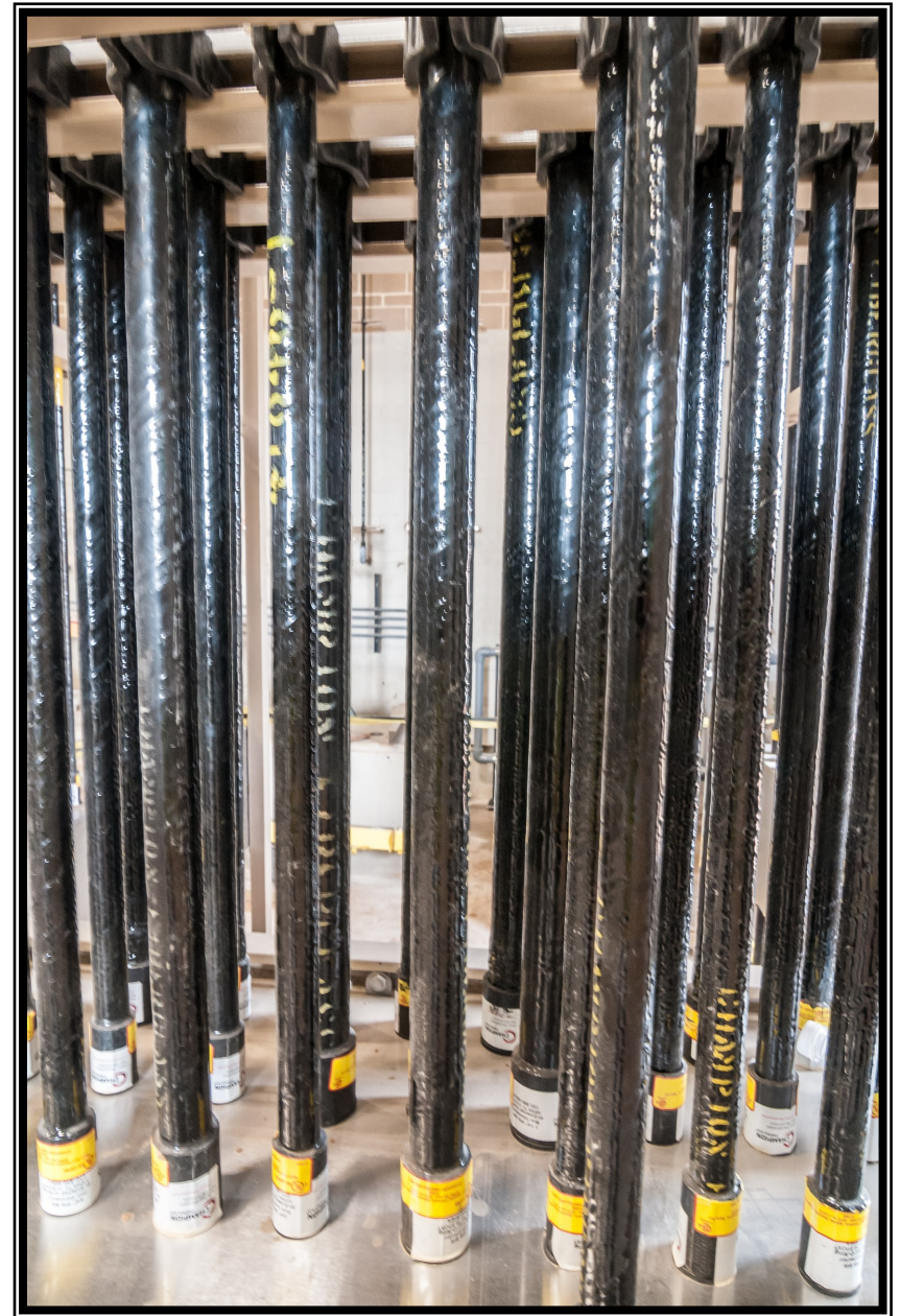
Fiberglass electrical conduit at the Chemical Building
