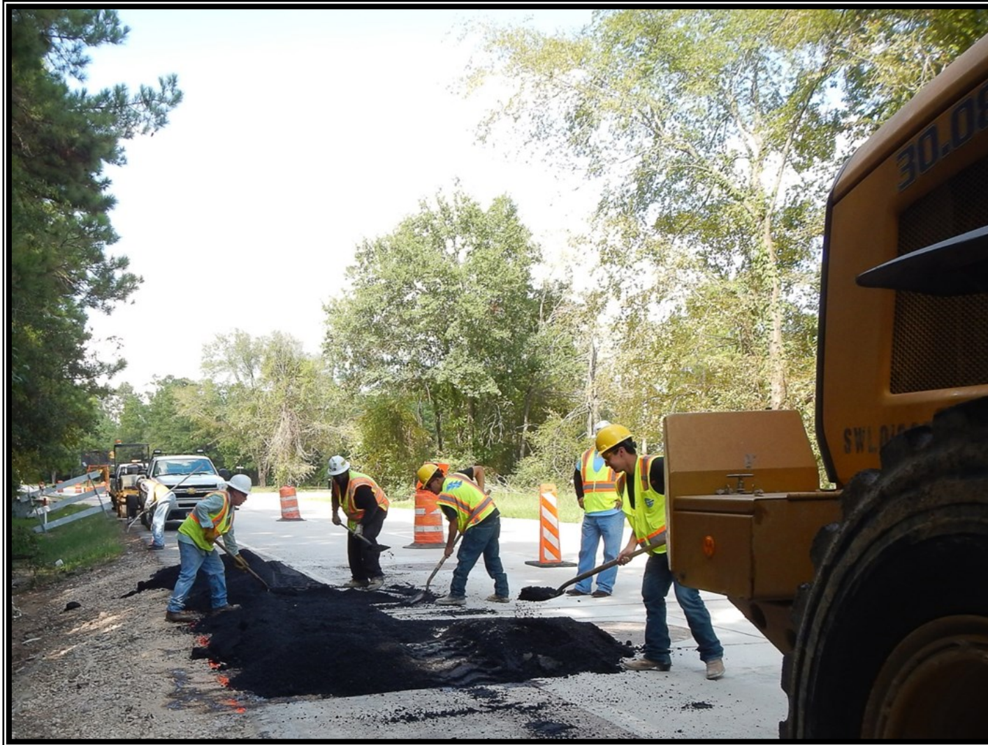
① Segment W2B - Asphalt shoulder restoration along Grogans Mill Road at Evergreen Circle
