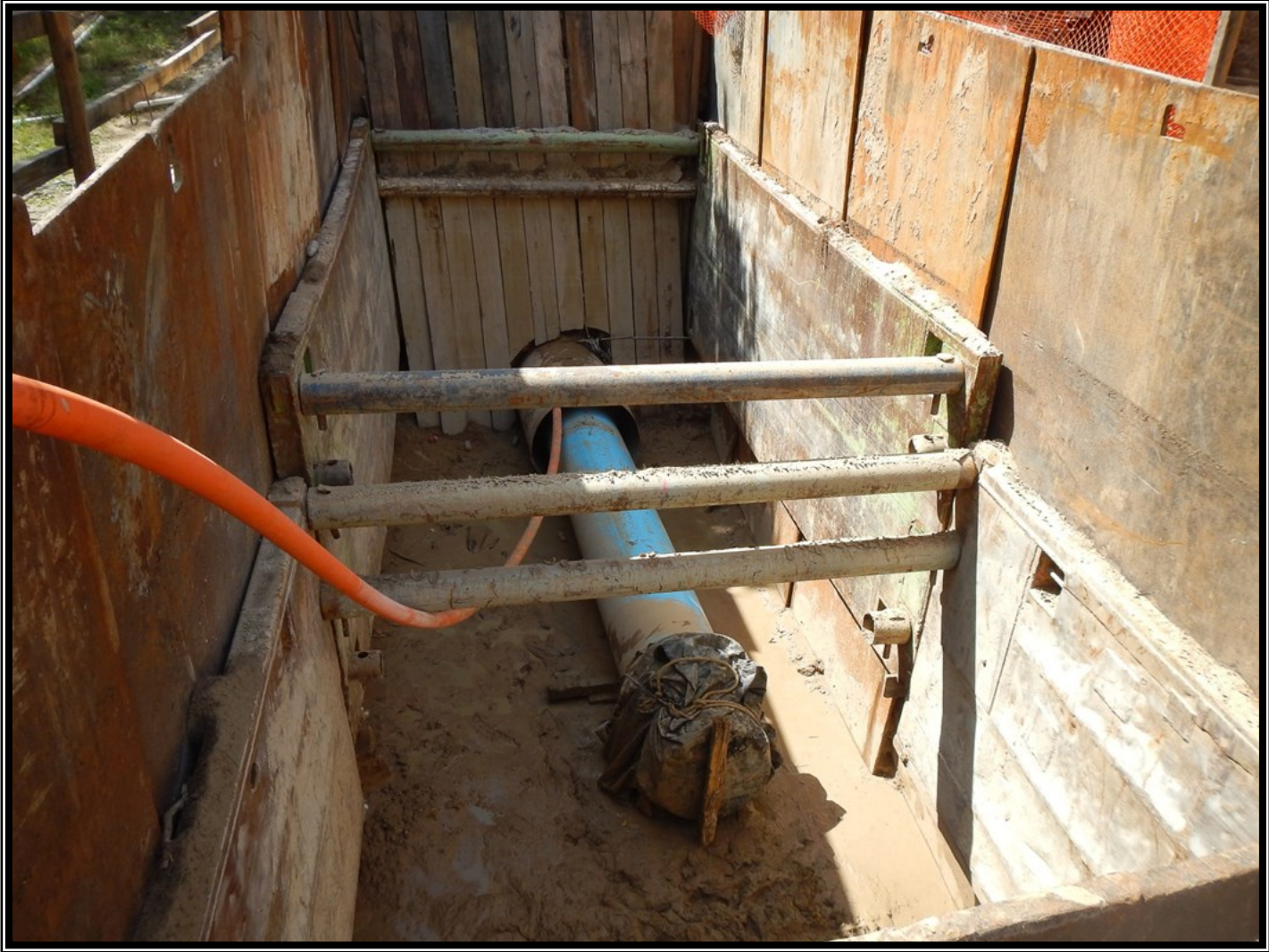
① Segment W2A— 30-inch pipe and fiber optic conduit installation along Research Forest
