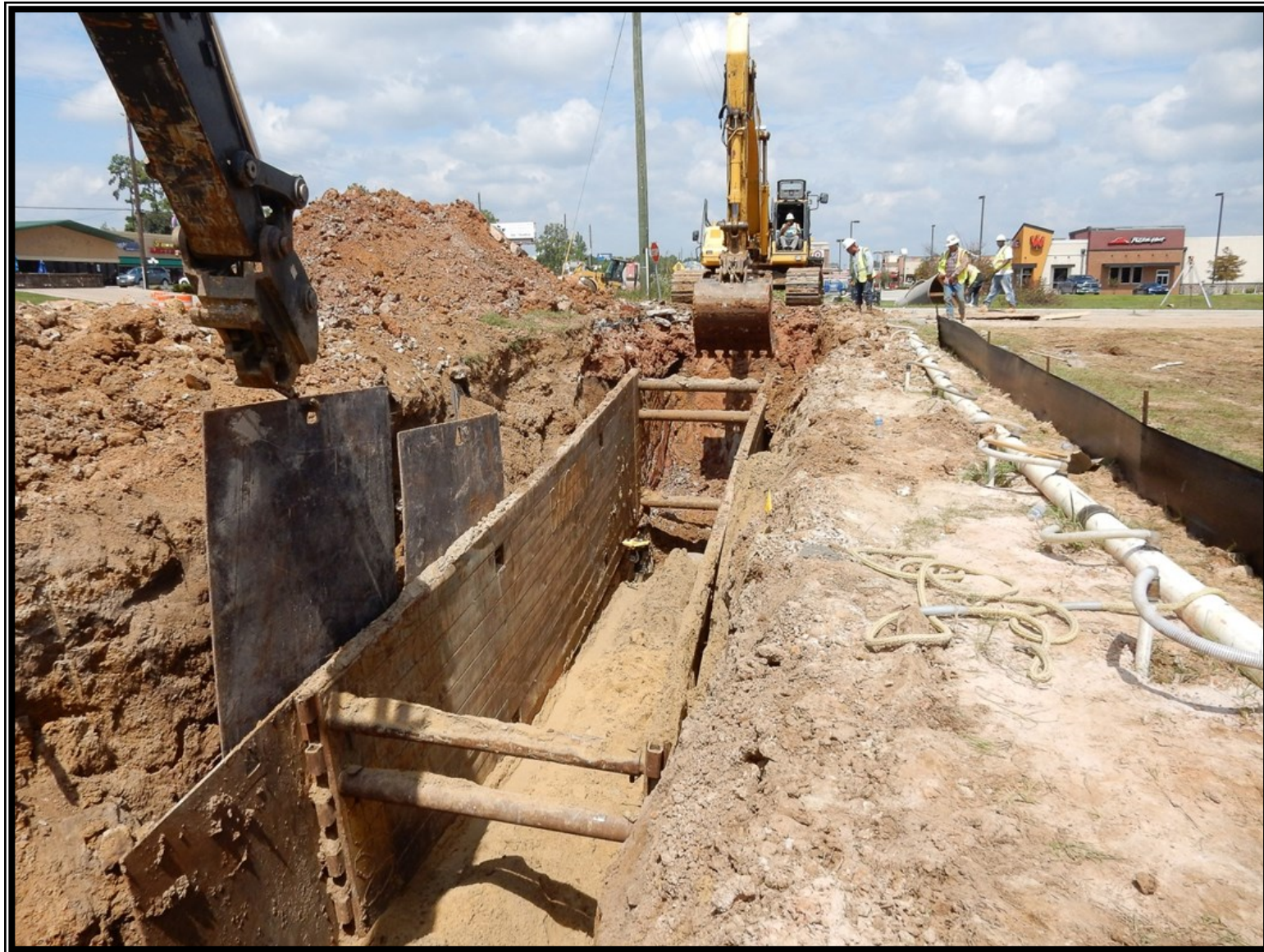
① Segment T3— 54-inch open-cut pipe installation along FM 2978 south of FM 1488
