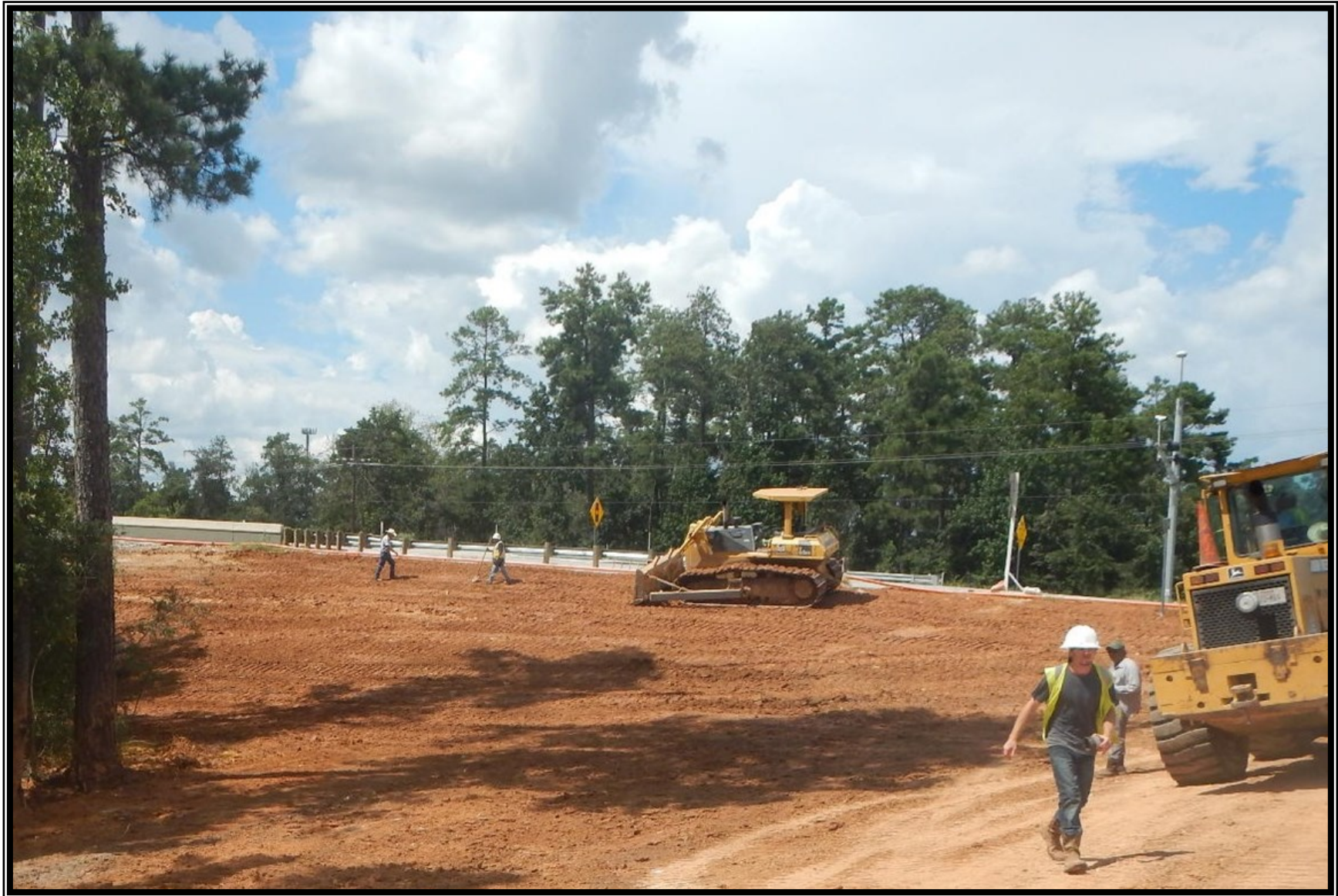
① Segment C4—Site restoration along FM 830 at I-45
