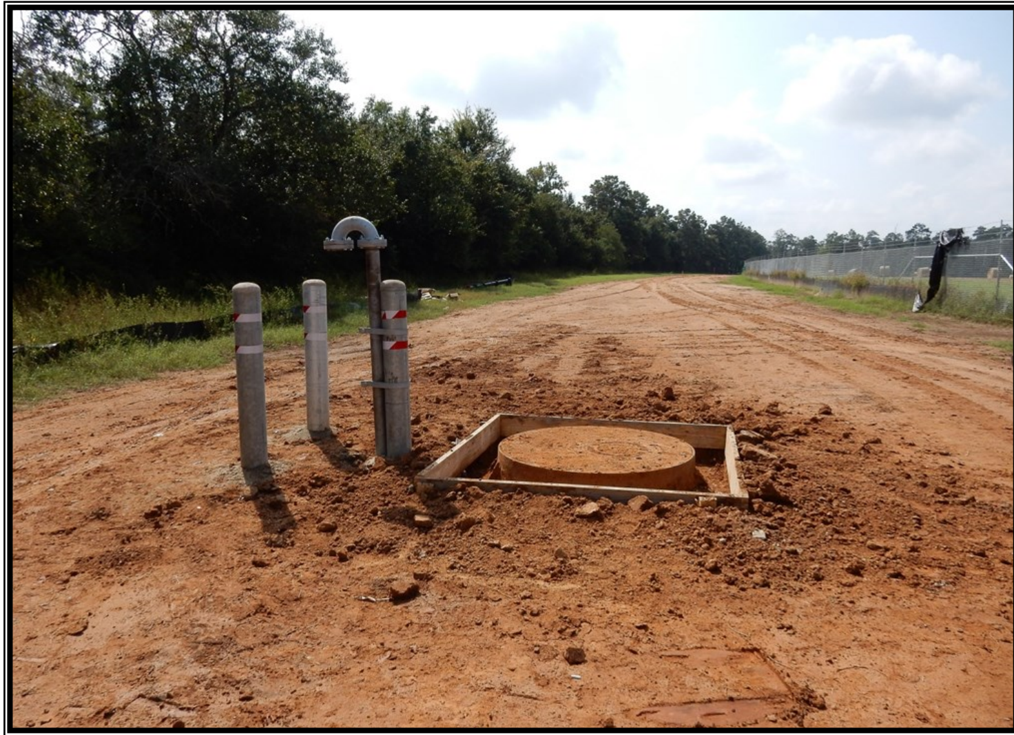
① Segment C3— Air release and vacuum relief valves along Girl Scout property
