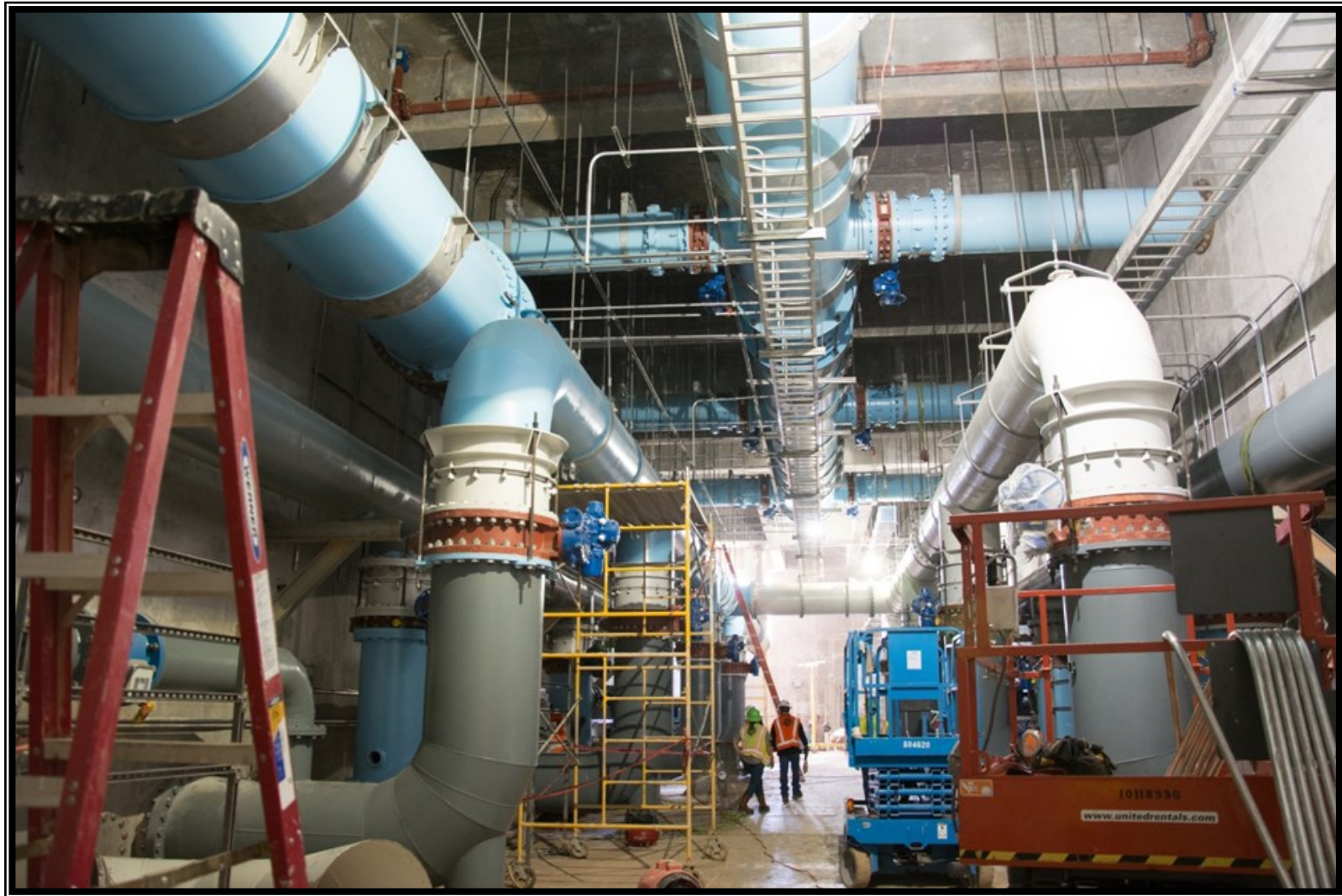
④ Piping and instrumentation installation at the Granulated Activated Carbon (GAC) Building
