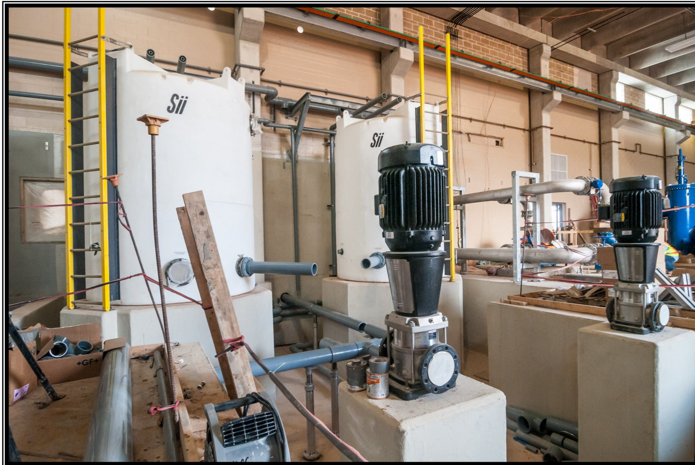
③ Chemical storage tank and feed pumps at the Membrane Building
