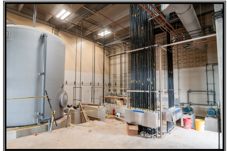
Fiberglass electrical conduit at the Chemical Building
