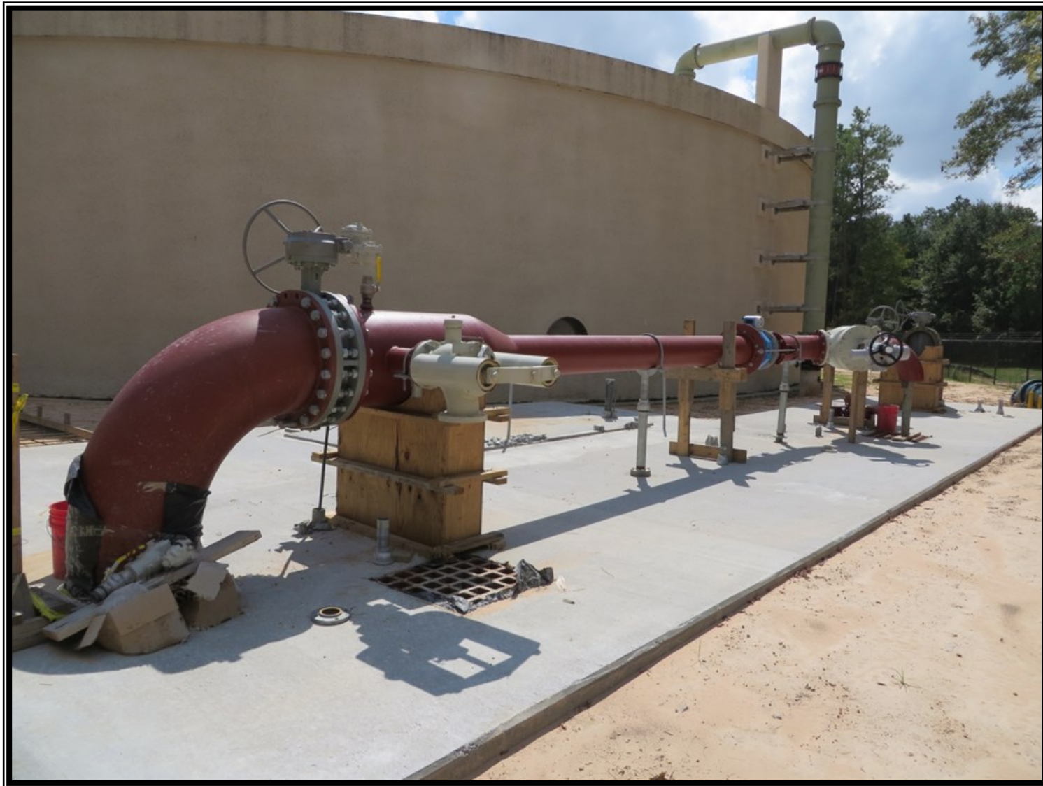
① Surface Water Receiving Facility – South — Flow Control Pressure Station at Woodlands Water Plant No. 1
