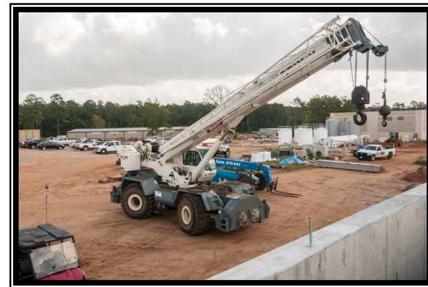
Crane utilized for placement of plate settlers at the Pretreatment Facilities
