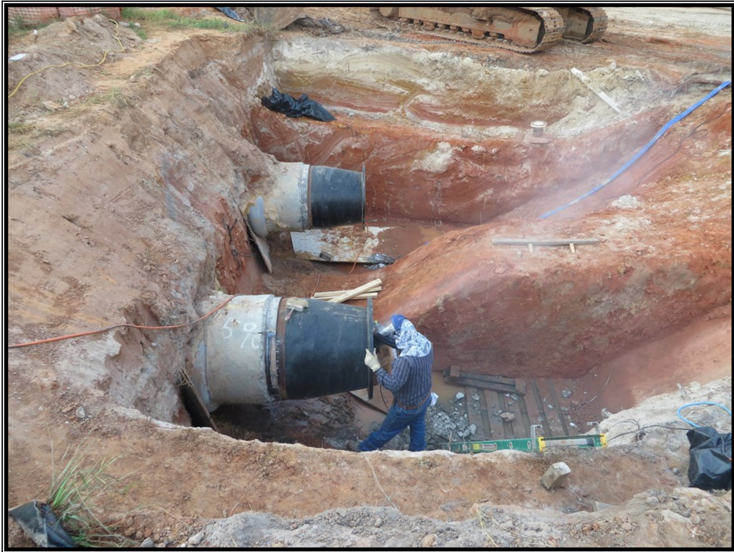
① Surface Water Standpipe—36-inch x 30-inch pipe reducer connections to Standpipe
