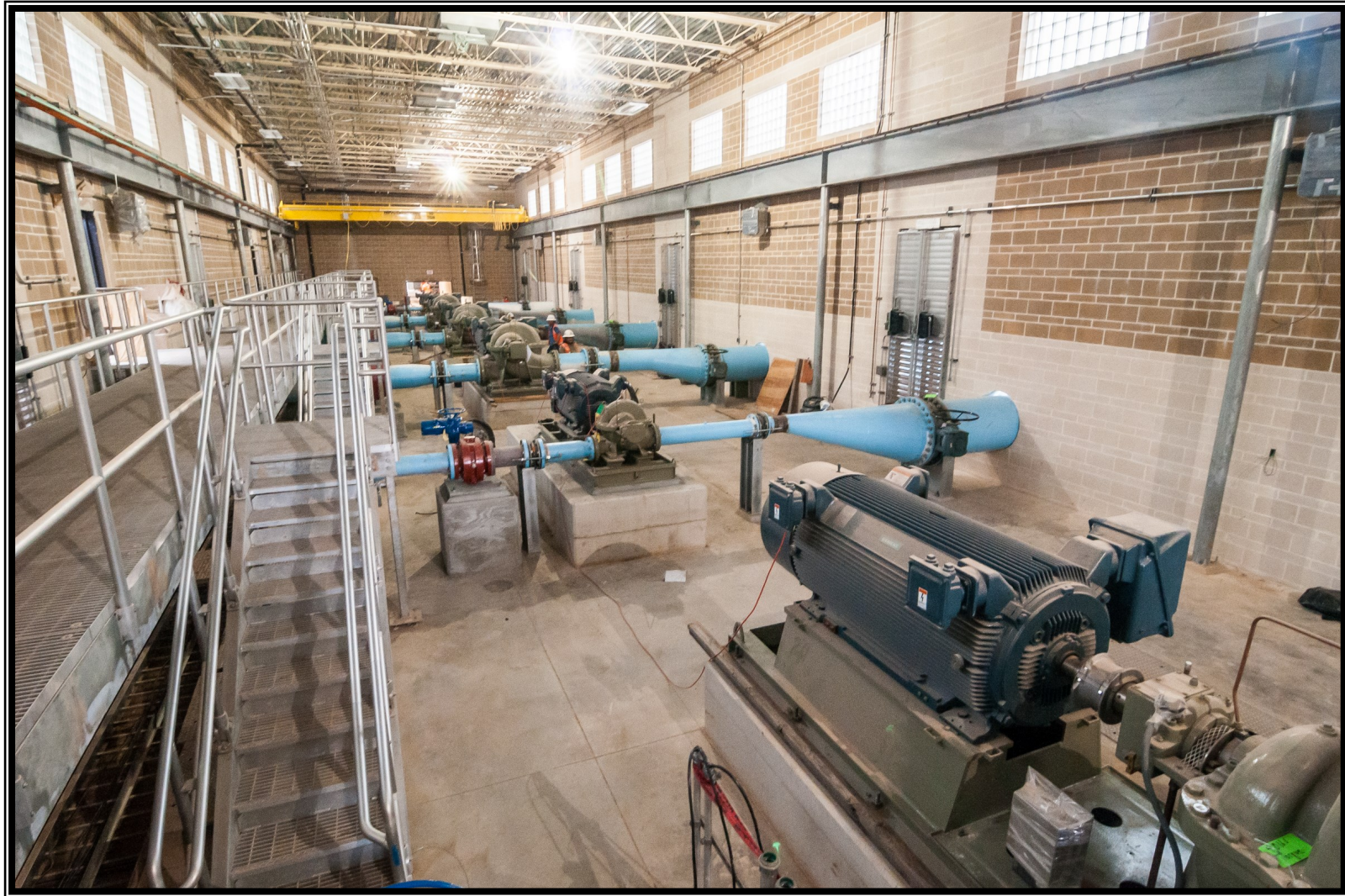
⑤ Pump and motor assemblies at the High Service Pump Station
