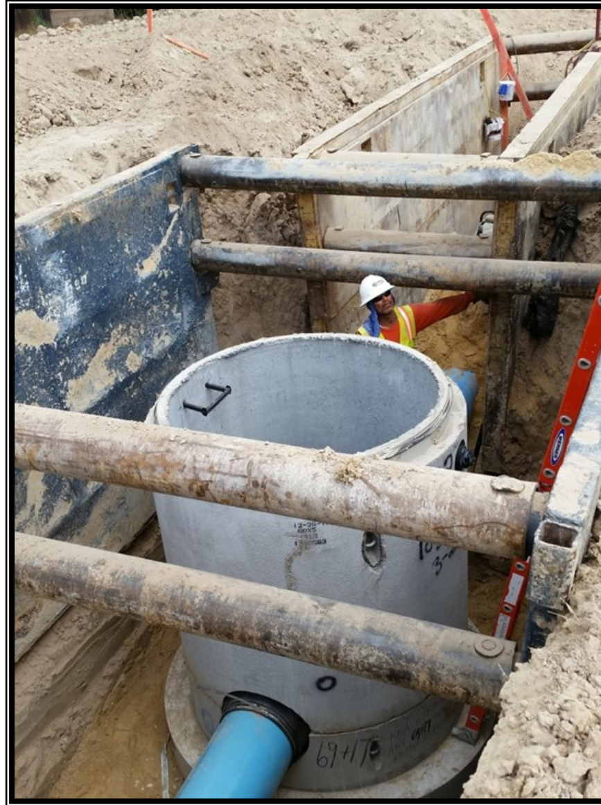
① Segment W3B - Air vacuum relief valve manhole installation
