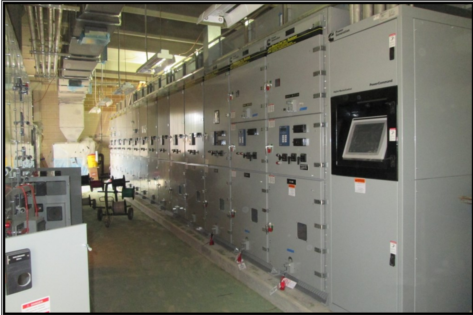
⑧ Paralleling switch gear installation in the Electrical Building
