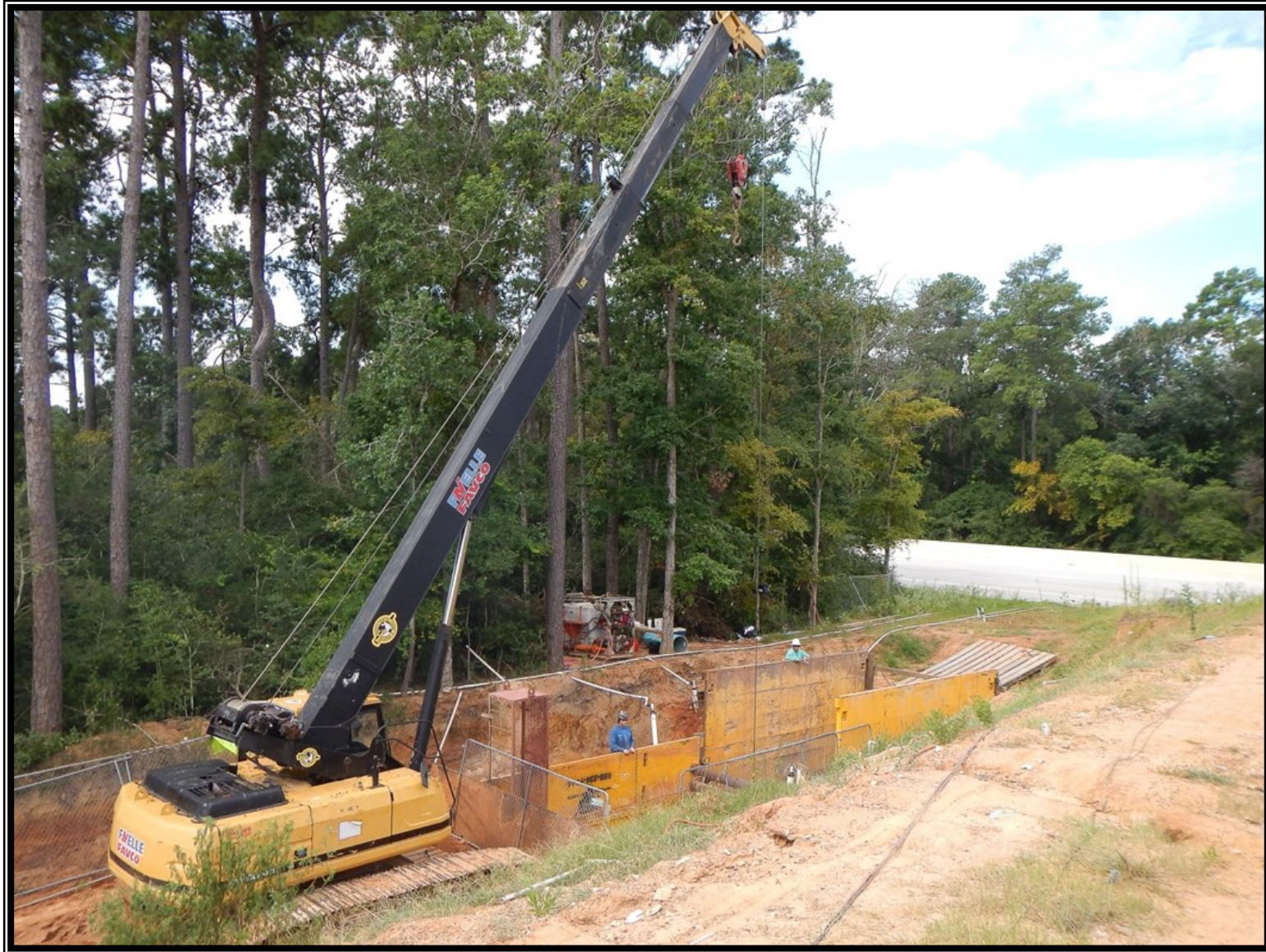
① Segment C4—Tunnel operation for 20-inch waterline installation under I-45
