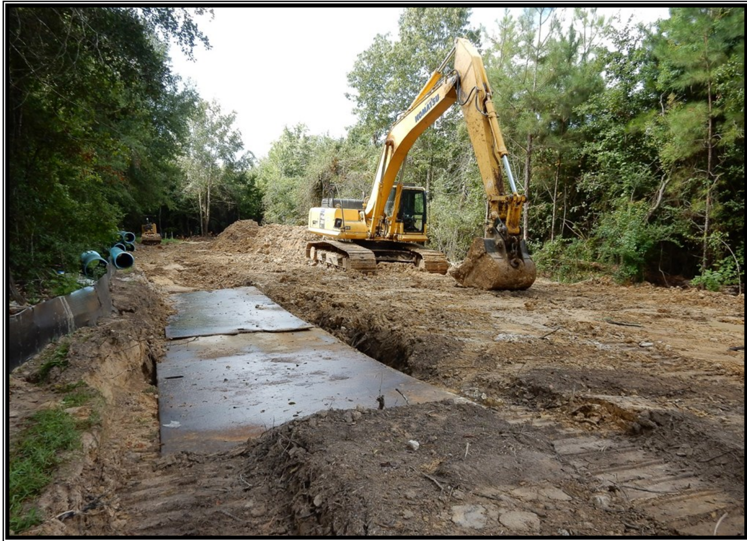
① Segment C3— Open-cut pipe installation adjacent to Union Pacific Railroad property
