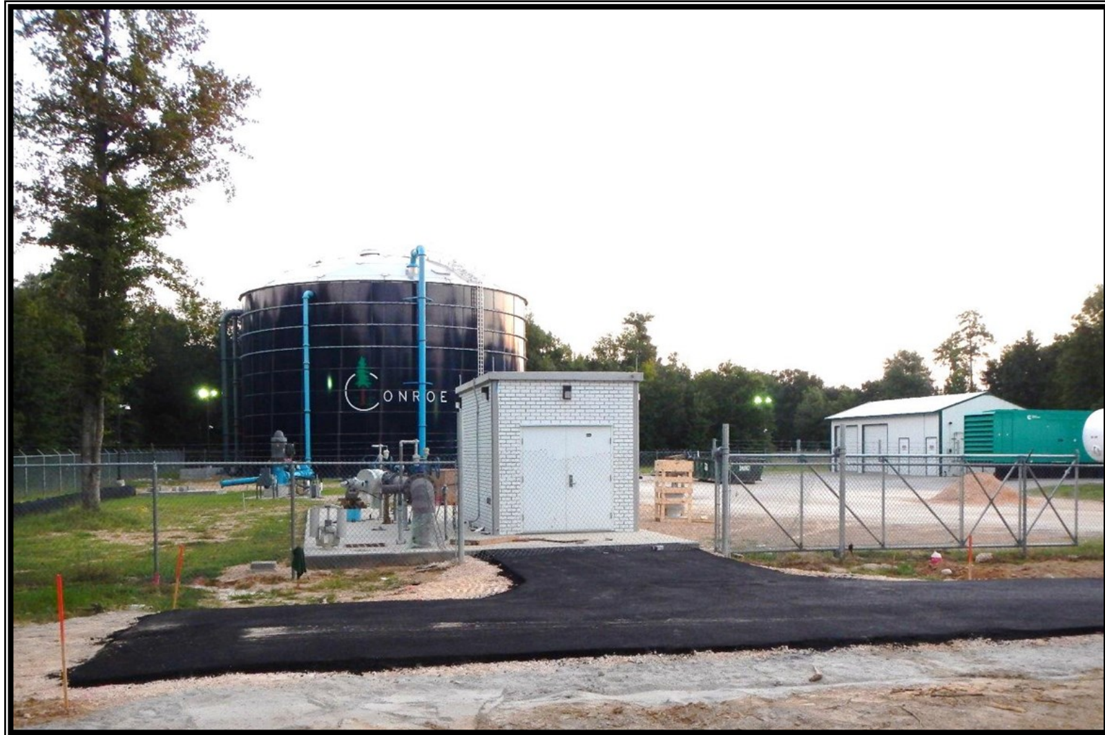
① Surface Water Receiving Facility – North— Site work at Conroe Water Plant No. 22
