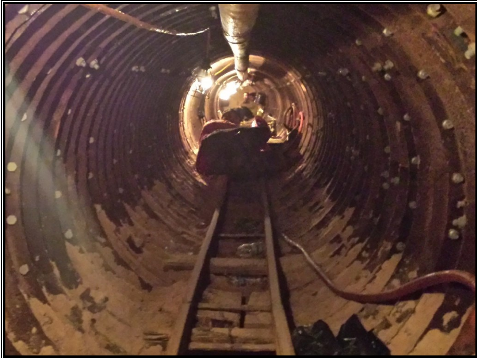
① Segment W3B - Interior view of 52-inch steel liner tunnel under I-45
