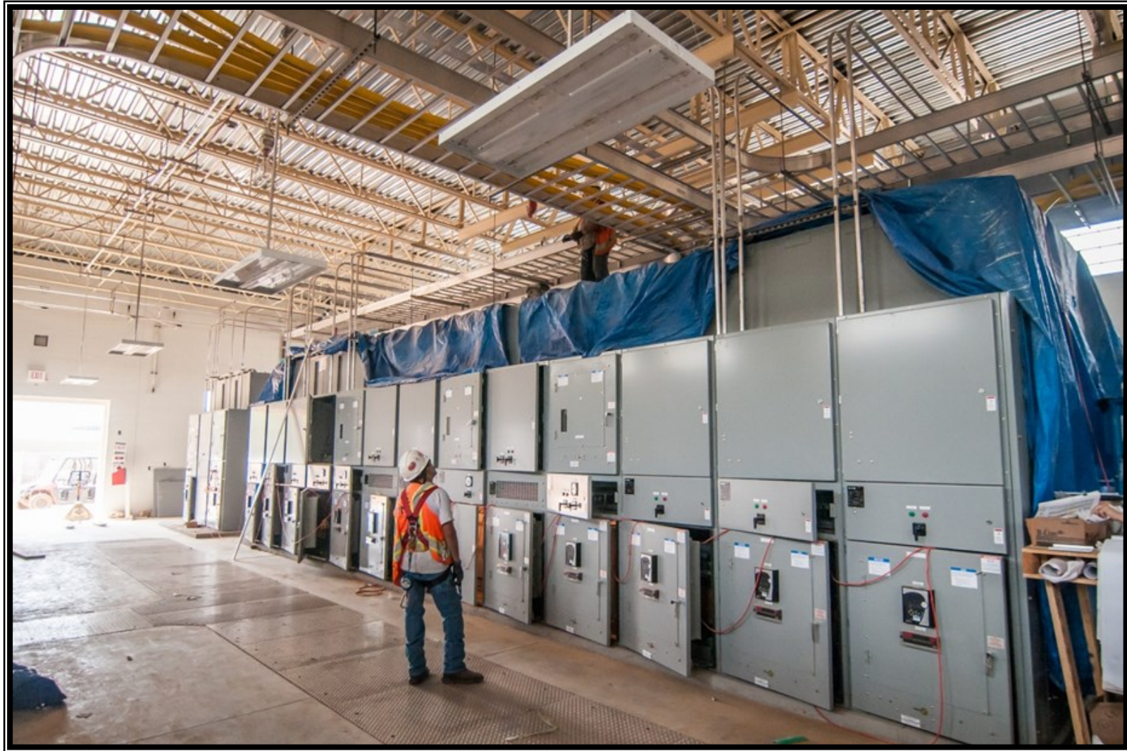
⑤ Electrical gear installation at the High Service Pump Station
