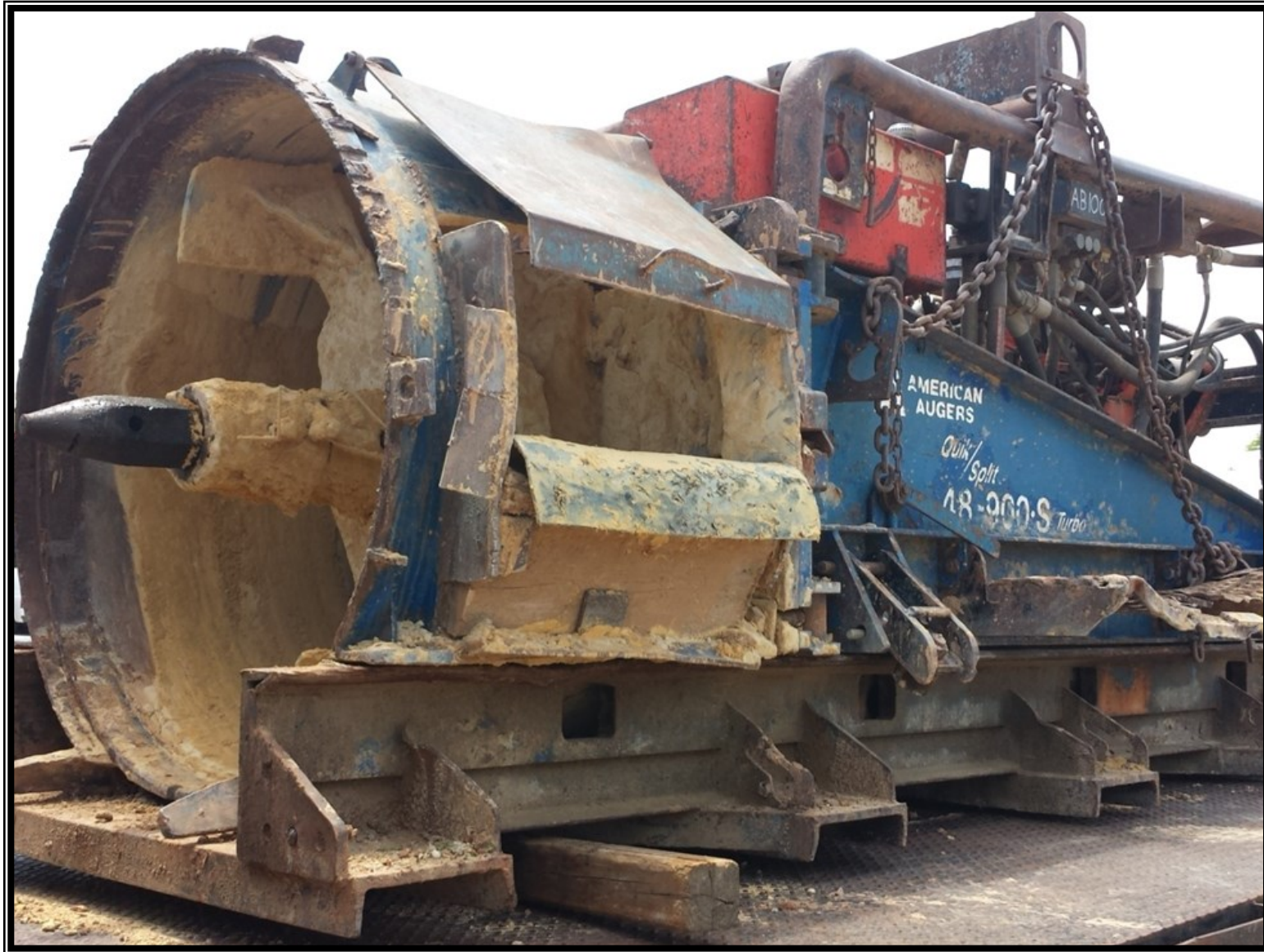
① Segment W3B - 36-inch dry bore auger machine for Rayford Road Crossing
