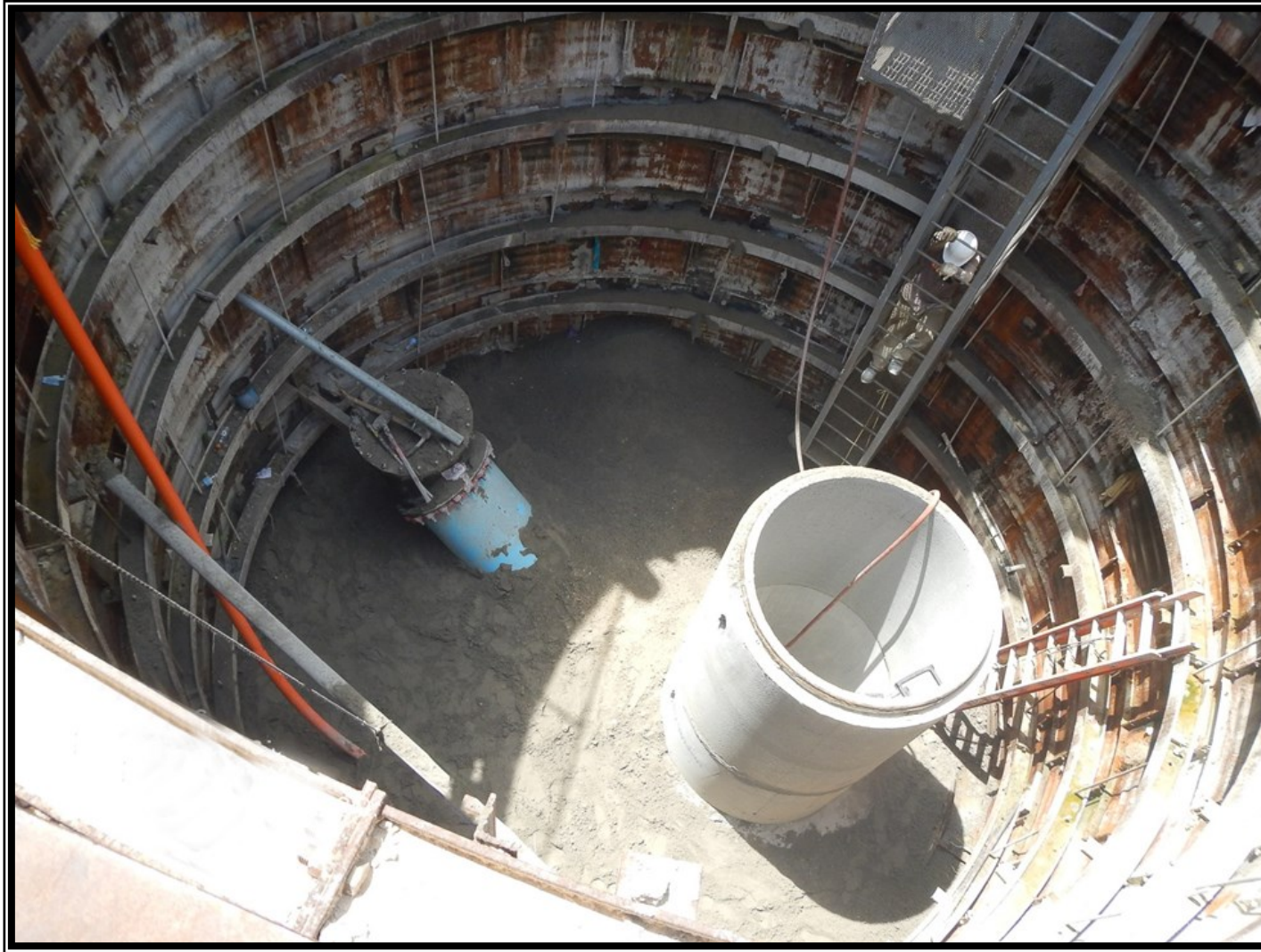
❶ Segment W2B - Backfilling of bore pit for Woodlands Waterway crossing
