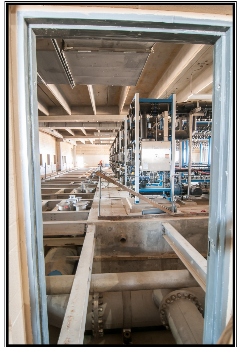
Left: Air relief and closure valve located in the Pump Room at the Membrane Building
