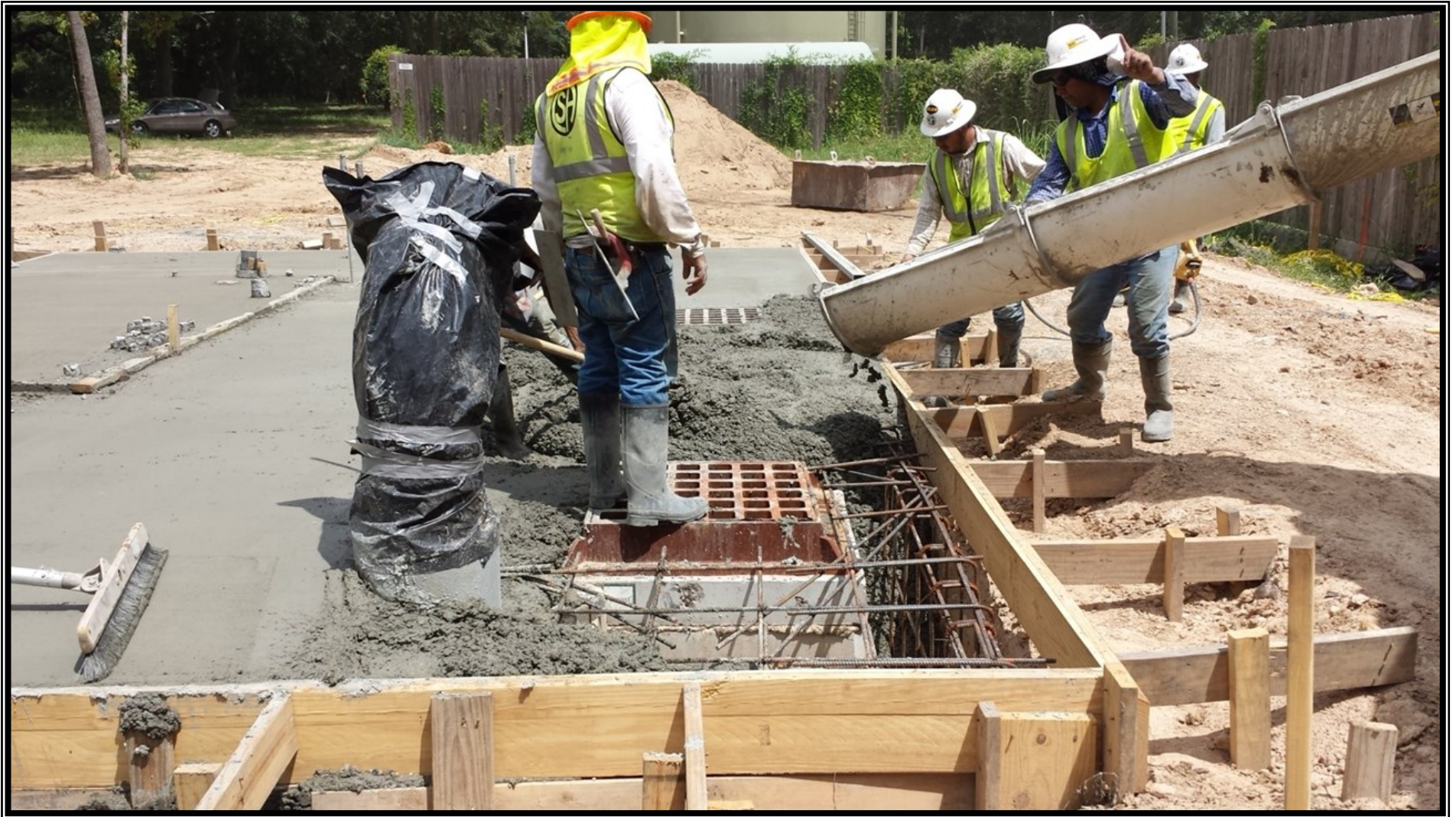
① Surface Water Receiving Facility – South — Flow Control Pressure Slab installation at Woodlands Water Plant No. 1
