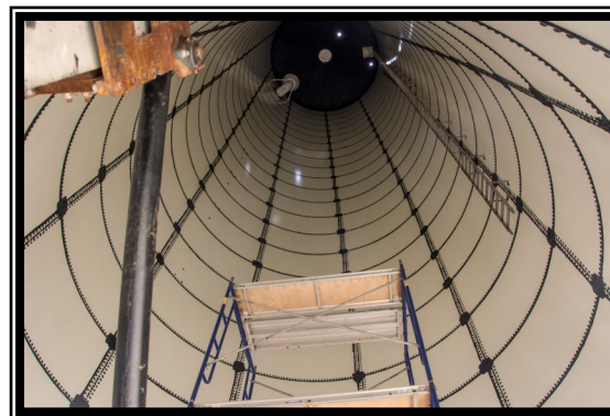
View from ground level to the top of Standpipe located near Conroe Water Plant No.
