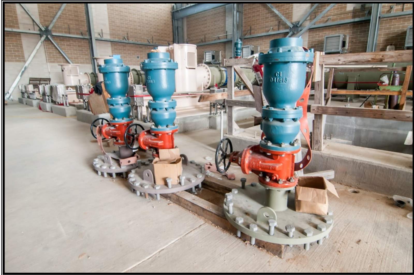
① Pressure reducing valve assemblies in the Raw Water Intake and Pump Station
