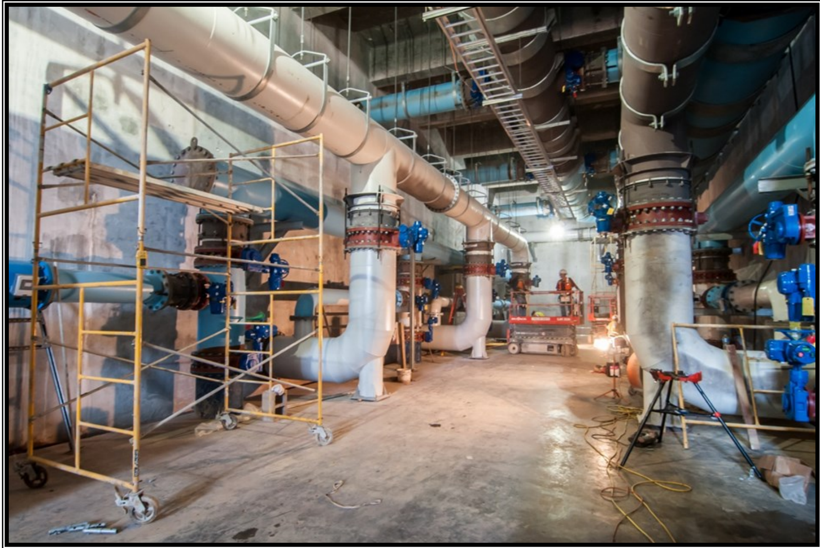
④ Process water piping installation at the Granulated Activated Carbon Building
