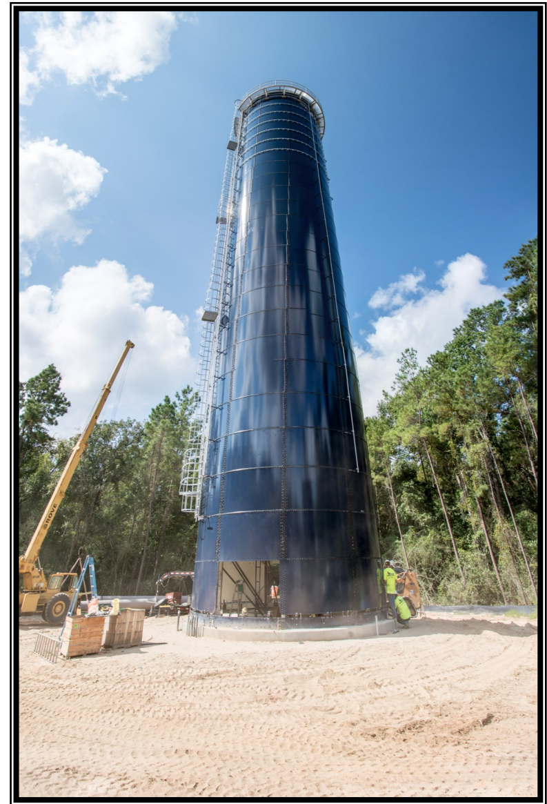
Standpipe construction near Conroe Water Plant No. 21
