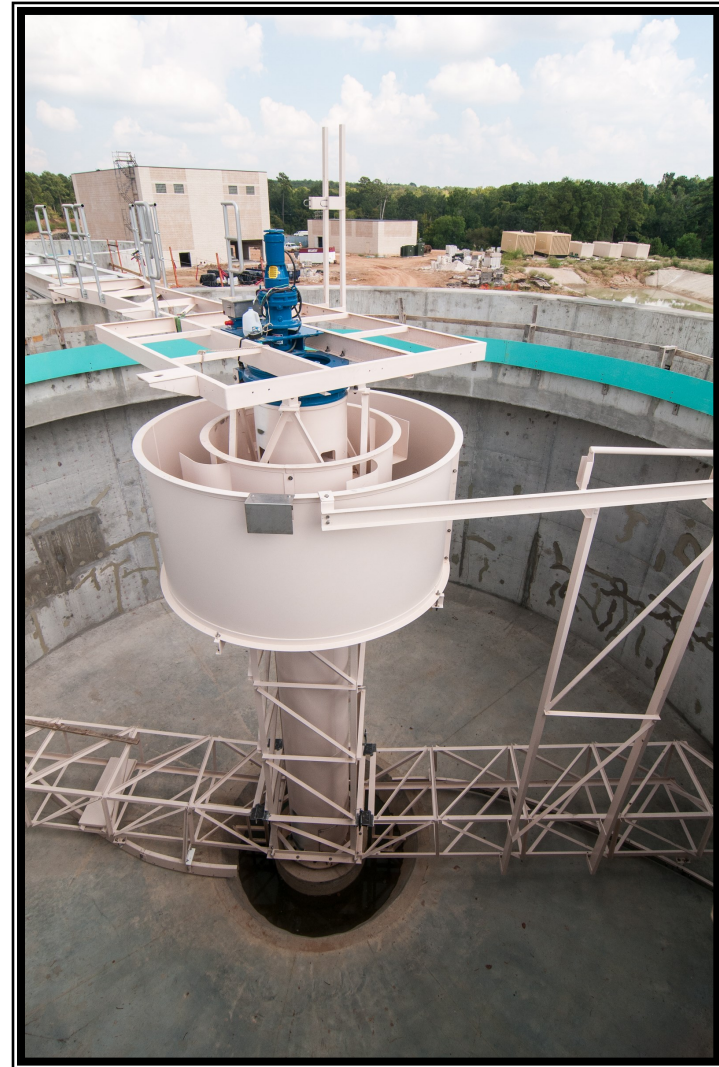
Center column of the sludge thickener at the Surface Water Facility
