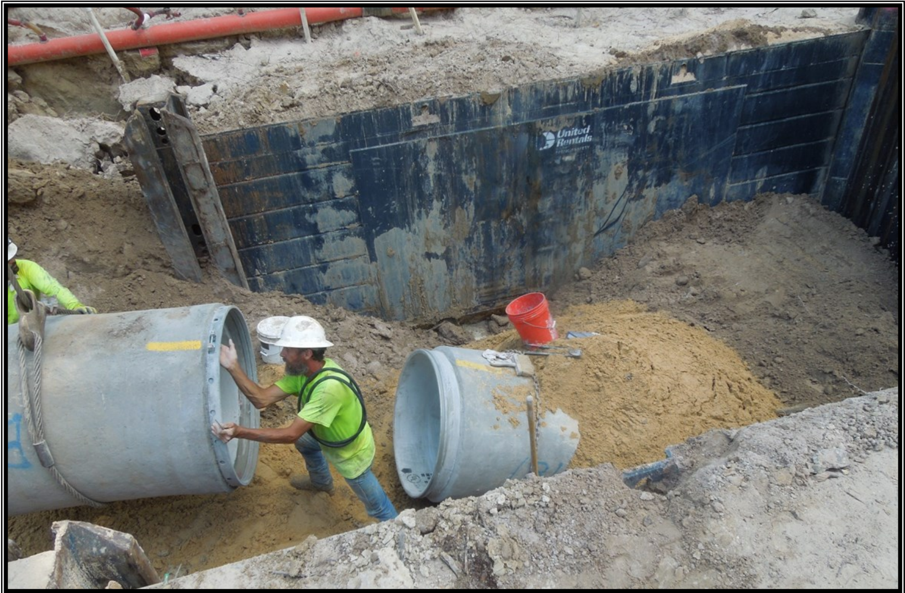
① Segment C2— 36-inch open-cut pipe installation along Entergy easement
