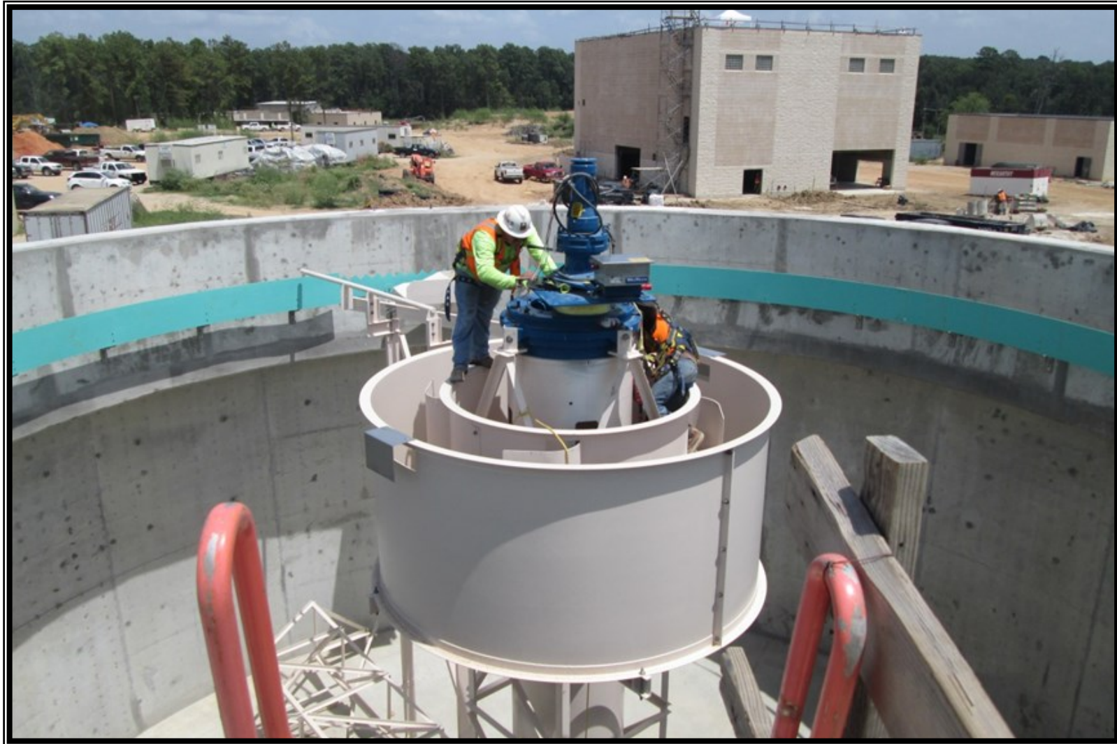
① Installation of mechanical equipment at the Sludge Thickeners
