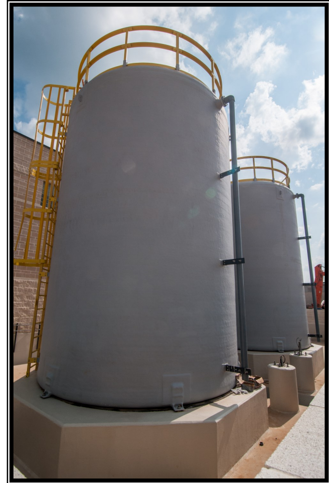
Aluminum Chlorohydrate storage tanks at the Chemical Storage Facility
