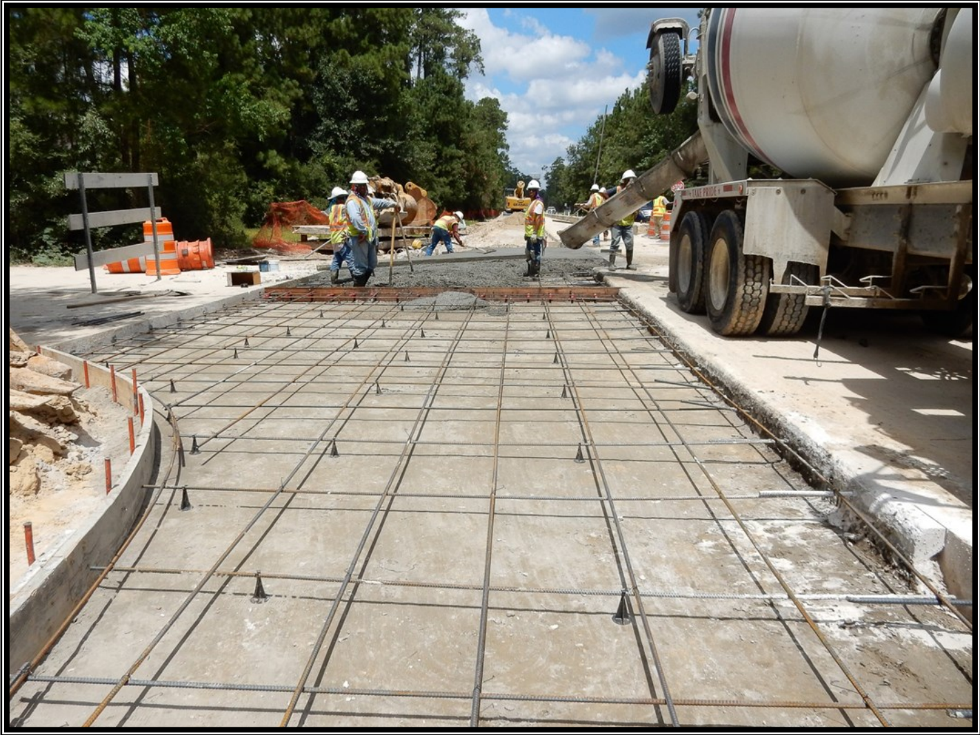
❶ Segment W2A— Pavement restoration along Research Forest
