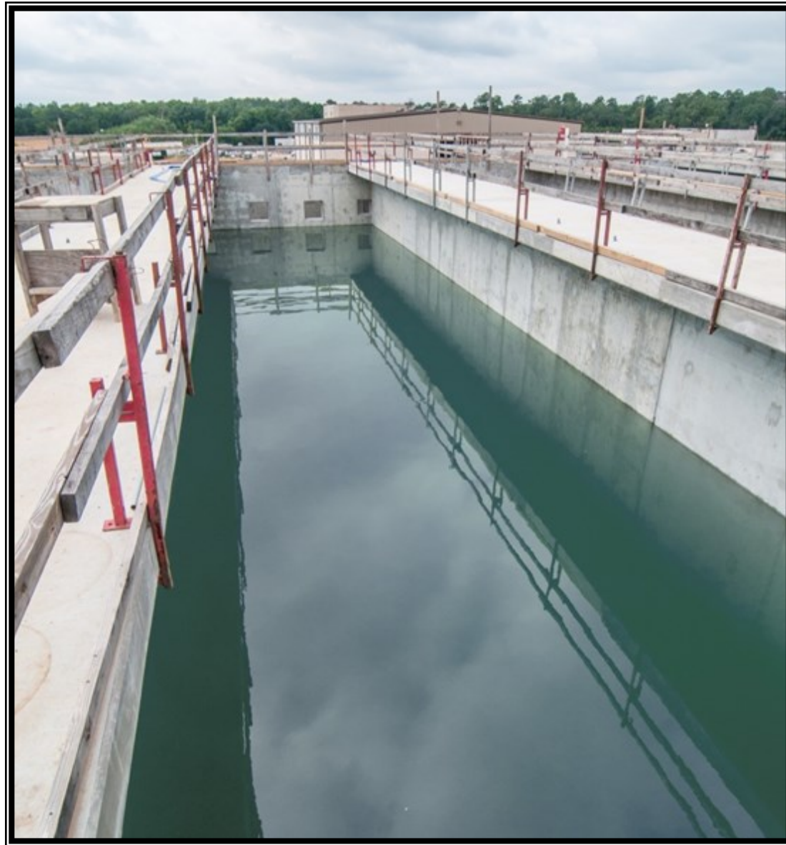
② Leak testing procedure at the Pretreatment Facility
