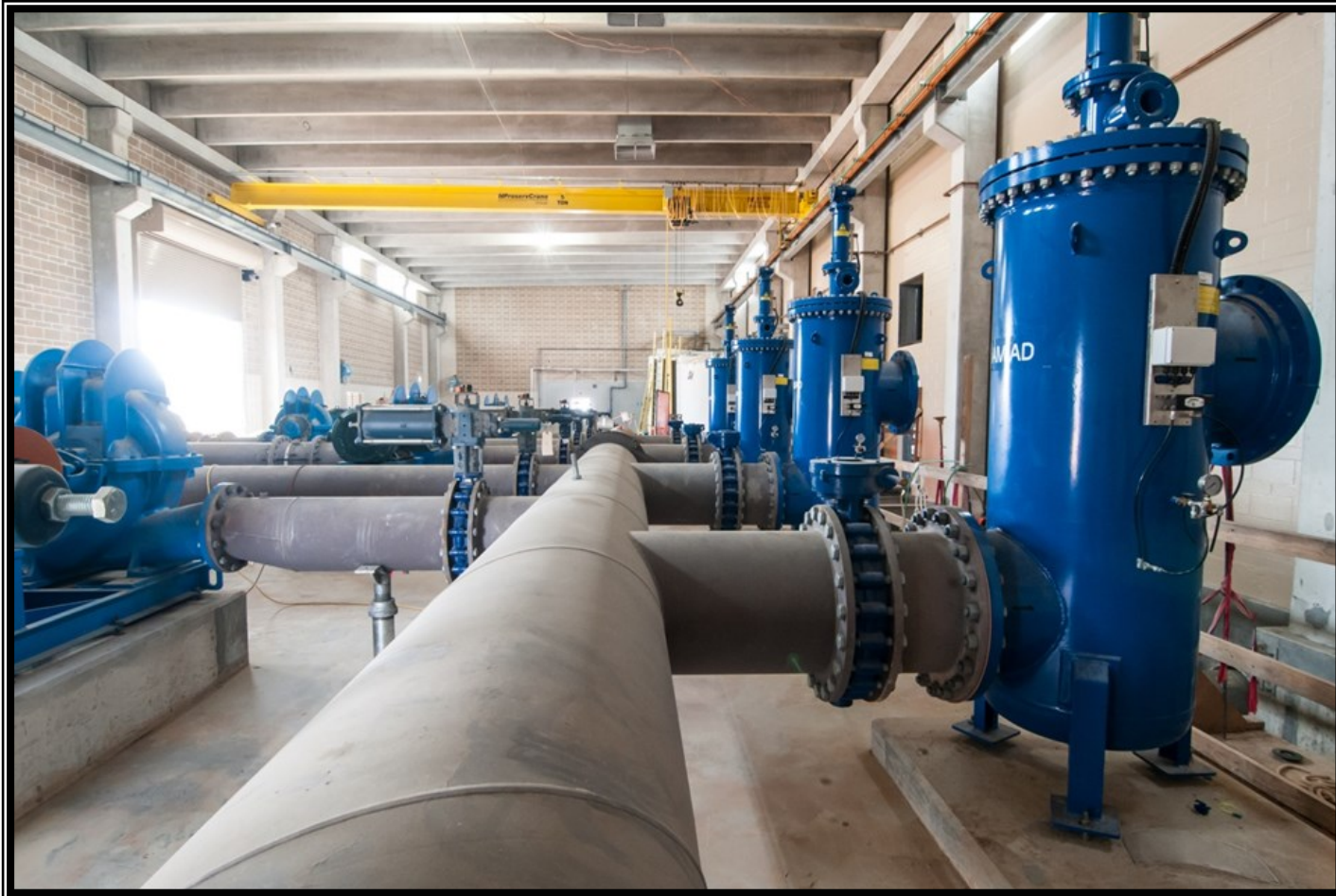
③ Supply header and strainer installation at the Membrane Building
