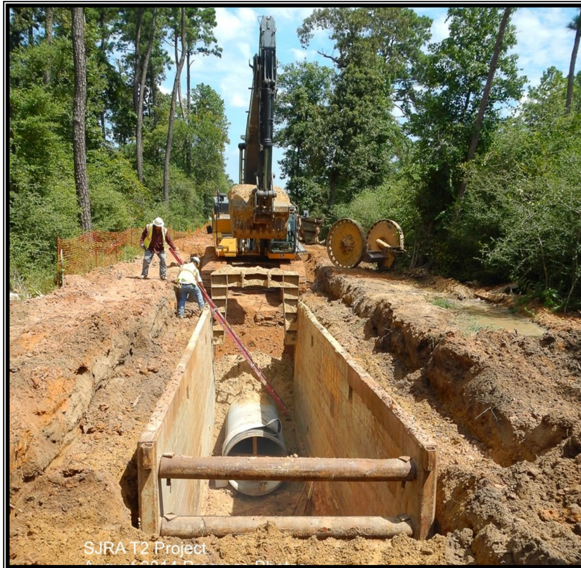
① Segment T3— 54-inch pipe installation along Sendera Ranch Road
