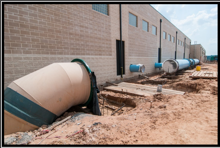
Intake suction header installation at the High Service Pump Station
