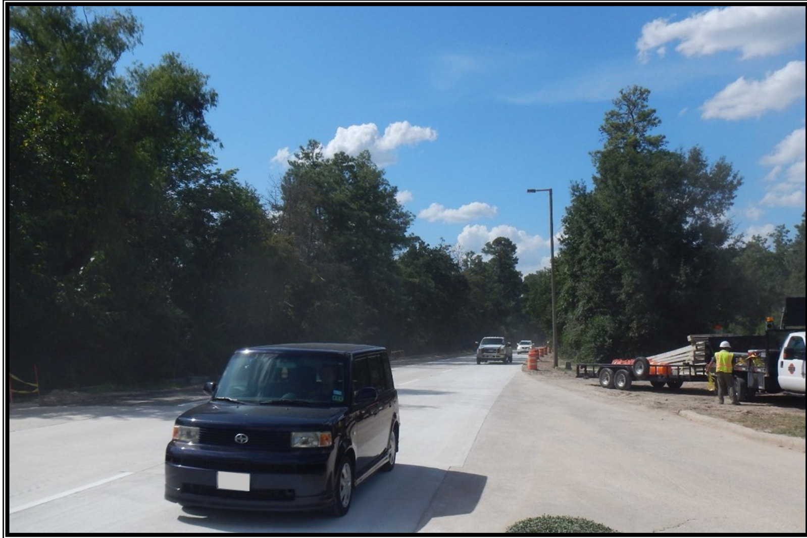
① Segment W3A - Traffic restoration at Grogans Mill Road and Millpark Drive
