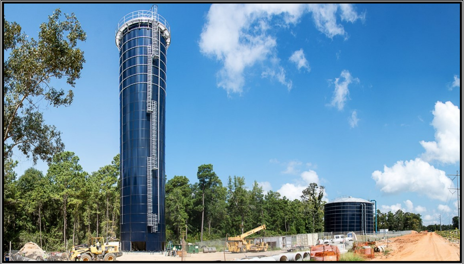
❶ Surface Water Standpipe—Standpipe tank installation (120 feet tall and 25 feet in diameter) at Conroe Water Plant No. 21
