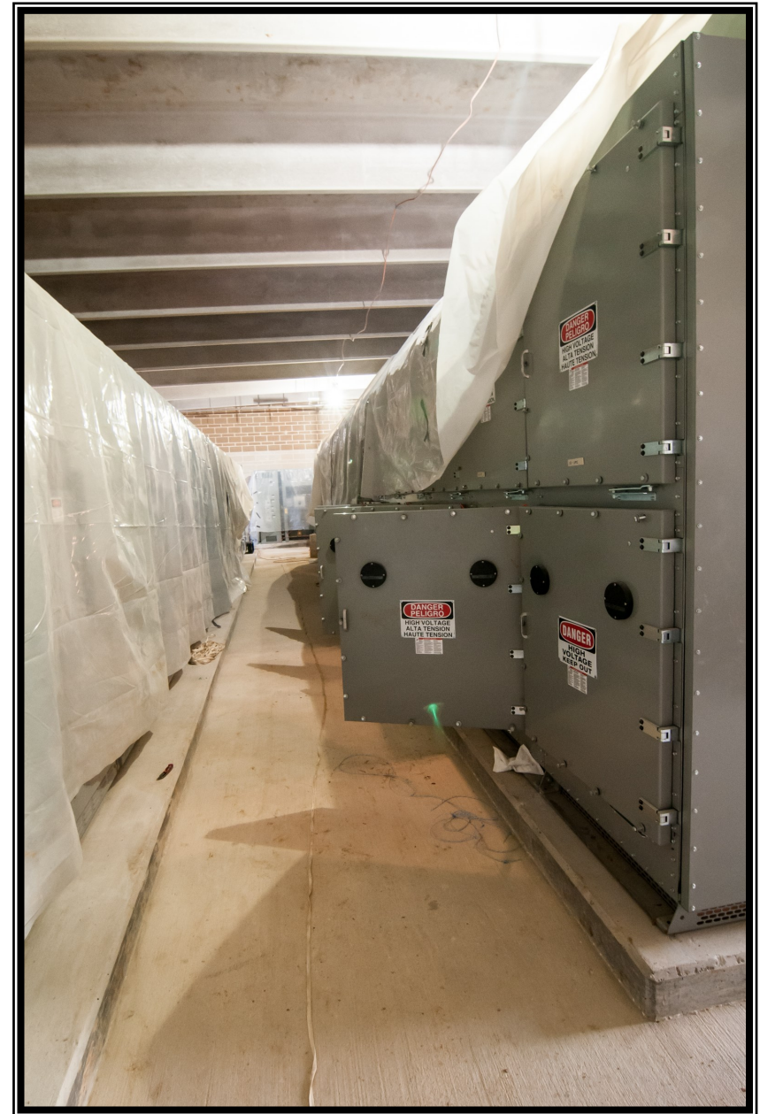
Switchgear installation at the Power Supply Building at Surface Water Facility
