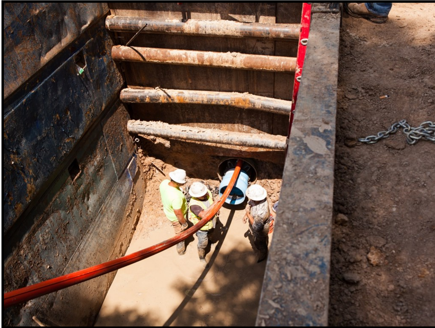
① Segment W3B— Pipe installation along Montgomery County Drainage District No. 6 right-of-way
