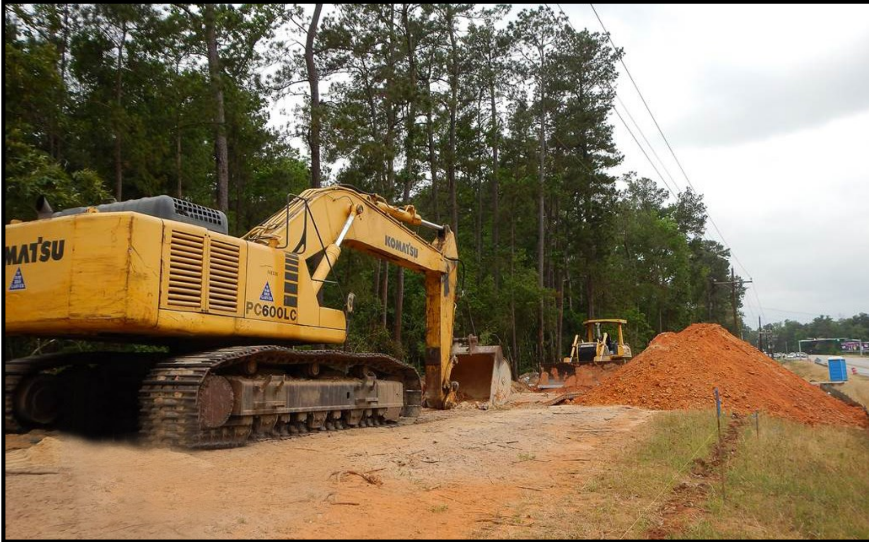
① Segment C4—24-inch pipe installation along FM 830
