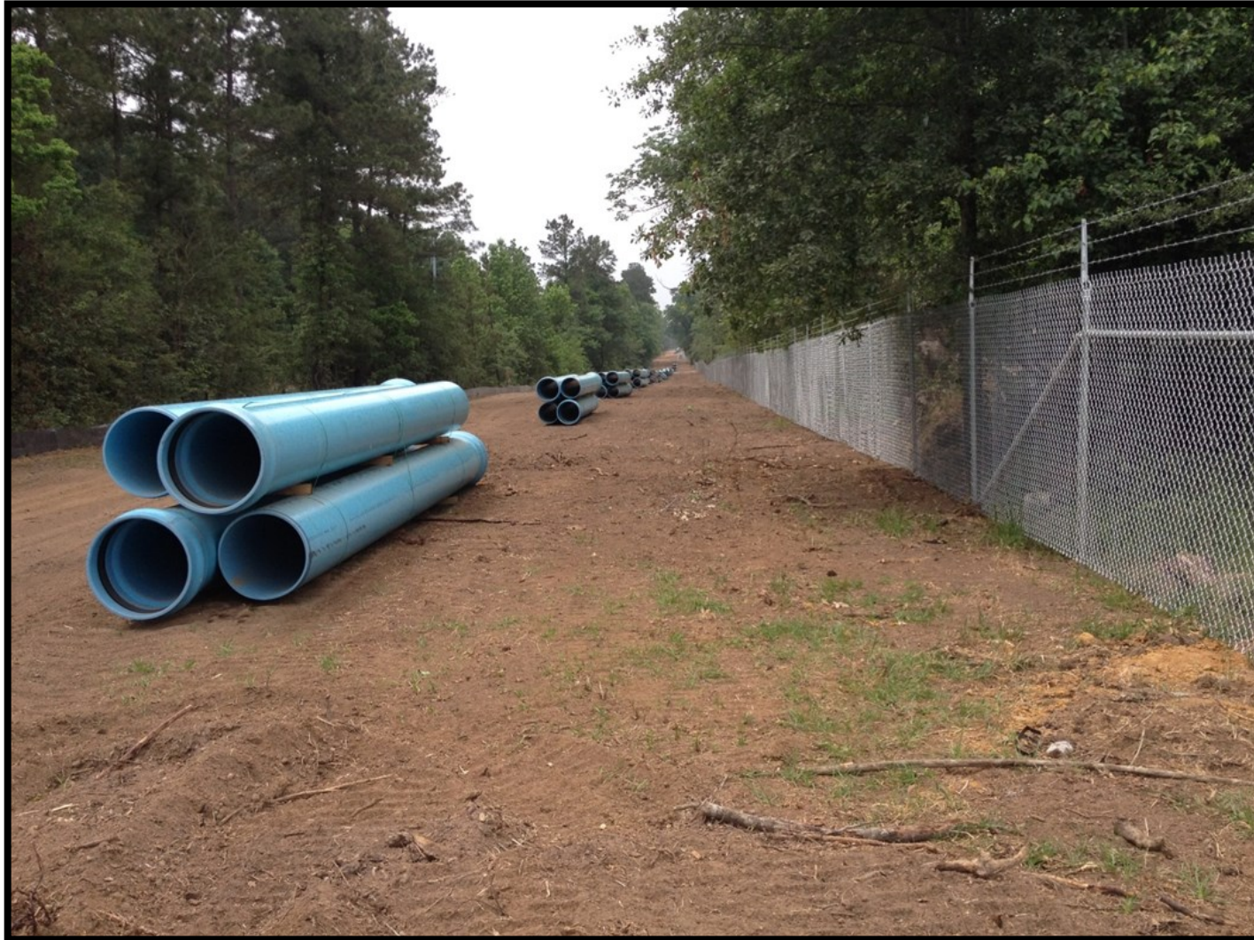
① Segment C3— Staging of pipe materials along Girl Scout property
