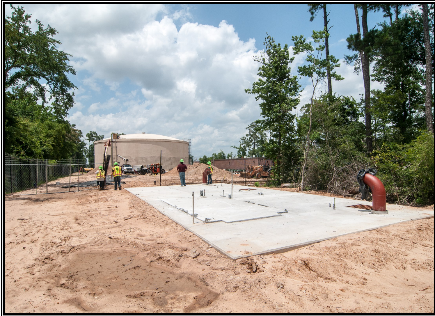
① Surface Water Receiving Facility – South —Control Building Foundation at SJRA Water Plant No. 5
