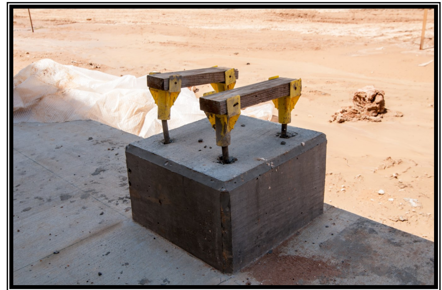
Column support outside of the Blower Building at Surface Water Facility
