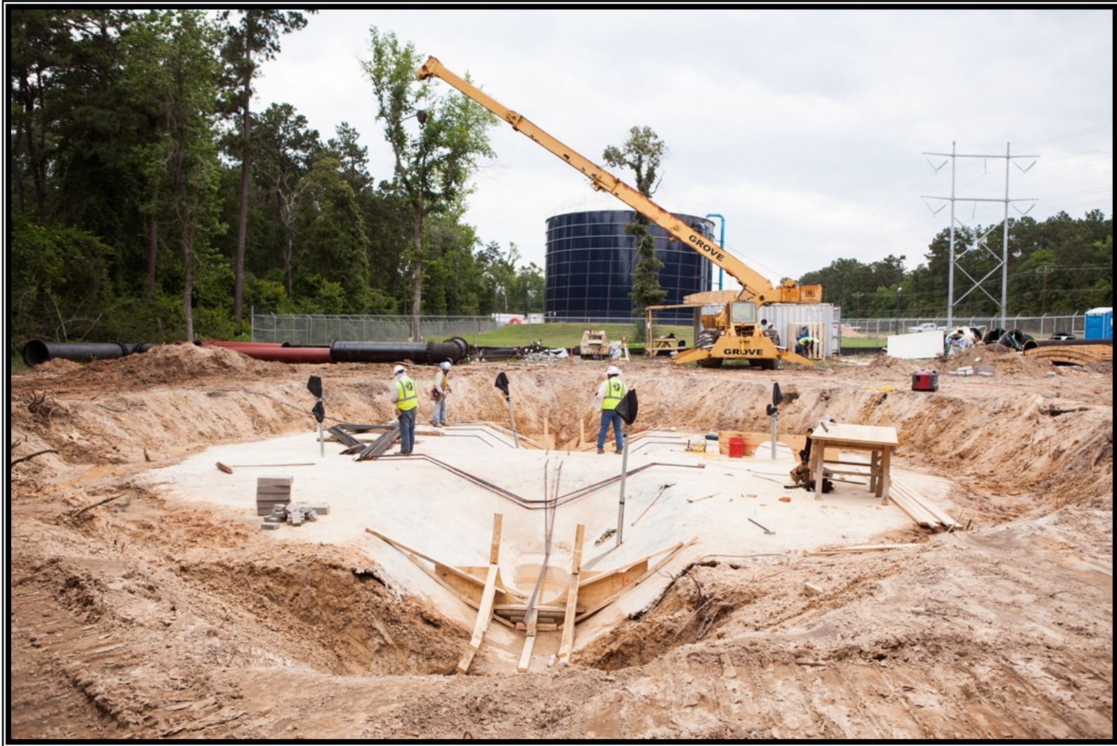
① Surface Water Standpipe—Reinforced steel and formwork installation
