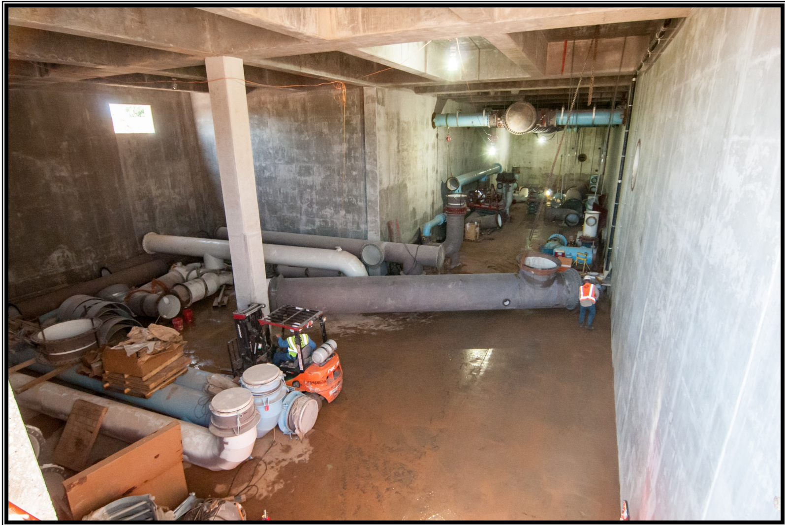
③ Pipe gallery installation at the Granulated Activated Carbon Building
