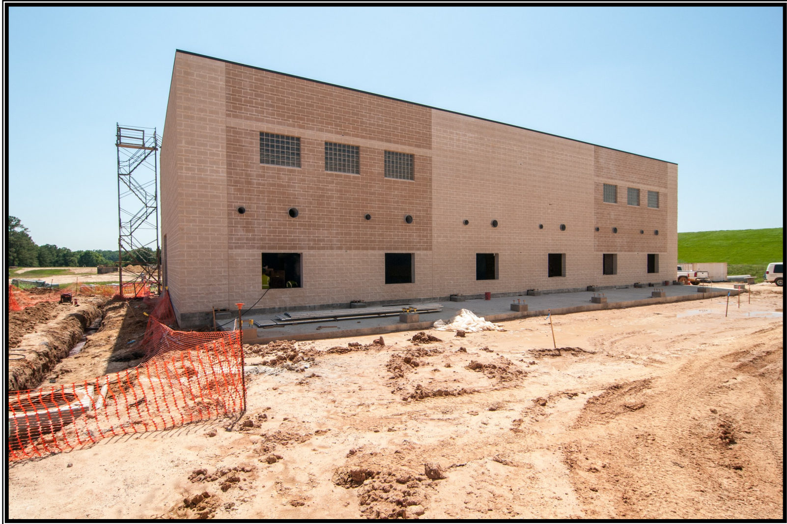
⑥ View of east side of Blower Building
