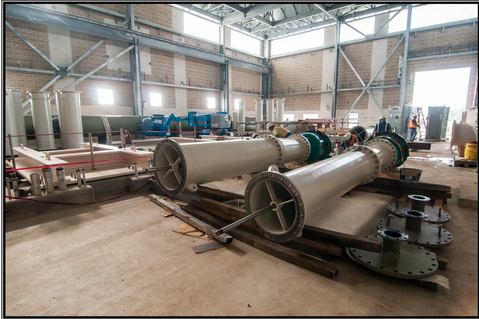
❶ Pump barrel installation at Raw Water Intake and Pump Station
