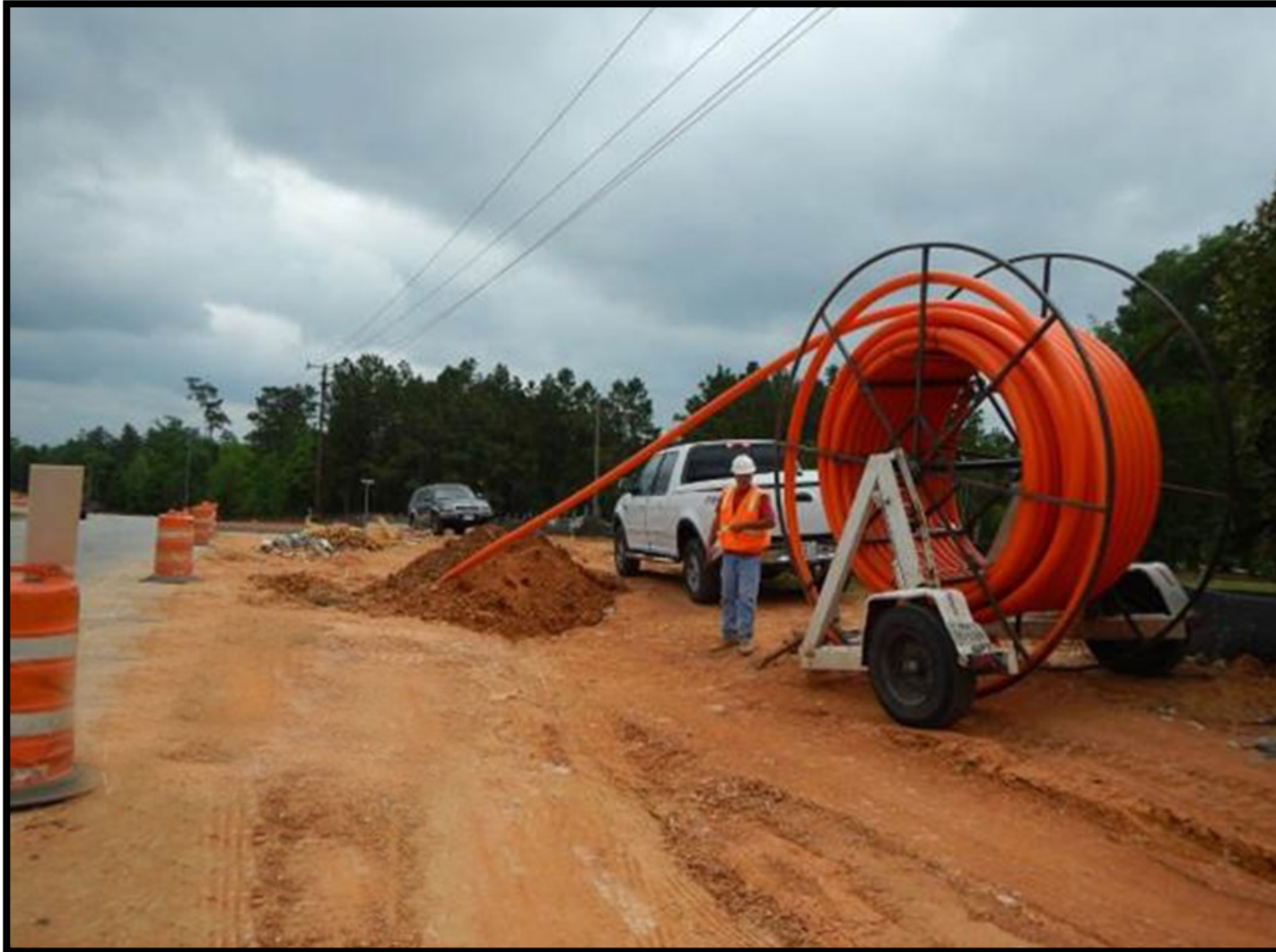
① Segment T2 - Fiber optic conduit installation along Fish Creek Thoroughfare
