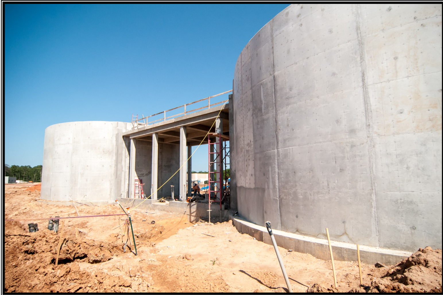
⑧ Pump Room concrete roof installation at the Sludge Thickeners
