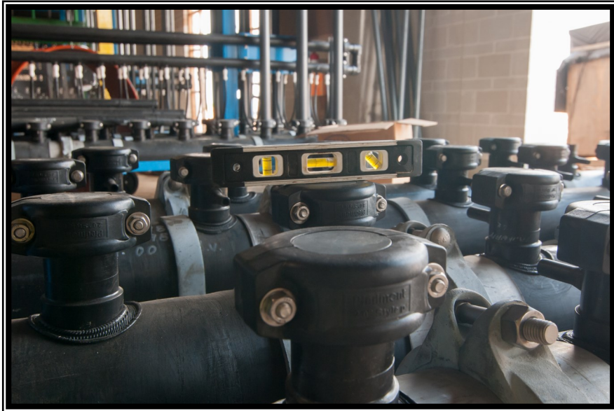
Membrane installation at the Membrane Building at Surface Water Facility
