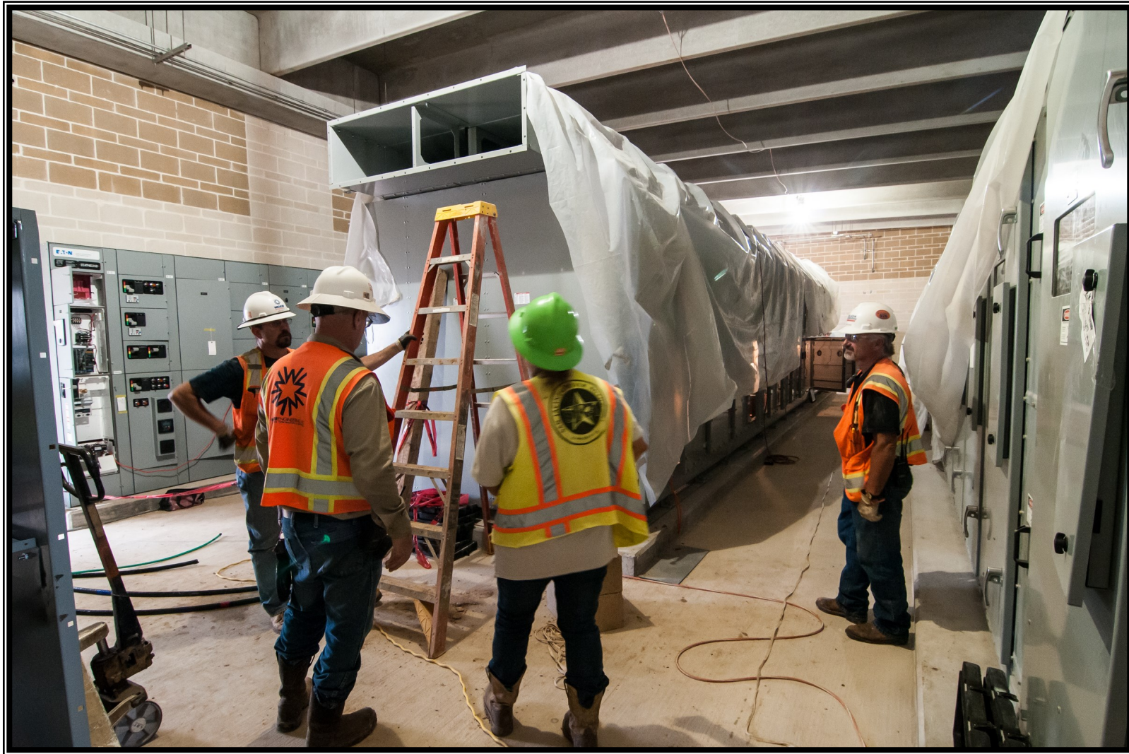
10 Main electrical switchgear installation at the Electrical Facilities
