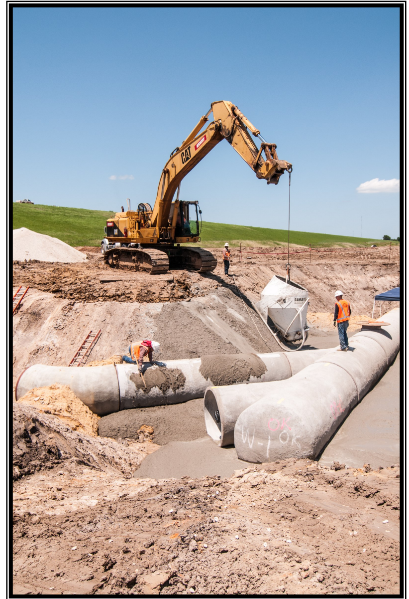
Raw Water Intake Pump Station plant piping at Surface Water Facilities
