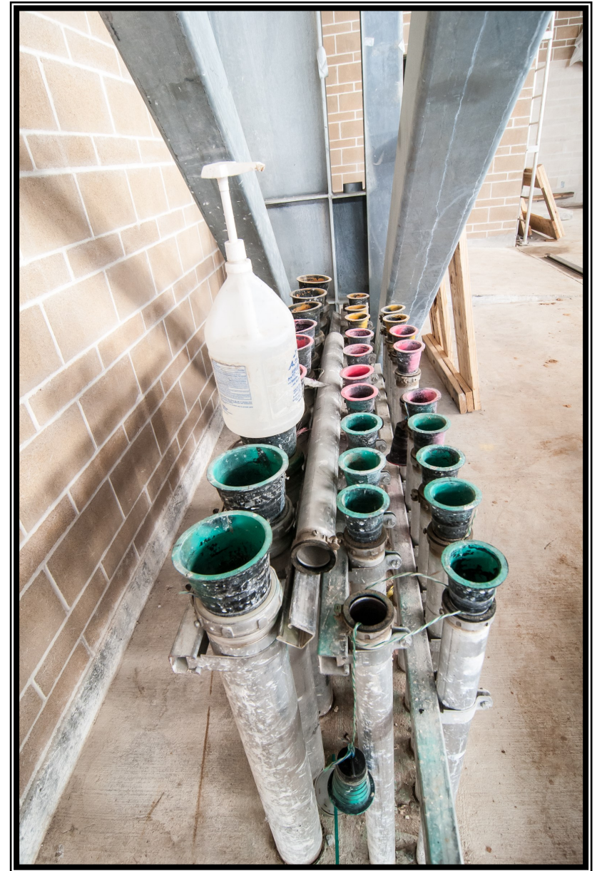
Conduit at the Raw Water Intake Pump Station at Surface Water Facility
