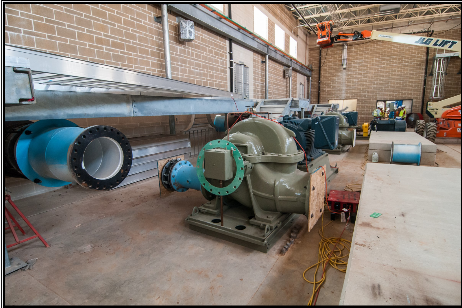
⑤ Pump installation at the High Service Pump Station
