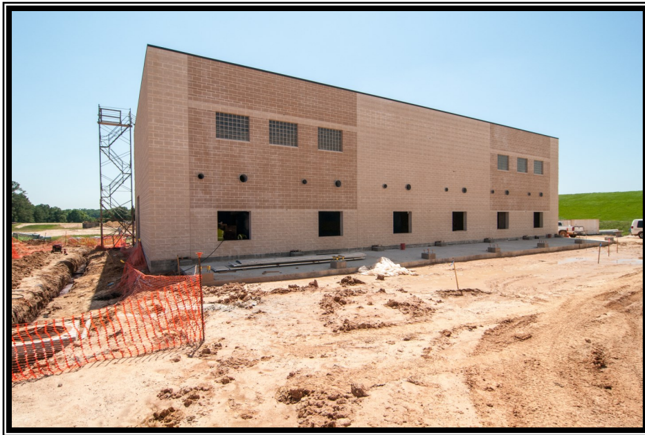
Above: View of Blower Building at Surface Water Facility
