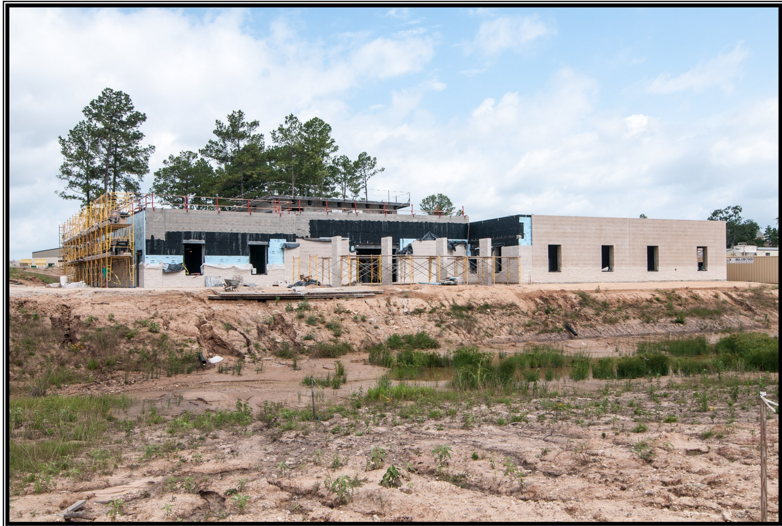
⑨ Completion of structural systems at the Operations Building
