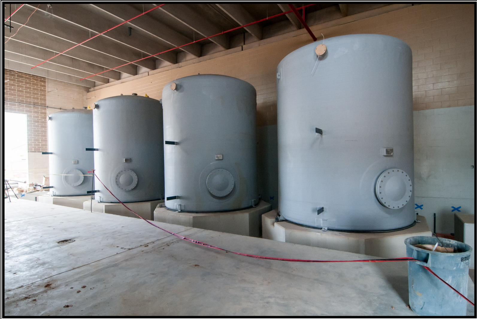
④ Installation of sodium hypochlorite tanks at the Chemical Storage Facilities
