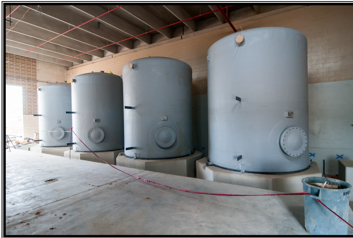
Chemical tanks at Chemical Storage Building at Surface Water Facilities
