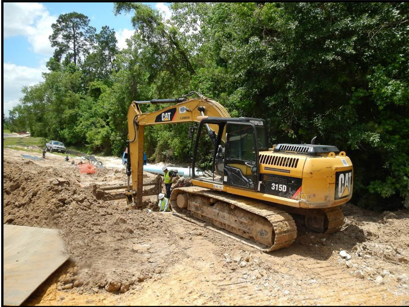
① Segment W4 - 24-inch pipe and fiber optic conduit installation on Gosling Road
