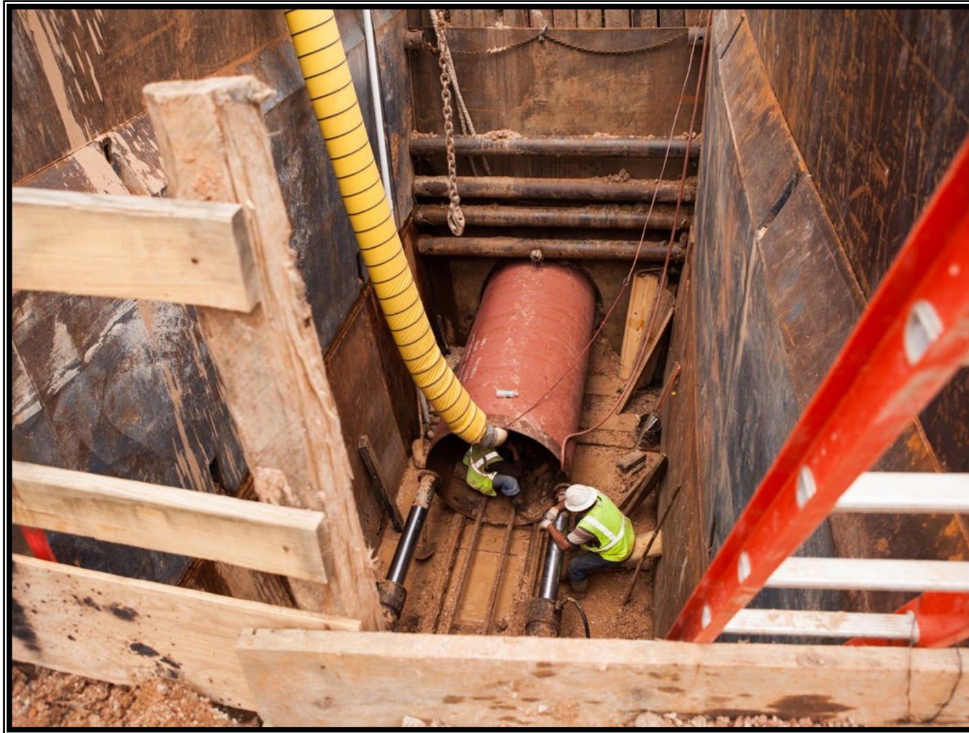
① Segment C2— 48-inch Steel Casing installation along Entergy easement
