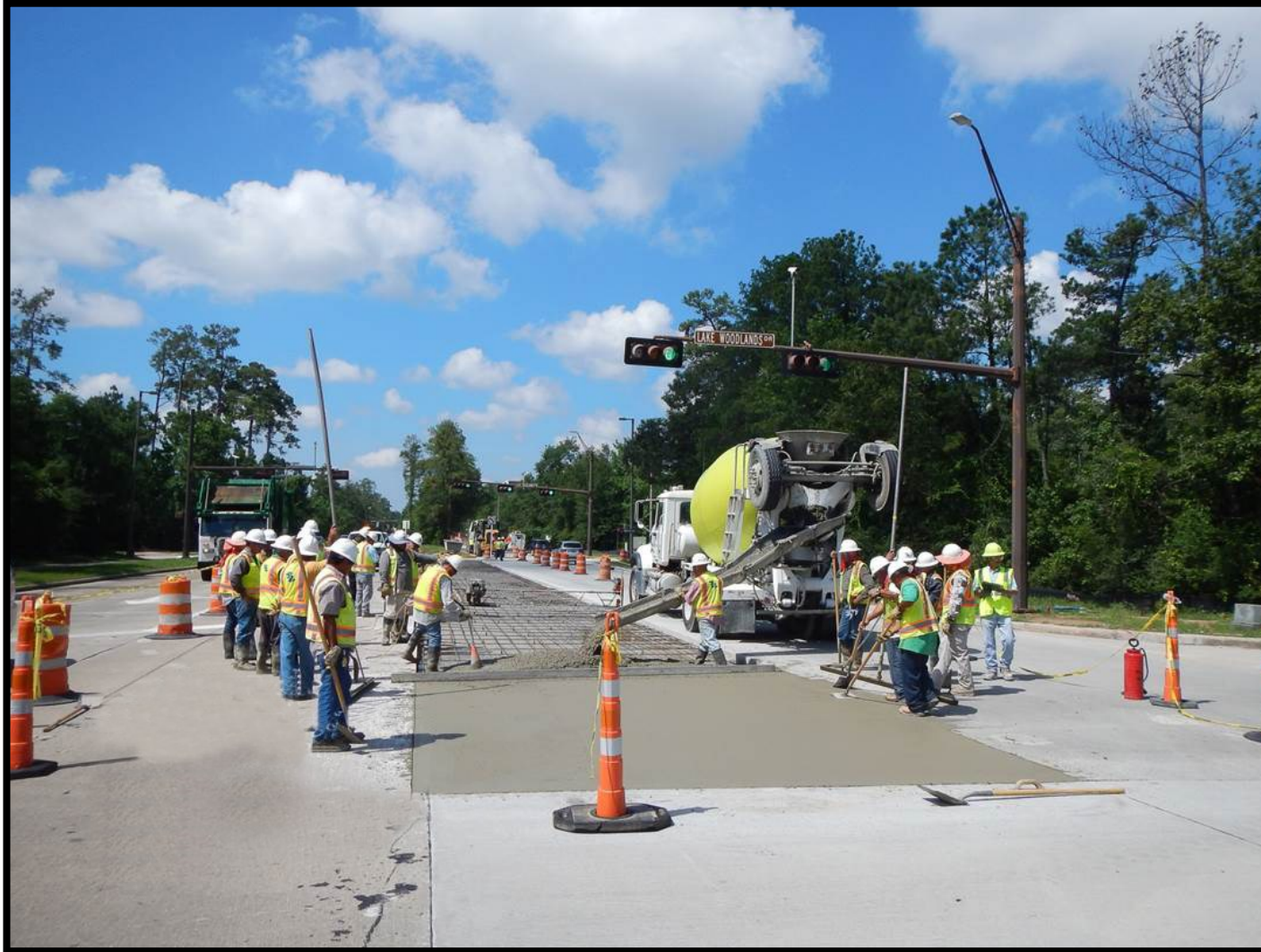
① Segment W2B - Concrete placement along Grogans Mill Road
