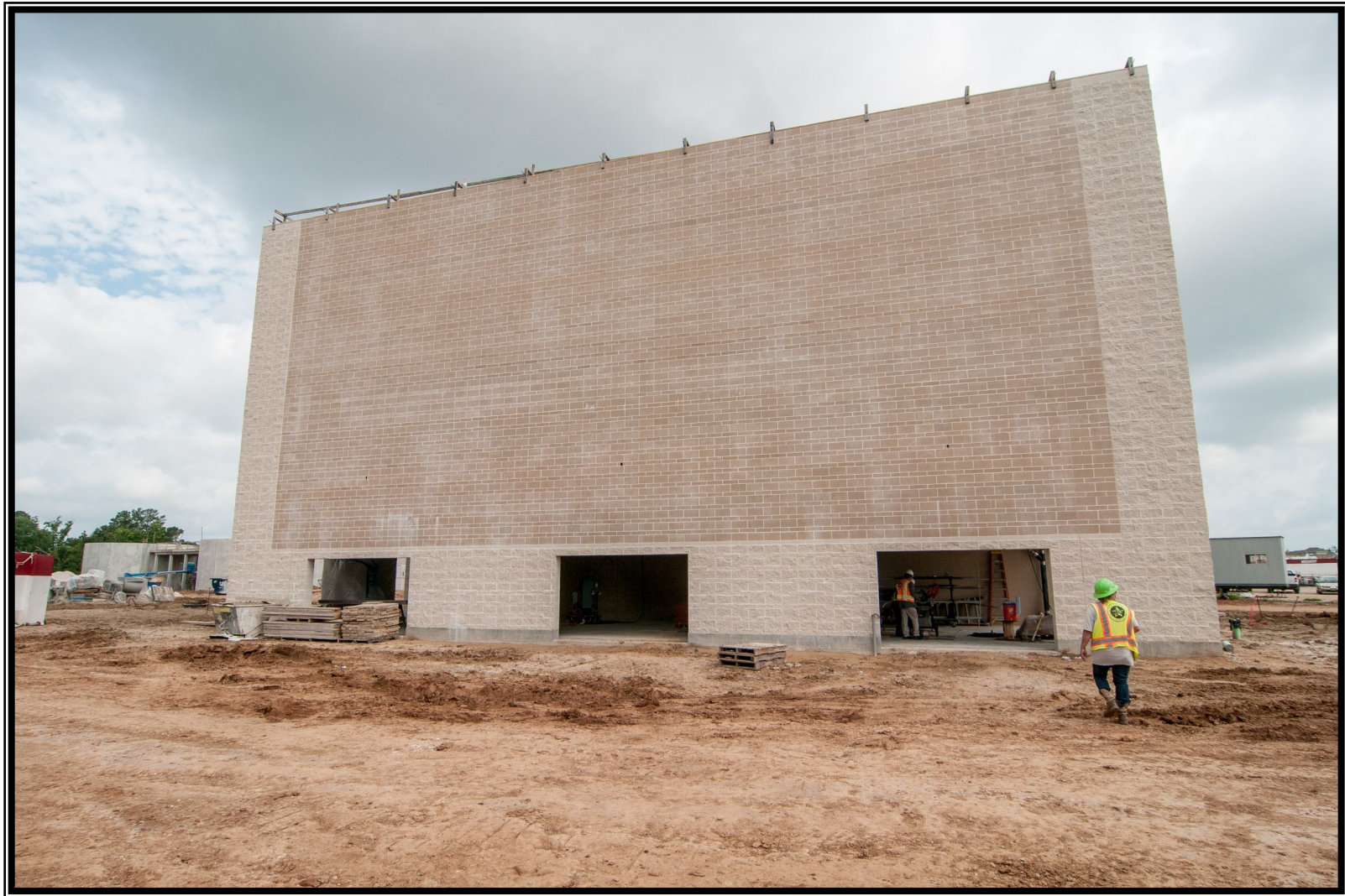
① Masonry installation at the Dewatering Building
