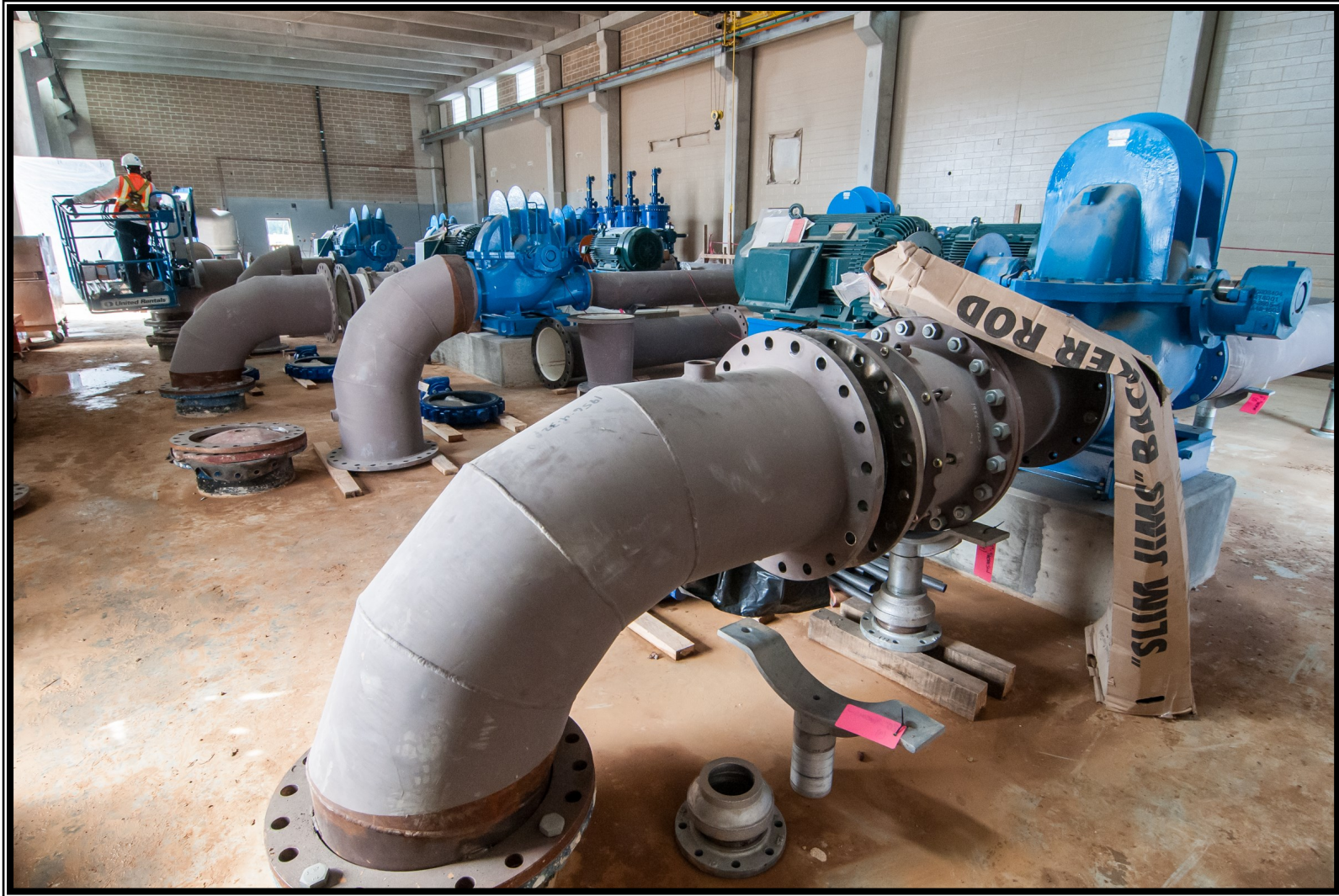
② Installation of membrane feed pumps at Membrane Building
