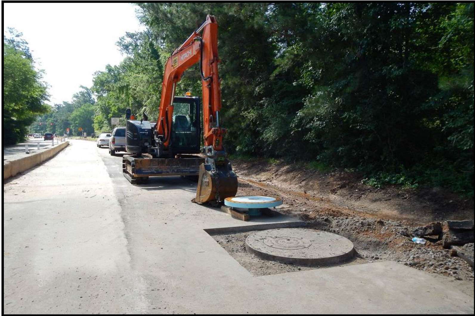
① Segment W1B - Manhole installation along Research Forest Drive
