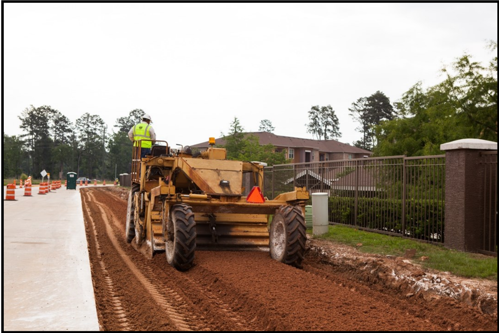
① Segment W1A—Pavement subgrade stabilization along Research Forest Drive
