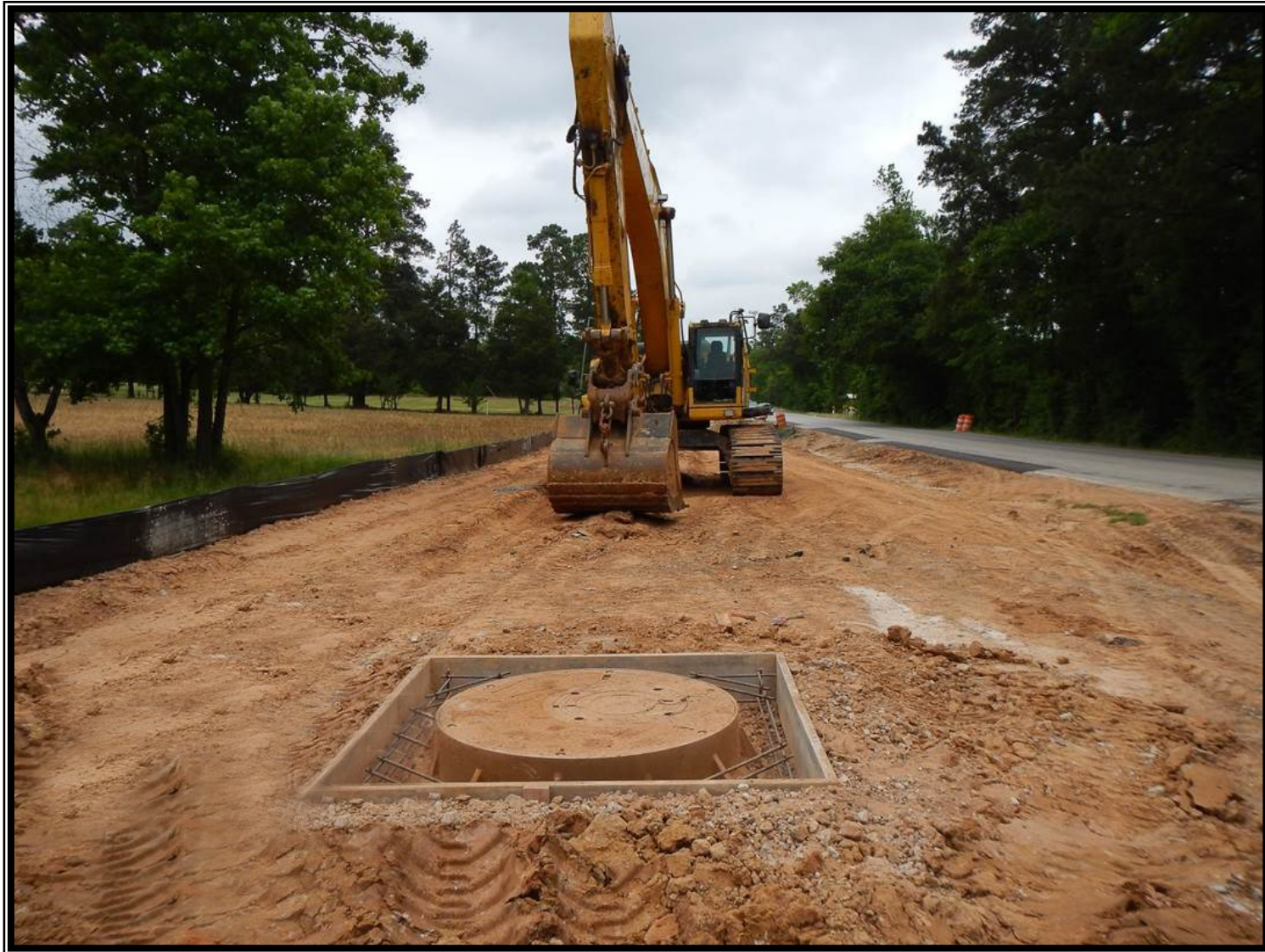
① Segment T1 - Manhole installation along McCaleb Road
