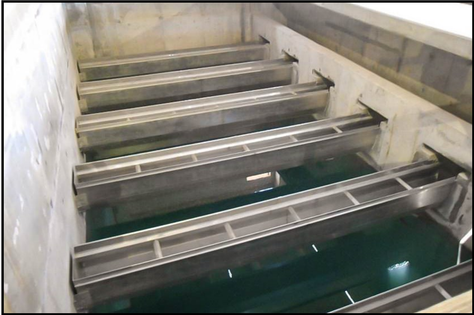
④ Leak testing contact basins in the GAC Building
