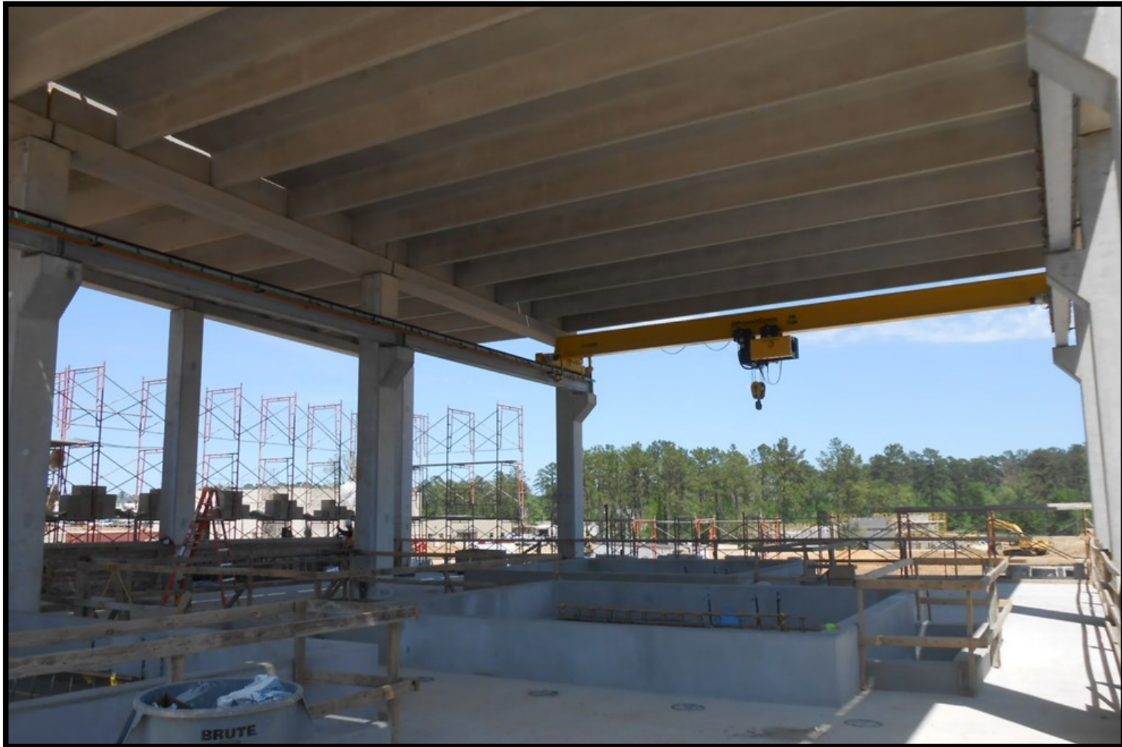
① Second floor masonry installation in the Dewatering Building
