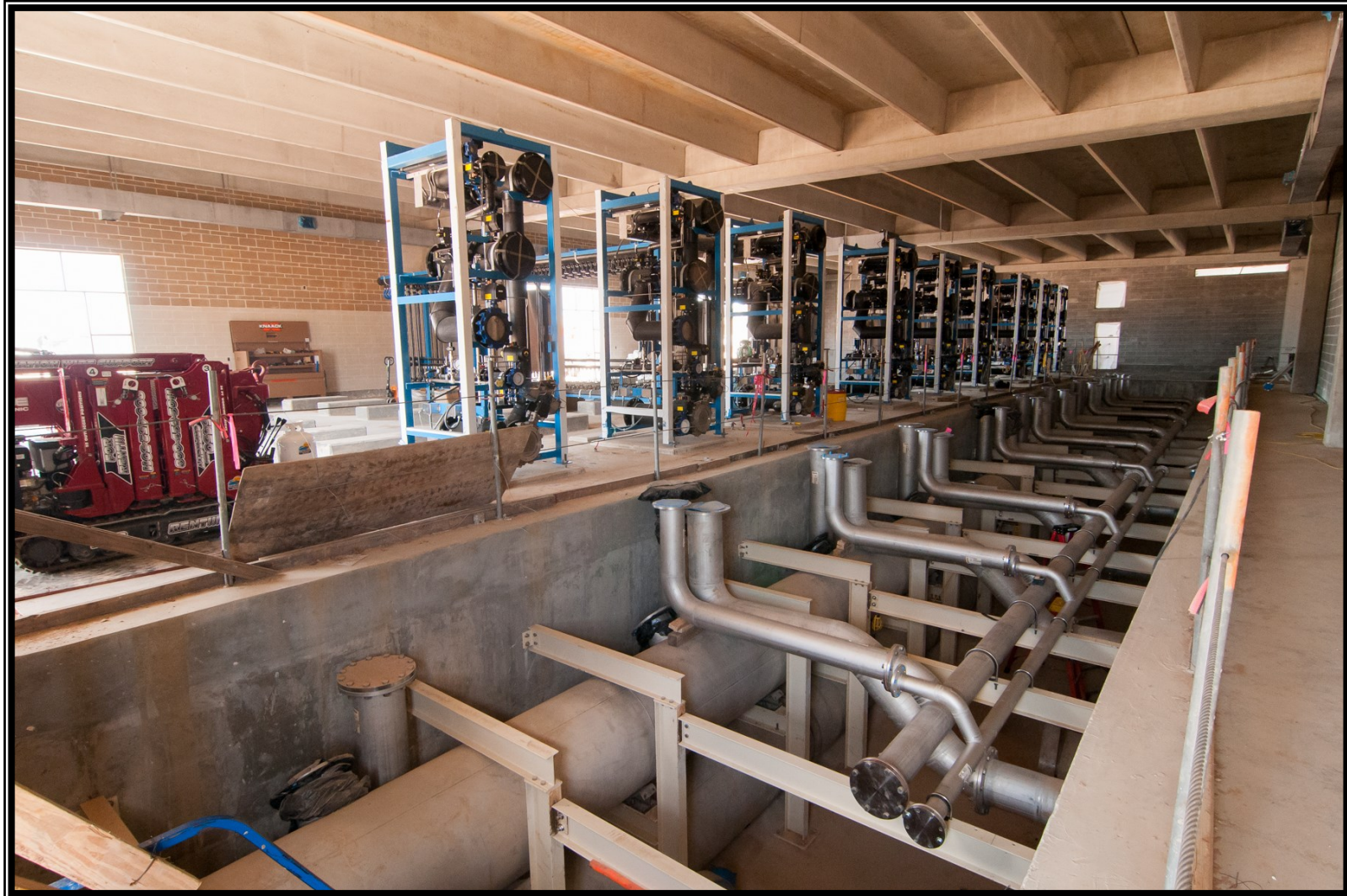
3 Installation of membrane equipment racks and piping in the Membrane Building
