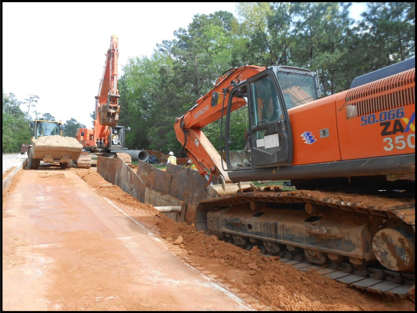
❶ Segment W2A - 42-inch pipe installation along Research Forest Drive
