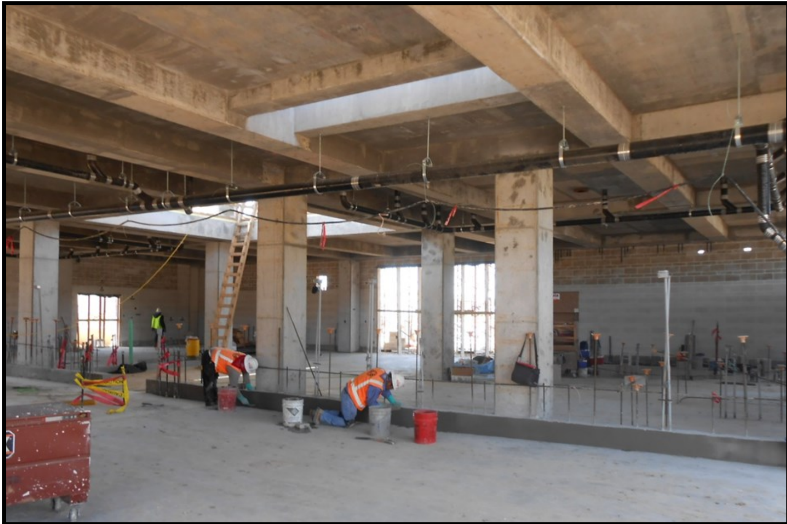
① First floor mechanical installation in the Dewatering Building
