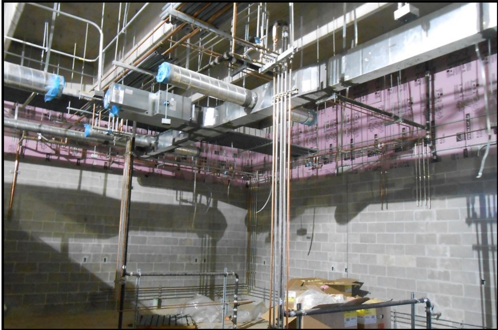
③ Mechanical and plumbing rough-in at the Membrane Building
