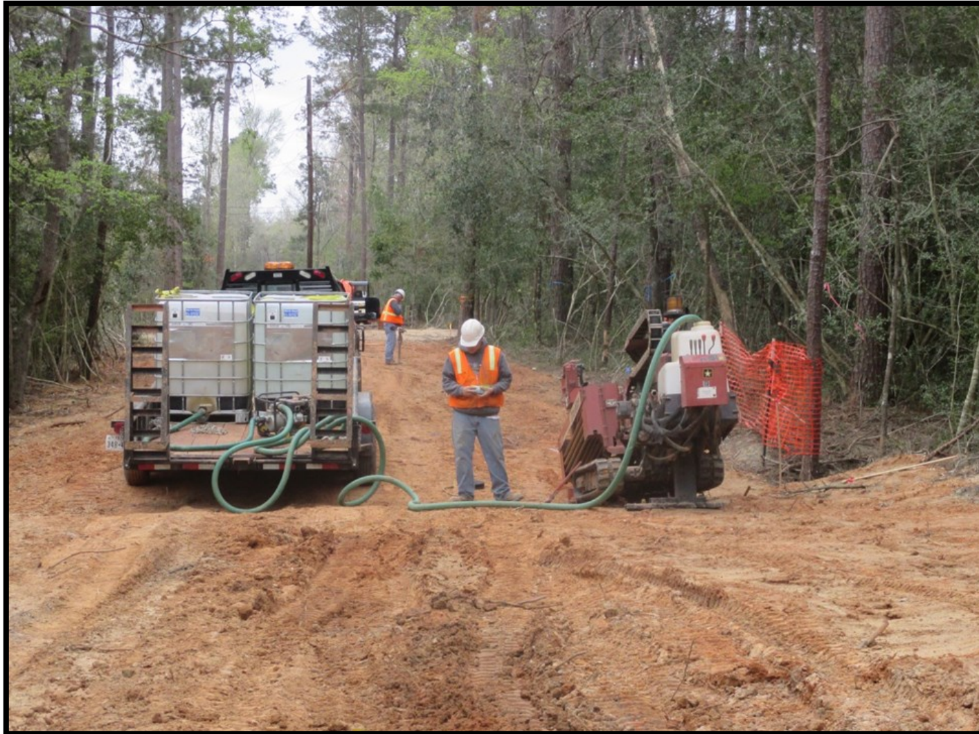
① Segment C1B - Horizontal directional drilling fiber optic conduit along Longmire Road
