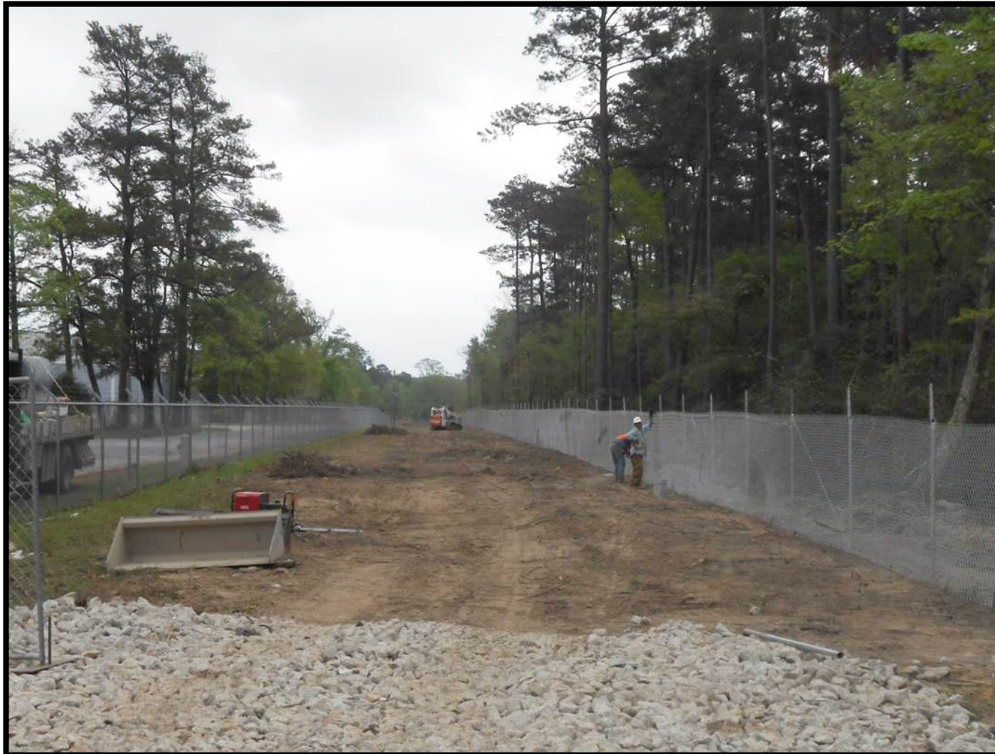
① Segment C3—Security fence installation along Silver Springs Road at Girl Scout property
