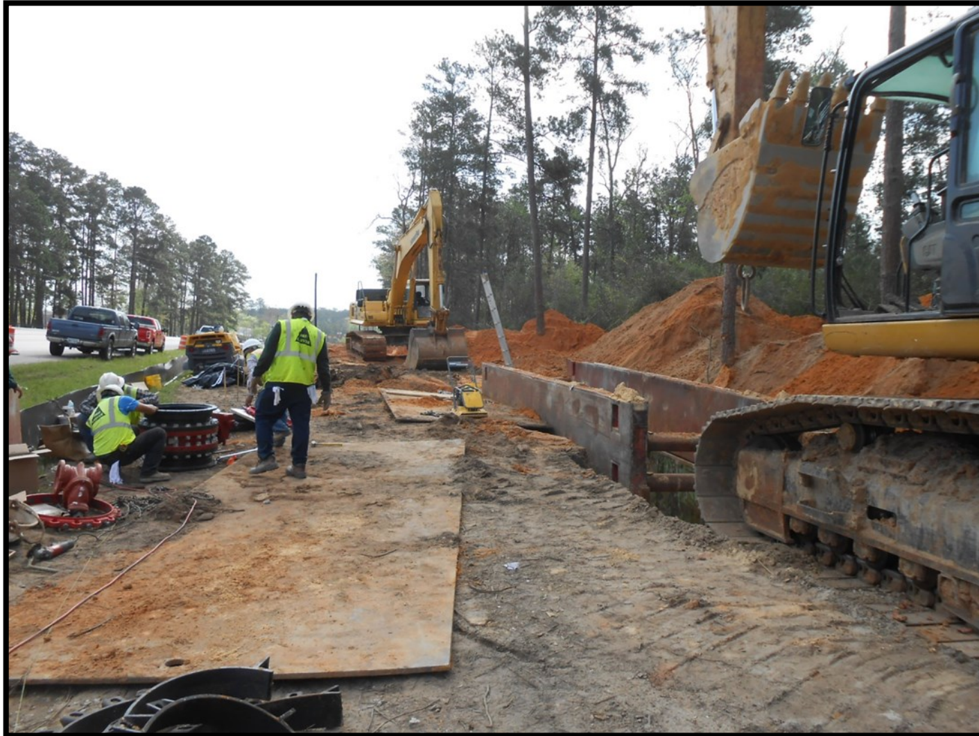
① Segment C4—24-inch pipe and restrained joint installation along FM 830
