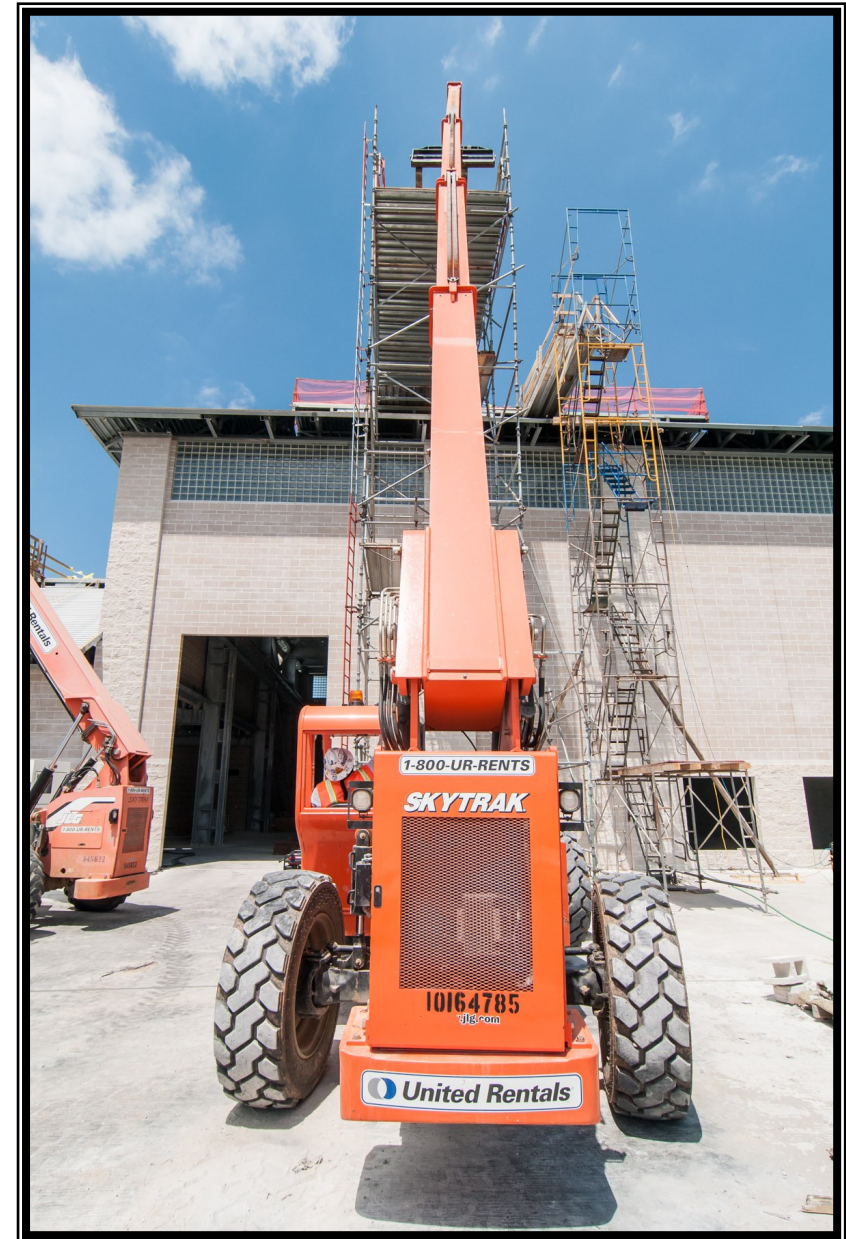
Installation of Roofing at Raw Water Intake at Surface Water Facility
