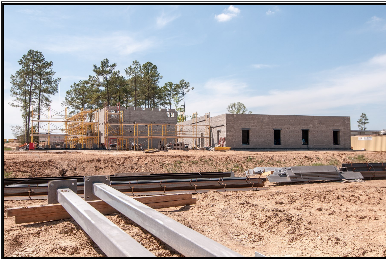
9 Outside view of Operations Building
