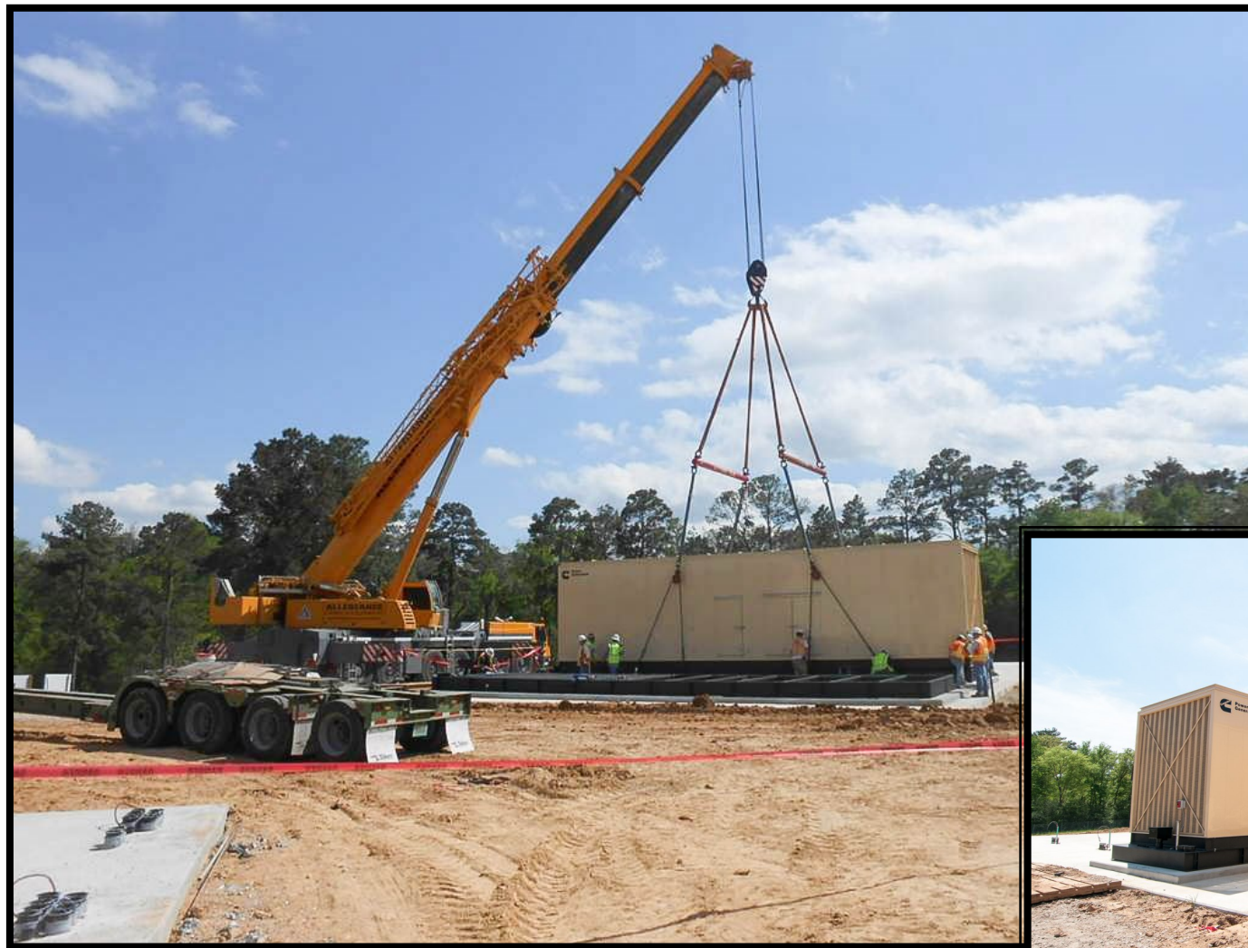
10 Backup Generator installation in progress at Electrical Facilities
