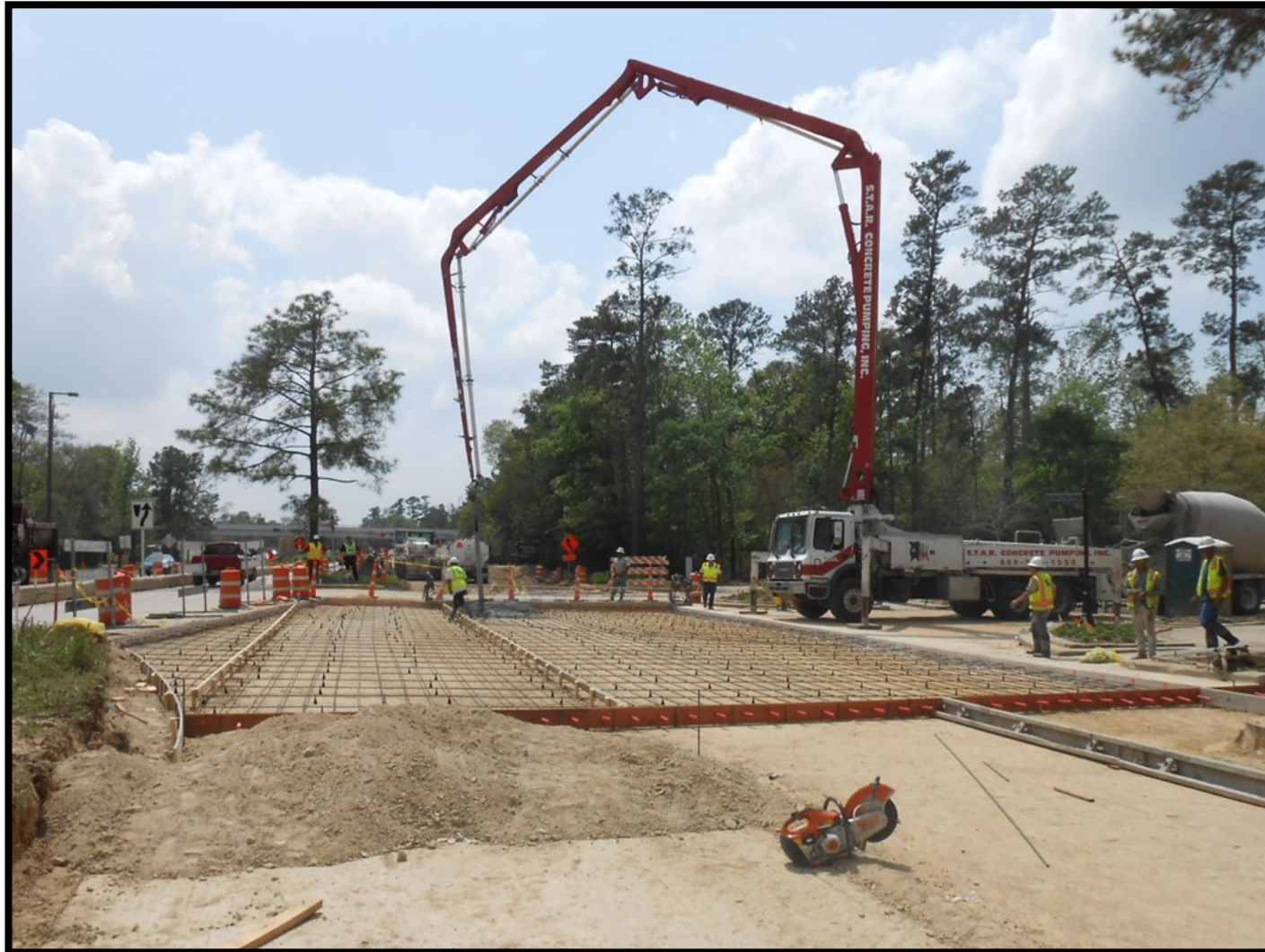
① Segment W2B - Concrete pavement installation at Grogans Mill Road and East Shore Drive
