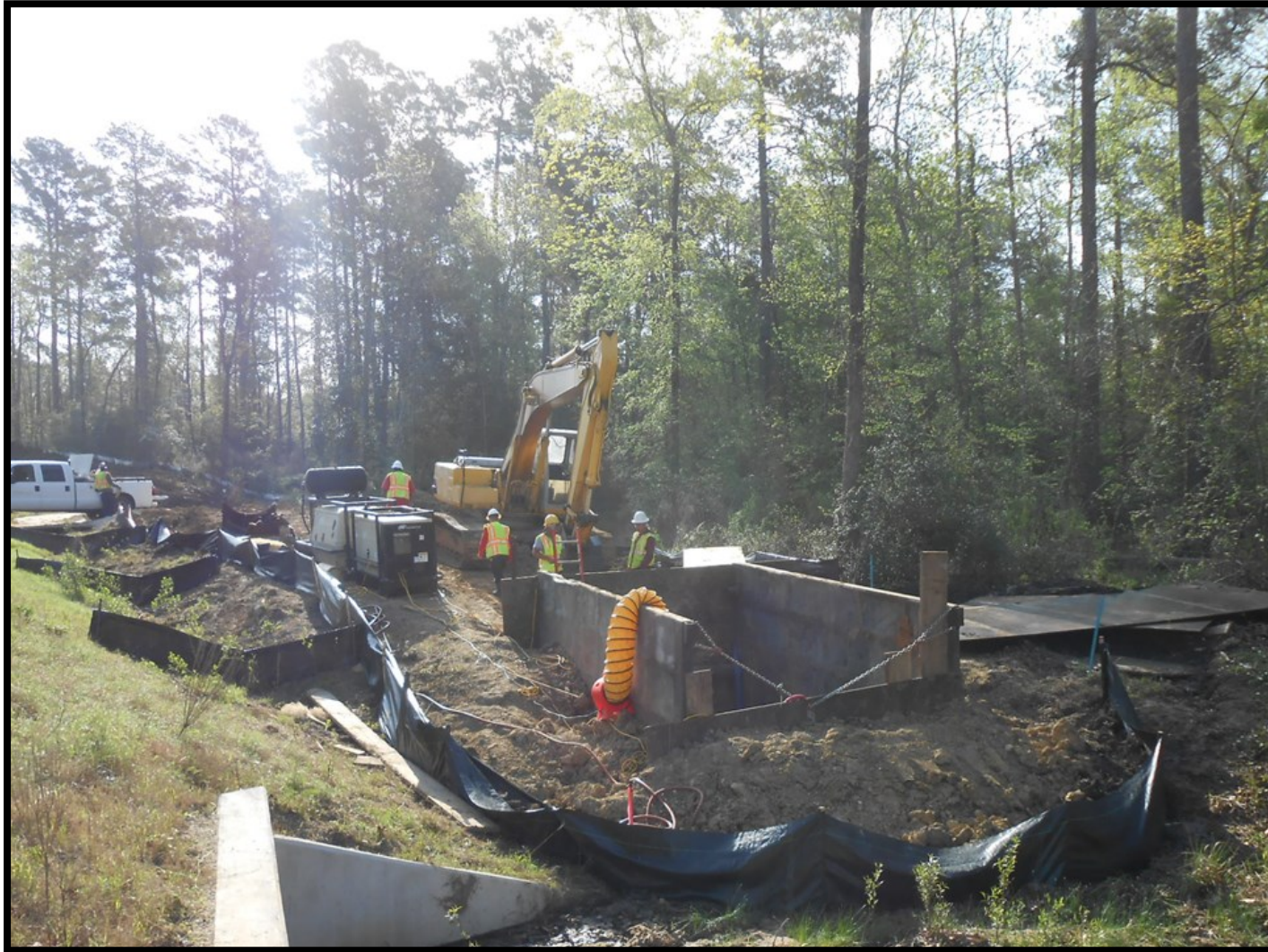
① Segment C1A - Tunnel installation at creek along GRP Access Road
