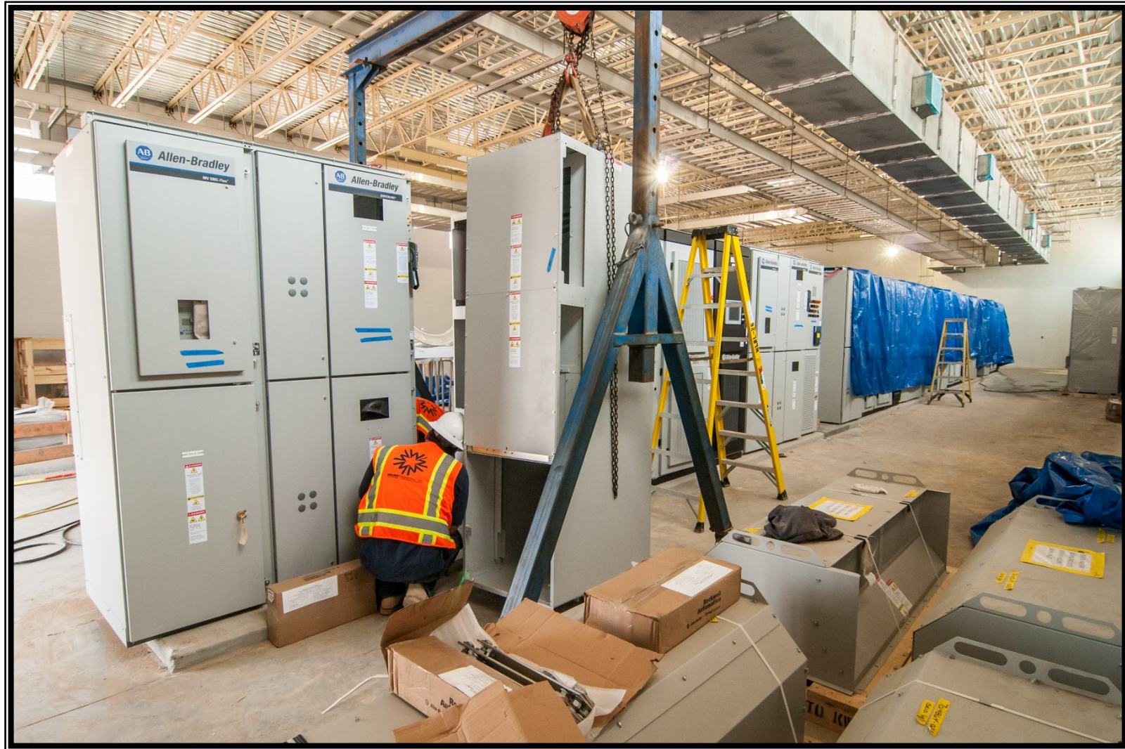
5 Installation of electrical room equipment at High Service Pump Station
