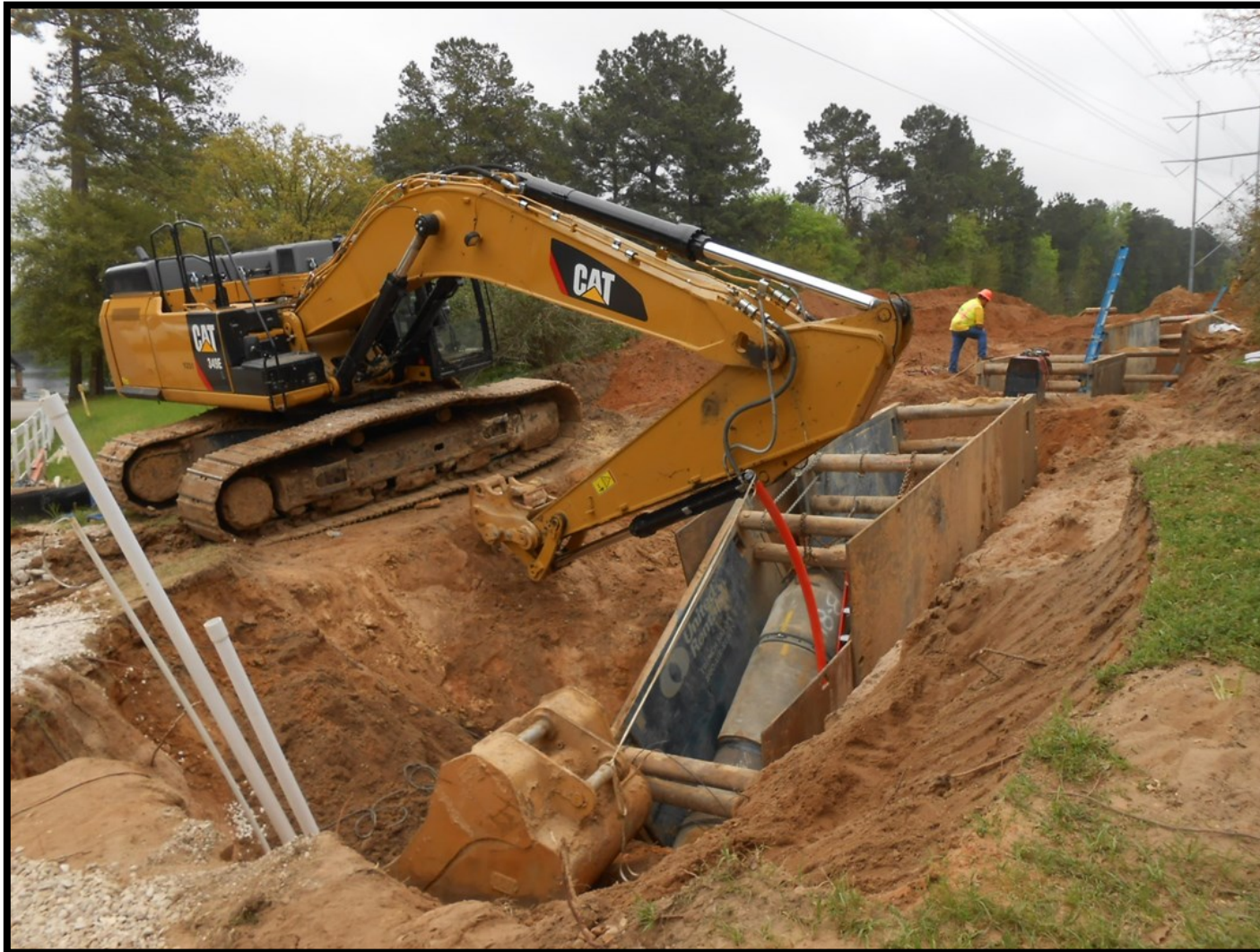
❶ Segment C2—Pipe installation along Entergy easement and Wayne Bennett Court
