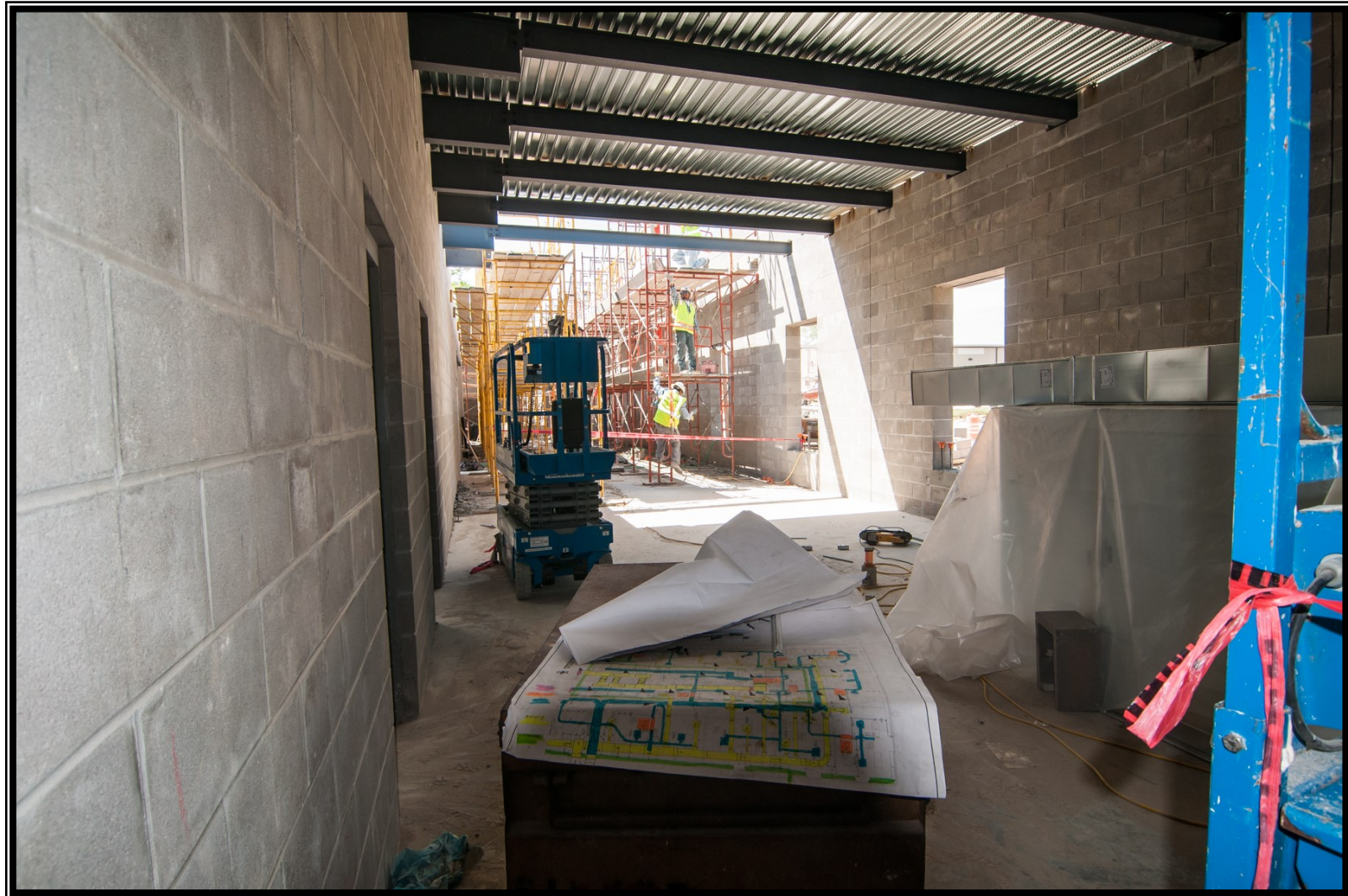
⑨ Masonry and structural steel installations at the Operations Building
