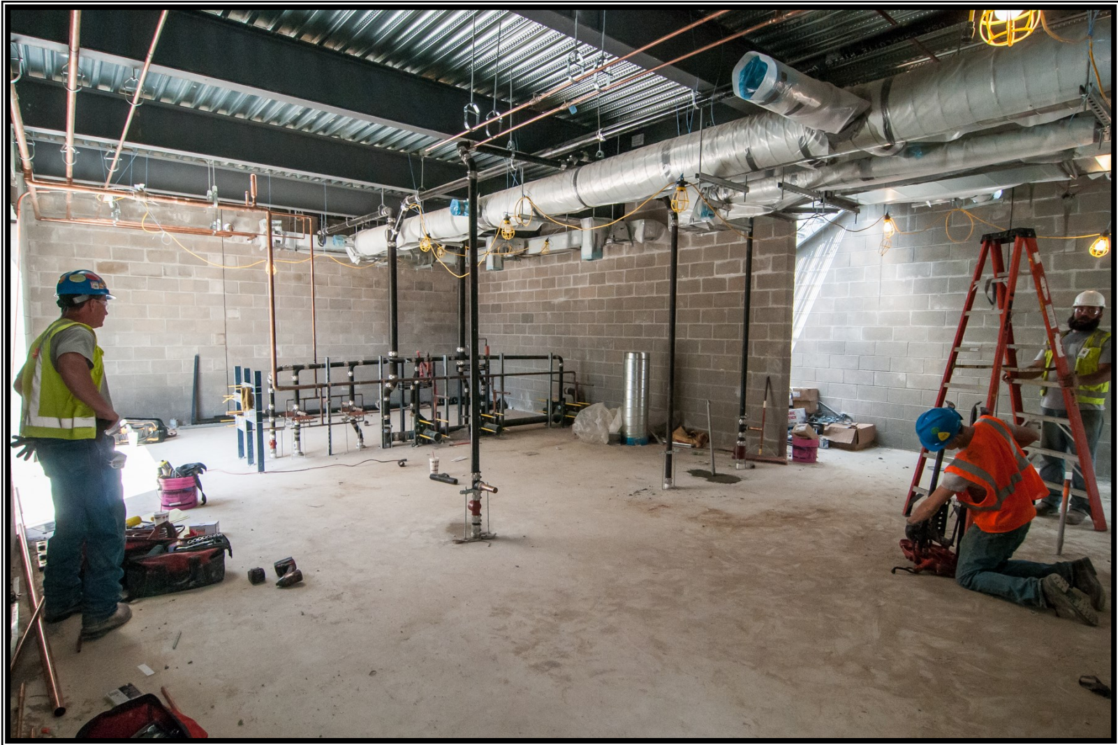
9 Mechanical and plumbing rough-in at the Operations Building
