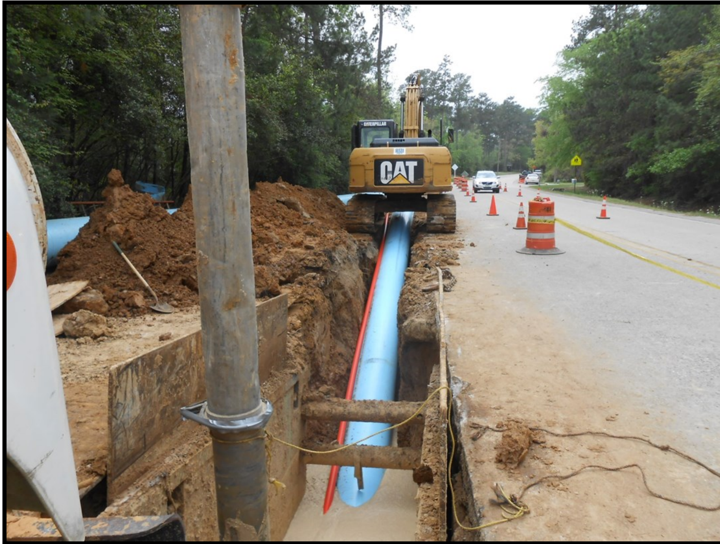
① Segment W4 - 24-inch pipe and fiber optic conduit installation at Shadowbend Place
