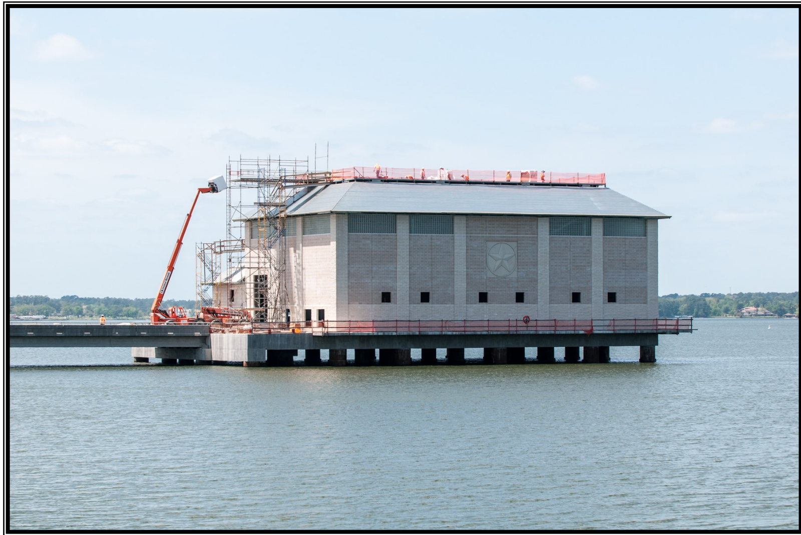
❶ Roof deck installation at the Raw Water Intake and Pump Station
