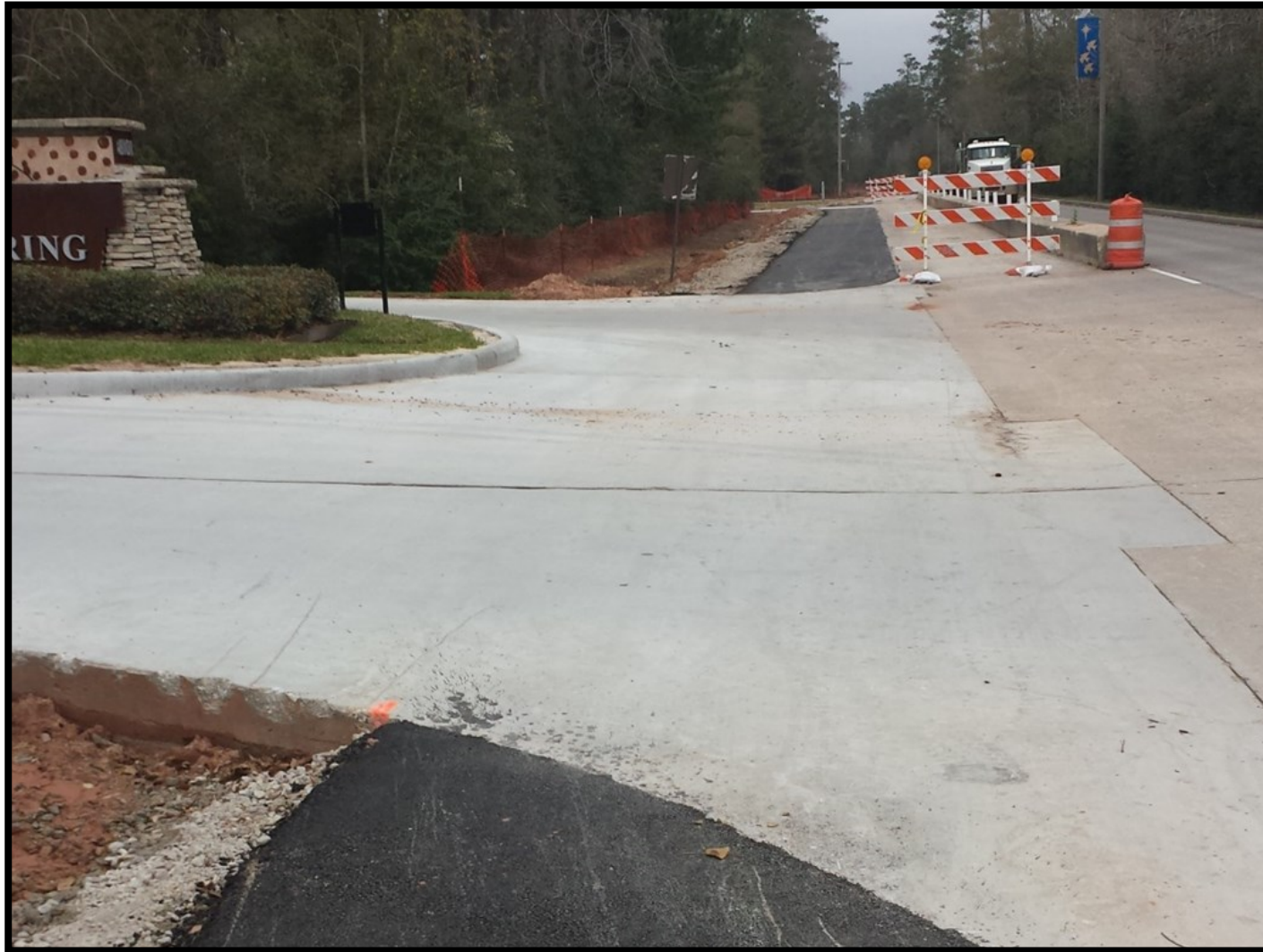
① Segment W1B - Asphalt shoulder repair along Research Forest Drive
