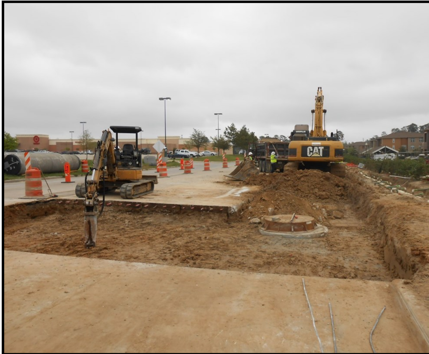
① Segment W1A—Concrete repairs along Research Forest Drive
