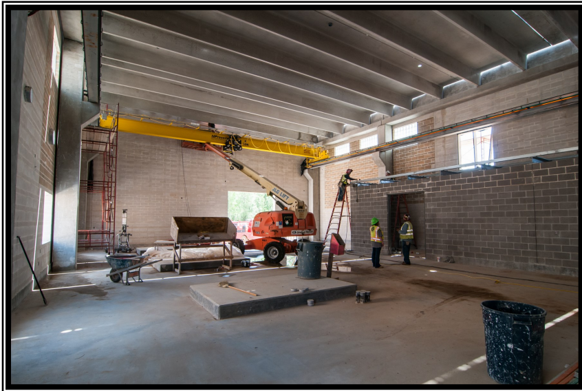
⑥ Masonry installation at Blower Building
