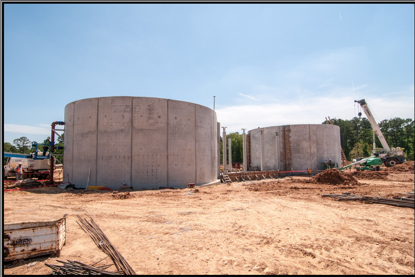
⑧ Concrete column installation at the Sludge Thickeners
