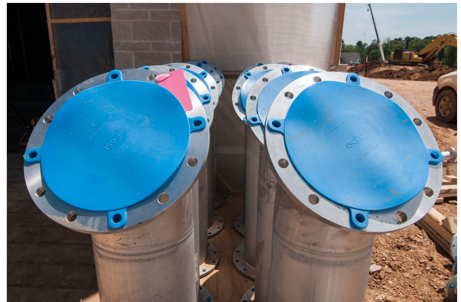
Pipes for Membrane Building at Surface Water Facility
