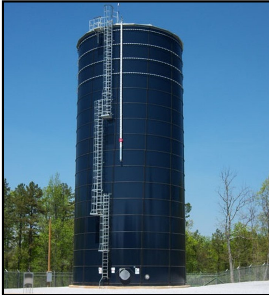
① Example Standpipe—SJRA Standpipe currently under fabrication
