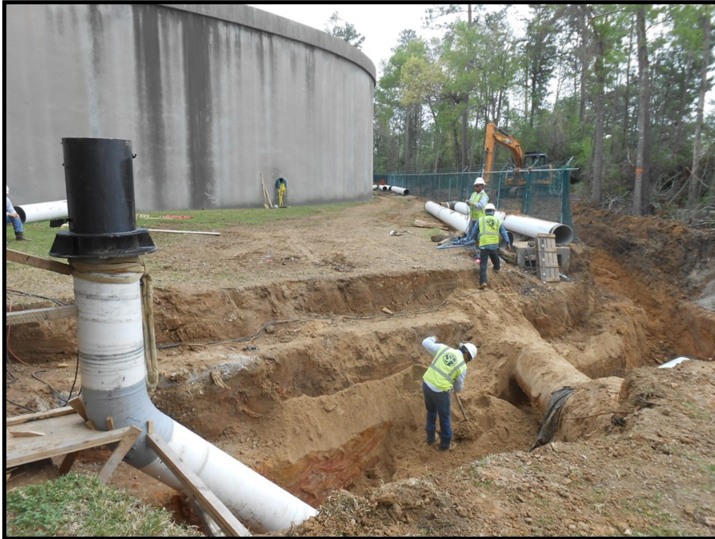
① Water Receiving Facilities—South—20-inch ground storage tank connection at SJRA Water Plant No. 2
