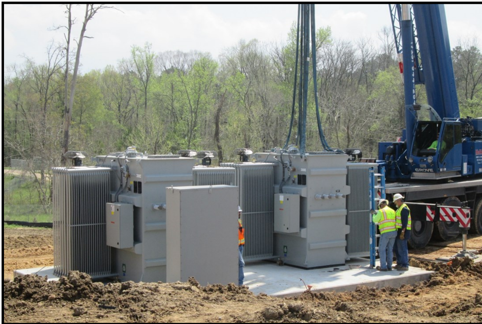
⑩ Main transformer installation in progress at Electrical Facilities
