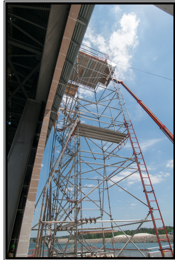
View from below of roofing installation at Raw Water
