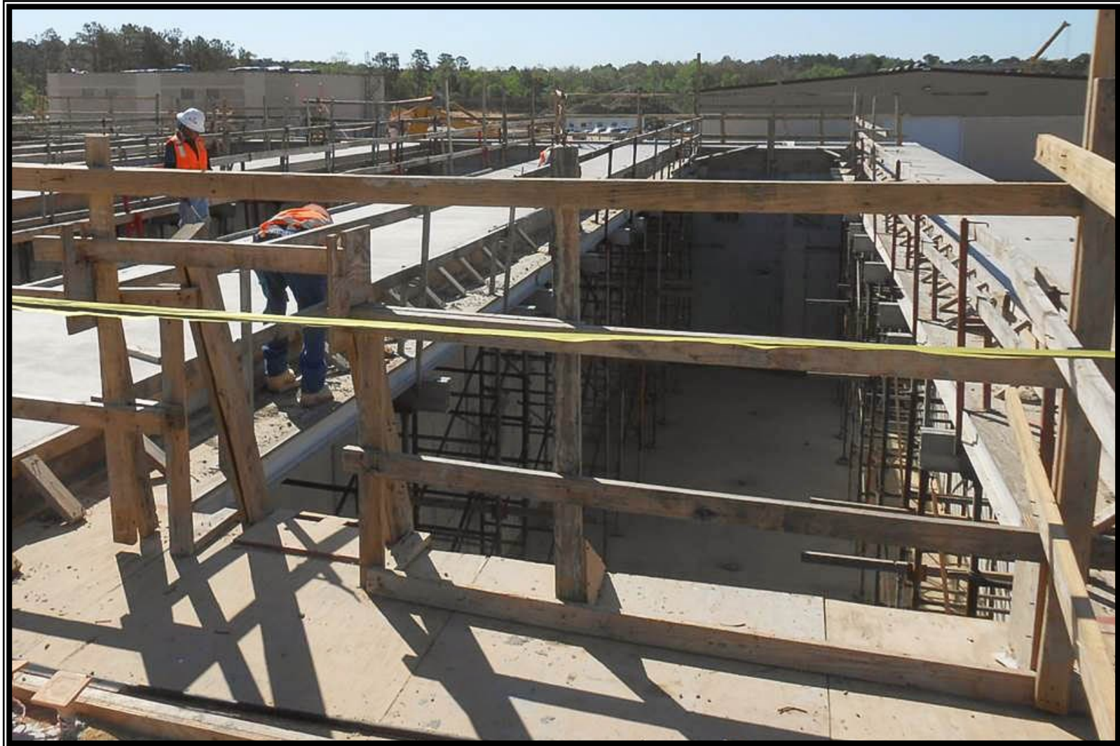
② Access walkway installation at the Pretreatment Facility
