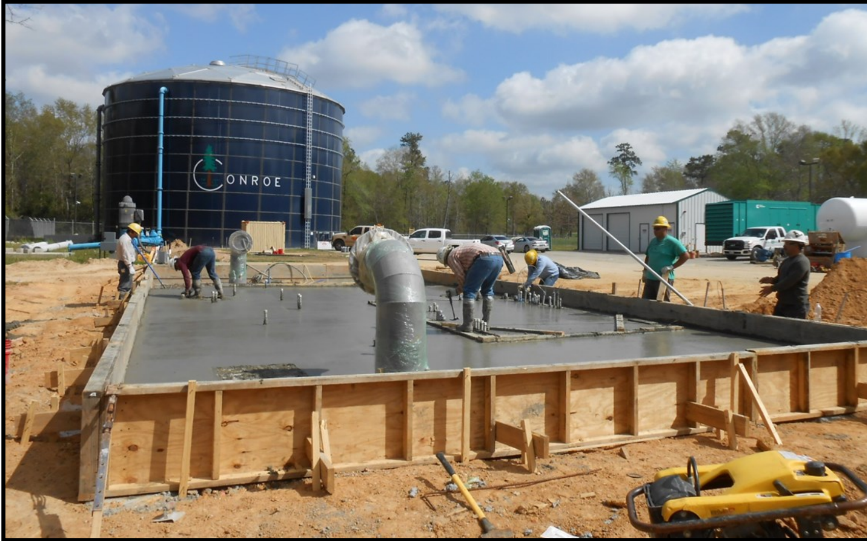
① Water Receiving Facilities—North— Flow and pressure control station slab installation at City of Conroe Water Plant No. 22
