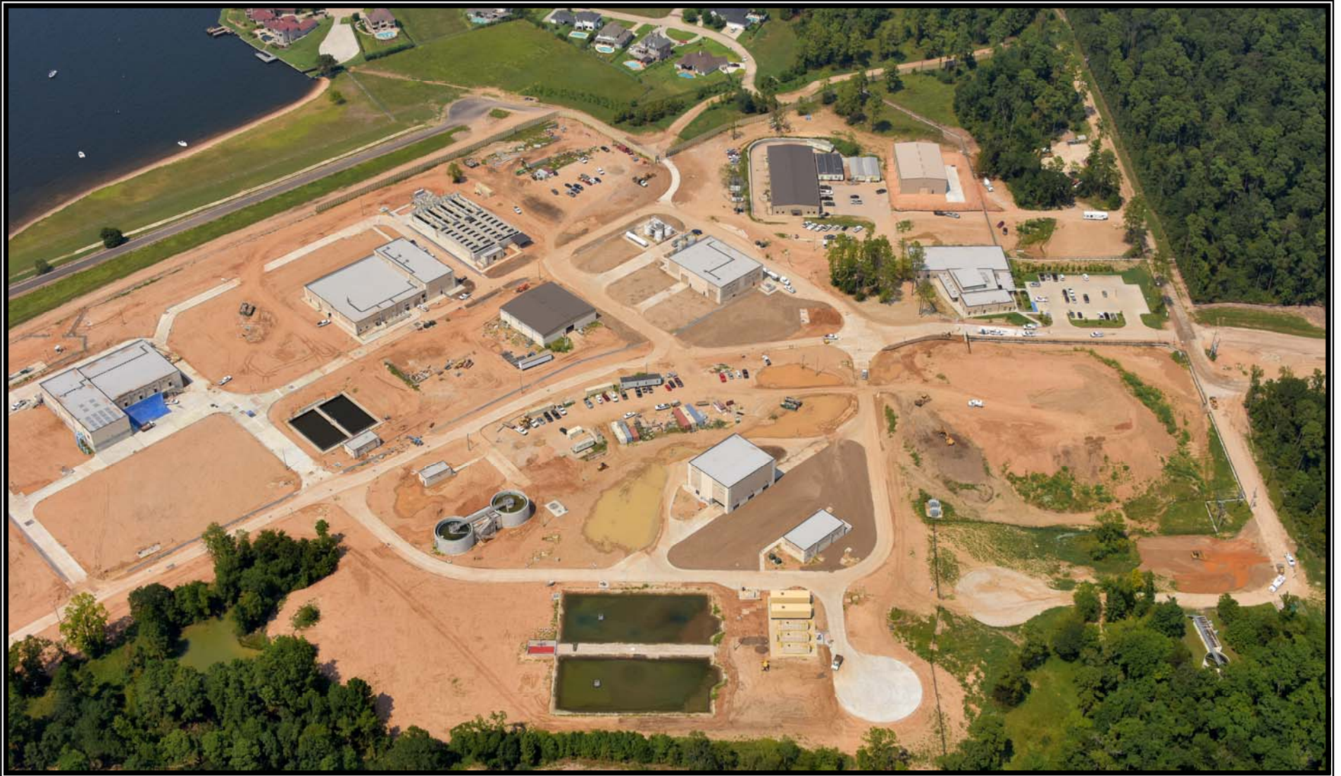
General Site - Aerial reflecting overview of site clean up at the Surface Water Treatment Facility
