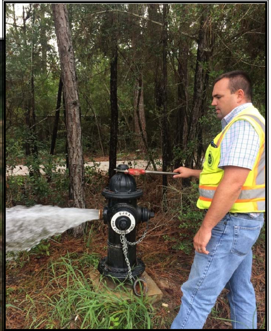
SJRA Staff — Flushing surface water transmission lines
