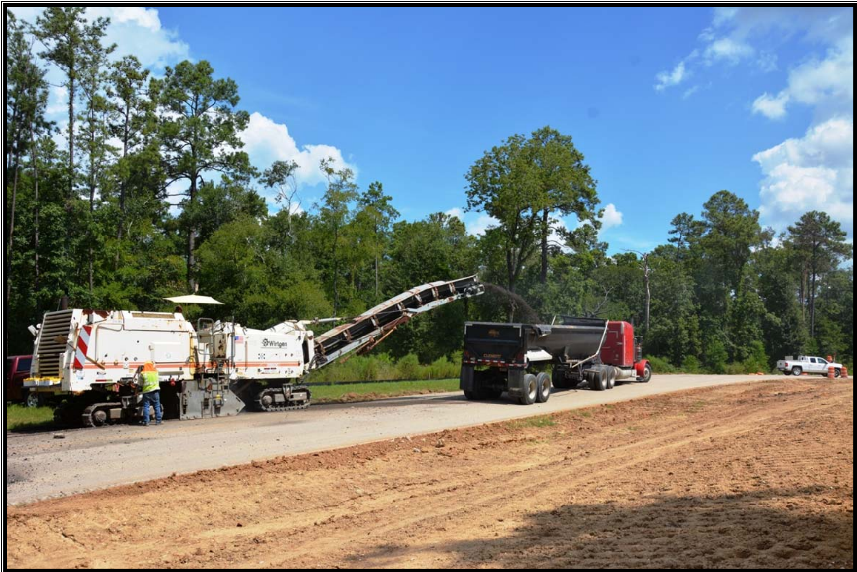
① Access Road—Milling of gravel for permanent access road
