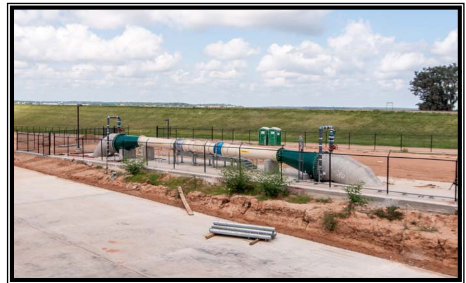
Clean up and installation of fencing around the Flow Meter Station
