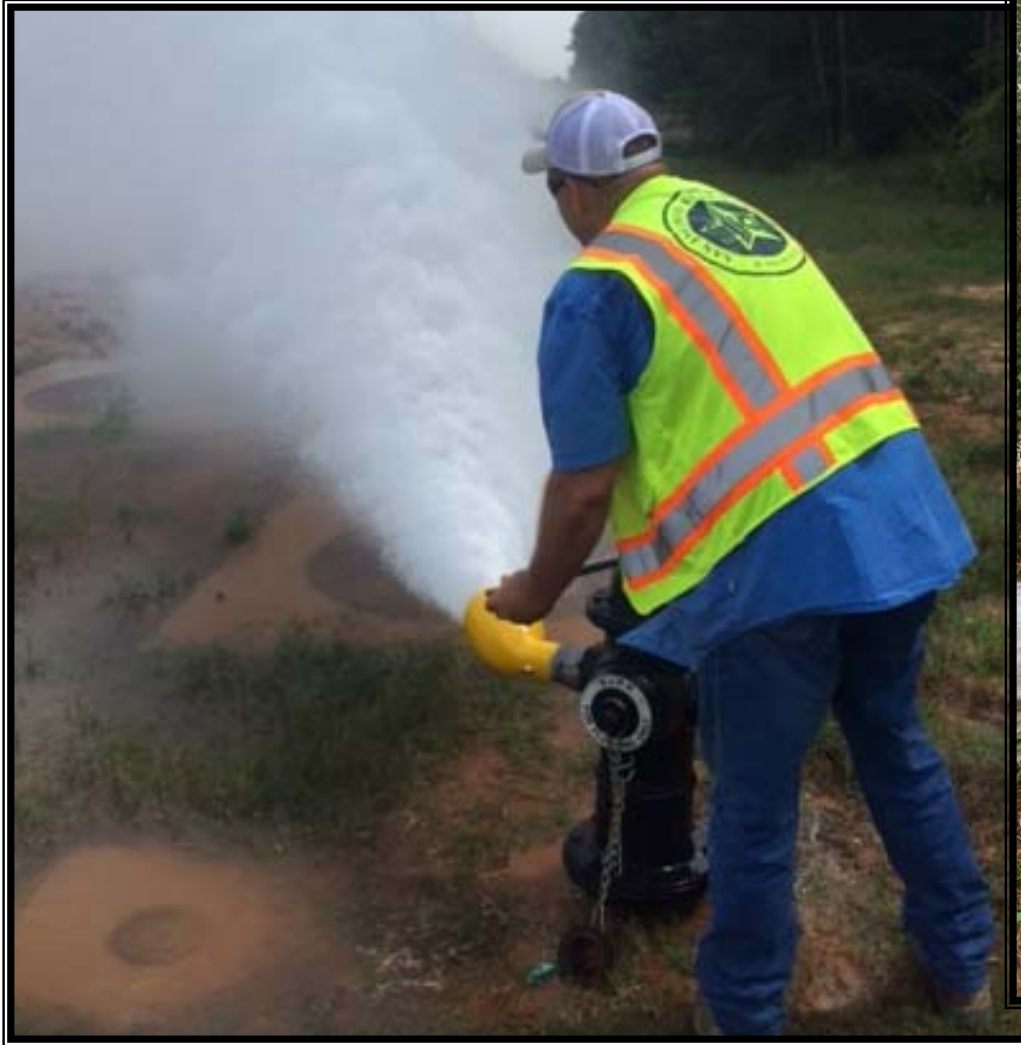
SJRA Staff — Flushing surface water transmission lines
