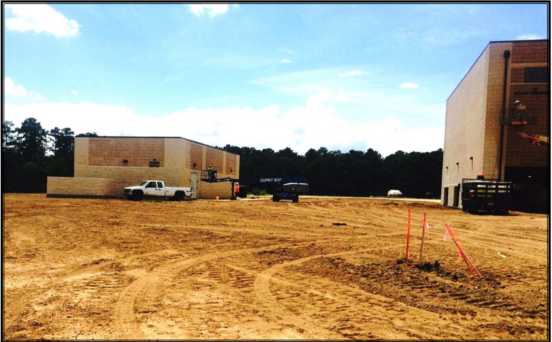
General Site—Site clean up, power washing, and sealing of exterior masonry
