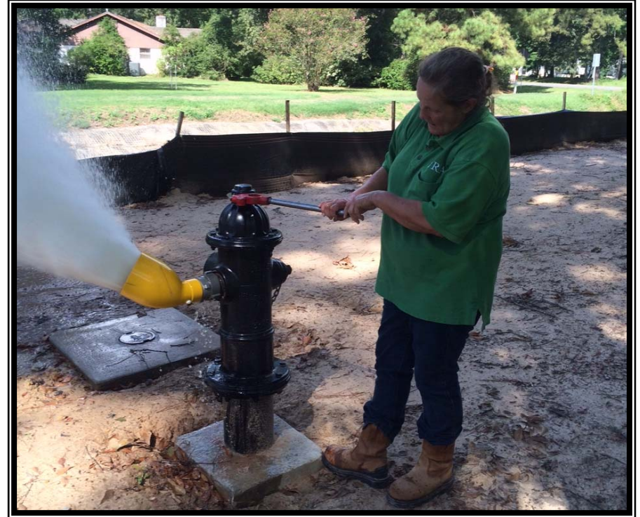
SJRA staff flushing surface water transmission lines
