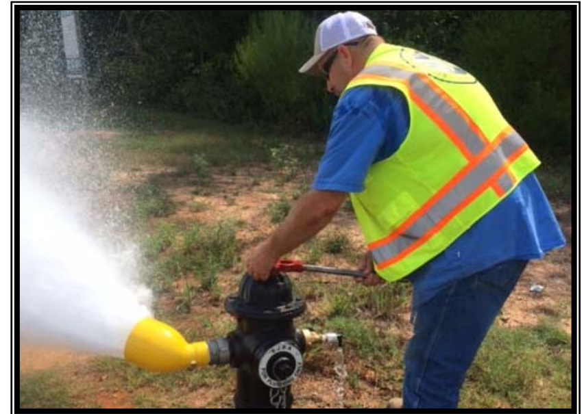
GRP staff flushing and taking samples along various surface water transmission line segments
