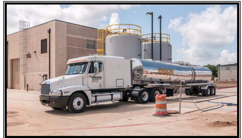
Coagulate delivery and storage at the Chemical Building
