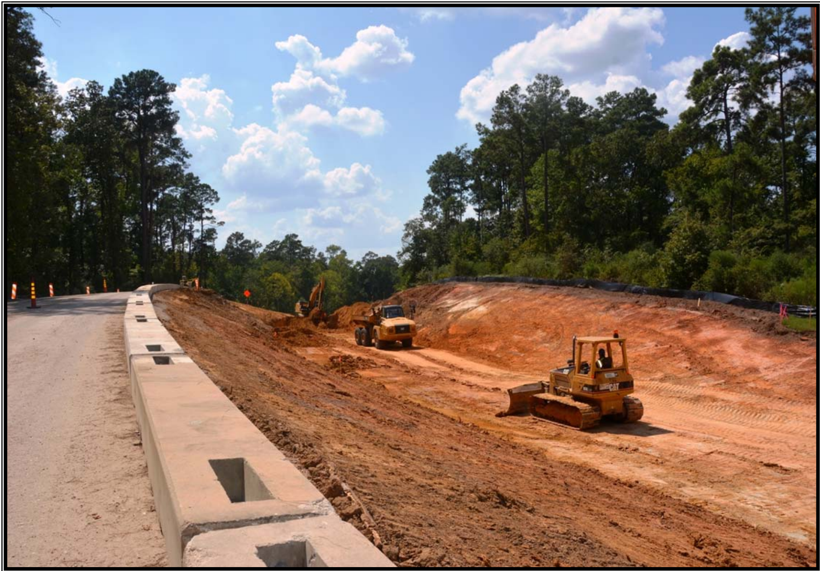
① Access Road—Excavation and grading to final subgrade
