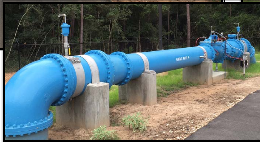
① Standpipe - Completed asphalt paving at site
