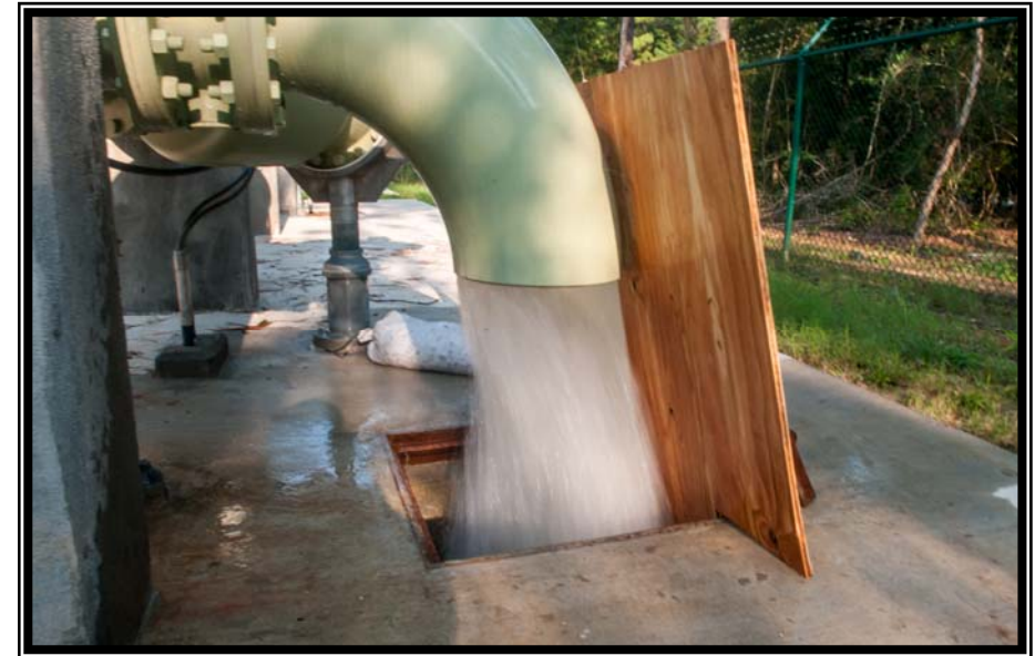
Left and Above—Flushing surface water transmission lines at the Woodlands Water Plant No. 2
