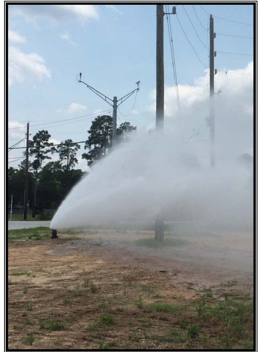
Flushing transmission line at the corner of Research Forest Drive and FM 2978
