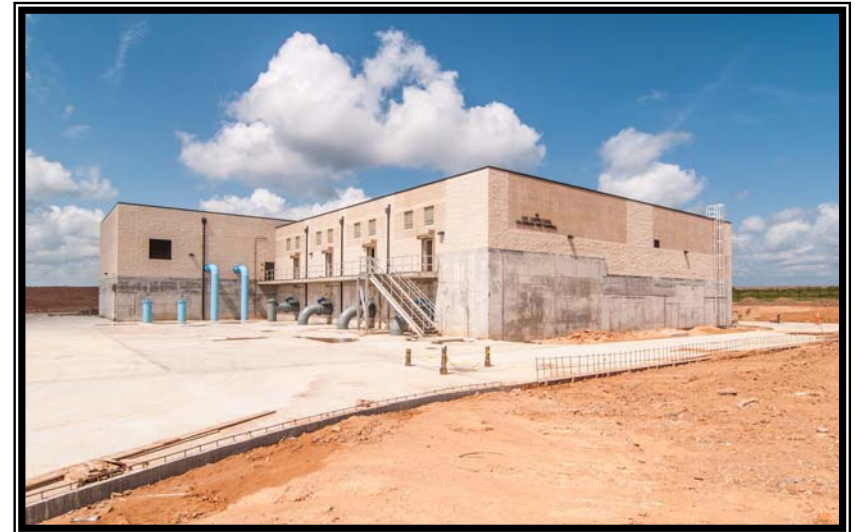
Above—Site grading and clean up at the Granular Activated Carbon (GAC) Building
