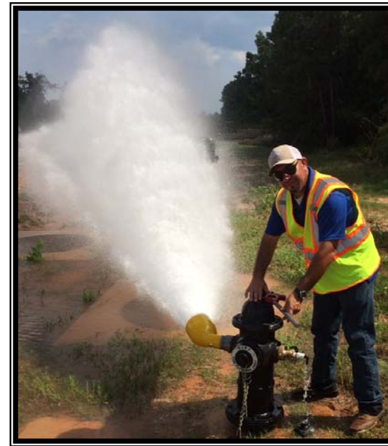
Above—SJRA staff flushing surface water transmission lines along Fish Creek Thoroughfare
