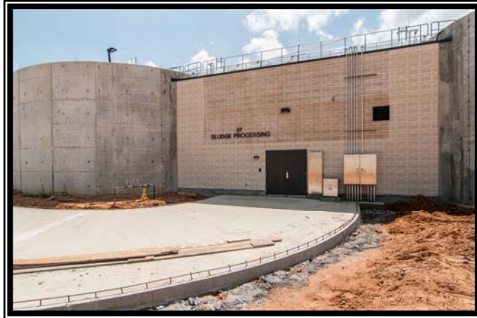
Concrete road to access the Sludge Processing Building
