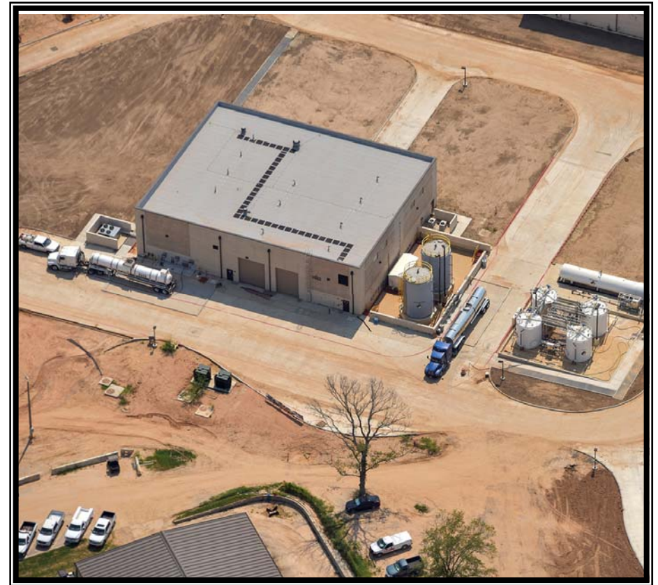
Aerial view of site grading and clean up at the Chemical Building
