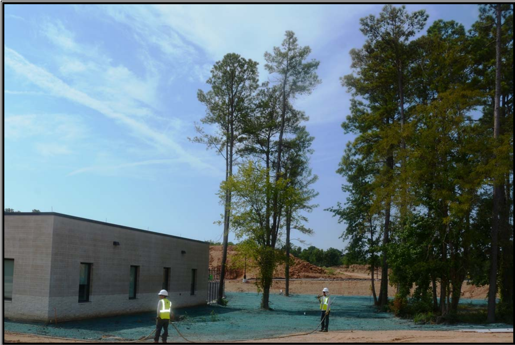
② Operations Building—Hydromulching and clean up
