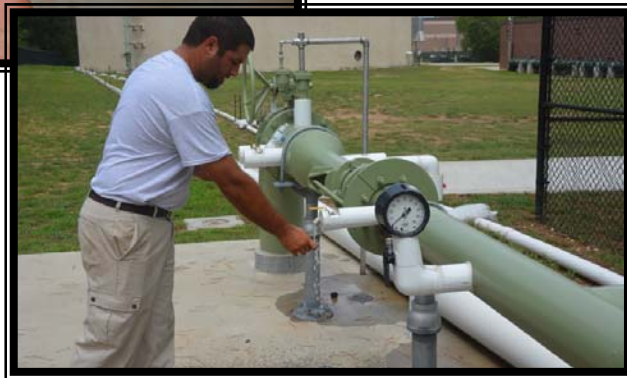
Transmission line dechlorination at the Woodlands Water Plant No. 5
