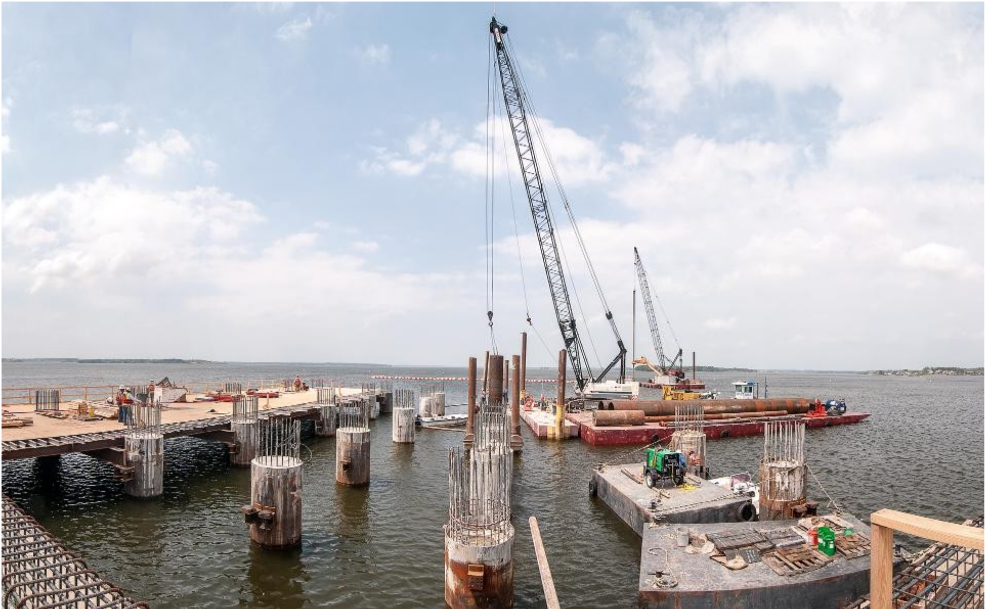
Pier Cylinder Placement at Raw Water Pump Station - April 10, 2013
