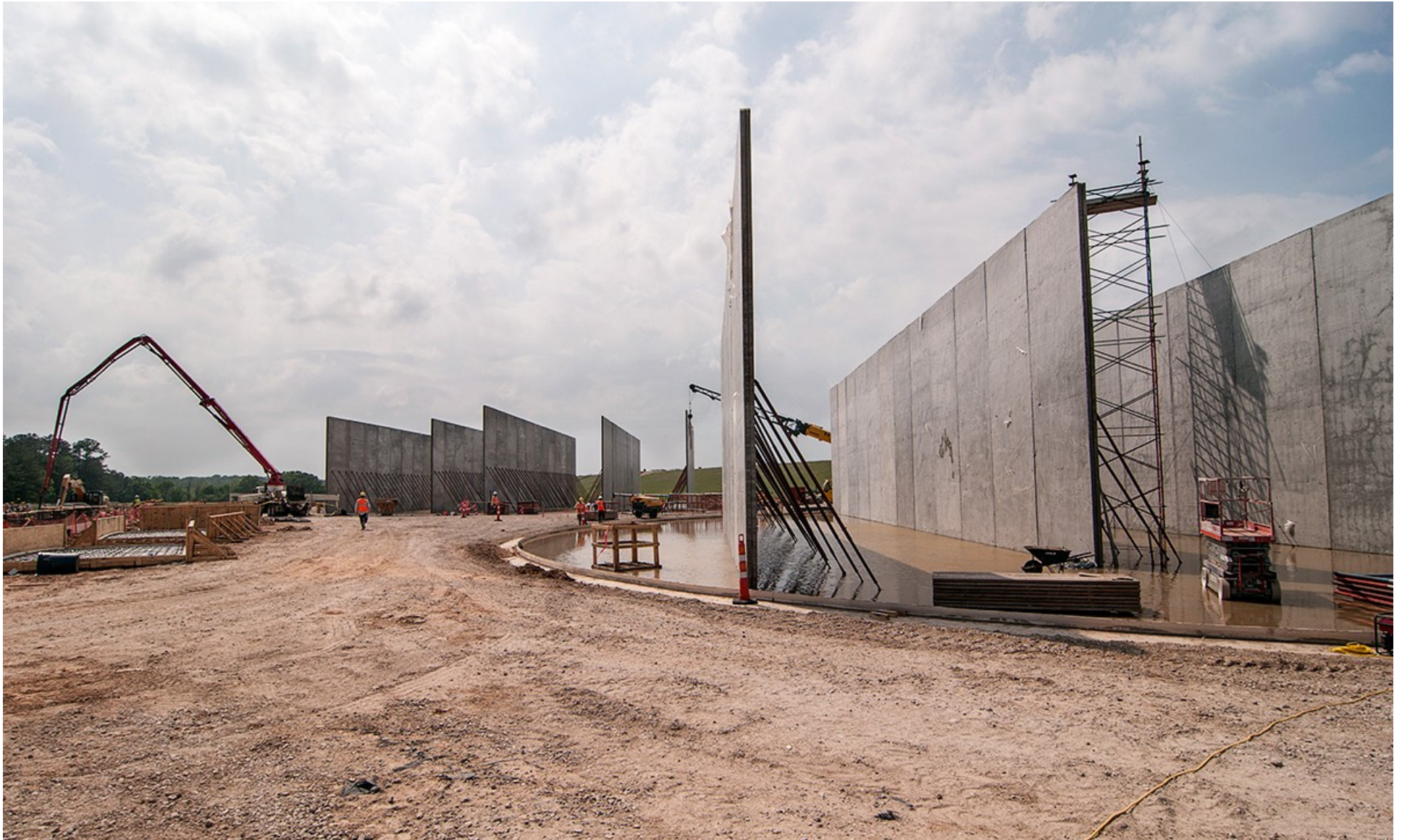
Ground Storage Tank Nos. 1 and 2 - Baffle walls complete and floors flooded for water curing of foundation - April 10, 2013
