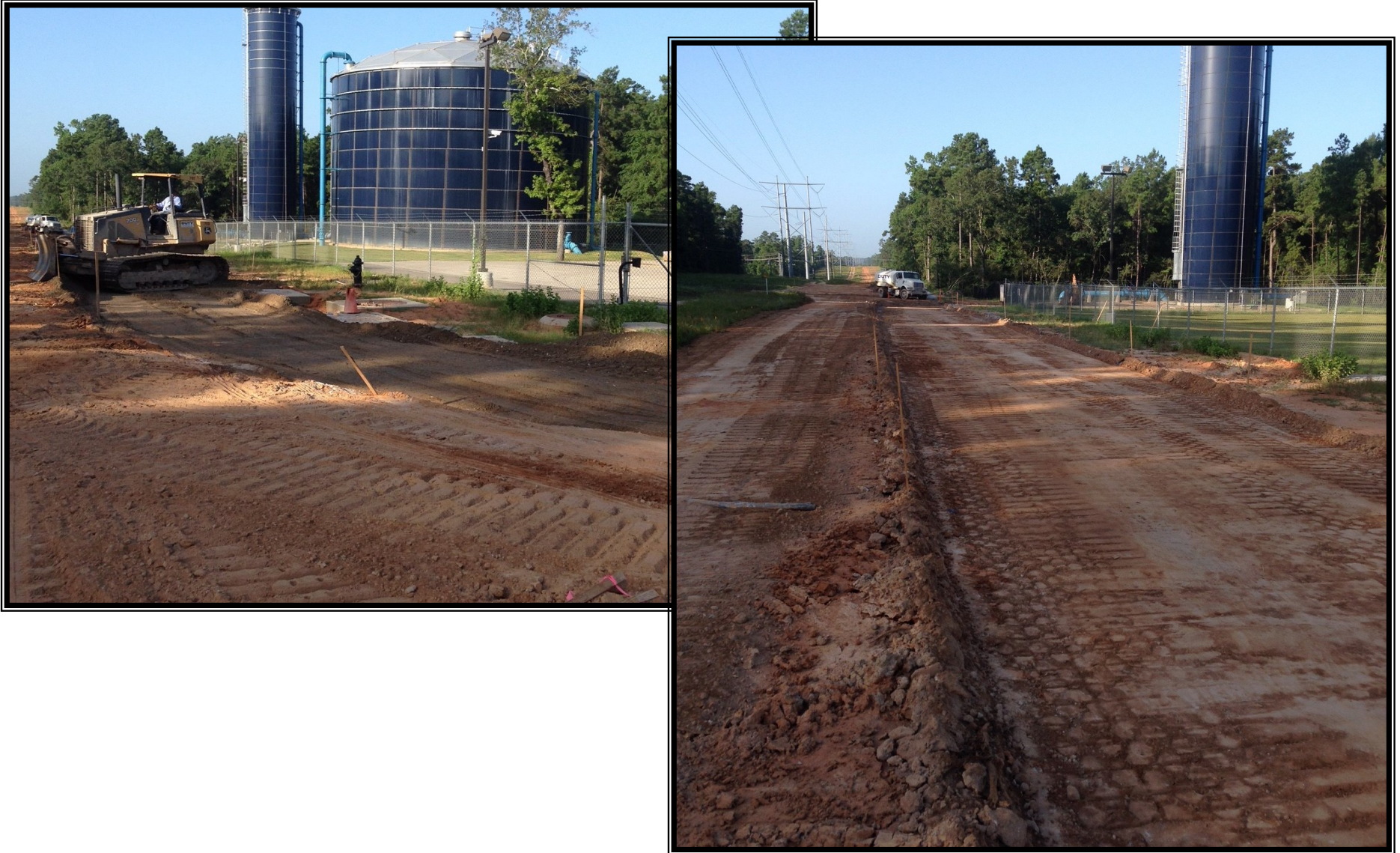
① Site grading in preparation of paving at the Standpipe
