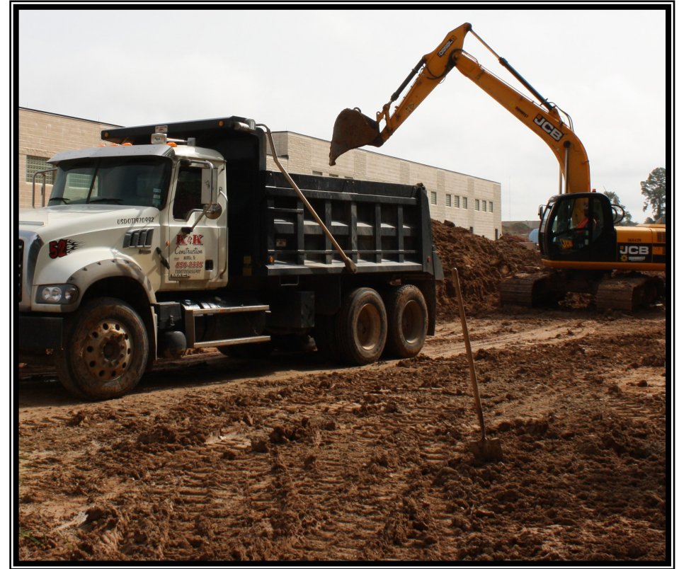
Left and Above—Contractors removing excess dirt from around High Service Pump Station
