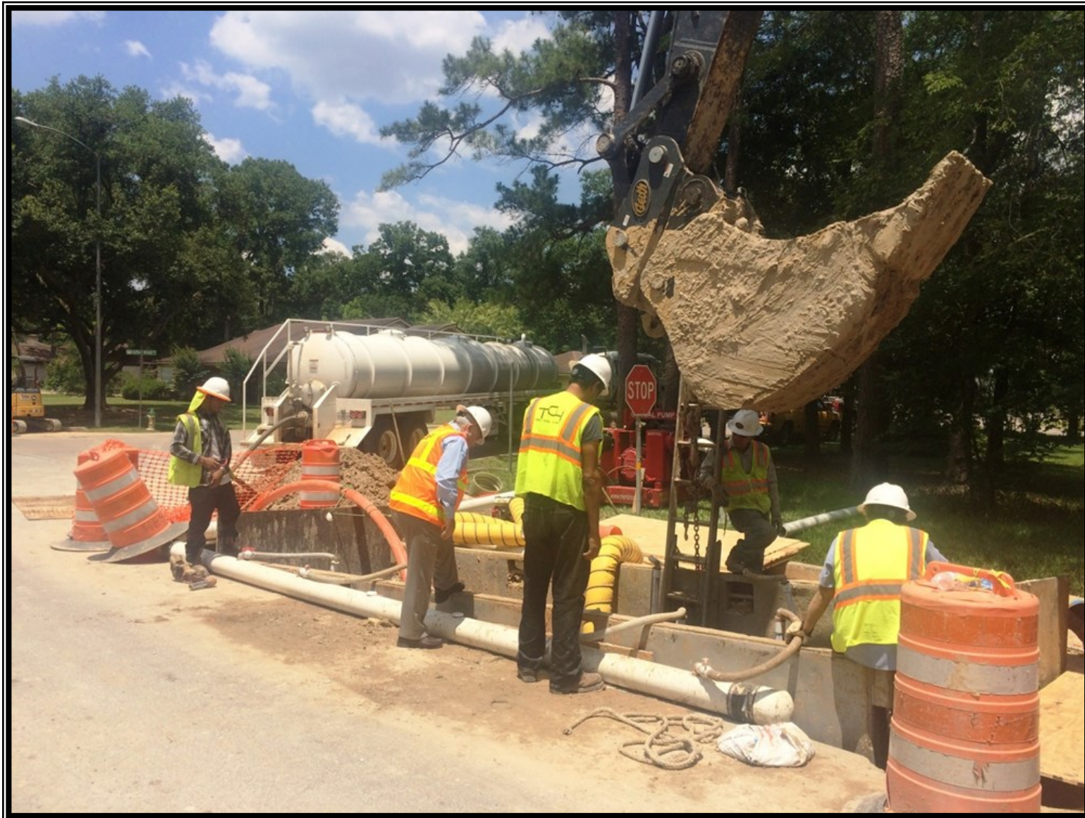
❶ Auger pit for installation of 30-inch steel casing under high pressure gas lines along Maplewood Drive
