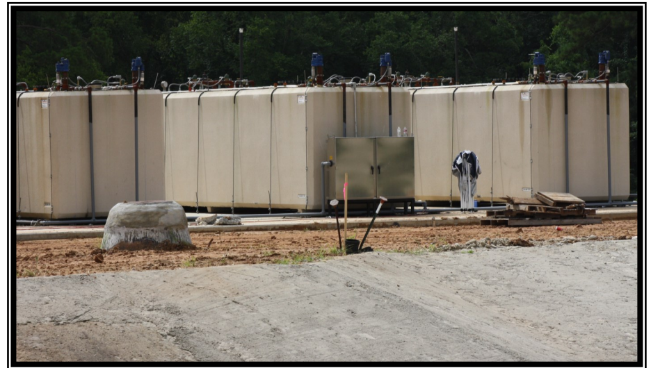
Fuel holding tanks located at the Power Supply Building
