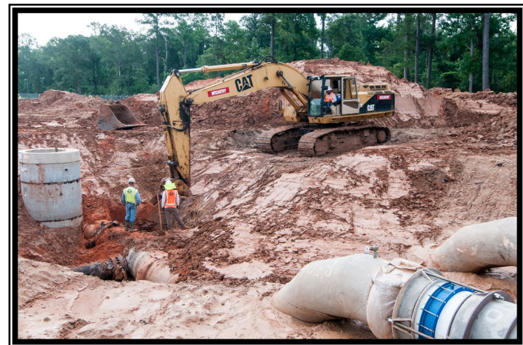
Workers backfilling transmission lines at the High Service Pump Station
