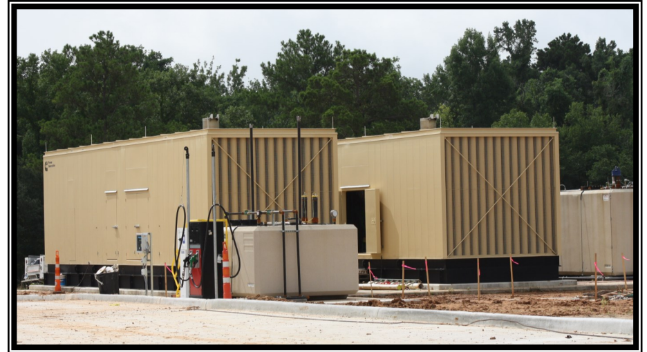
Facility generators located at the Power Supply Building
