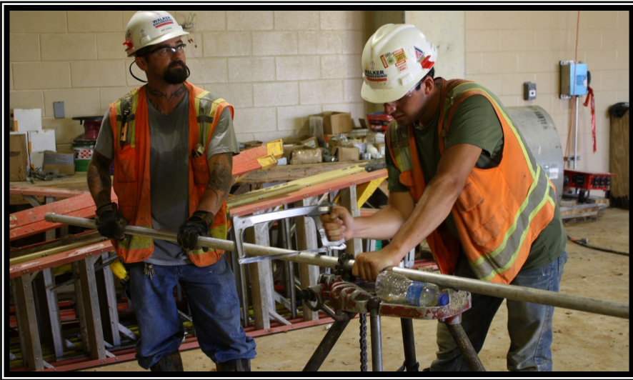
Workers cutting and threading pipe in the Solids Dewatering Building
