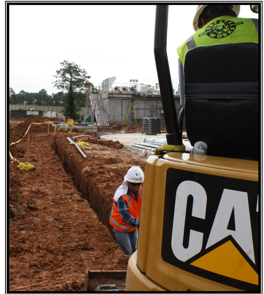
Workers installing conduit to the water meter for the City of Houston's raw water pumpage
