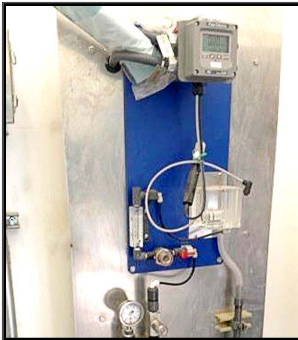
Water Receiving Facility chlorine analyzer
