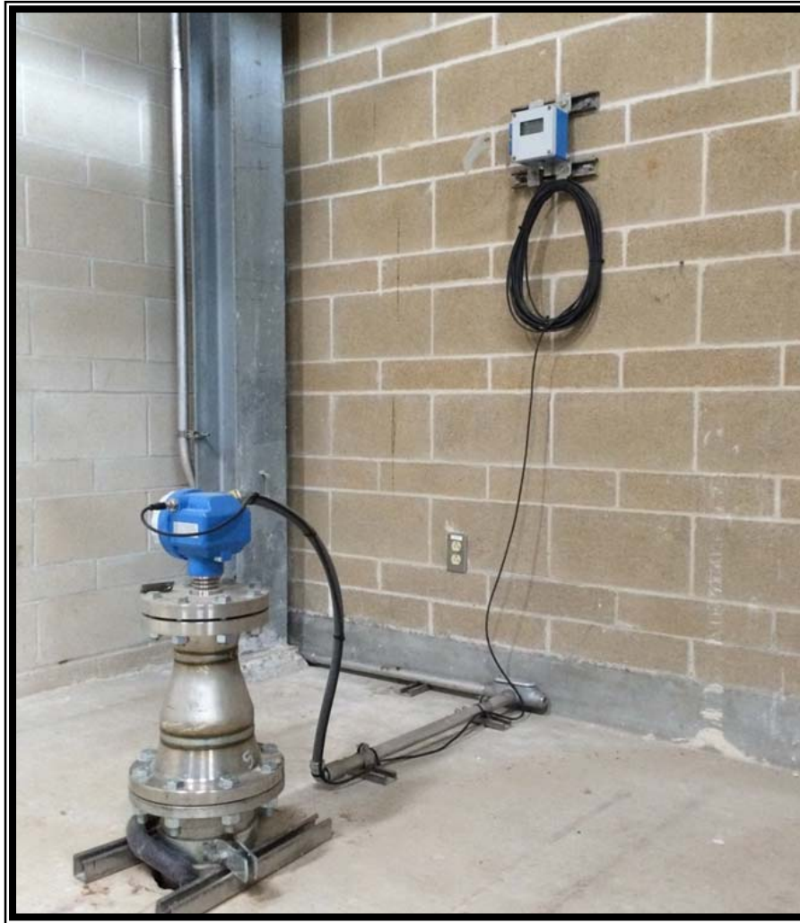
Level transmitters (lake and chemical tank)
