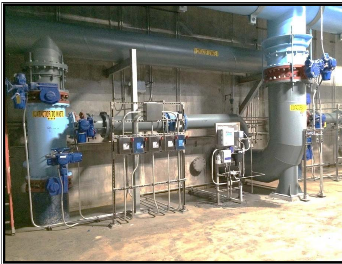
Granular Activated Carbon (GAC) control valves, flow meter, turbidimeter, and UV254 analyzer
