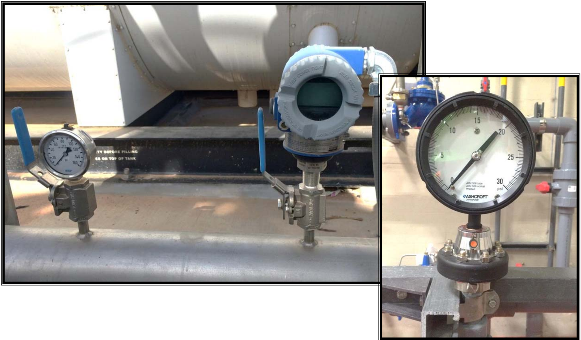
Pressure gauges and transmitters
