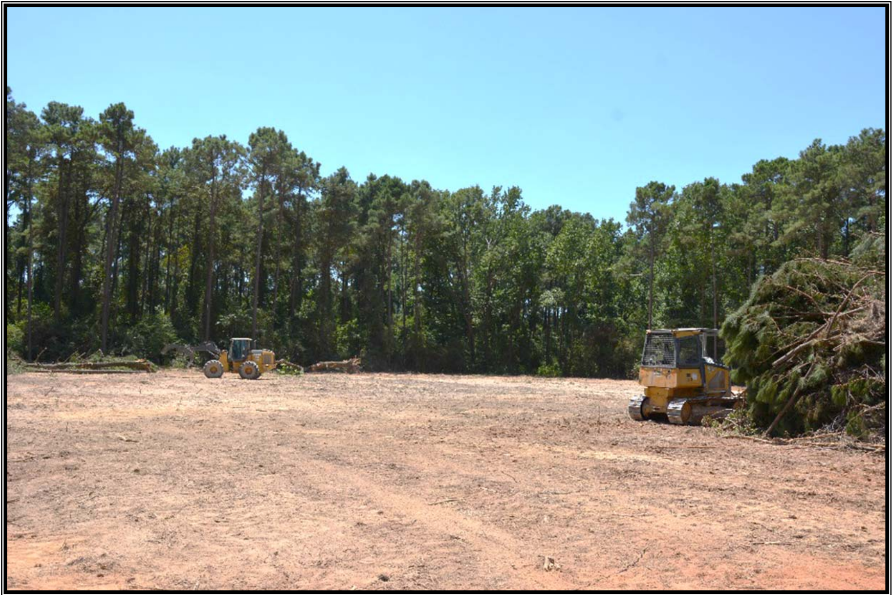
① Access Road—Detention pond clearing and grubbing
