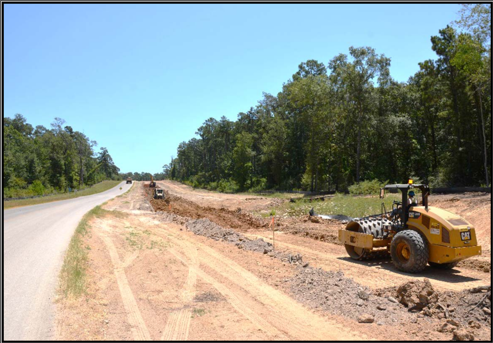
❶ Access Road—Subgrade preparation for eastbound boulevard section
