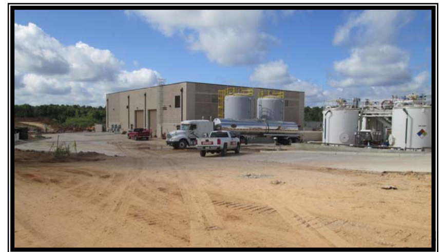
Lime delivery and storage at the Chemical Building
