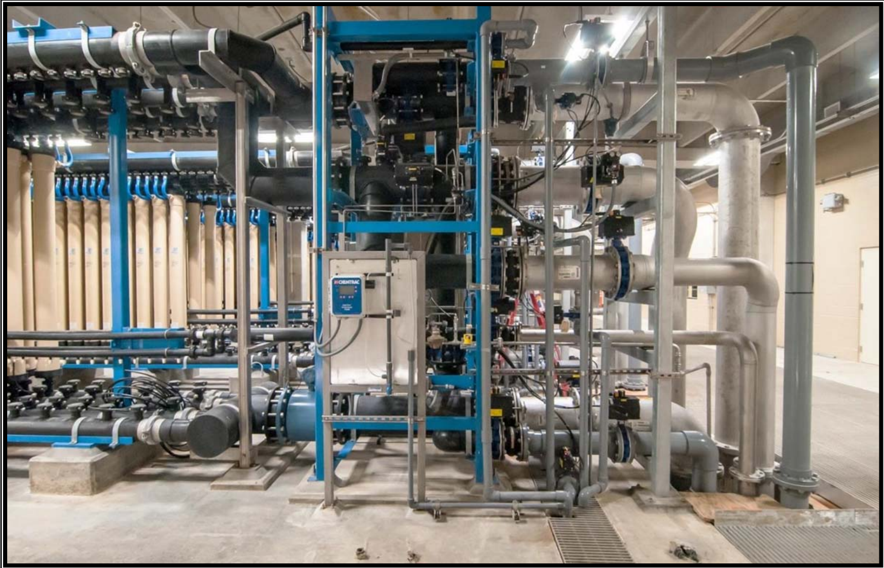
Membrane rack with valves, flow meter, and particle counter
