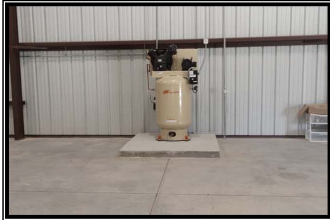
Air compressor system installed in the Maintenance Building
