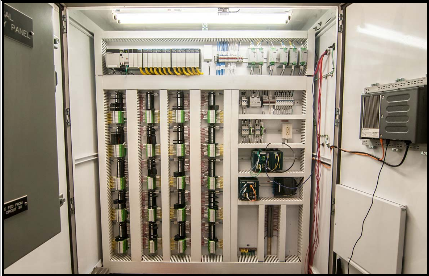
Programmable Logic Controller (PLC) Panel—Programmed by SJRA staff
