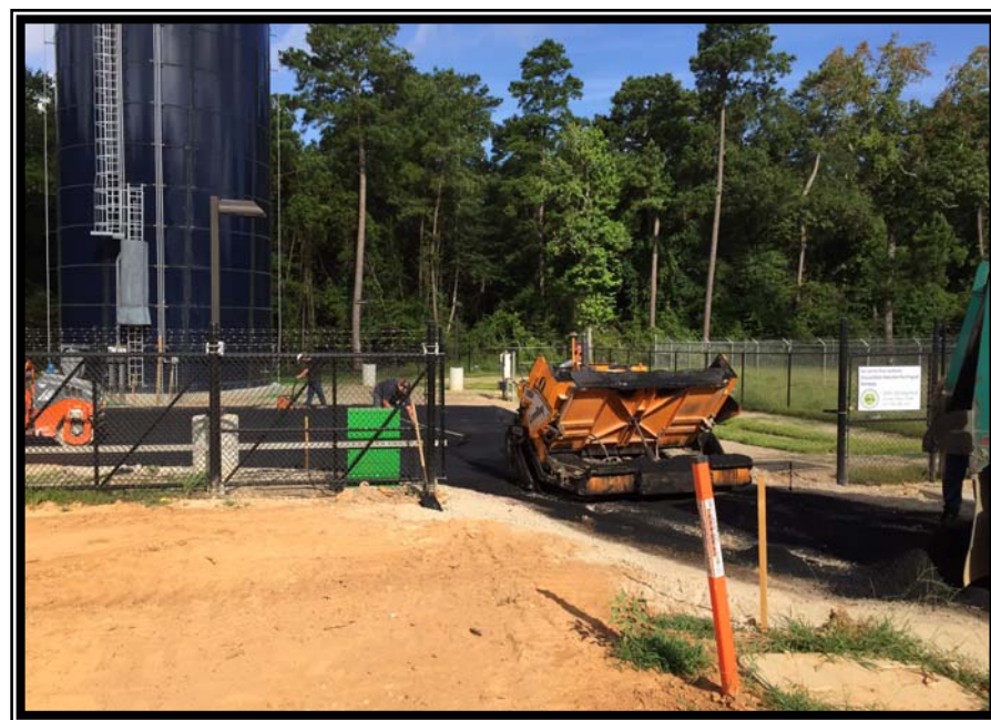
Workers paving site with asphalt at the Standpipe
