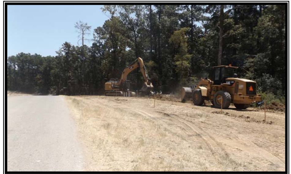
Above—Clearing and grading of temporary access road Left— Gravel placement on temporary access road
