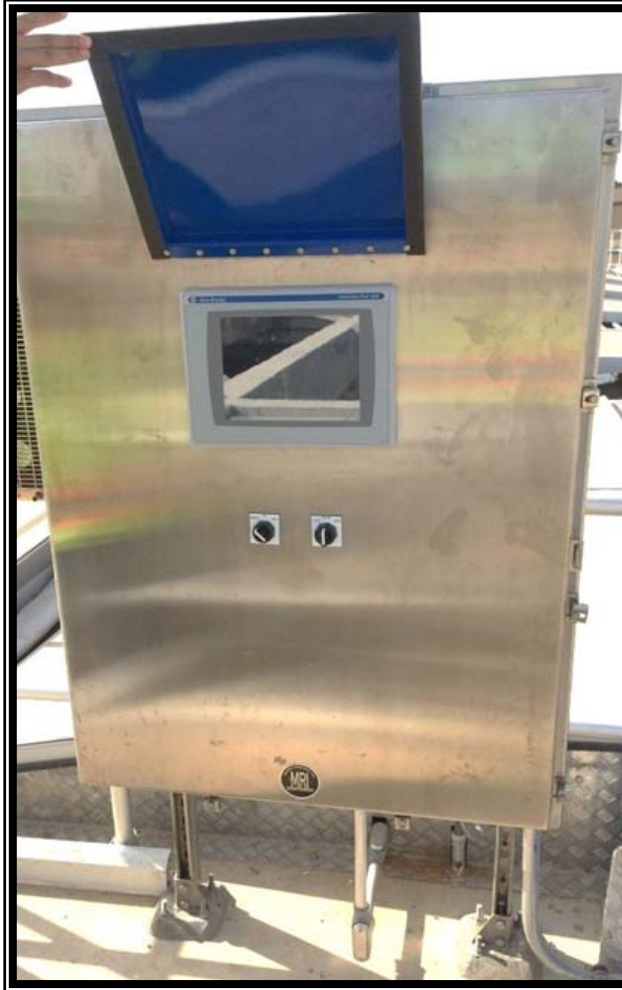
Programmable Logic Controller (PLC) panels—Programmed by vendor
