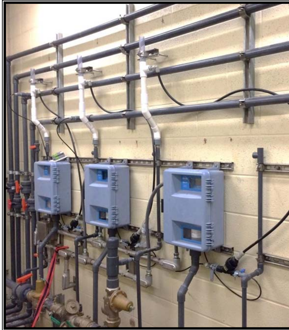
Surface Water Treatment Facility chlorine analyzers
