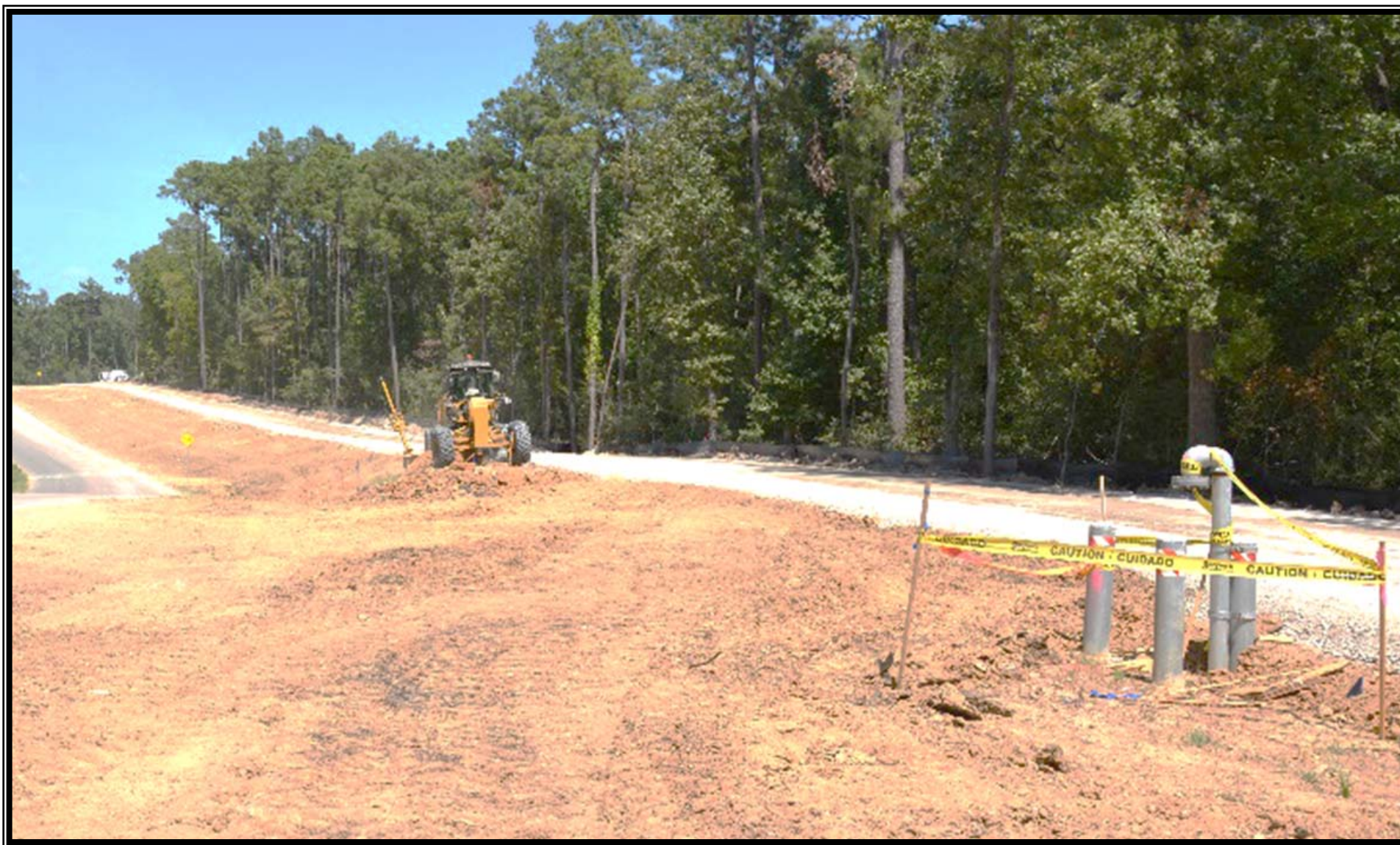
① Access Road—Temporary bypass roadway installation
