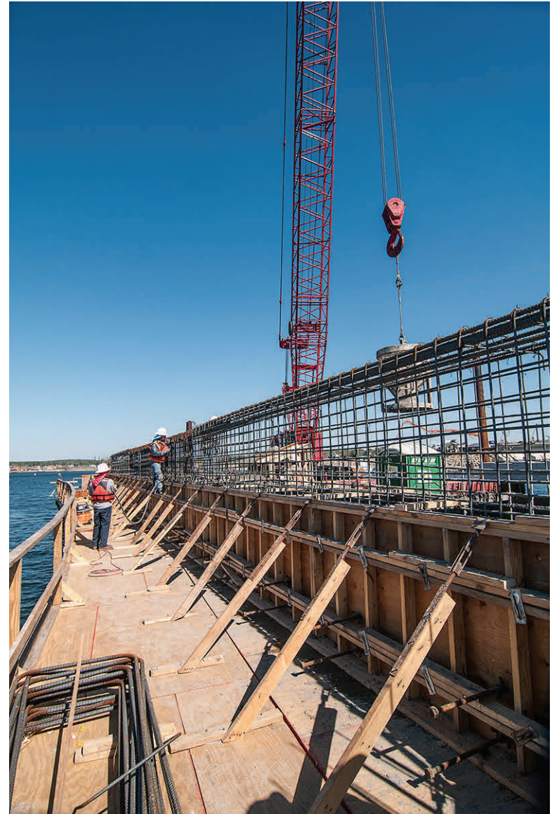
Raw Water Pump Station - Concrete pour at new beam - March 15, 2013
