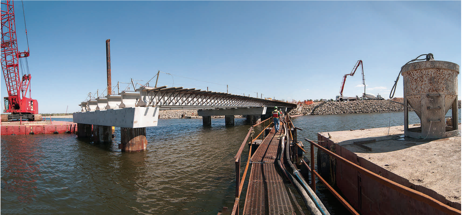
Raw Water Pump Station - View from current end of bridge structure looking toward the Dam - March 15, 2013
