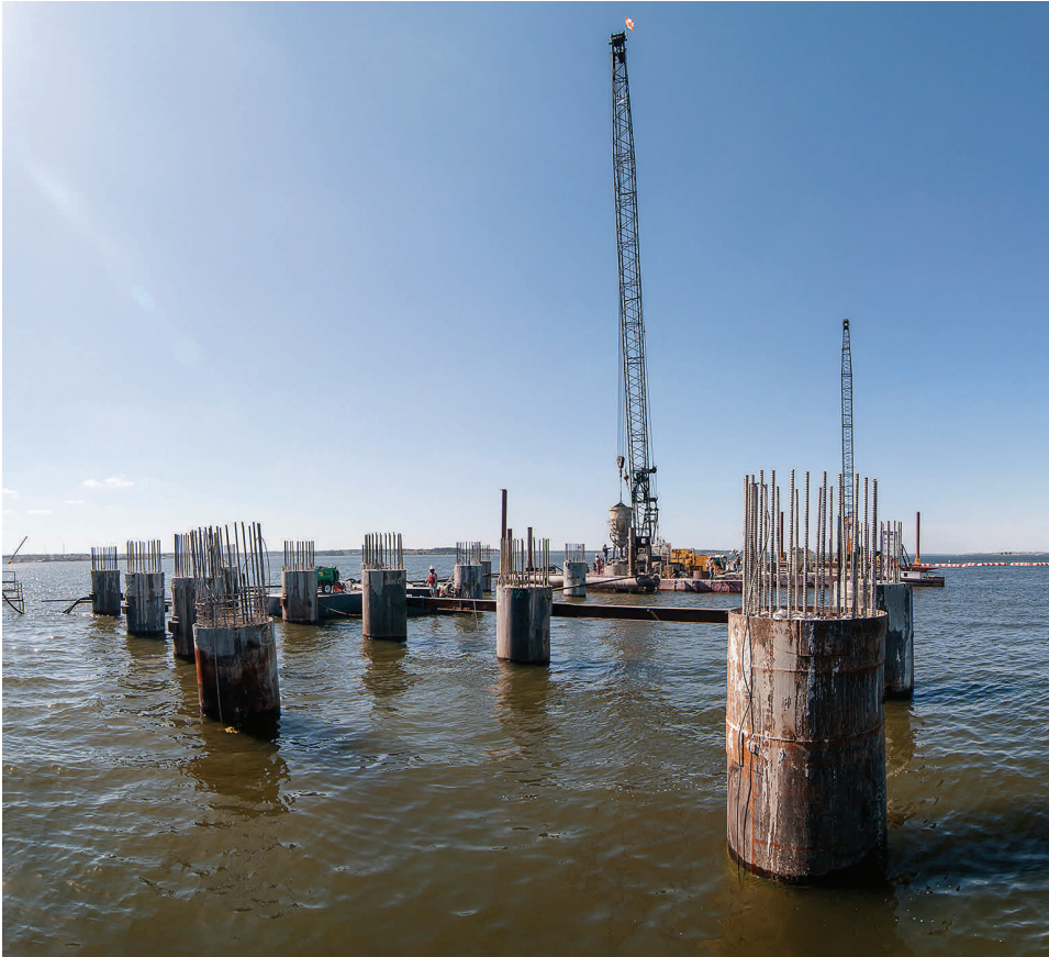
Raw Water Pump Station - Continuation of pier installation - March 15, 2013
