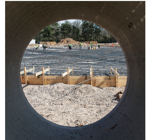
Reinforcement steel installation at Ground Storage Tank No. 2
