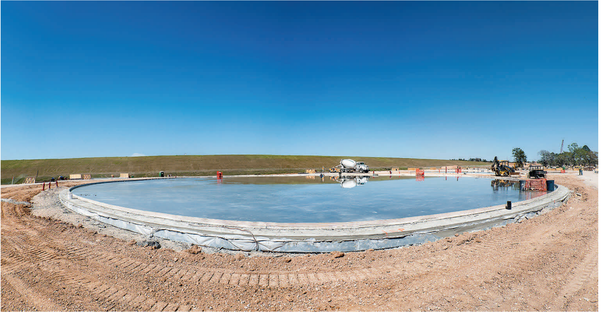
Ground Storage Tank No. 1 flooded for water curing of foundation- March 15, 2013
