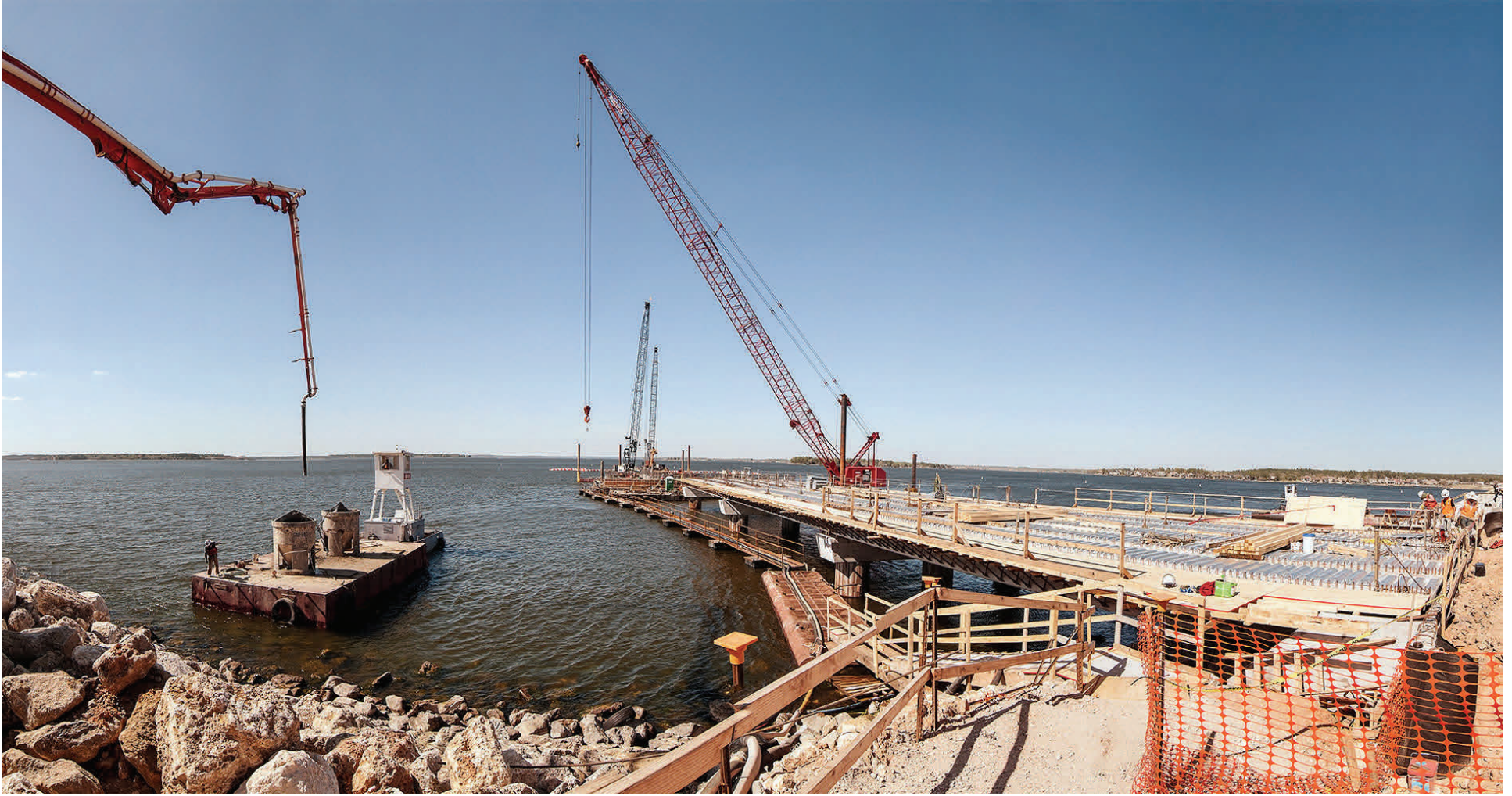
Concrete pouring operation at Raw Water Pump Station - March 15, 2013
