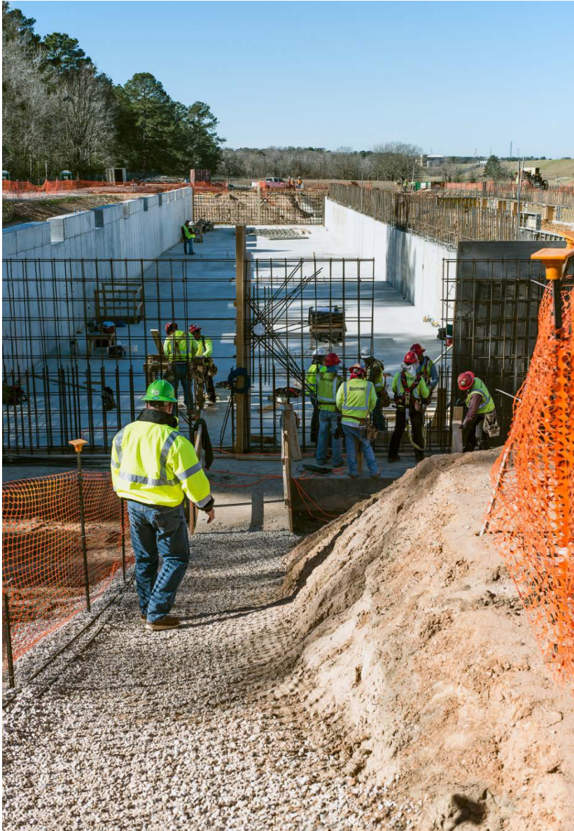
High Service Pump Station – Pipe Discharge Bay
