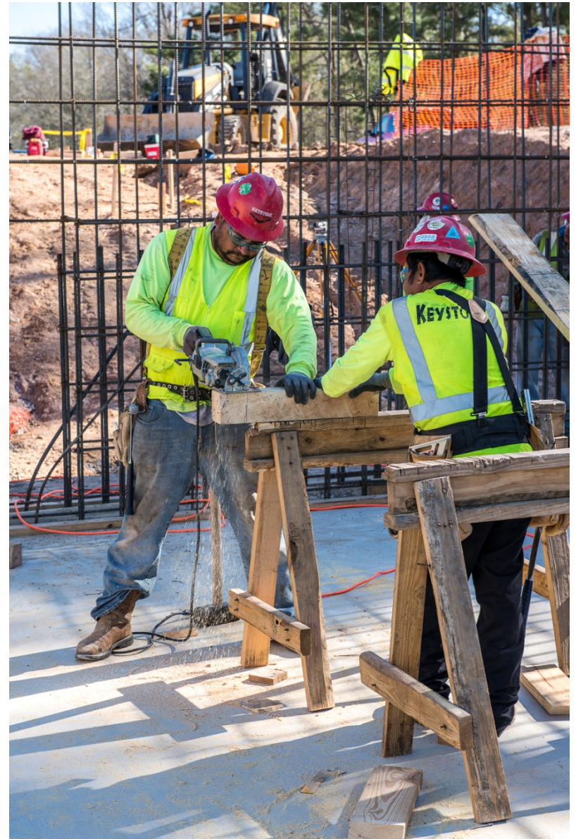
Workers install forms prior to concrete placement
