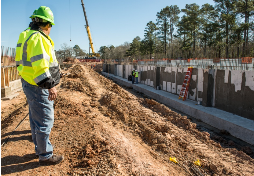
High Service Pump Station pipe discharge bay looking east
