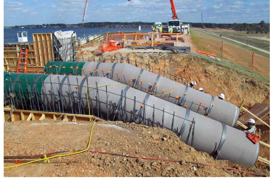
Dual 48-inch pipe crossing over Lake Conroe Dam
