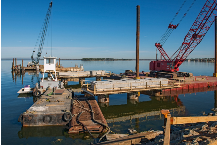
Bent caps in place on piers at Raw Water Pump Station
