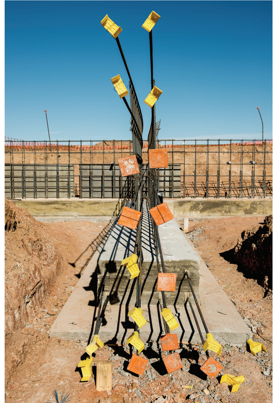
Future wall at High Service Pump Station Discharge Structure
