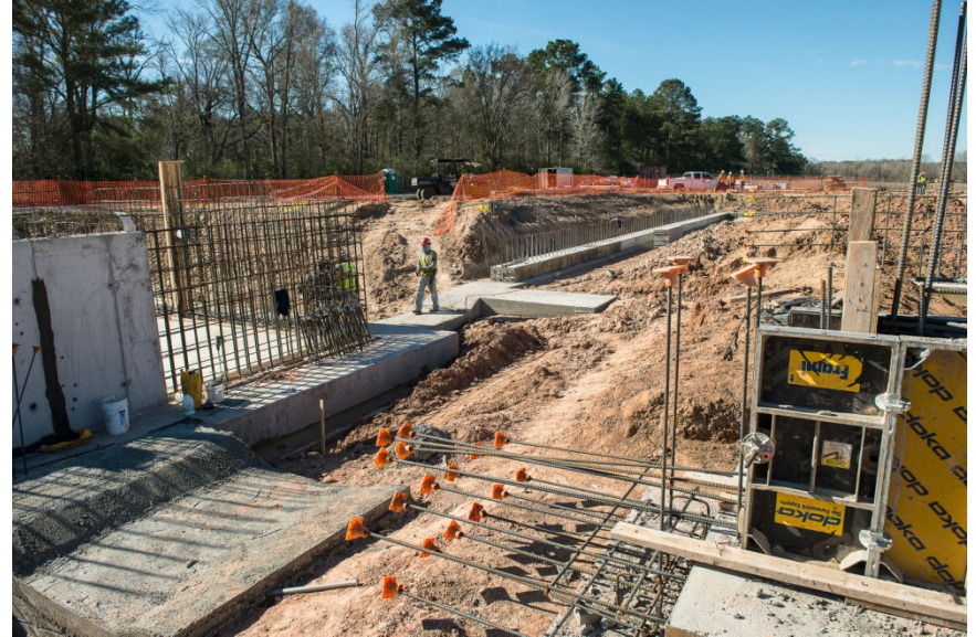
High Service Pump Station pipe discharge bay looking west
