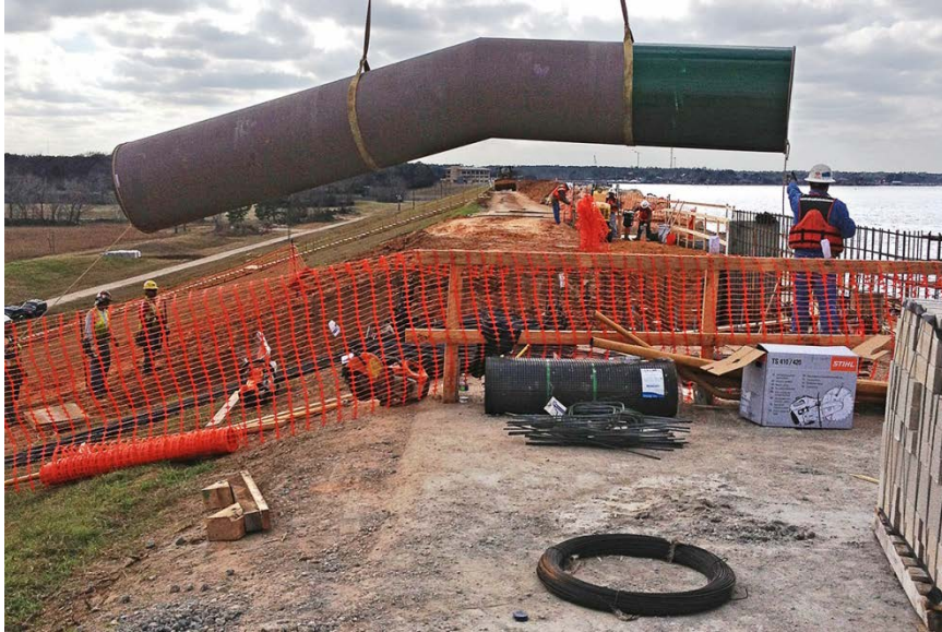
First of two 48-inch pipe crossings over Lake Conroe Dam
