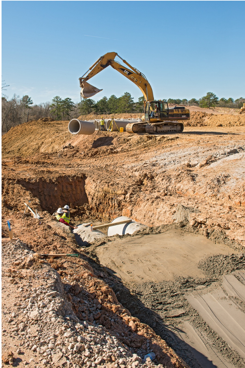
Drainage culvert installation at main entrance road
