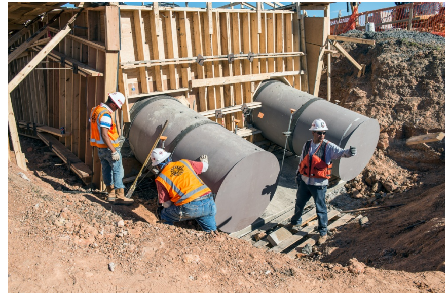
Workers examine pipe installation
