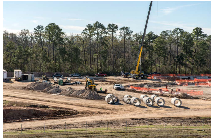
Ground Storage Tank site preparation
