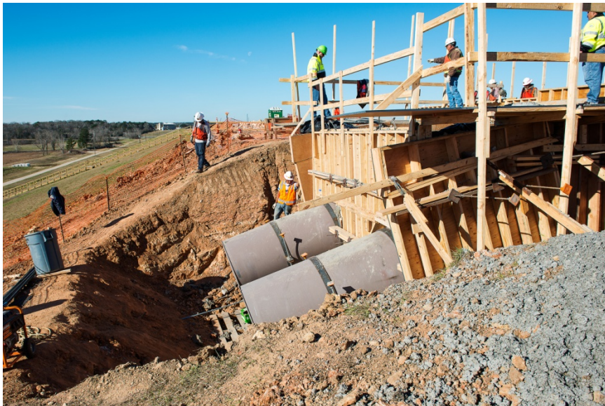
Forming for dual 48-inch pipe encasement
