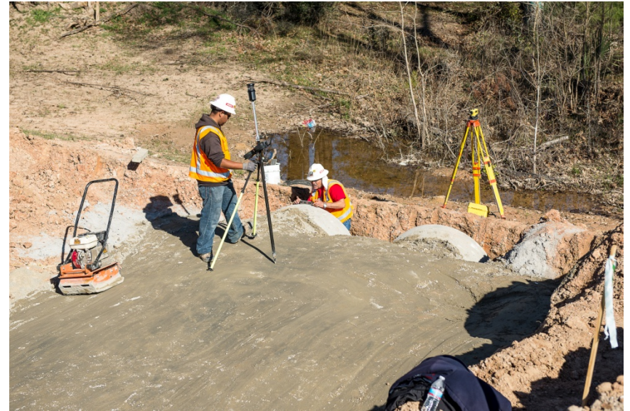
Workers check grade of drainage culverts
