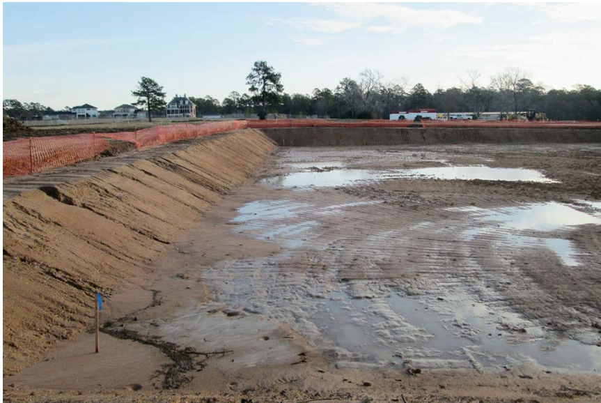
Excavation at Membrane Facility
