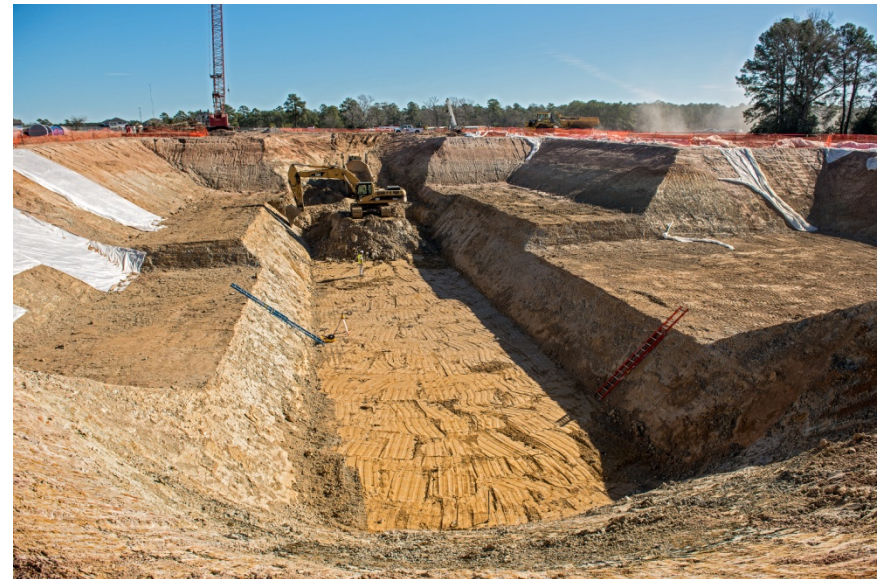
Excavation for Granular Activated Carbon Facility
