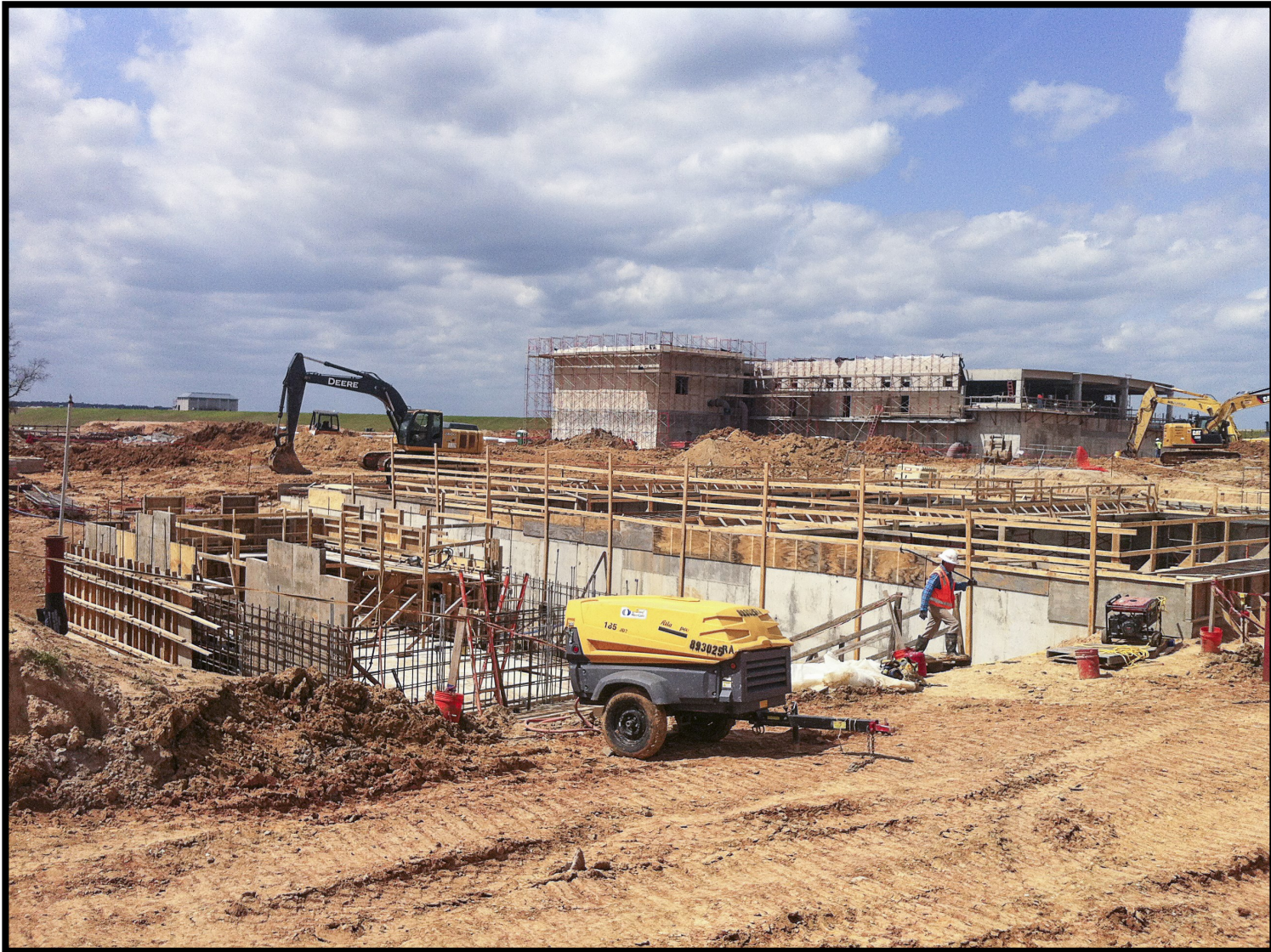
⑧ Concrete installation at Backwash Equalization
