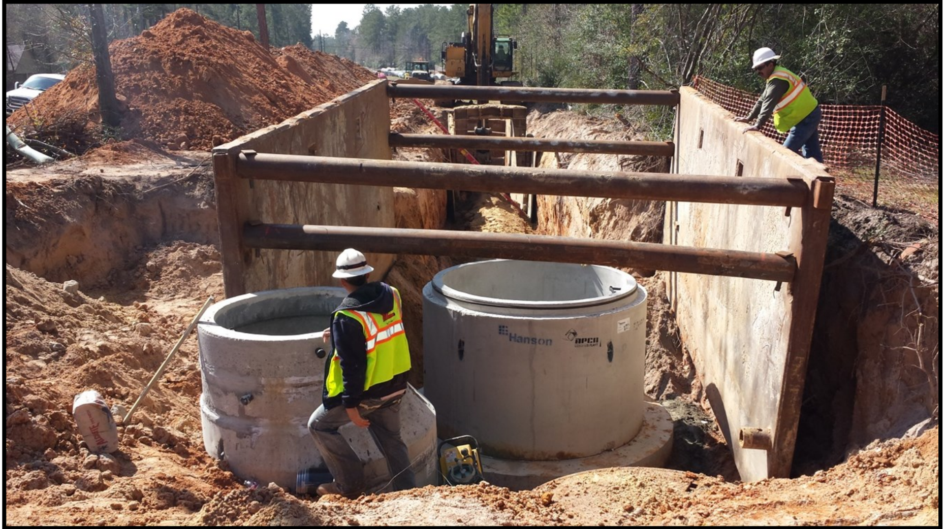
① Segment T3—Manhole installation along Sendera Ranch Road
