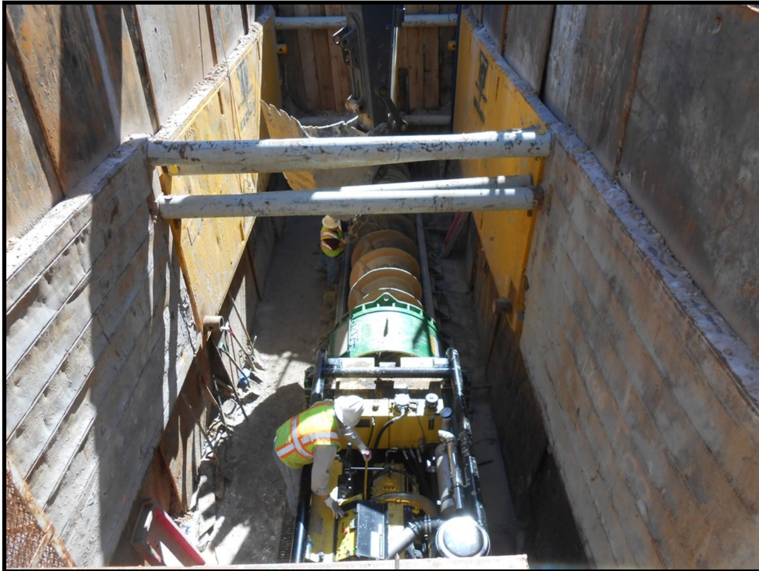
① Segment W2B - Tunnel operation at Grogans Mill Road and High Timbers Drive
