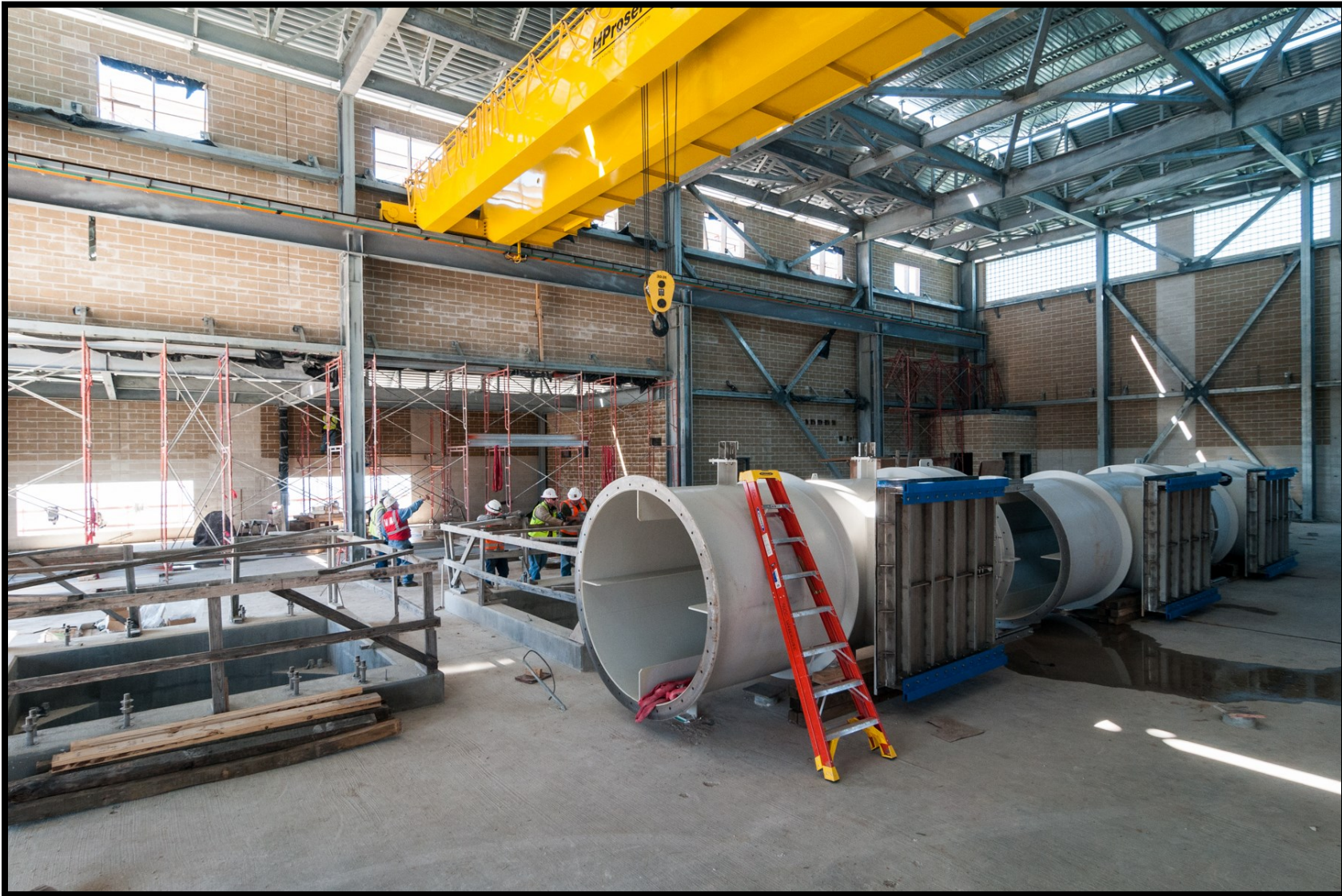
① Interior view of masonry installation at Raw Water Intake
