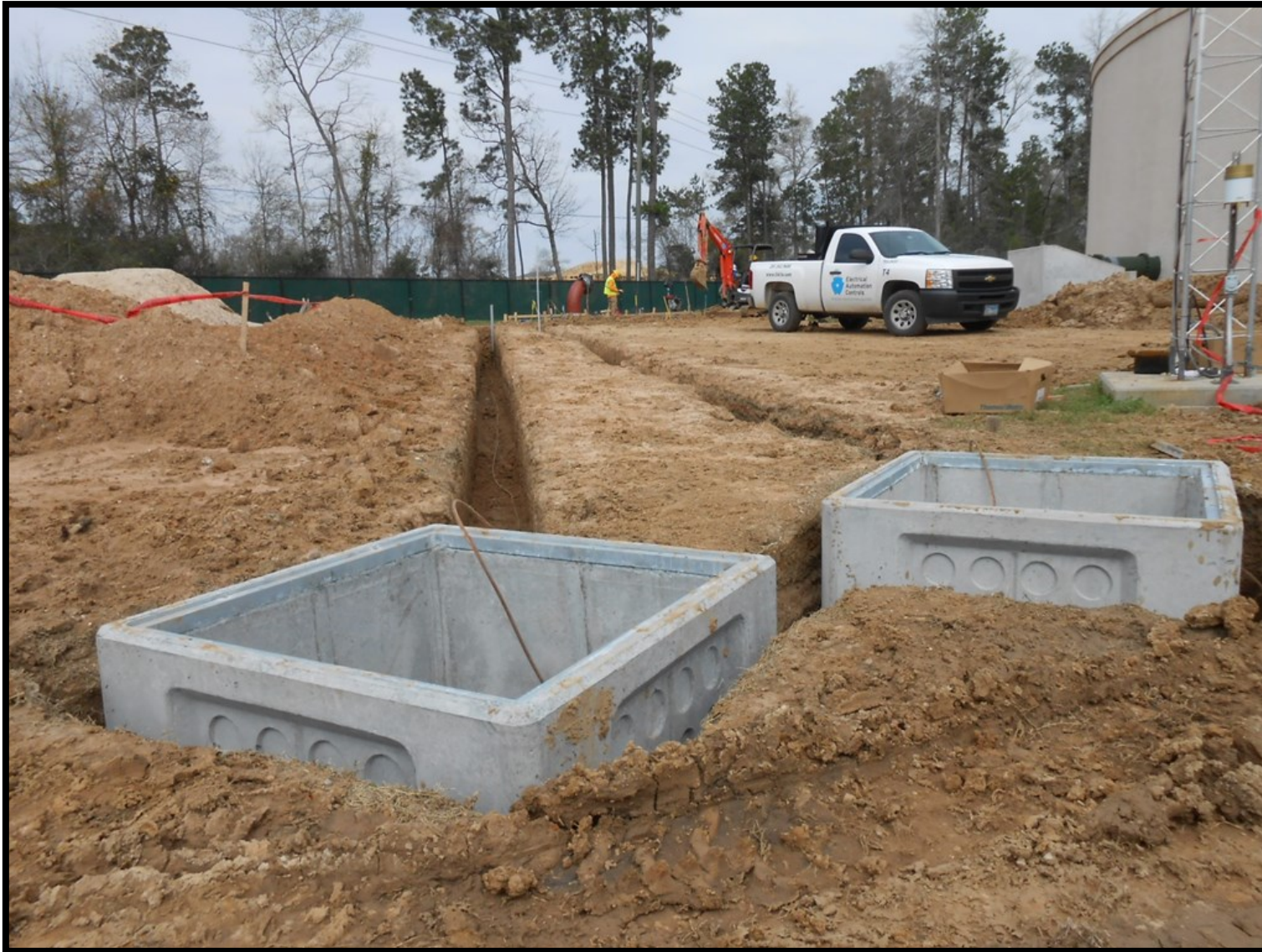
① Water Receiving Facilities—South—Electrical junction box installation and duct bank excavation at SJRA Water Plant No. 4
