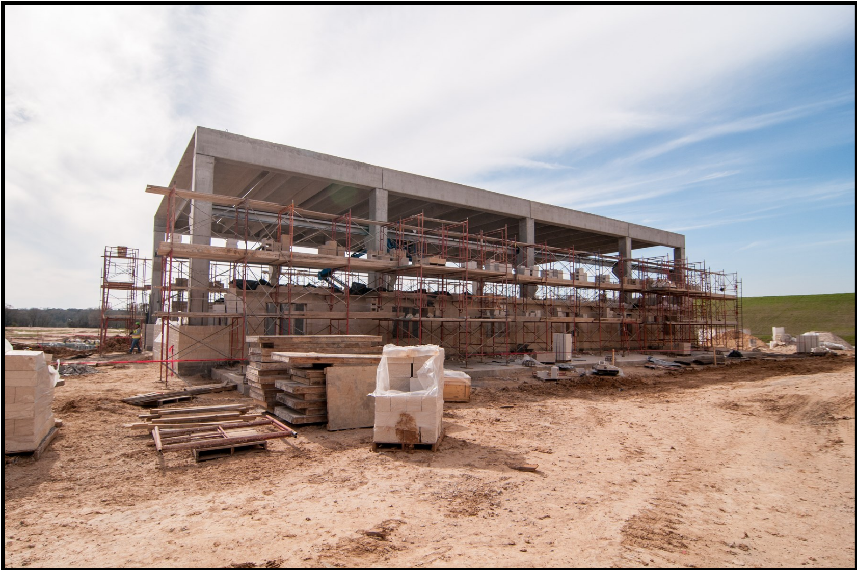
⑥ Masonry installation at Blower Building
