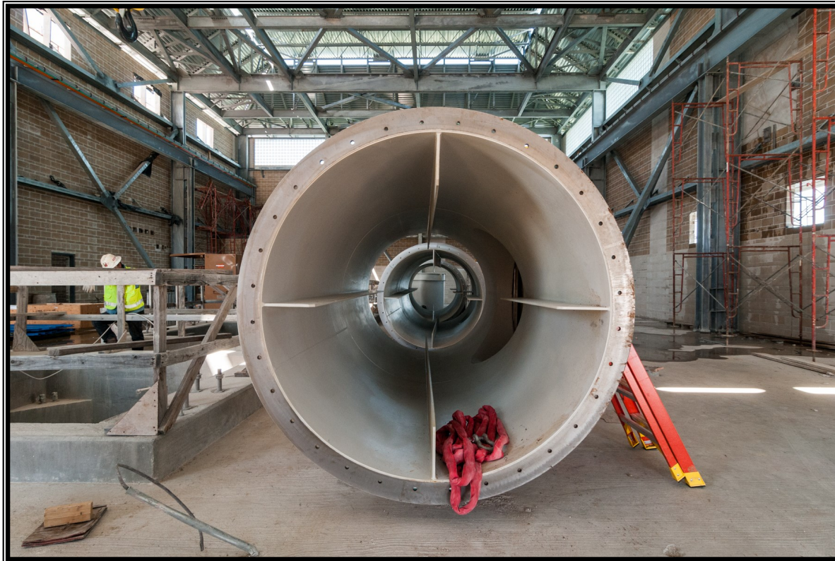
Pump barrel being stored at Raw Water Intake at Surface Water Facilities
