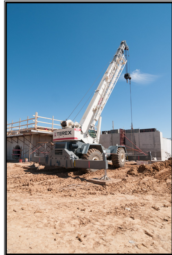
Progress at GAC Building at Surface Water Facilities
