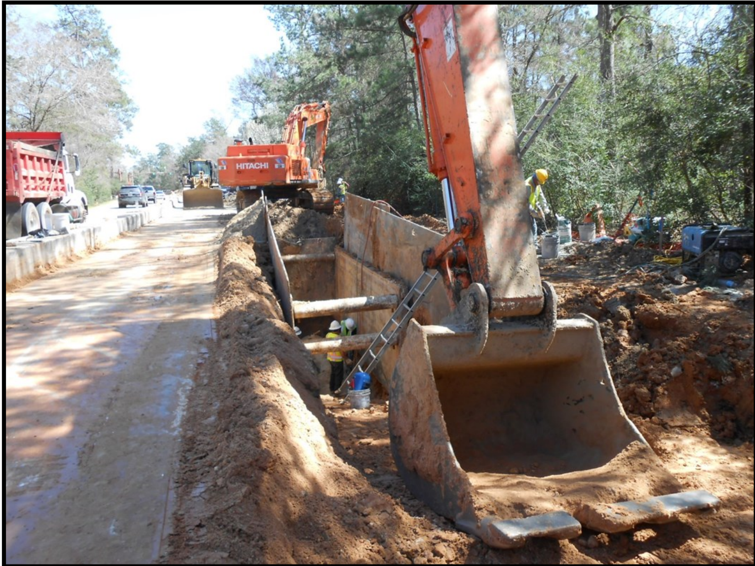
① Segment W1B - Open cut operations along Research Forest Drive
