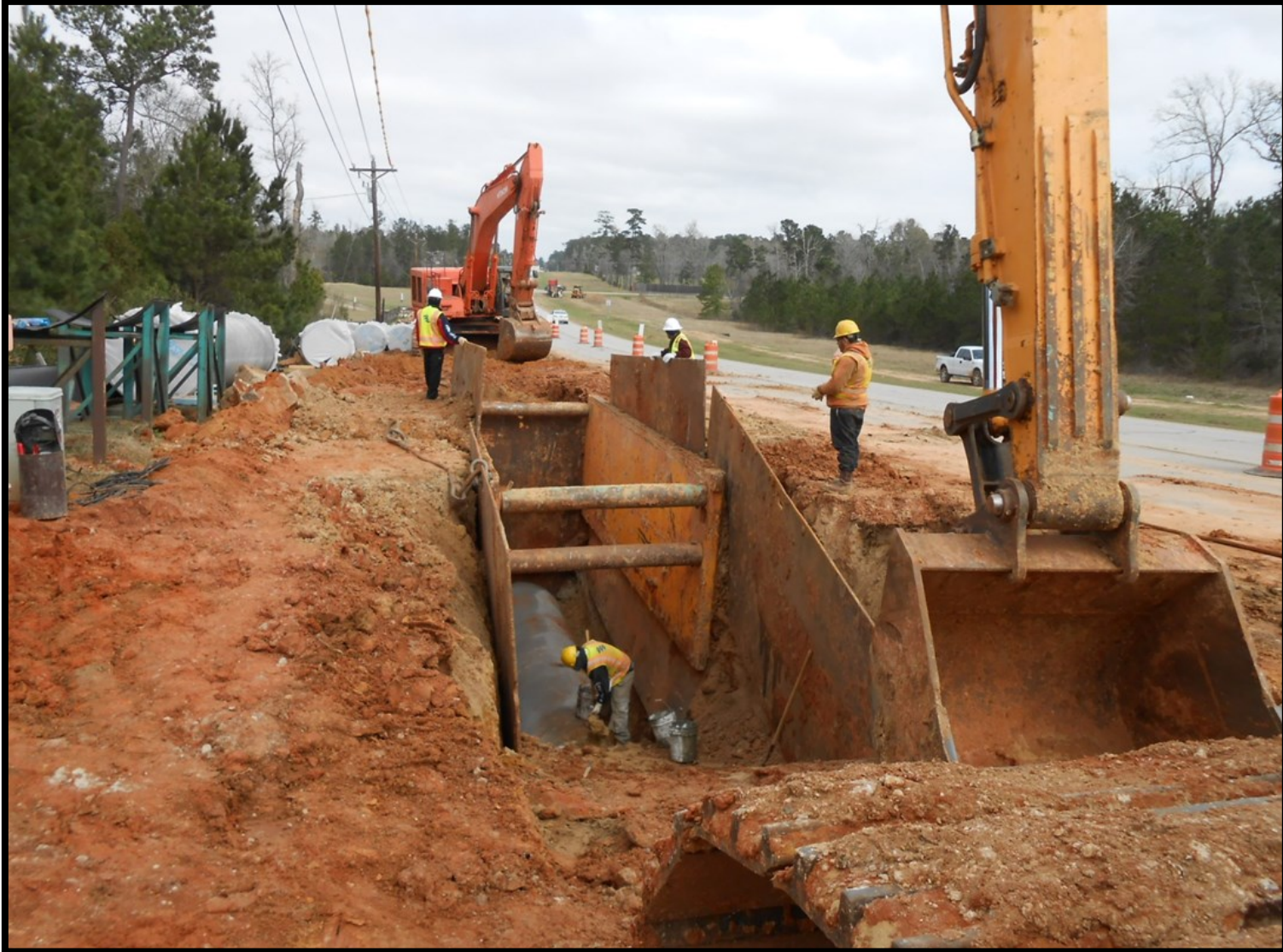
① Segment T2 - 54-inch pipe installation along Fish Creek Thoroughfare
