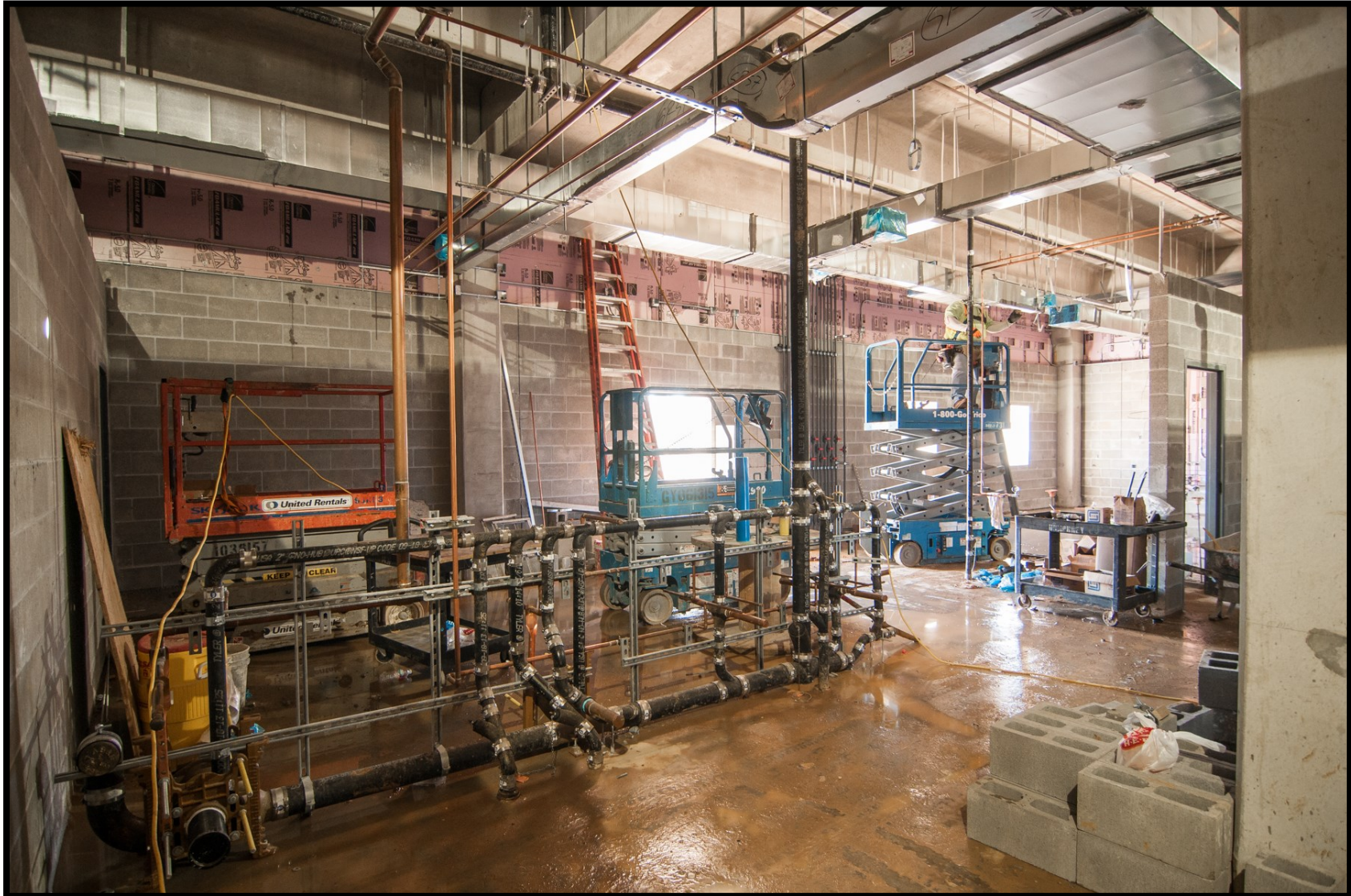
3 Mechanical and plumbing rough-in at Membrane Building
