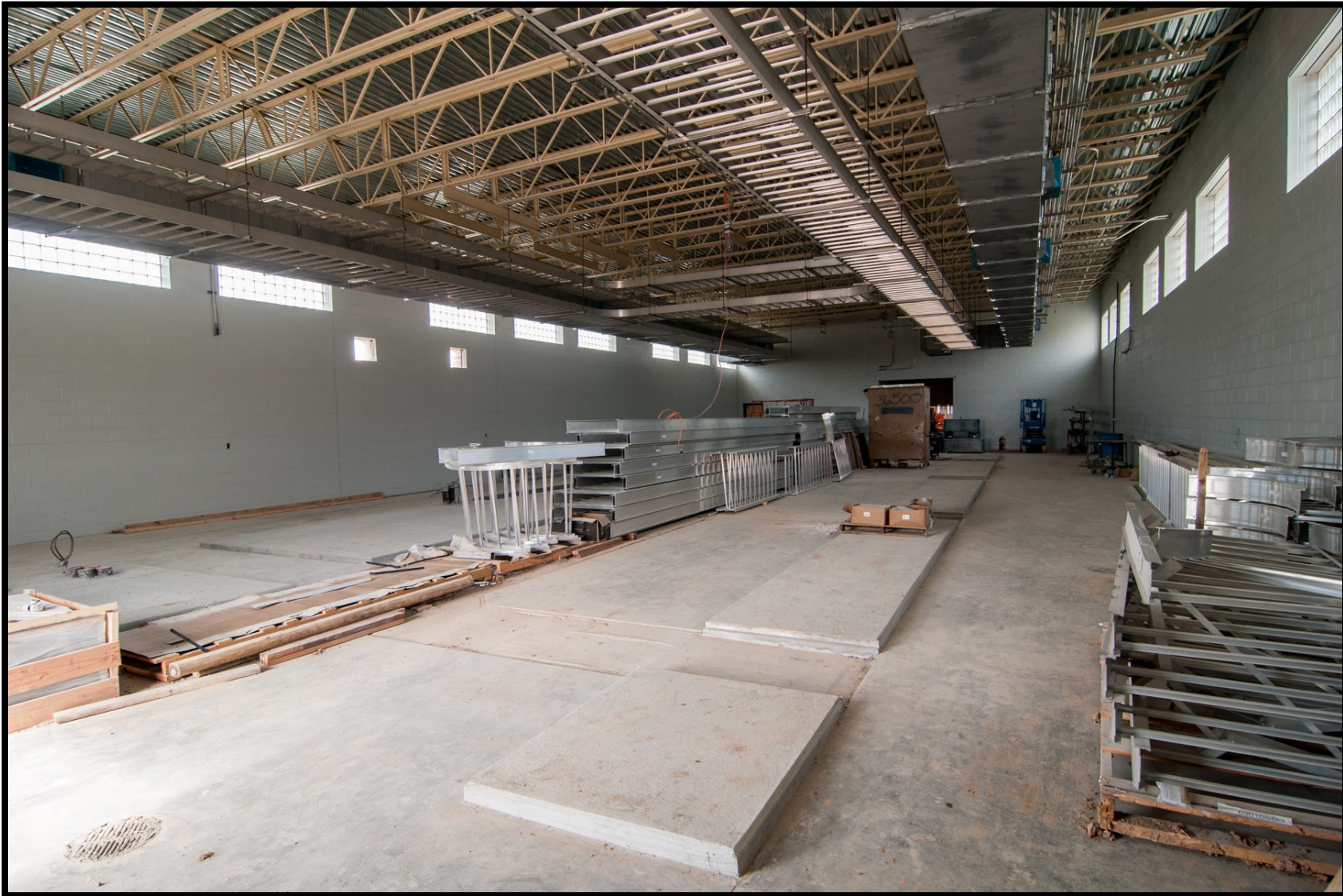
⑤ Electrical room at High Service Pump Station
