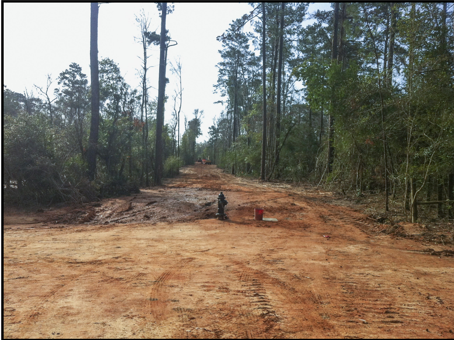
① Segment C1B - Site restoration along Longmire Road
