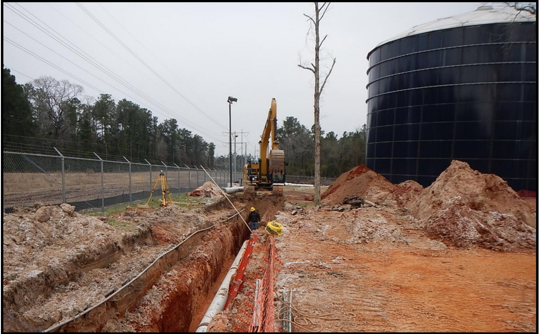
❶ Water Receiving Facilities—North— Yard piping installation at City of Conroe Water Plant No. 21
