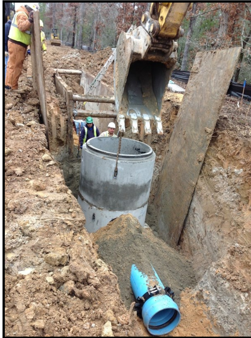
① Segment C3—Manhole and 20-inch pipe installation along Pollok Drive
