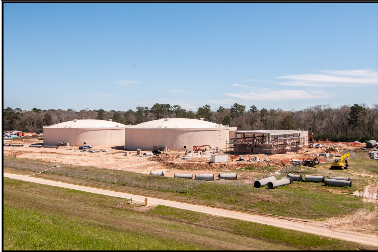
View of Groundwater Storage Tank Nos. 1 and 2 and Blower Building at Surface Water Facilities
