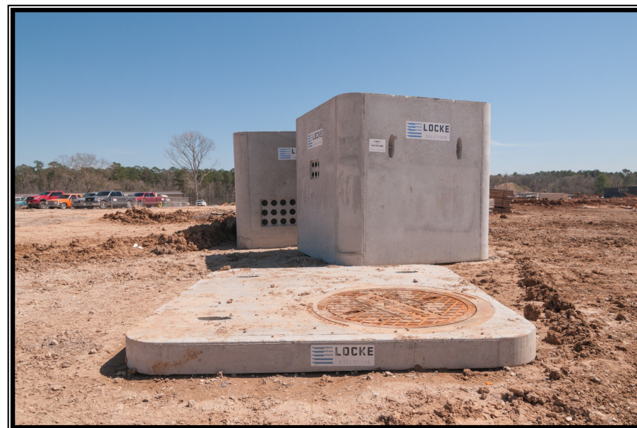
Electrical manholes on site at Surface Water Facilities
