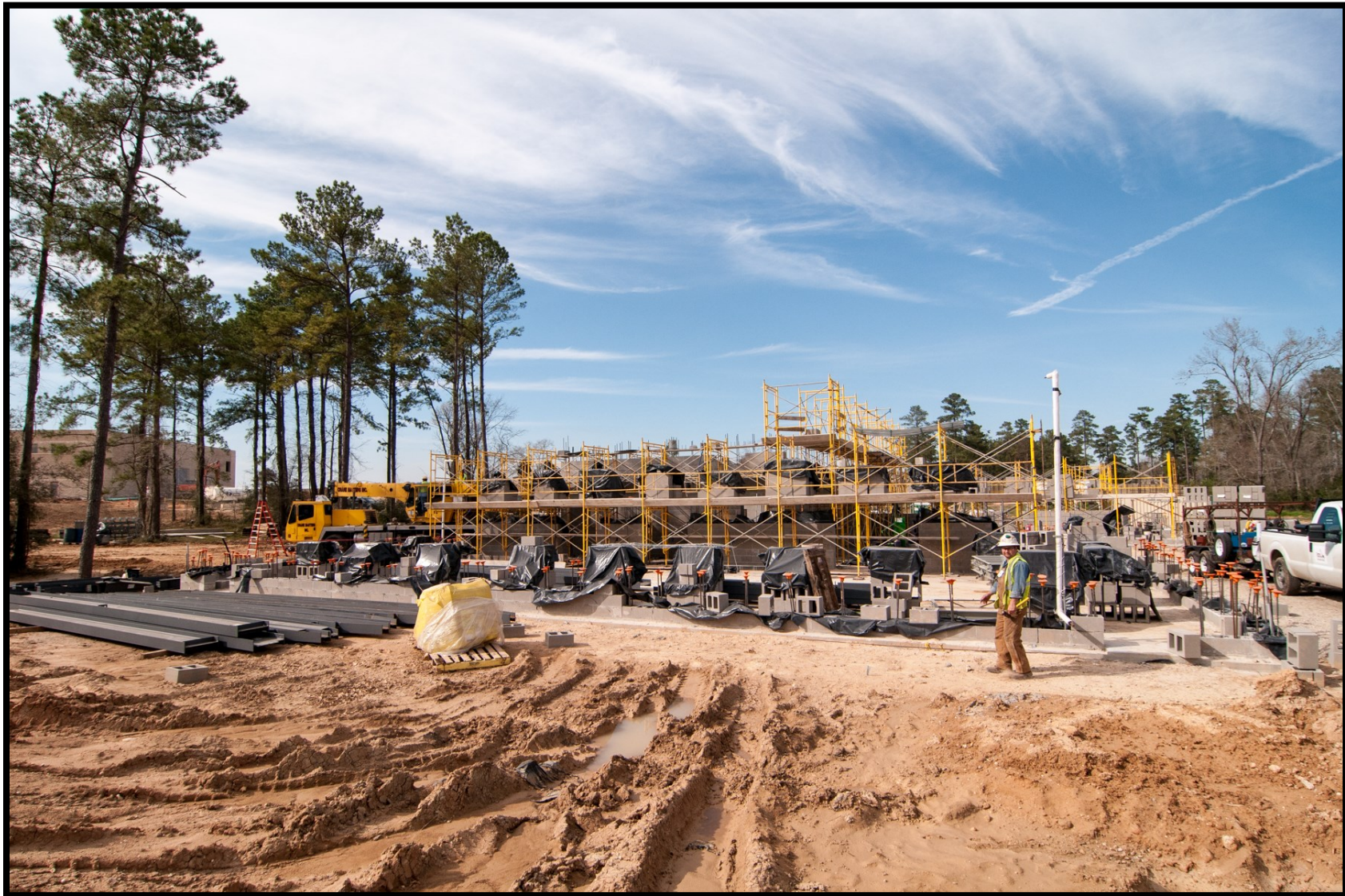
⑩ Masonry installation in progress at Operations Building
