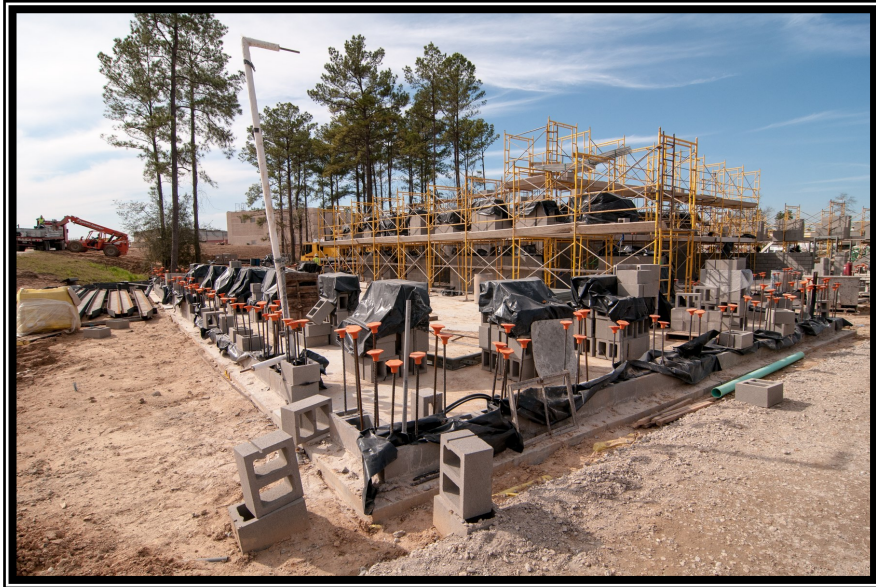
Construction progress at GRP Operations Building
