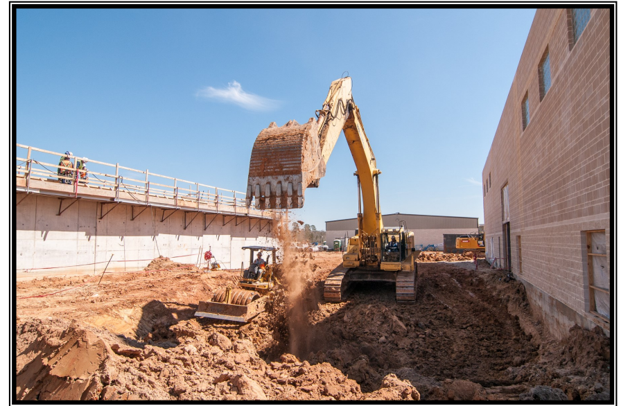
Construction between Pretreatment and Membrane buildings at Surface Water Facilities
