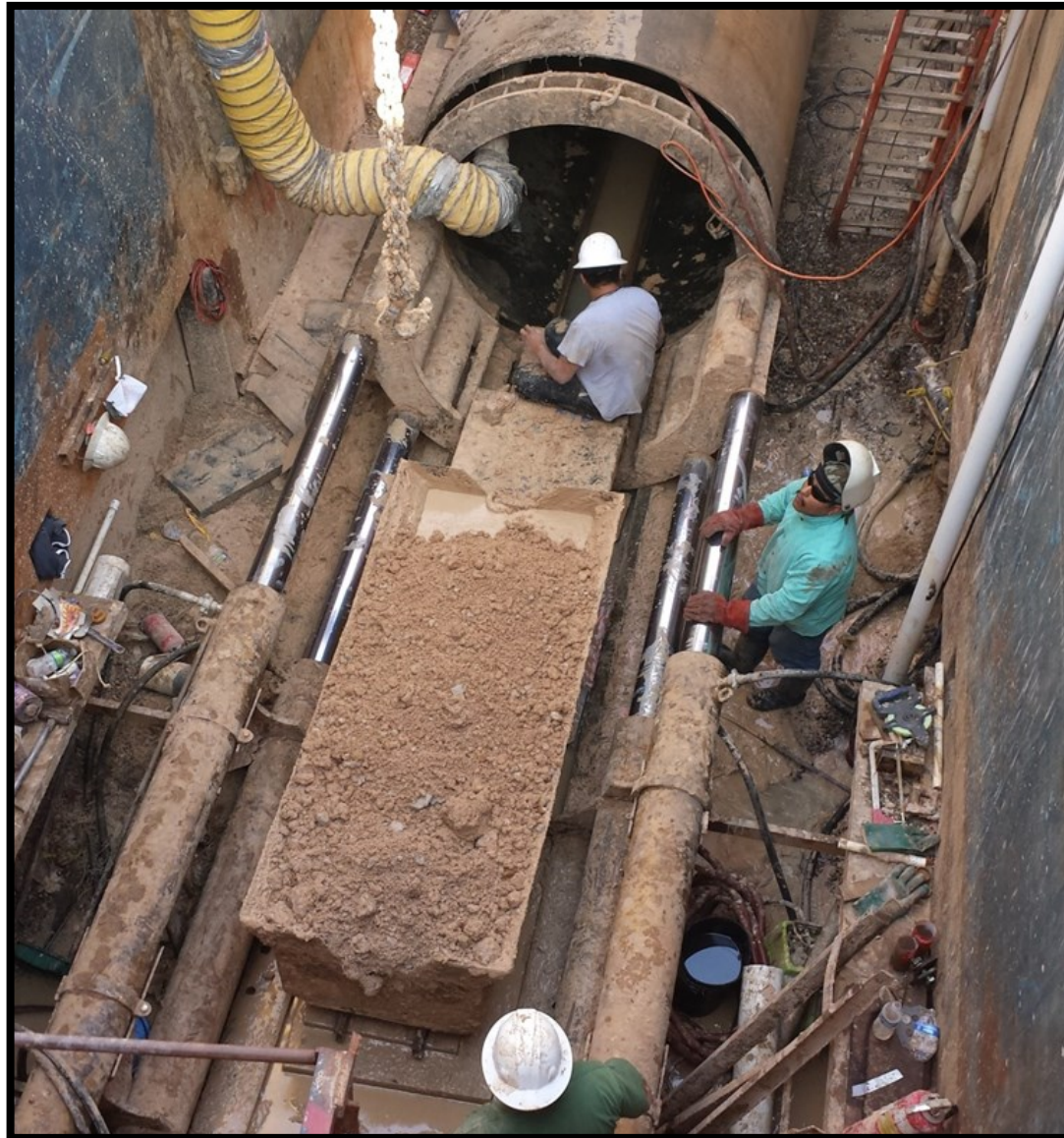
① Segment W1A—Tunnel operation along Research Forest Drive
