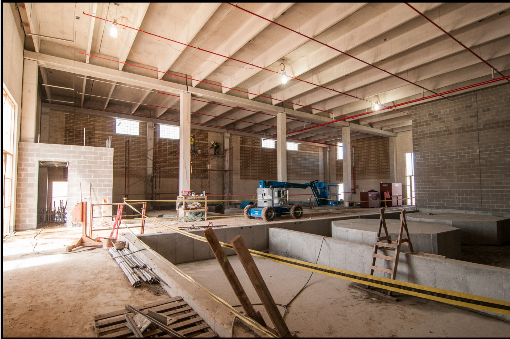
⑦ Interior view of fire suppression system at Chemical Facilities
