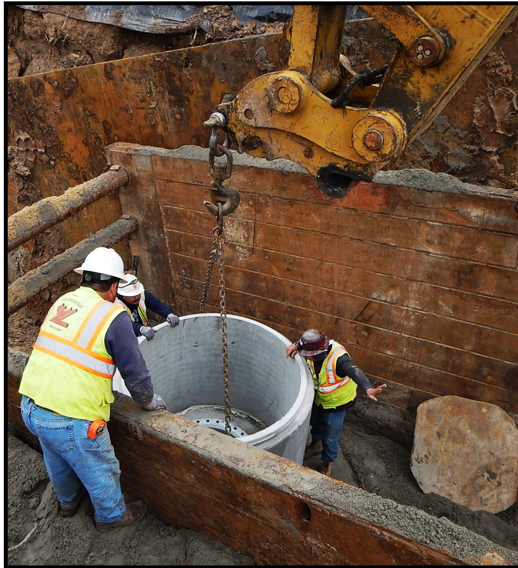
① Segment T1 - Manhole installation along McCaleb Road
