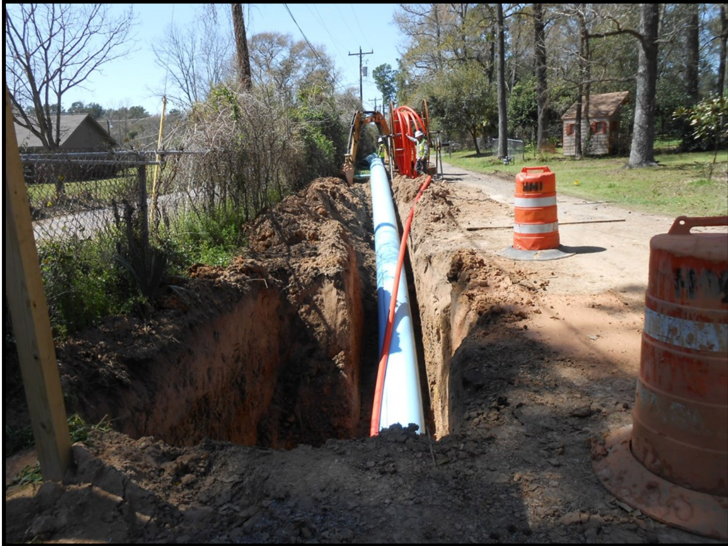
① Segment W4 - Manhole installation and compaction testing along Sun Perch Road
