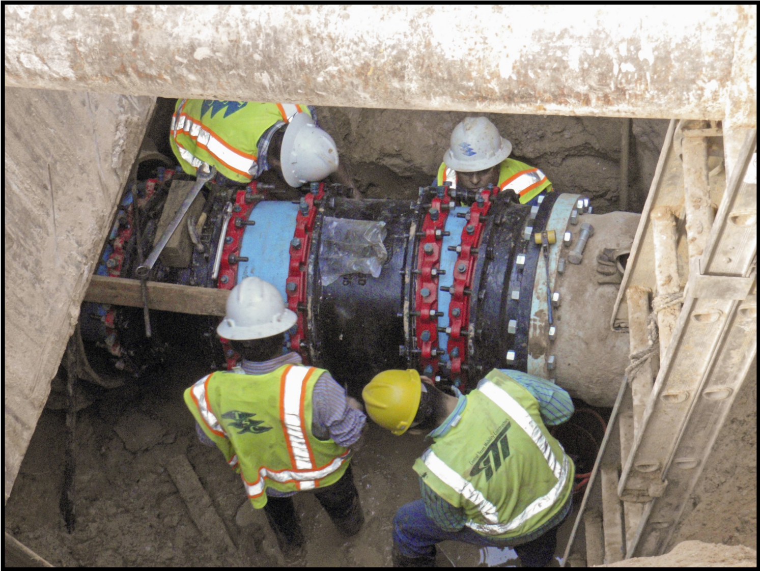
1 Segment W2A - Restrained joint installation along Research Forest Drive
