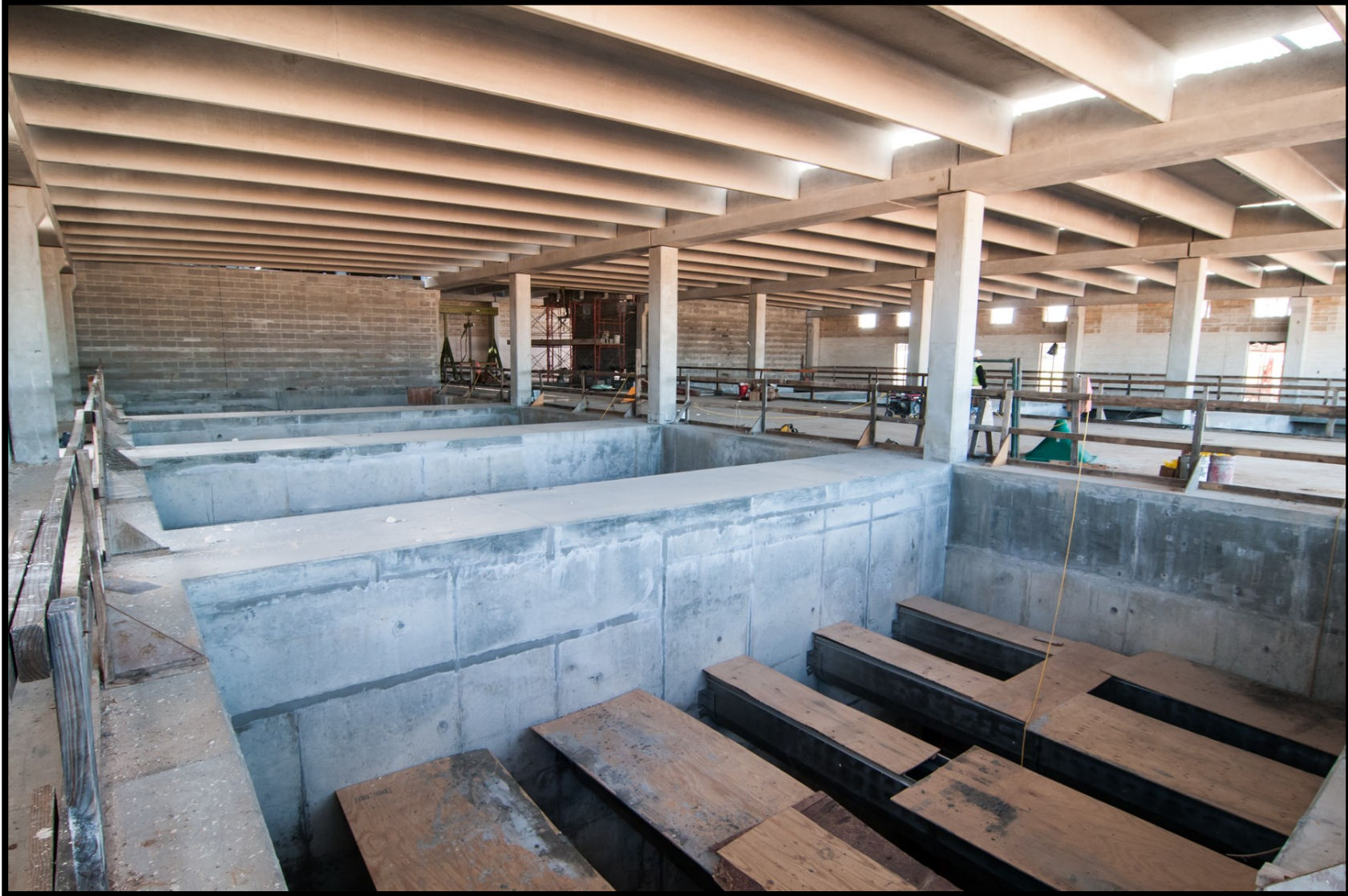
④ Interior view of GAC Building
