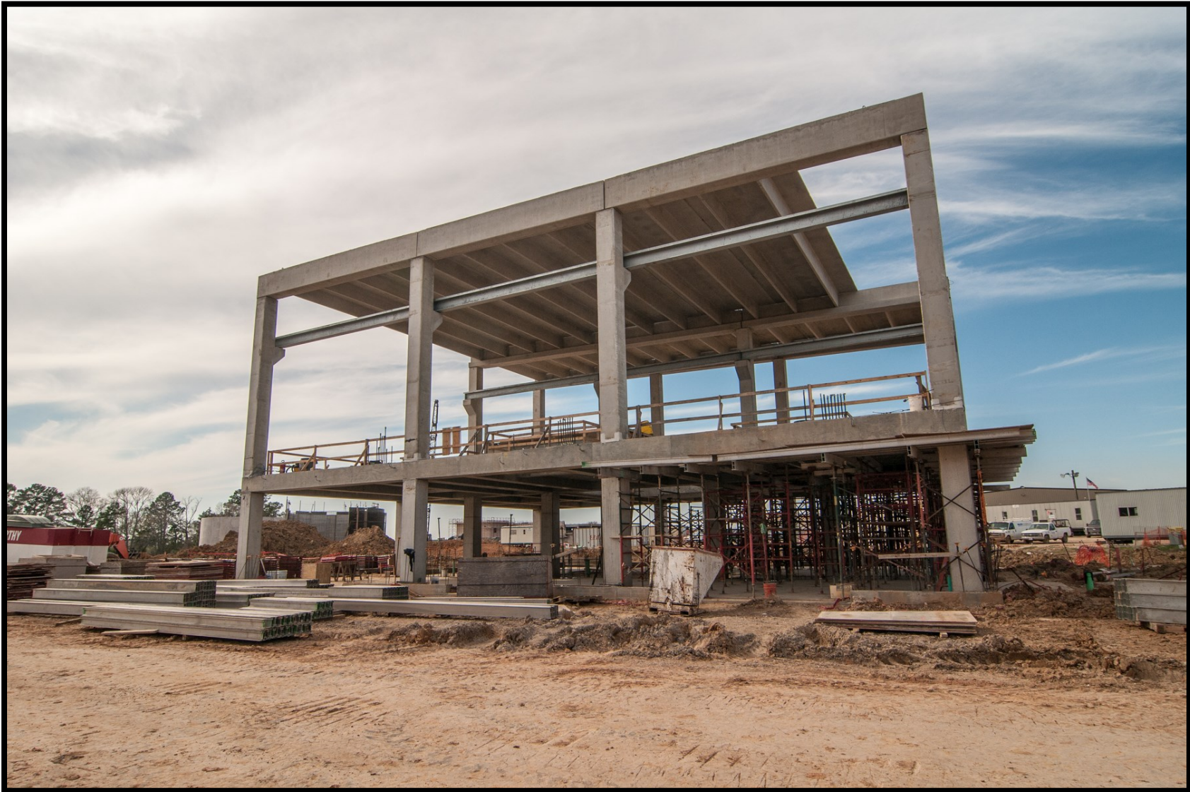
9 Second floor deck installation at Dewatering Building
