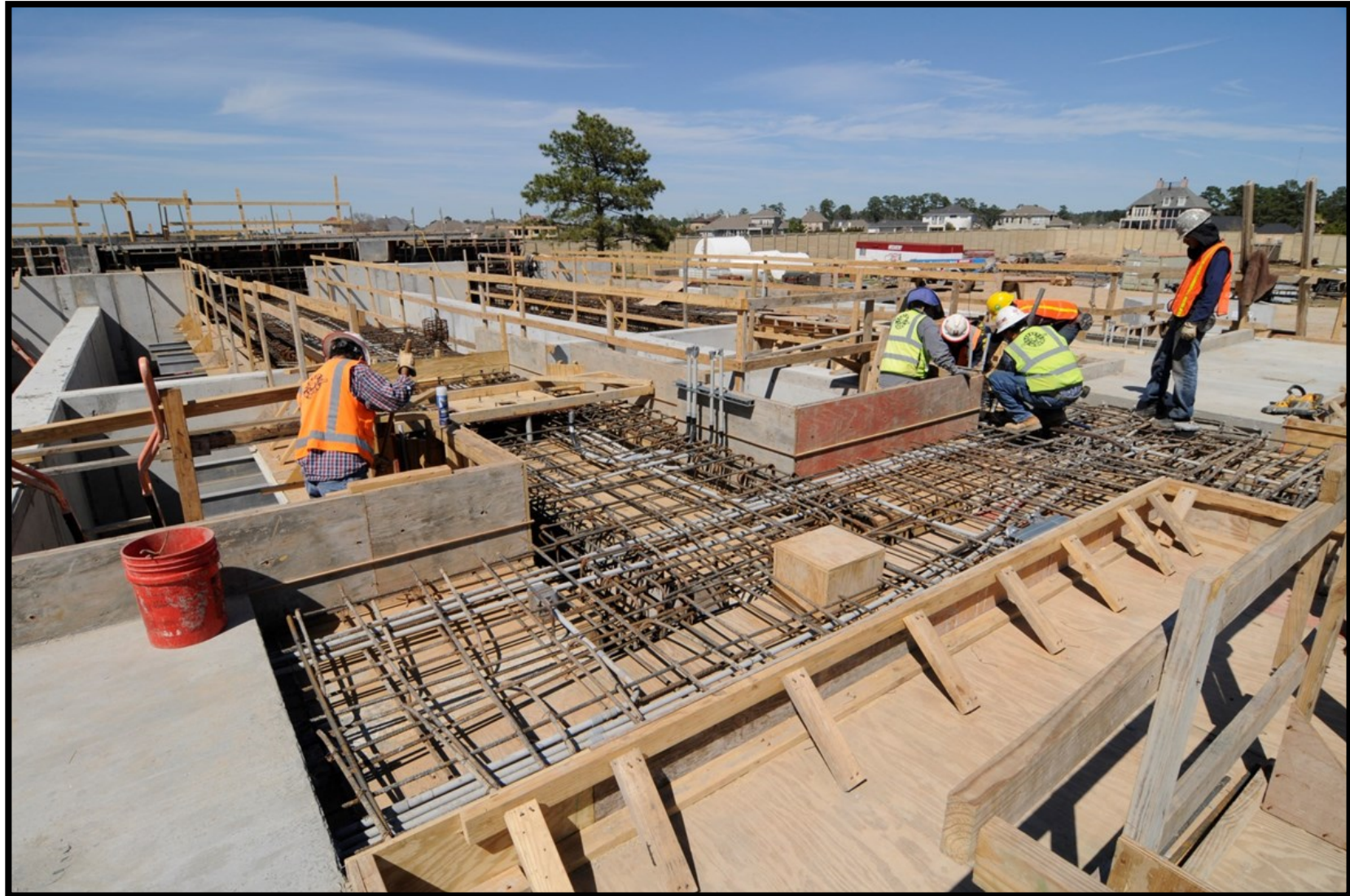
② Access walk way installation at Pretreatment Facility
