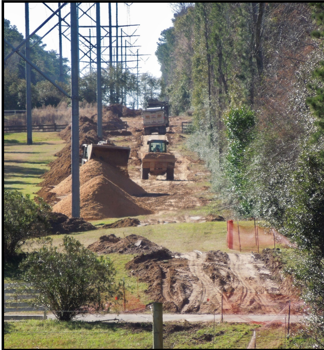
❶ Segment C2—Pipe installation along Entergy easement
