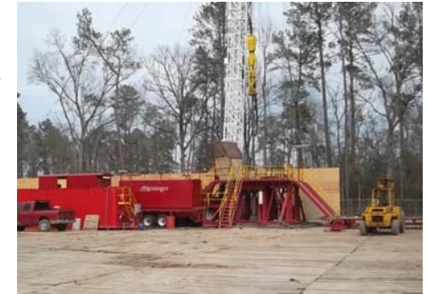
Water Well No. 39 construction
