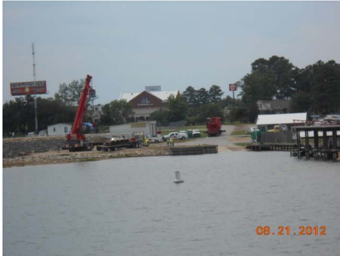
August 21, 2012 – Crane delivery
