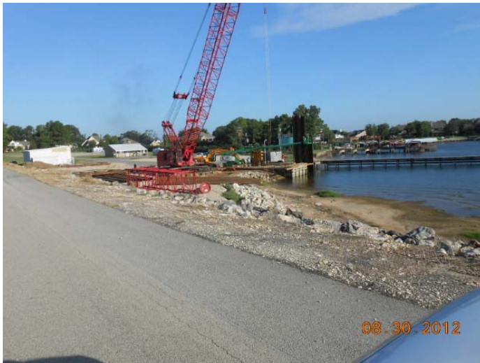
August 30, 2012 – Bulkhead construction @ west end of dam
