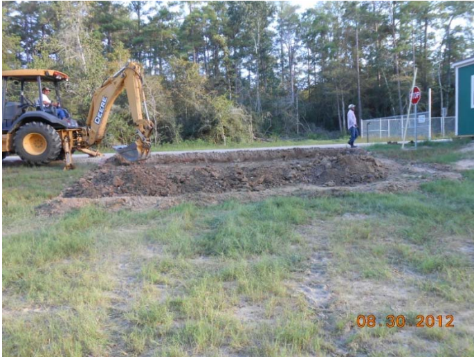
August 30, 2012 – Entrance guard house parking construction
