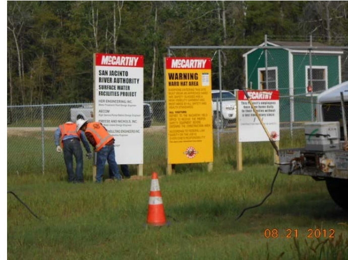
August 21, 2012 – Installation of construction site signs @ SWF site entrance
