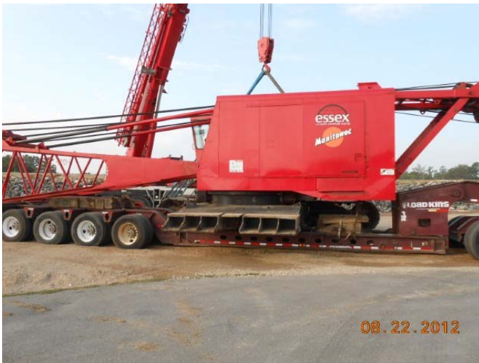
August 22, 2012 – Crane delivery
