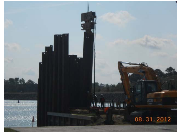
August 30, 2012 – Bulkhead construction @ west end of dam
