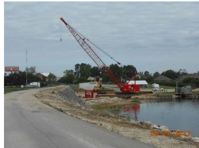
August 27, 2012 – Crane assembly complete
