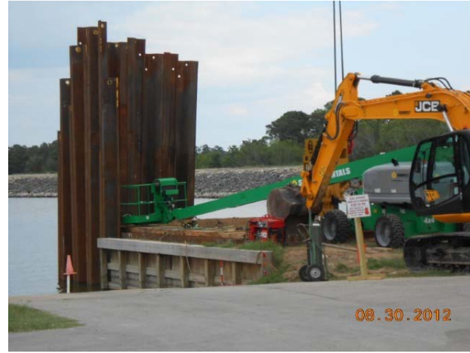
August 30, 2012 – Bulkhead construction @ west end of dam
