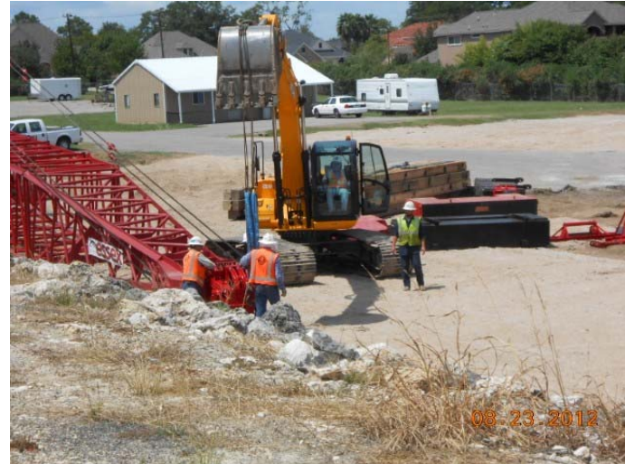
August 23, 2012 – Crane assembly
