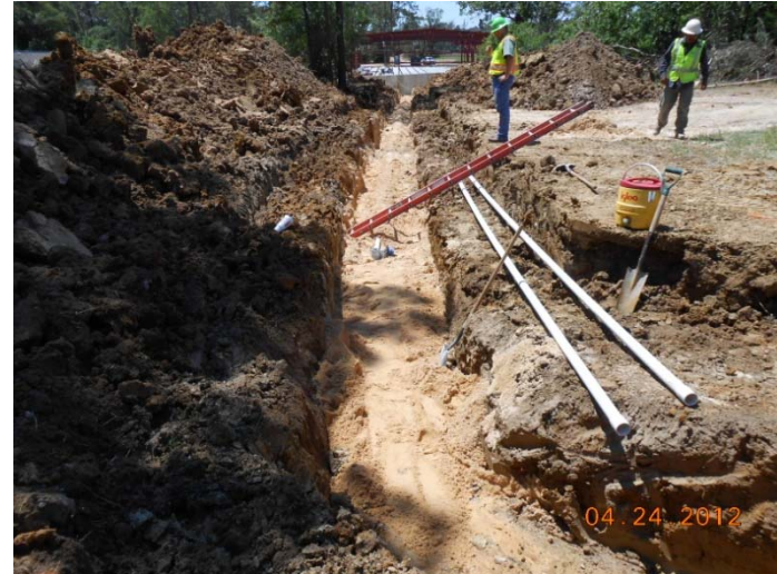
April 24, 2012 – GRP Building No. 1 2-inch waterline installation
