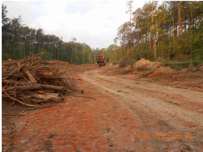
April 3, 2012 – SWF Temporary Access Road clearing
