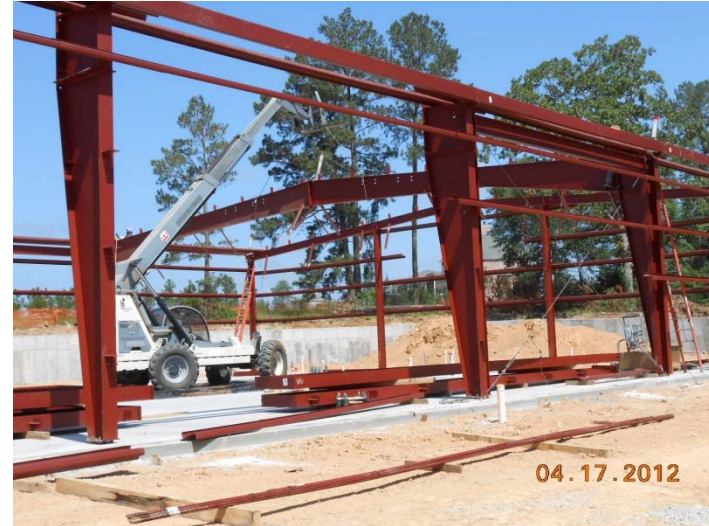
April 13, 2012 – GRP Building No. 1 roof truss installation
