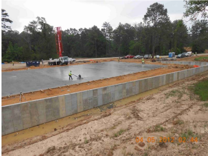
April 5, 2012 – GRP Building No. 1 foundation concrete pour
