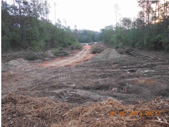
April 3, 2012 – SWF Temporary Access Road clearing
