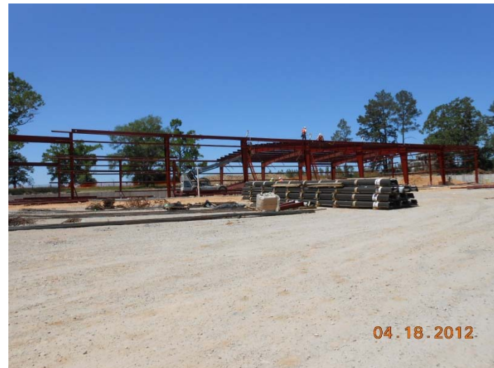
April 18, 2012 - GRP Building No. 1 roof truss and beam installation
