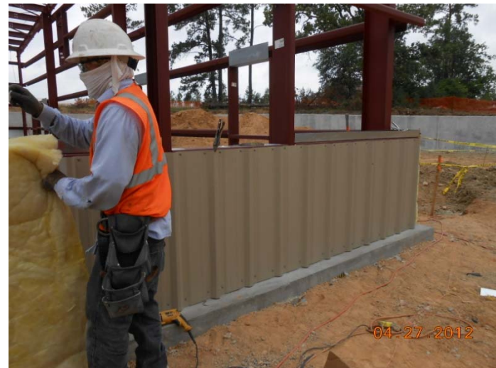
April 27, 2012 – GRP Building No. 1 exterior wall construction
