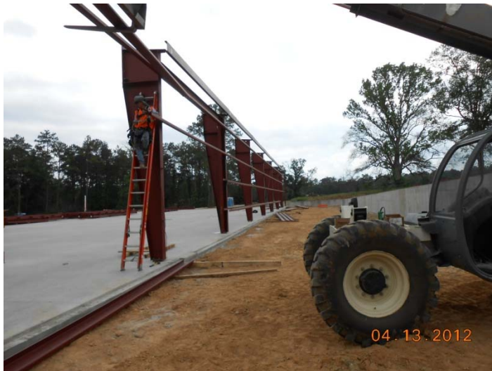
April 13, 2012 – GRP Building No. 1 steel column and beam erection
