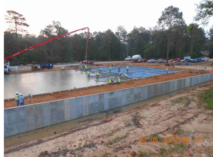
April 5, 2012 – GRP Building No. 1 foundation concrete pour
