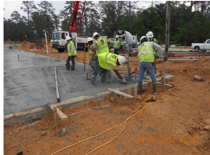
April 5, 2012 – GRP Building No. 1 foundation concrete pour
