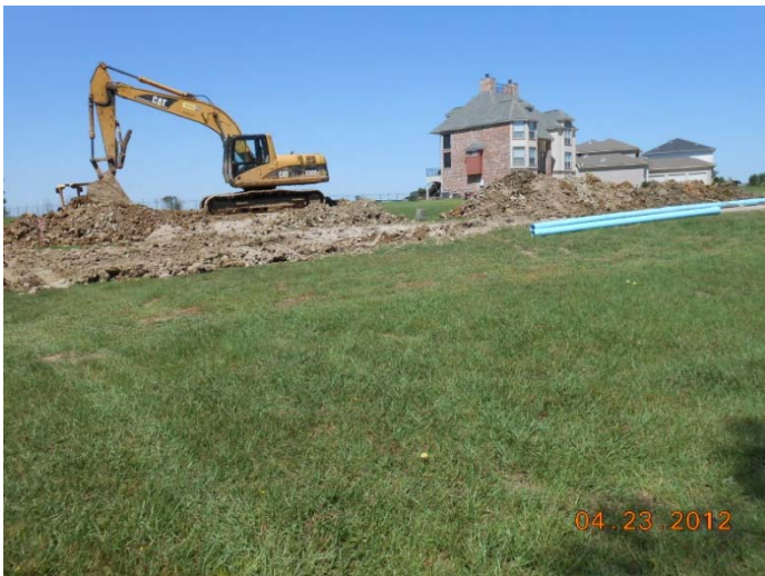
April 23, 2012 – GRP Building No. 1 6-inch waterline installation
