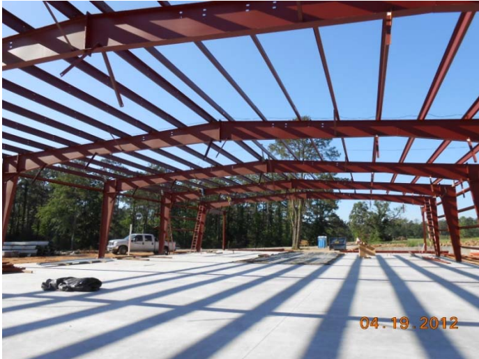
April 19, 2012 – GRP Building No. 1 roof trusses and beams
