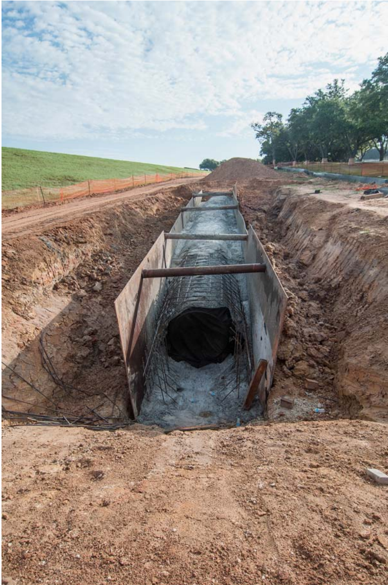
2 Segment T1 Section Below Dam Showing 60-inch Pipe Concrete Encasement
