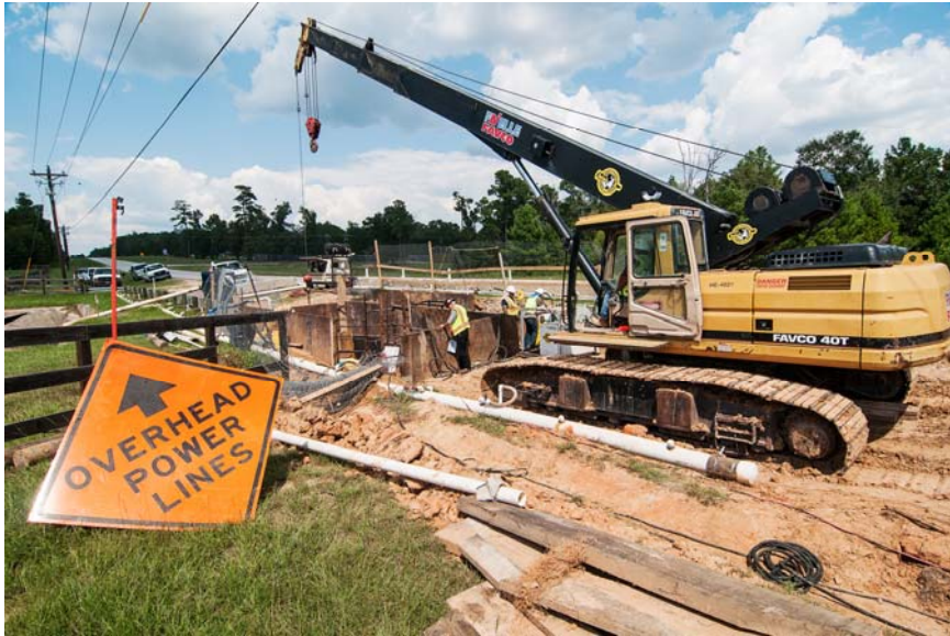
② Tunnel Pit Installation near Overhead Power Lines
