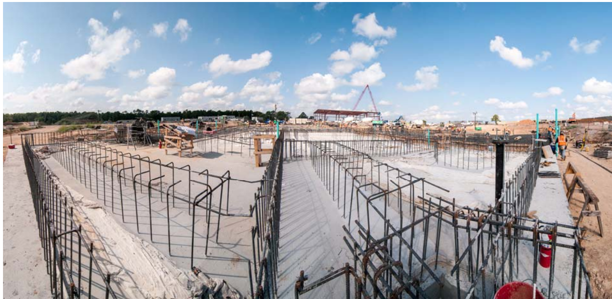
16 17 18 Conduit and Rebar Installation at Chemical Facilities
