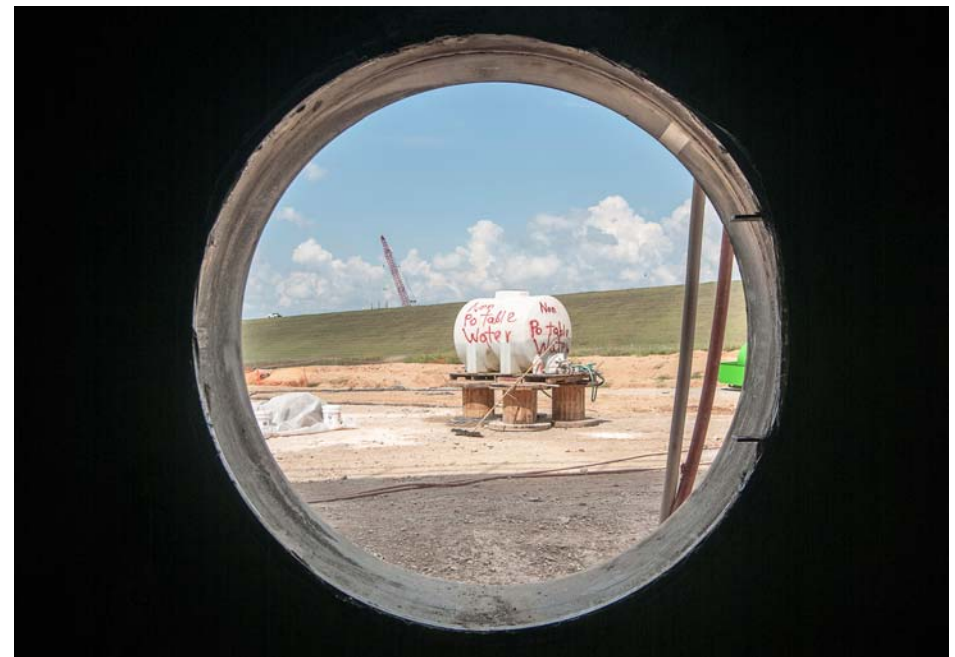
Surface Water Facilities—View from the Inside of the Ground Storage Tank
