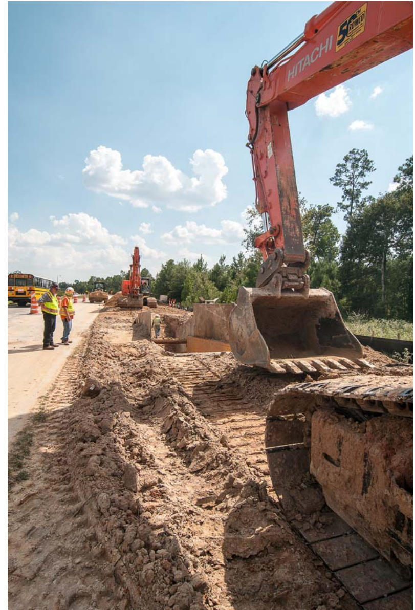
789 60-inch Pipe Installation Along Fish Creek Thoroughfare
