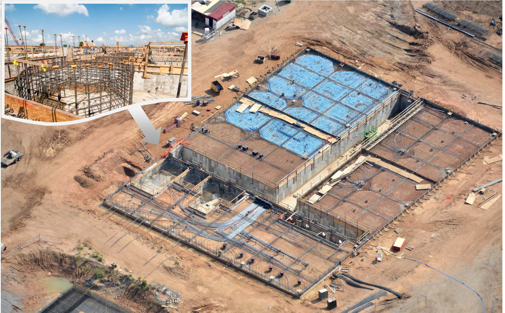
⑩ Backfilling and Initial Wall Installation at Membrane Facilities; Inset Shows Foundation for Future Chemical Tank
