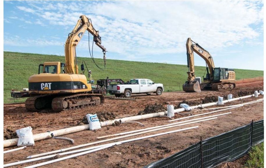
3 Segment T1 Dewatering System Installation
