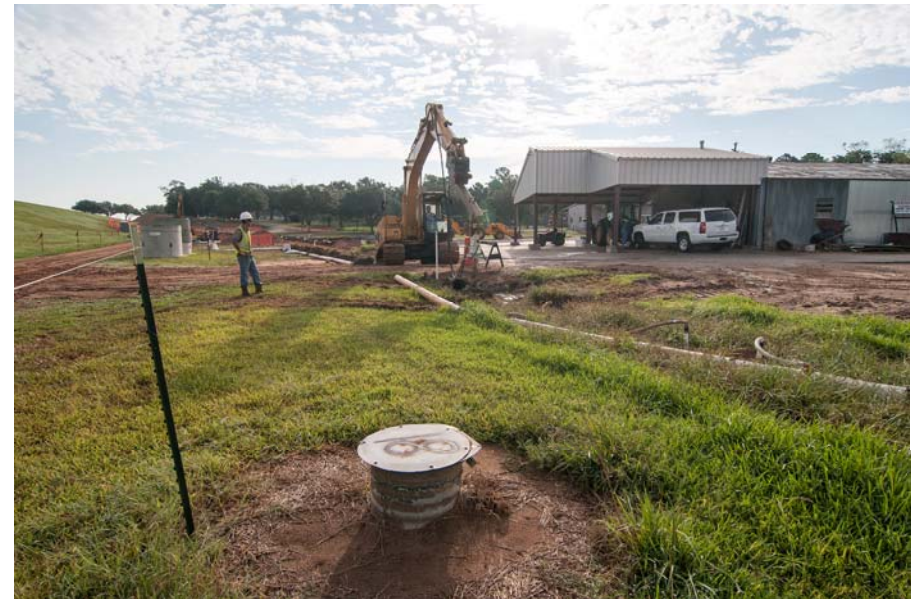
4 Segment T1 Dewatering Operation
