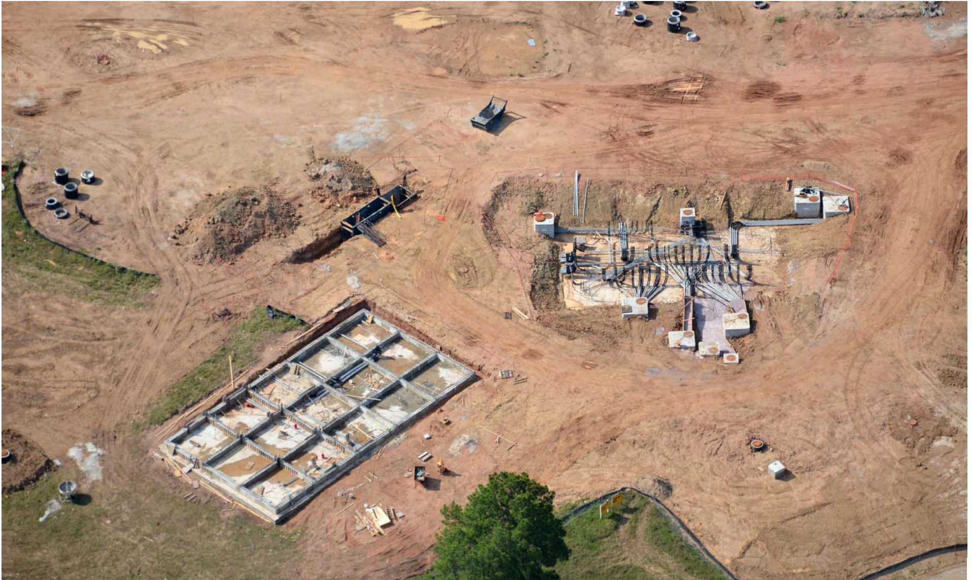
14 15 Aerial View of Generator and Switchgear Building Foundations
