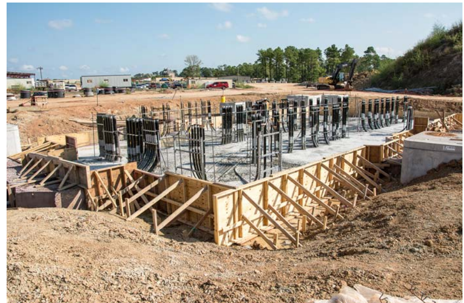
15 Conduit Installation at Electrical Switchgear Building
