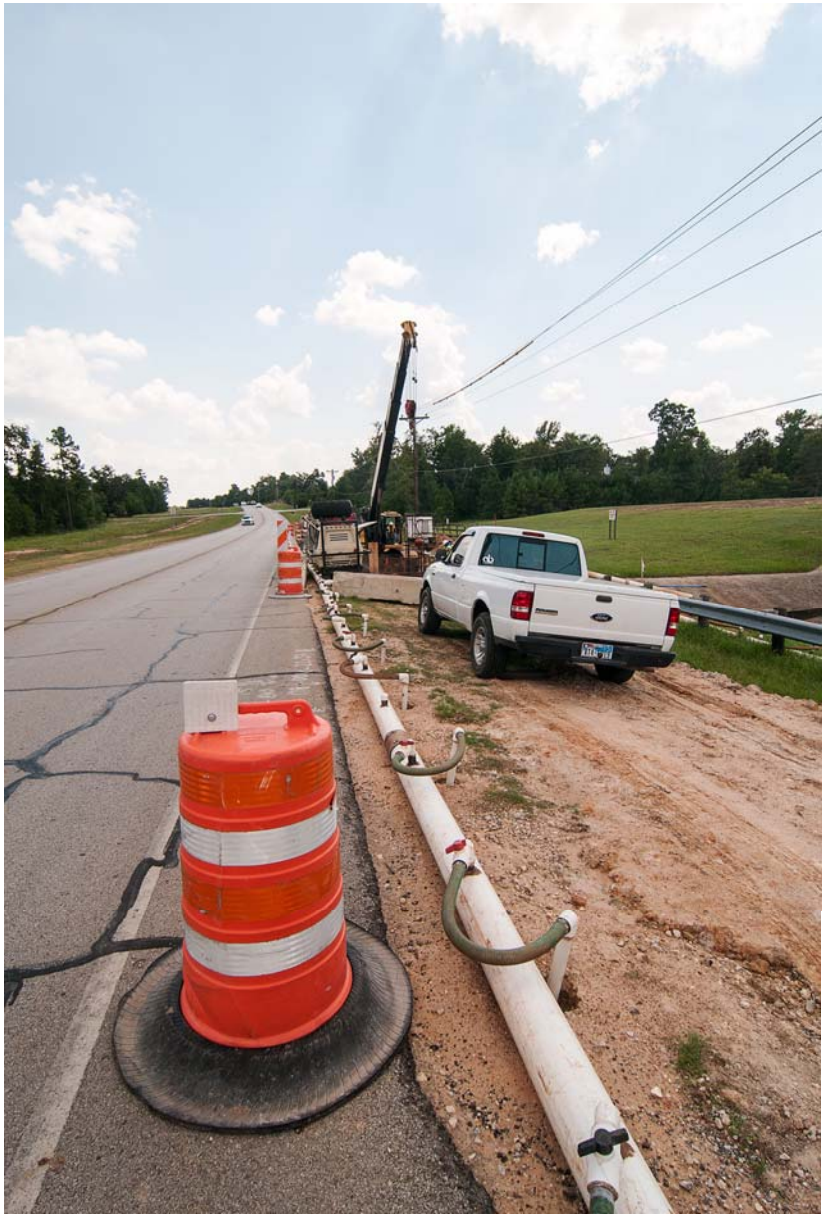
1 Groundwater Dewatering Along Segment T2
