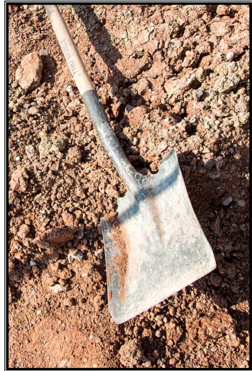
Surface Water Facilities - Construction Site
