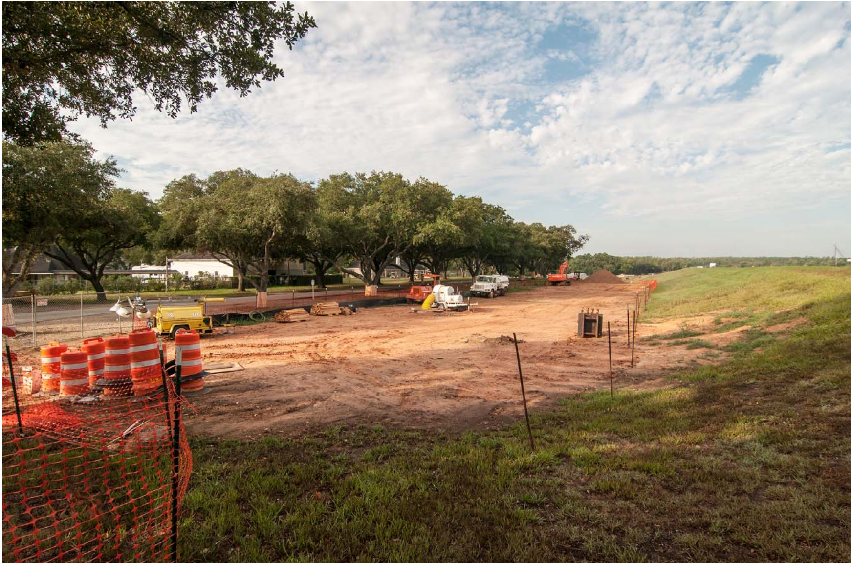
① Completed Segment T1 Pipe Installation at G&A Building
