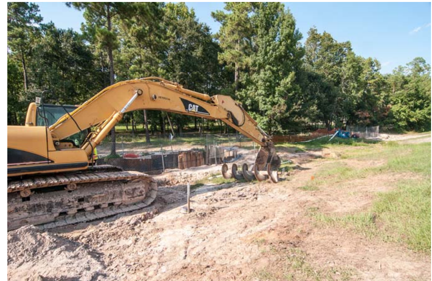
③ Segment W1B Installation of Tunnel Shaft for Boring Under Creek Along Alden Bridge
