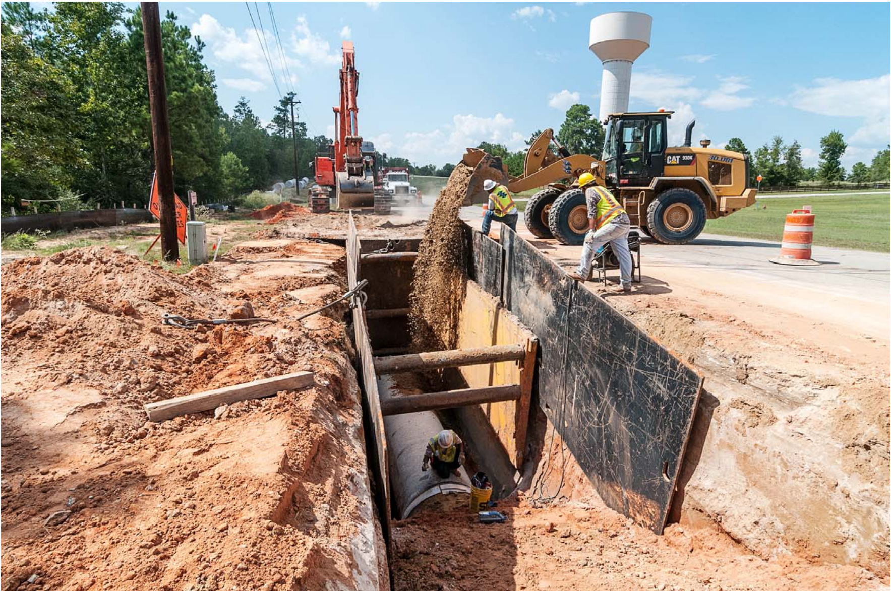
⑥ 60-inch Pipe Installed by Open Cut Construction Along Fish Creek Thoroughfare
