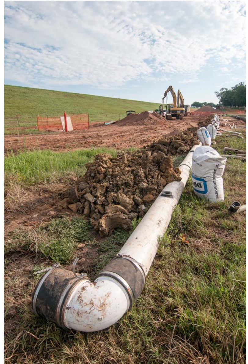
Segment T1 - Well Point Installation
