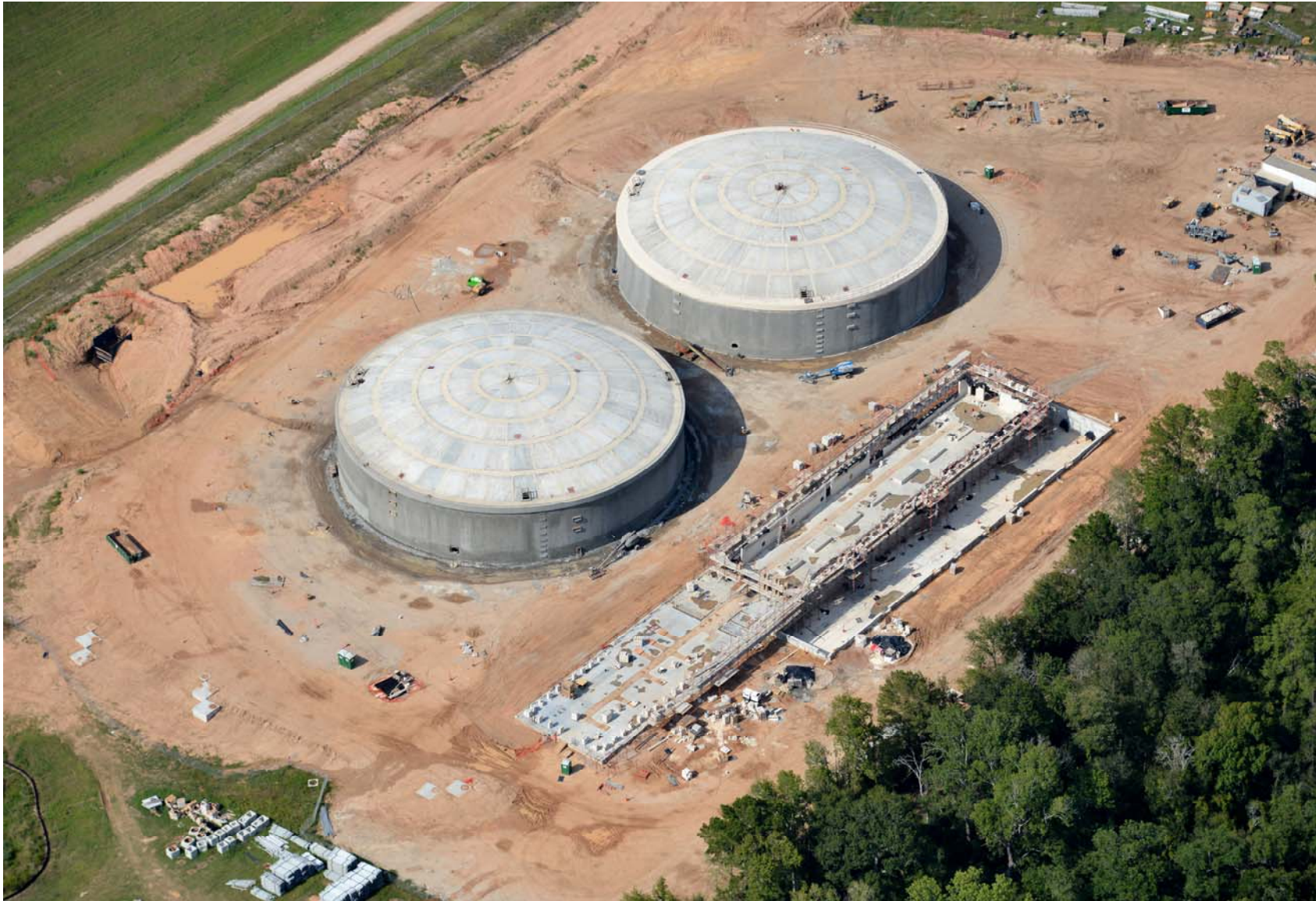
7 8 9 10 Aerial View of Ground Storage Tanks And High Service Pump Station
