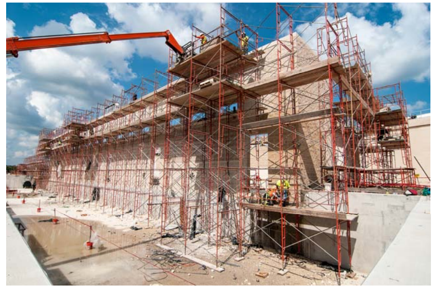
10 High Service Pump Station - Scaffolding and Building Masonry Work
