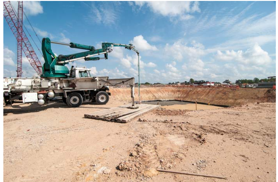
13 Seal Slab Installation at Equalization Basin
