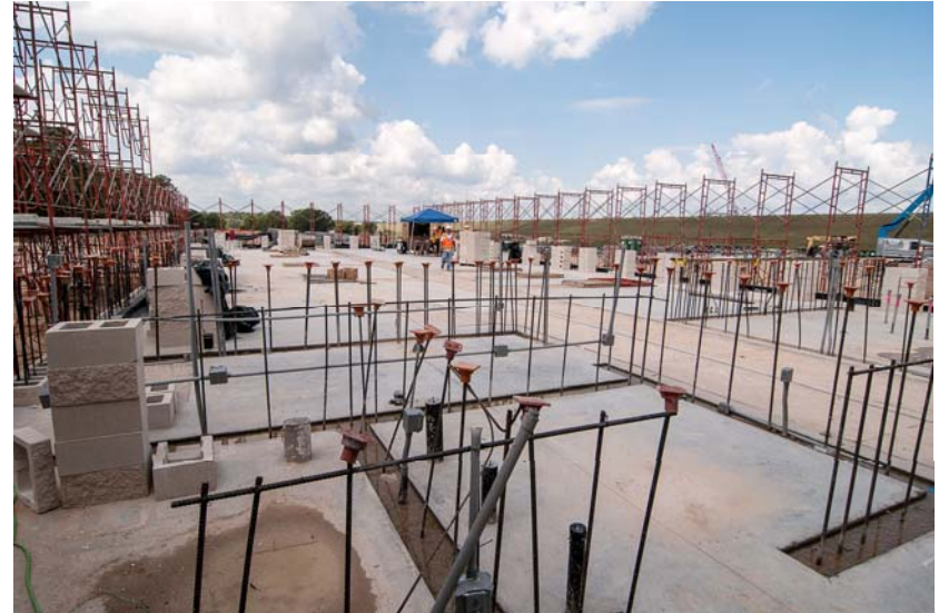
9 High Service Pump Station - Electrical Room
