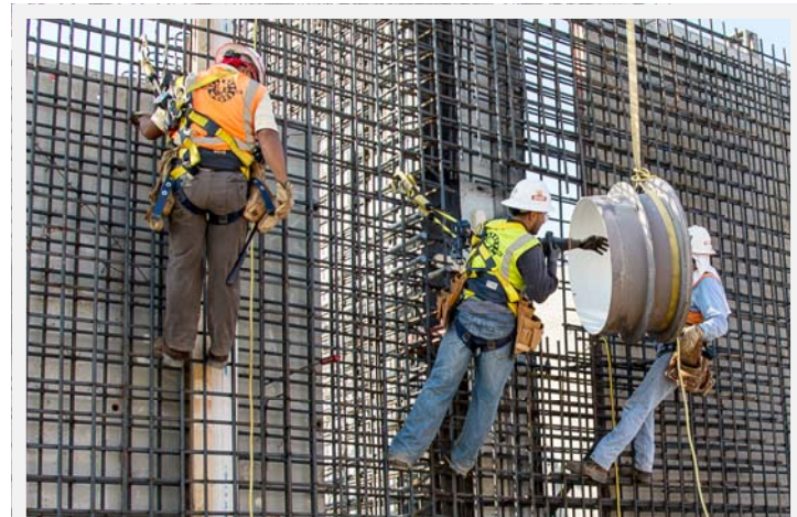
Below, Rebar Installation at GAC Building
