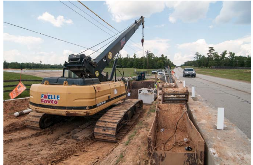
③ Construction Proximity to Traffic Along Fish Creek Thoroughfare
