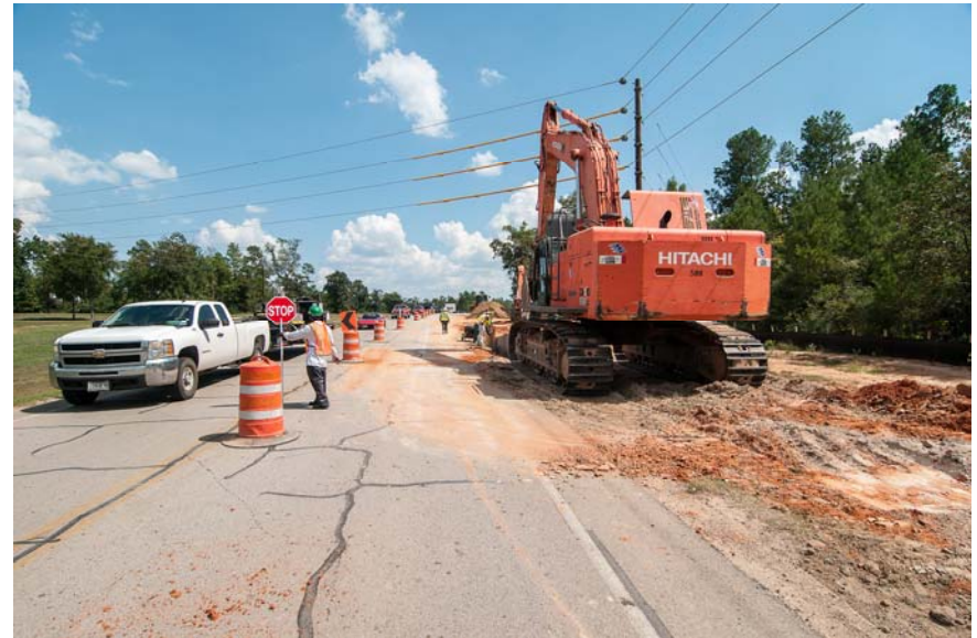
⑤ Workers Divert Traffic Along Fish Creek Thoroughfare
