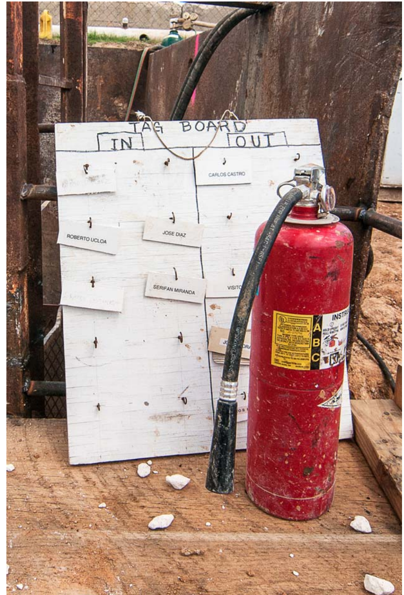
Safety Precautions - Worker Sign In/Sign out for Tunnel Pit Entry and Fire Extinguisher
