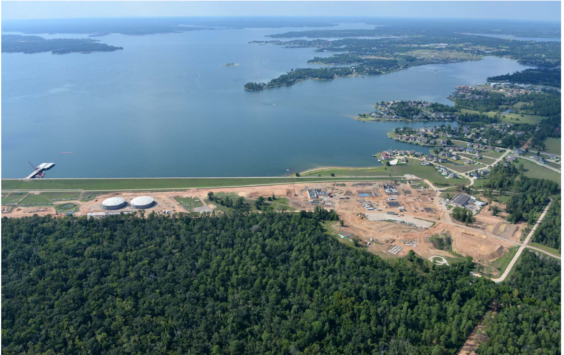
Overall Aerial View of Surface Water Plant Site - August 23, 2013
