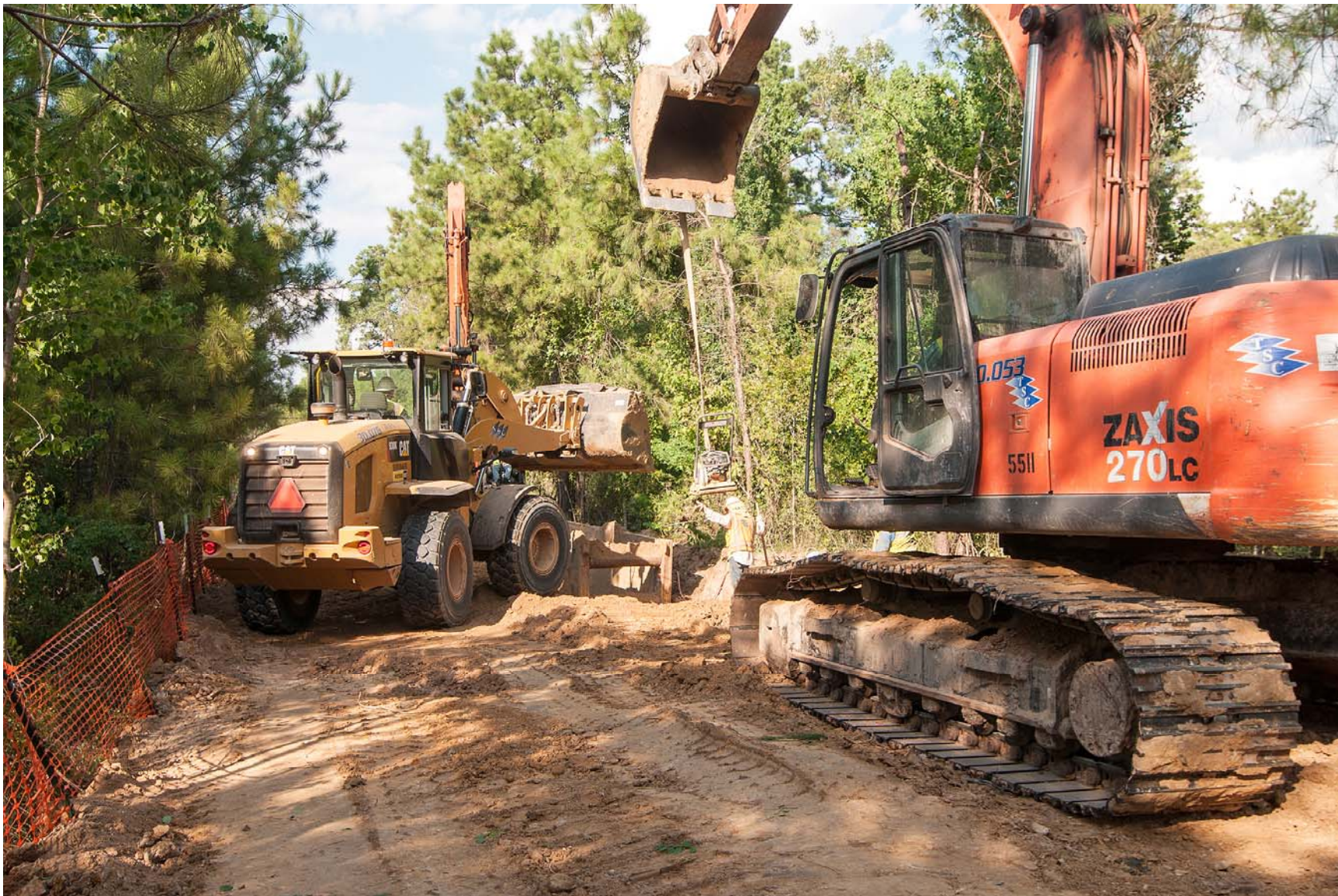
④ Segment W1B Narrow Construction within Easement along Kuykendahl
