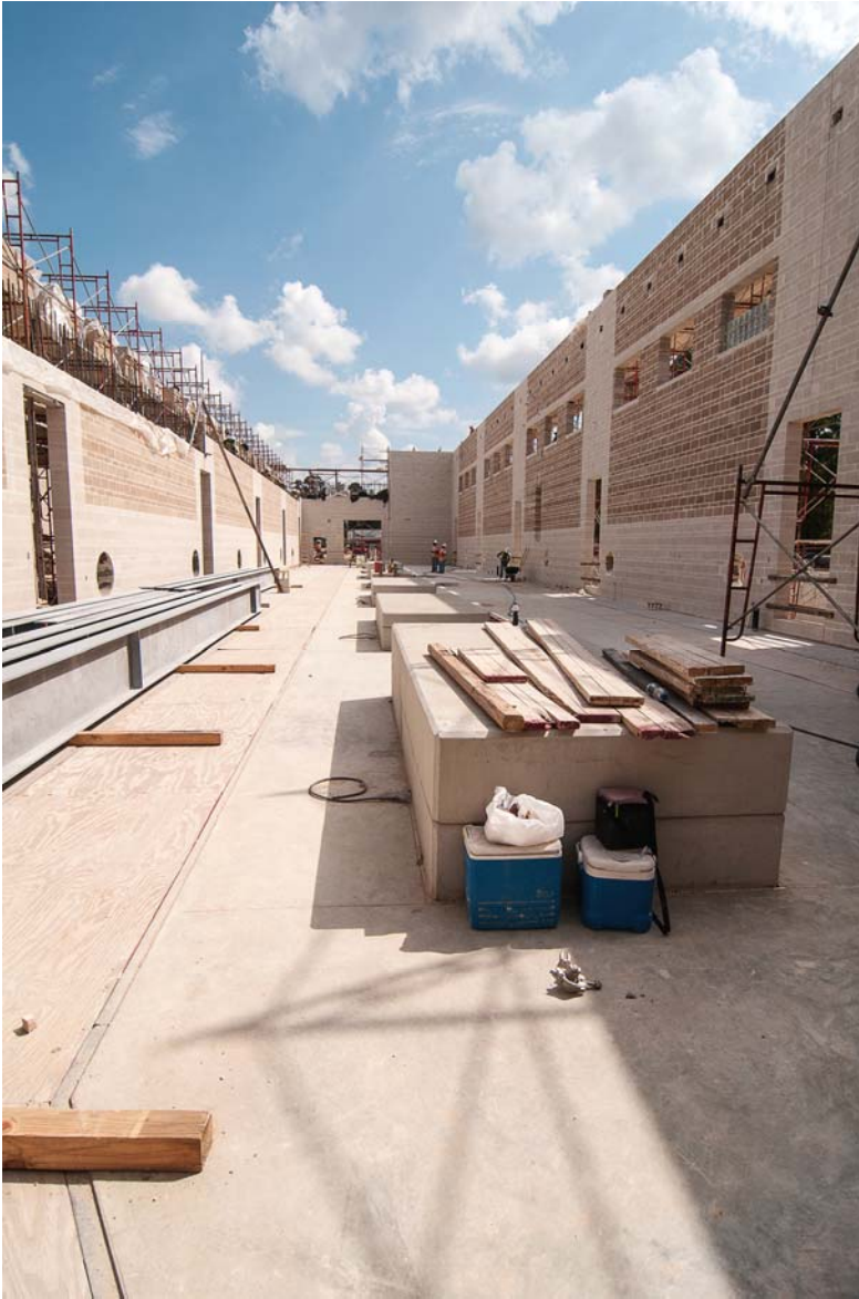
8 High Service Pump Station - Inside the Pump Room
