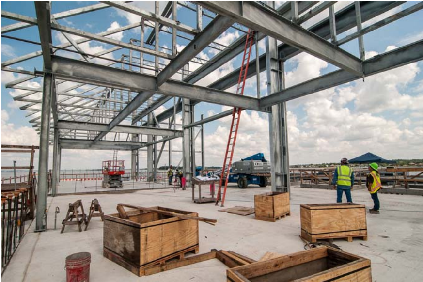
①②③④ Building Steel Erection Begins at Raw Water Pump Station
