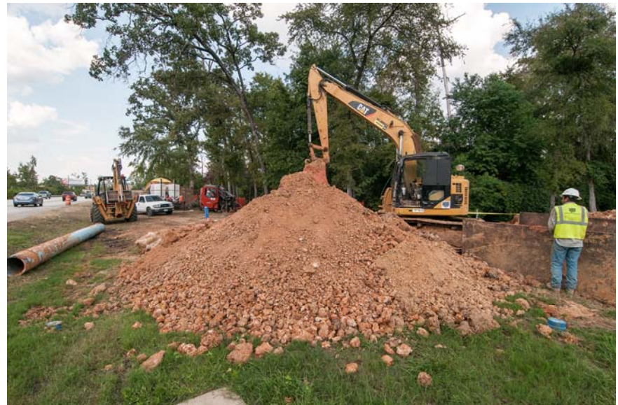
① ② ③ Segment W1A Along FM 2978 - Trenchless Construction of 16-inch Waterline
