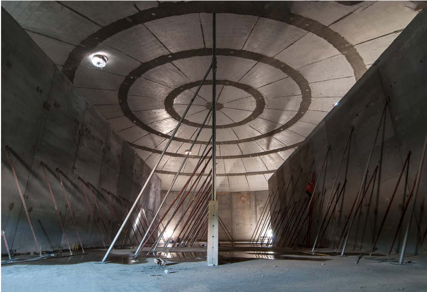
⑥ Inside Ground Storage Tank No. 2 Showing Baffle Walls and Supports
