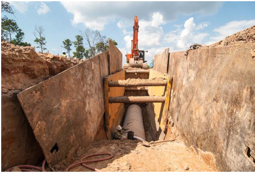
789 60-inch Pipe Installation Along Fish Creek Thoroughfare
