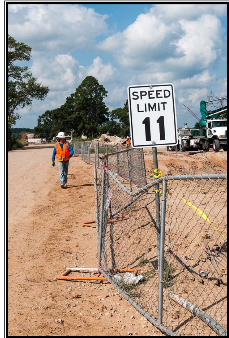
Surface Water Facilities—Speed Limit Sign
