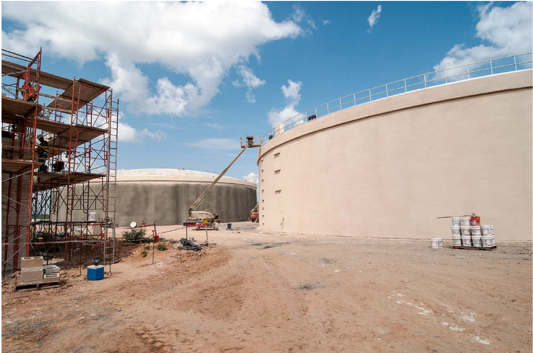
① Ground Storage Tank Nos. 1 and 2 - Exterior Coating Near Completion on Ground Storage Tank No. 2
