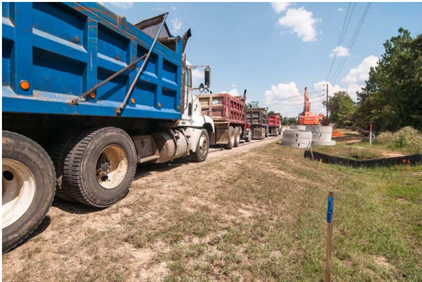
④ Dump Trucks Wait to Remove Spoils from Open-cut Construction
