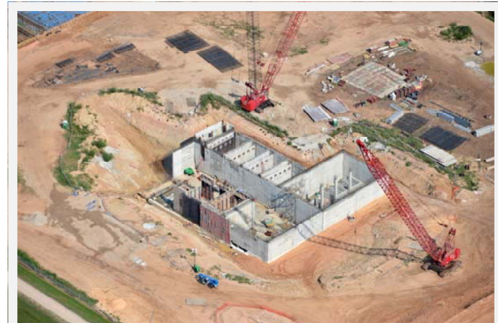
Above, Aerial View of the GAC Building
