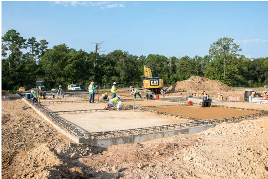
14 Installation of the Generator Building
