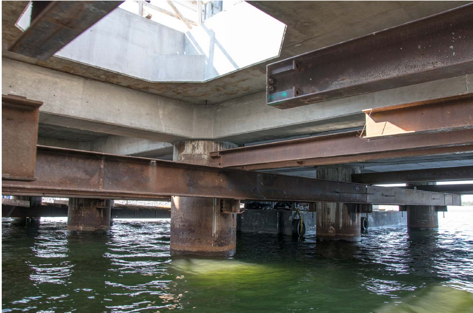
⑤ Raw Water Pump Station - Steel Supports Used for Deck Construction (to be removed) and Deck Opening for Future Pump
