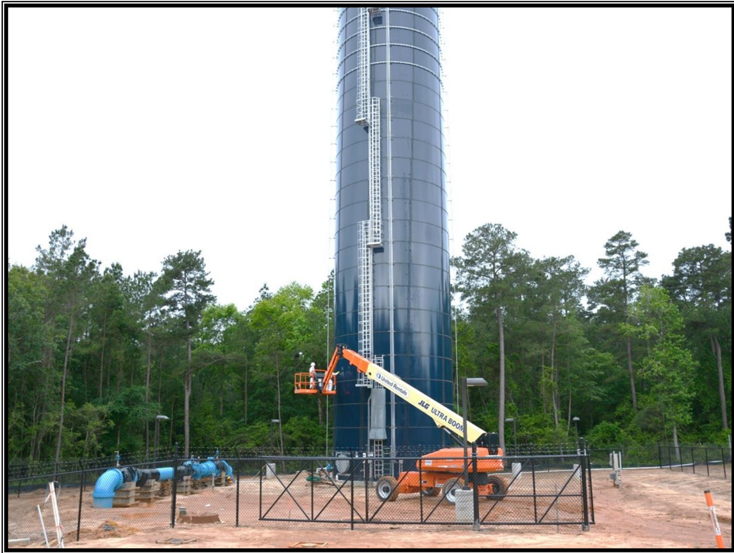
① Exterior cleaning of the Standpipe
