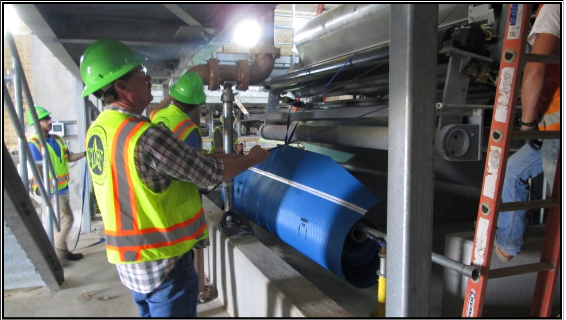
② Dewatering Building—Operations and maintenance staff installing belts during training
