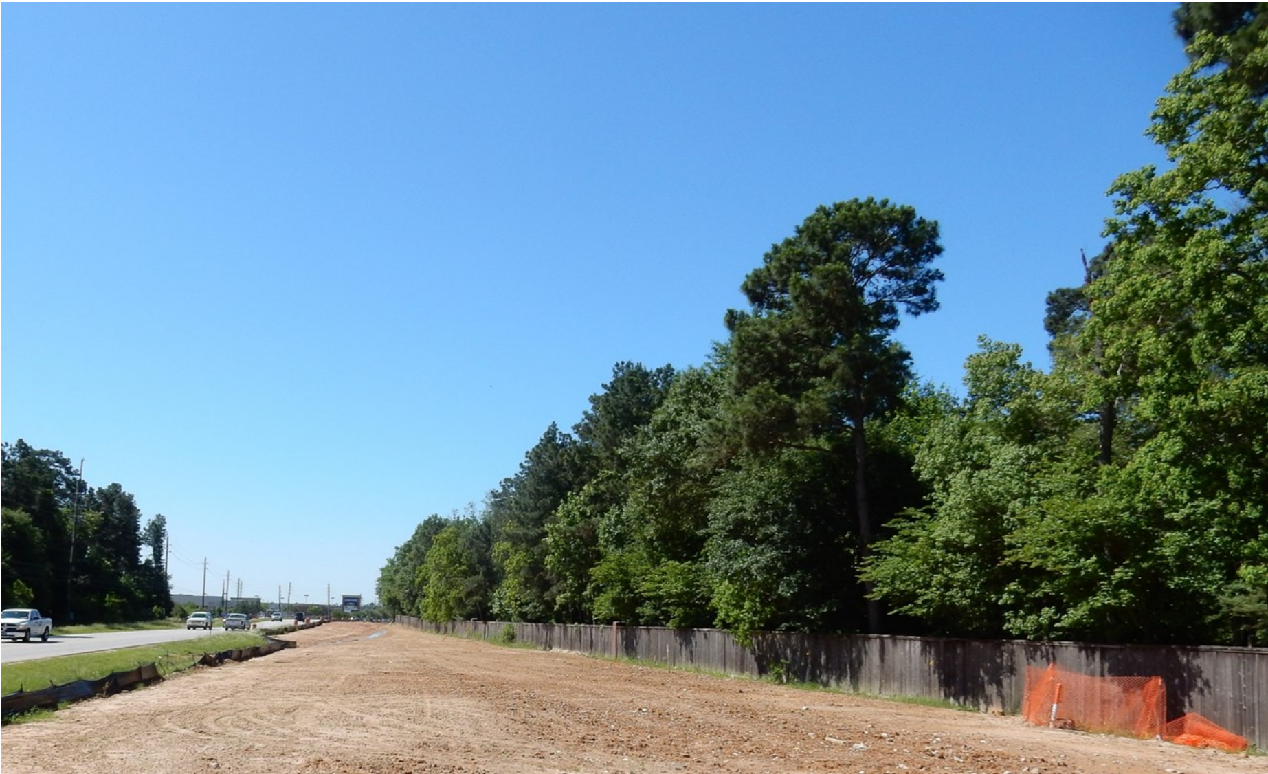
① Site restoration along Sendera Ranch Road north of FM 1488
