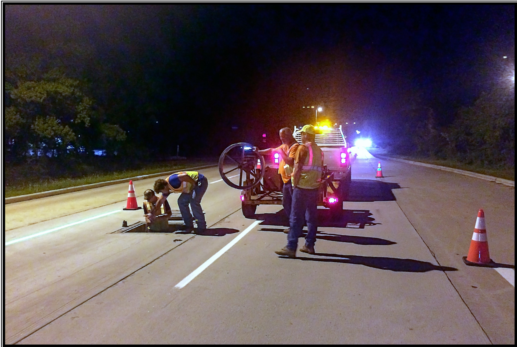
Night time installation of fiber optic cable along Research Forest Drive
