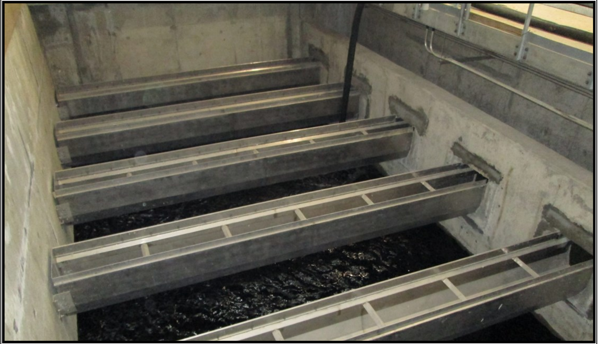
① Granulated Activated Carbon (GAC) Building—Installation of GAC material into contactor basin
