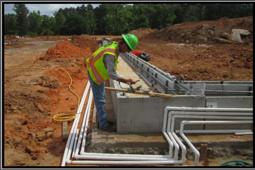
Worker inspecting chemical trench piping at the Surface Water Treatment Facility
