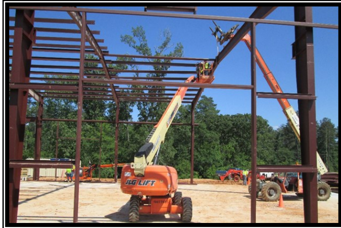
Crews erecting steel beams at the Maintenance Building
