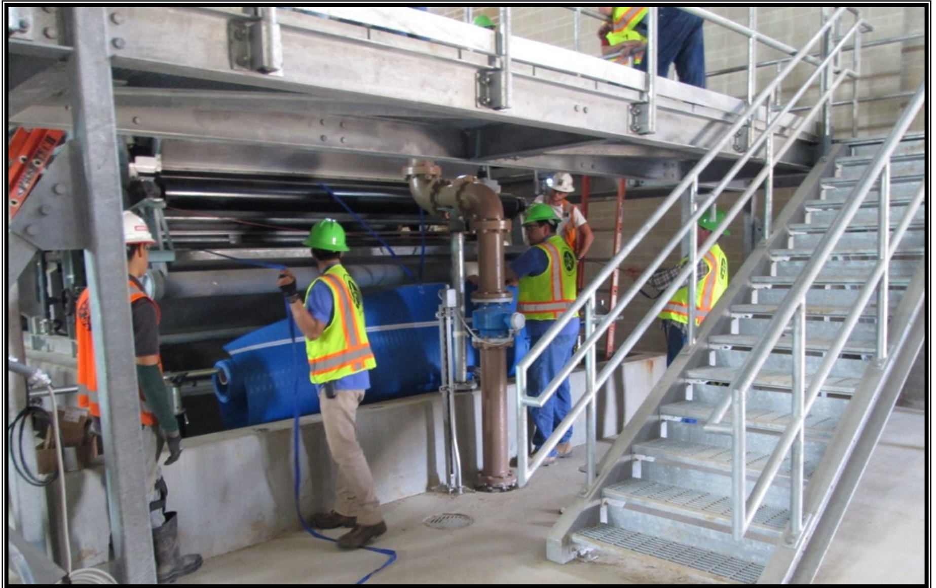
② Dewatering Building—Operations and maintenance staff installing belts during training
