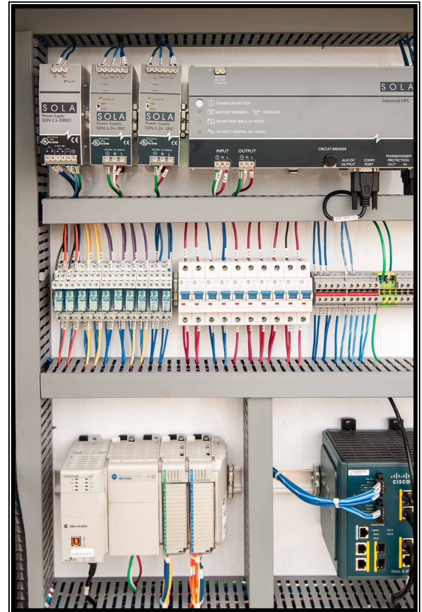
Control panel for the sludge system located in the Pretreatment Facility
