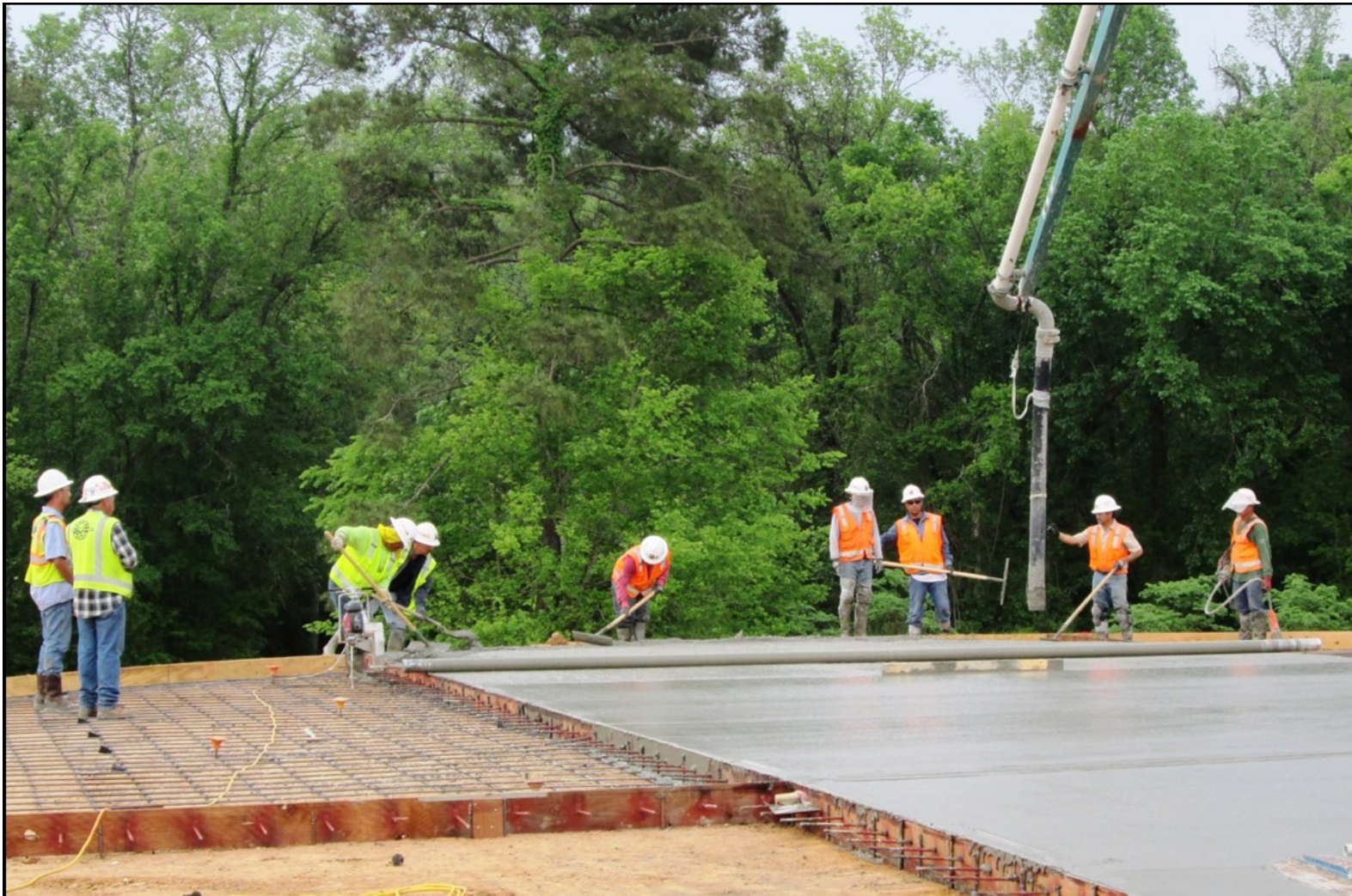
General Site—Form work, reinforcing steel, and concrete placement
