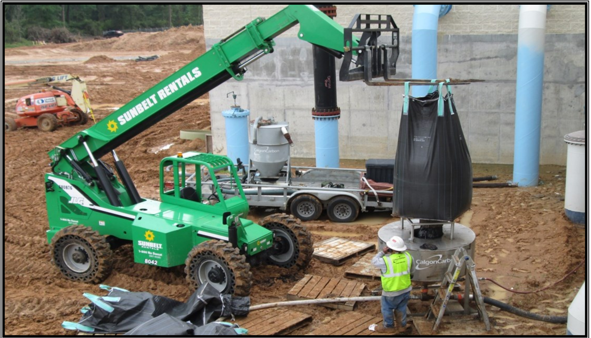
❶ Granulated Activated Carbon Building—Eductor system installation of GAC media
