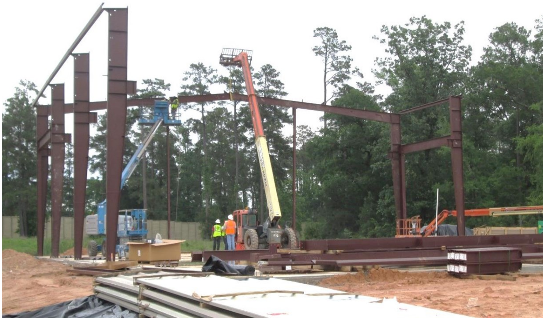
③ Maintenance Building—Erection of structural steel framing system
