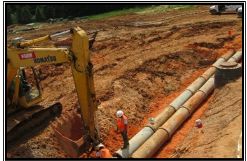
Workers installing twin storm sewer pipe west of the Surface Water Facility
