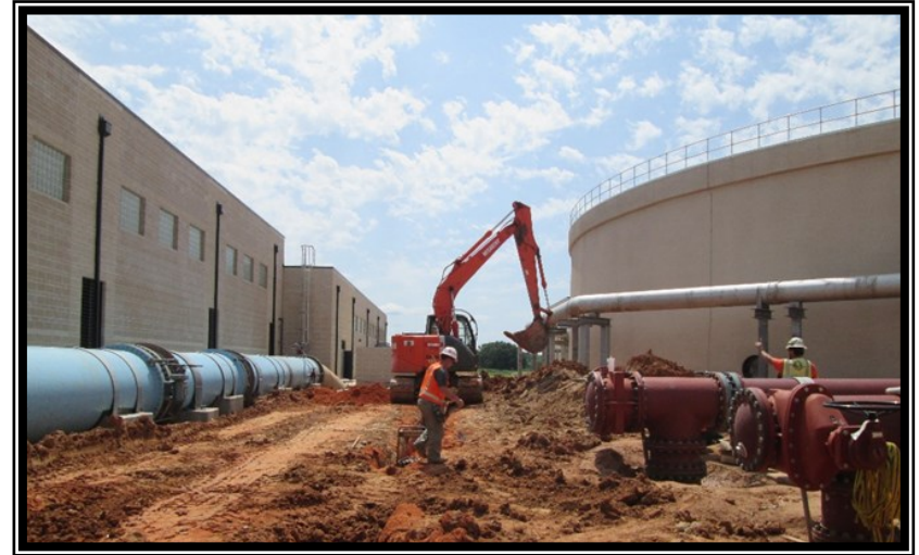
Workers installing sample lines at the High Service Pump Station
