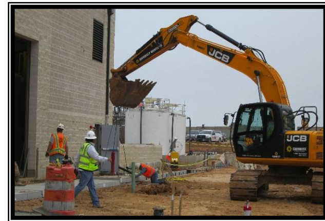
Workers installing chemical trench covers at the Chemical Building
