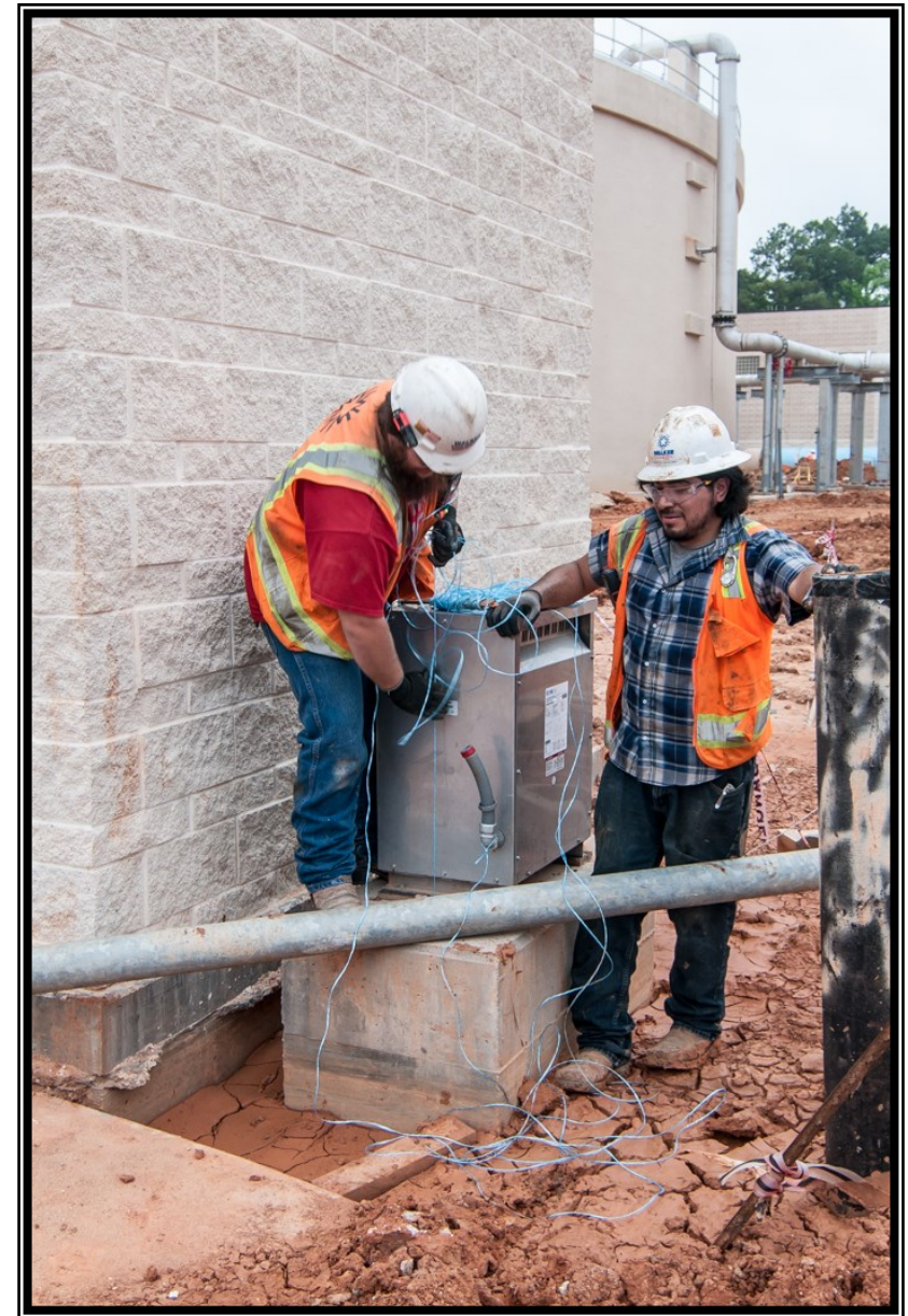
Left—Belt filter press at the Solids Dewatering Building Above—Workers pulling wire at the Sample Building
