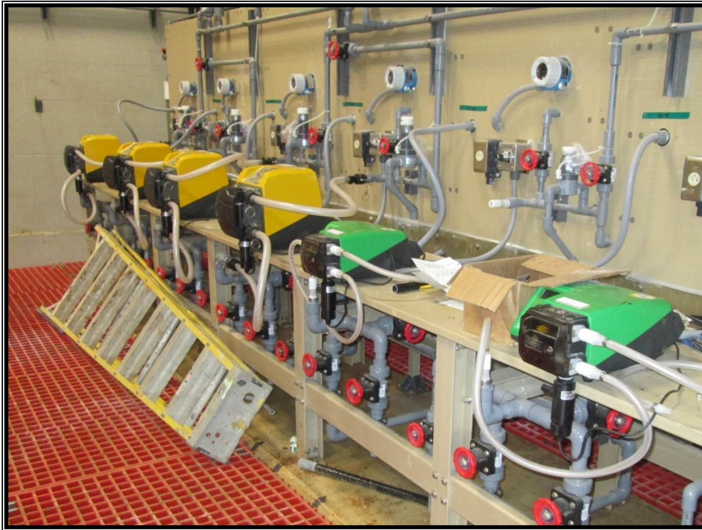
④ Chemical Building — Chemical metering station
