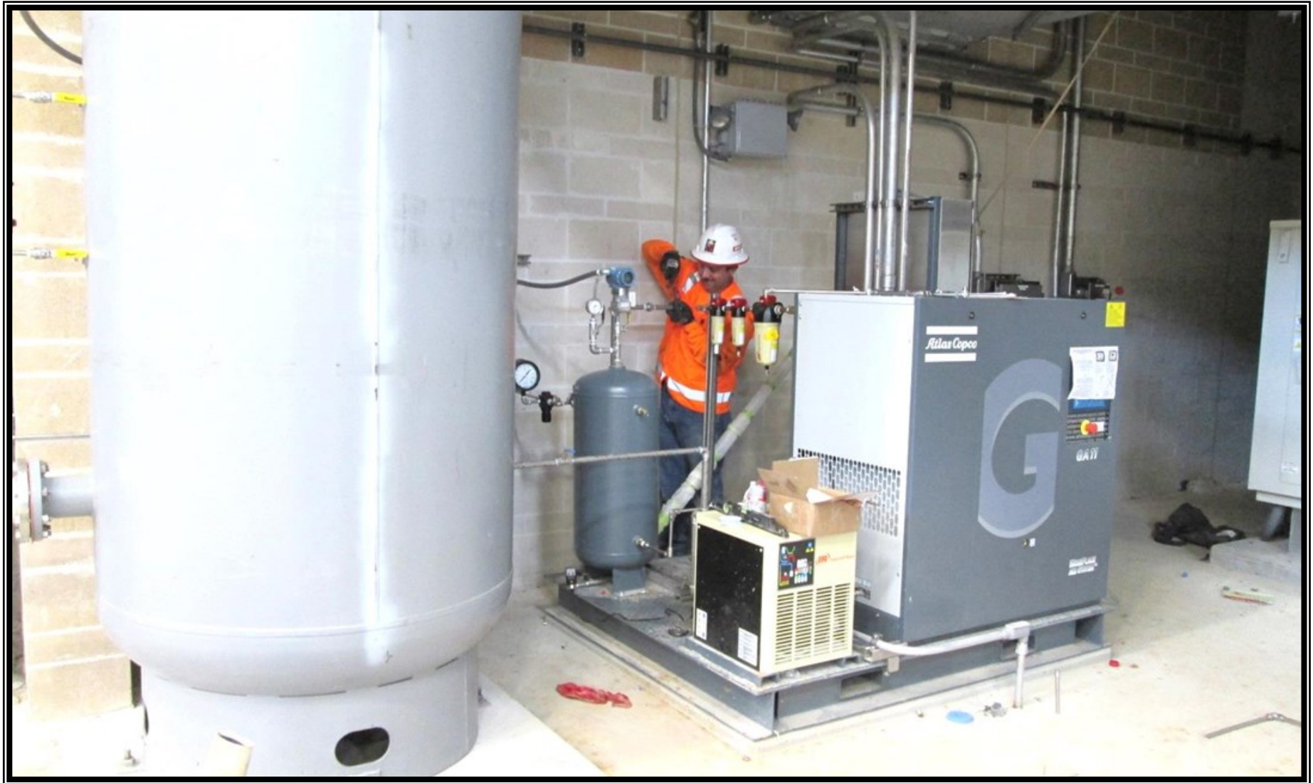
① Raw Water Intake and Pump Station—Air burst system checkout
