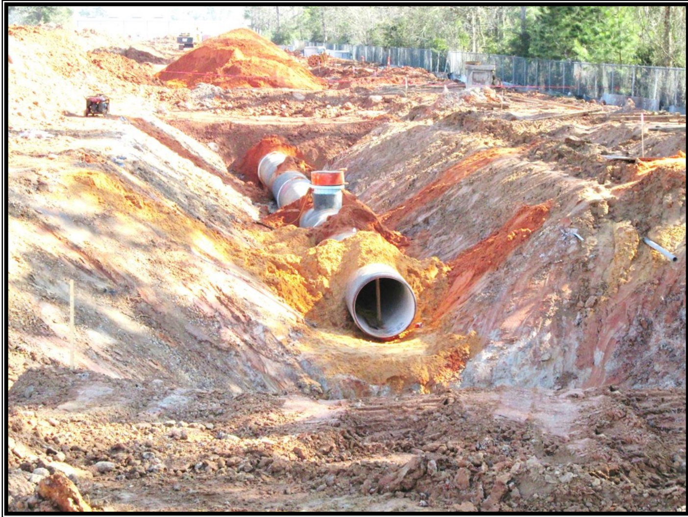
General Site—Installation of 42-inch transmission line
