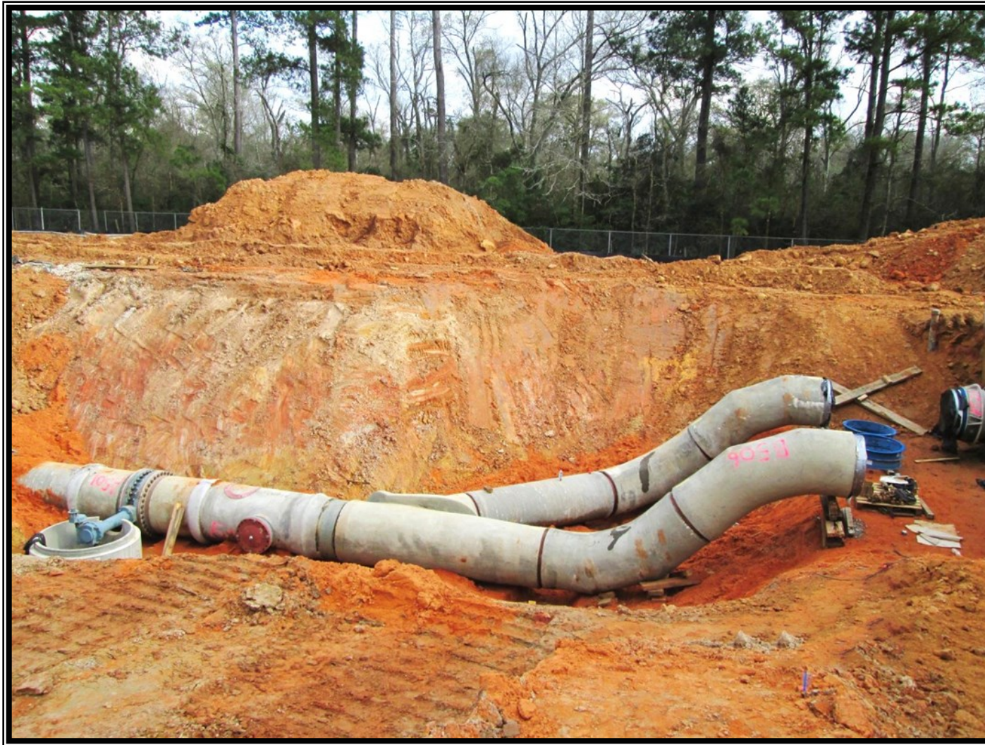
General Site—Connection of 42-inch transmission line to the High Service Pump Station (HSPS) discharge header
