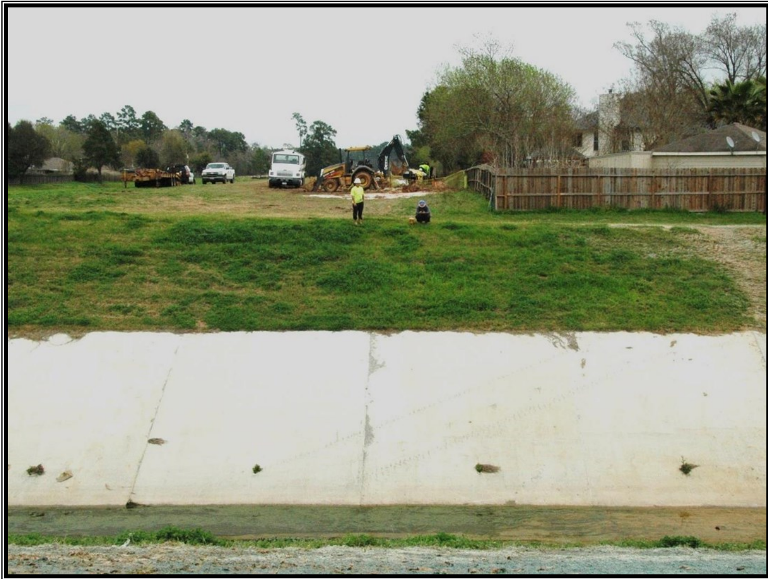
① Tunnel operations for 20-inch pipe under drainage ditch
