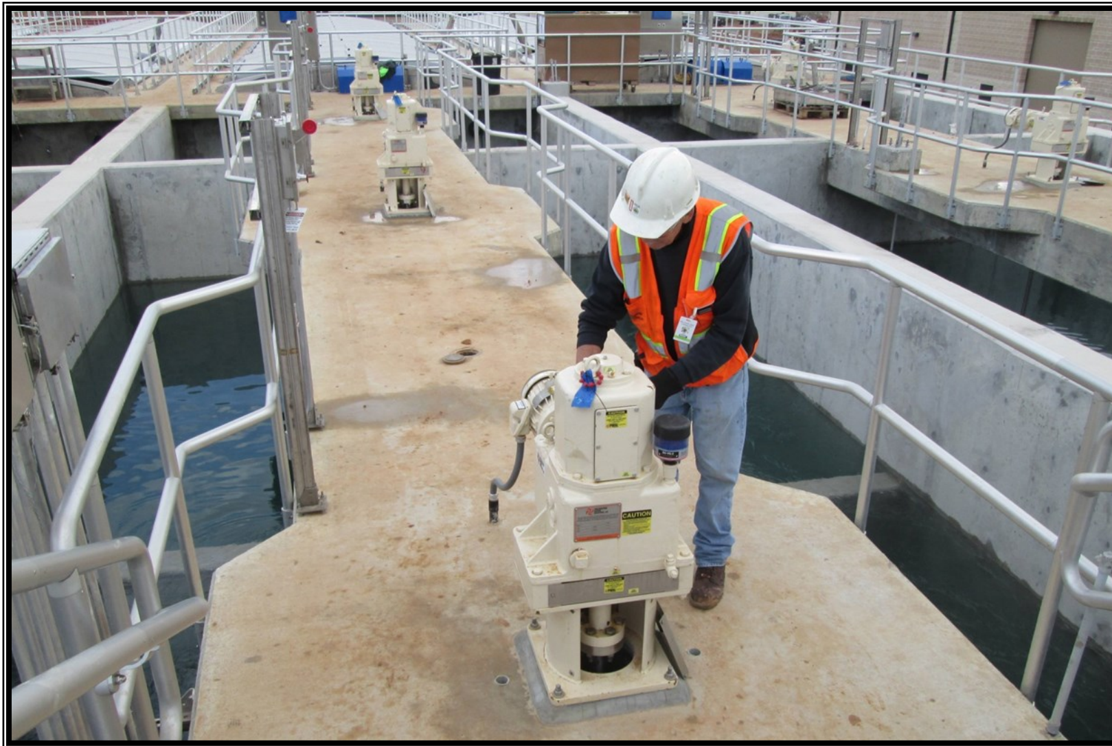
② Pretreatment Facilities — Mixer motor rotation inspection
