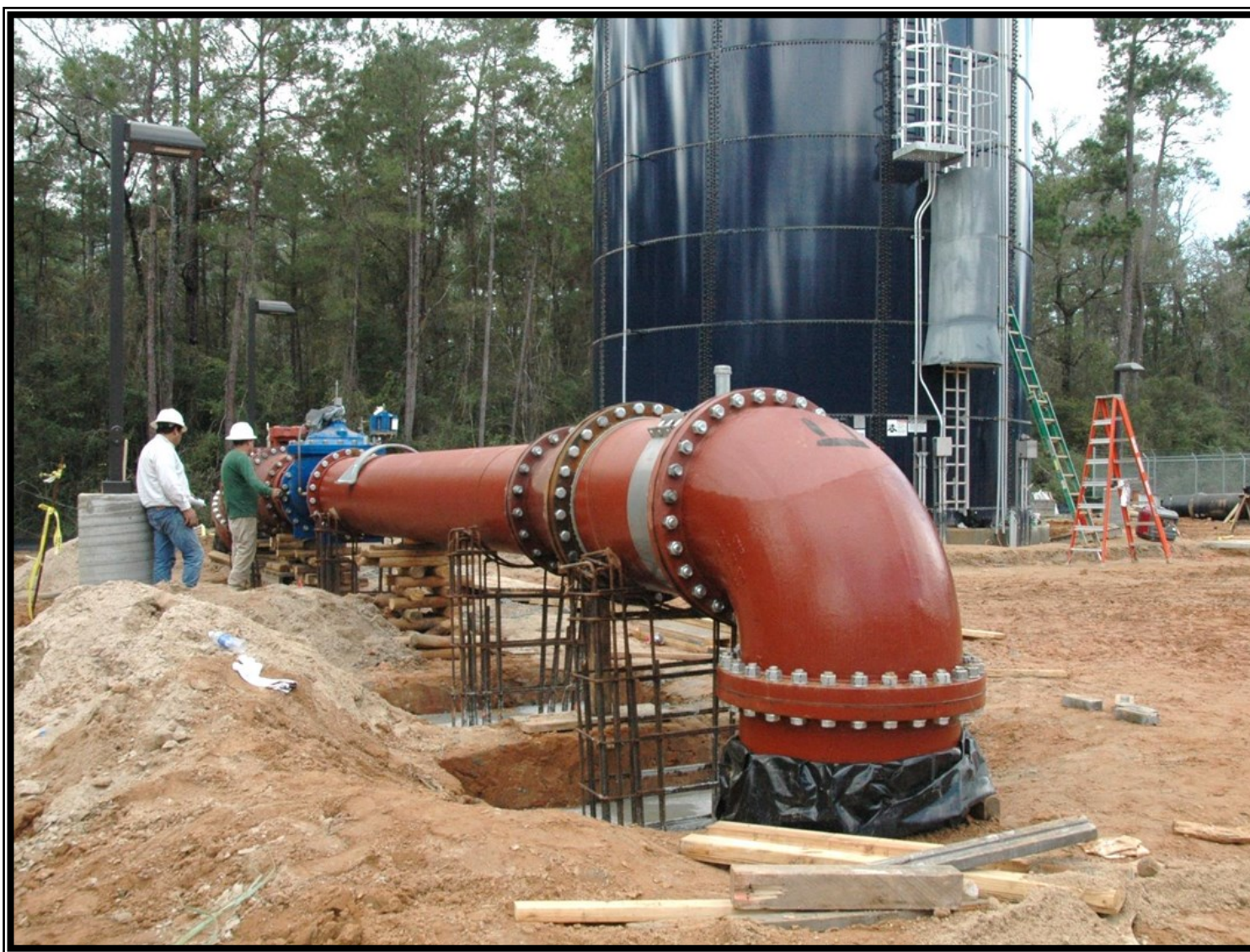
❶ Above ground piping and pipe support installation at Standpipe
