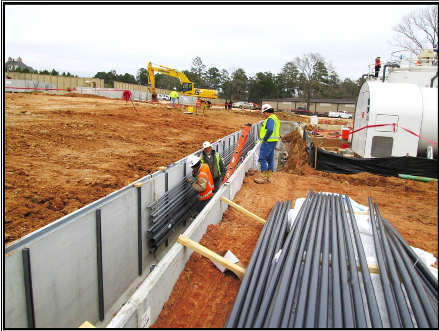
General Site—Installation of chemical piping in chemical trench
