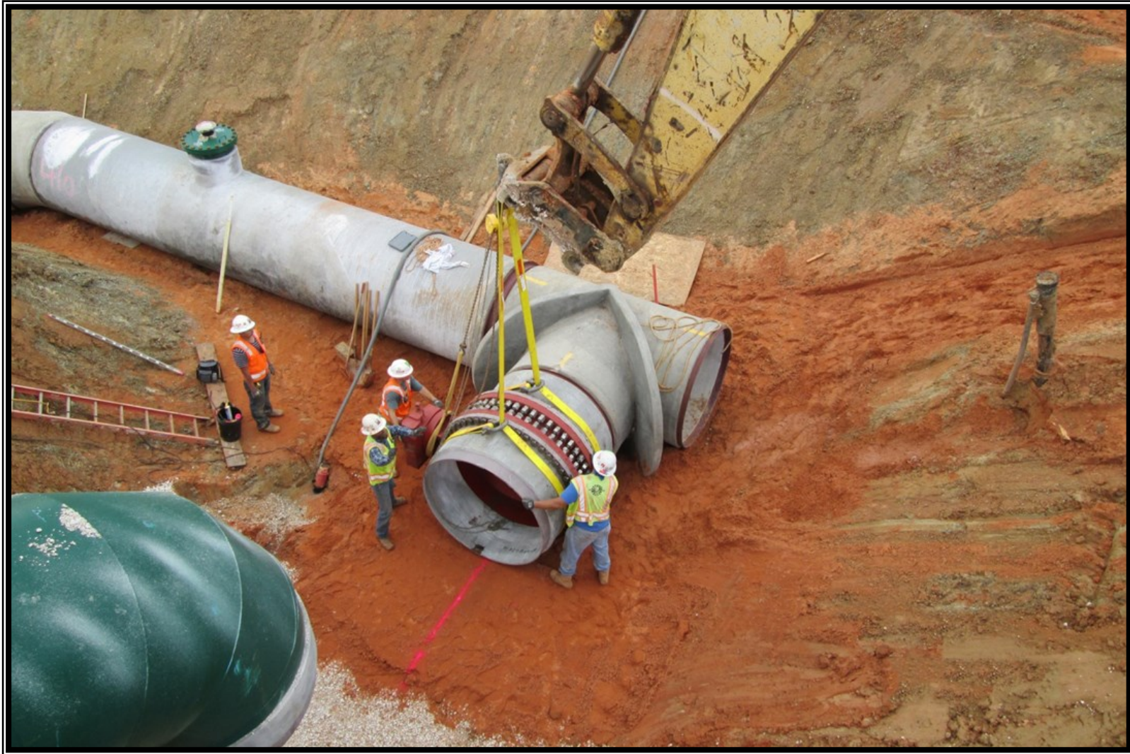
② Pretreatment Facilities — 60-inch raw water connection to rapid mix basin
