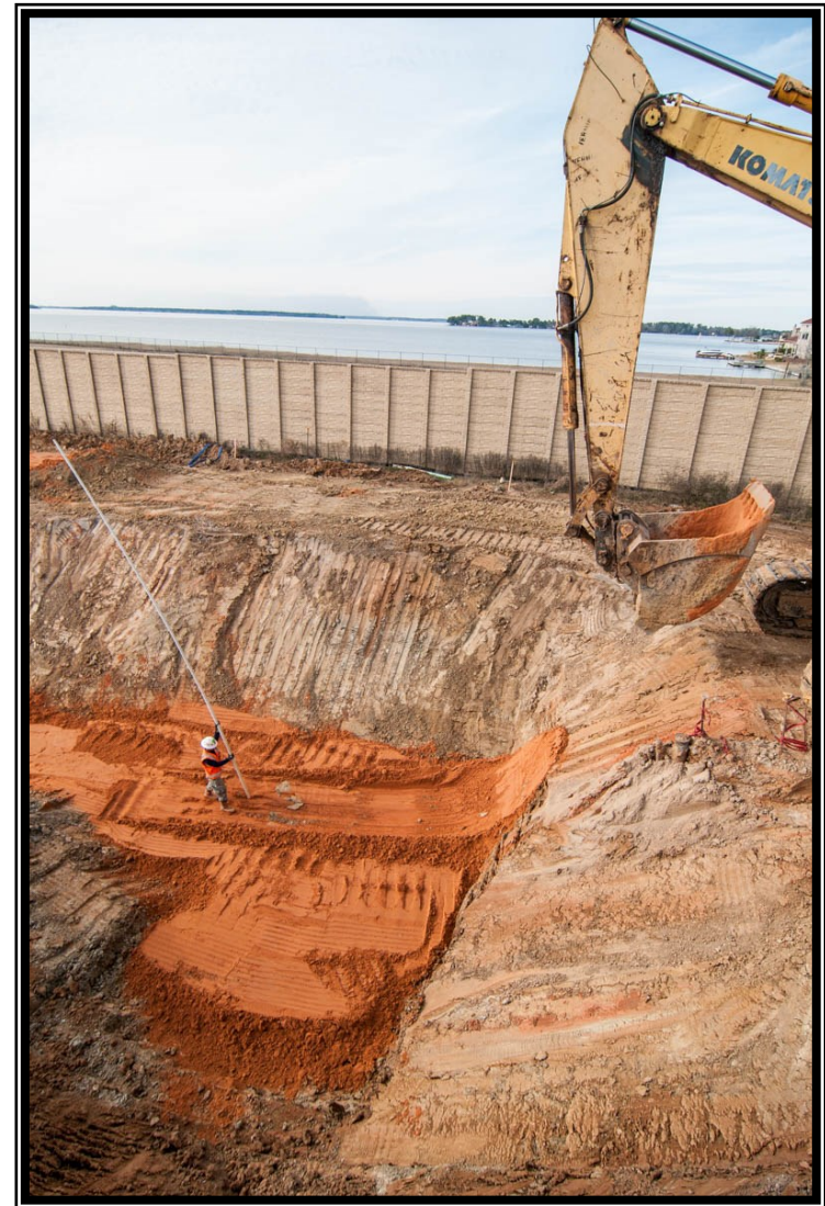
Workers installing a base for intake waterline connection at the Pretreatment Facility
