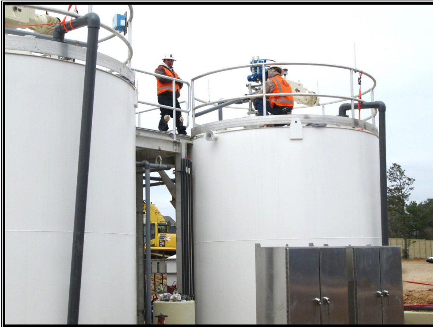
④ Chemical Building — Installation of lime mixing system piping
