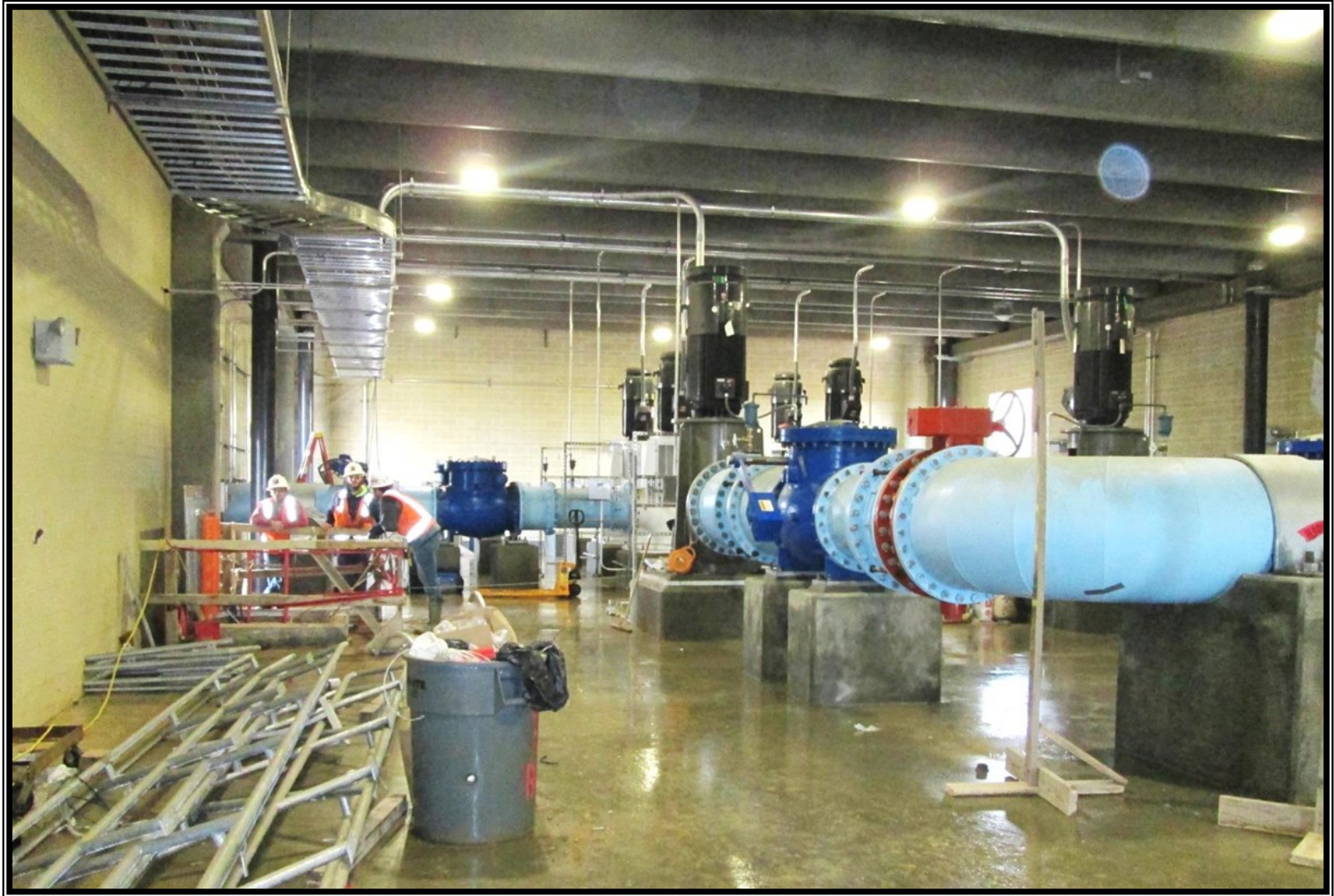
③ Granulated Activated Carbon Building — Treated water transfer pumps and piping
