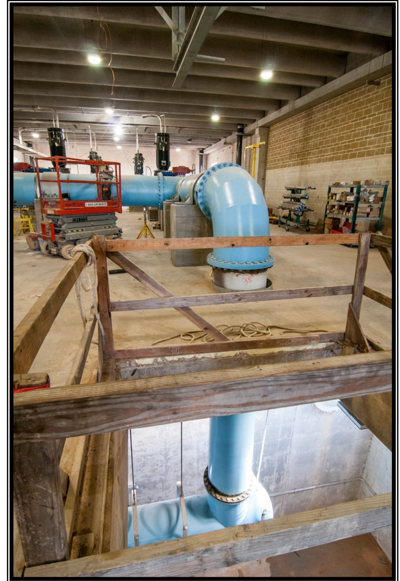
Upper and lower level view of process piping in the Granular Activated Carbon (GAC) Building
