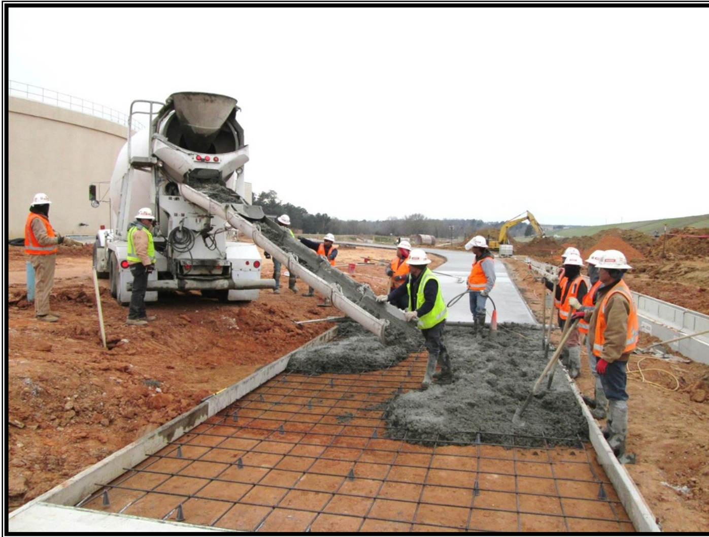
General Site—Placement of concrete roadway from Granular Activated Carbon (GAC) to the Blower Building
