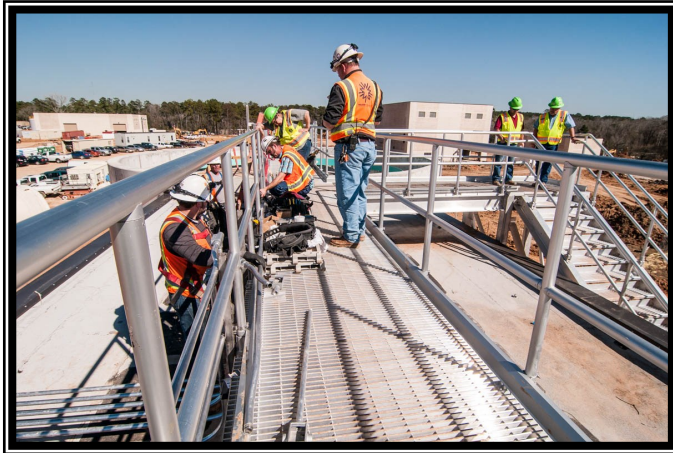
Electricians installing conduit at the Sludge Thickeners
