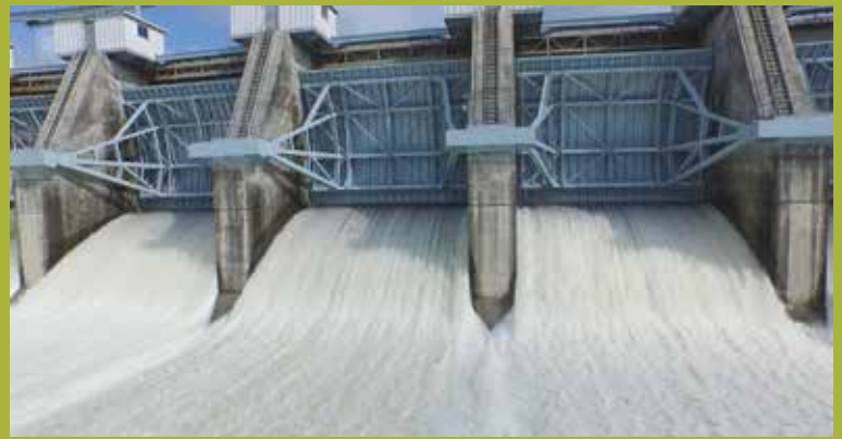
Figure 5. Back side of the main spillway gates showing storm water being released. Photo courtesy of Firefly UAV Services, LLC – www.fireflyuav.com .
