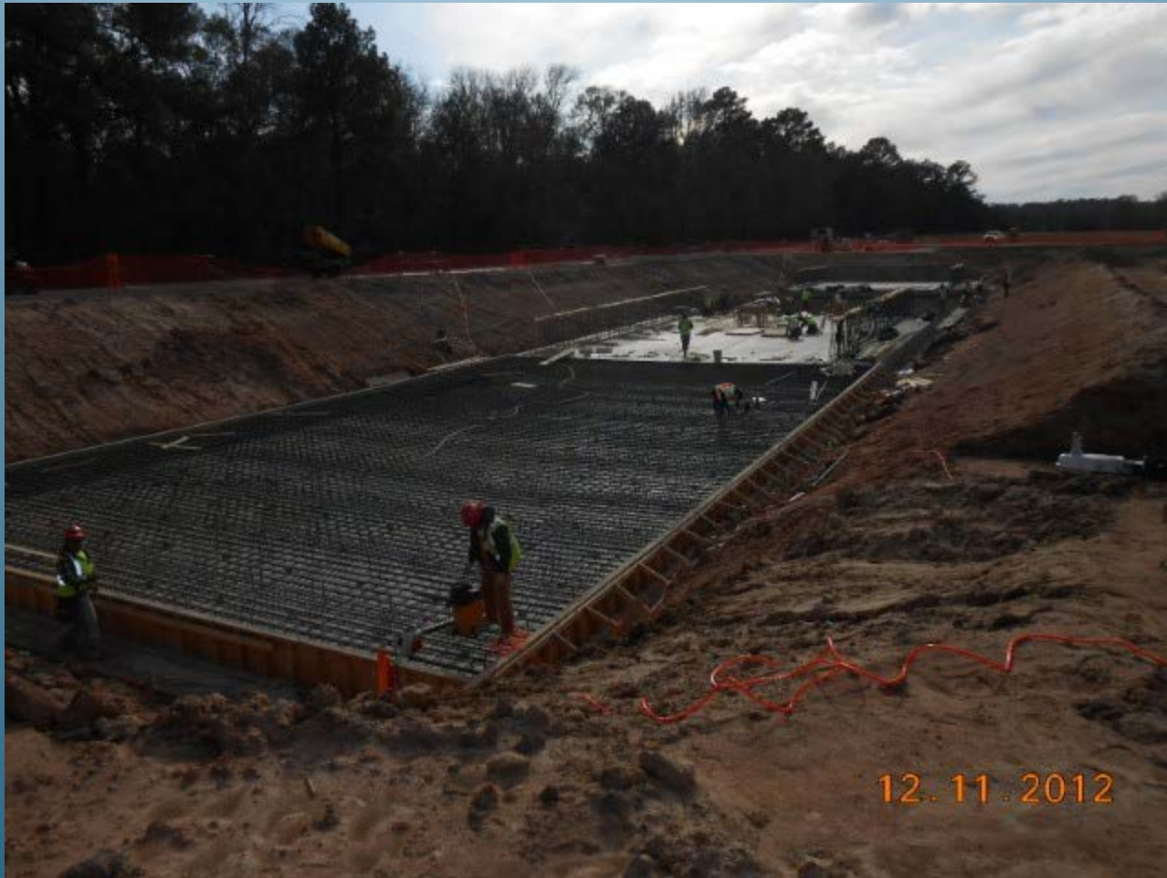
Forming and Placing Reinforcing Steel for HSPS
