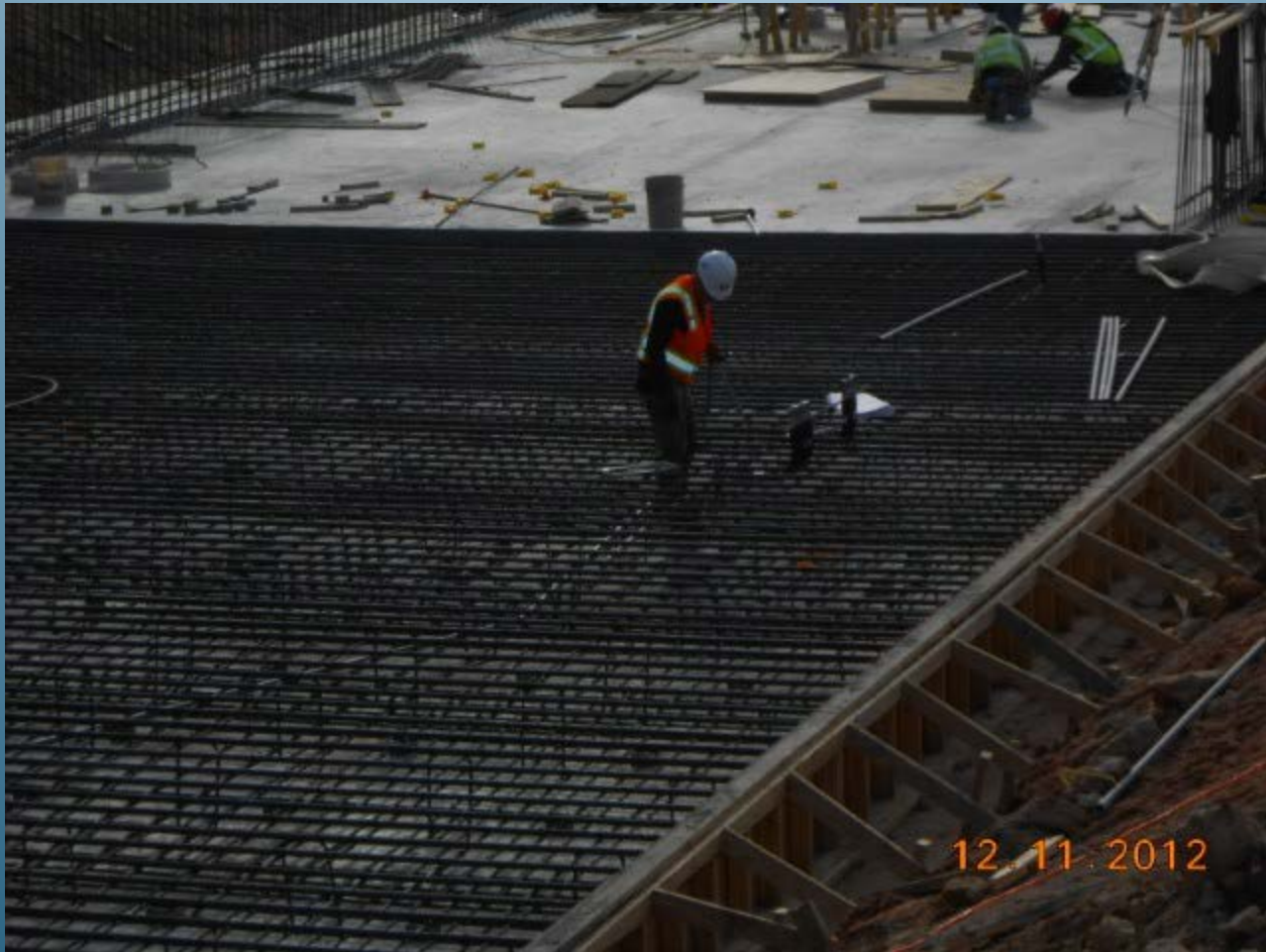
Reinforcing Steel for HSPS Discharge Bay Slab
