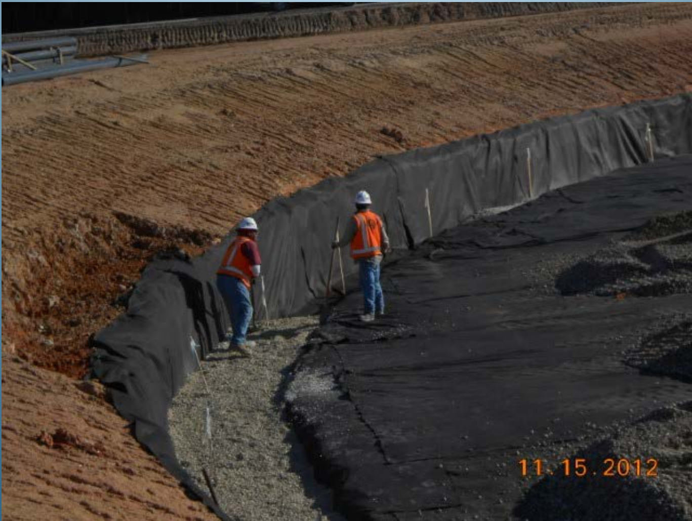
GST Under Drain Rock Installation
