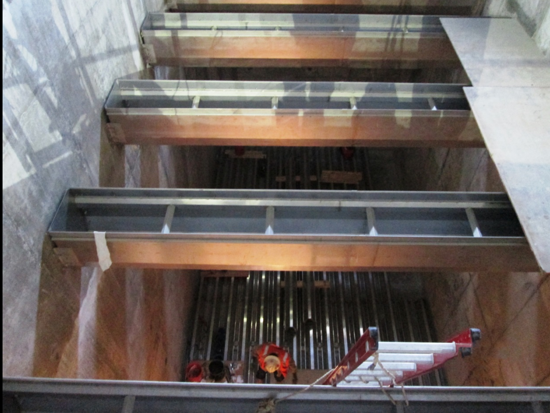
Granulated Activated Carbon Building – GAC trough and underdrain installation
