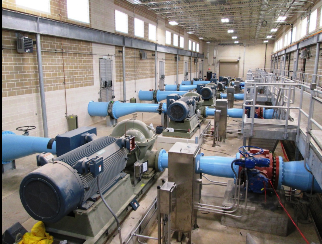
High Service Pump Station – Pump room overview
