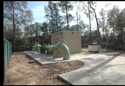
SJRA Water Plant No. 2
