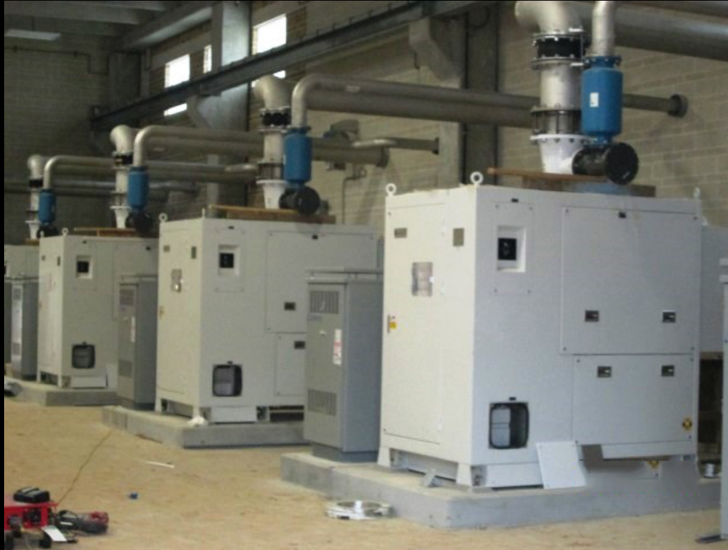
Blower Building – Installation of turbo blowers
