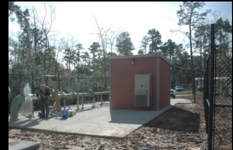
SJRA Water Plant No. 5
