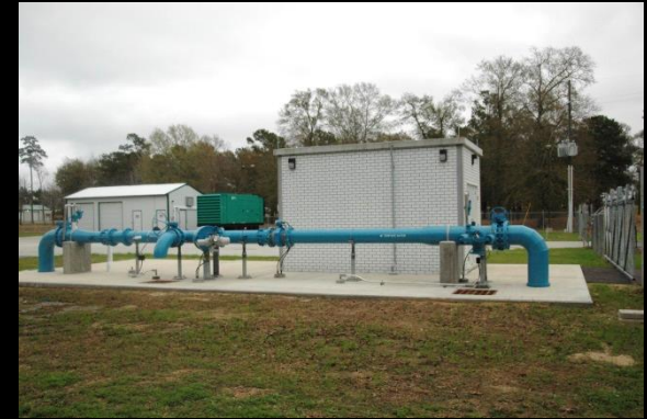
City of Conroe Water Plant No. 22
