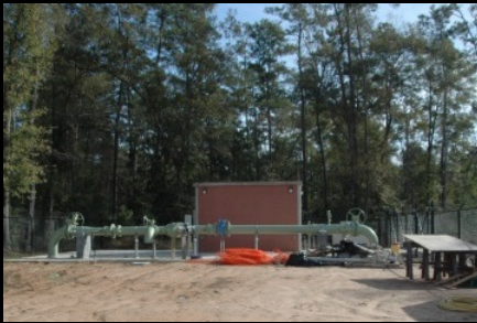
SJRA Water Plant No. 3
