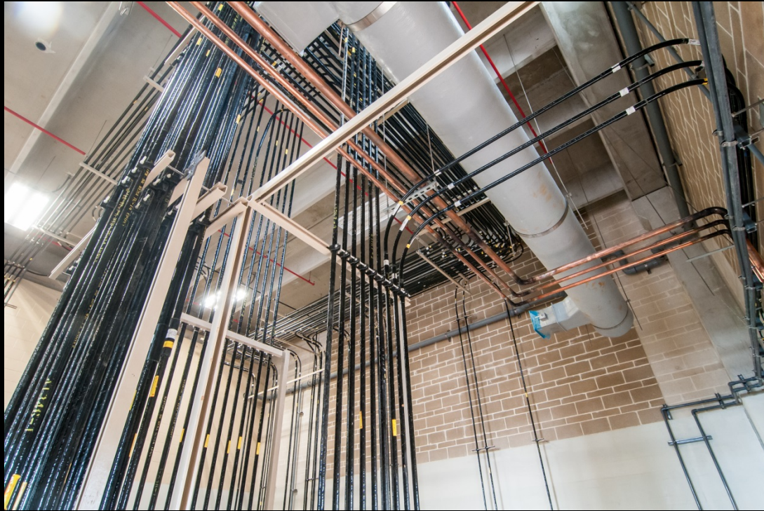
Chemical Building – Electrical conduit installation
