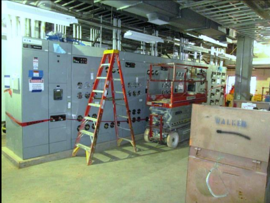
Membrane Building – Electrical equipment installation
