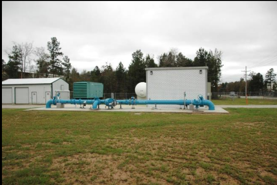
City of Conroe Water Plant No. 20
