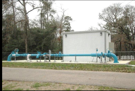
City of Conroe Water Plant No. 14W
