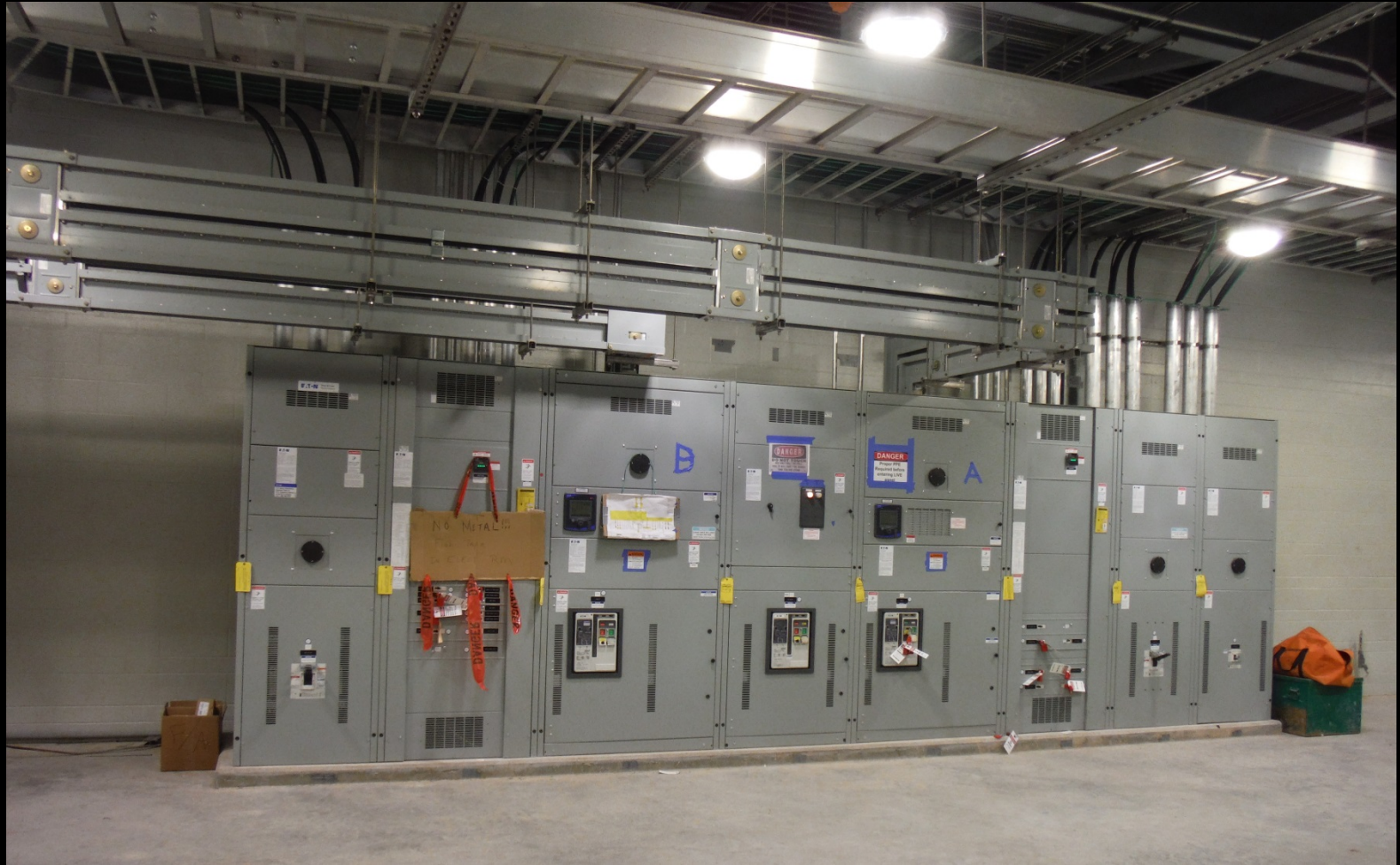
Raw Water Intake – Electrical equipment installation
