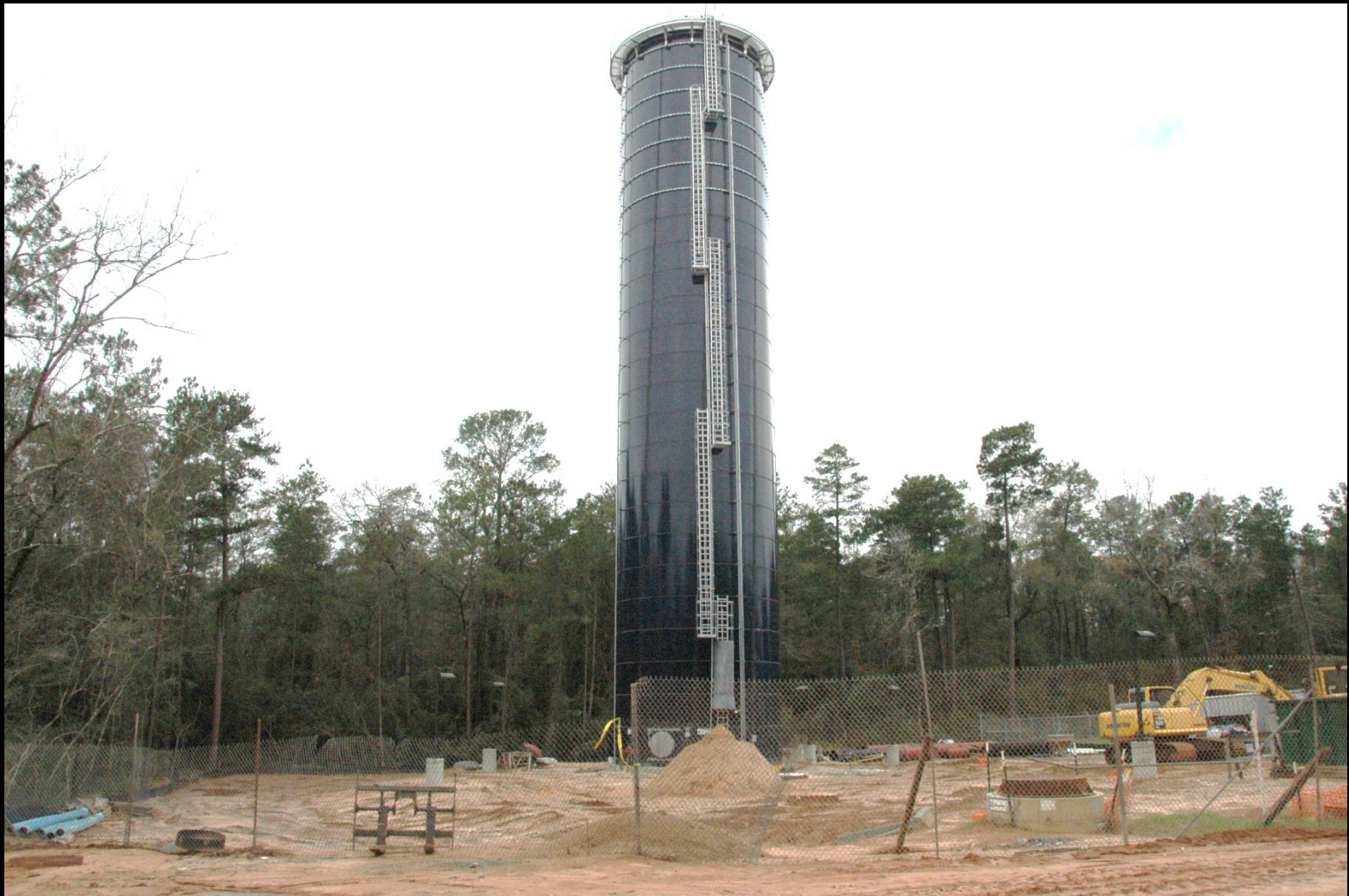
Continuation of yard piping at Standpipe
