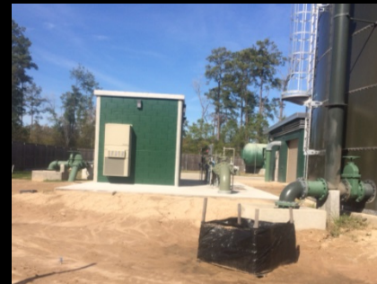
SMCMUD Water Plant No. 3
