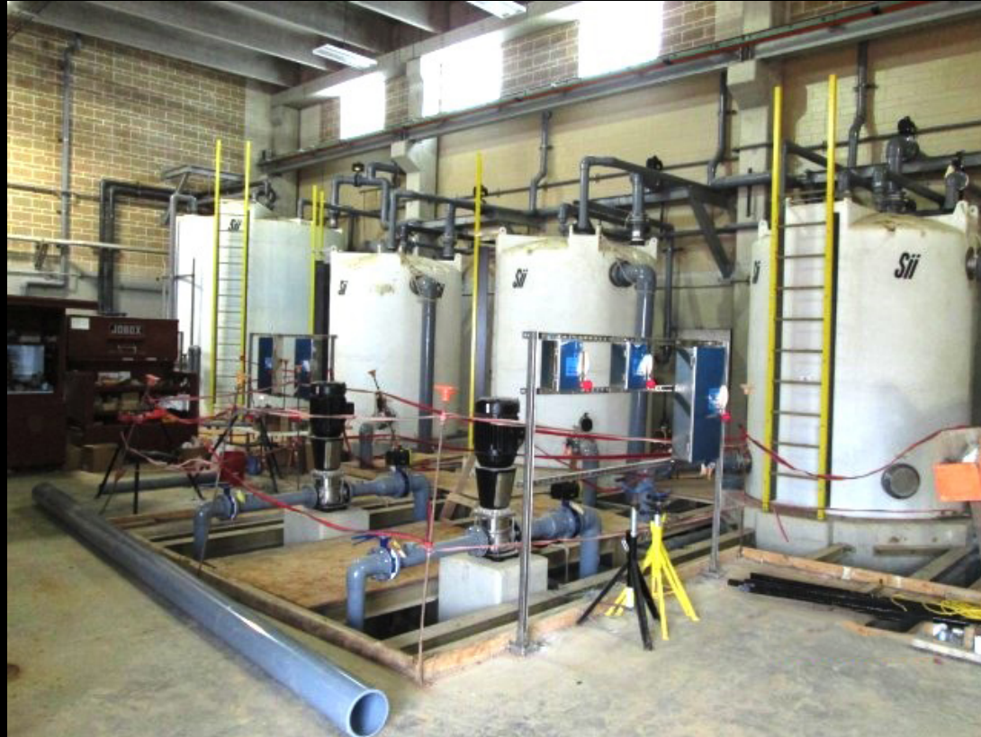
Membrane Building – Chemical storage and pumping systems
