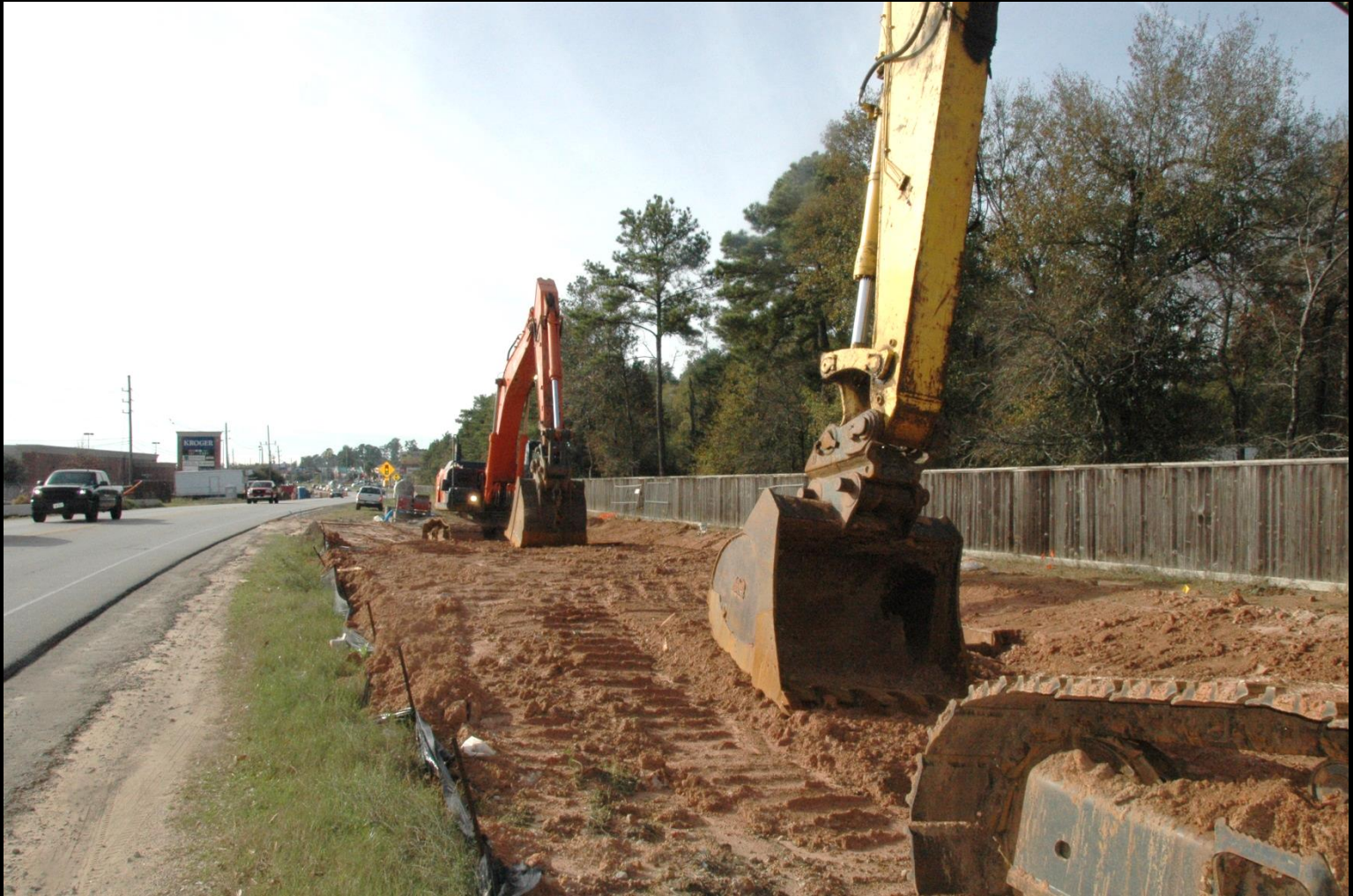
Staging for open cut construction along Sendera Ranch Road
