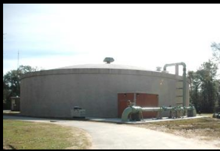
SJRA Water Plant No. 1
