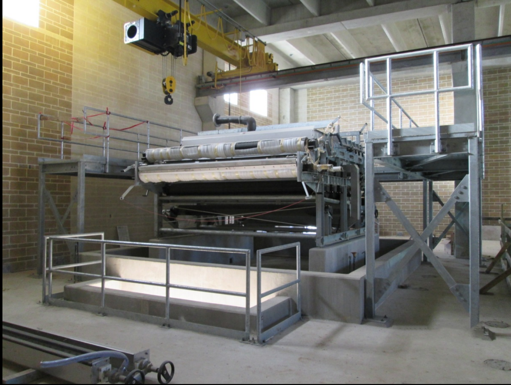
Dewatering Building – Belt filter press and walkway
