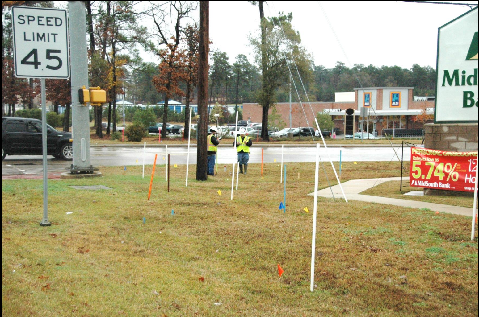
Utility locates for tunnel construction at Longmire Road and Loop 336
