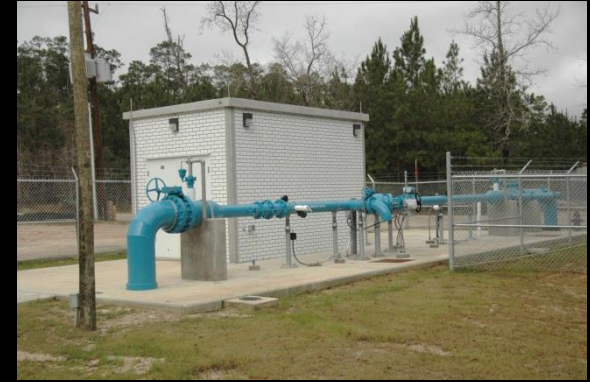
City of Conroe Water Plant No. 15
