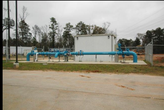
City of Conroe Water Plant No. 21
