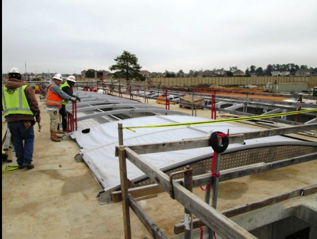
Pretreatment – Installation of basin covers
