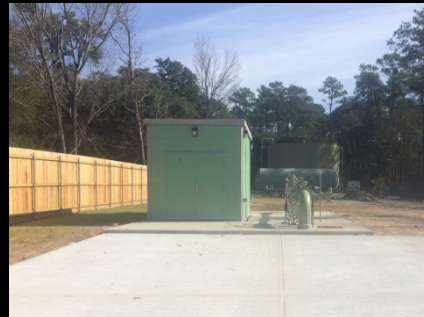
SMCMUD Water Plant No. 2
