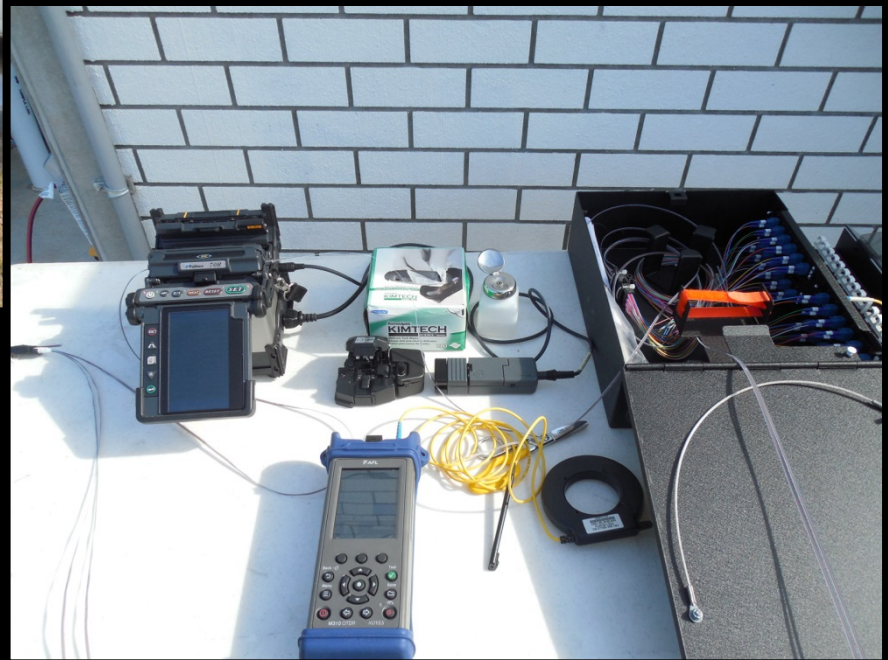
Fiber Optic splicing and testing at City of Conroe Water Plant No. 20
