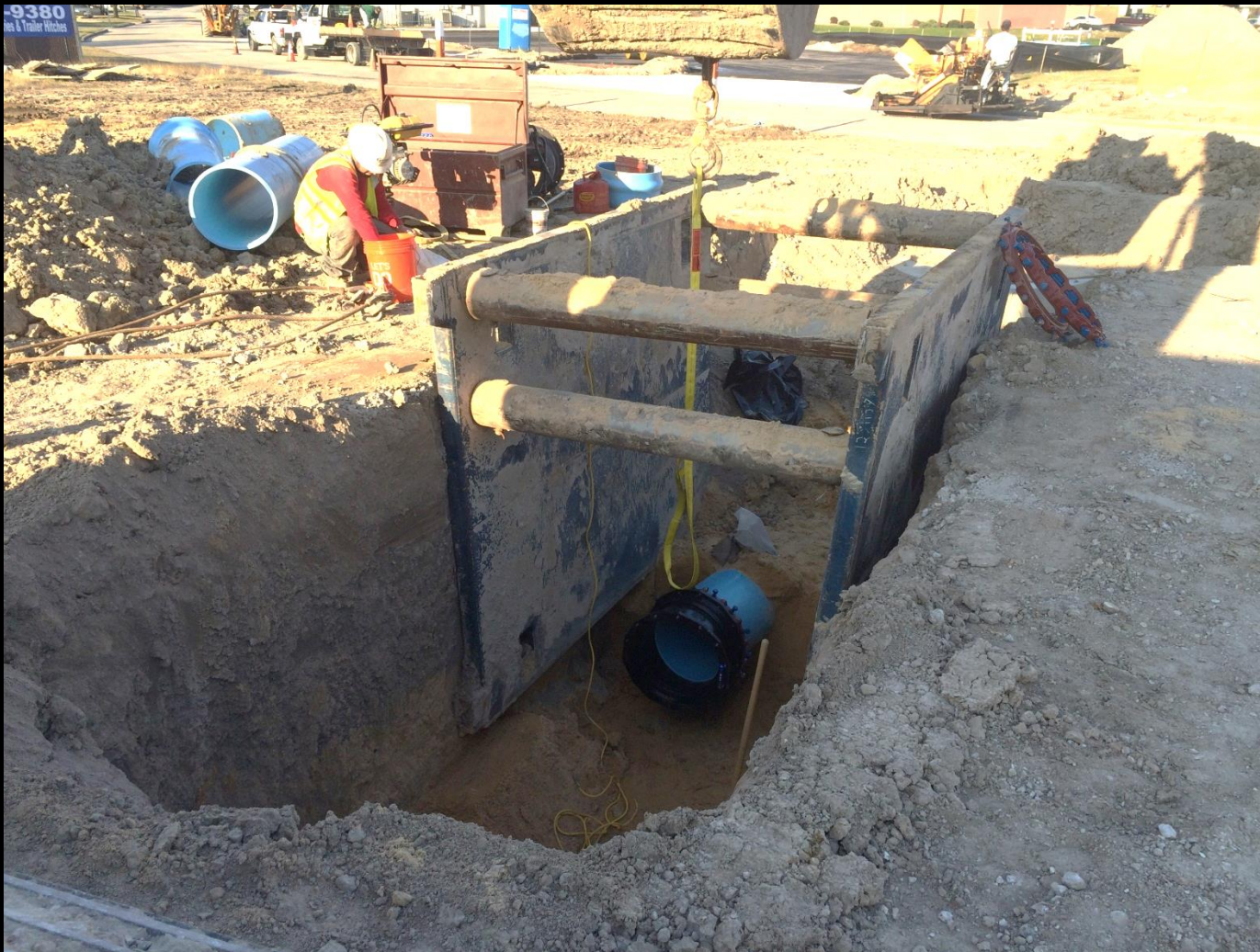
Open cut construction along Kinder Morgan pipeline easement
