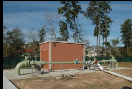
SJRA Water Plant No. 4
