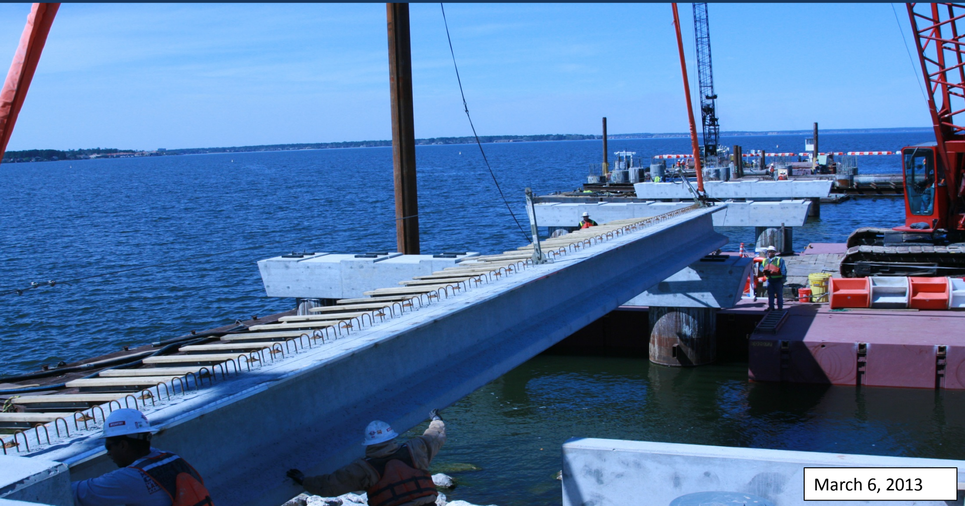
Placement of 75 feet long precast concrete bridge girders
