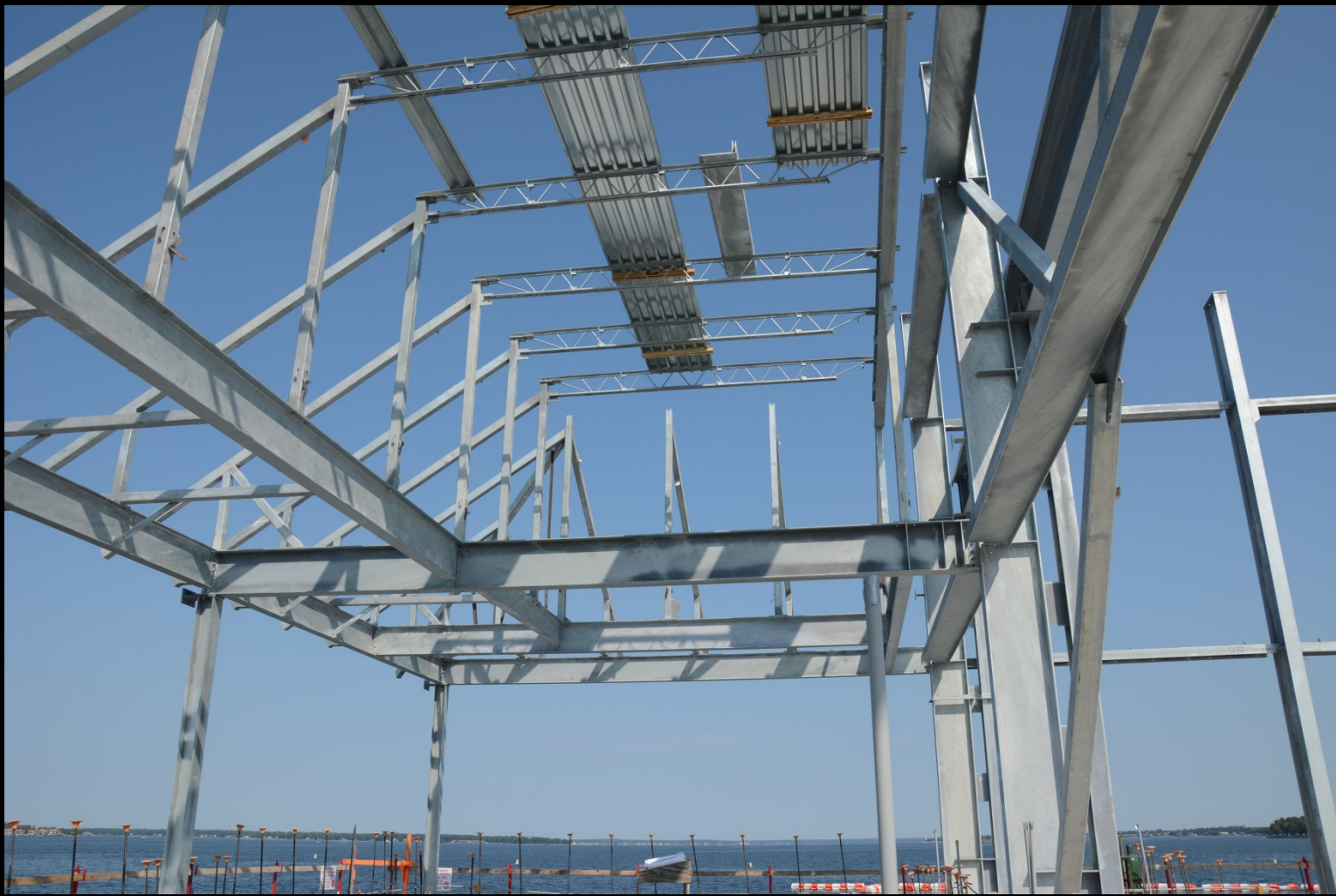
Steel erection and staging at Raw Water Pump Station
