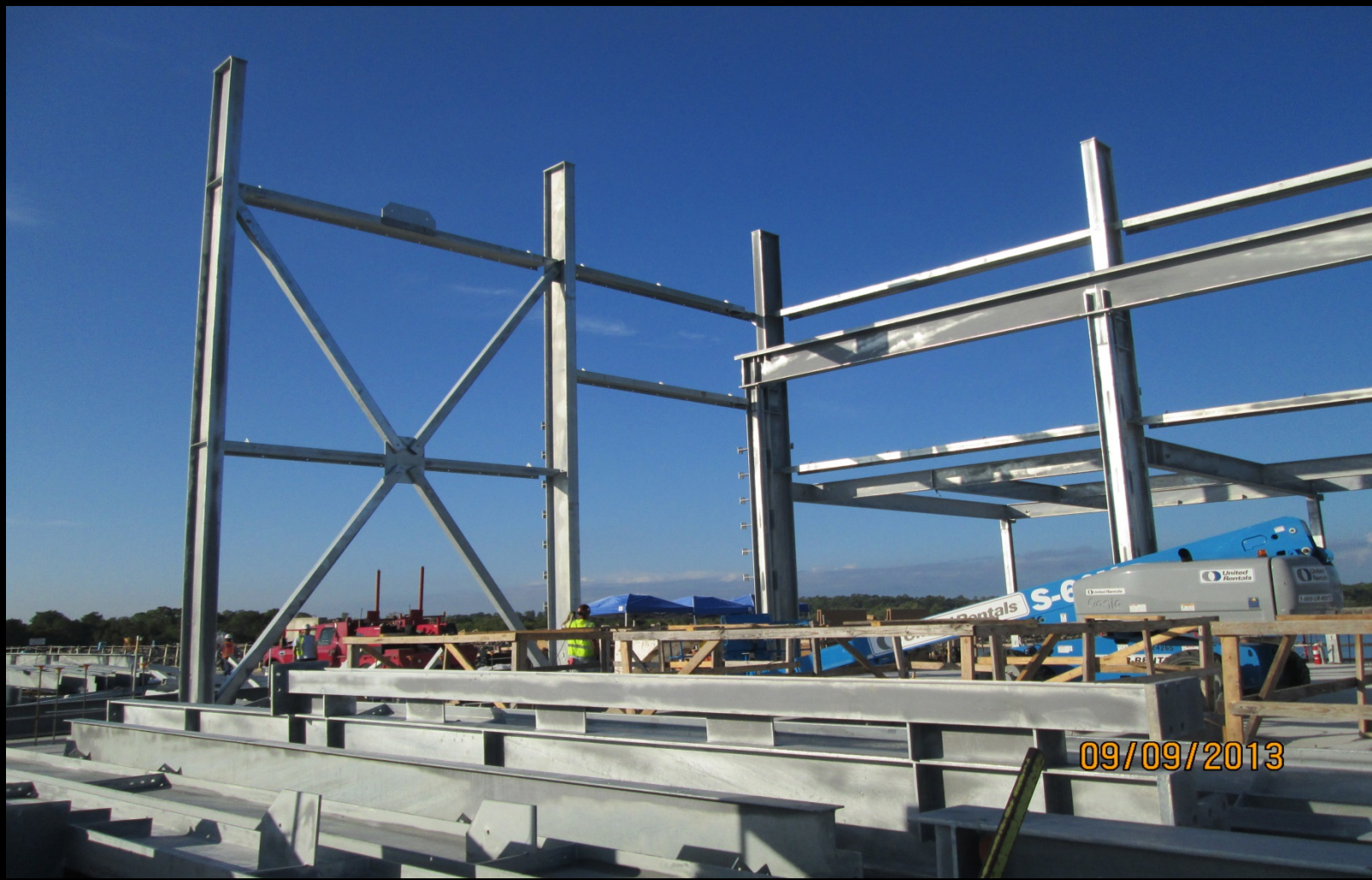
Steel erection and staging at Raw Water Pump Station
