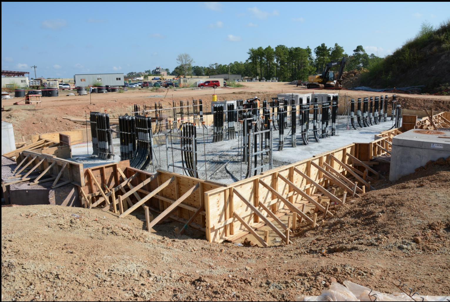
Electrical rough-in at Power Supply Building
