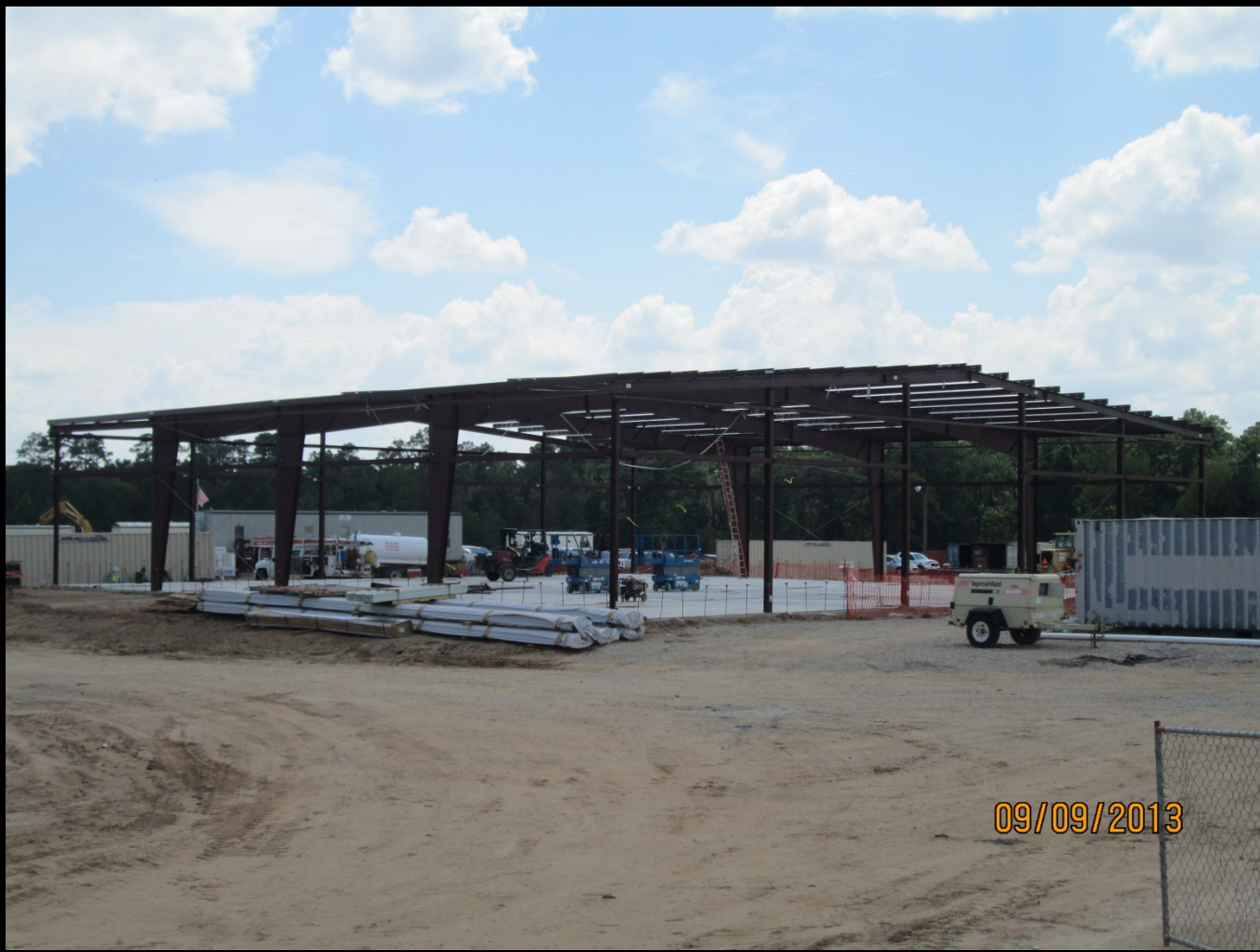
Steel erection complete at Warehouse
