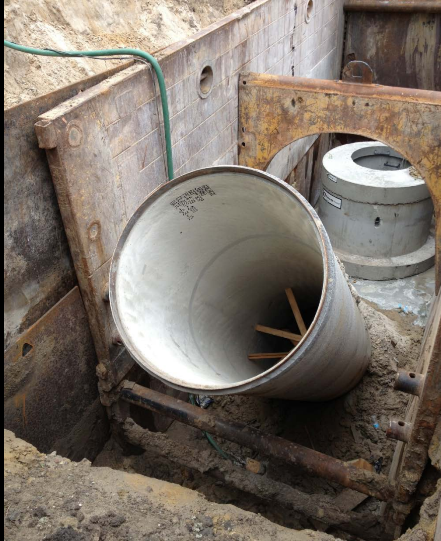
Open cut tie-in at the spillway
