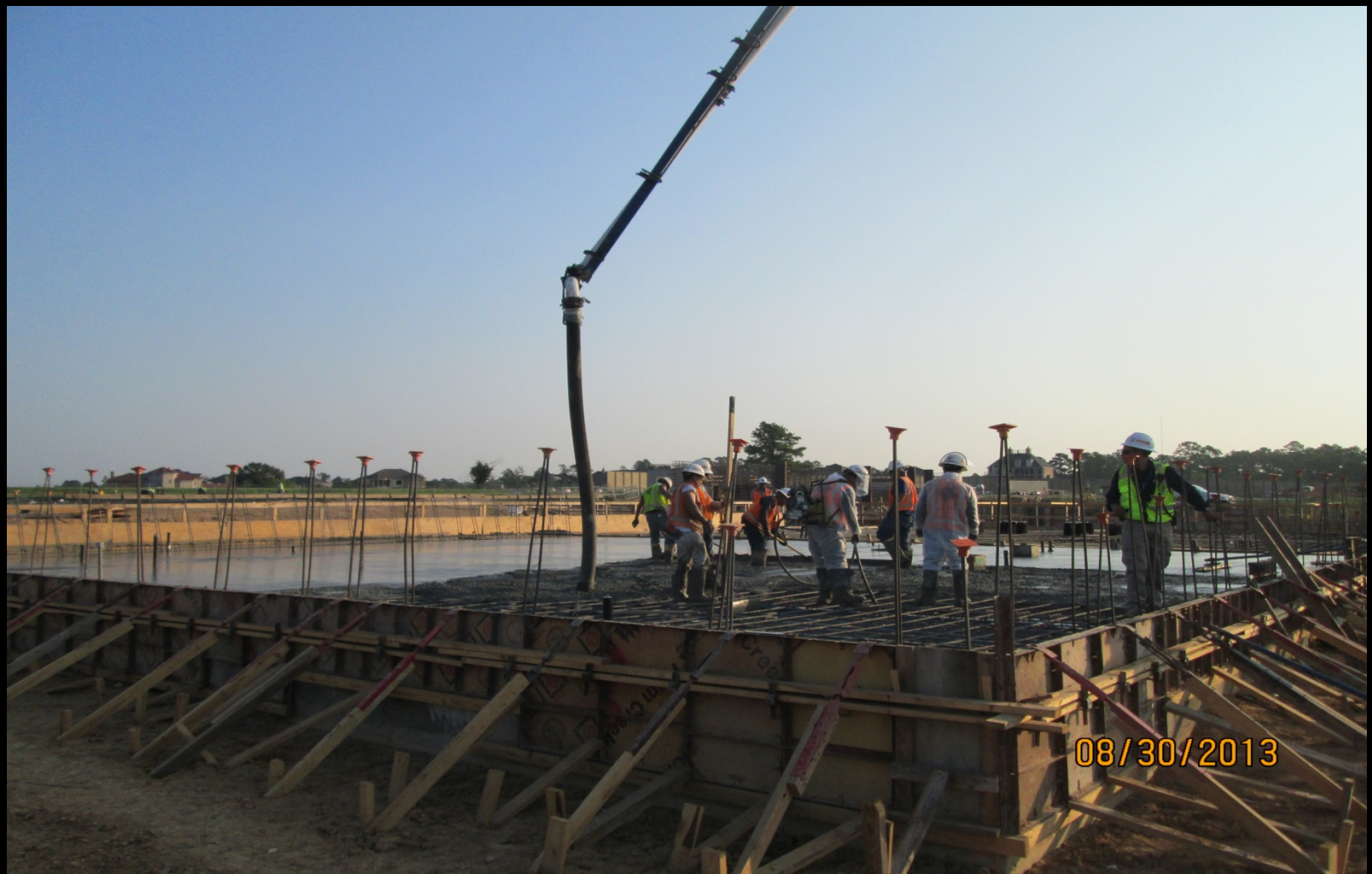
Foundation placement at Membrane Building
