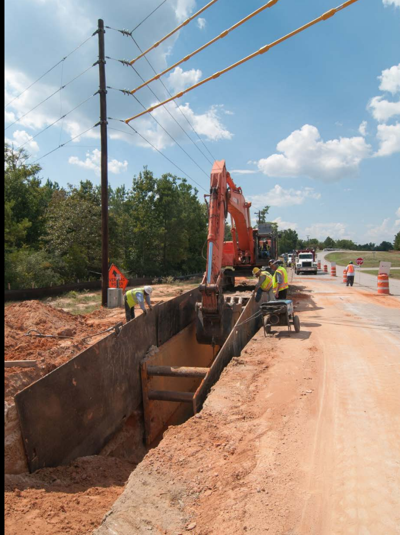
Open cut installation – Fish Creek Thoroughfare
