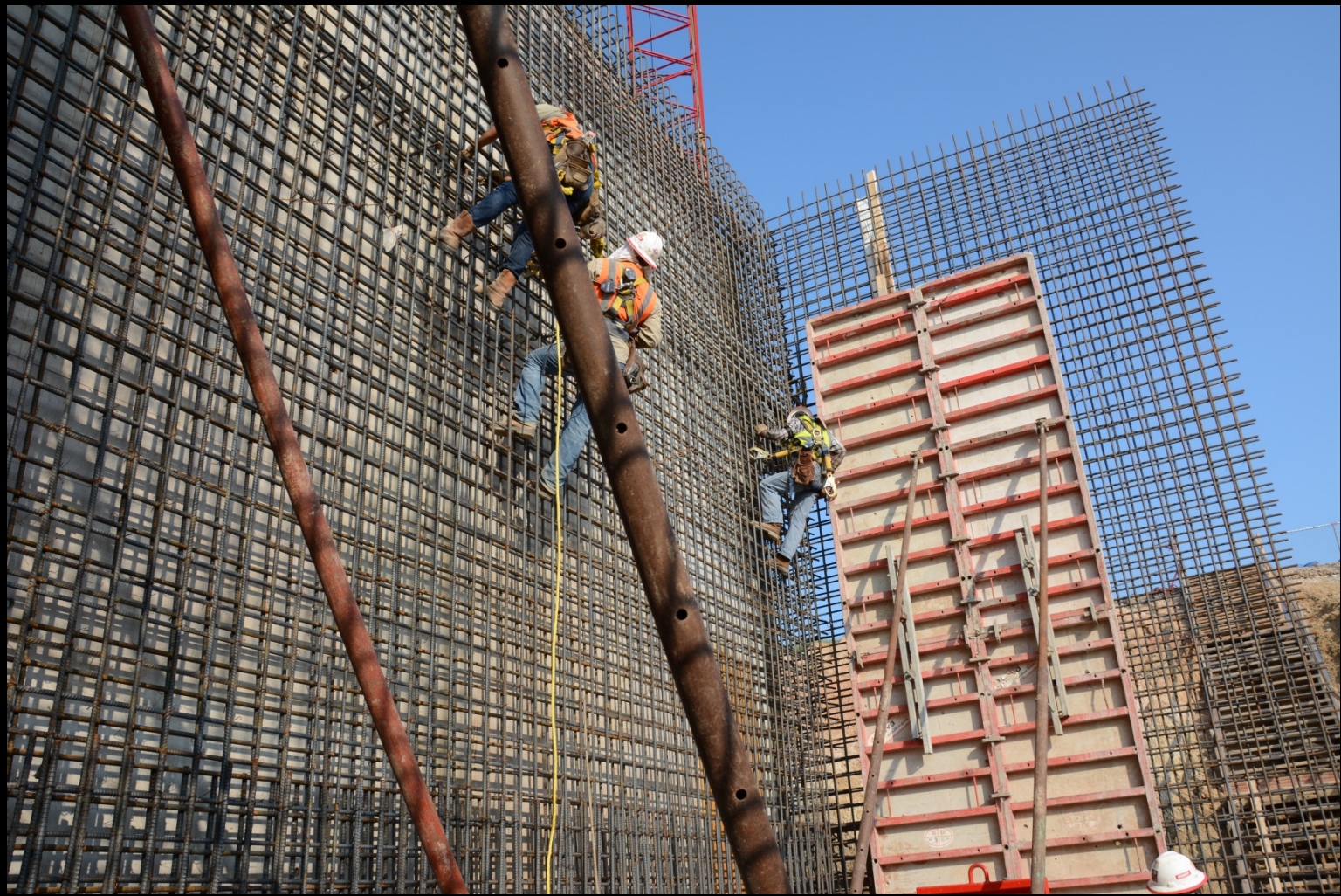
Rebar installation for contactor wall
