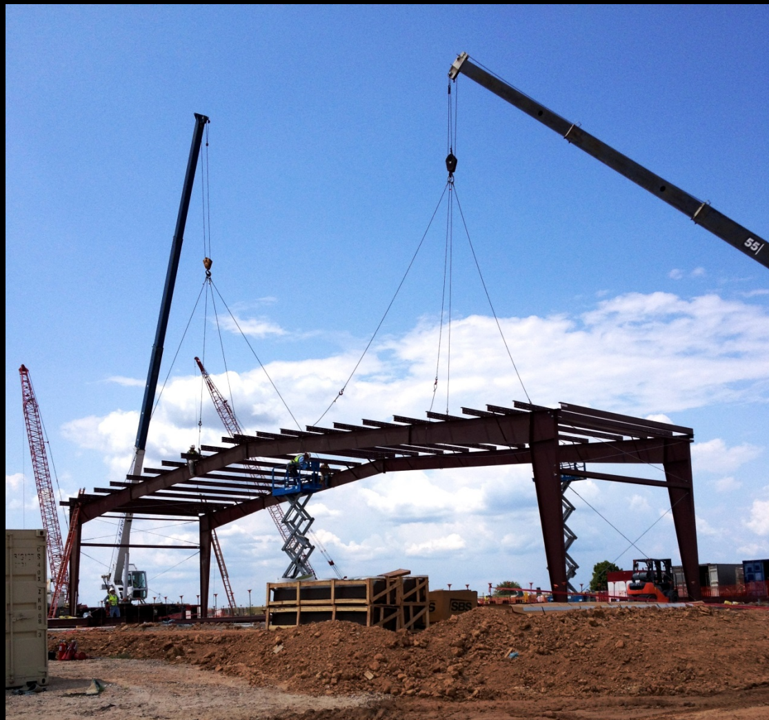
Steel erection at Warehouse
