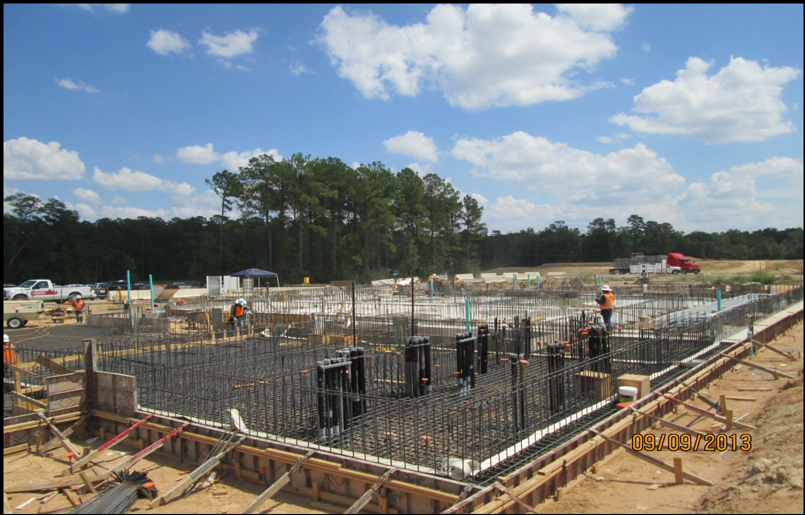
Concrete and rebar placement at the Chemical Building
