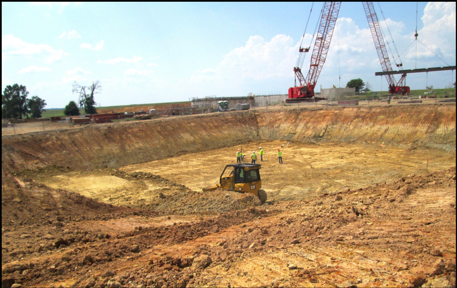
Mass excavation at the Backwash Equalization Basin
