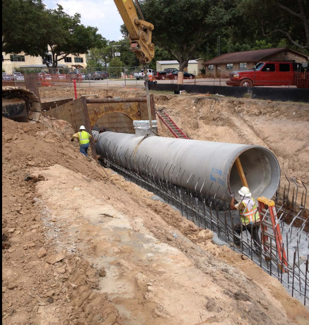
Concrete encasement of 60" line west of G&A Building
