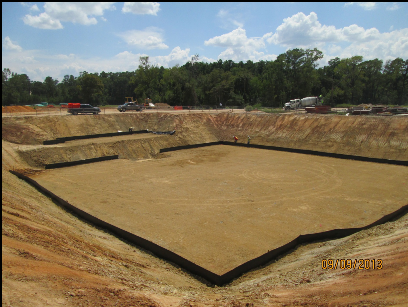
Subgrade preparation complete at the Backwash Equalization Basin
