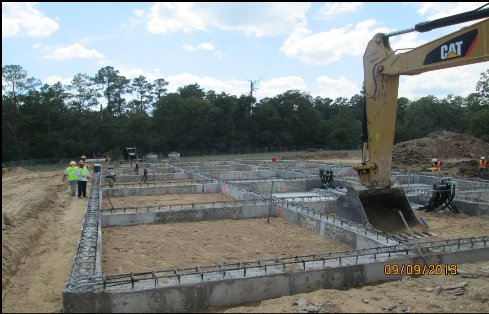
Structural backfill at Power Supply Building
