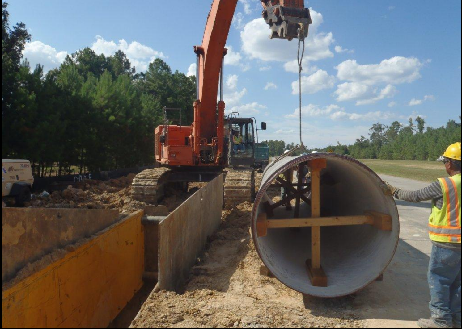
Open cut pipe installation – Fish Creek Thoroughfare
