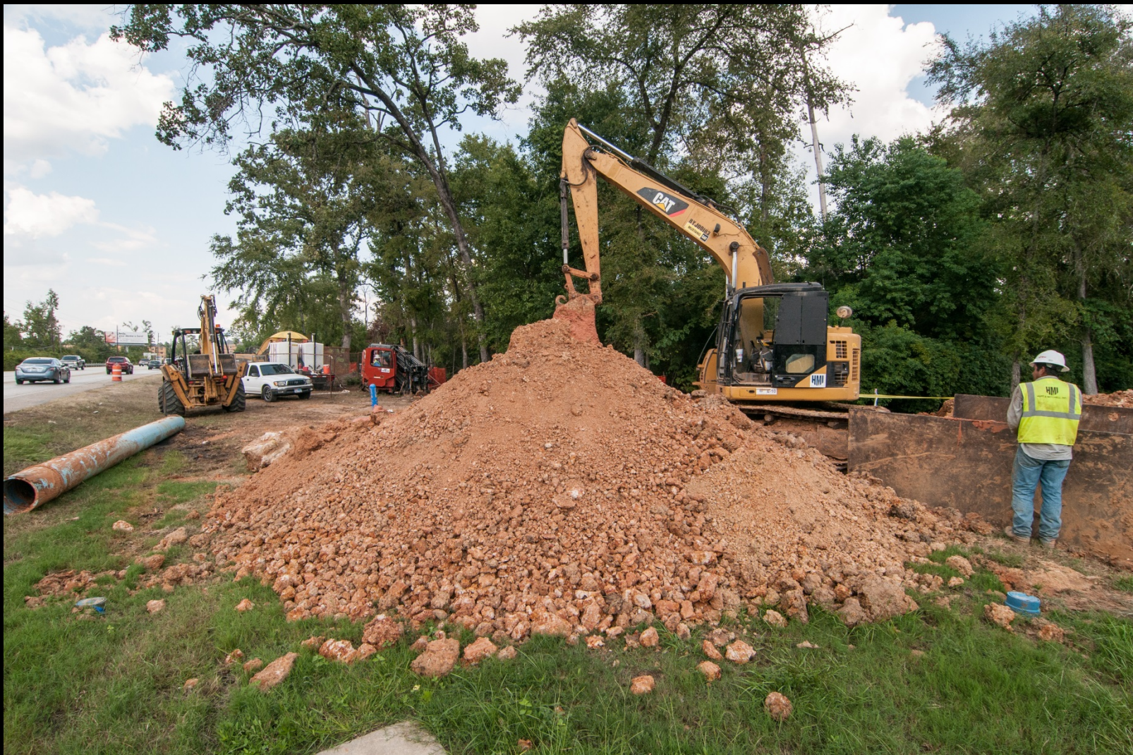
Excavation for 16" PVC pipe along FM 2978
