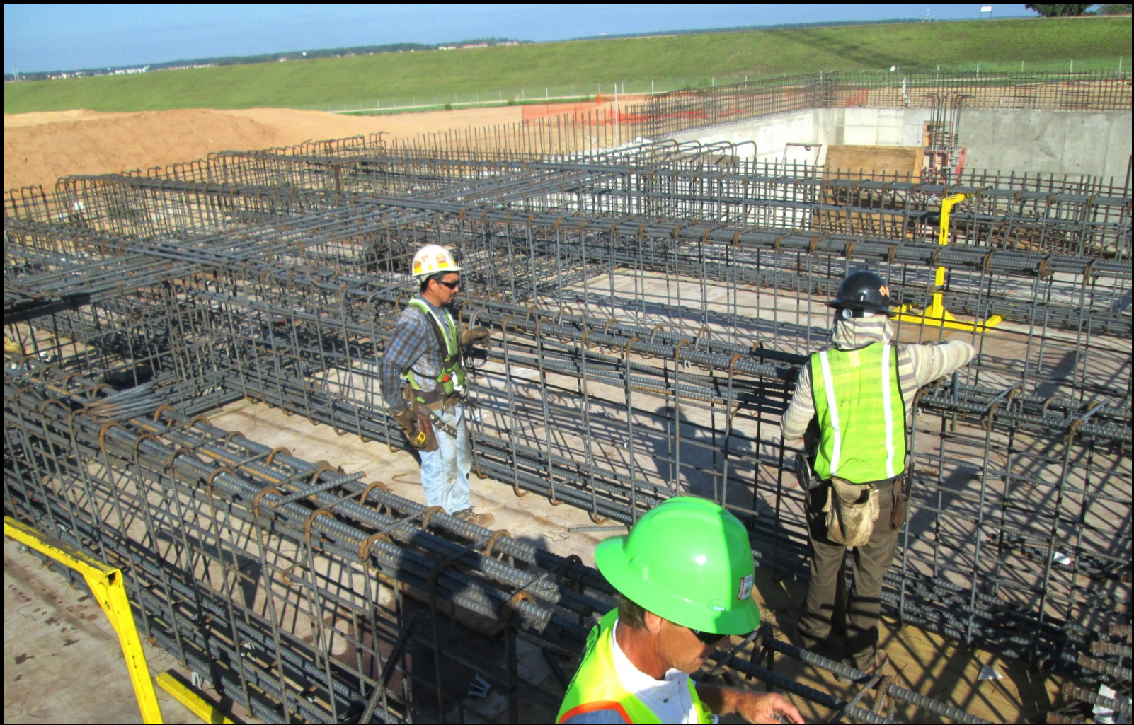
Rebar installation for the 2 nd floor concrete deck
