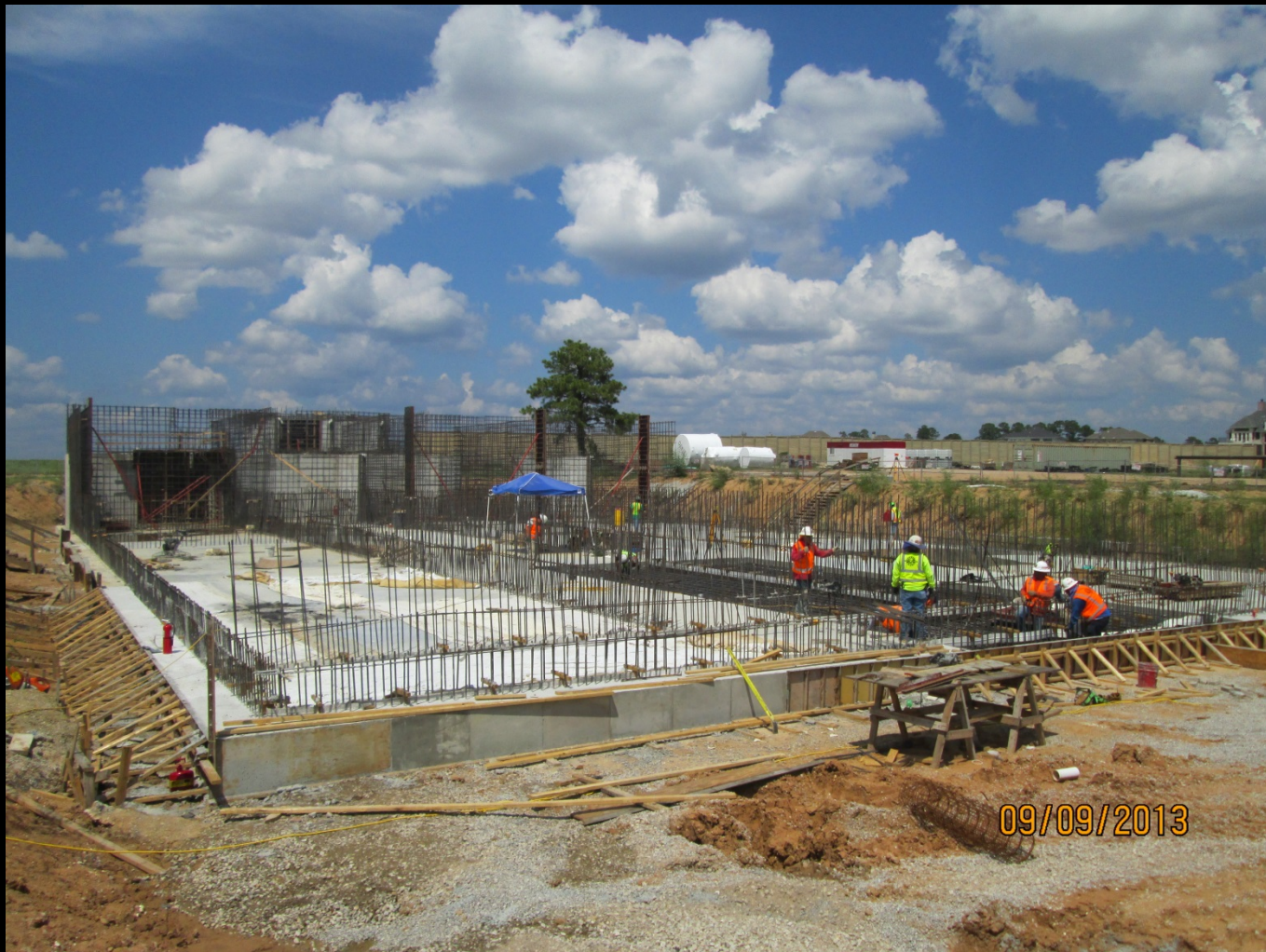
Continuation of Pretreatment Structure foundation installation
