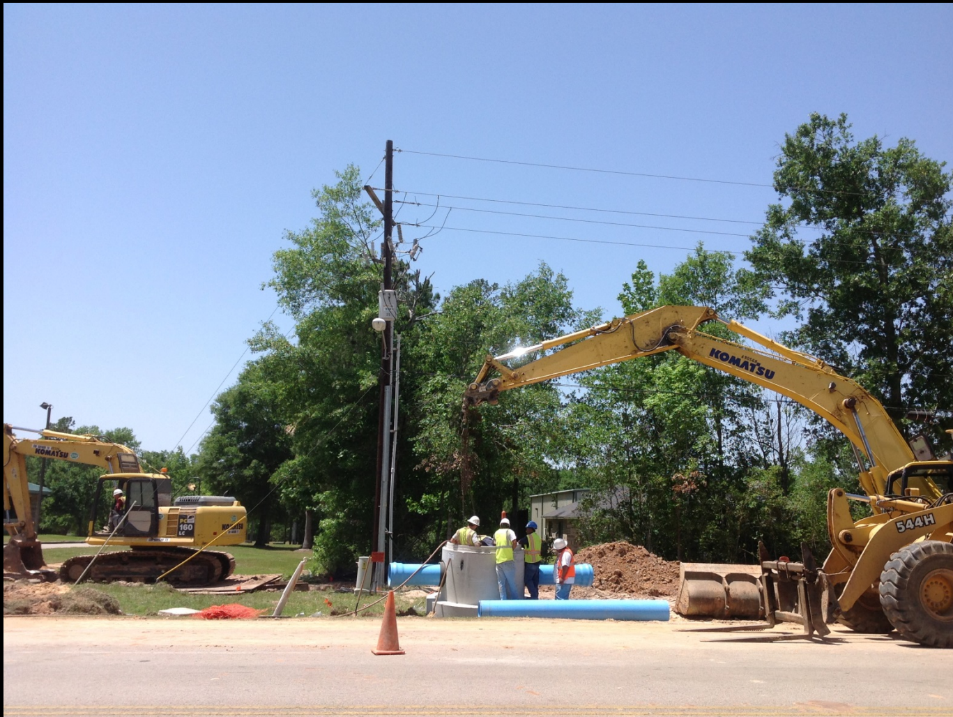
Valve access manhole installation along Pollock Road
