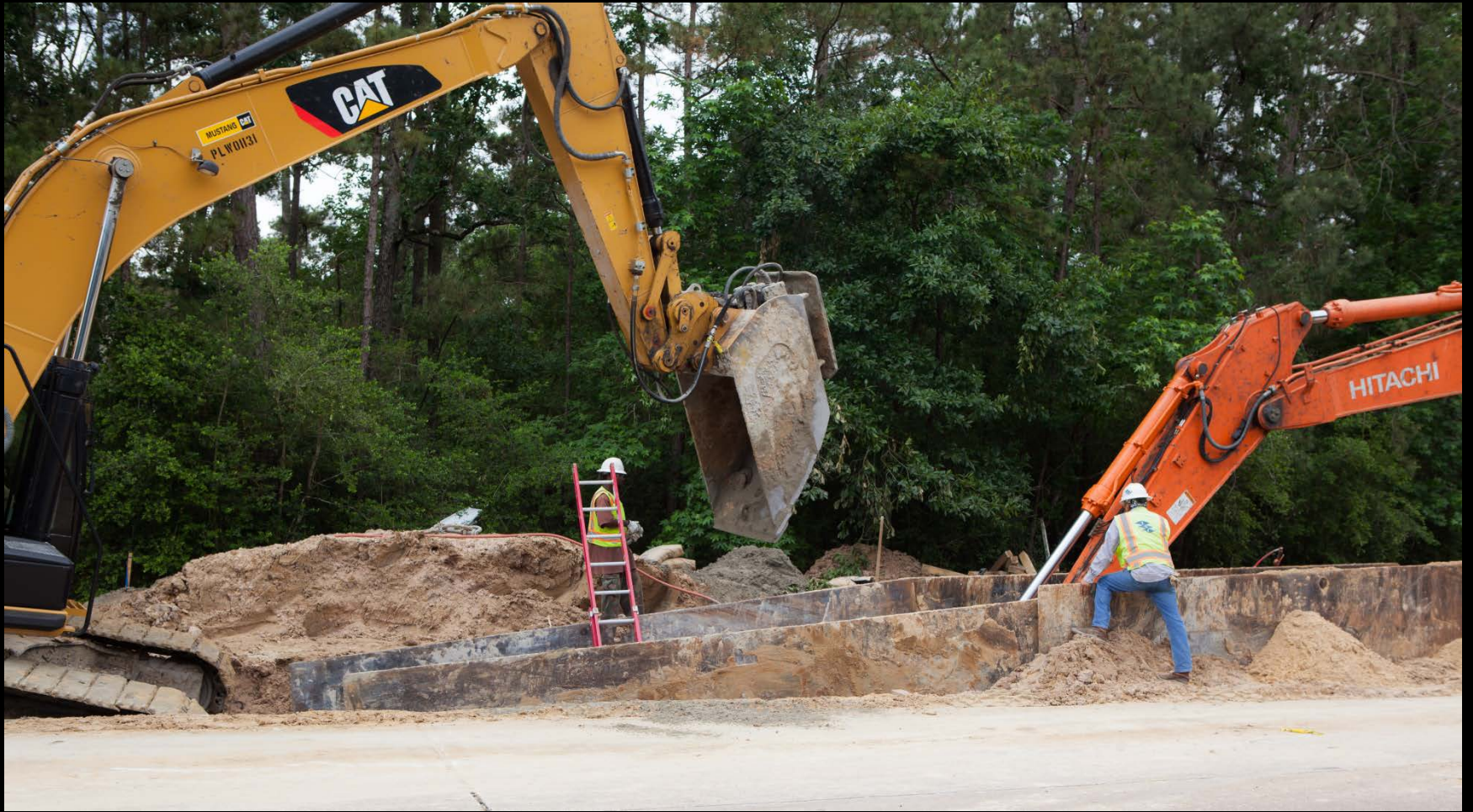
42-inch pipe installation along Research Forest Drive
