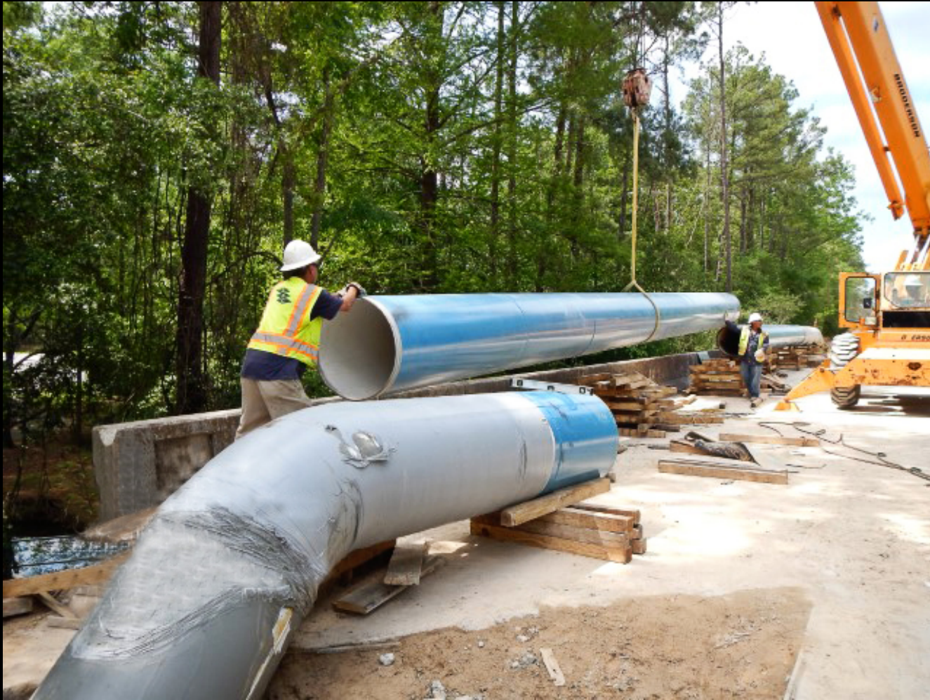
30-Inch aerial pipe installation on Grogan's Mill at bridge crossing
