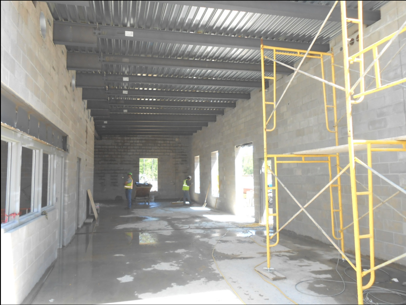
Operations Building – Previous progress photograph
