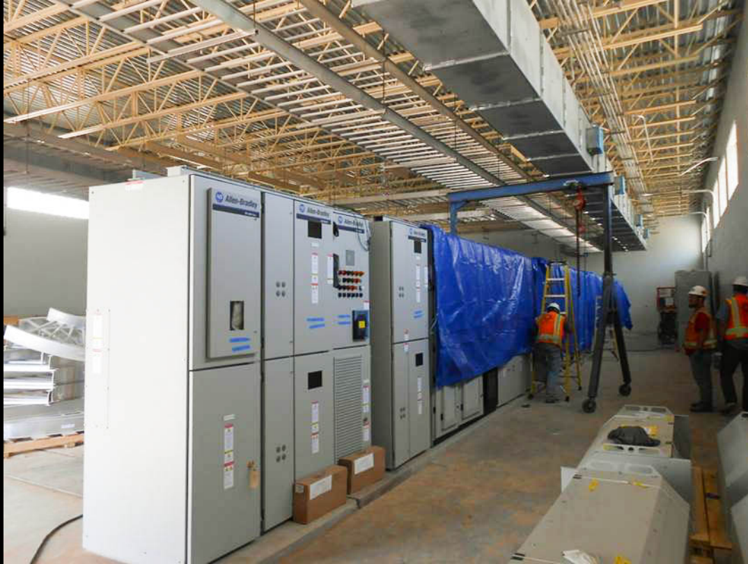
High Service Pump Station - Previous progress photograph
