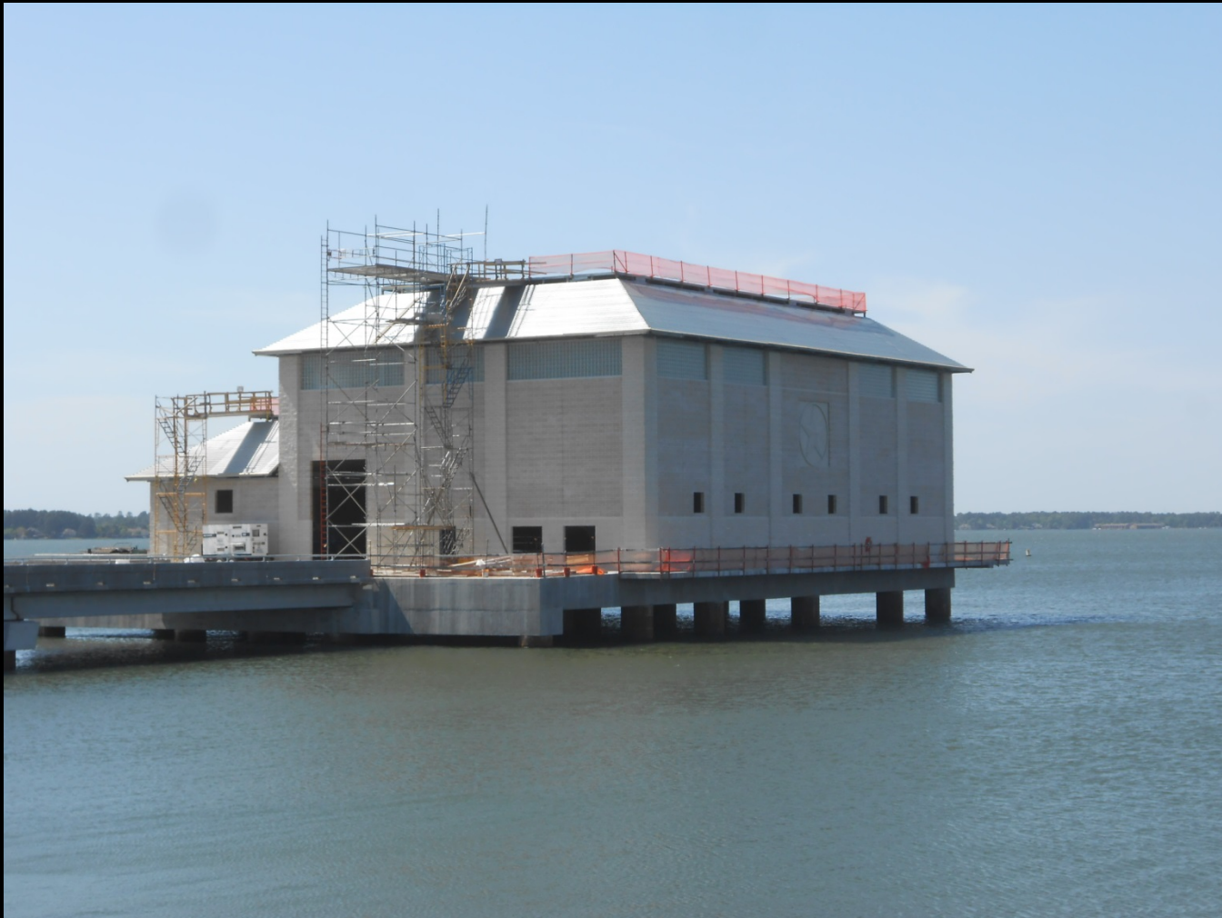
Raw Water Intake & Pump Station - Previous progress photograph
