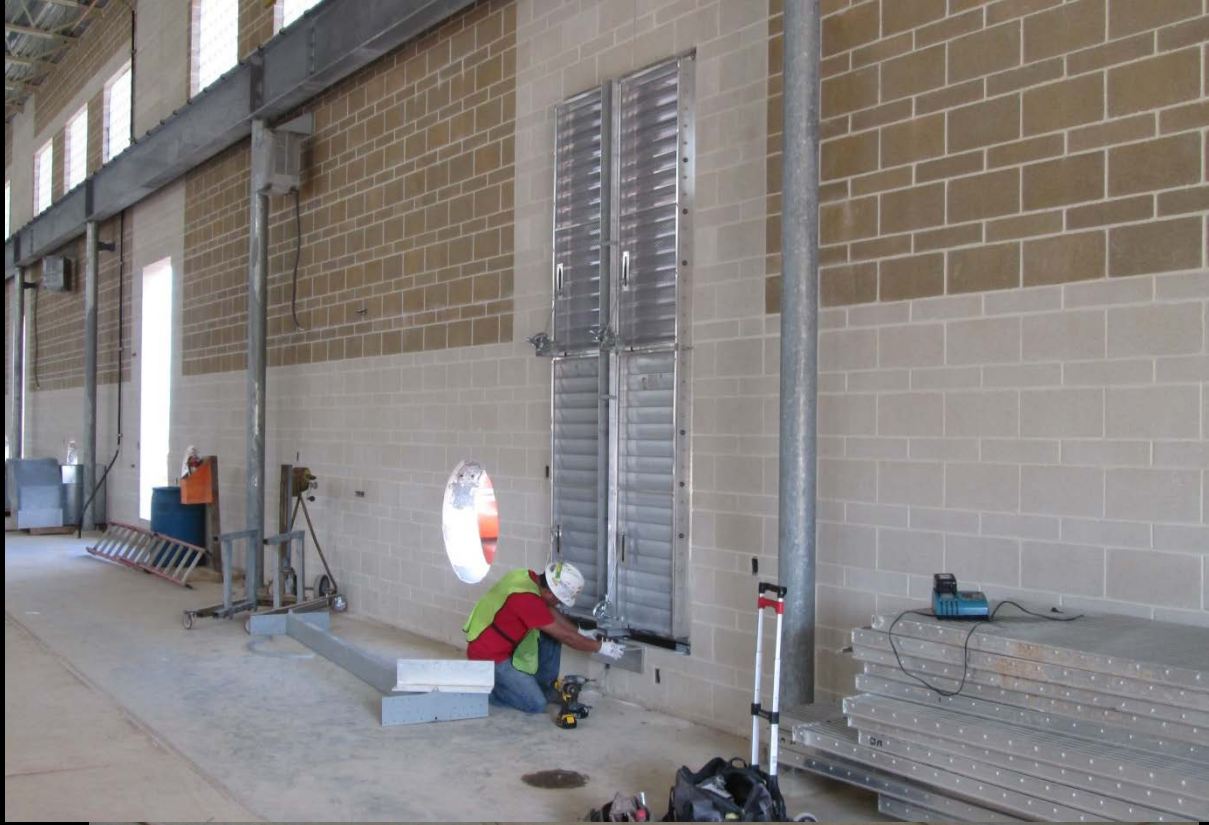
High Service Pump Station – Installation of mechanical louvers
