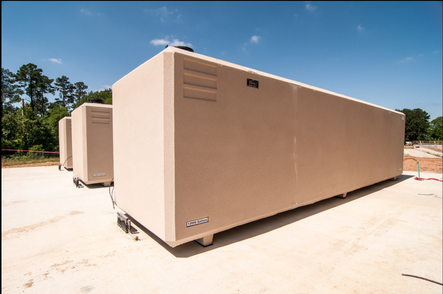
Electrical Facilities – Diesel fuel reservoirs
