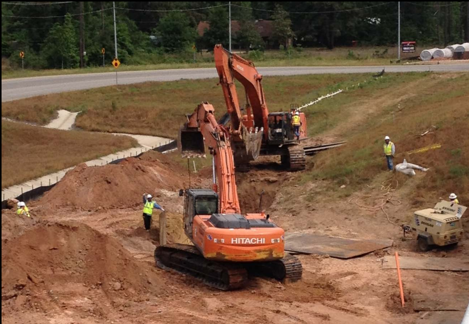
54-inch pipe installation at FM 2854
