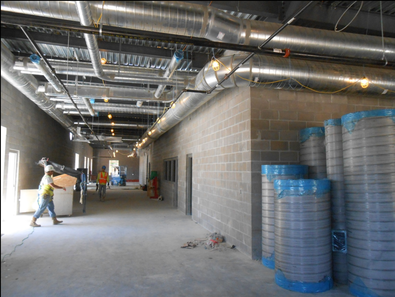
Operations Building – Mechanical and plumbing installation
