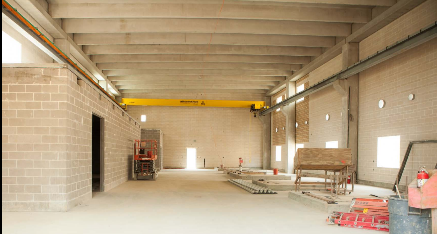
Blower Building – Cleaning and preparation for blower equipment installation
