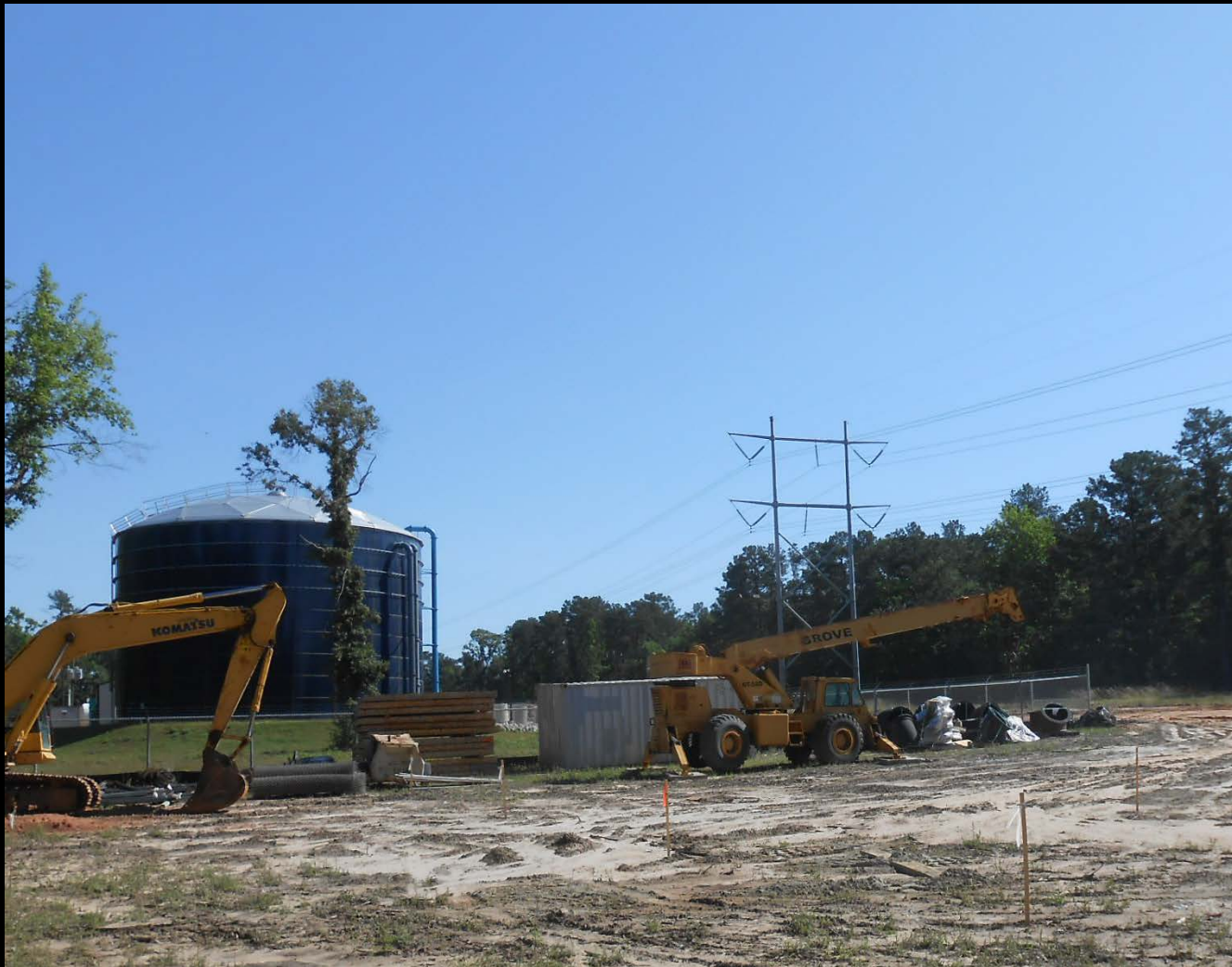
Equipment mobilization and delivery of construction materials
