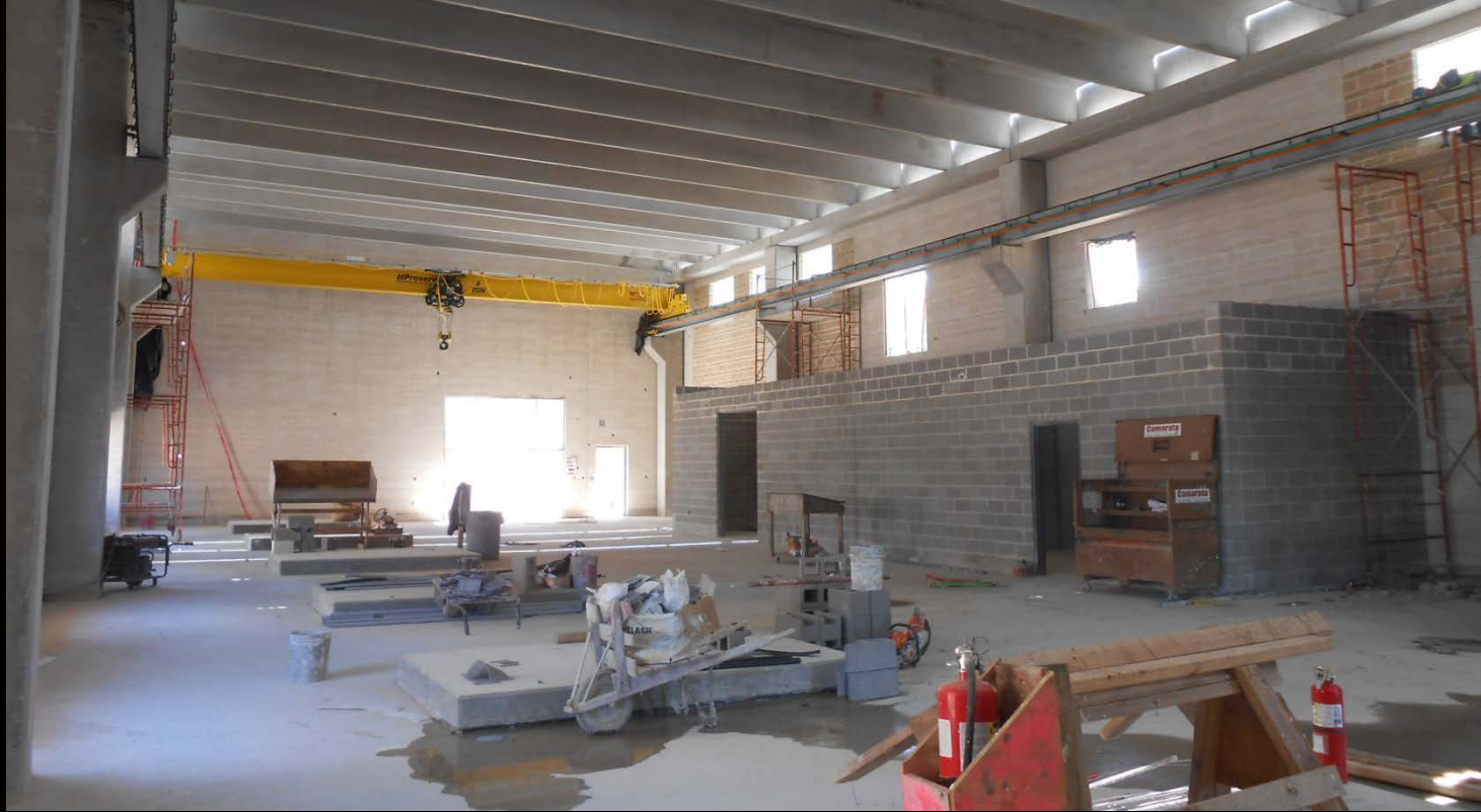
Blower Building – Previous progress photograph
