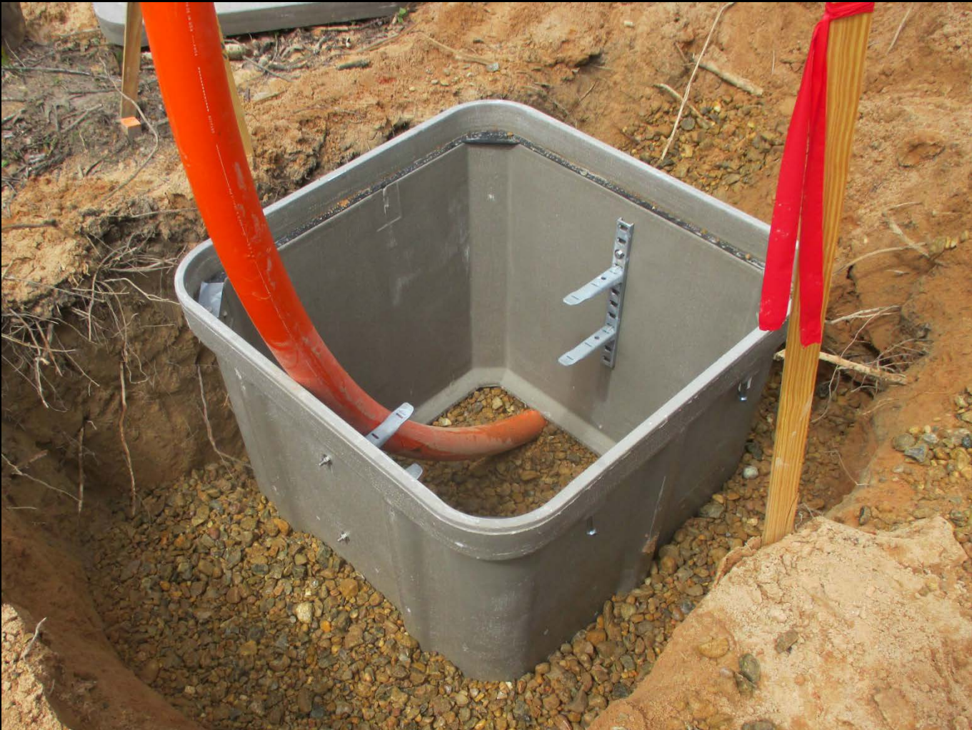
Ground box and fiber optic conduit installation
