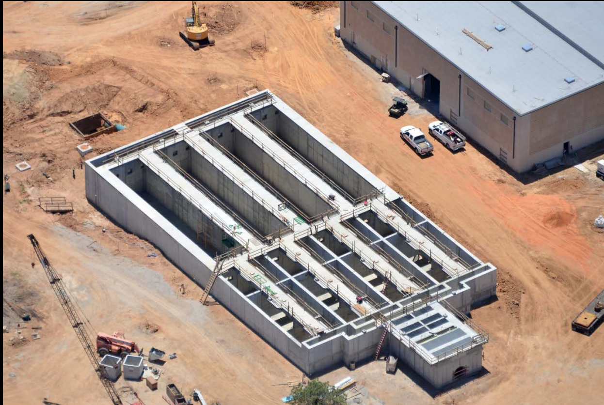
Pretreatment Facility – Preparation of equipment installation
