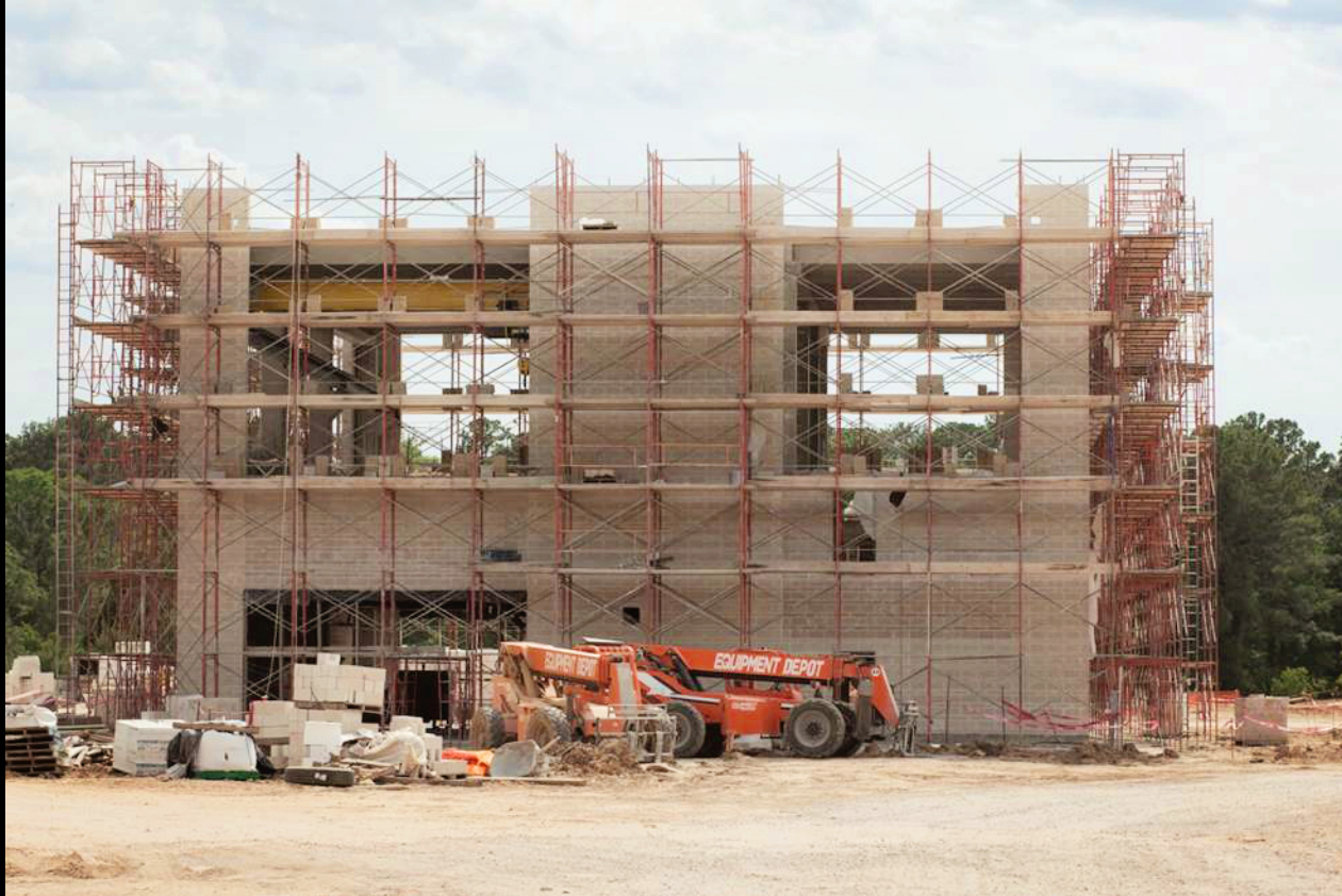
Dewatering Building – Masonry installation
