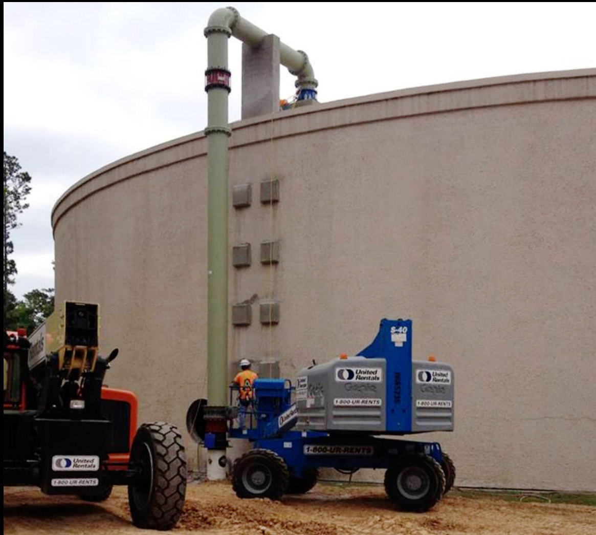
20-inch ground storage tank connection at SJRA Water Plant No. 4
