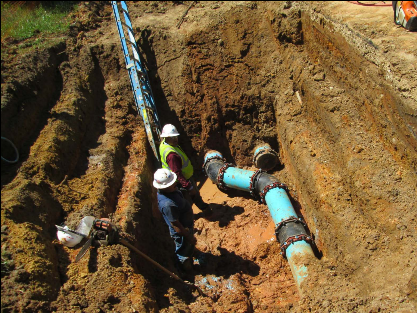
12-inch water line relocation at the intersection of Branch Crossing and Research Forest
