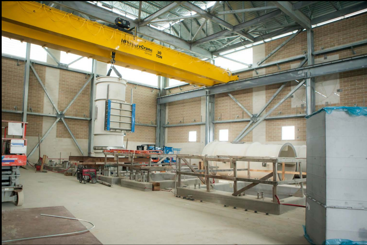
Raw Water Intake & Pump Station – Pump barrel installation
