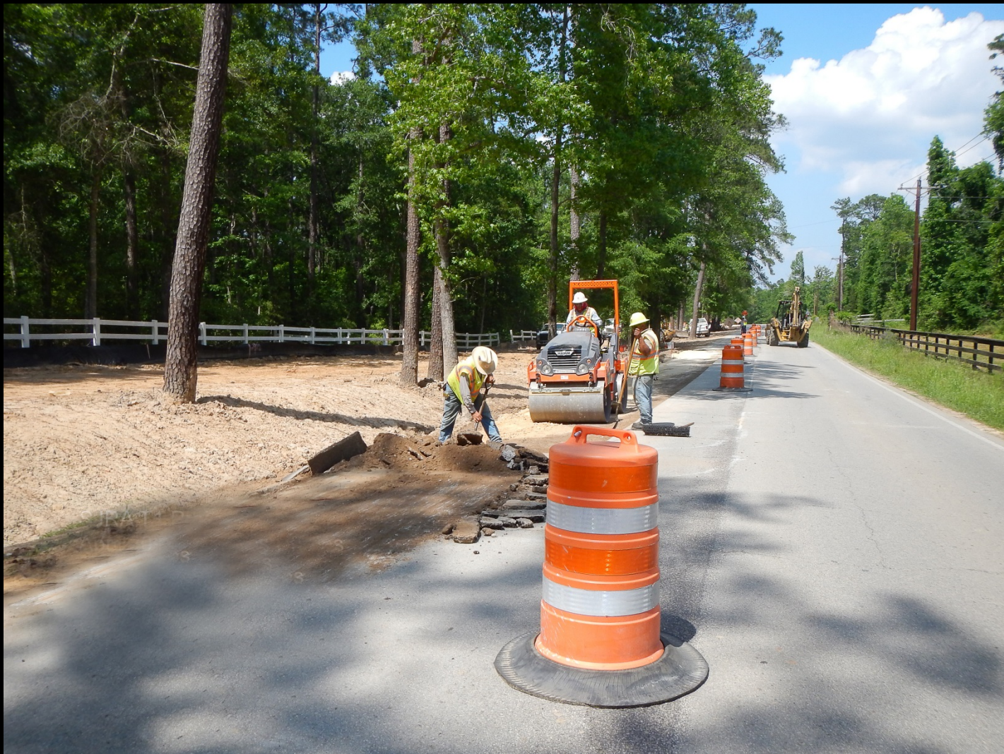
Asphalt pavement repairs along McCaleb Road
