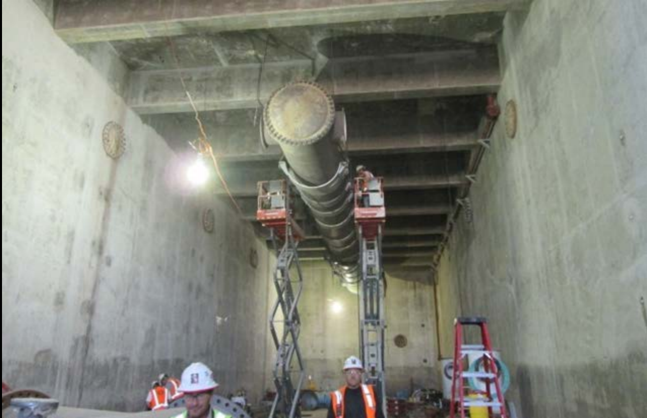
Granulated Activated Carbon Contactors – Pipe gallery installation
