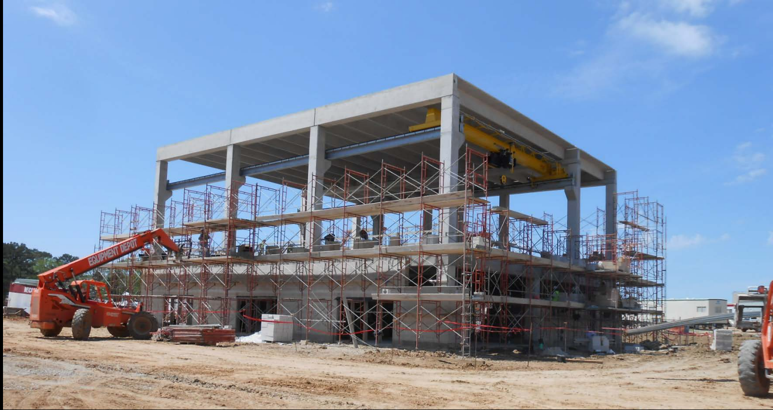
Dewatering Building – Previous progress photograph
