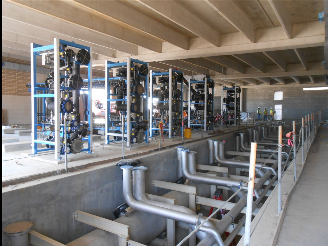
Membrane Building – Previous progress photograph
