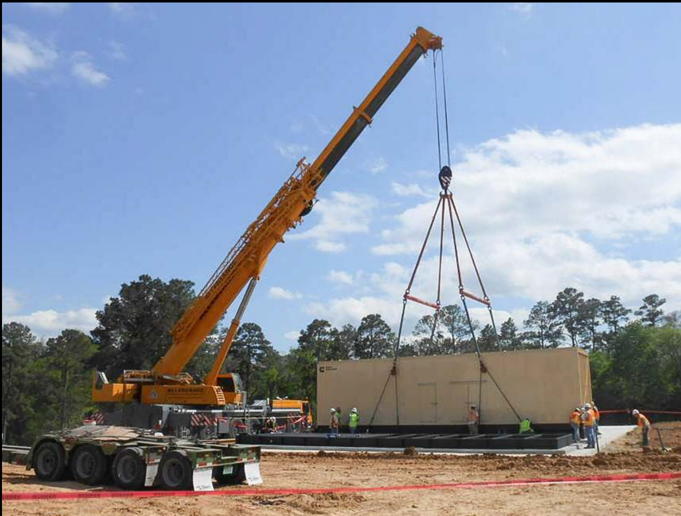
Electrical Facilities – Previous progress photograph
