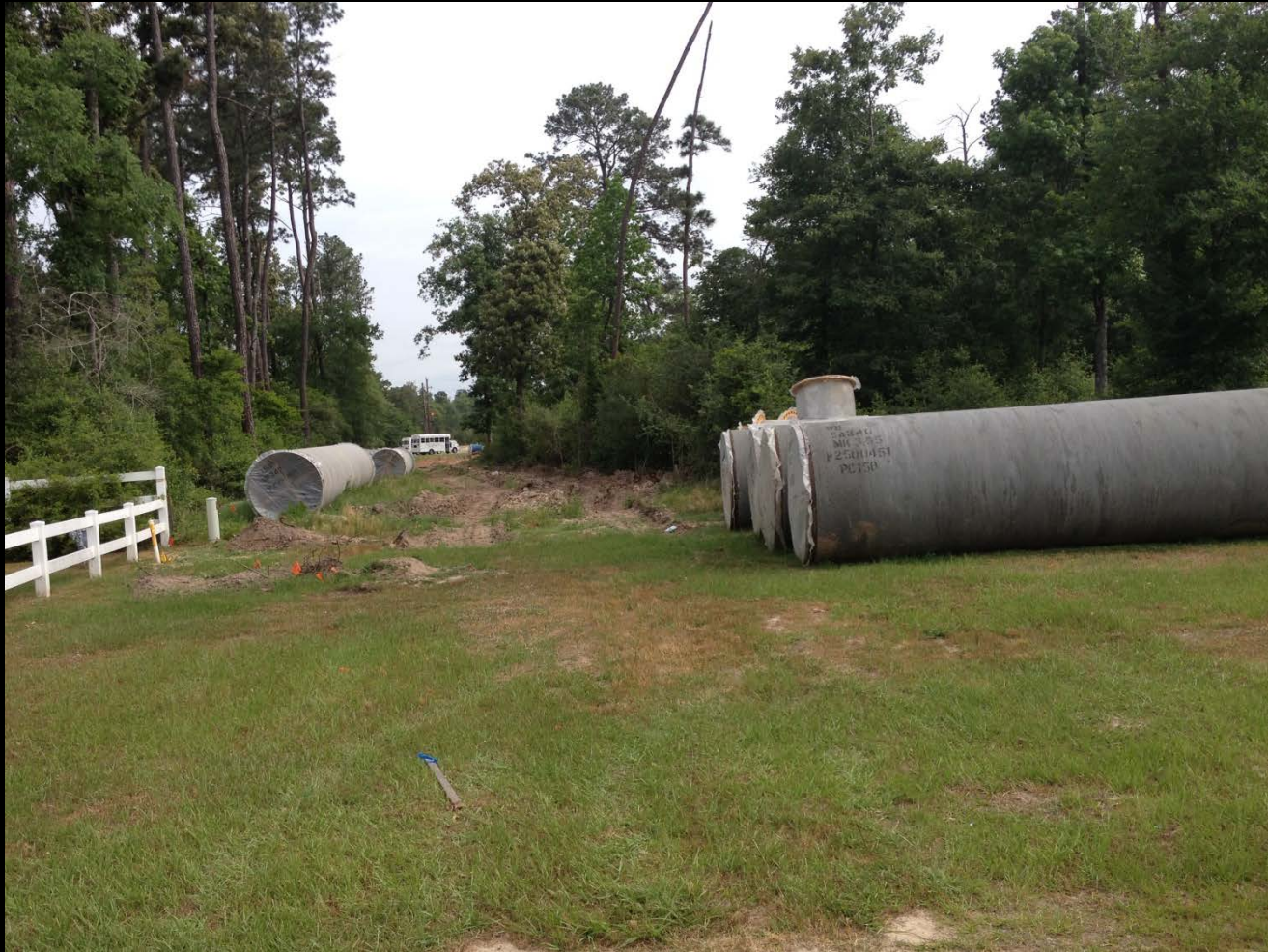
54-inch pipe installation along Sendera Ranch Road
