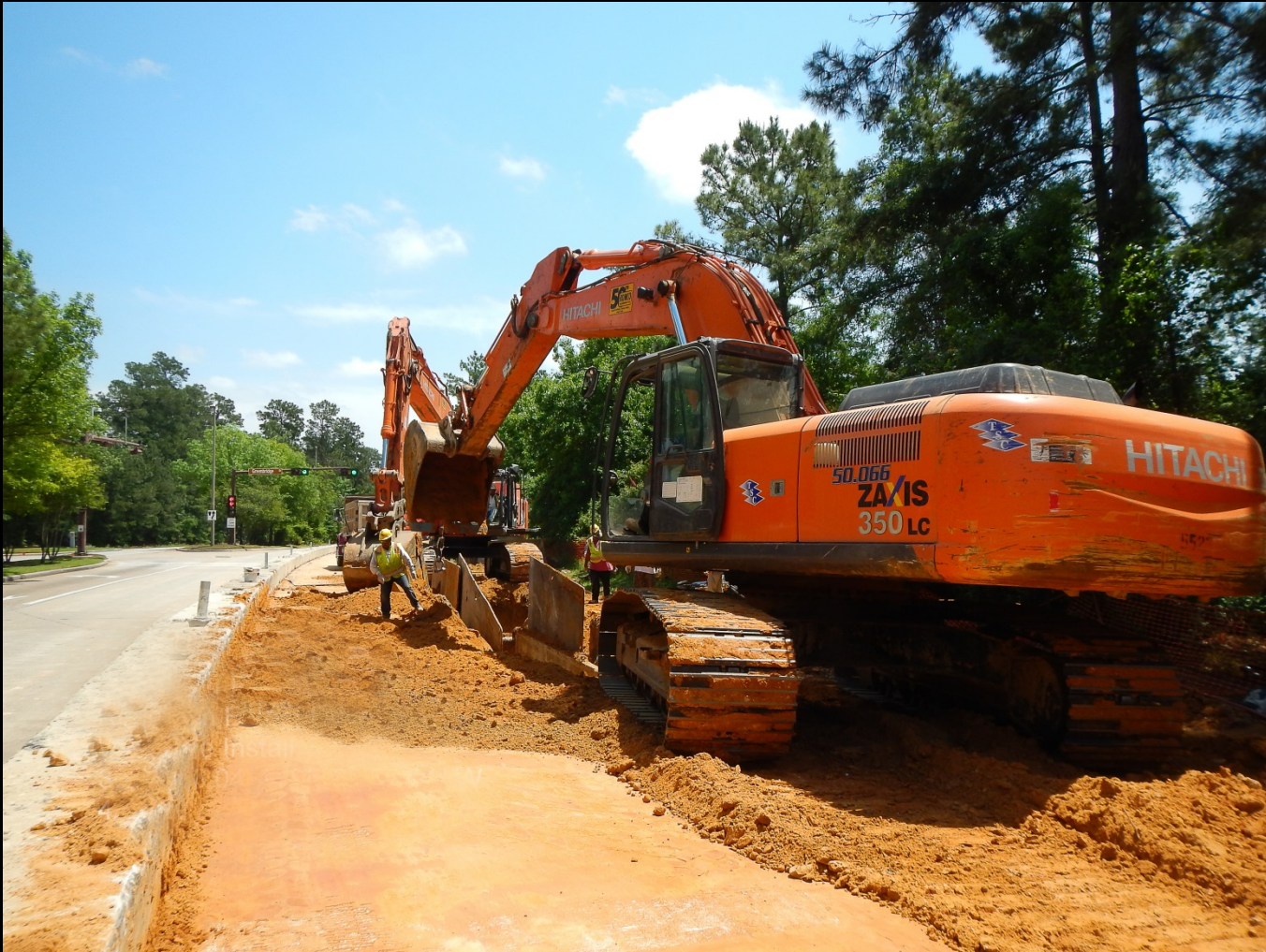
42-inch pipe installation along Research Forest Drive
