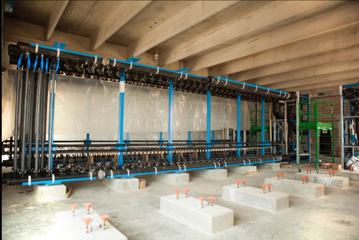
Membrane Building – Installation of membrane equipment racks and piping
