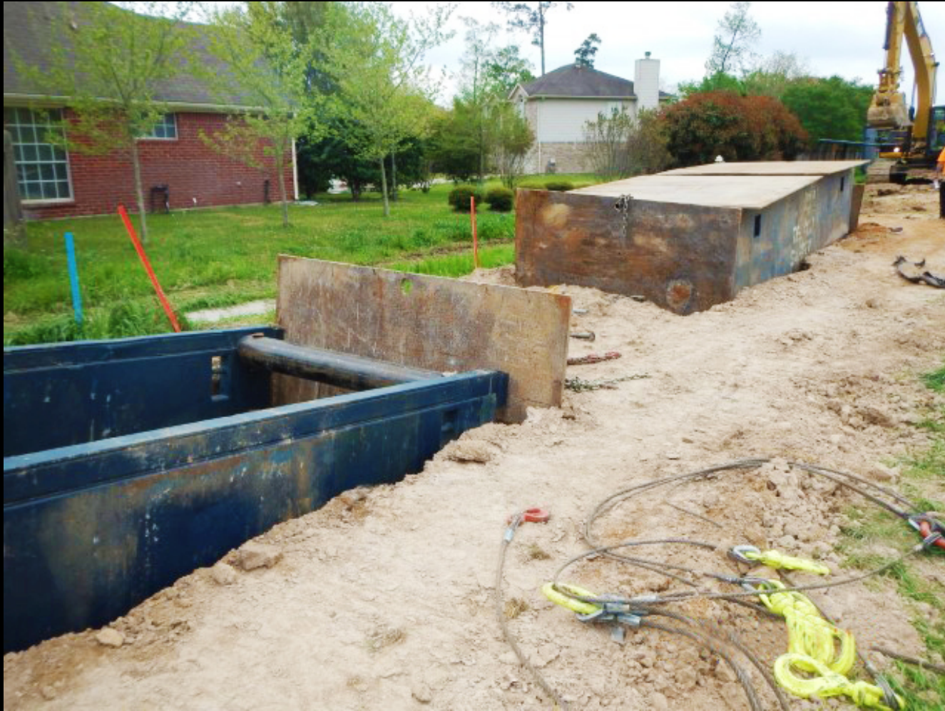
Pipe installation along Montgomery County Drainage District right-of-way
