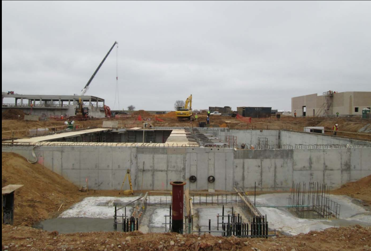
Backwash Equalization Basin— Previous progress photograph
