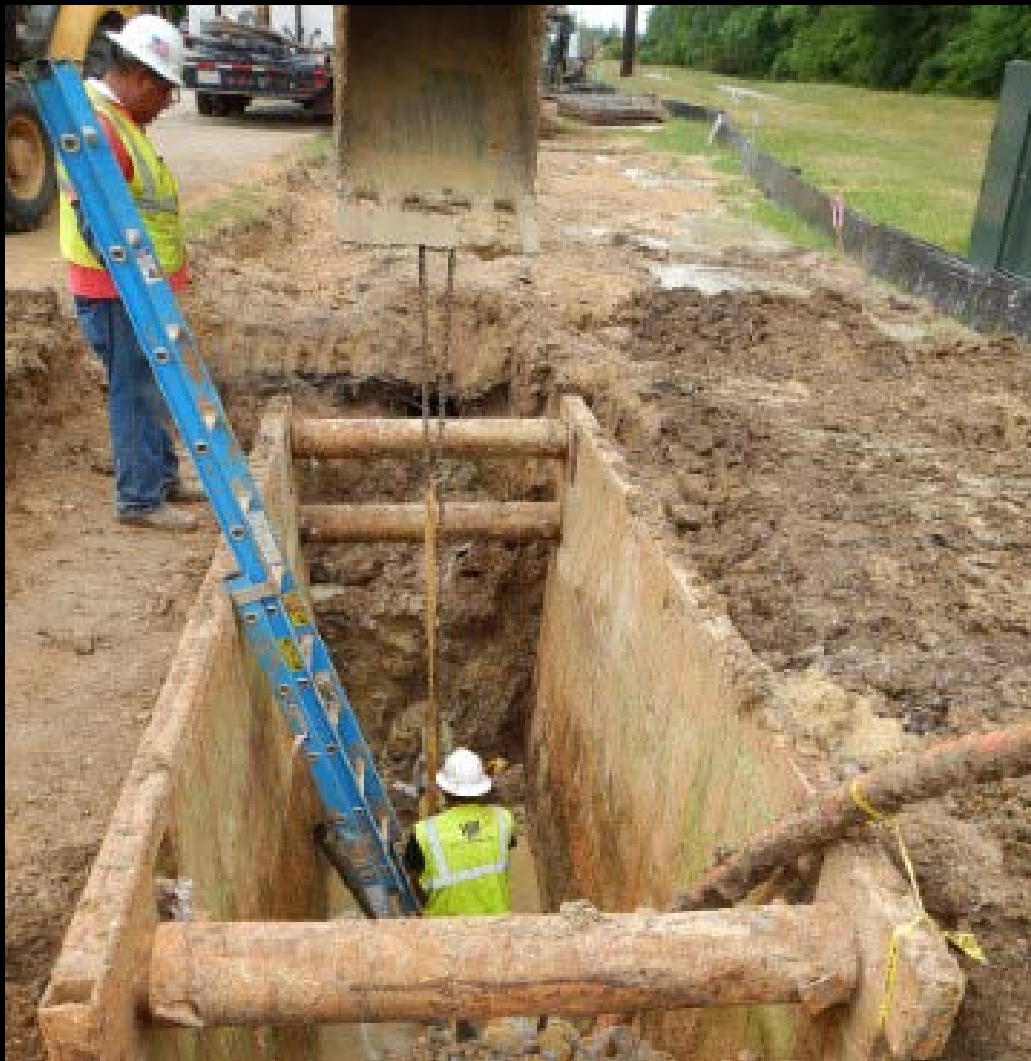
24-inch pipe and fiber optic conduit installation on Gosling
