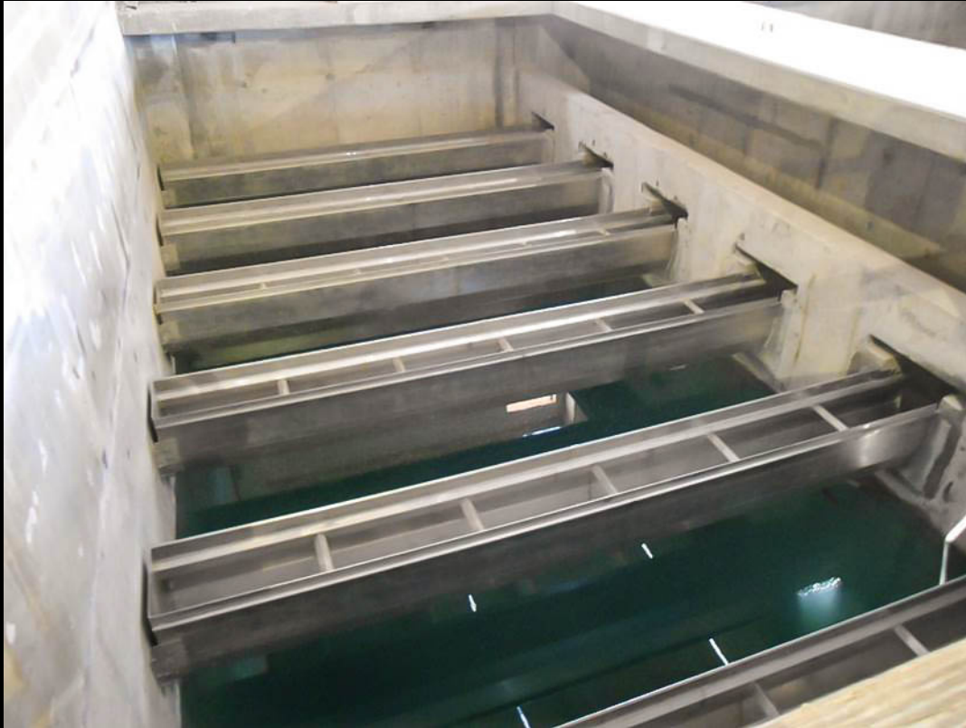
Granulated Activated Carbon Contactors – Previous progress photograph
