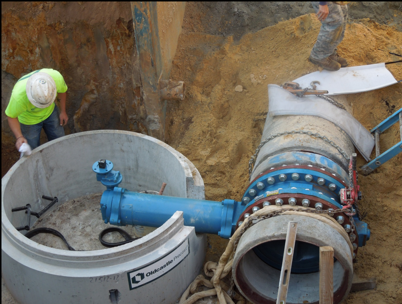
Butterfly valve installation along Entergy easement
