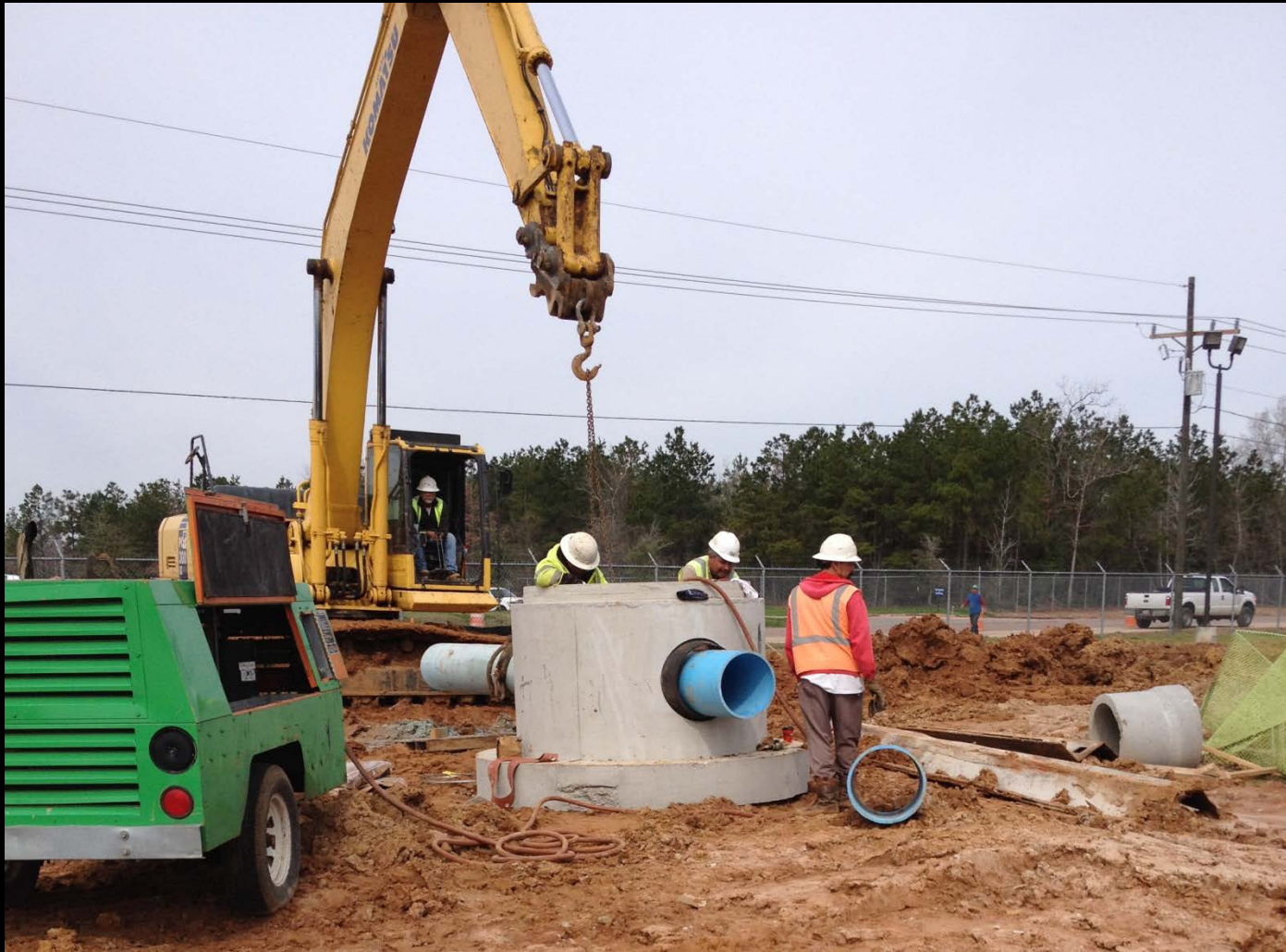
Valve access manhole installation at Conroe Water Plant No. 20
