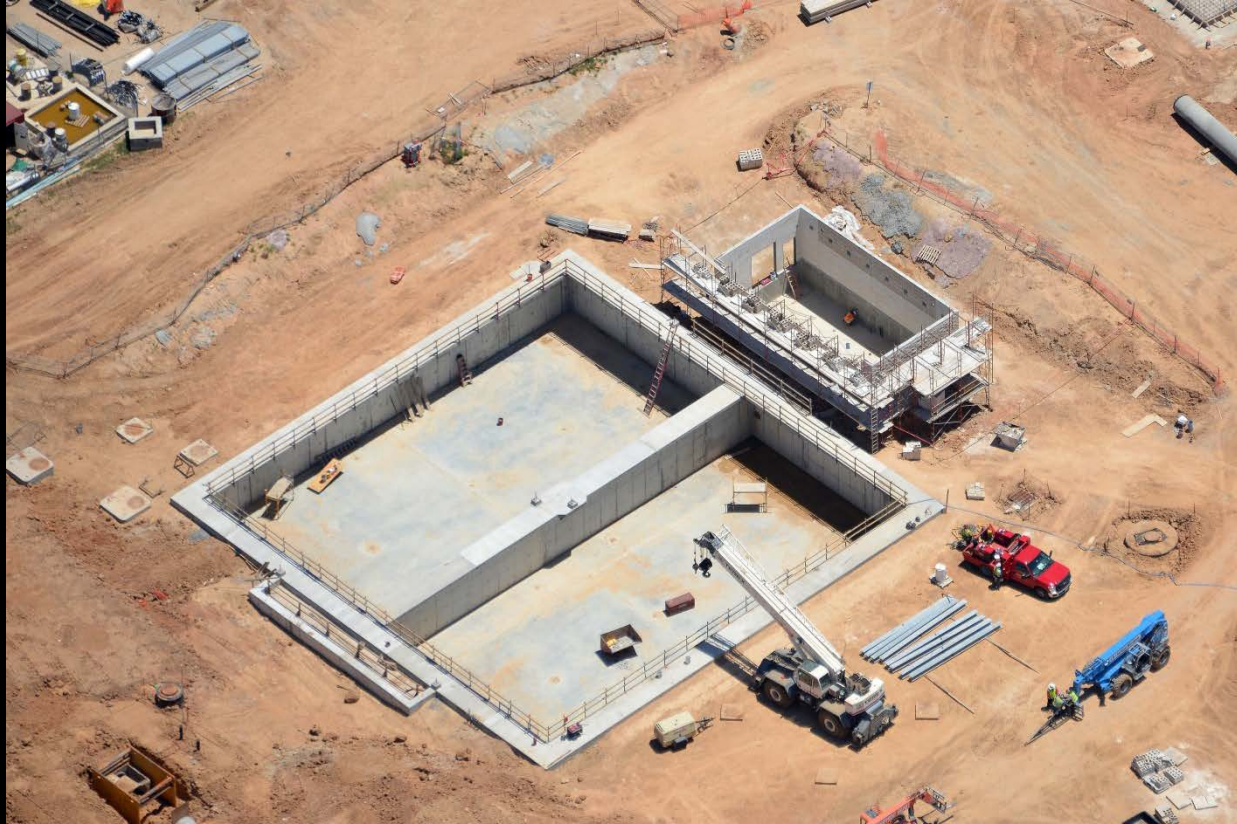
Backwash Equalization Basin— Pump Station masonry installation
