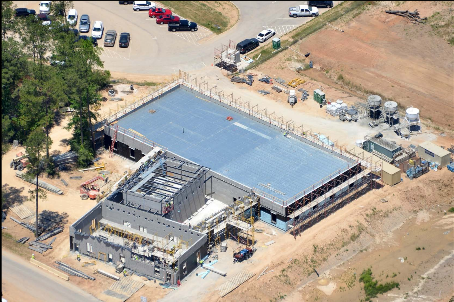
Operations Building – Roof framing and masonry installation
