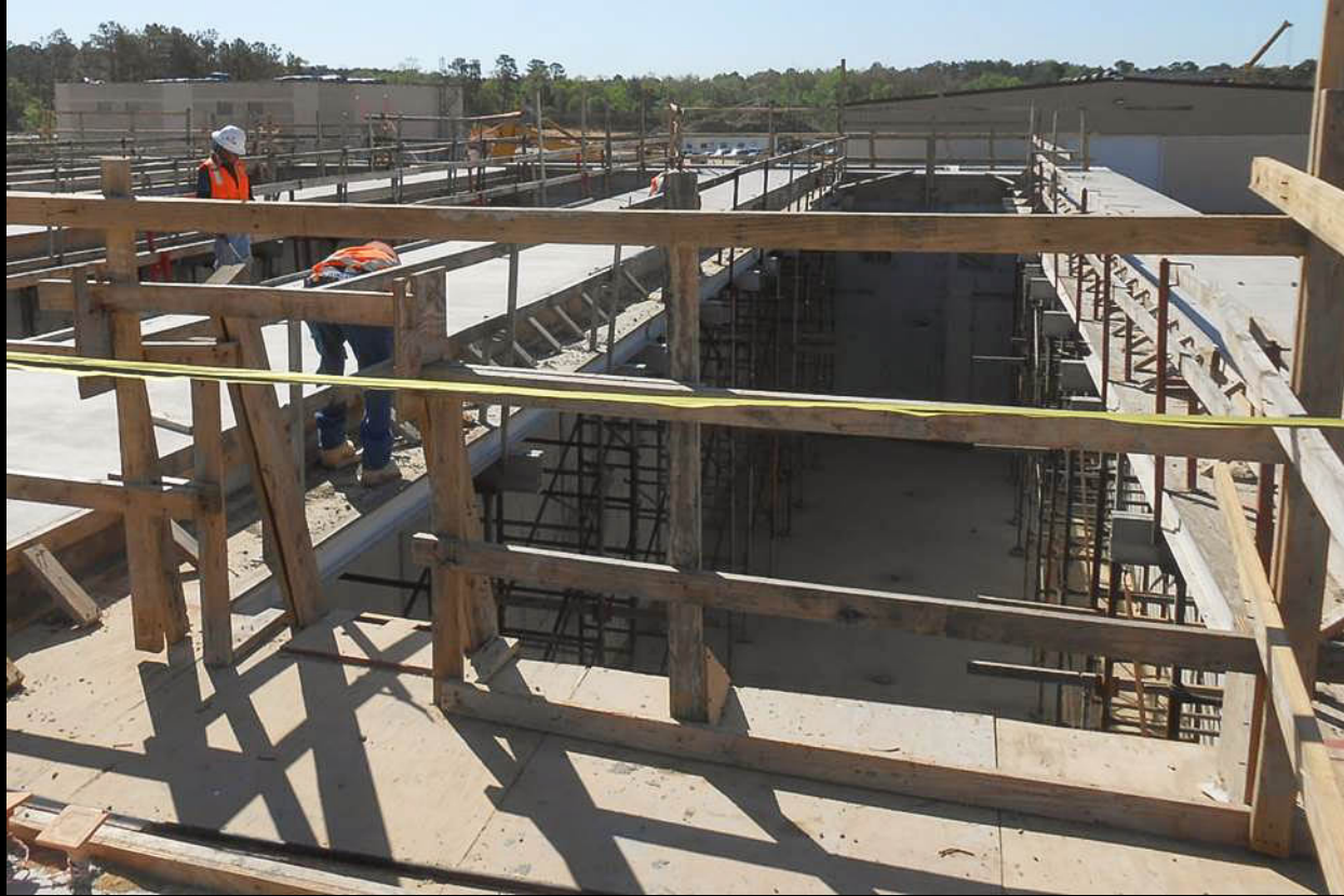
Pretreatment Facility – Previous progress photograph
