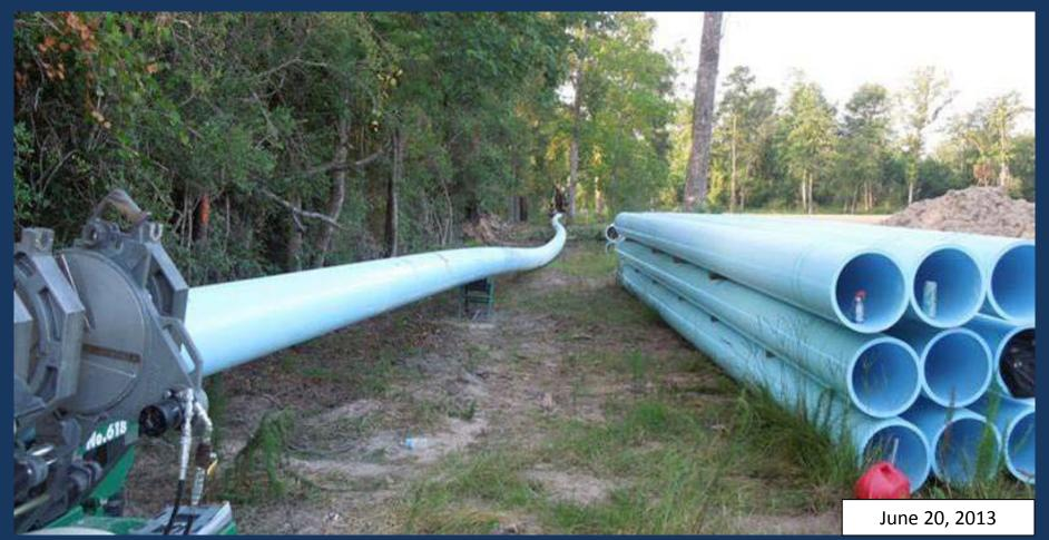
Fusing of 16" fusible PVC water line at FM2978
