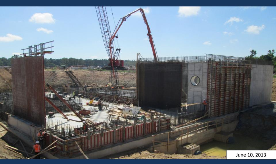
Lower foundation concrete placement at the GAC Building
