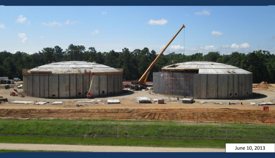
Installation of wall and roof panels at GST1 and GST2
