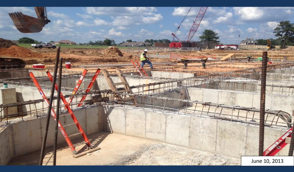
Grade beam installation at Membrane Building
