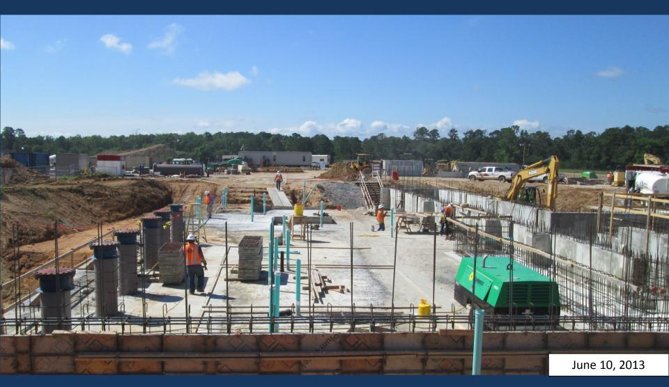
Seal slab at Pump Room in the Membrane Building
