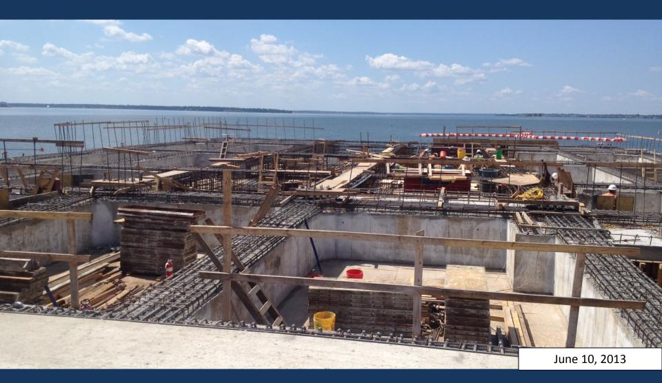
Rebar and formwork installation for the building foundation
