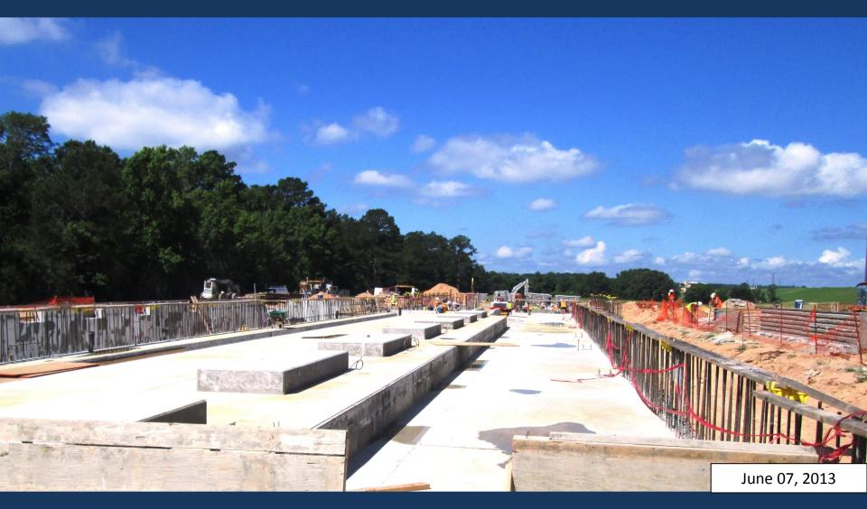
Slab on grade complete at the Pump Room
