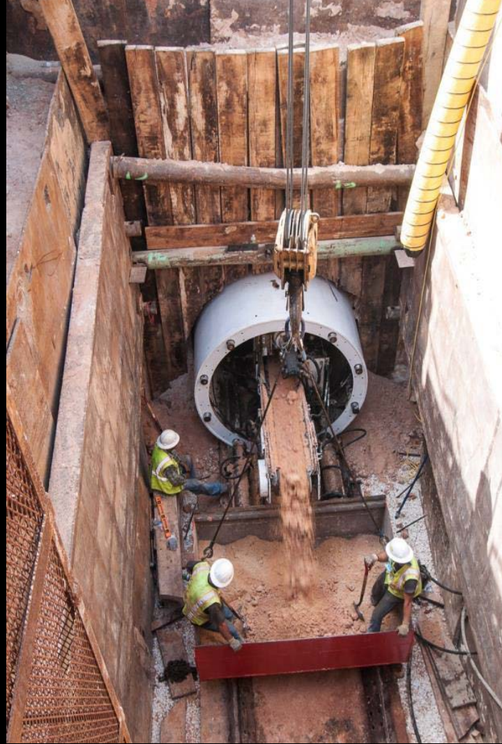
Tunnel boring machine in operation
