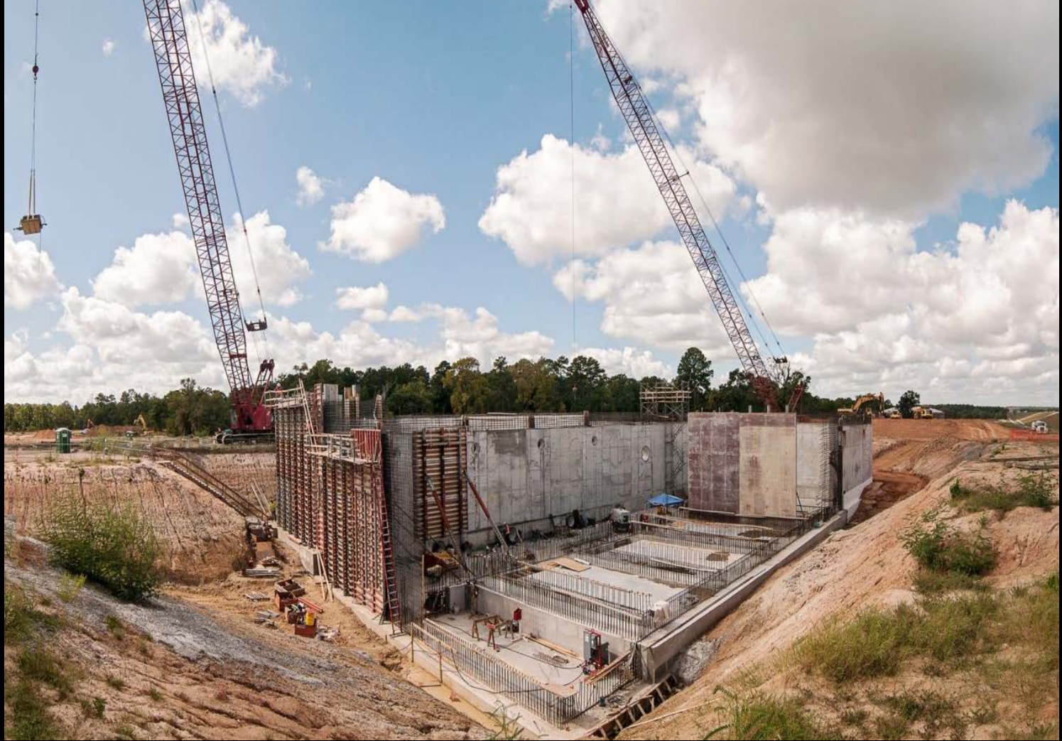
Lower foundation and concrete wall installation at the GAC Building
