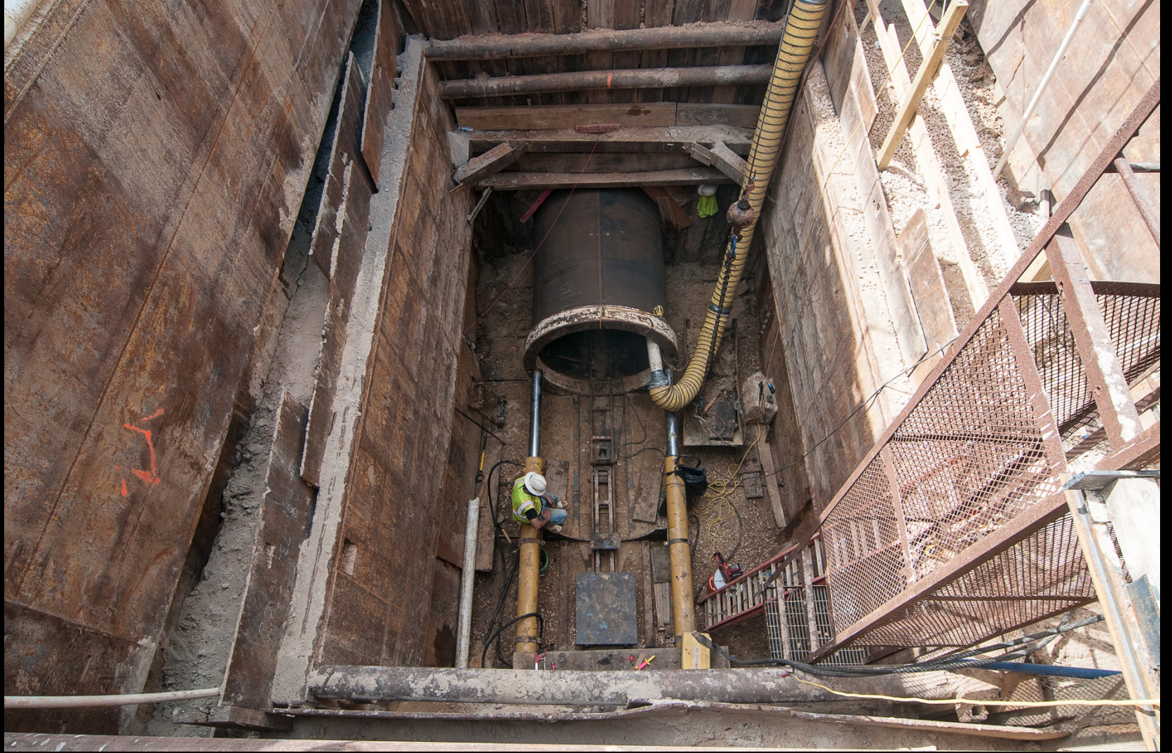
Jacking of steel casing
