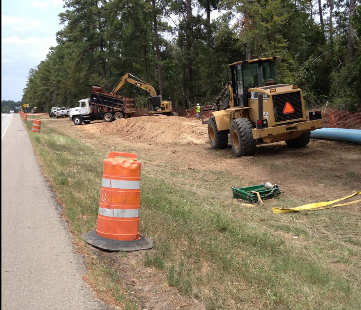
Water line installation along FM 2978
