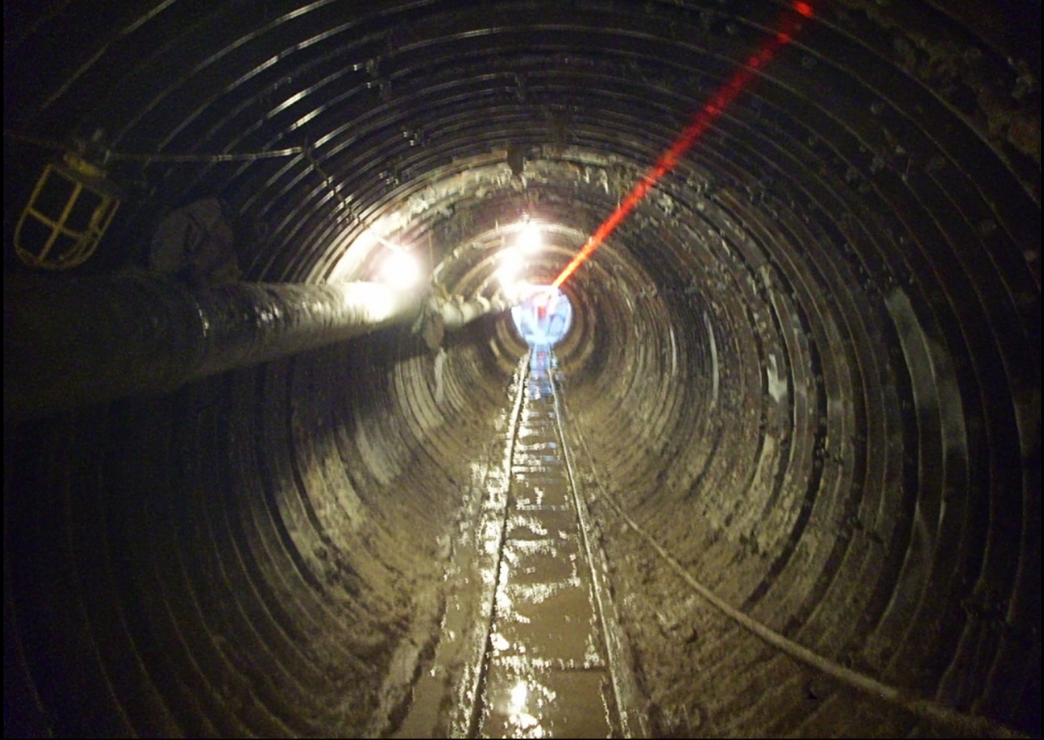
Interior view of tunnel – SH 105
