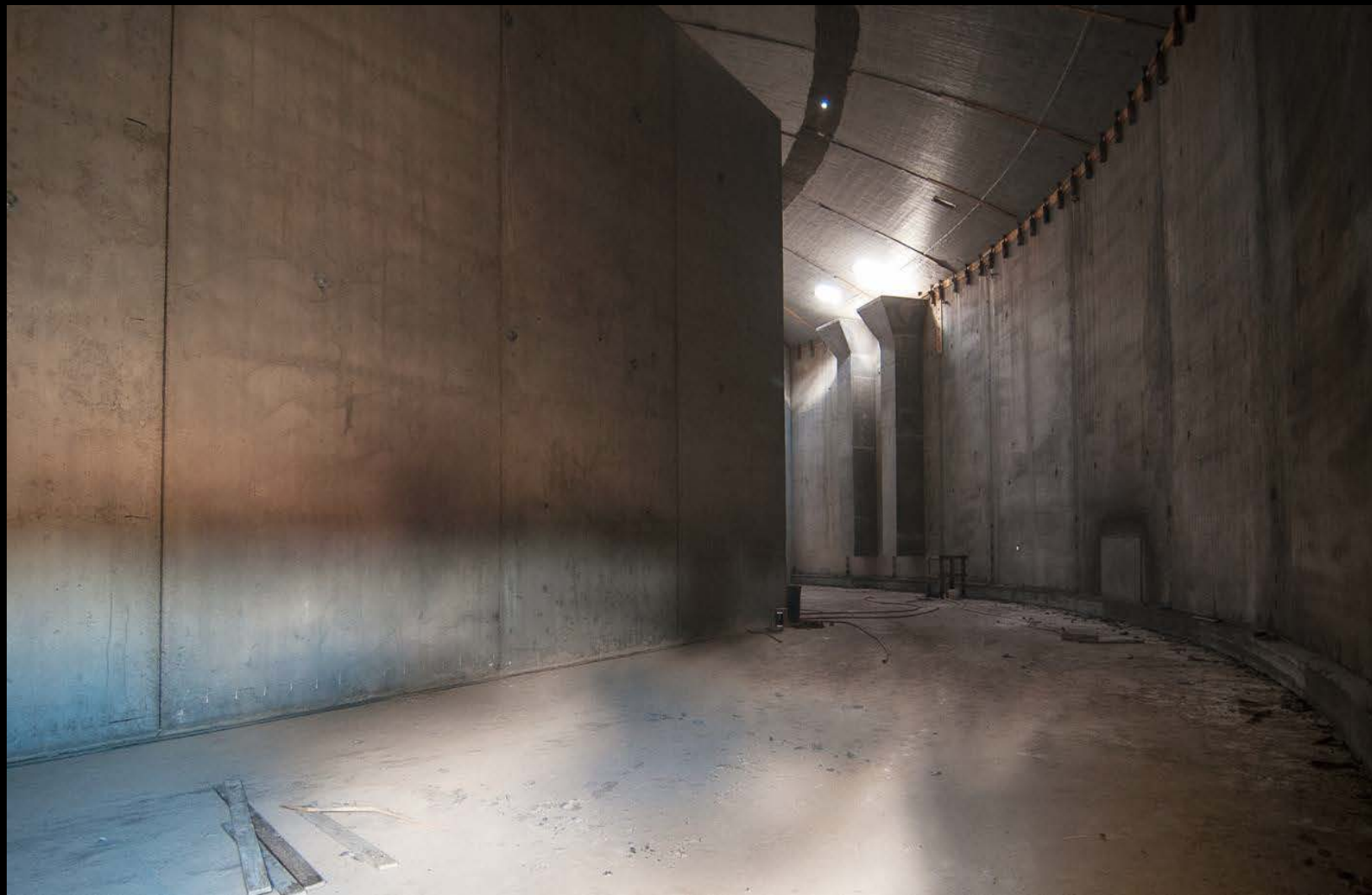
Interior tank view
