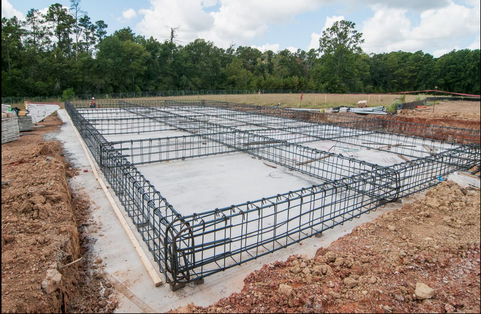
Seal slab complete with grade beam installation underway at the Generator structure
