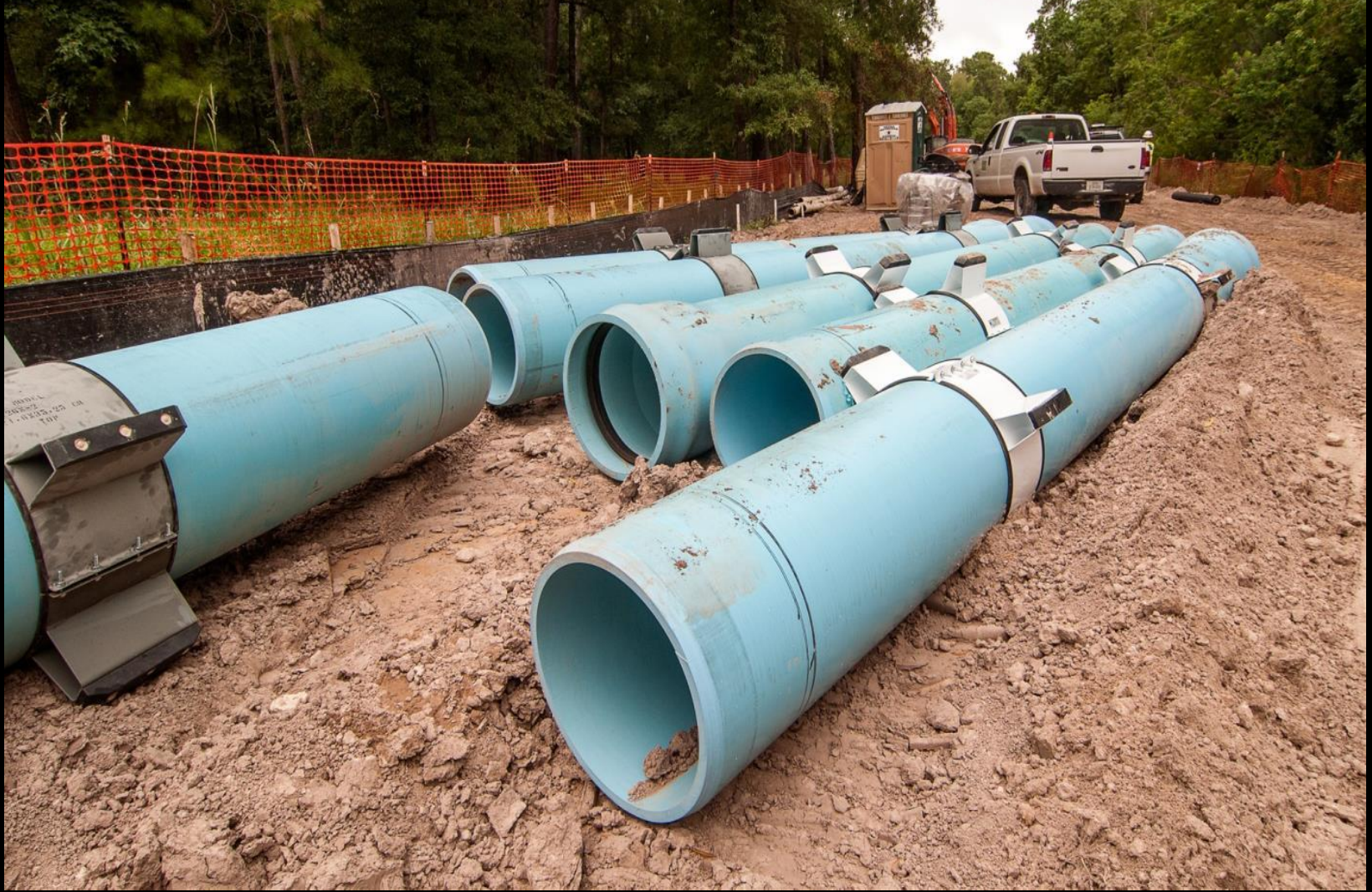
Staging of 20 inch PVC pipe along Kuykendahl Road extension
