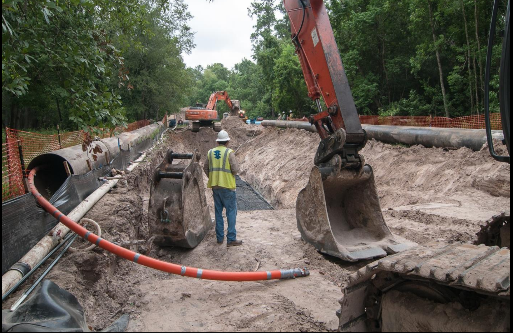
Open cut pipe installation at Kuykendahl Road extension
