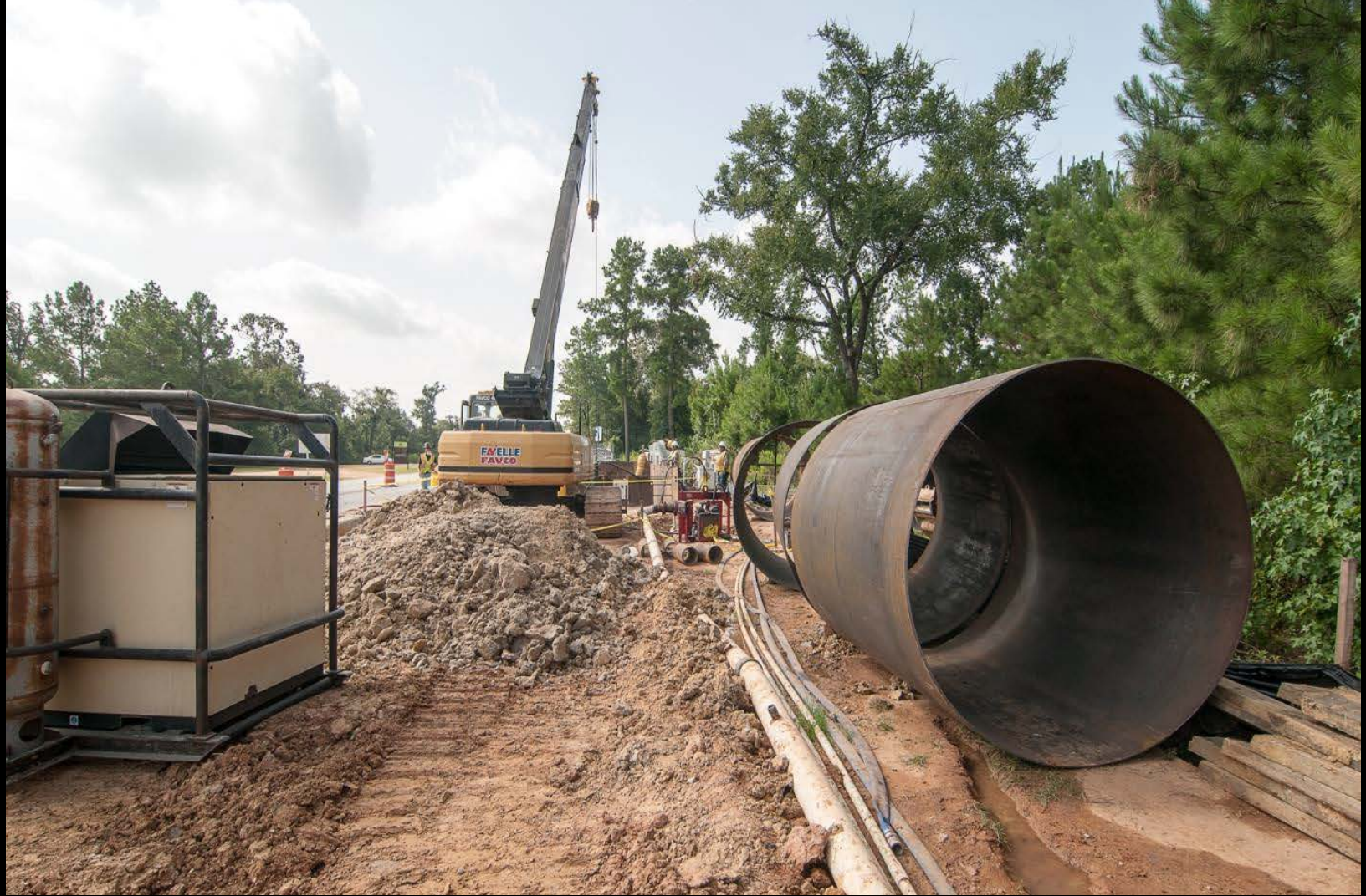
Steel casing for tunnel section
