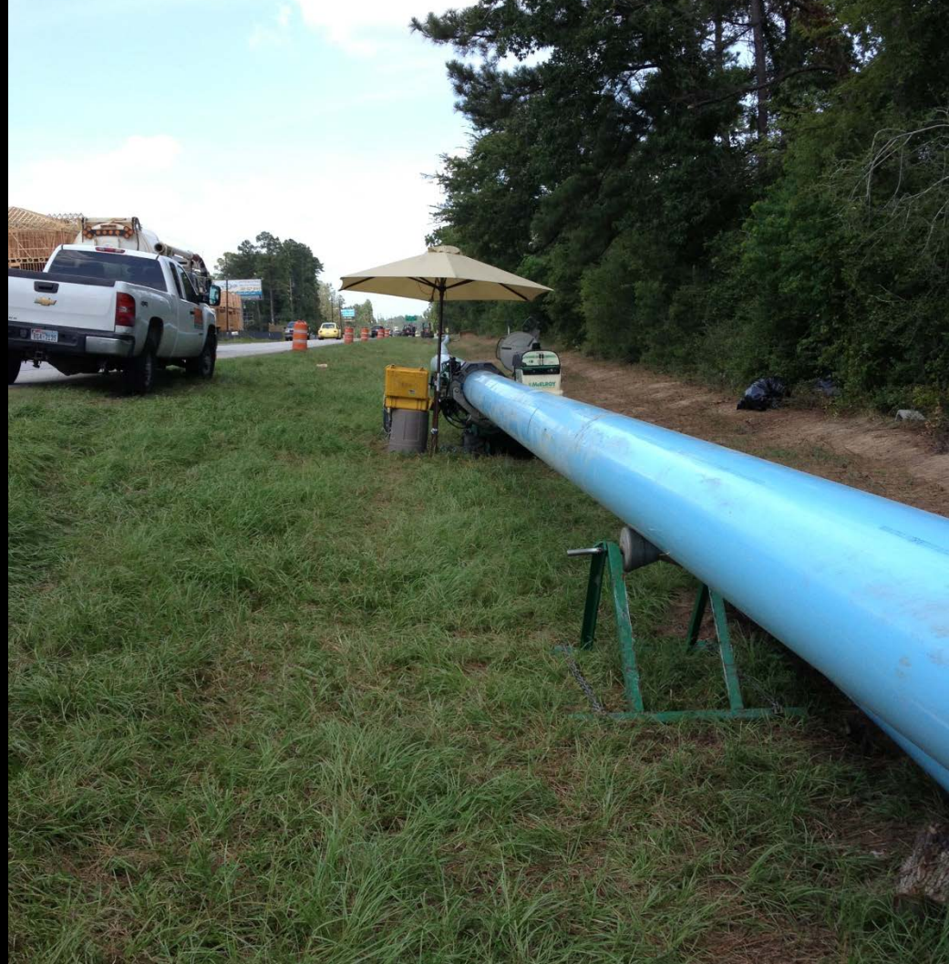
Fusing 16 inch PVC Pipe – FM 2978
