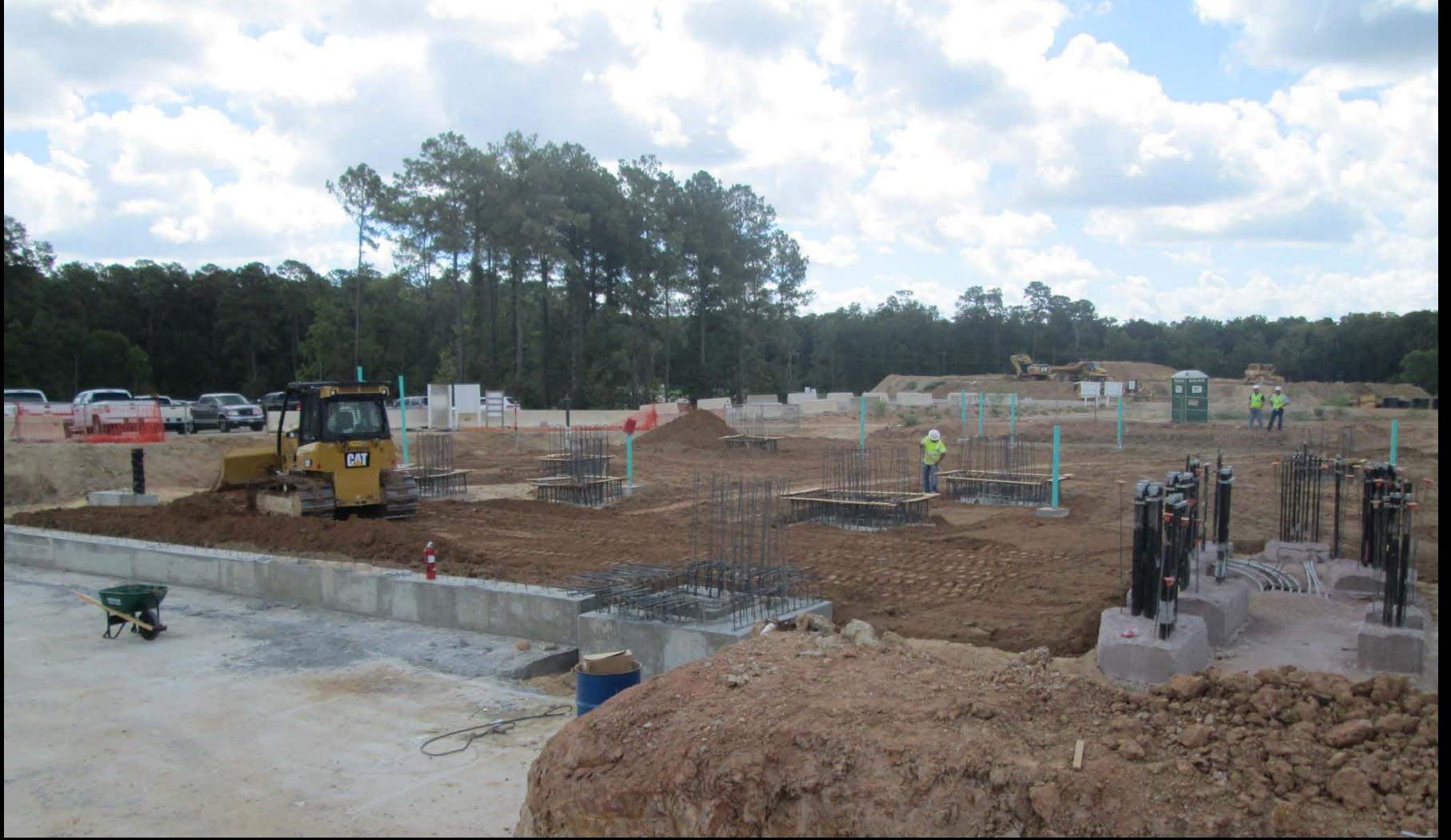
Select fill installation at the Chemical Facility
