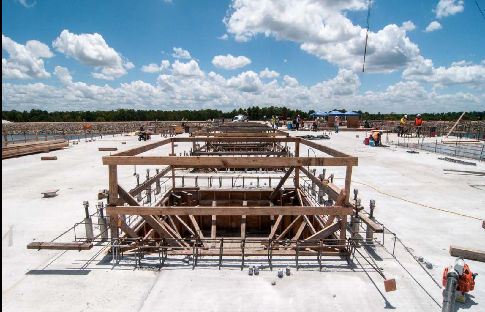
Pump foundation complete
