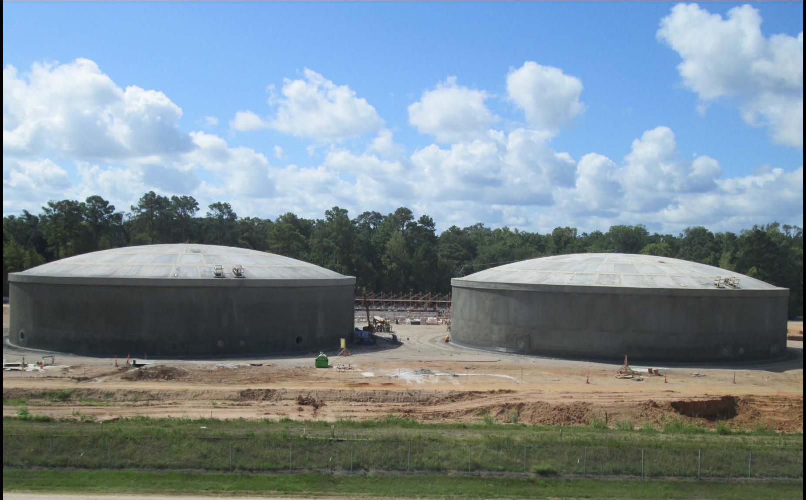
Wire winding complete
