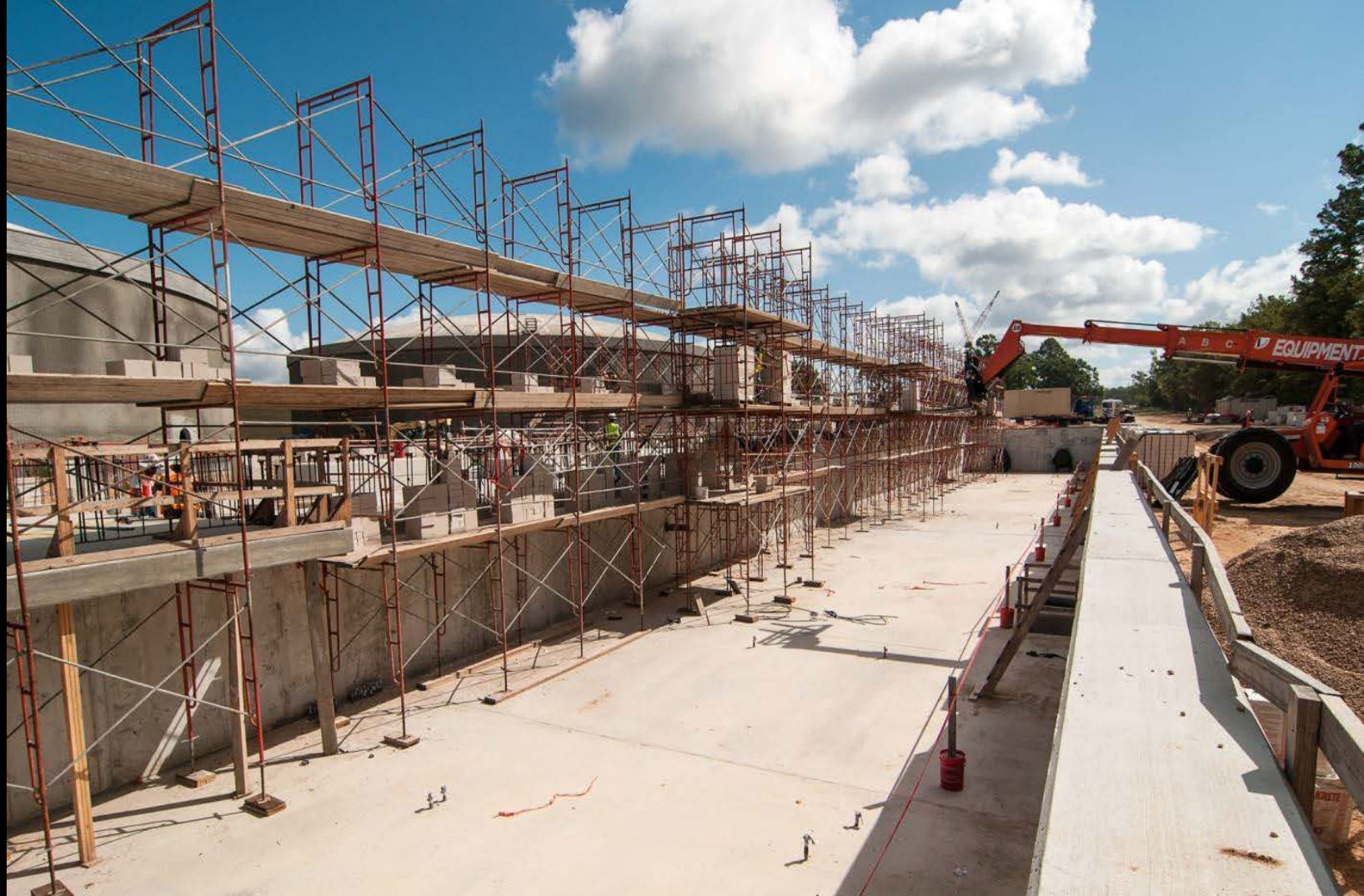
Exterior masonry installation
