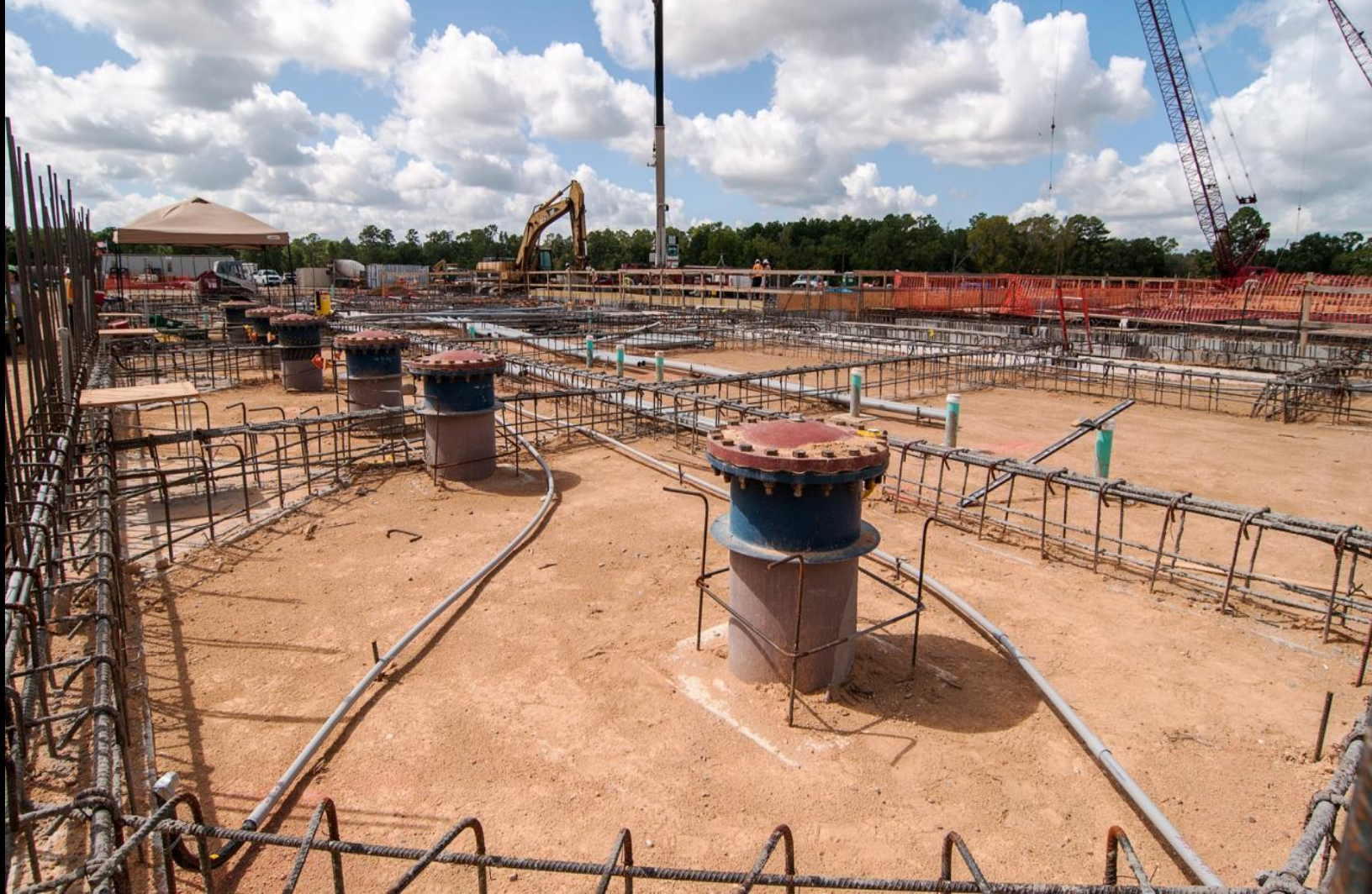
Foundation backfill complete at Membrane Building
