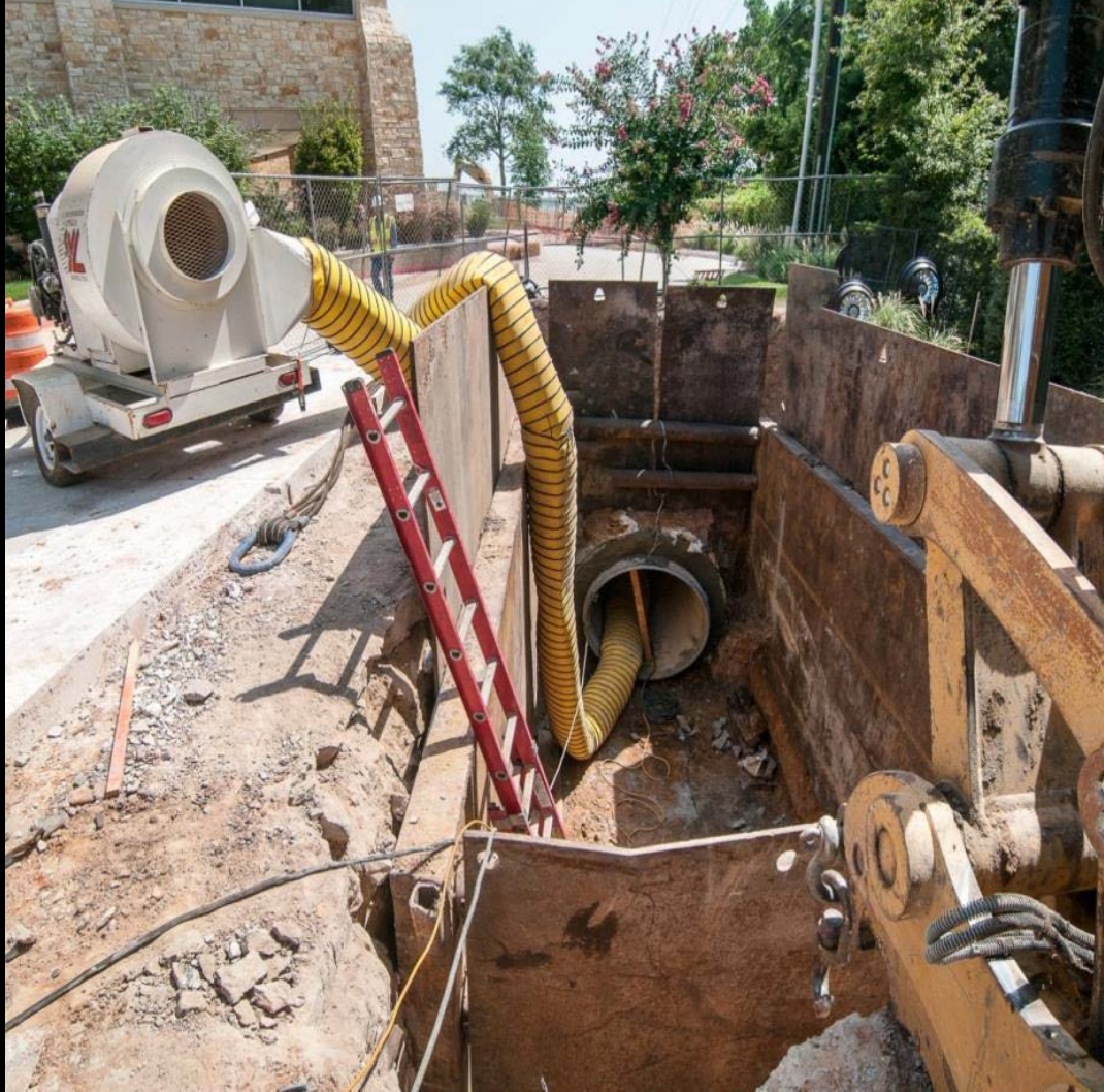
Tunnel operation - G&A parking lot
