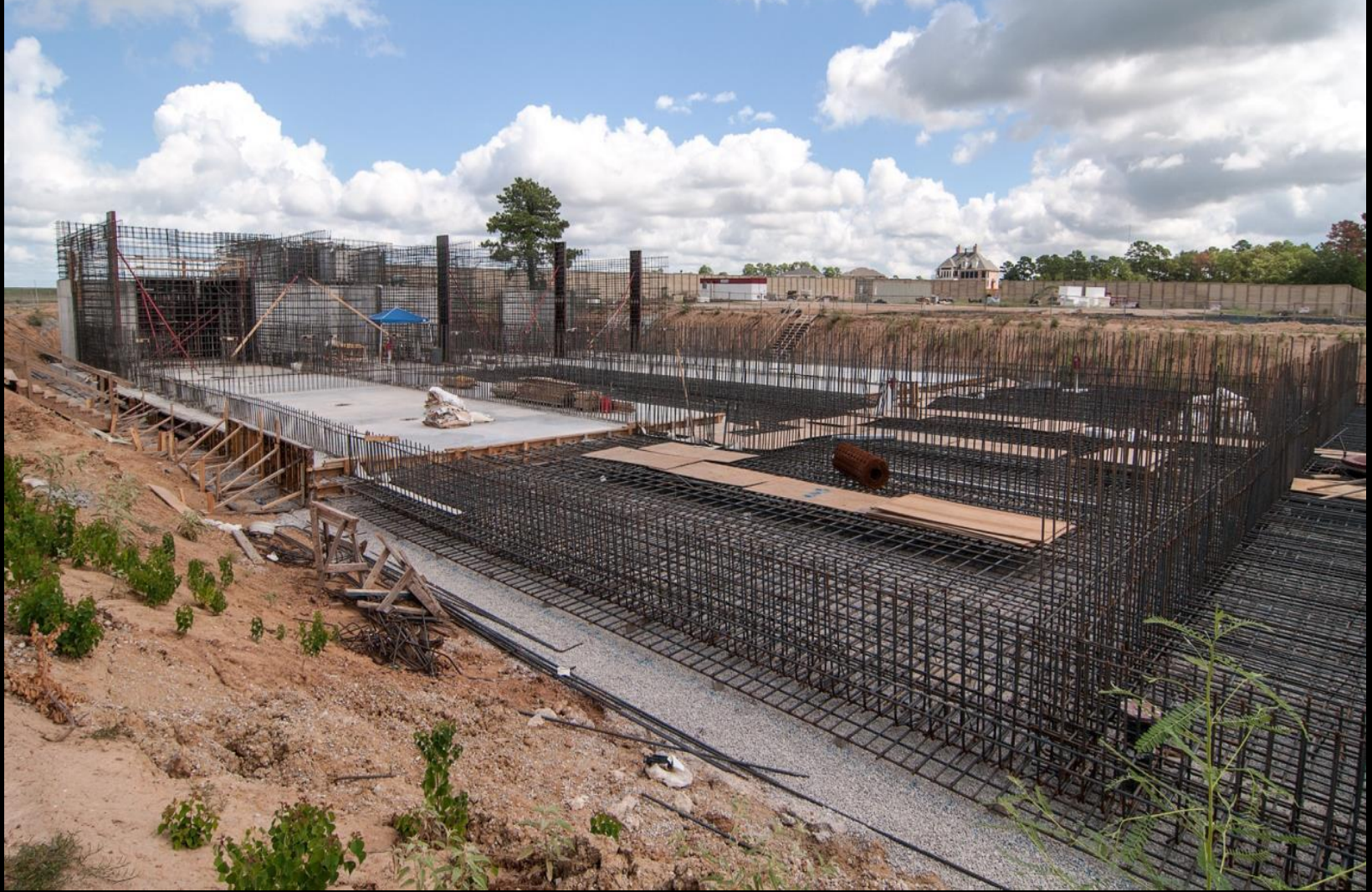
Installation of Pretreatment foundation rebar complete
