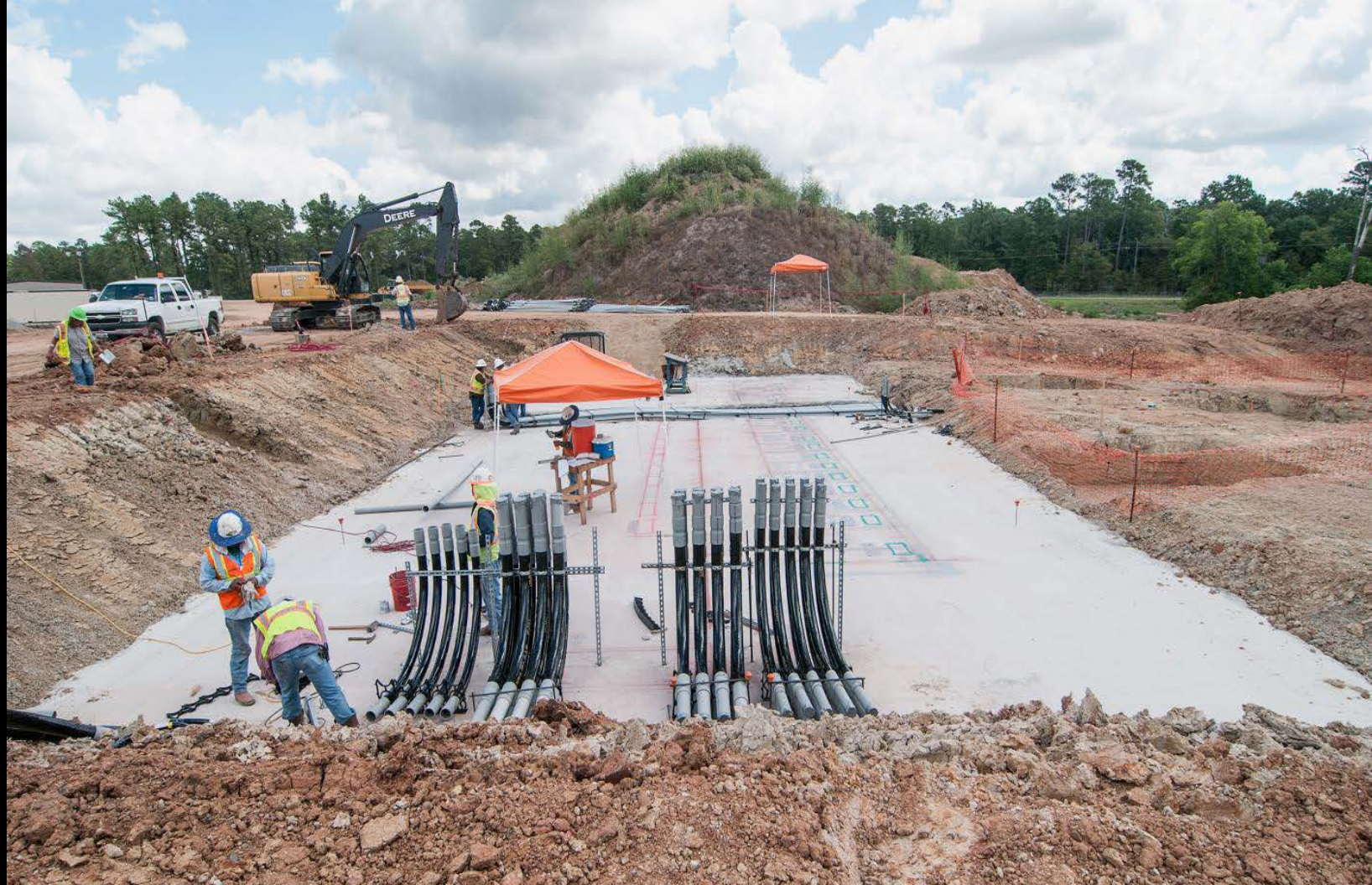
Seal slab complete at Electrical Building and early stages of electrical rough-in
