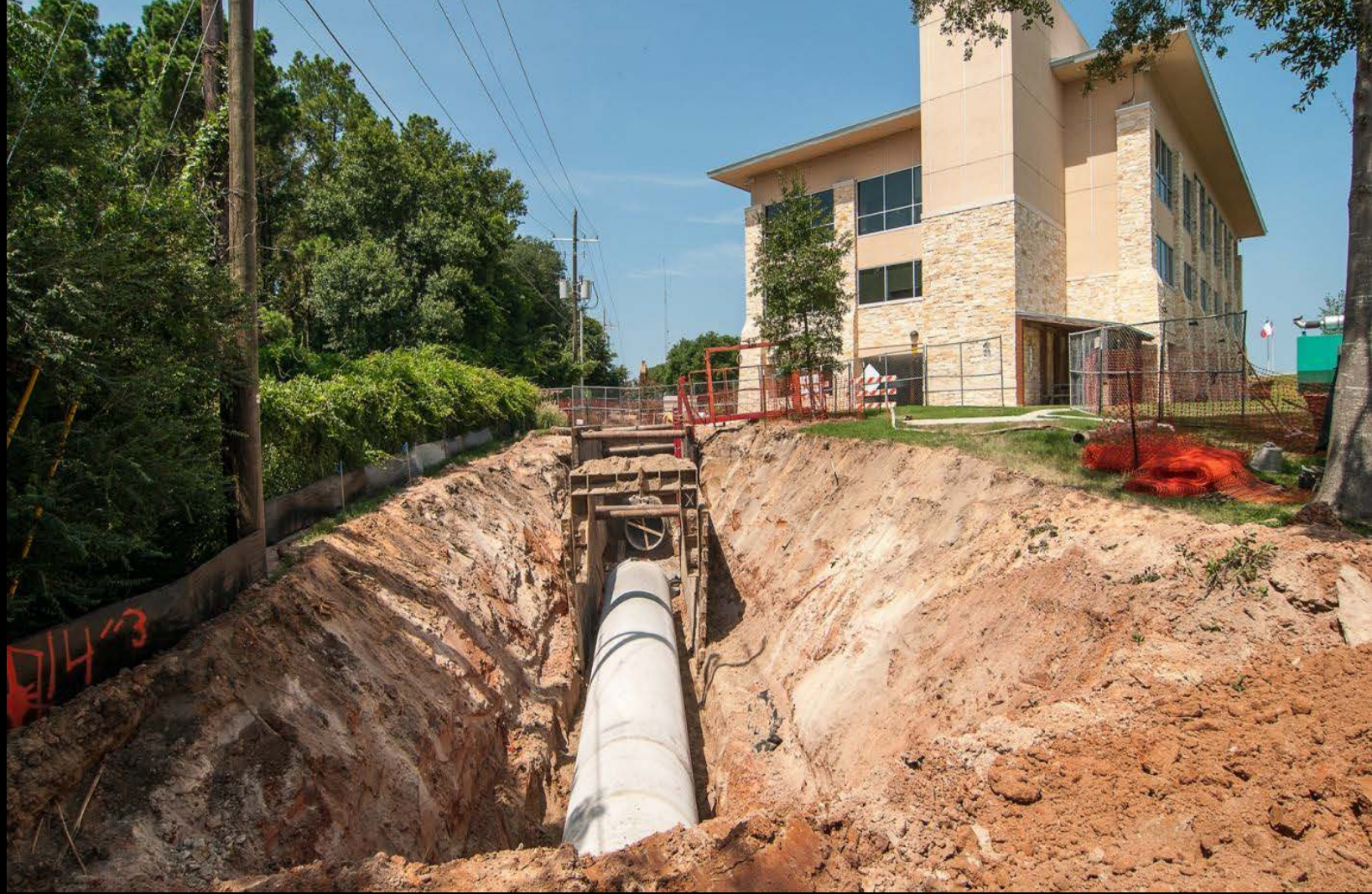
Open cut installation of 60 inch line adjacent to G&A Building
