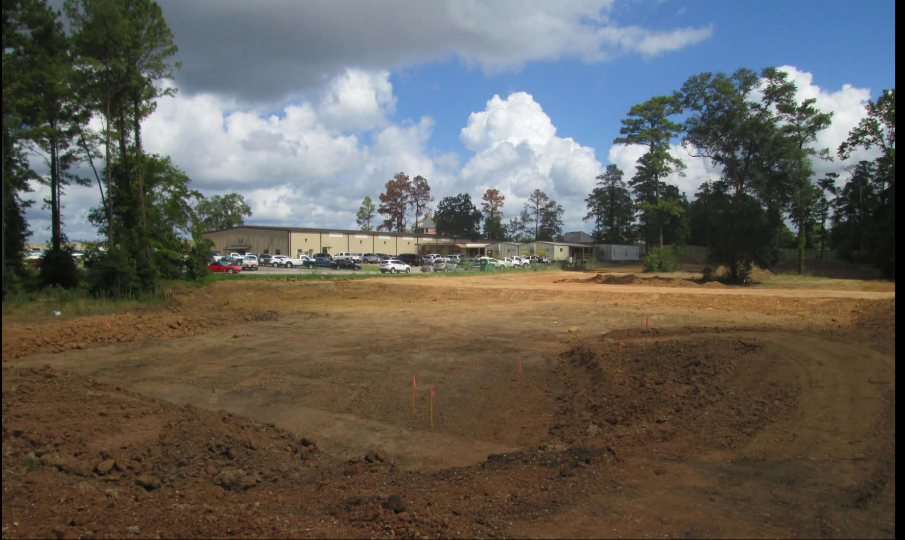
Subgrade preparations at Operations Building
